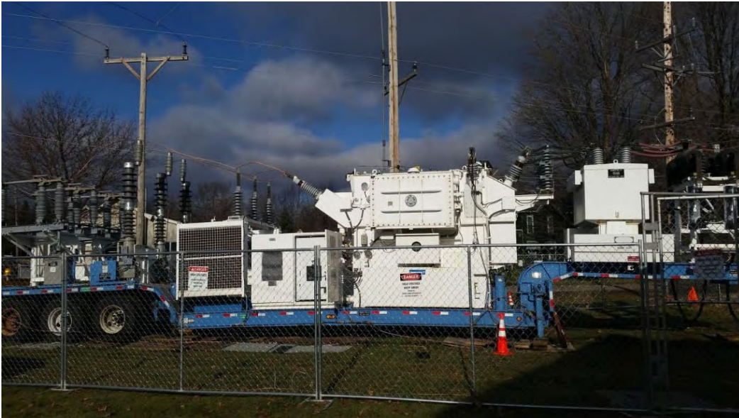
FIGURE 91 MOBILE SUBSTATION
