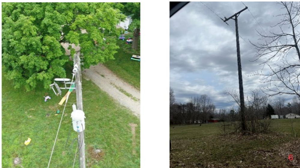
IMAGERY FROM DRONE INSPECTION COMPARED TO VISUAL GROUND INSPECTION
