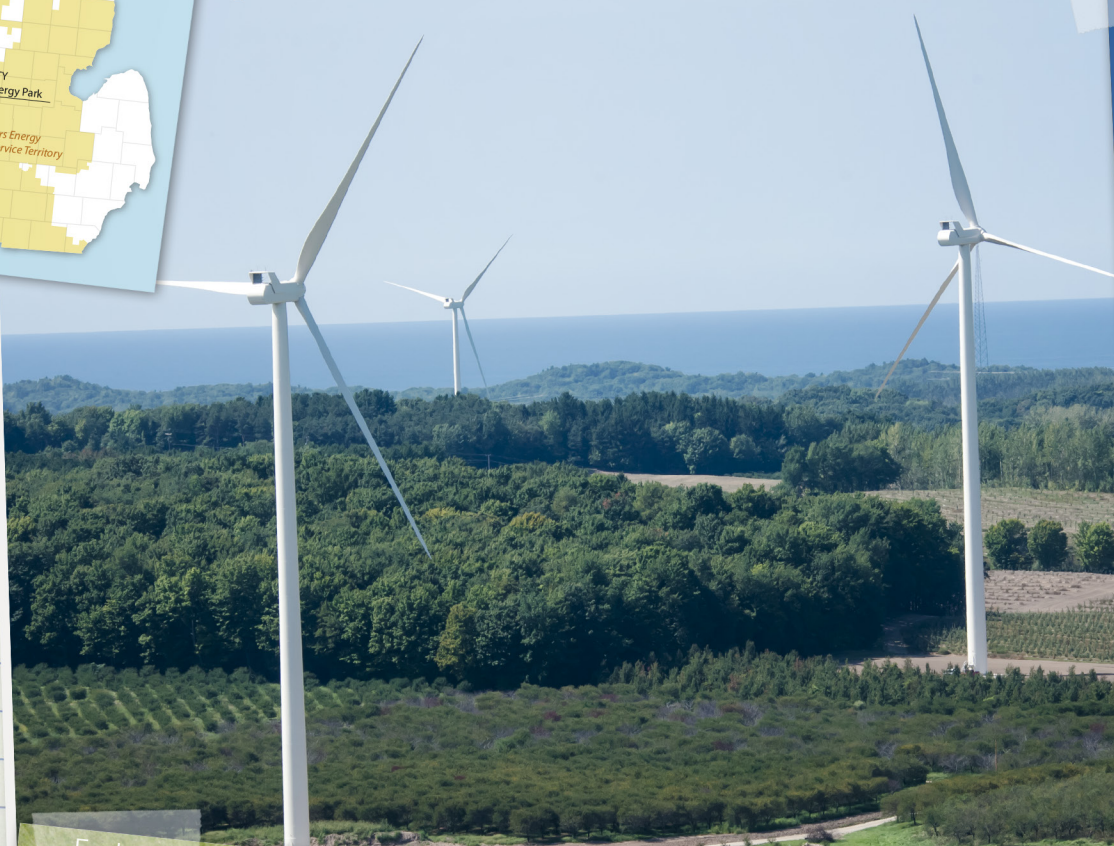
Each wind turbine blade is 150 feet long.
