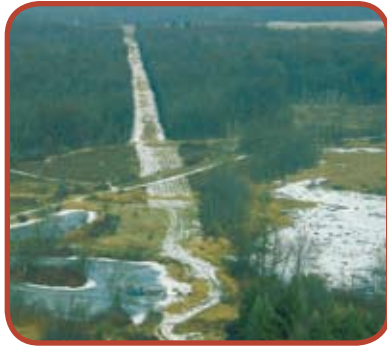
Obstruction-free corridors help us to safely deliver natural gas to our customers.
