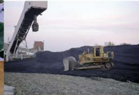
Below: About 1.4 million tons of coal a year helps Whiting produce the electricity you depend on. Bottom: The plant generates power throughout the days, nights, weekends and holidays.
