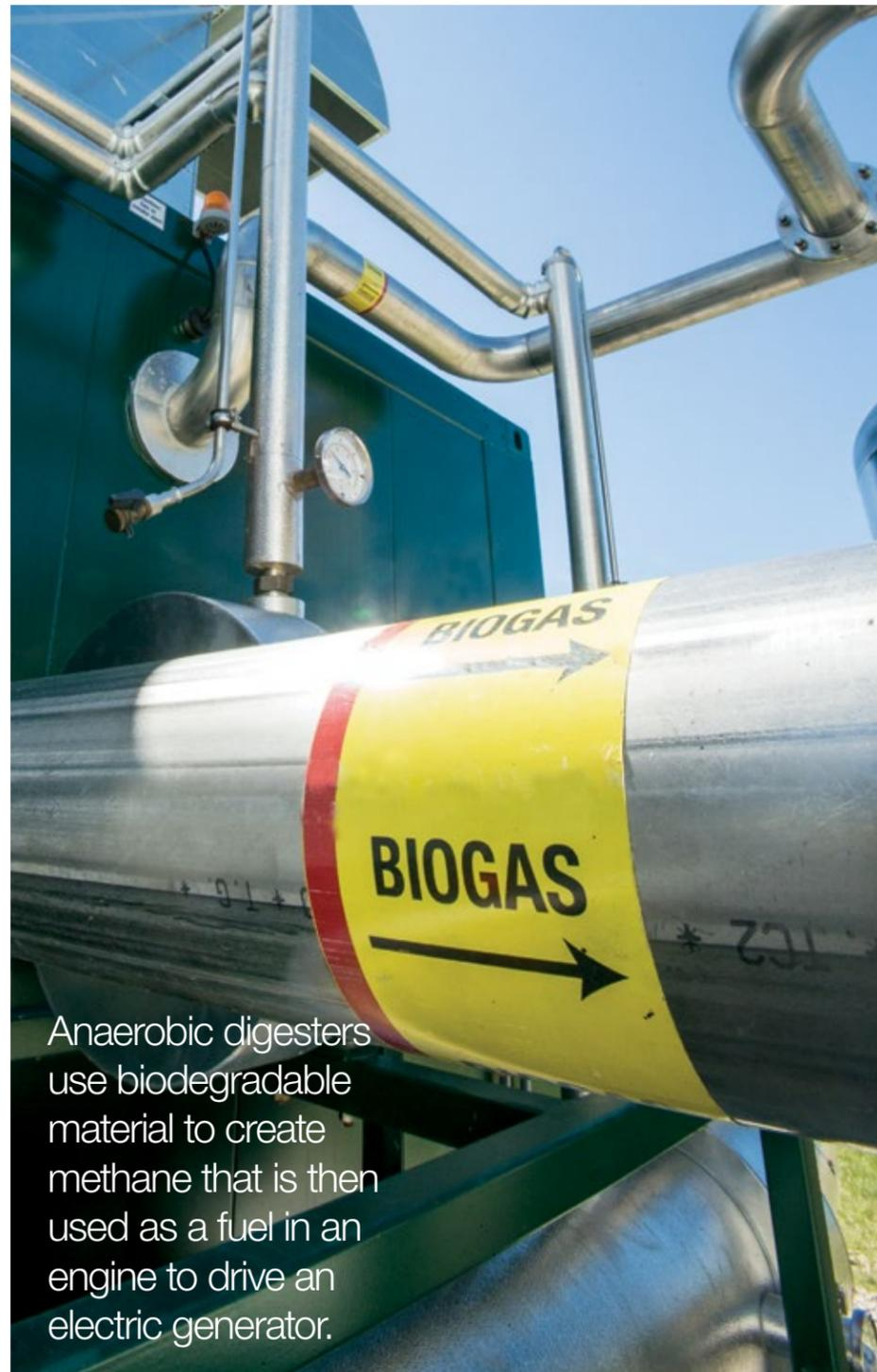
Anaerobic digesters use biodegradable material to create methane that is then used as a fuel in an engine to drive an electric generator.
