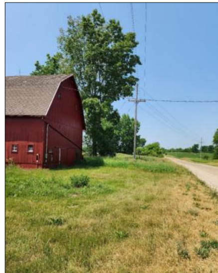
Approved overhead permanent service and clear path.
