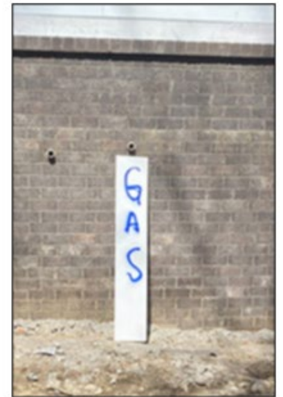
Meter location marked with plywood marked Gas.
