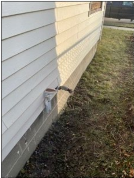
New meter location visible with stubbed out fuel line.
