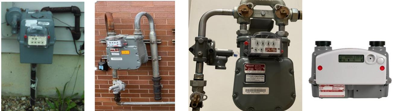
Regulated Meter (RM)    Top Connect (TC) Meter    Top Connect (TC) Meter w/Bypass    Itron Intellis USM
