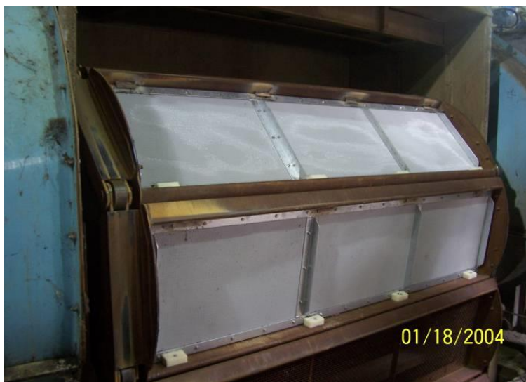
Figure 4-7 Traveling Water Screen with Fine-mesh Overlays (Courtesy of Alden)
