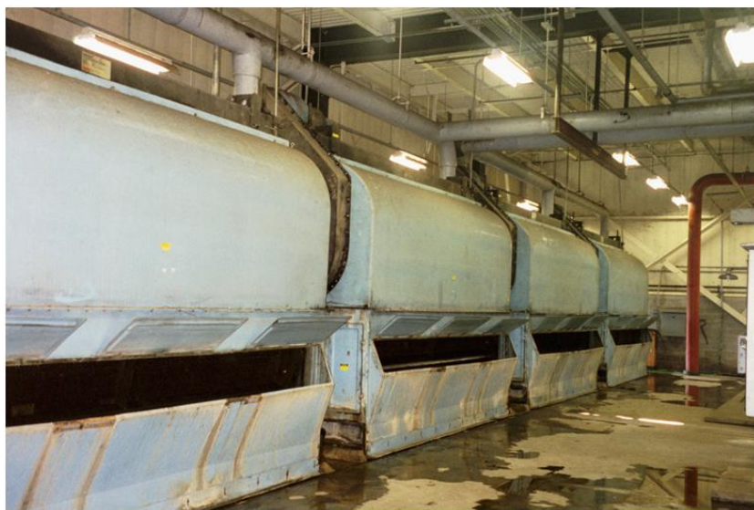
Figure 4-15 Typical Through-flow Traveling Water Screen Arrangement
