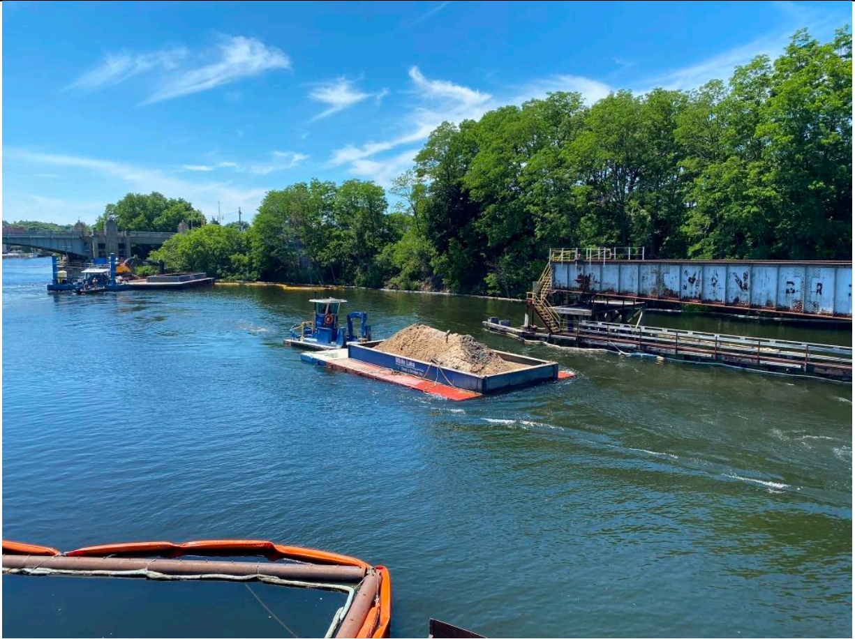
Photo No. 3: Transporting dredged sediment for dewatering (photo taken facing northwest)
