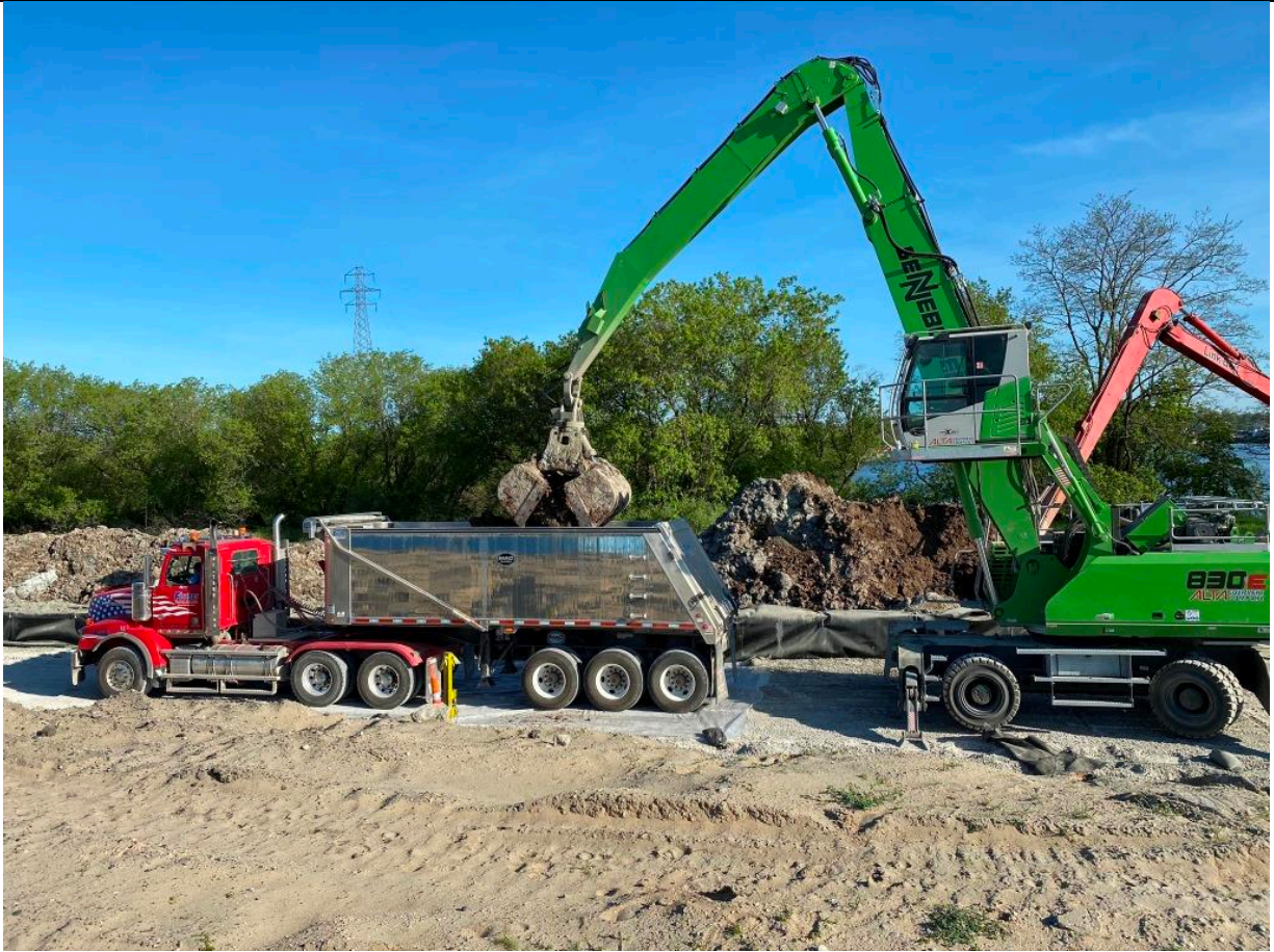
Photo No. 3: Loading dewatered sediment for transportation and disposal offsite (photo taken facing north)
