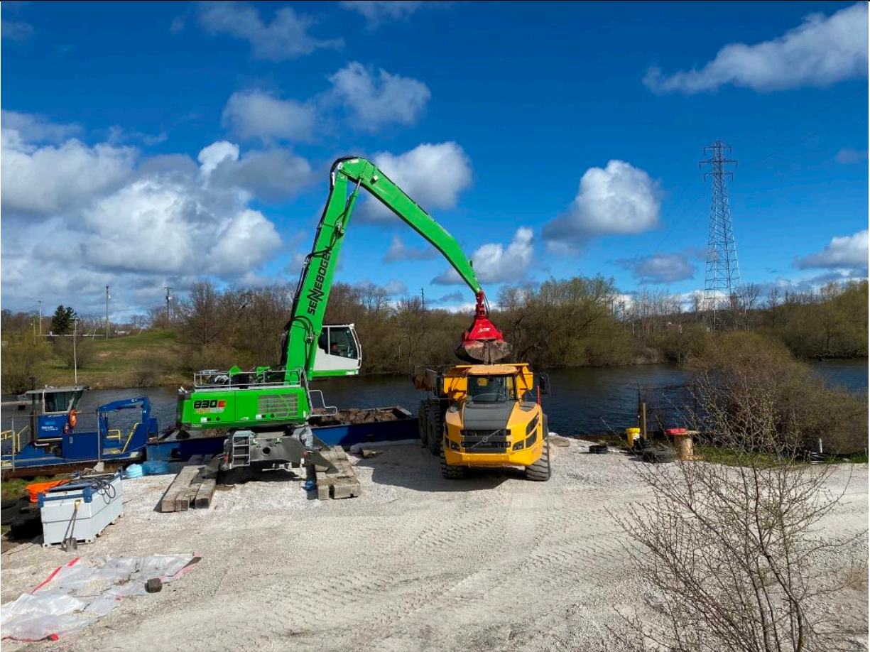
Photo No. 2: Unloading dredged sediment for transportation to the dewatering pad (photo taken facing north)
