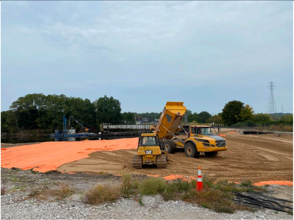
Photo No. 2: Restoration Activities – Installation of Orange Demarcation Fabric and Sand (photo taken facing northeast)
