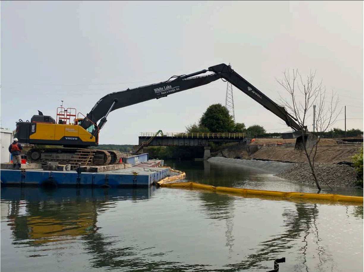
Photo No. 1: Restoration Activities – Installation of Bank Armoring Stone (photo taken facing north)
