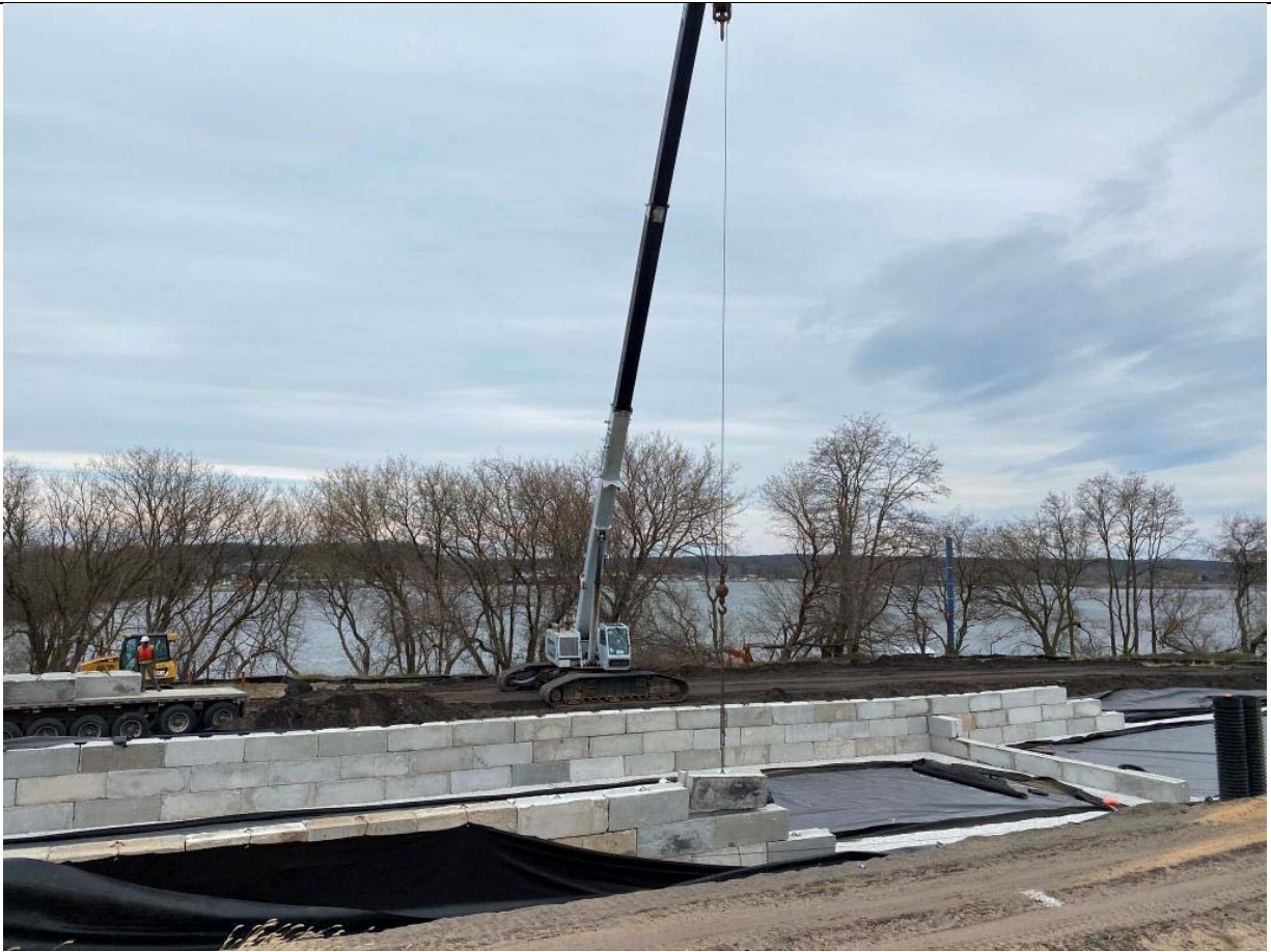
Photo No. 3: Dewatering pit construction (photo taken facing north)
