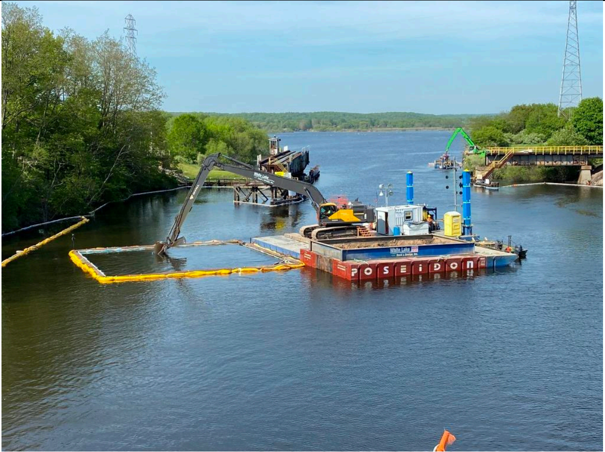
Photo No. 1: Sediment dredging (photo taken facing east)
