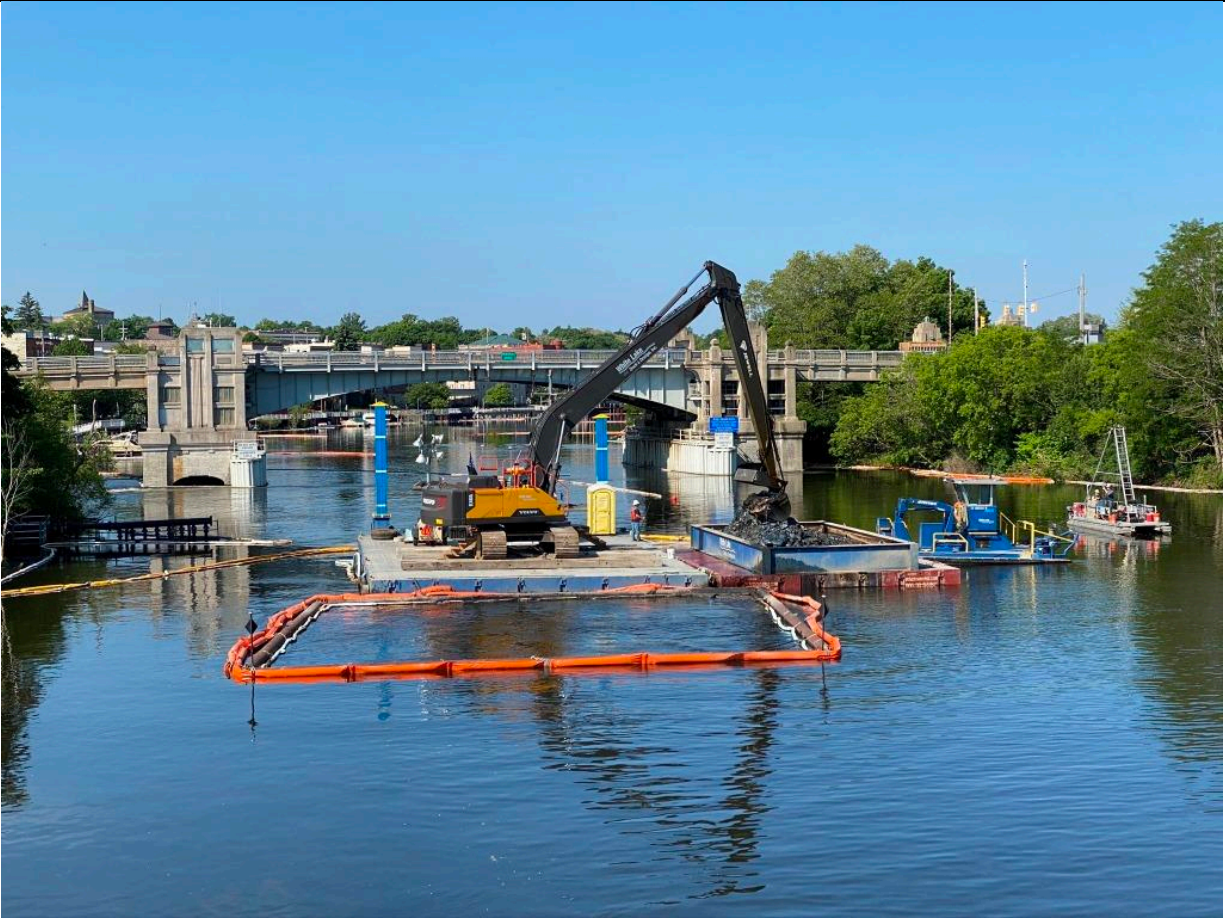
Photo No. 2: Sediment dredging (photo taken facing west)
