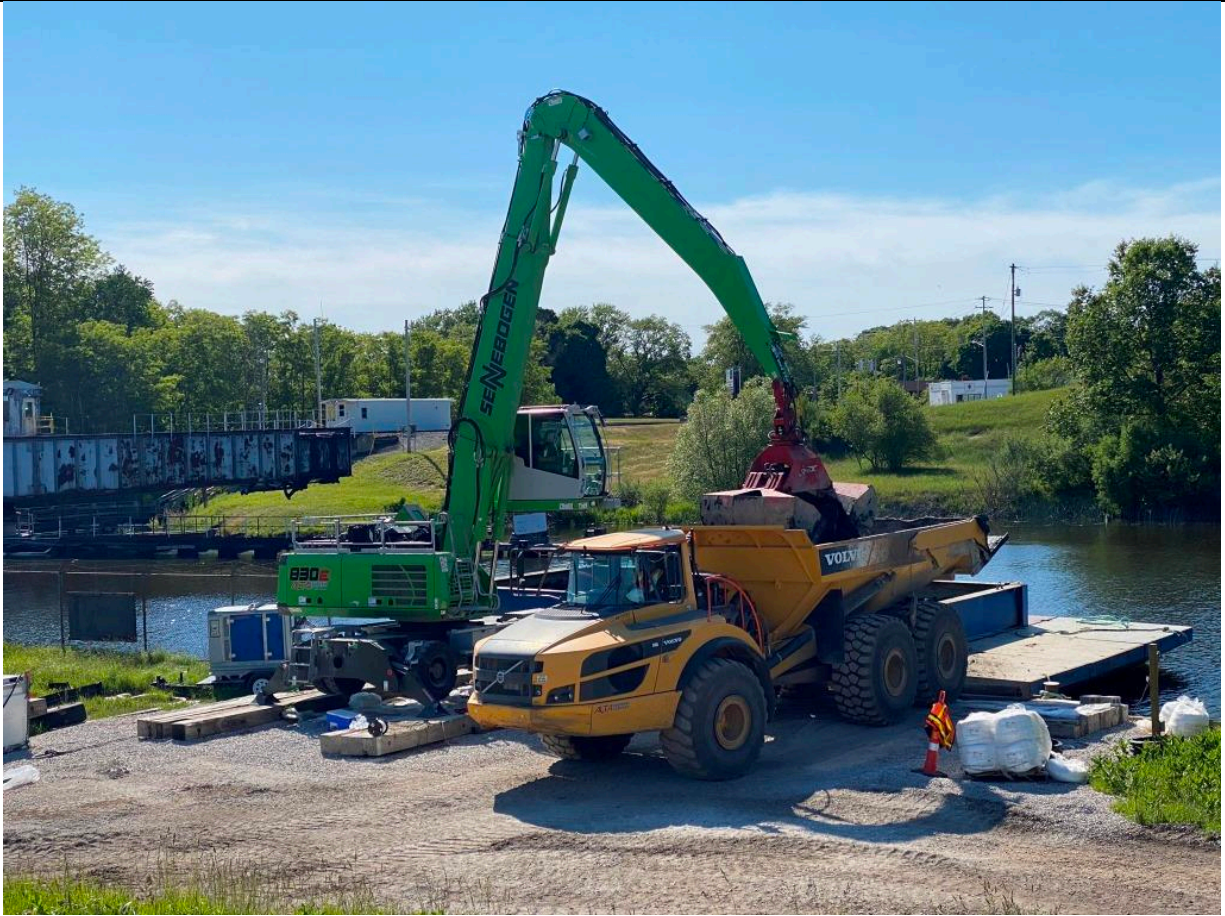
Photo No. 3: Unloading dredged sediment for transportation to the dewatering pad (photo taken facing north)
