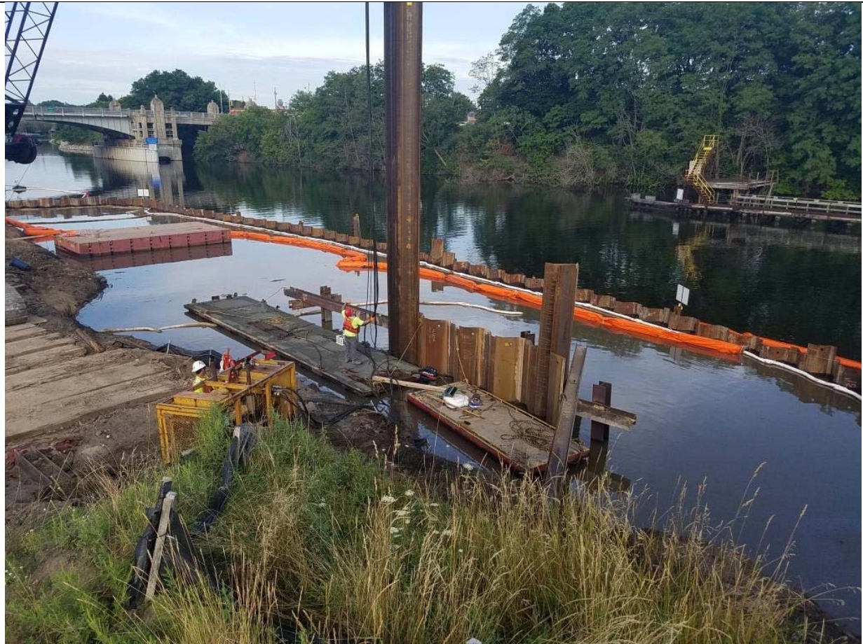
Photo No. 2: Operational Site cofferdam and support platform installation. (photo taken facing west)
