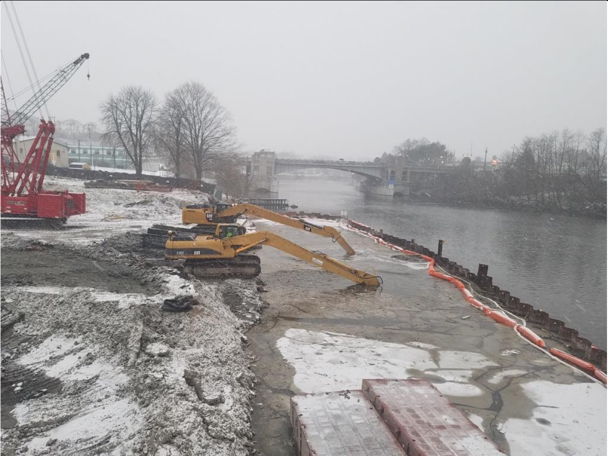
Photo No. 2: Operational Site- ISS swell removal. (photo taken facing west)
