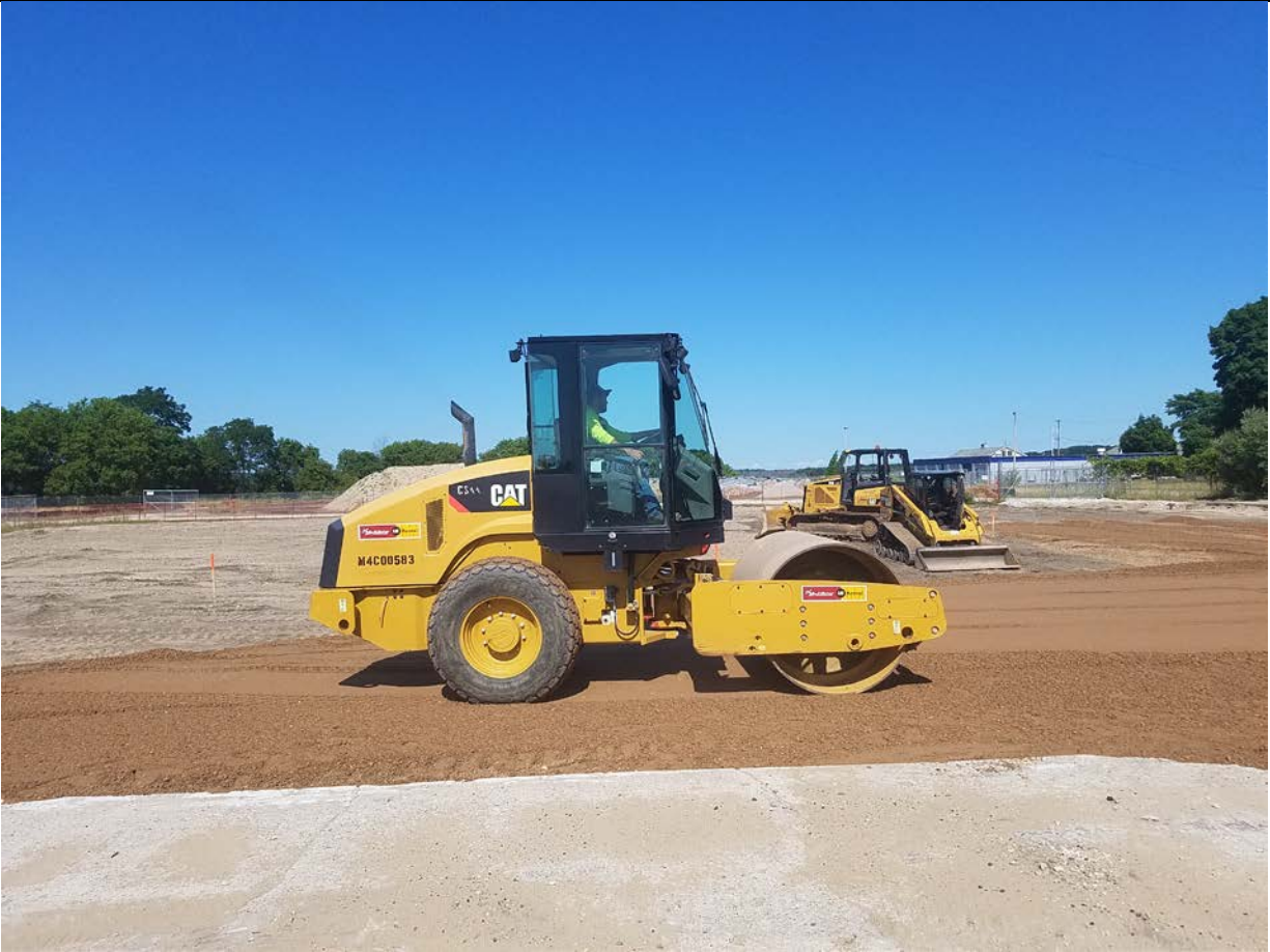
Photo No. 2: Former Relief Holder asphalt subgrade preparation. (photo taken facing east)
