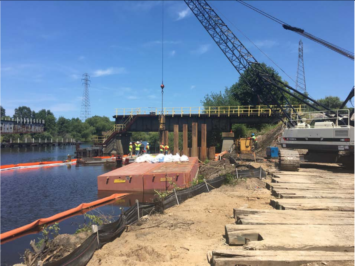
Photo No. 3: Operational Site resuspension control installation. (photo taken facing north)
