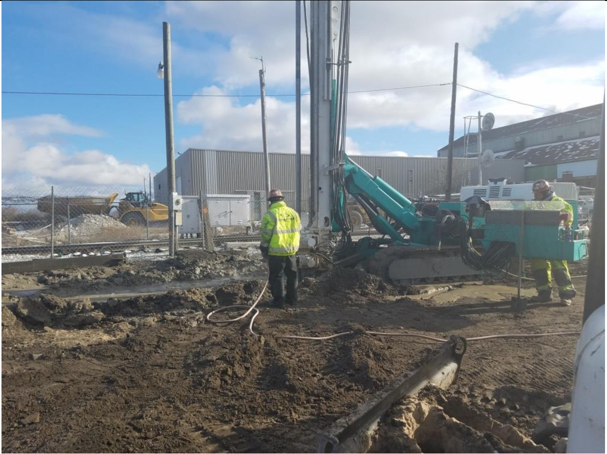
Photo No. 3: ISS via jet grouting (photo taken facing east)
