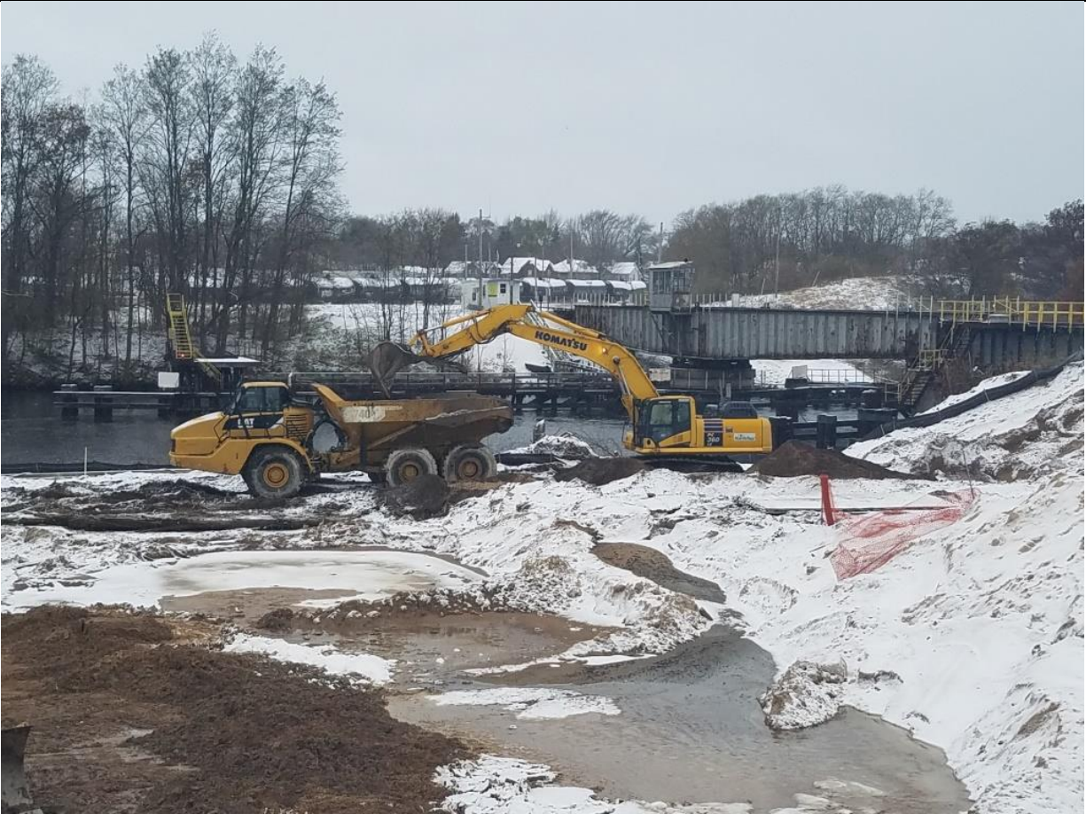
Photo No. 2: Loading overburden material for transportation and stockpiling. (photo taken facing north)
