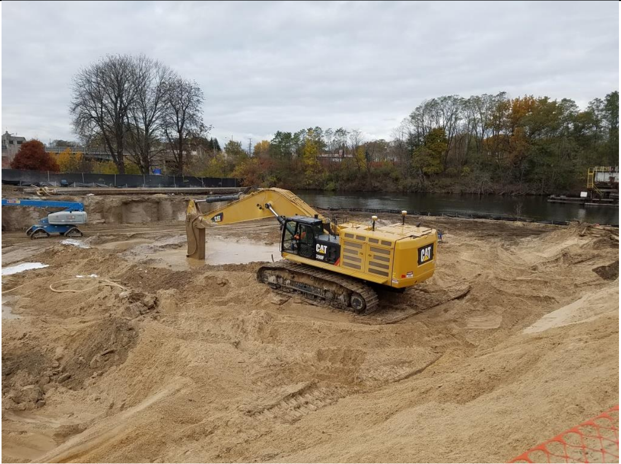
Photo No. 1: Bucket mixing ISS (photo taken facing northwest)
