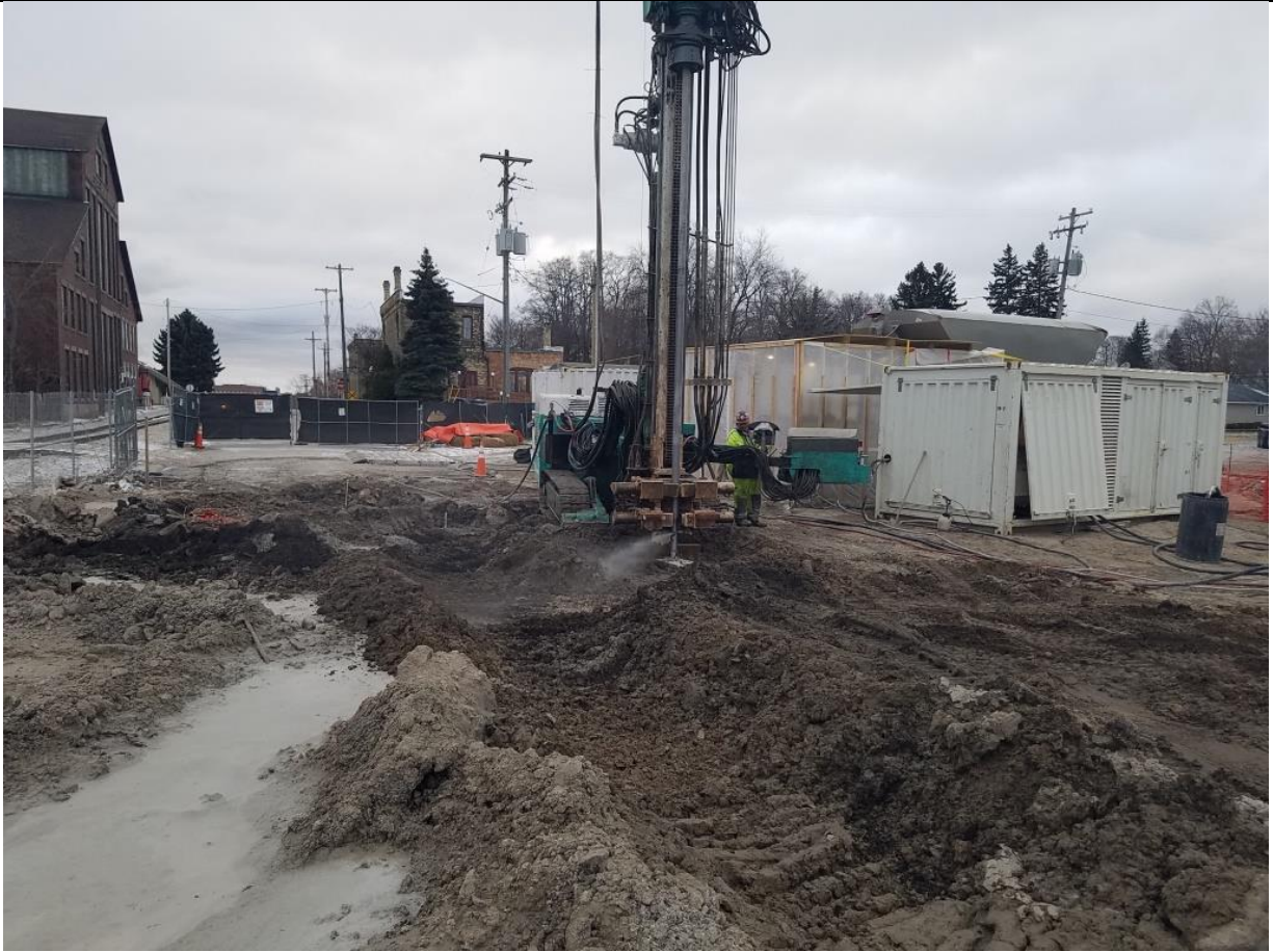
Photo No. 3: ISS via jet grouting (photo taken facing south)
