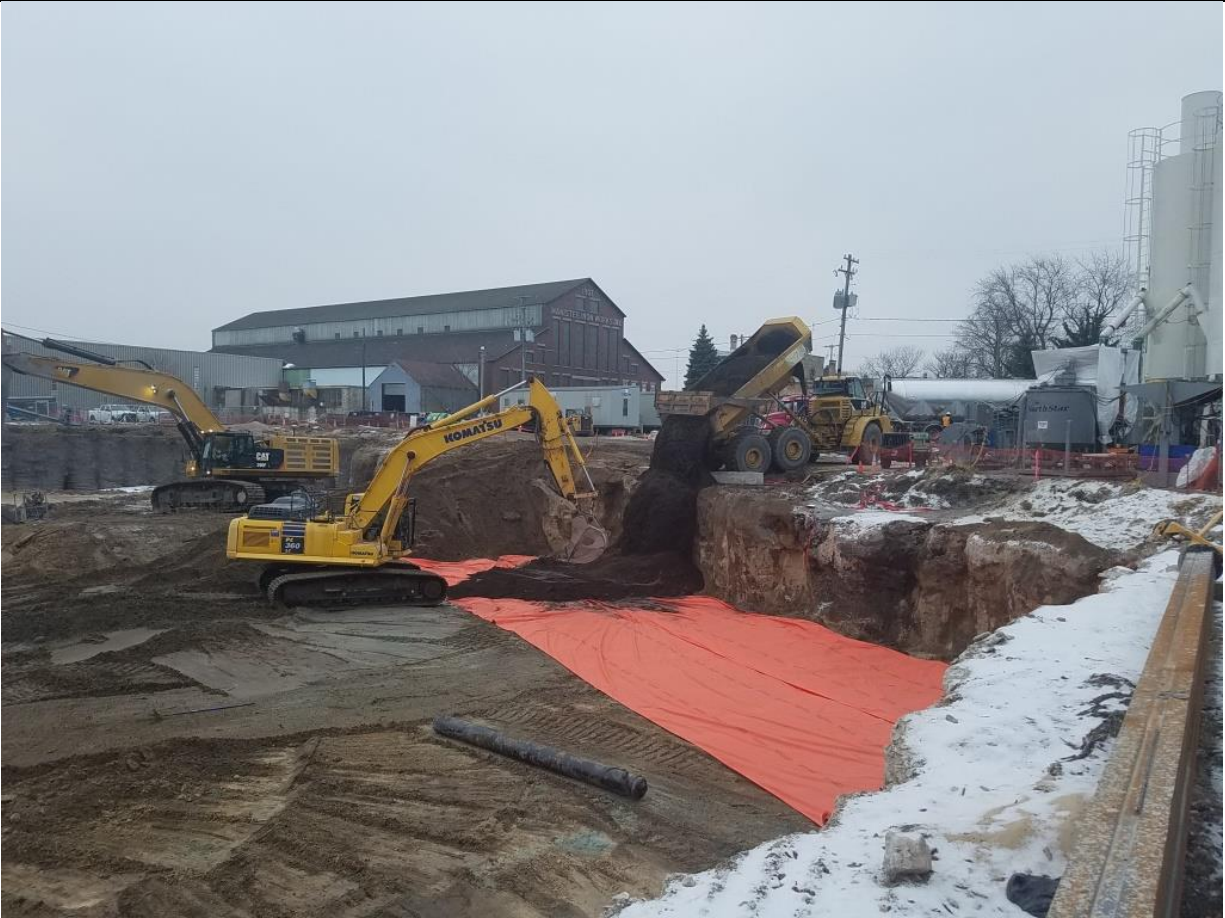
Photo No. 2: Placing backfill over demarcation fabric on the top of ISS. (photo taken facing southeast)
