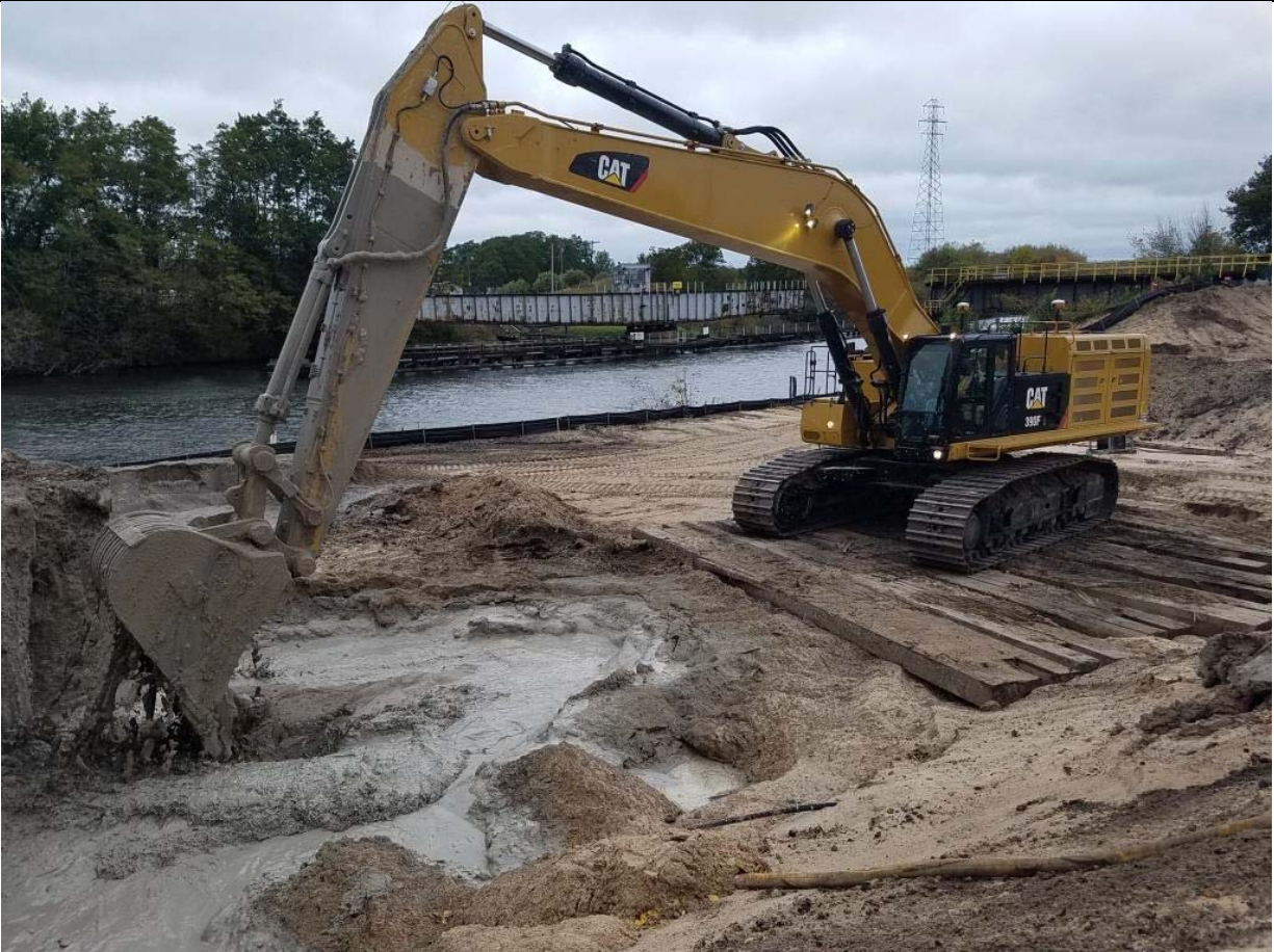
Photo No. 2: Performing bucket mixing ISS. (photo taken facing northeast)
