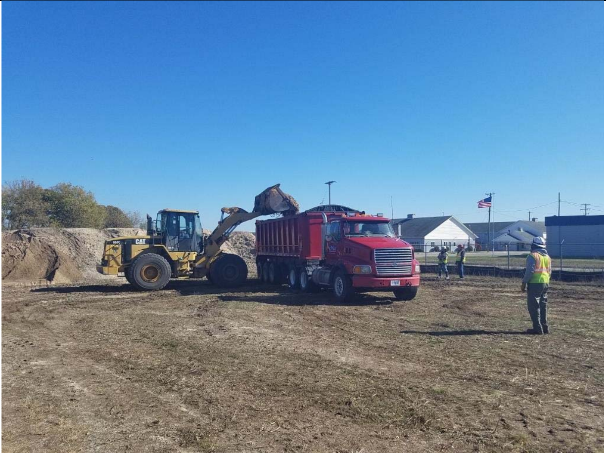
Photo No. 3: Loading soil for disposal offsite. (photo taken facing east)
