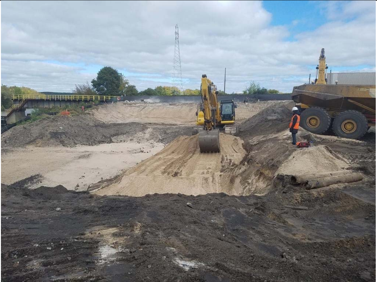
Photo No. 1: Removing overburden material. (photo taken facing east)
