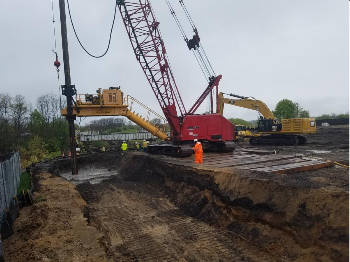
Photo No. 2: ISS column drilling (photo taken facing north)
