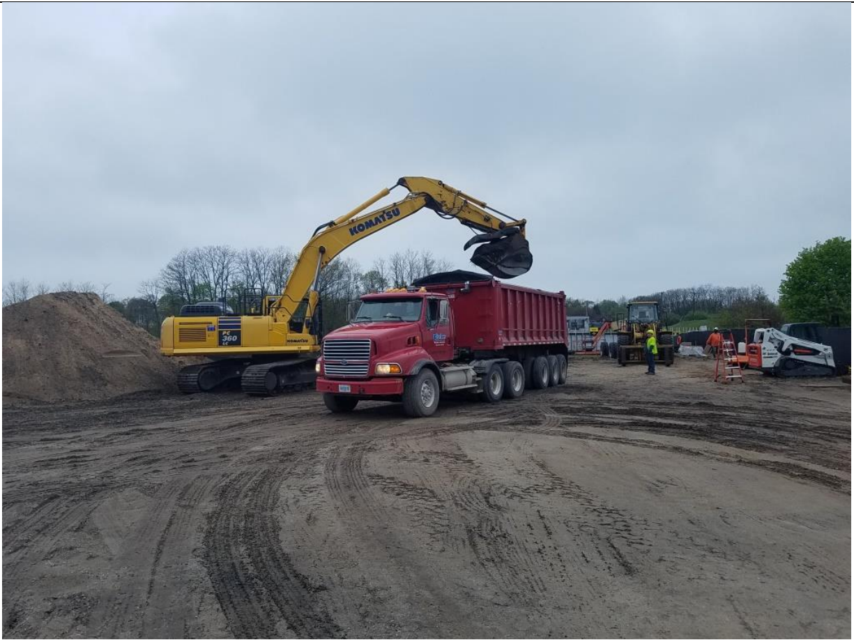
Photo No. 3: Loading unsuitable soil for transportation and disposal offsite (photo taken facing north)
