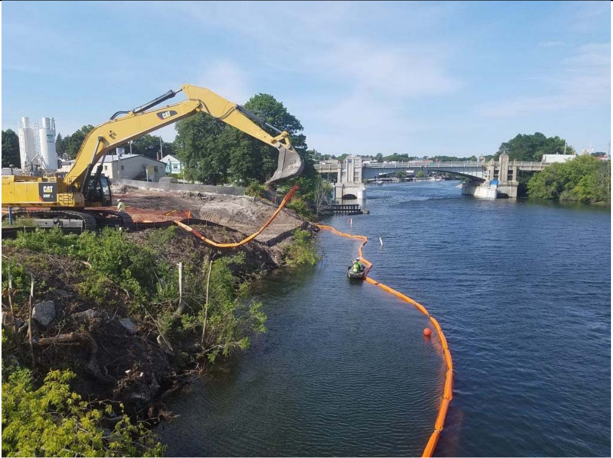
Photo No. 3: Turbidity curtain installation (photo taken facing west)
