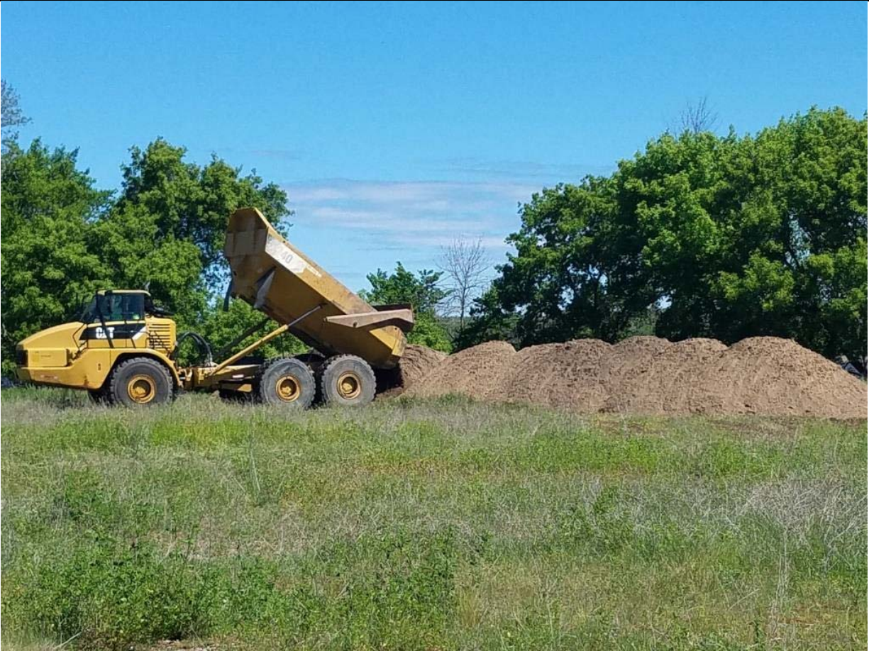
Photo No. 2: Overburden soil stockpiling (photo taken facing north)
