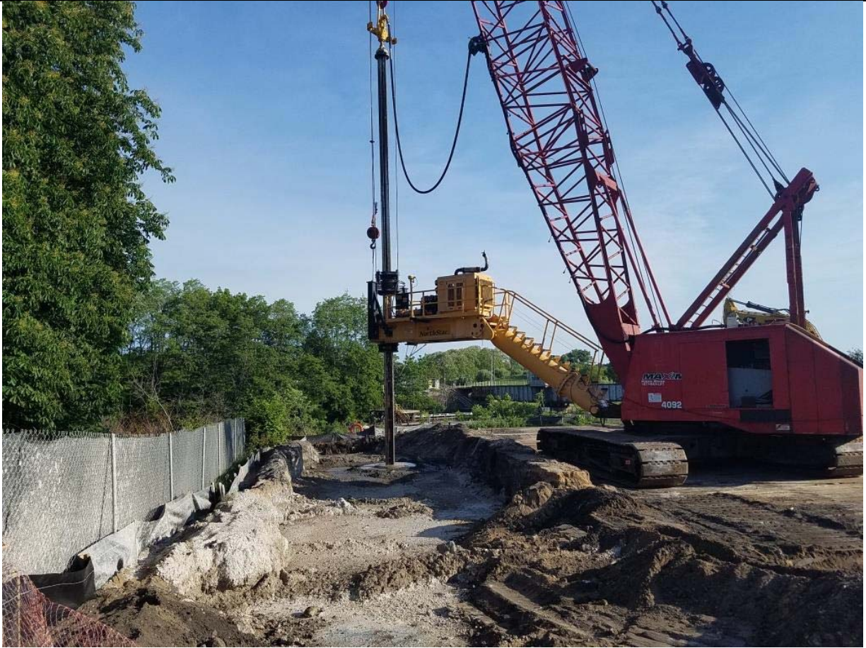
Photo No. 1: Performing perimeter ISS column installation along west side of the site (photo taken facing north)
