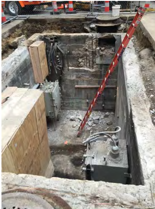
FIGURE 69 – VAULT OR MANHOLE ROOF REPLACEMENT
