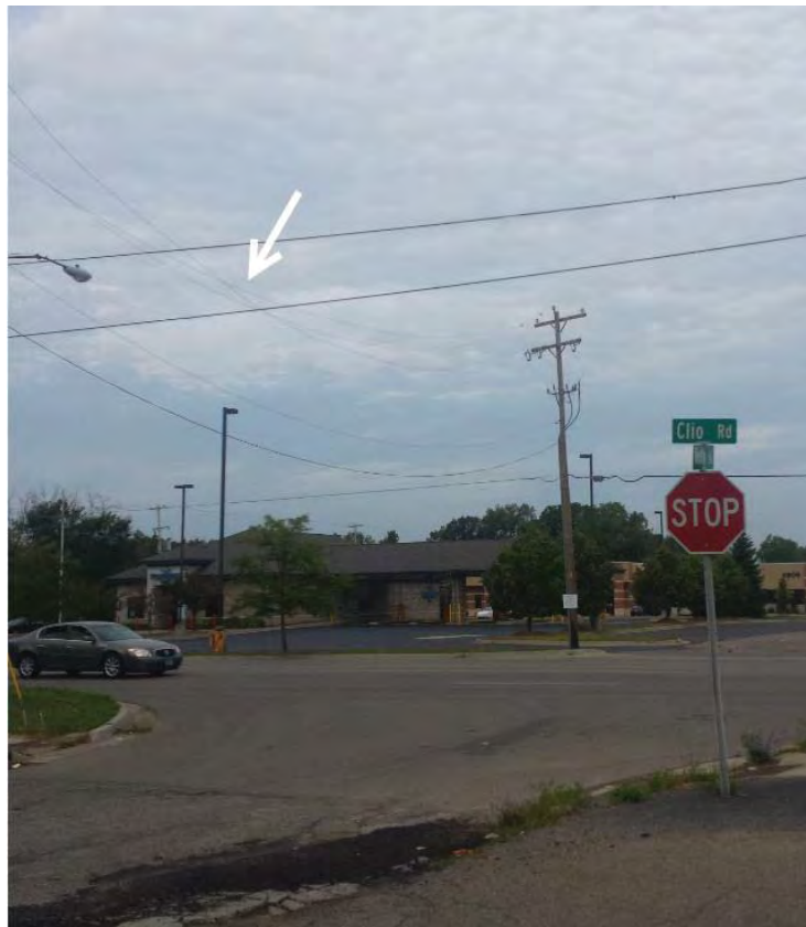
FIGURE 98 – SAGGED WIRES ON PIERSON FEEDER
