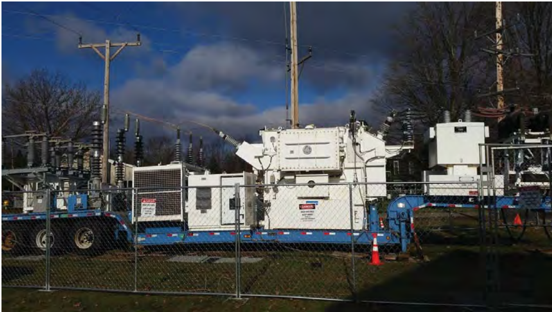
FIGURE 86 – MOBILE SUBSTATION
