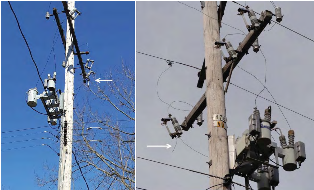
FIGURE 97 – BLOWN CAPACITOR FUSES
