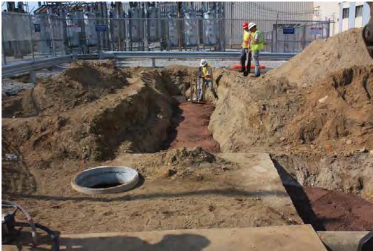
FIGURE 78 – INSTALLATION OF NEW DUCT BANK AND MANHOLE
