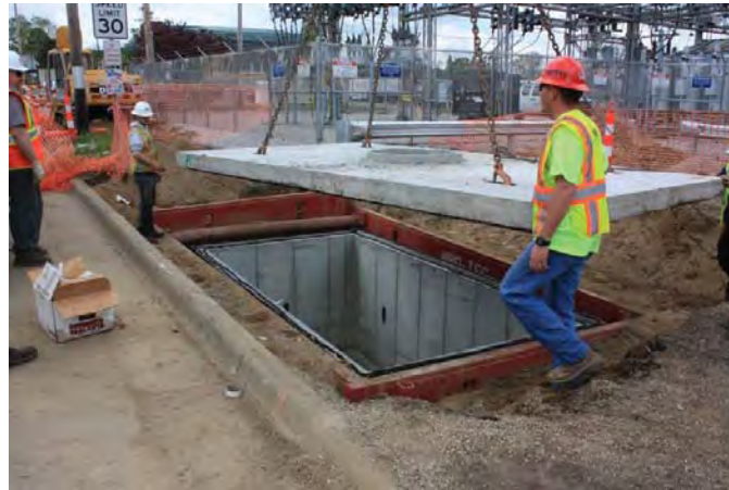
FIGURE 79 – INSTALLATION OF MANHOLE ROOF
