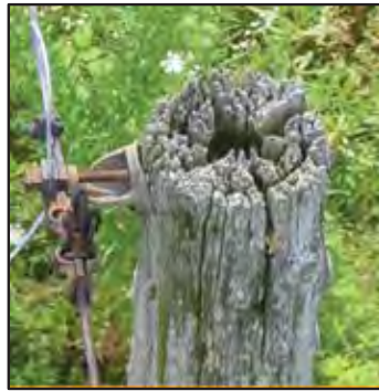
FIGURE 84 – DETERIORATION OF HVD POLE TOP FROM HELICOPTER INSPECTION
