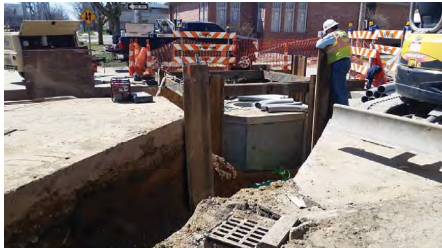
FIGURE 70 – INSTALLATION OF NEW MANHOLES OR VAULTS
