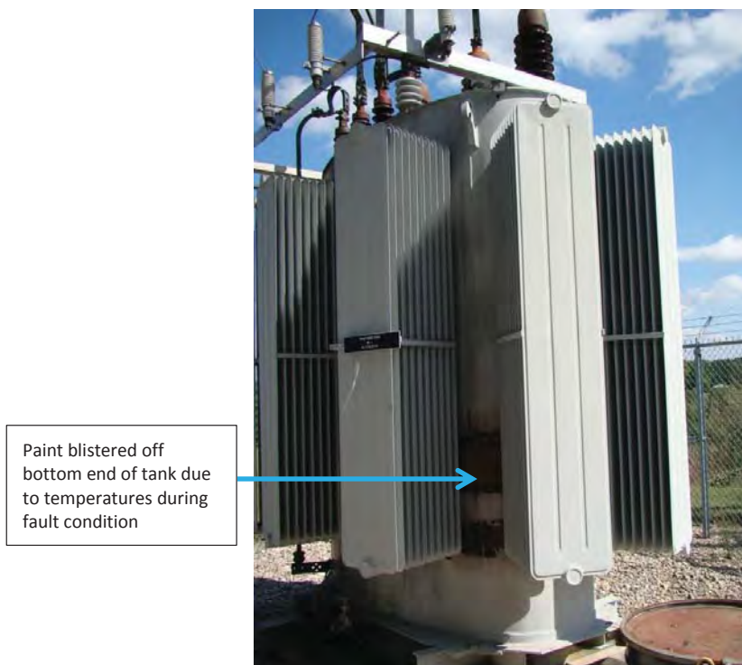
FIGURE 61 – FAILED TRANSFORMER AT SHANTY CREEK SUBSTATION
