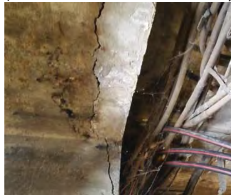
FIGURE 66 – DETERIORATED MANHOLE/VULT ROOFS
