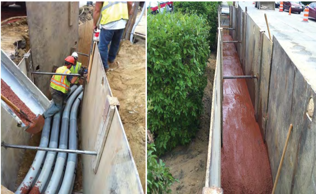
FIGURE 71 – INSTALLING NEW CONCRETE ENCASED DUCT BANK
