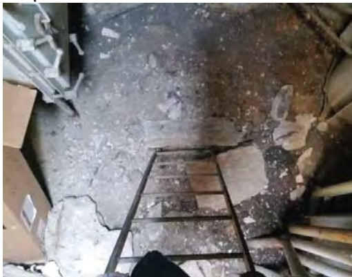
FIGURE 66 – DETERIORATED MANHOLE/VULT ROOFS
