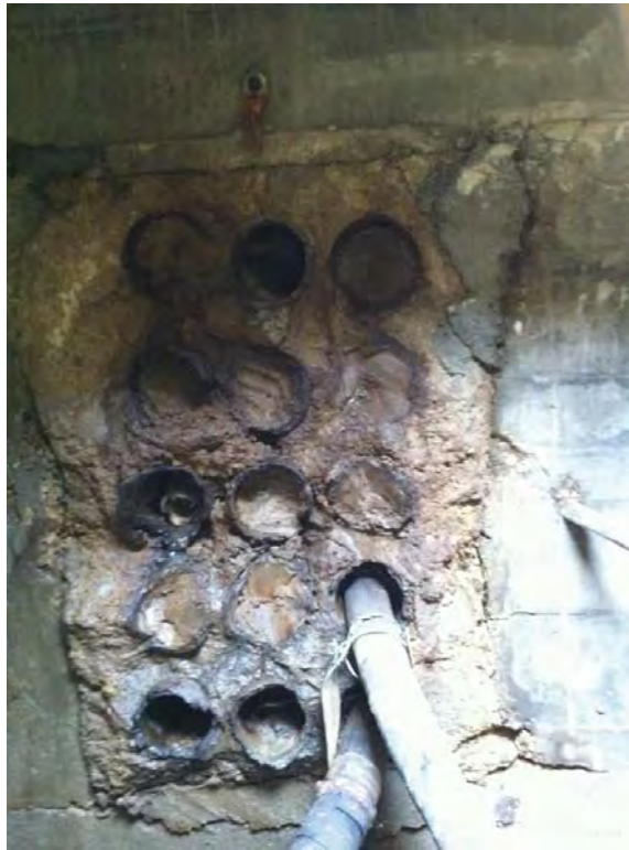
FIGURE 65 – DAMAGED / CRUSHED DUCT BANKS
