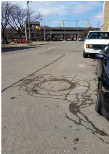
FIGURE 67 – SUNKEN/DETERIORATED MANHOLE ACCESS
