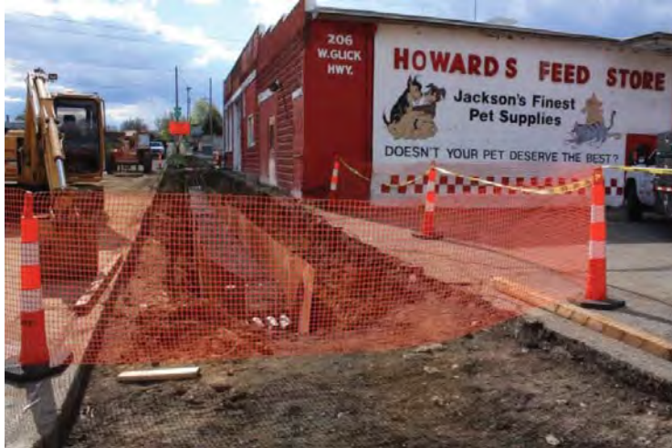
FIGURE 77 – NEW DUCT BANK BUILT IN SIDEWALK AREA
