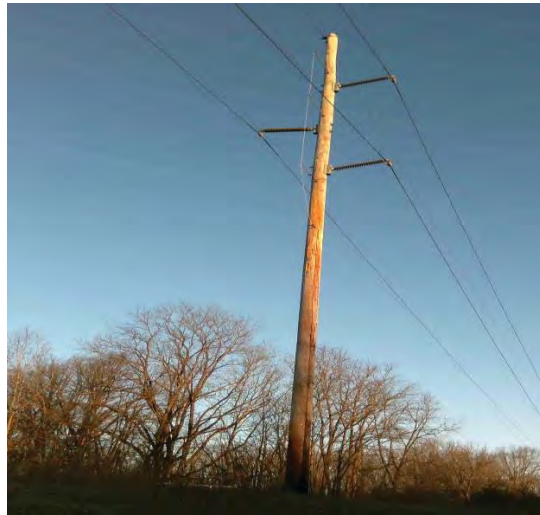
FIGURE 47 – HORIZONTAL HVD POLYMER POST DESIGN
