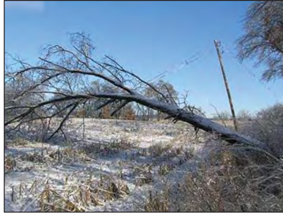
FIGURE 46 – ASC SUPPORTING A FALLEN TREE
