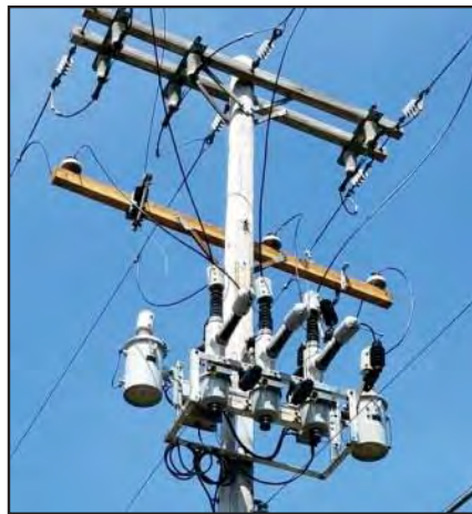
FIGURE 32 – INSTALLED AUTOMATIC TRANSFER RECLOSER
