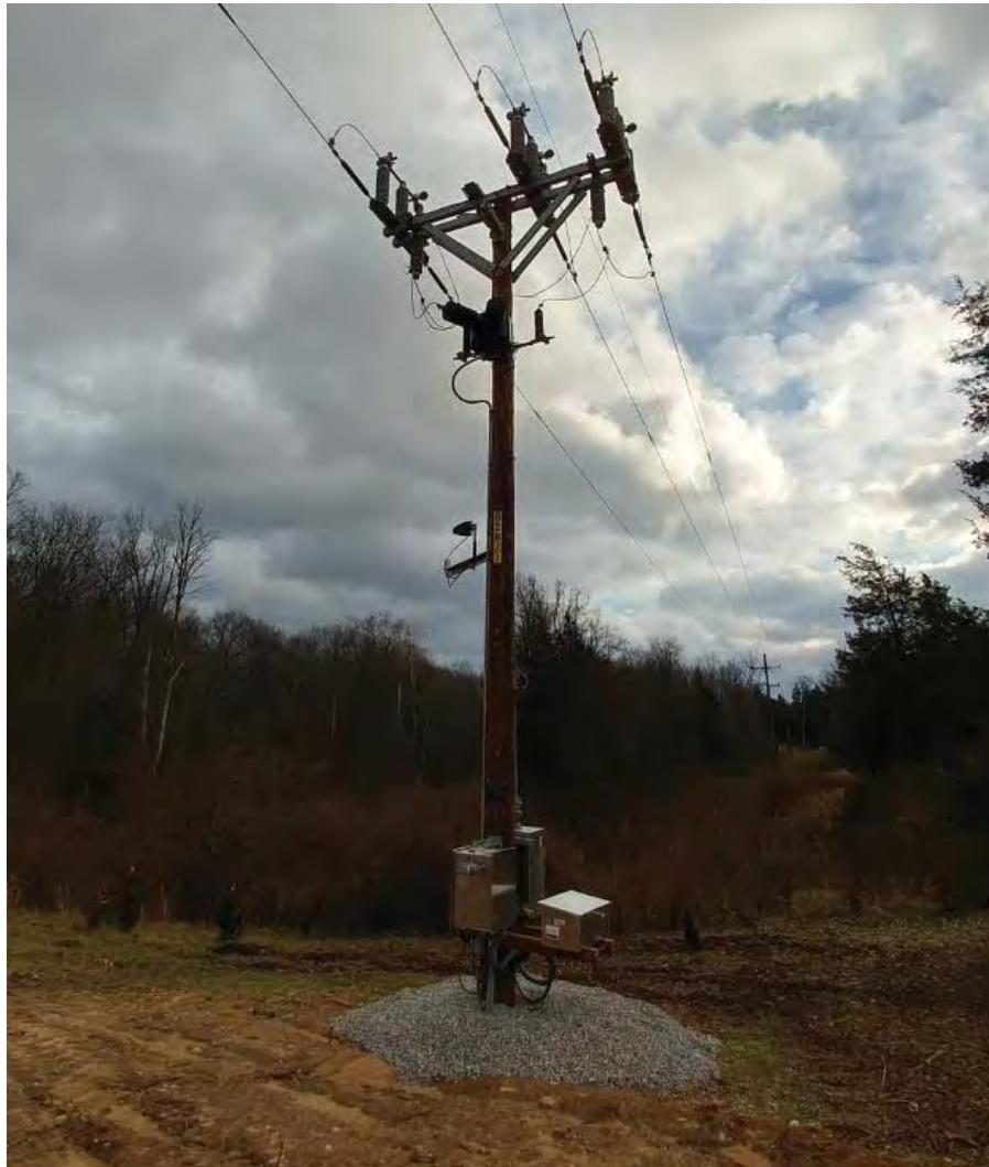
FIGURE 63 – TYPICAL 46 kV MOAB SWITCH
