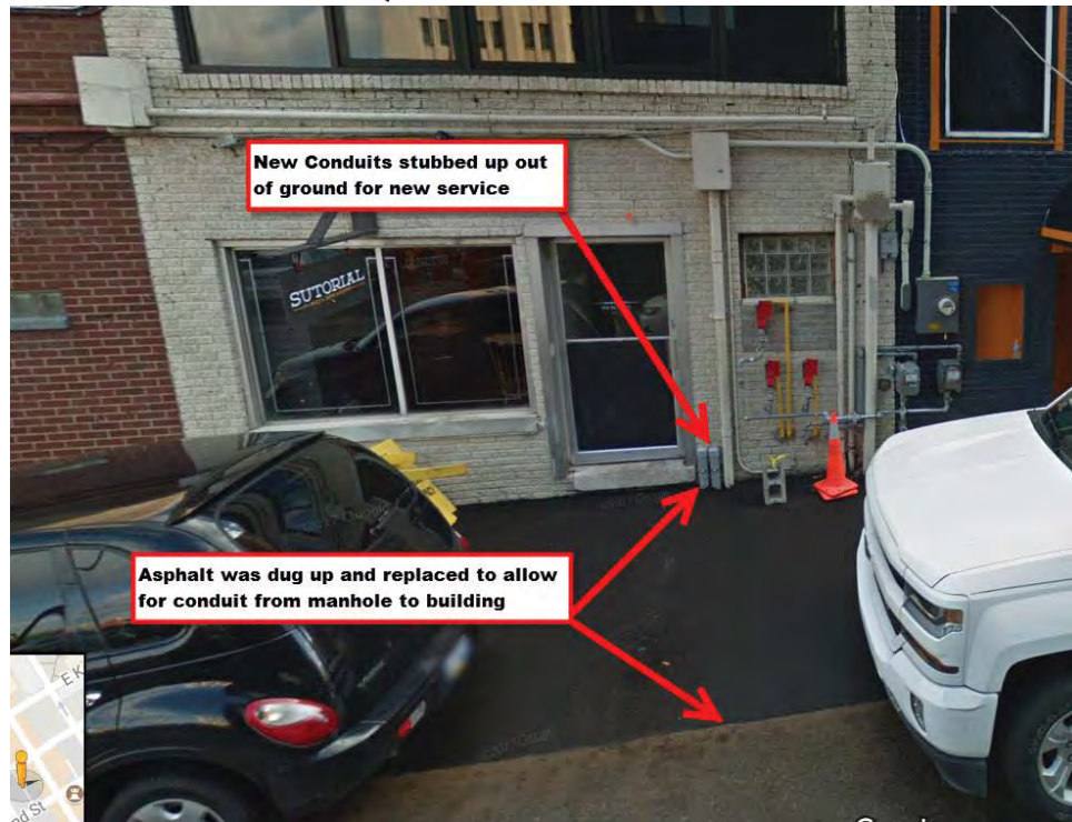
FIGURE 57 – AREA REQUIRING INSTALLATION OF NEW CONDUIT
