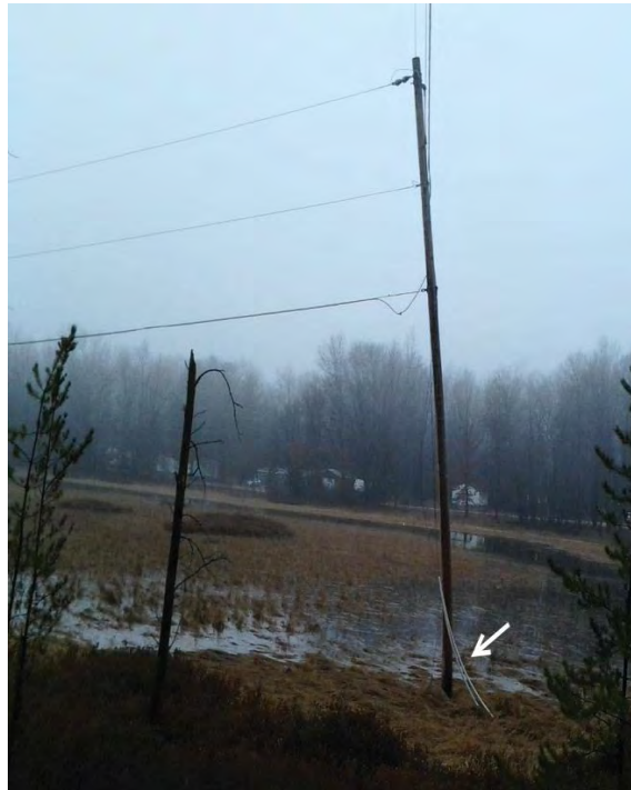
FIGURE 103 – PRIMARY POLE WITH BROKEN GUY
