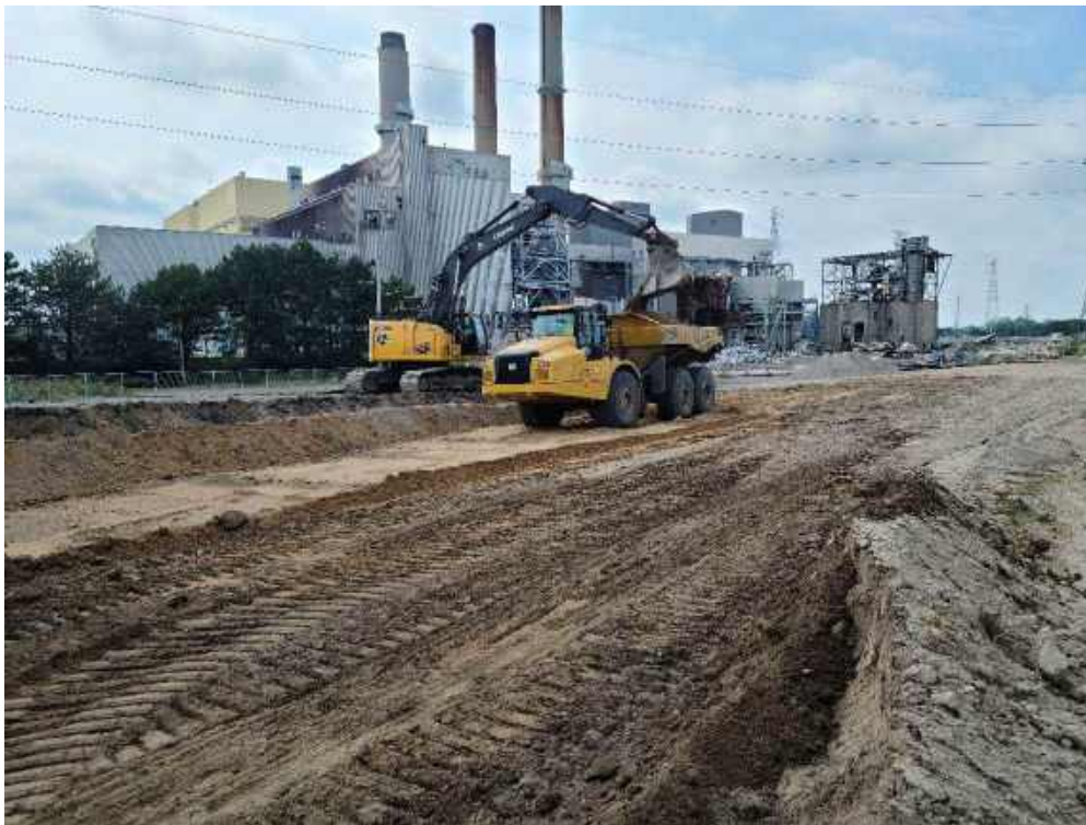
Photo 1: Fisher excavating excess berm material from the west end of the Lined Impoundment.
