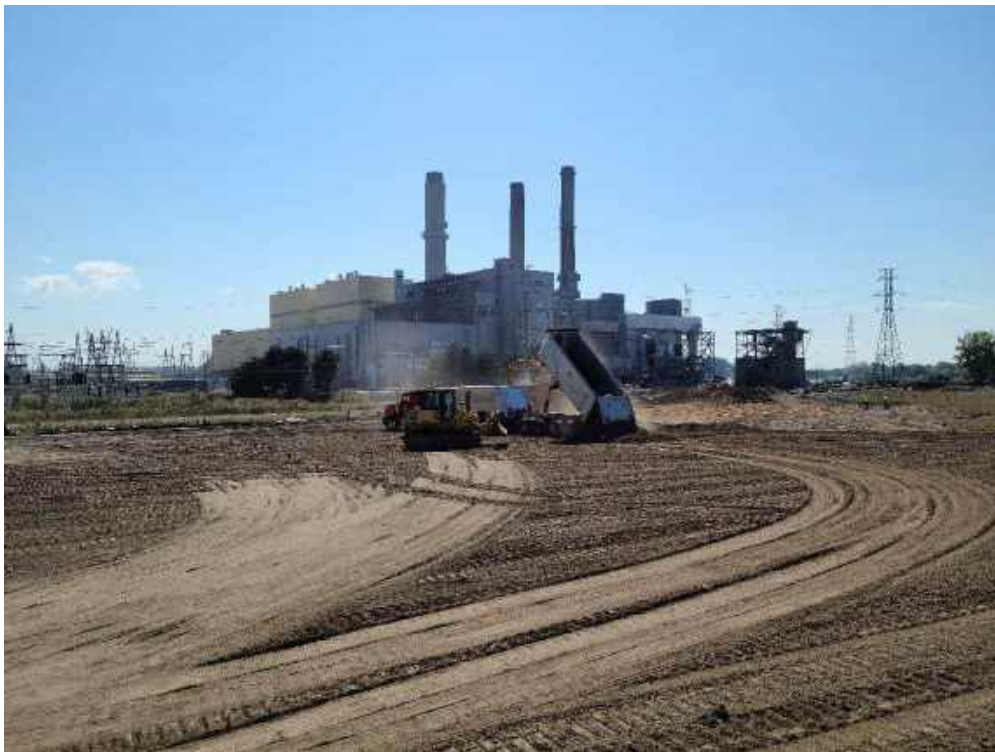
Photo 2: Fisher placing topsoil on the restoration.
