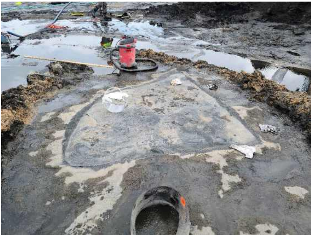
Photo 2: Fisher completes a repair to the primary geomembrane liner system in the Settling Basin.
