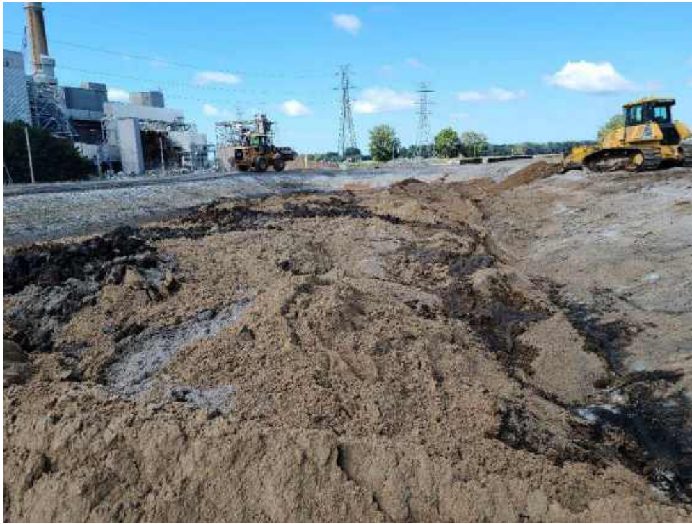
Photo 1: Fisher is mixing sand into the ash in the concrete-lined portion of the Settling Basin.
