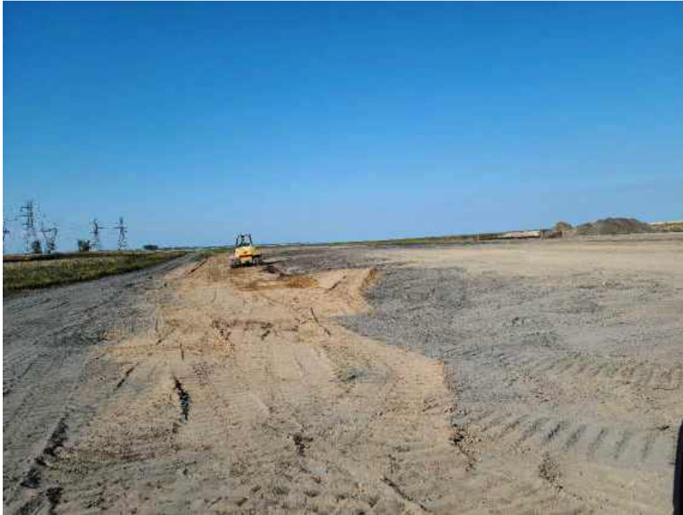
Photo 2: Fisher covering the placed ash located adjacent to the north/south road in the Weadock Landfill.
