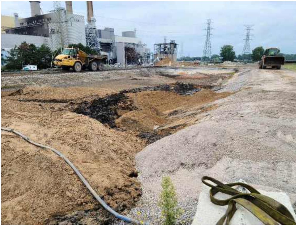
Photo 1: Fisher starts mixing sand in with the ash in the concrete-lined portion of the Settling Basin.
