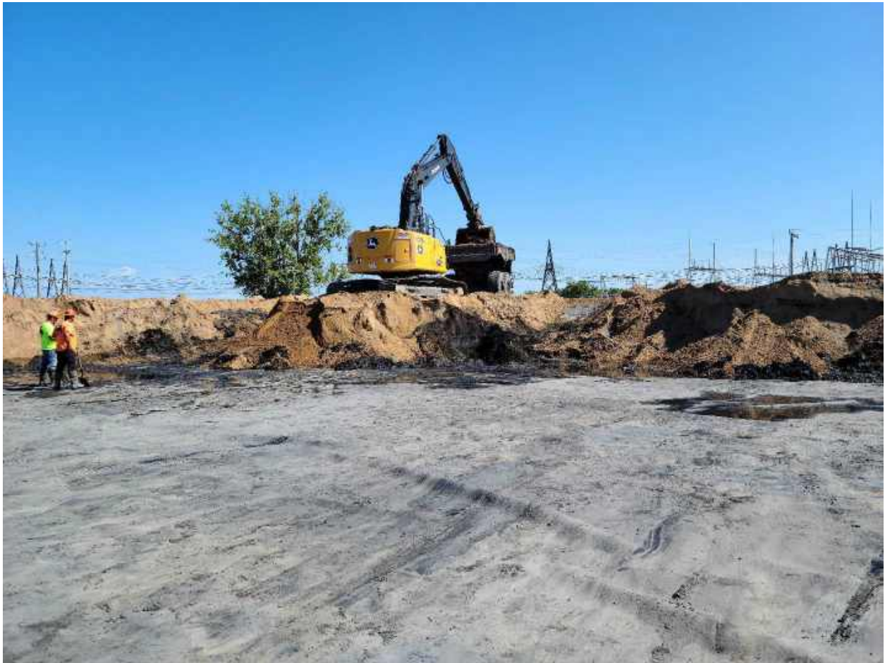
Photo 2: Fisher loading out ash/sand mix above the primary liner of the Settling Basin.
