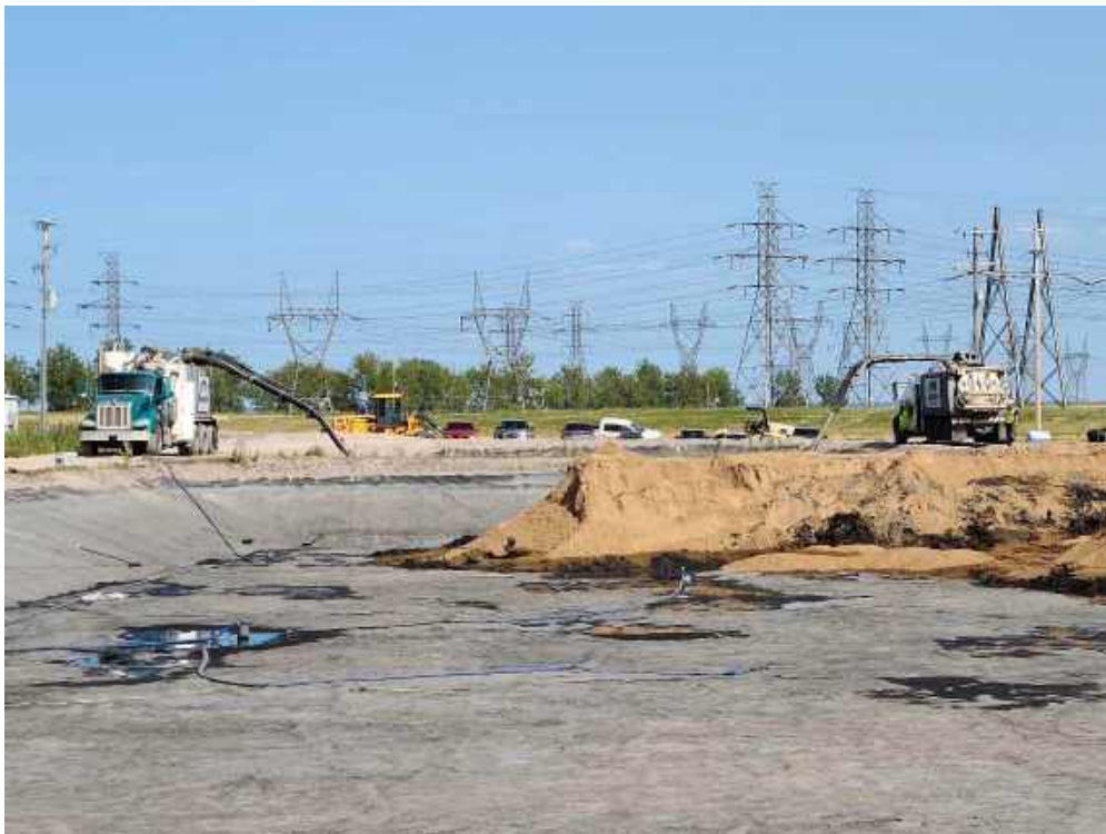
Photo 2: Fisher's progress on the Settling Basin.
