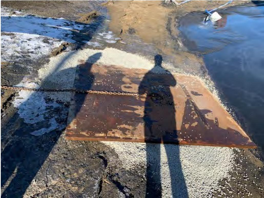
*Figure 2 - Temporary AquaBlok Backfill and Steel Plate Placement*
