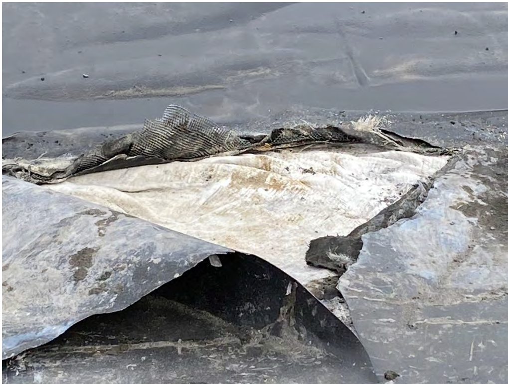
Picture 10 – Liner Repair at Visual Observation Point No. 2
