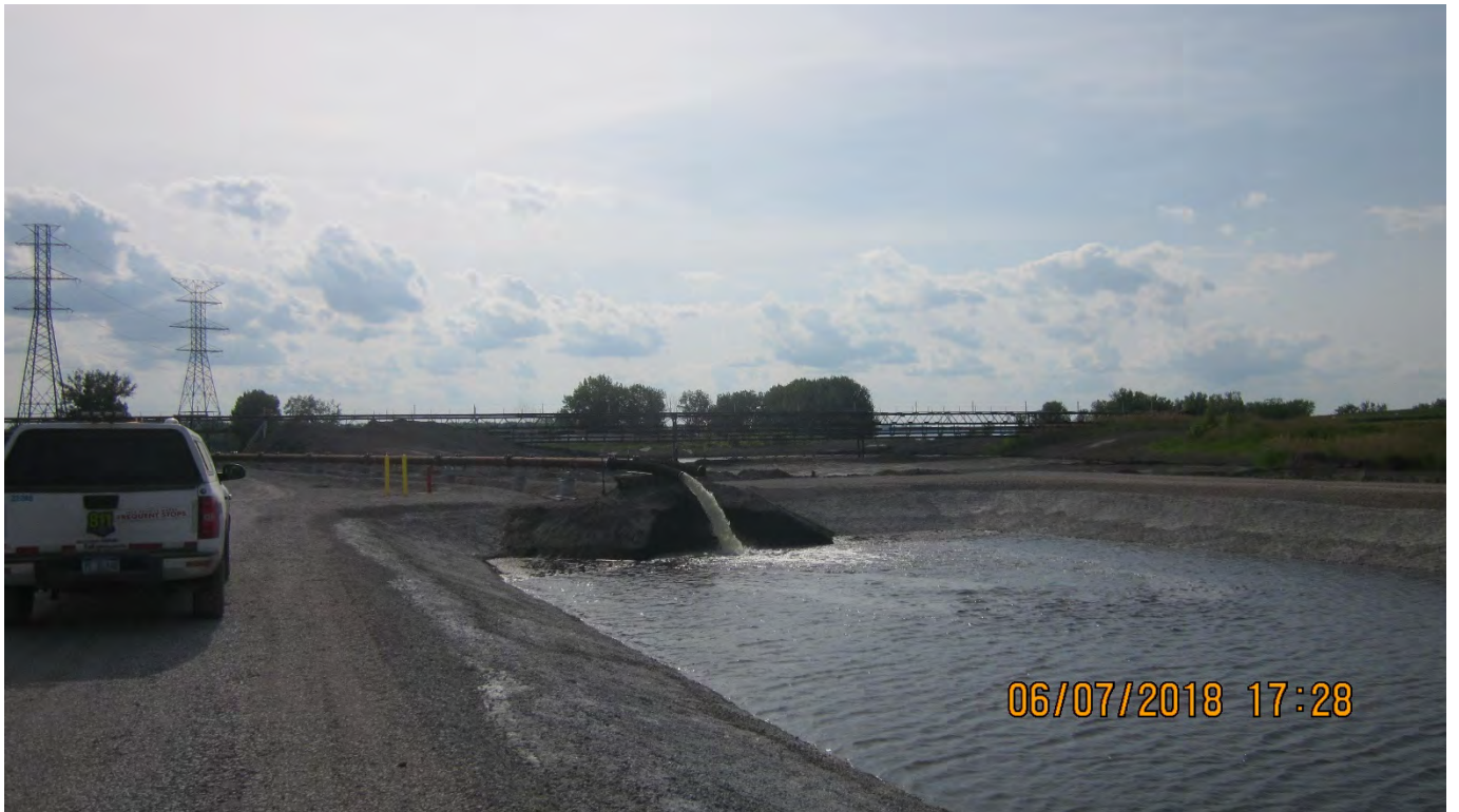
Picture 02 – View of Karn Lined Impoundment Looking West, Bottom Ash Discharge Point into Primary Basin
