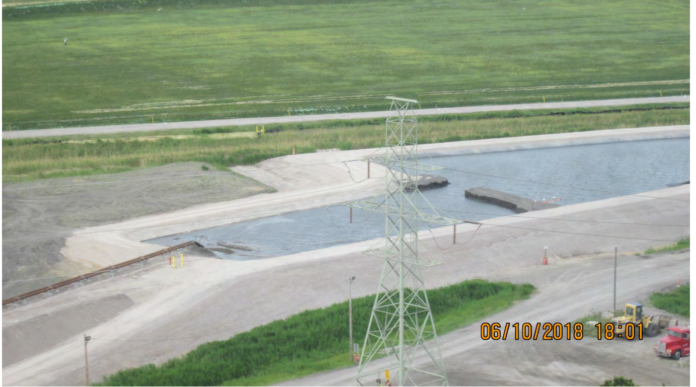
Picture 01 – View of Karn Lined Impoundment Looking North
