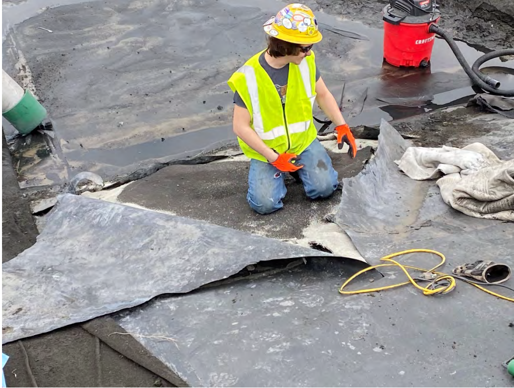
Picture 11 – Liner Repair at Visual Observation Point No. 2
