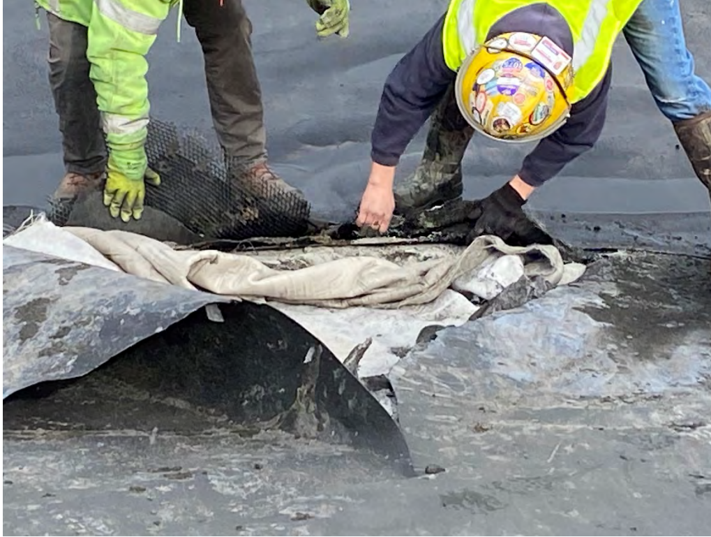
Picture 09 – Liner Repair at Visual Observation Point No. 2
