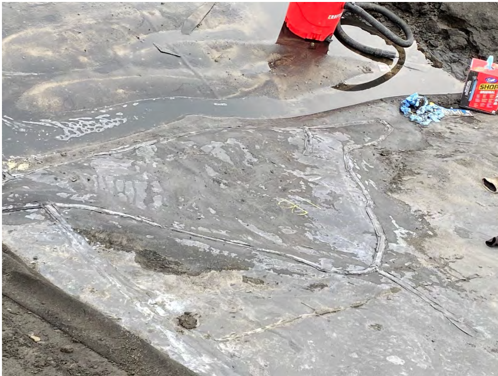
Picture 12 – Liner Repair at Visual Observation Point No. 2
