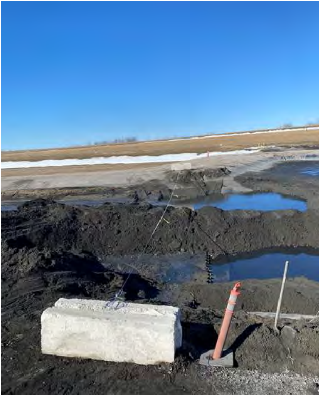
Picture 08 – Installation of Cable Wire and Concrete Jersey Barrier Engineering Control
