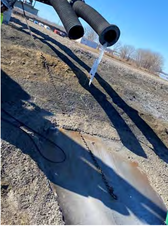
Picture 07 – Final Repair Completed at Visual Observation Point No. 1
