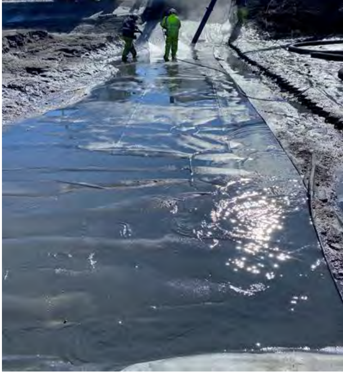
Picture 05 – Walkdown and Inspection of Locations of Previous Bottom Ash Storage
