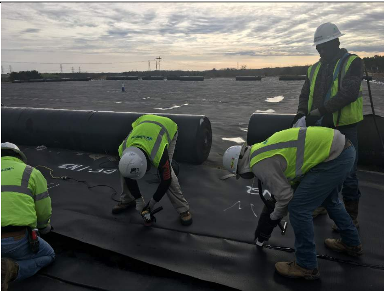
Performing extrusion welding of repairs.
