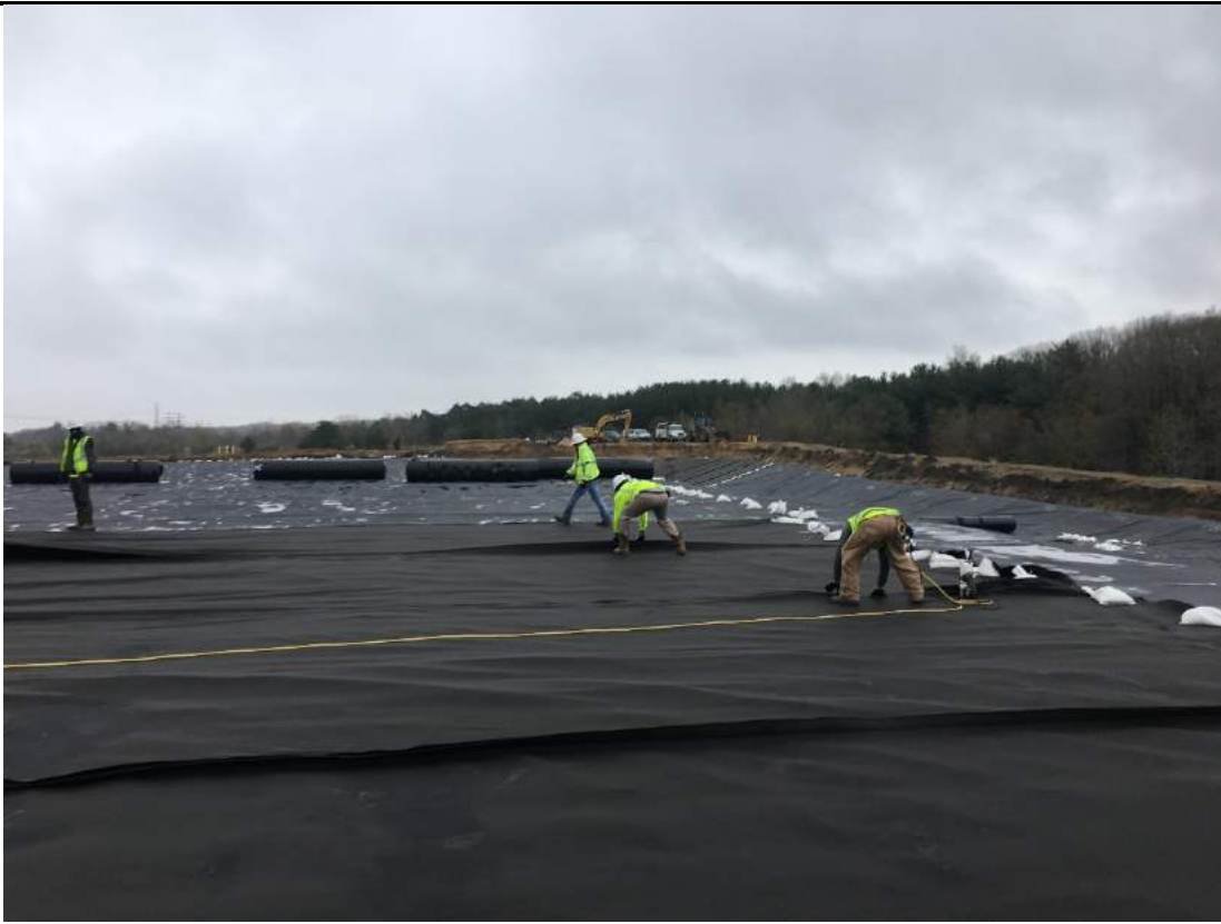
Deploying and sowing geotextile.
