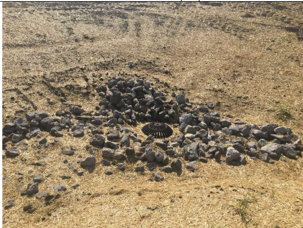
Eastern manhole with rip-wrap.
