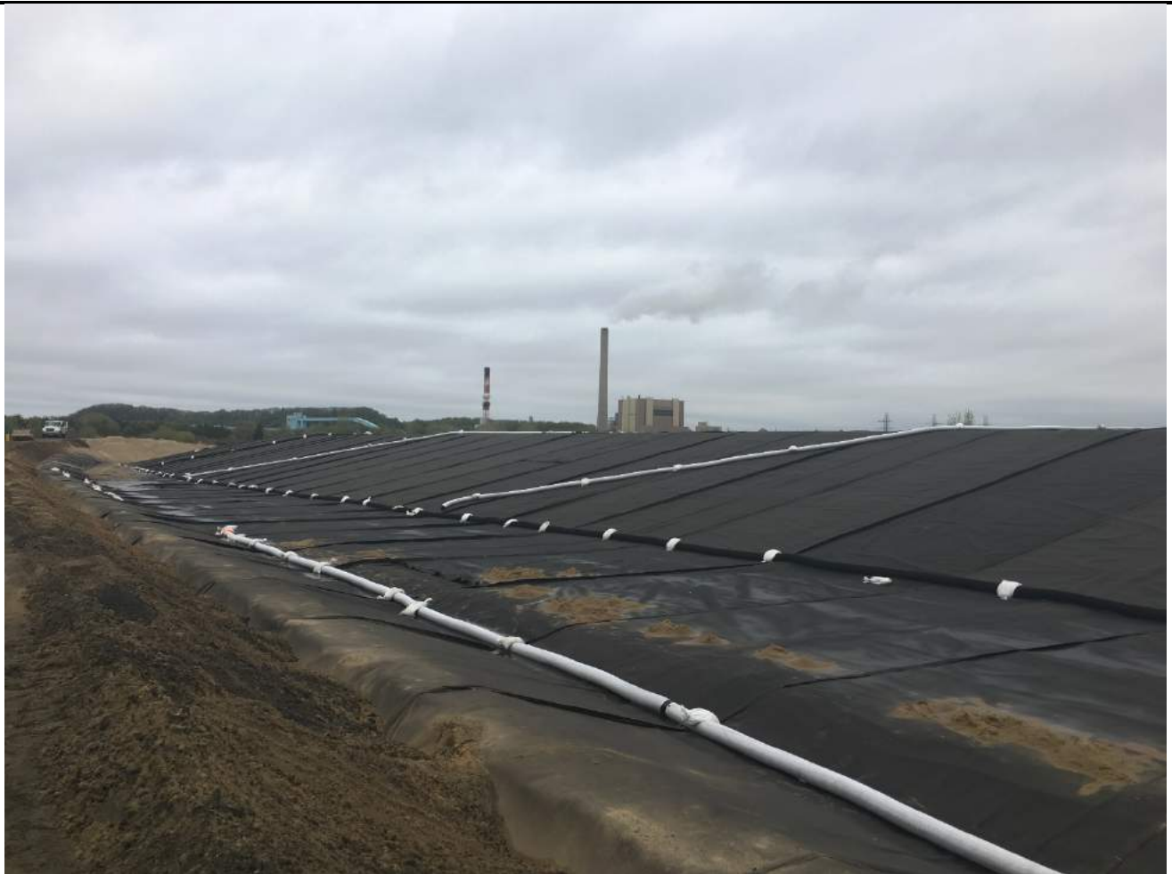
Placing 6-inch drainage tile.
