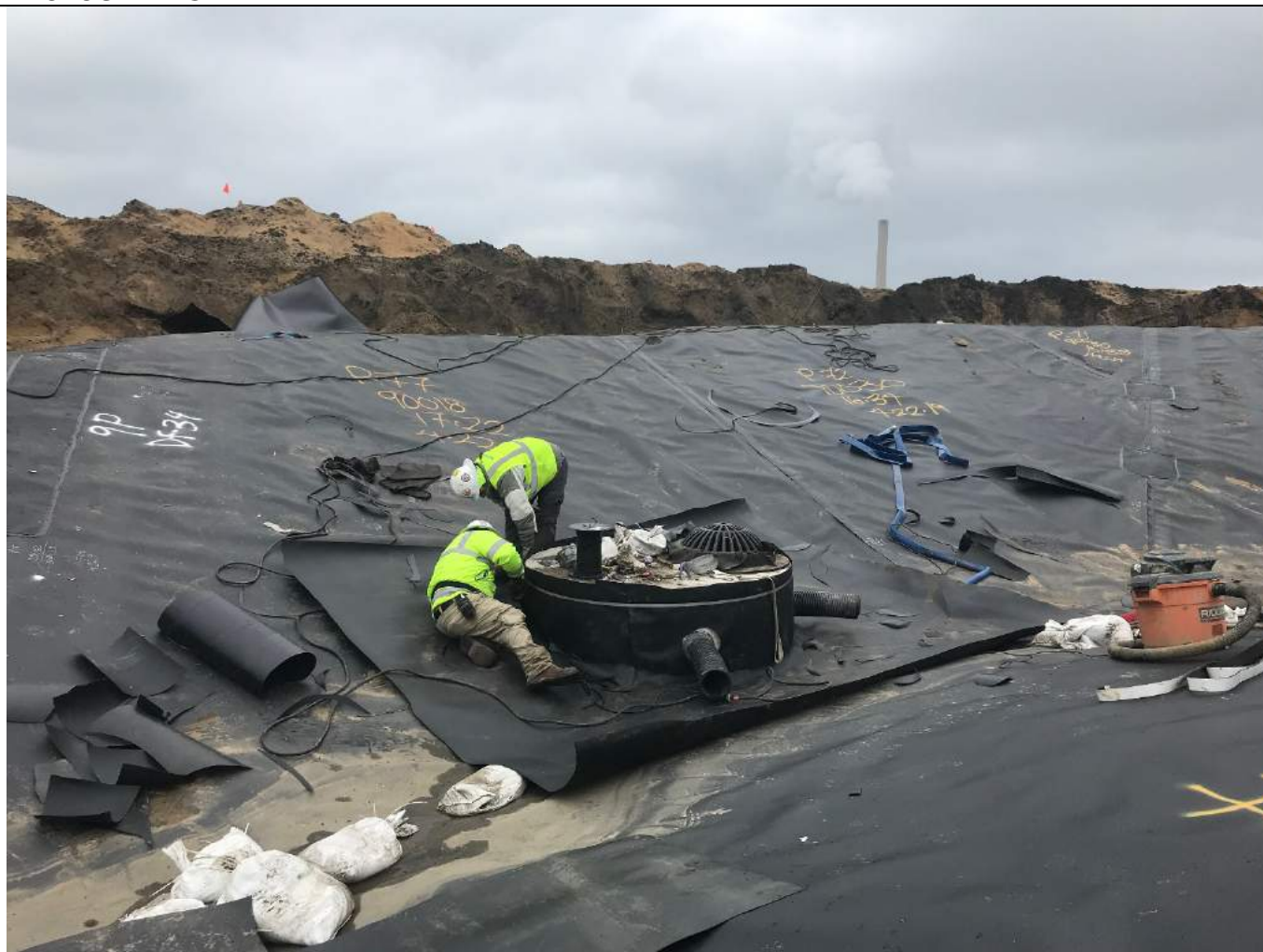
Welding repair around western stormwater drain.
