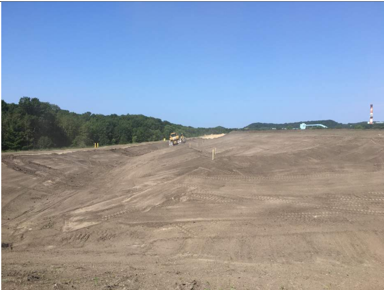
Dozer preparing top of topsoil on the northern side of Pond A.
