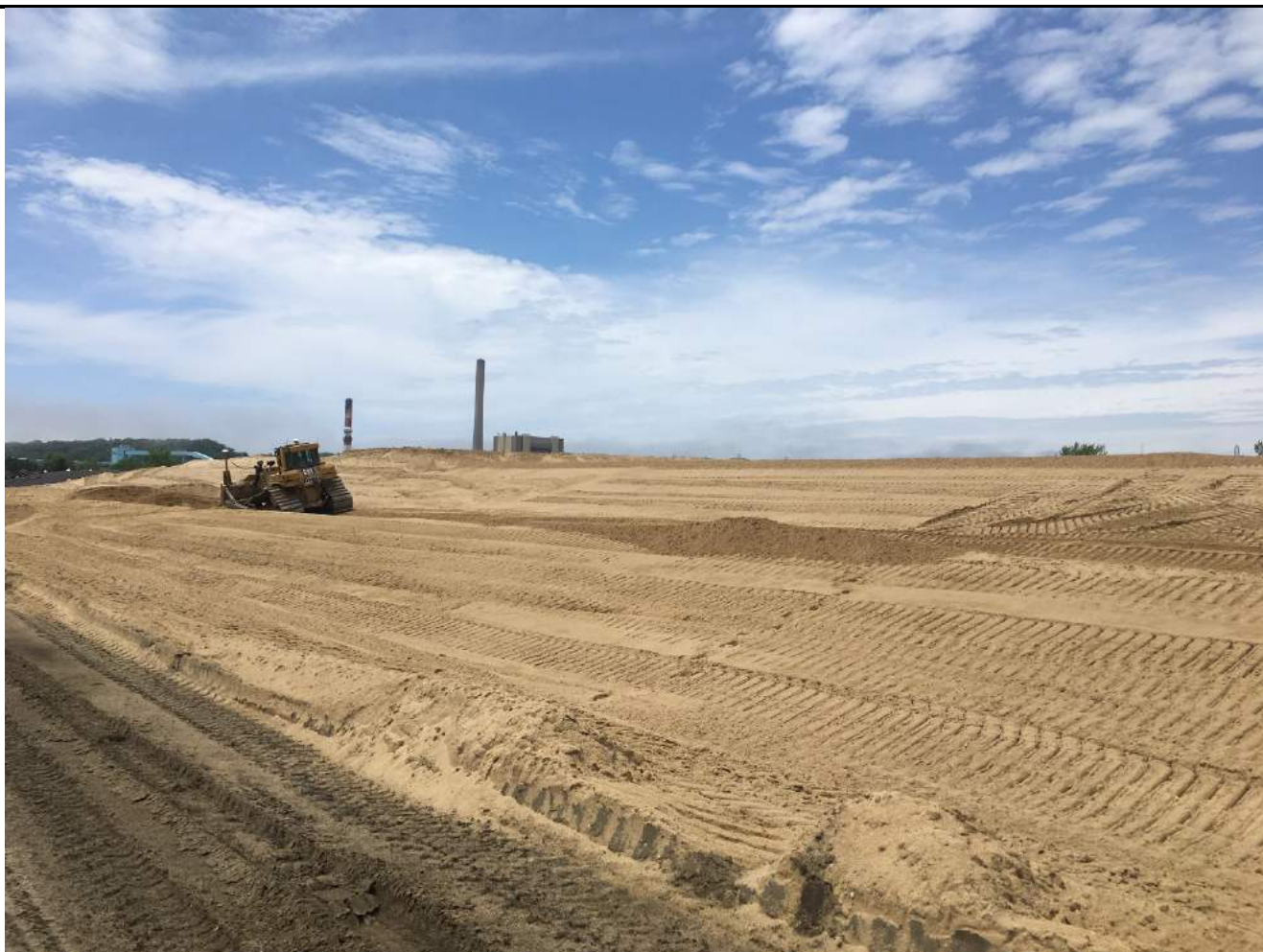
Dozer grading cover material of Pond A.
