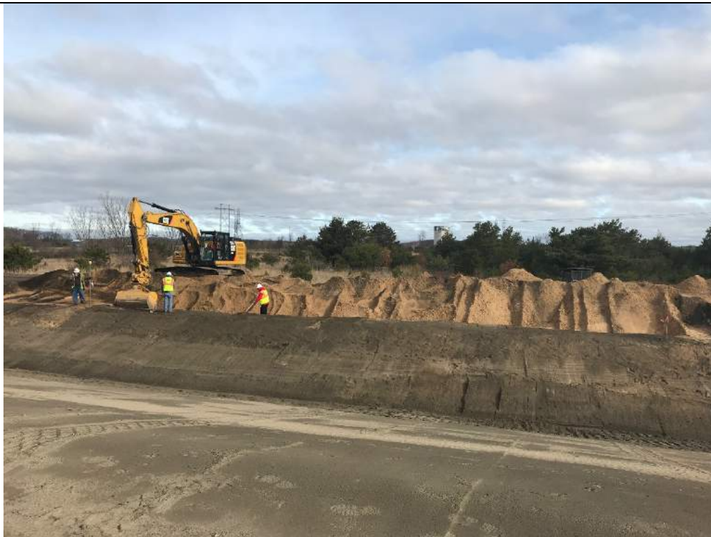
Ryan excavating anchor trench on the north side of Pond A.
