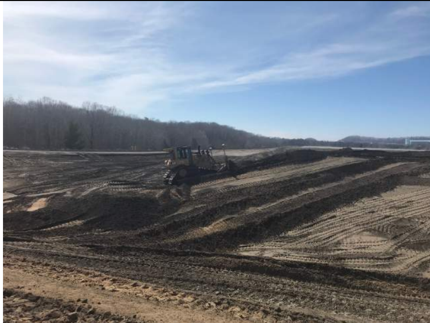
Dozing subgrade to meet tolerance.
