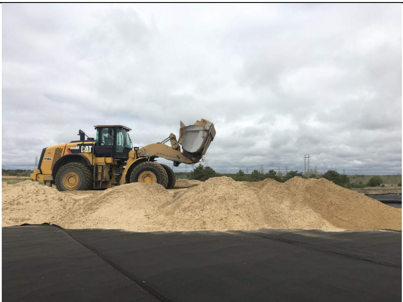
Placing cover material on top of Pond A.
