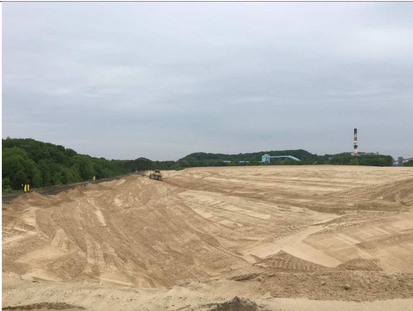
Dozer grading cover material of Pond A.
