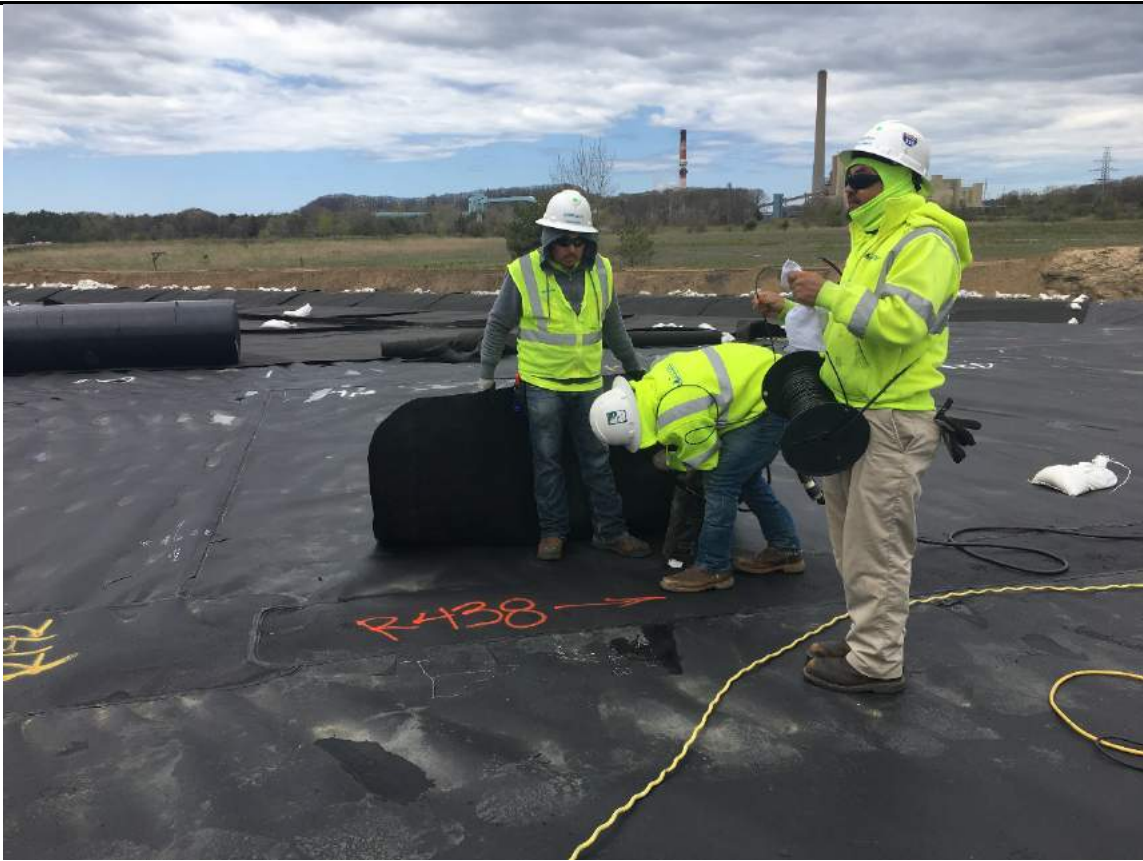
Extrusion welding cap on top of Pond A.
