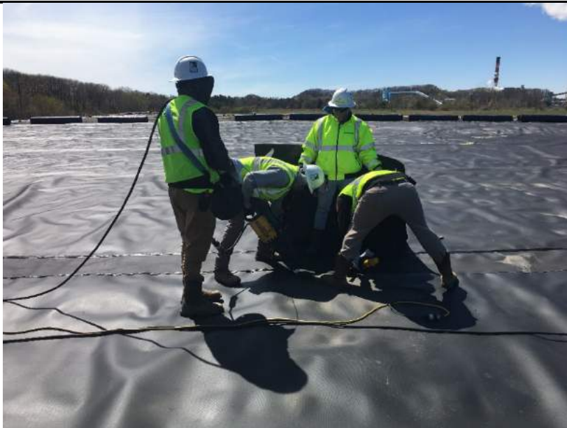
Extrusion welding caps.
