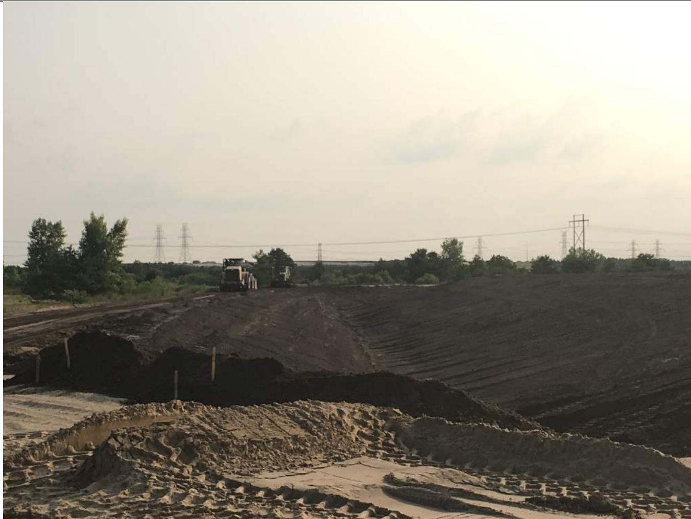
Grading of topsoil at the west end of Pond A.
