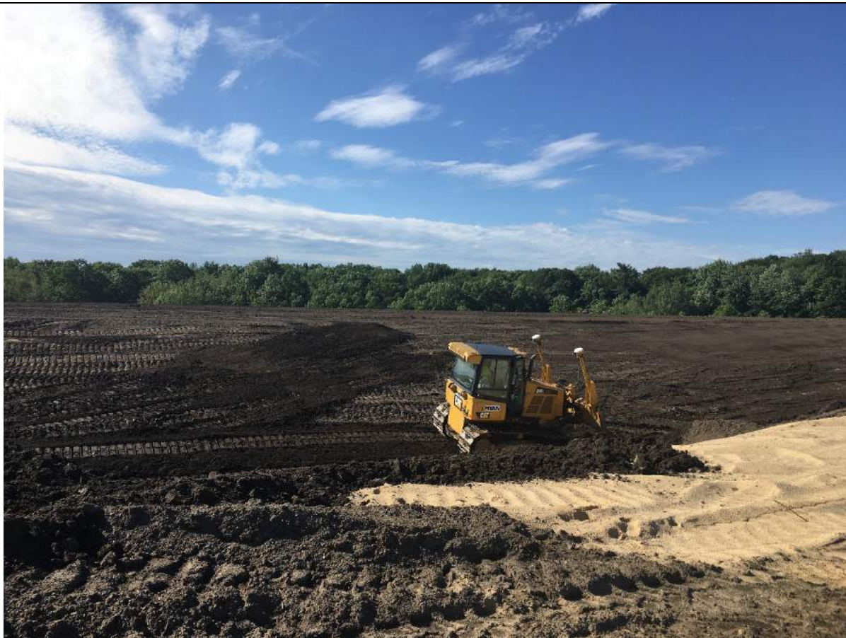
Grading topsoil at the west end of Pond A.
