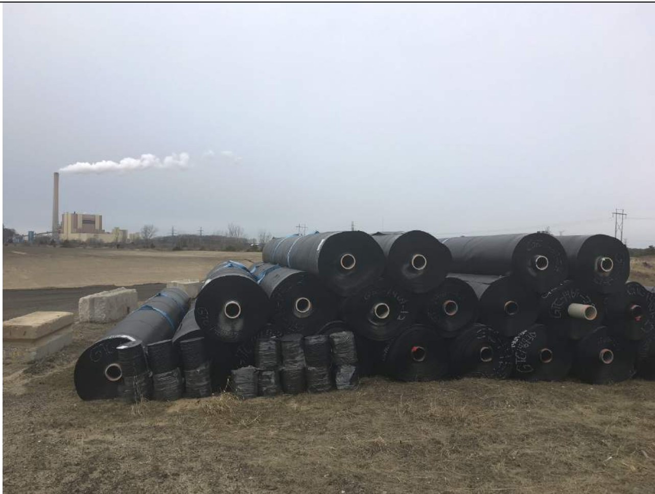
Stockpiled Geosynthetic Material for Pond A.
