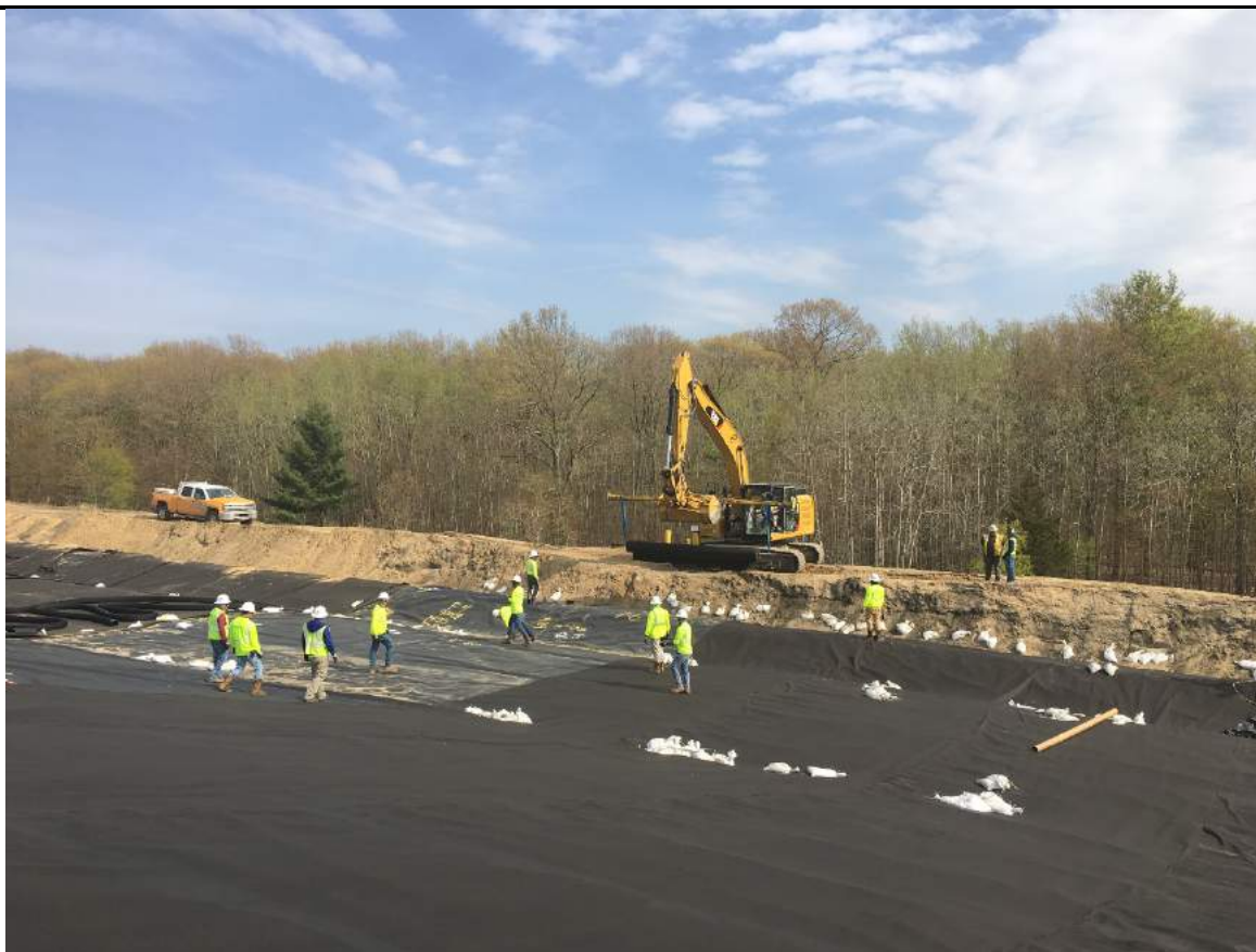
Geotextile being placed over 4/13 welded seams.
