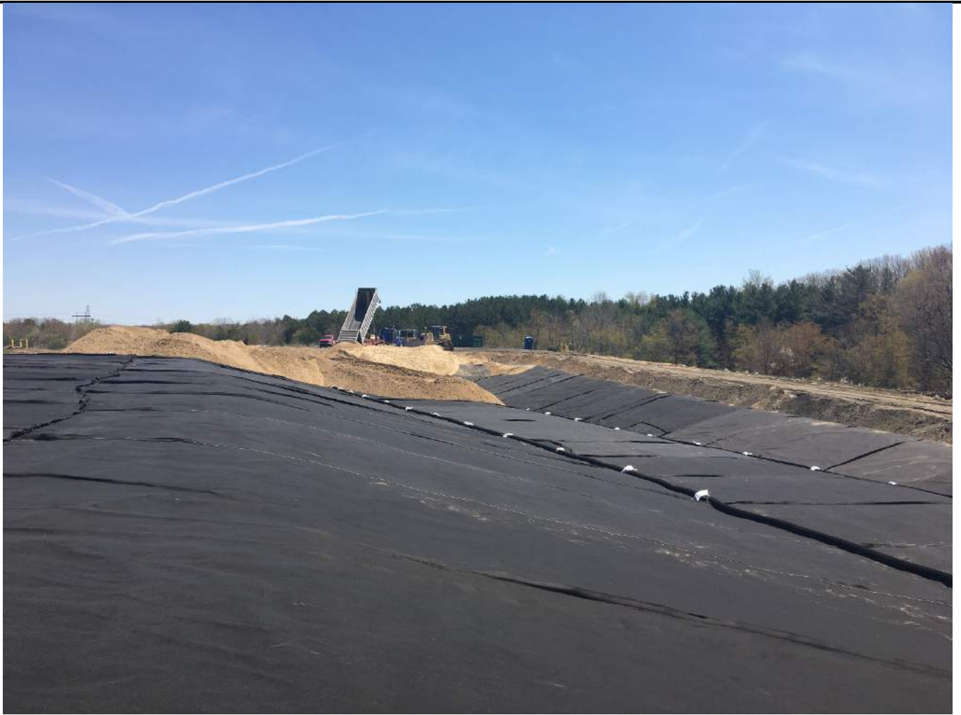
Cover material and 6-inch drain tile.
