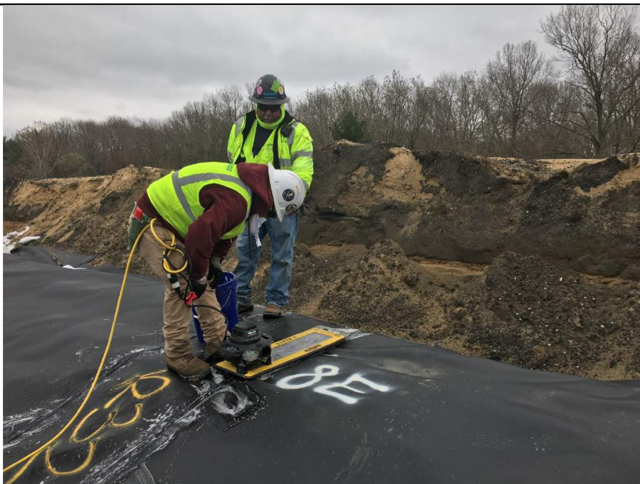
Vacuum testing repairs
