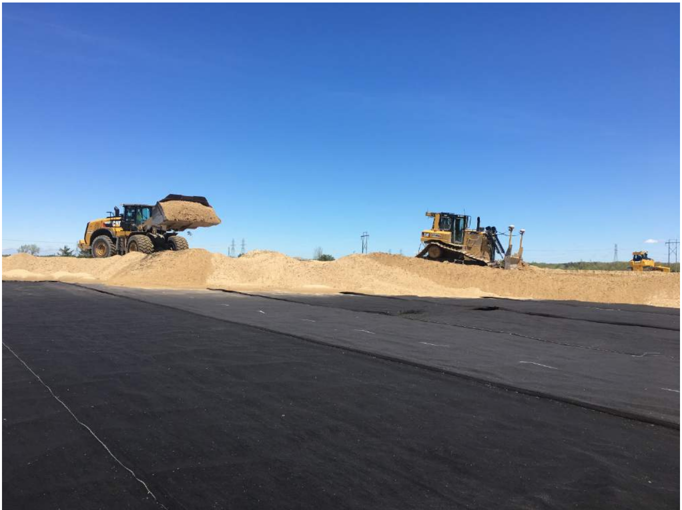
Grading and placing cover material in the northwest corner of Pond A.
