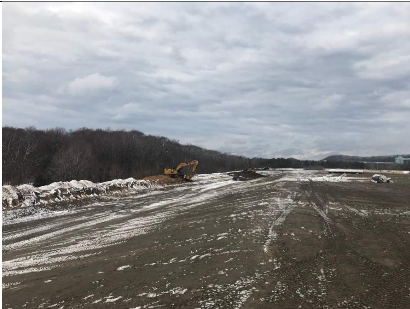
Ryan excavating the anchor trench on the south side of Pond A.
