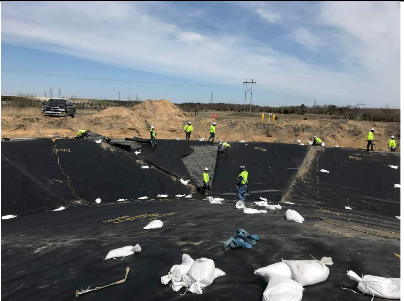
Fusion welding geosynthetics in the northeast corner of Pond A.
