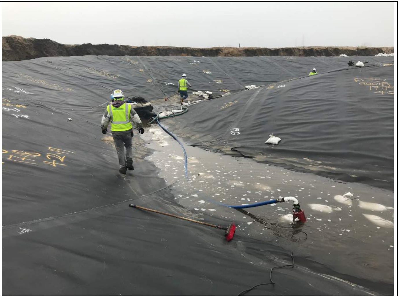
Sump-pump dewatering western end of Pond A
