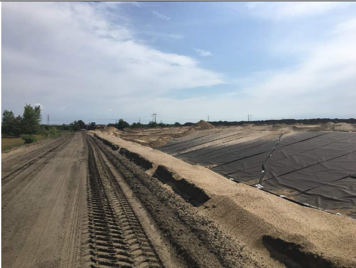
Placing cover material at the west end of Pond A.
