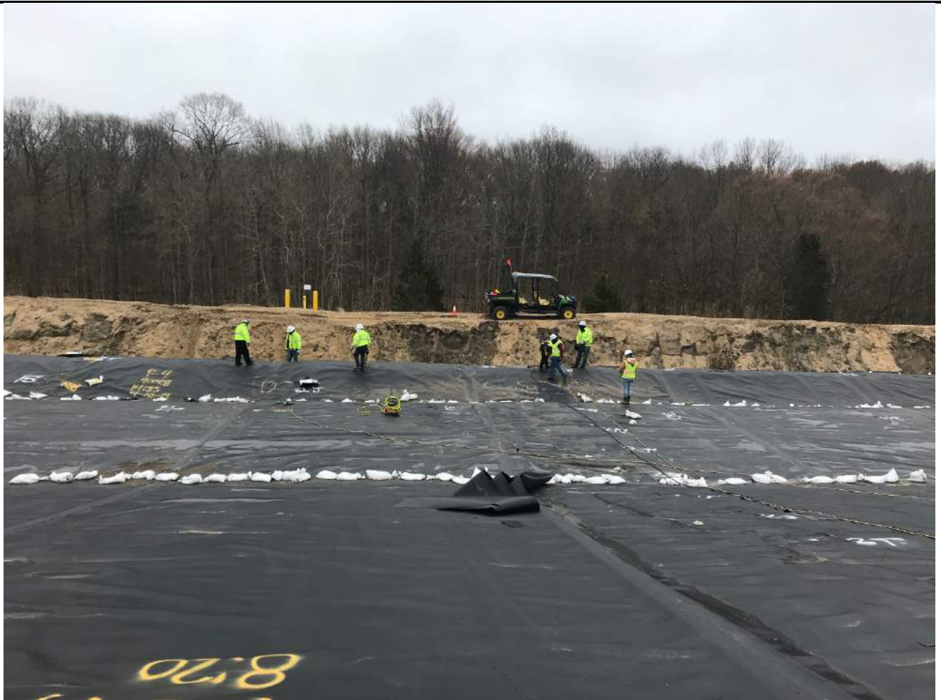
Extrusion welding repairs along south side of Pond A.
