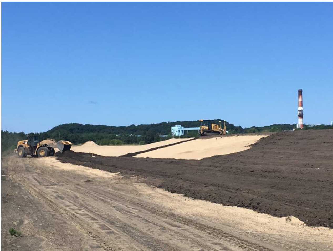
Placing and grading topsoil at the west end of Pond A.
