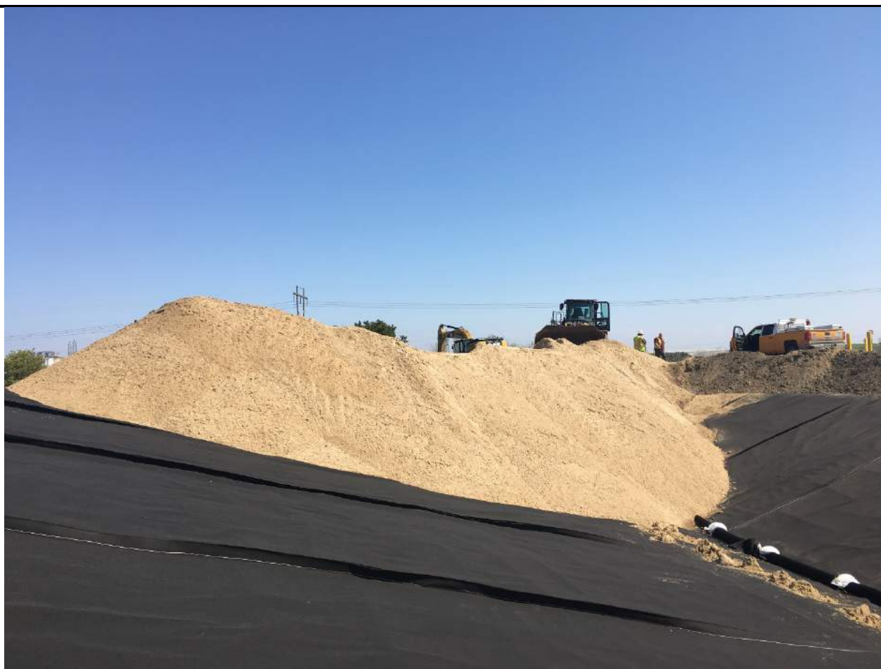
Cover material being placed in the northeast corner.
