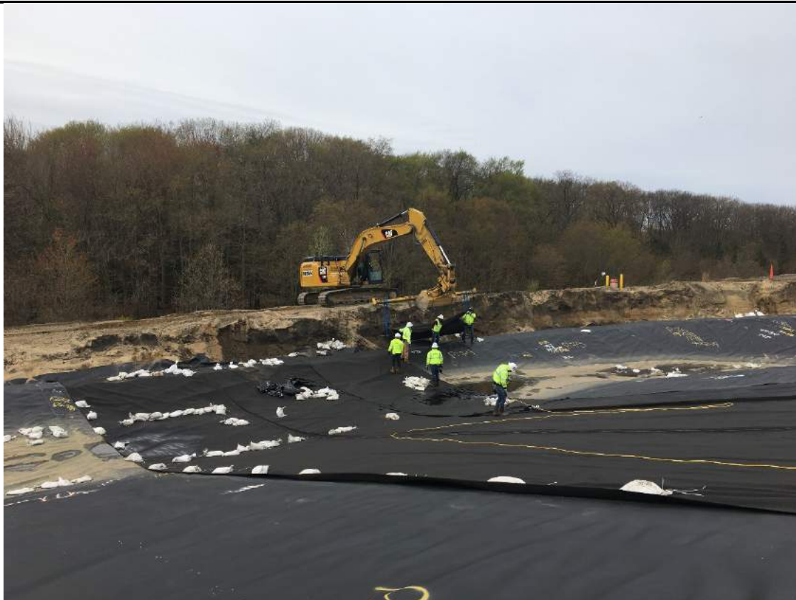
Placing and sowing seams of textile on west end of Pond A.
