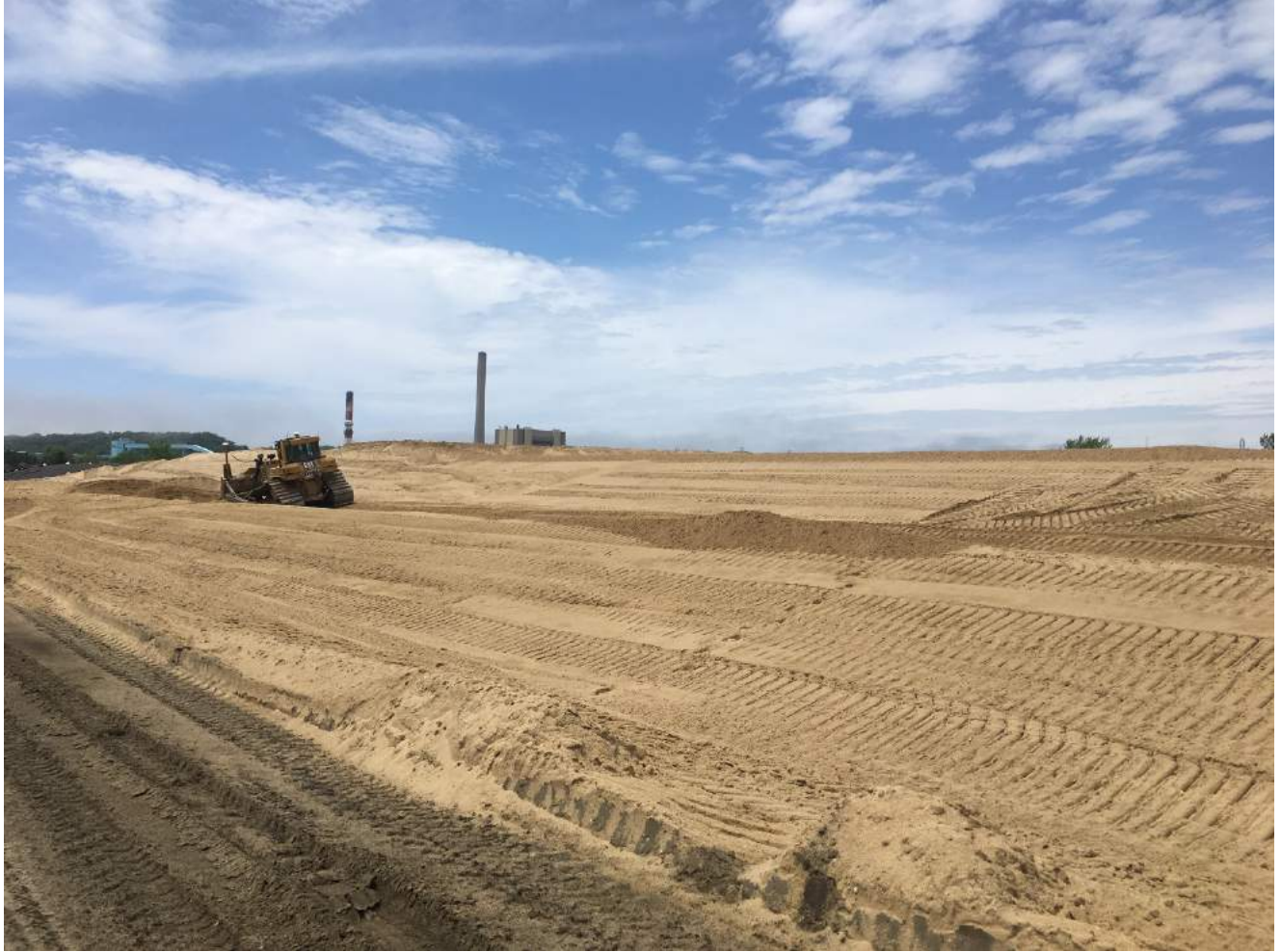
Dozer grading cover material of Pond A.
