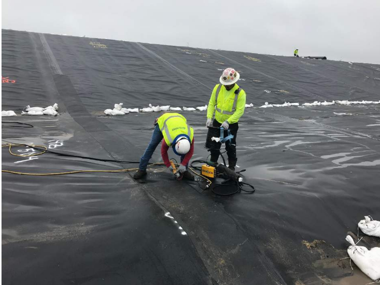
Extrusion welding repairs.
