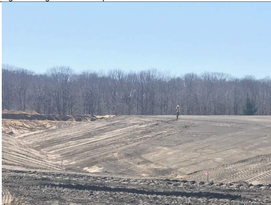
Ryan laborer rock-picking subgrade.
