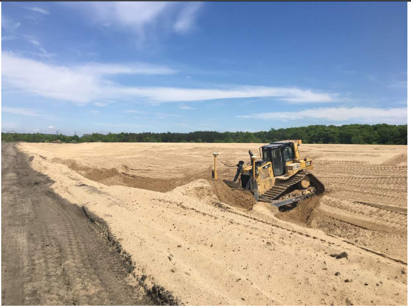
Dozer placing cover material over repaired area.
