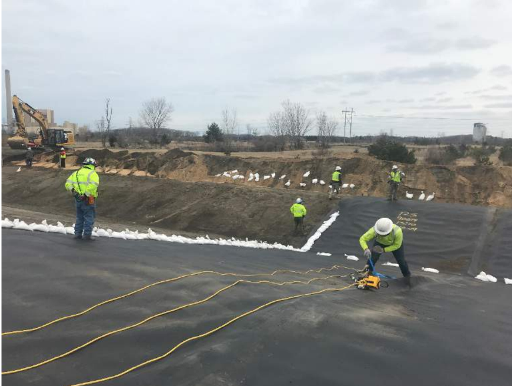
Fusion seaming along the north slope of Pond A.
