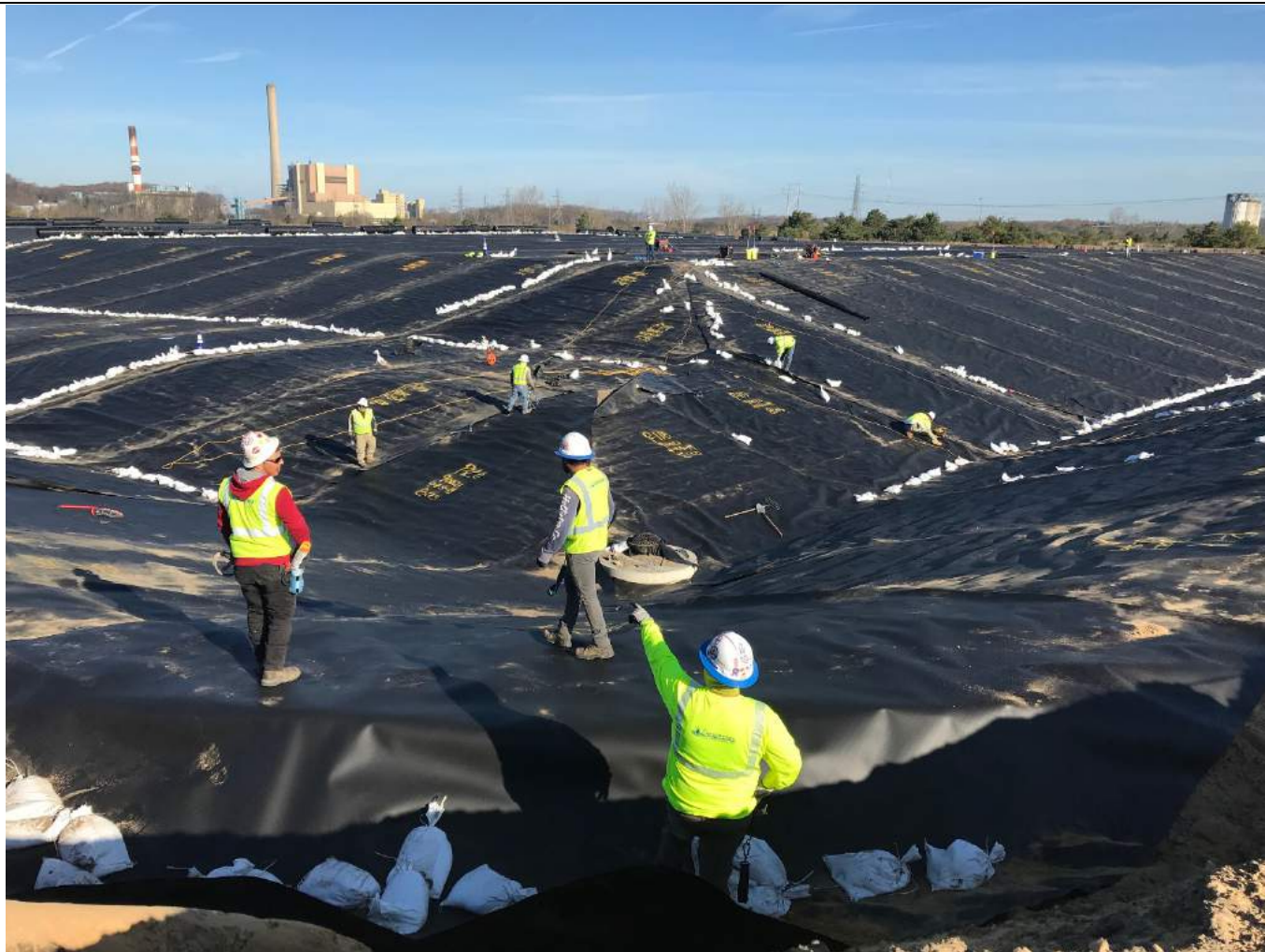
Fusion seaming the last of the geomembrane for Pond A.
