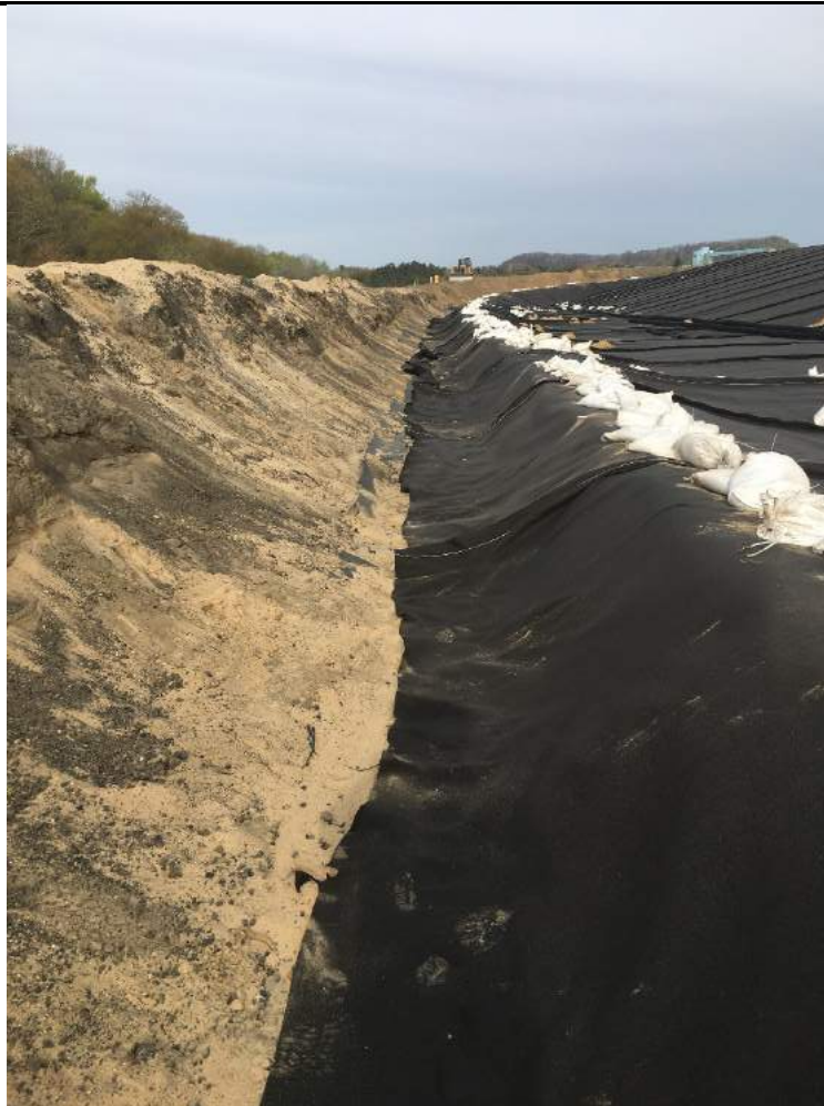
Sandbags removed from the anchor trench.
