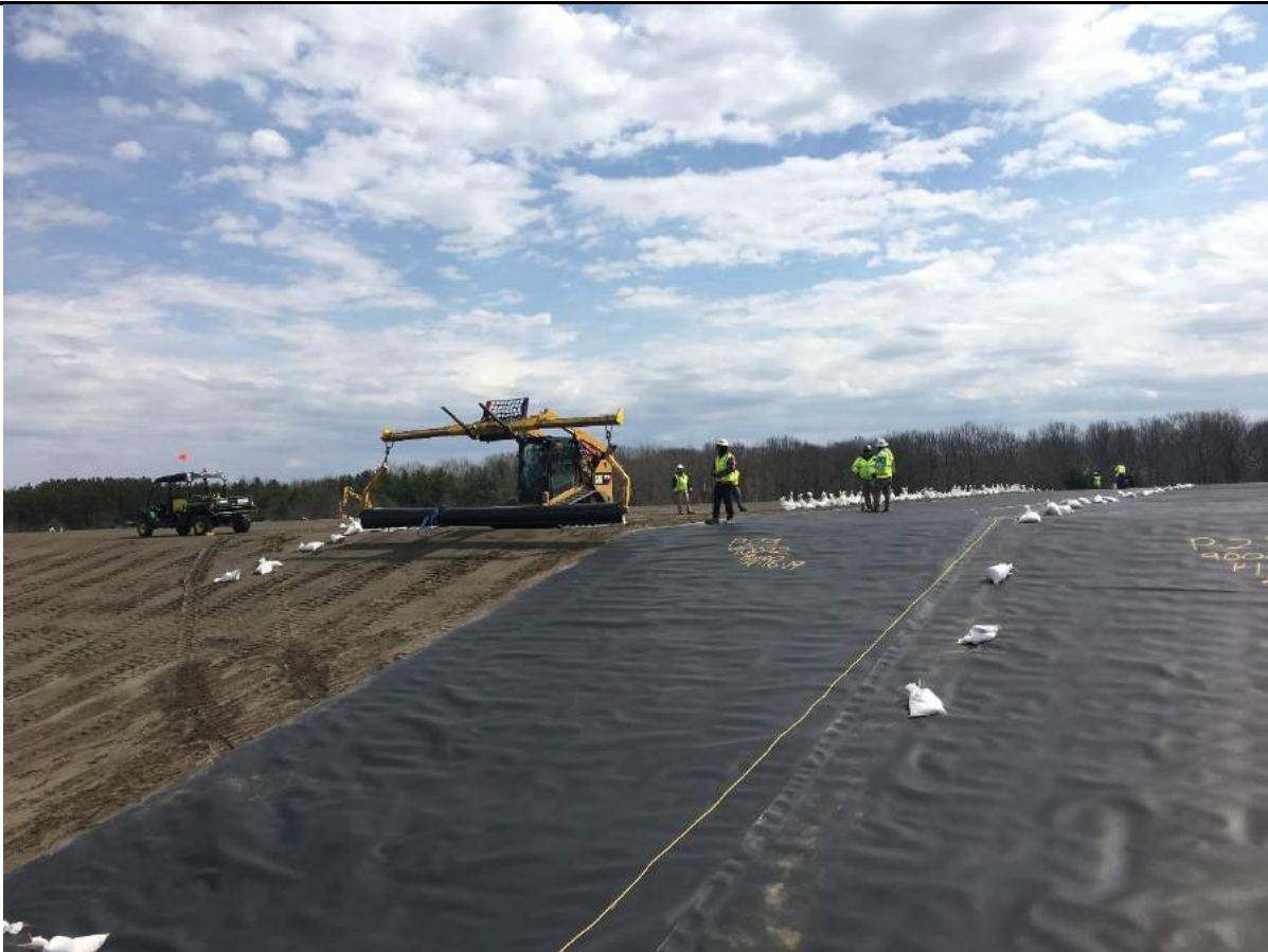
Cat skid-steer deploying geomembrane.
