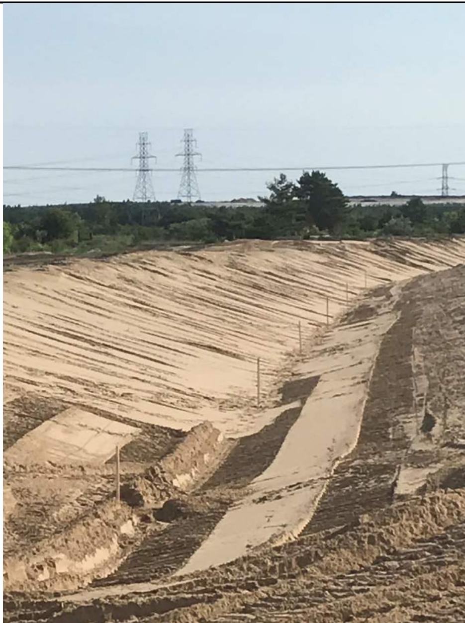
Cert points along the toe of slope.
