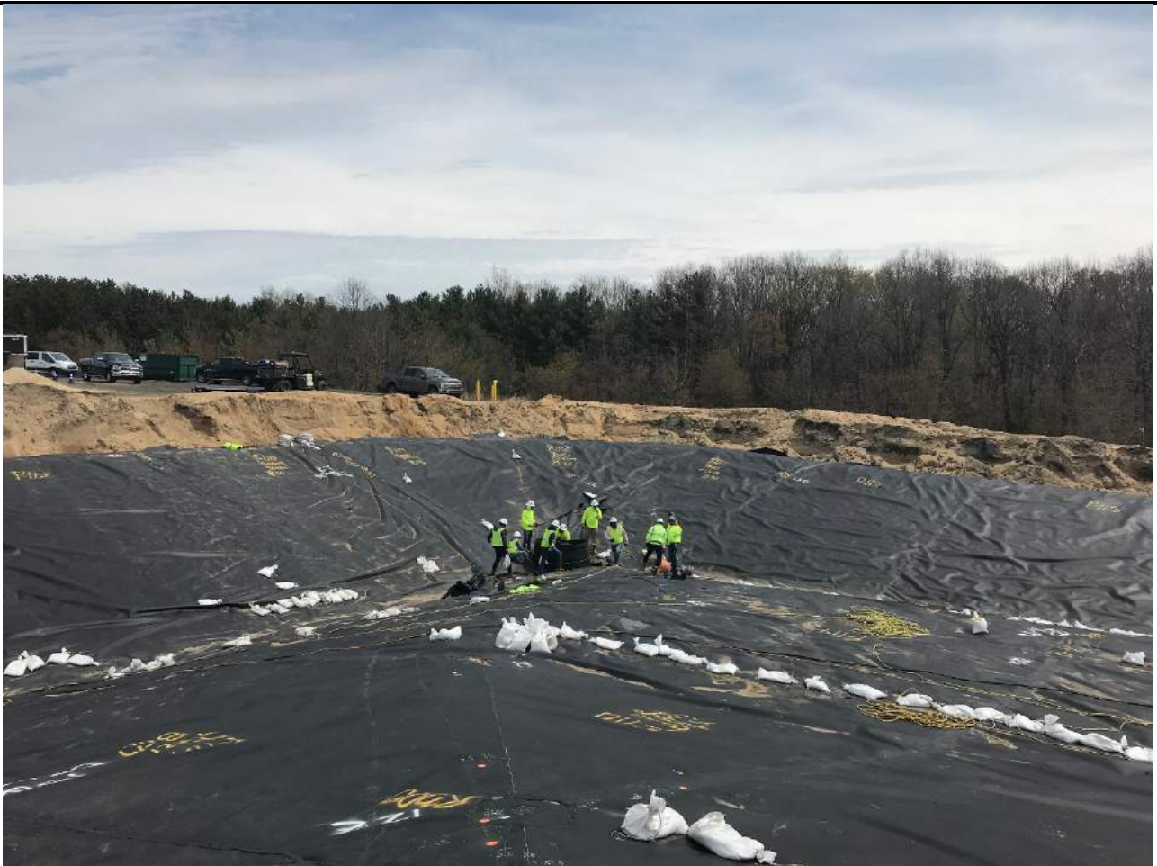
Began welding boot for eastern stormwater manhole
