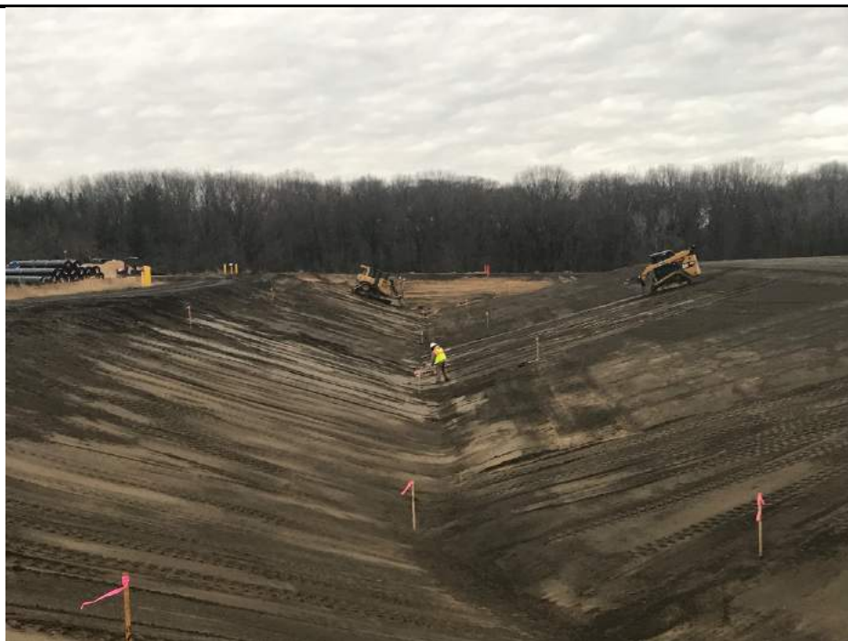
Ryan preparing subgrade along the eastern slope of Pond A.
