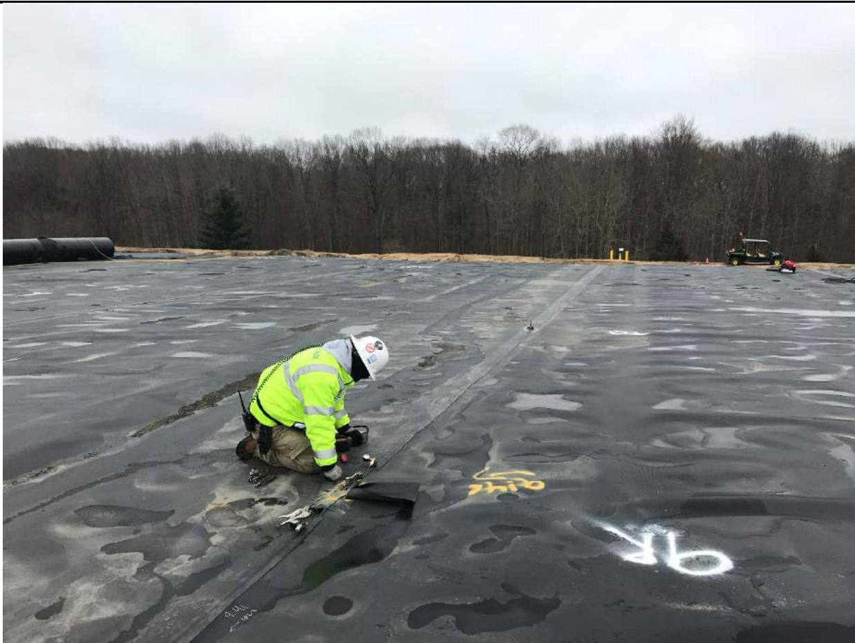
Pressure testing seams.
