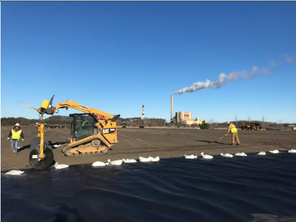
CAT Skid-steer about to deploy liner and Ryan laborer raking subgrade prior to deployment.
