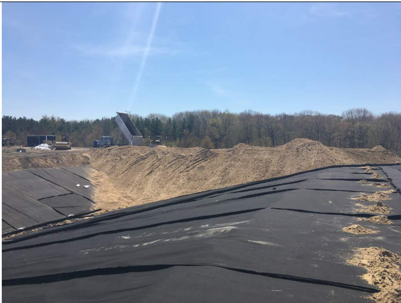
Cover material being placed in the southeast corner.
