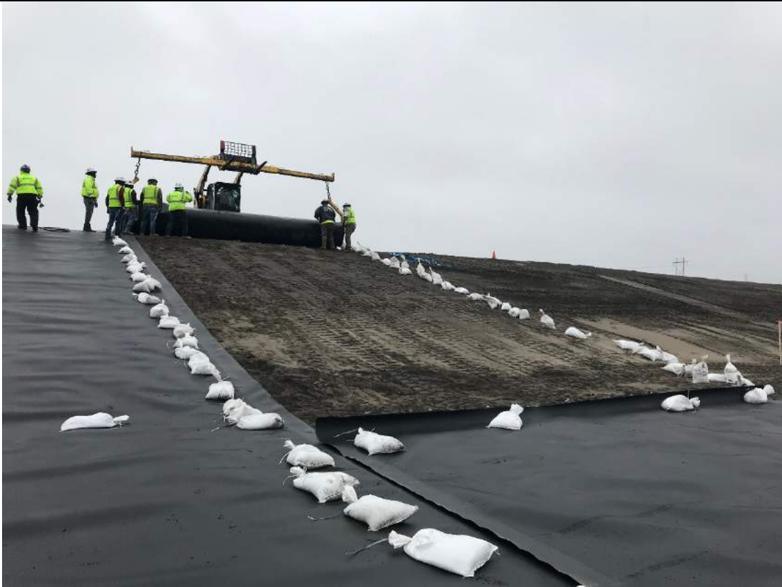
CAT Skid-steer deploying geomembrane.
