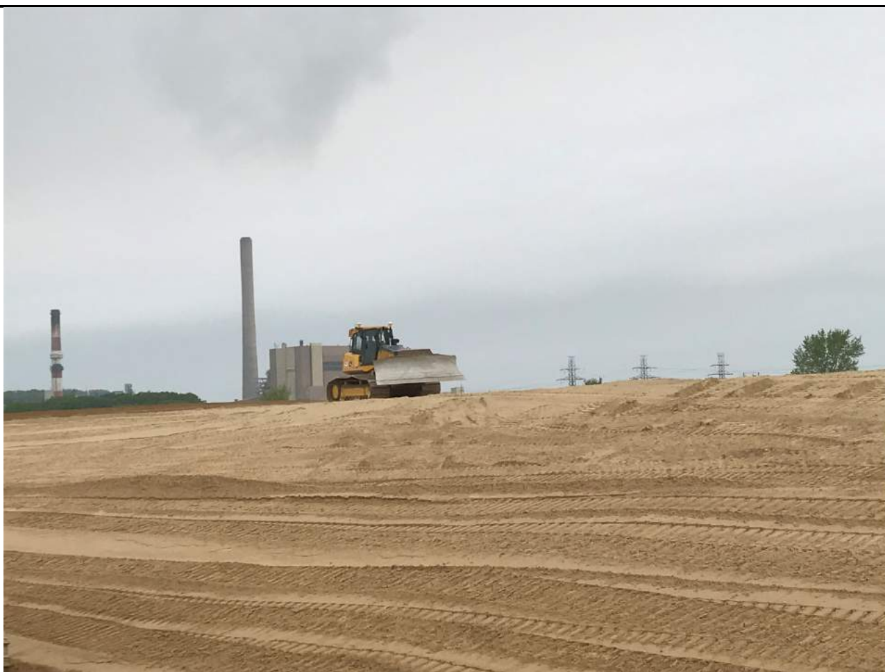
Grading cover material in Pond A.
