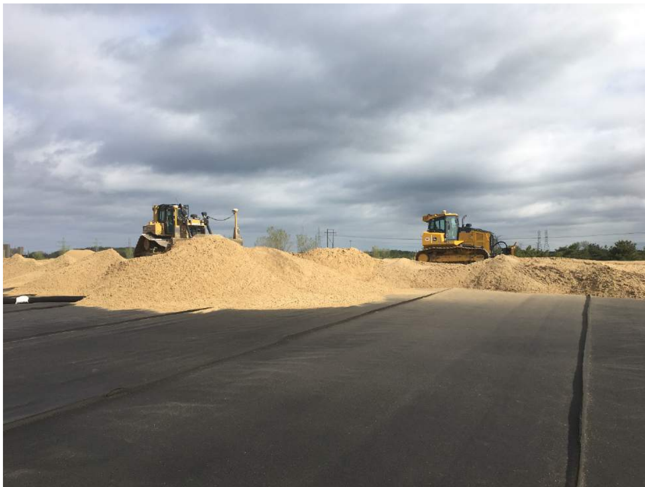
Grading cover material in the northwest corner of Pond A.
