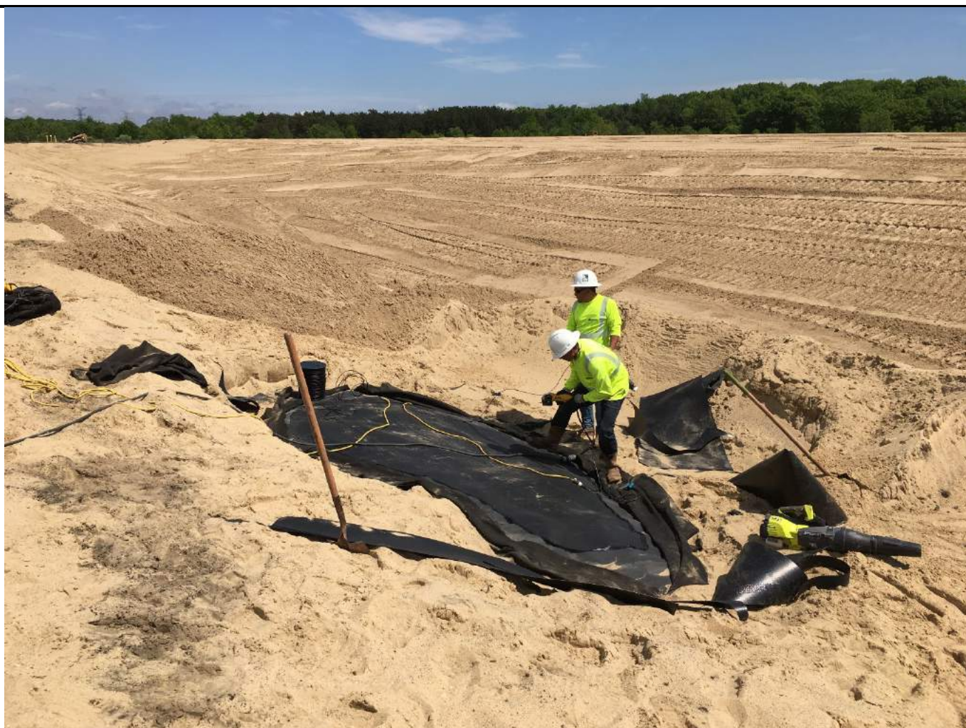
Chesapeake extrusion welding patch over repair.
