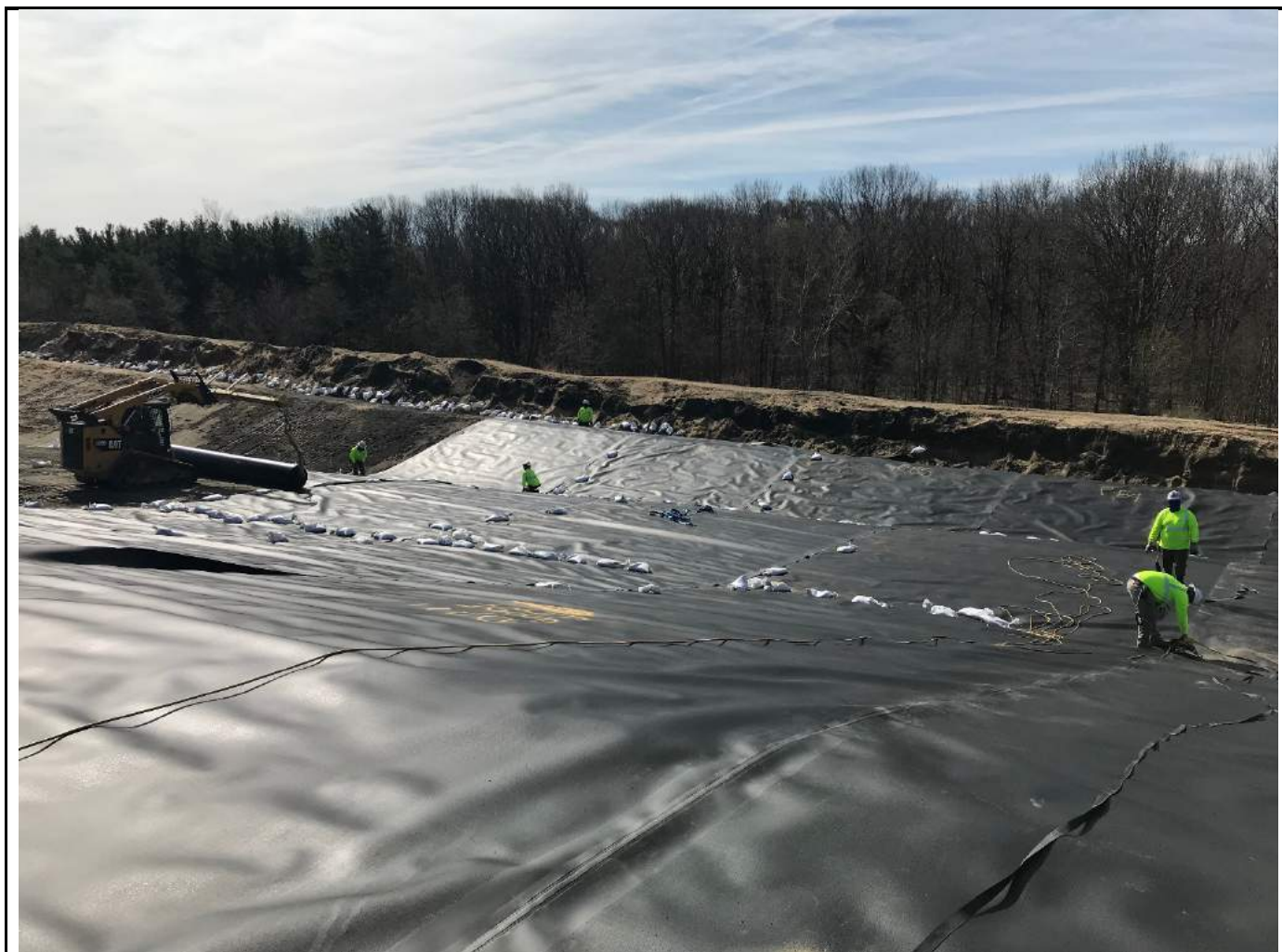
Fusion welding and deploying geosynthetics along the south side of Pond A.
