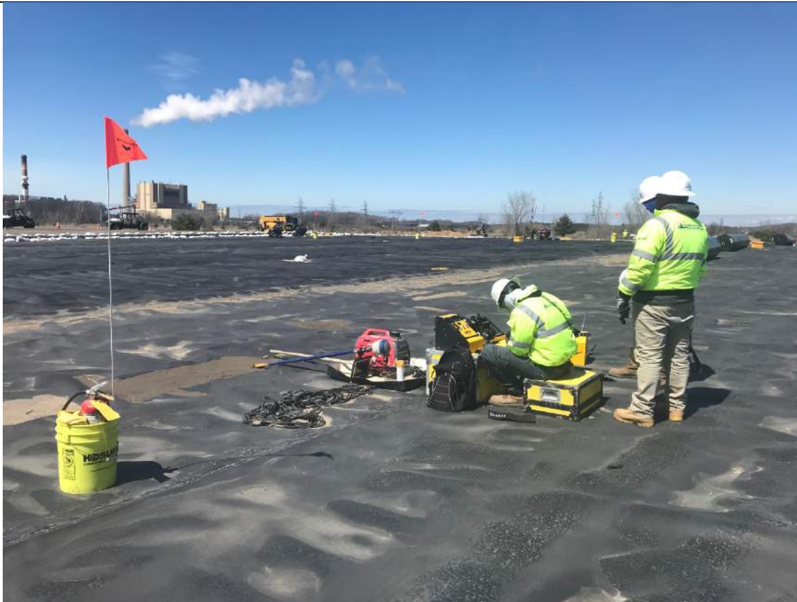
Testing fusion trial seams.
