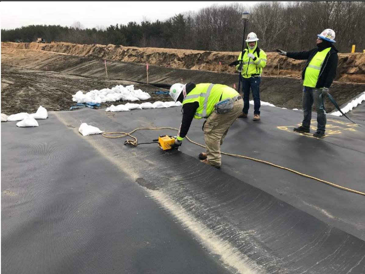
Fusion Seaming of cross seam.
