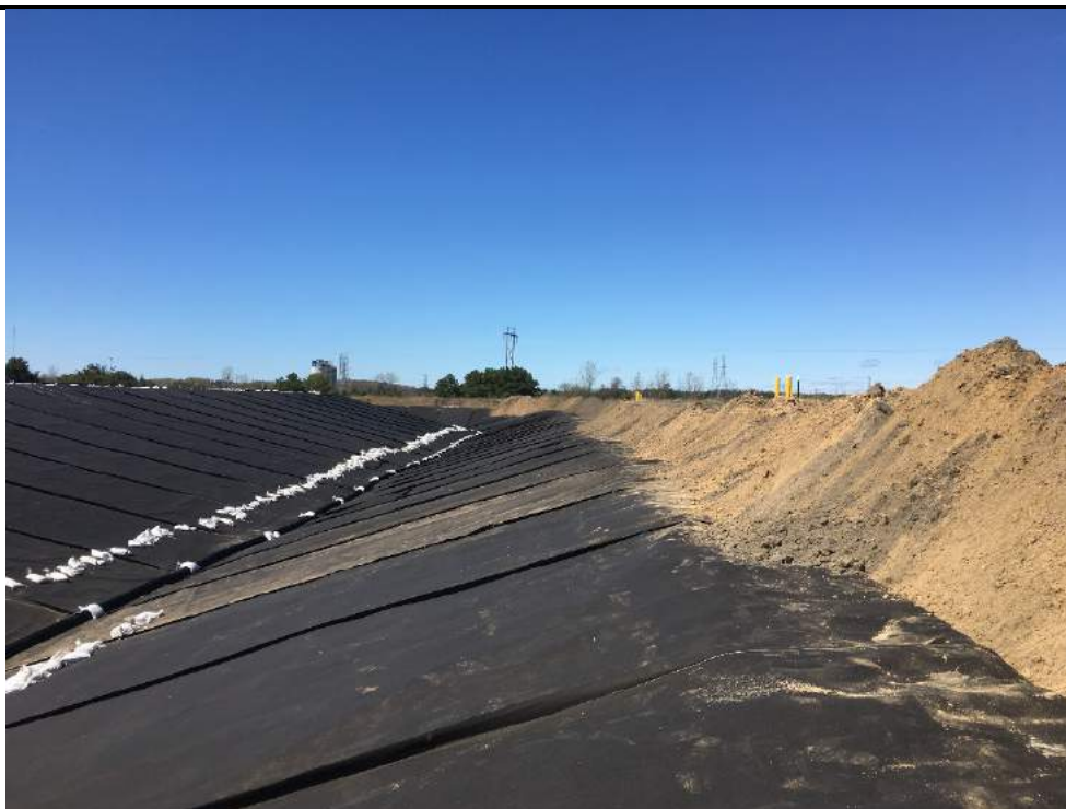
Backfilled anchor trench along the eastern edge of Pond A.
