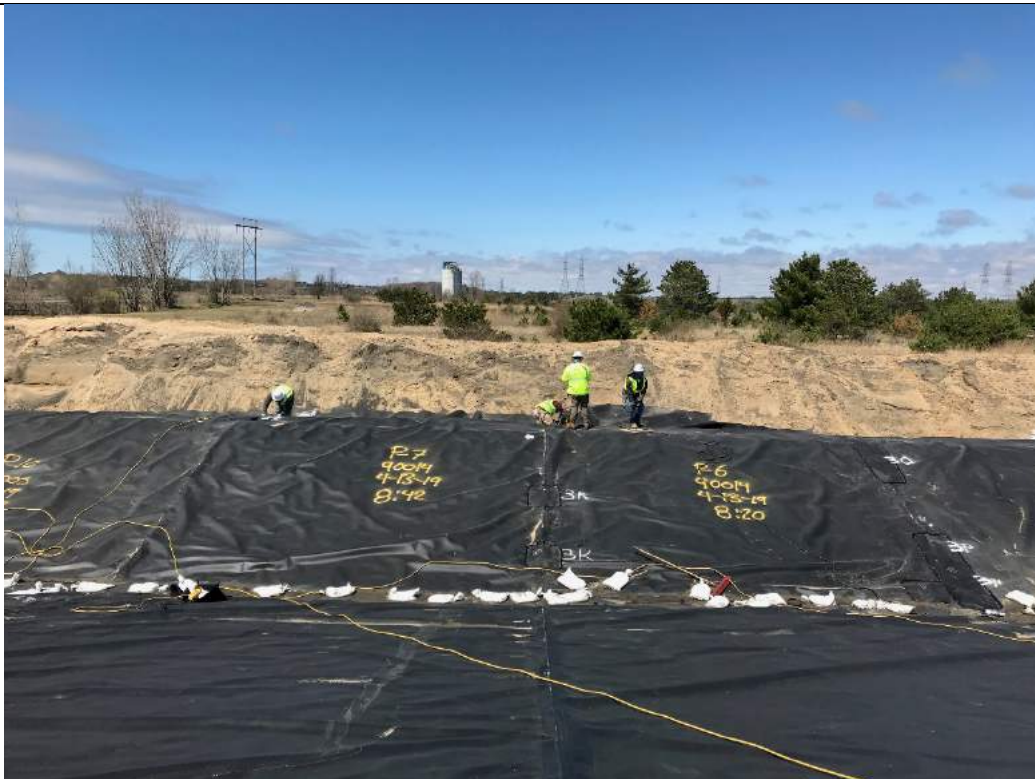
Extrusion welding repairs along the north side of Pond A.
