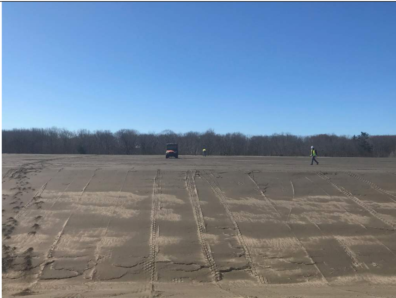
Ryan laborers rock-picking Pond A subgrade
