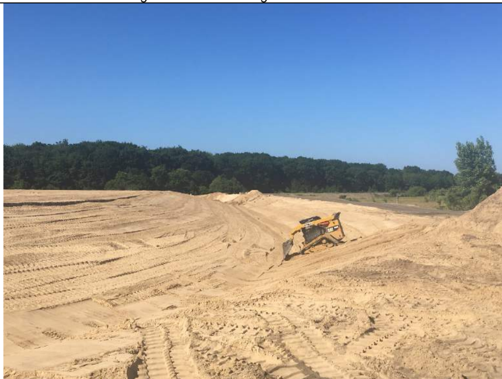
Skid-steer preparing subgrade
