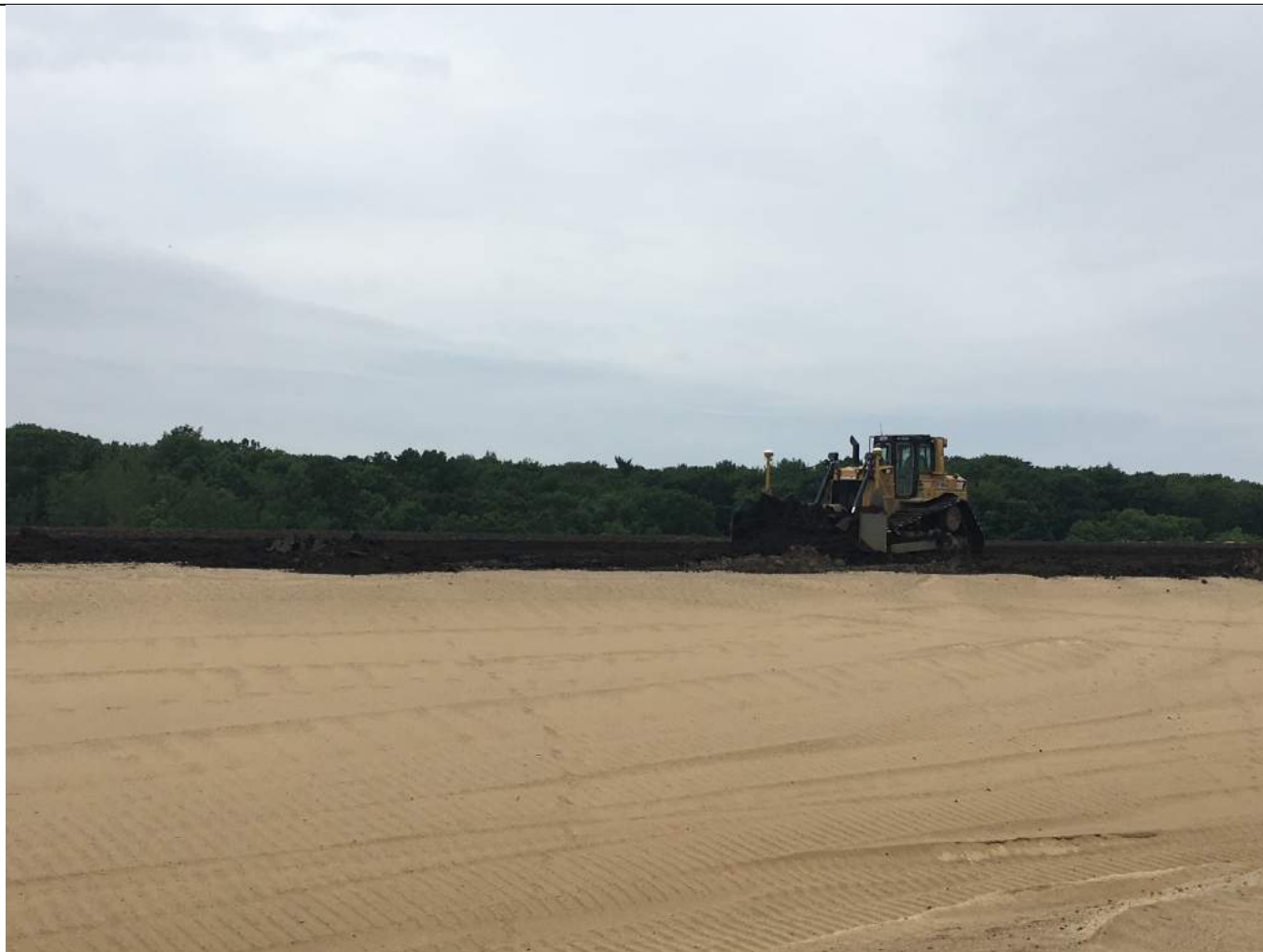
Delivery and grading of topsoil.
