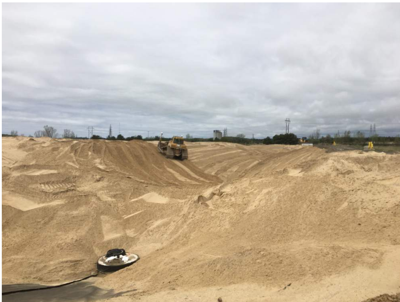
Pushing out cover material in the southeastern corner of Pond A.
