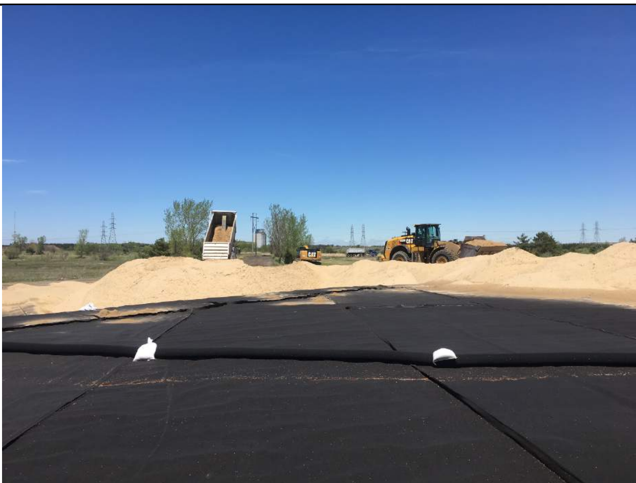
Placing and receiving cover materials in the northwest corner of Pond A.
