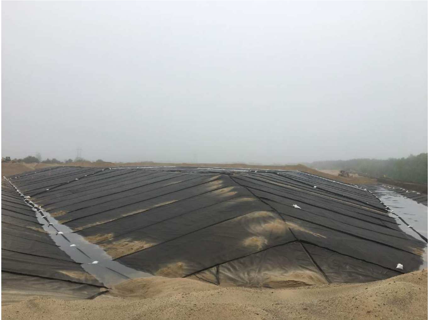
Placing and grading cover material.
