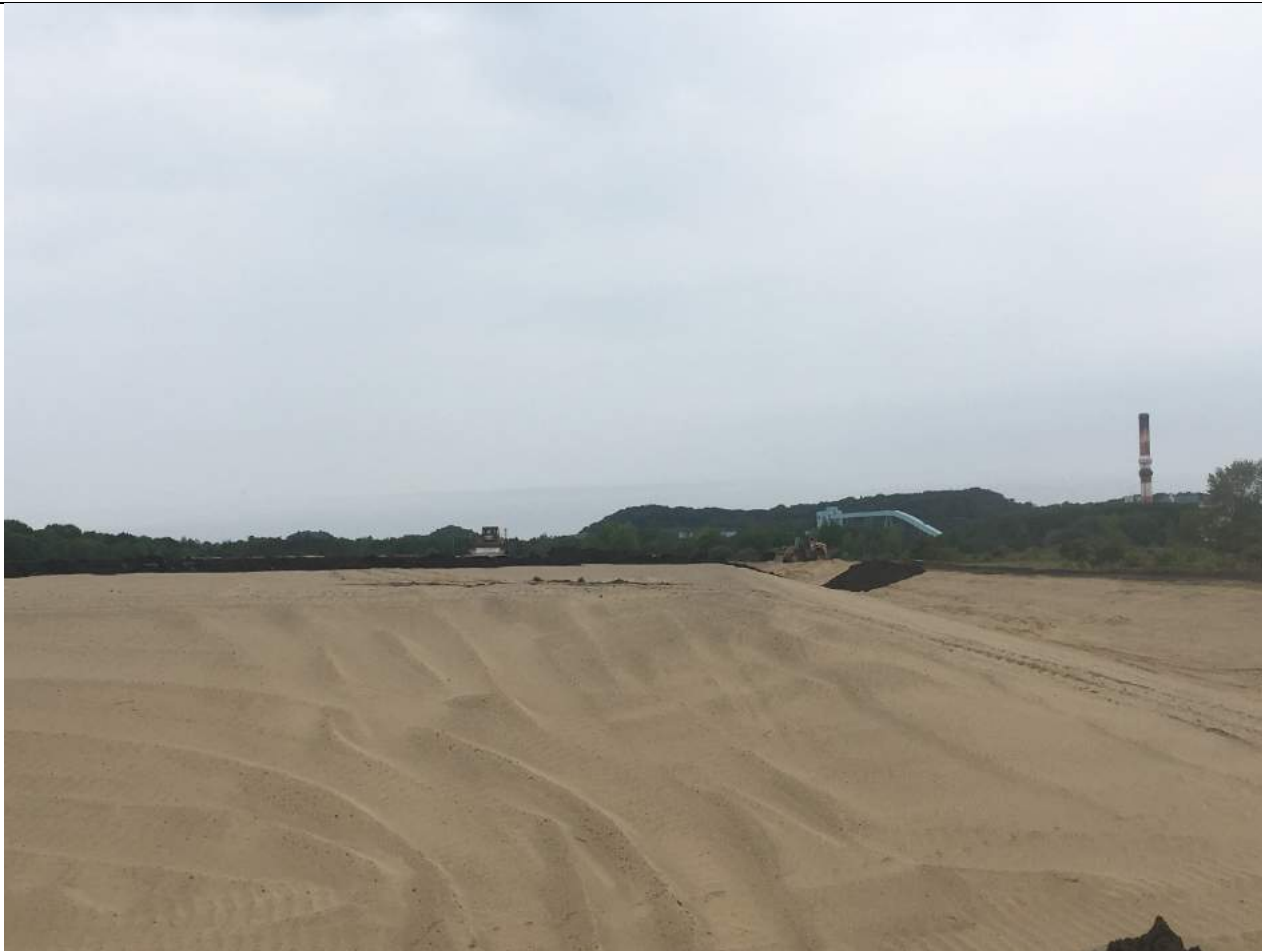
Dozer grading cover material of Pond A.
