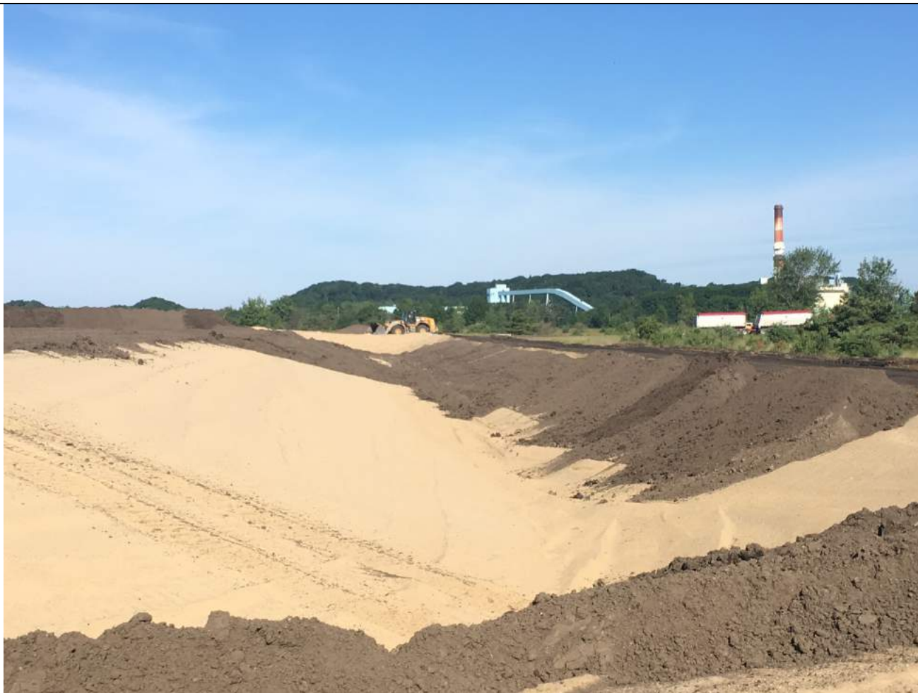
Delivery and grading of topsoil.
