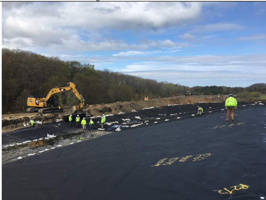
Placing and sewing seams of geotextile in the southwest corner of Pond A.
