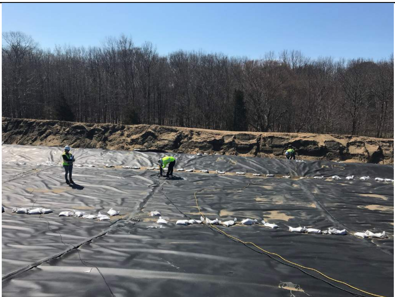
Extrusion welding repairs.
