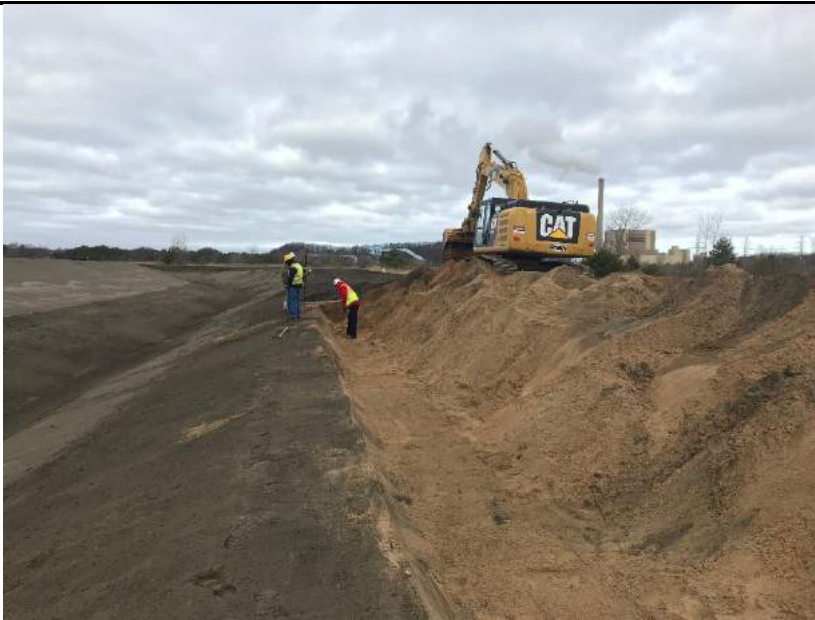
Anchor trench along the north side of Pond A.
