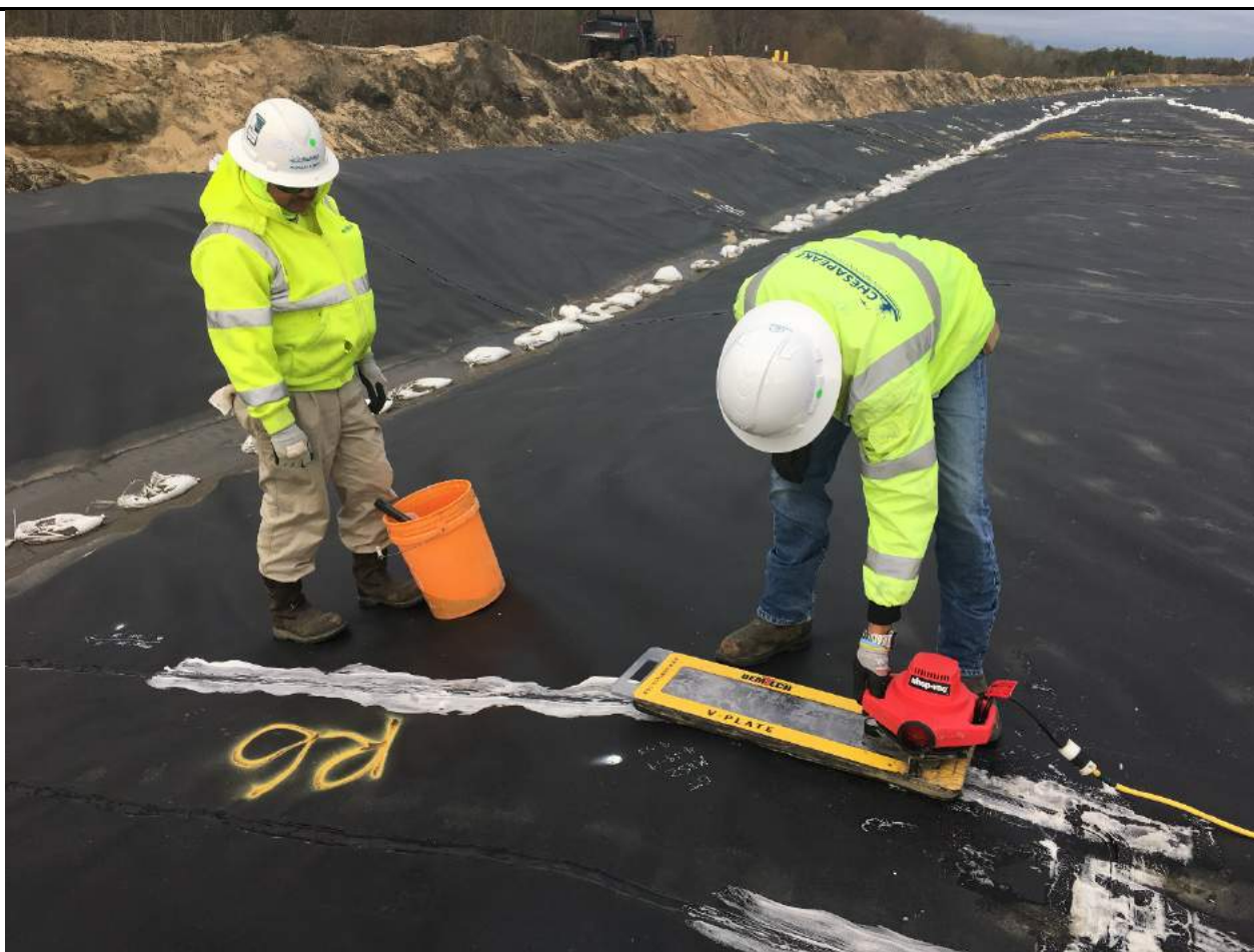
Vacuum testing of repairs.
