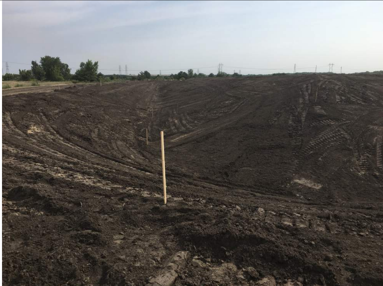
Graded of topsoil at the west end of Pond A.
