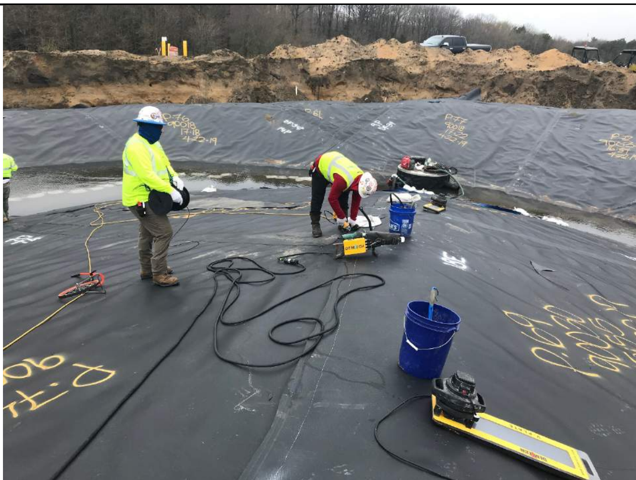
Extrusion welding repairs.
