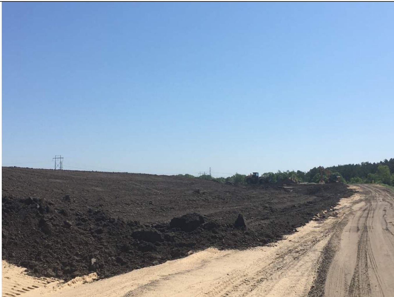
Delivery and grading of topsoil.
