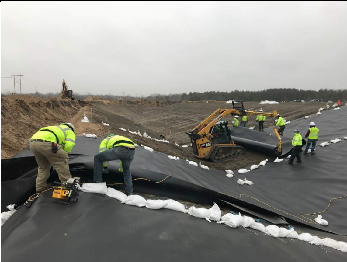
Fusion seam and deploying geomembrane.
