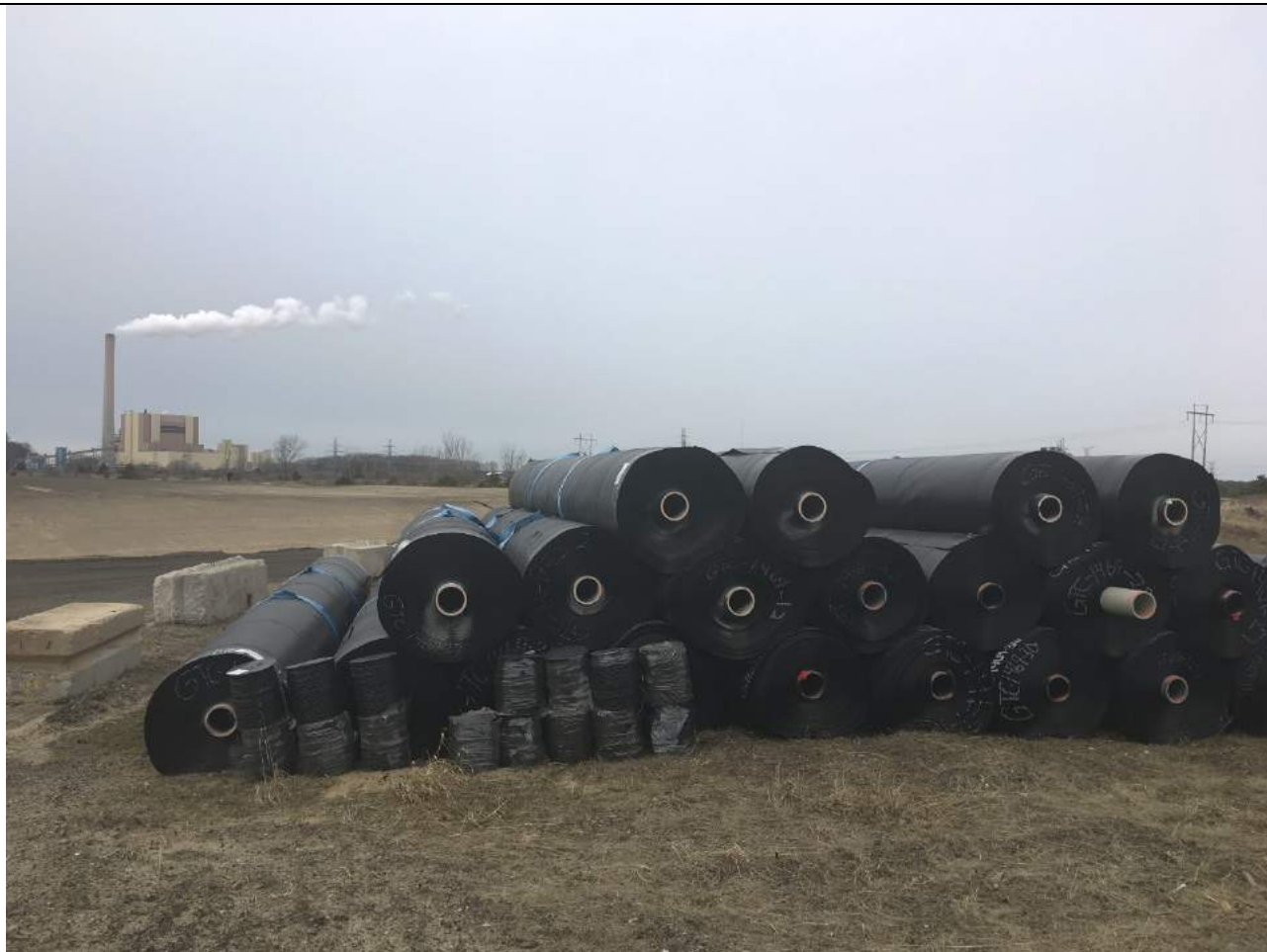
Stockpiled Geosynthetic Material for Pond A.
