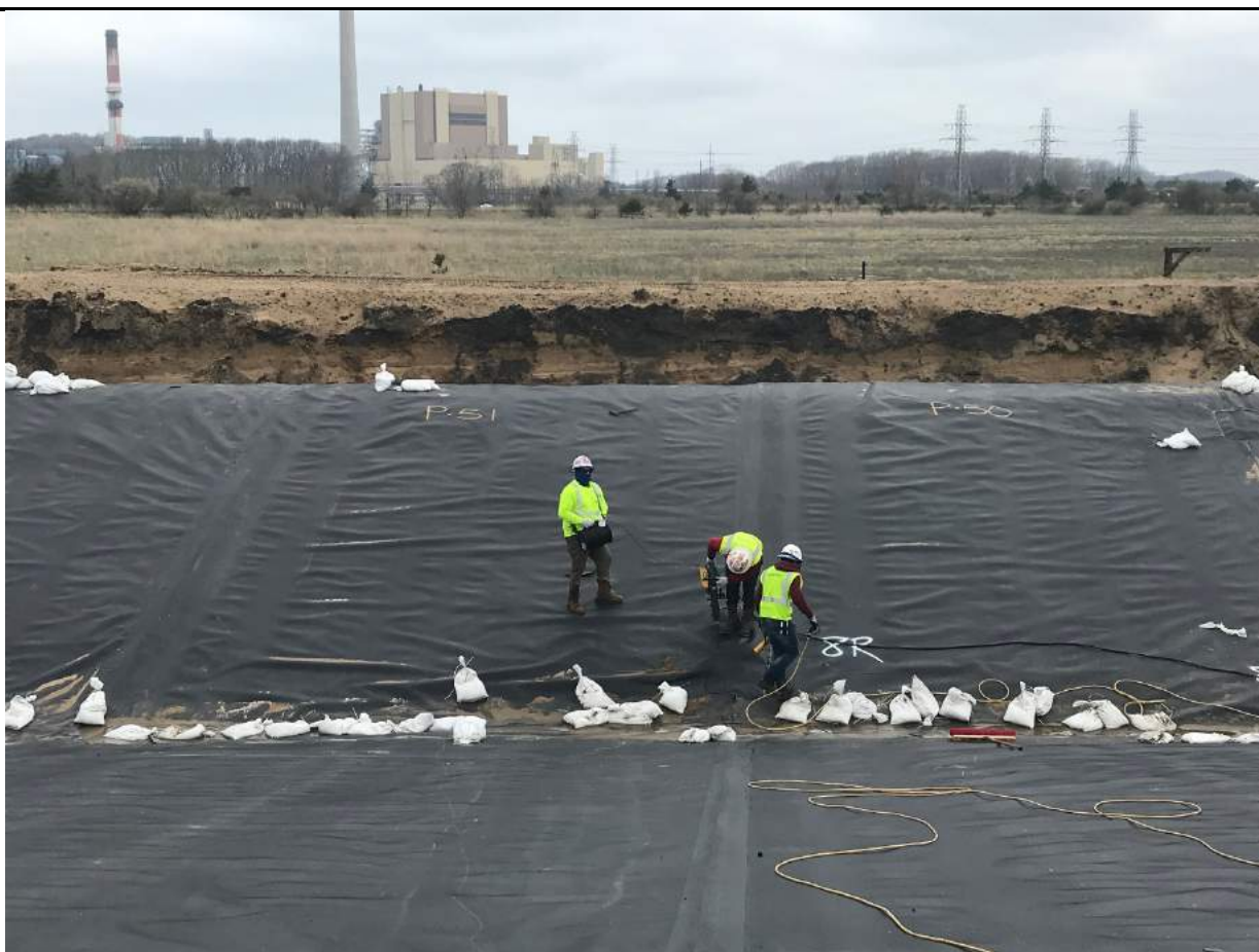
Extrusion welding repairs.
