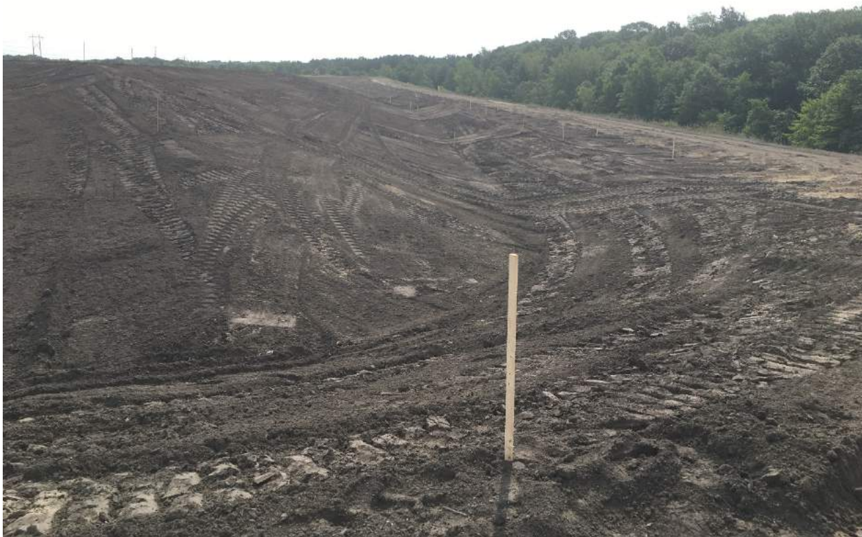
Graded topsoil on the south side of Pond A.
