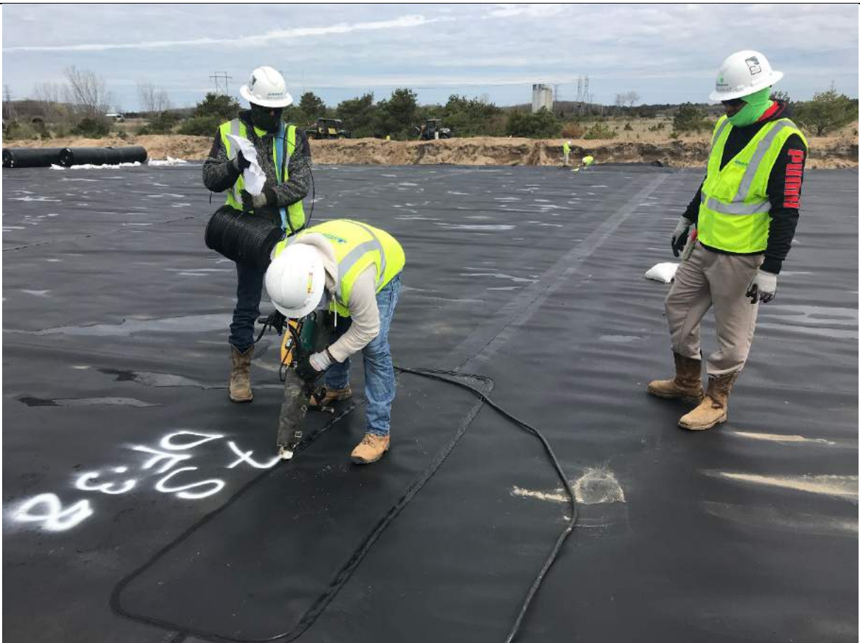
Performing extrusion welding of repairs.
