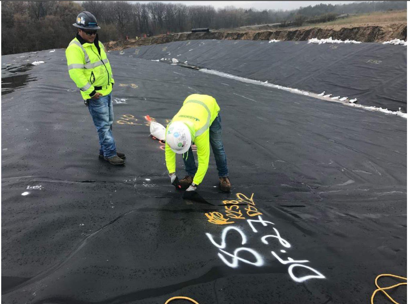
Pulling extrusion destruct DX-6P
