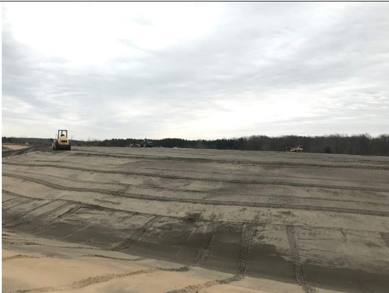
Dozer and drum roller repairing subgrade.
