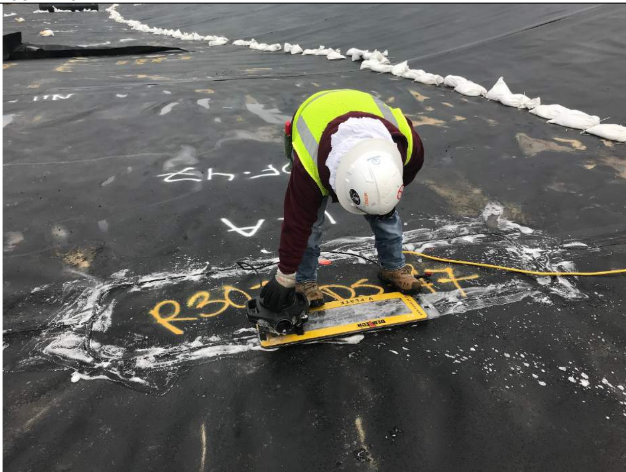
Vacuum testing repairs.
