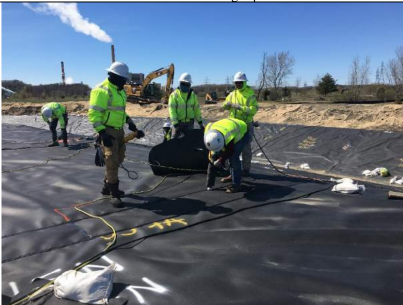
Extrusion welding caps.
