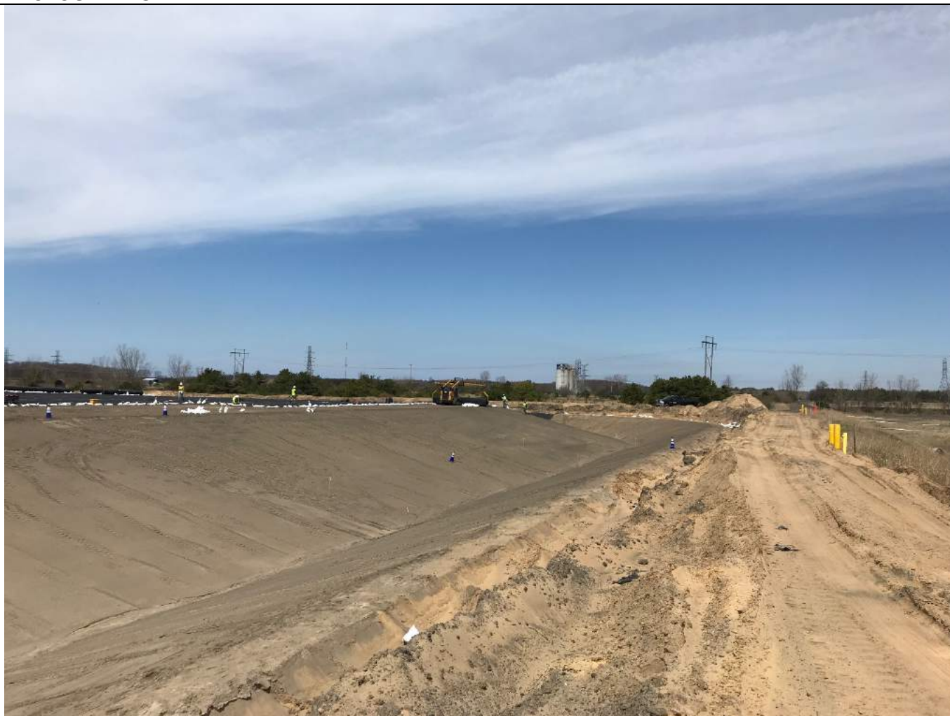
Deploying geosynthetics along the northeast corner of Pond A.
