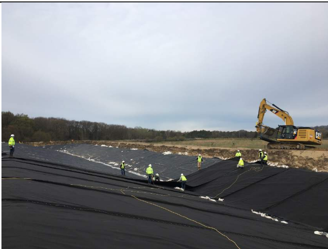
Placing and sowing seams of textile on the west end of Pond A.
