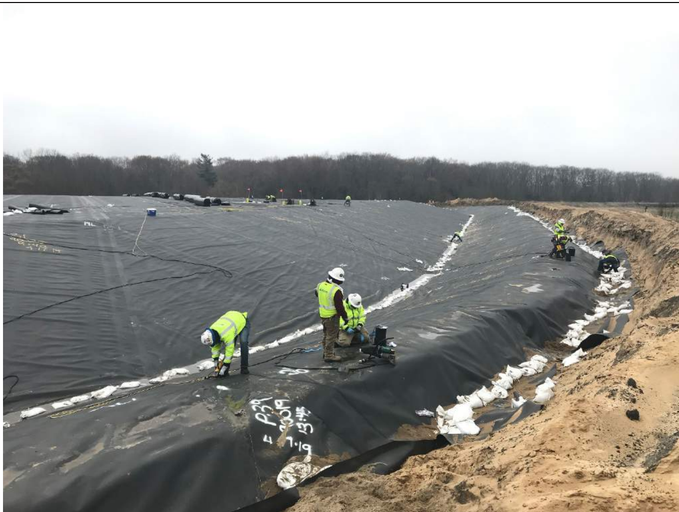
Extrusion welding of repairs.
