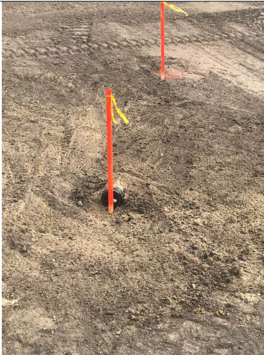
Installed screens on the drain tile.
