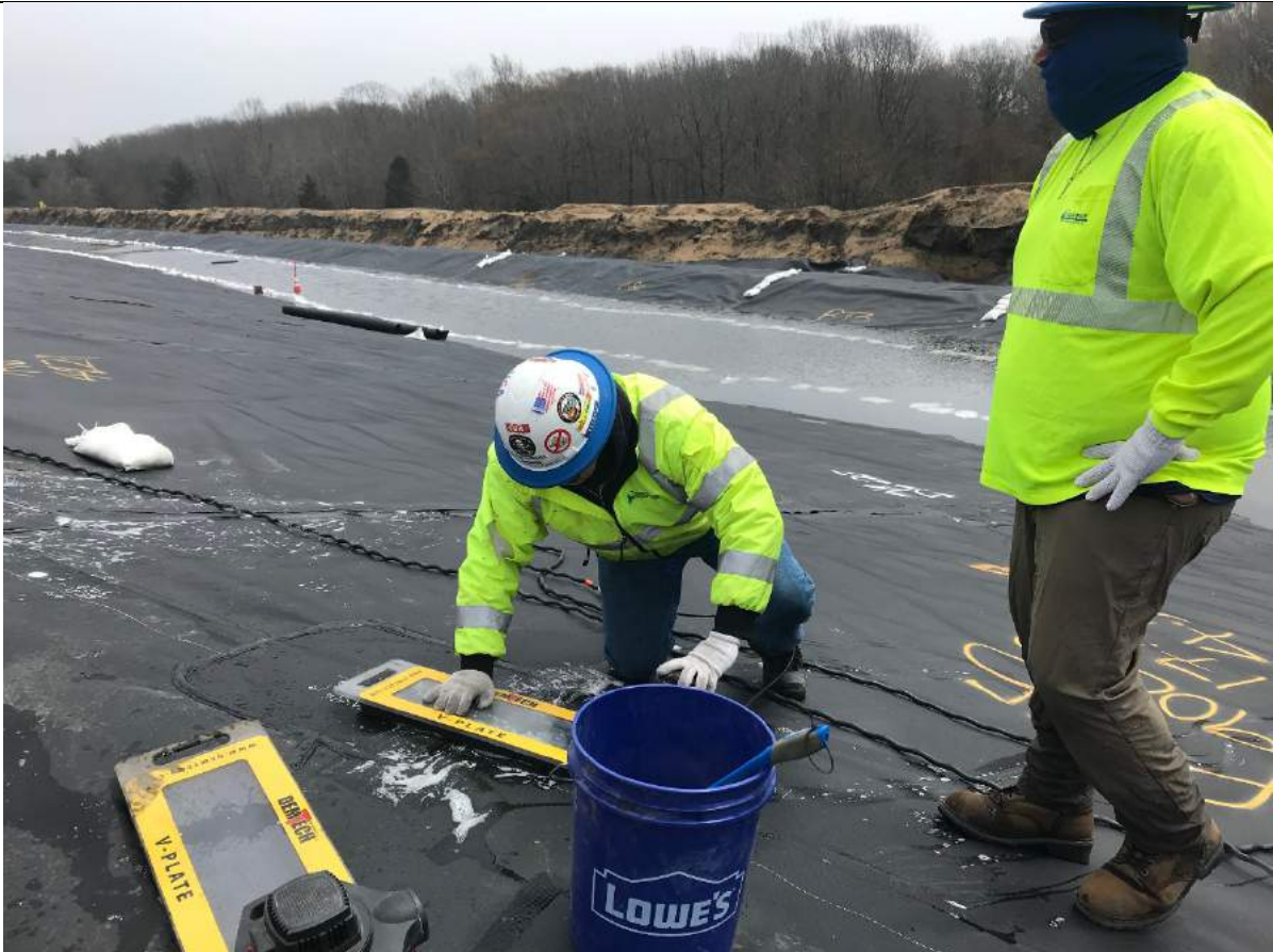
Welding repair around western stormwater drain.
