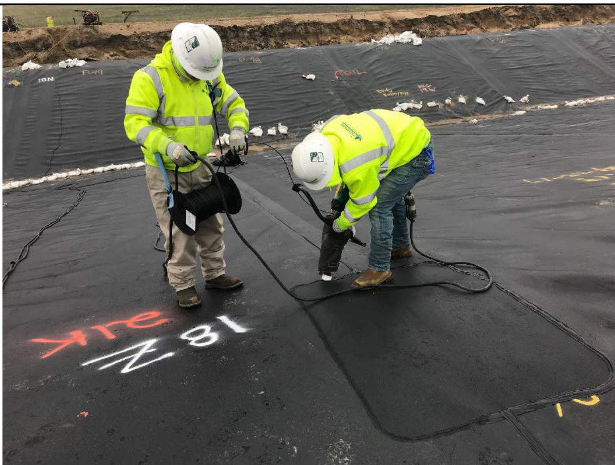
Extrusion welding repairs.
