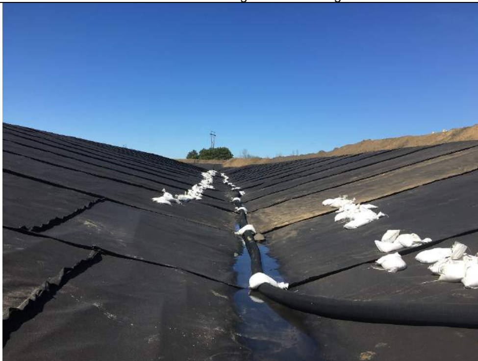
Installed 6-inch drainage tile.
