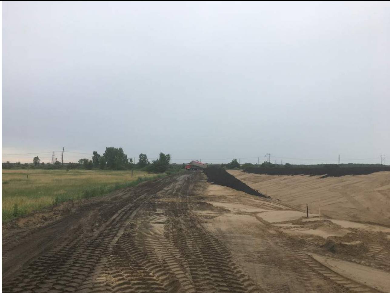
Receiving topsoil at the west end of Pond A.
