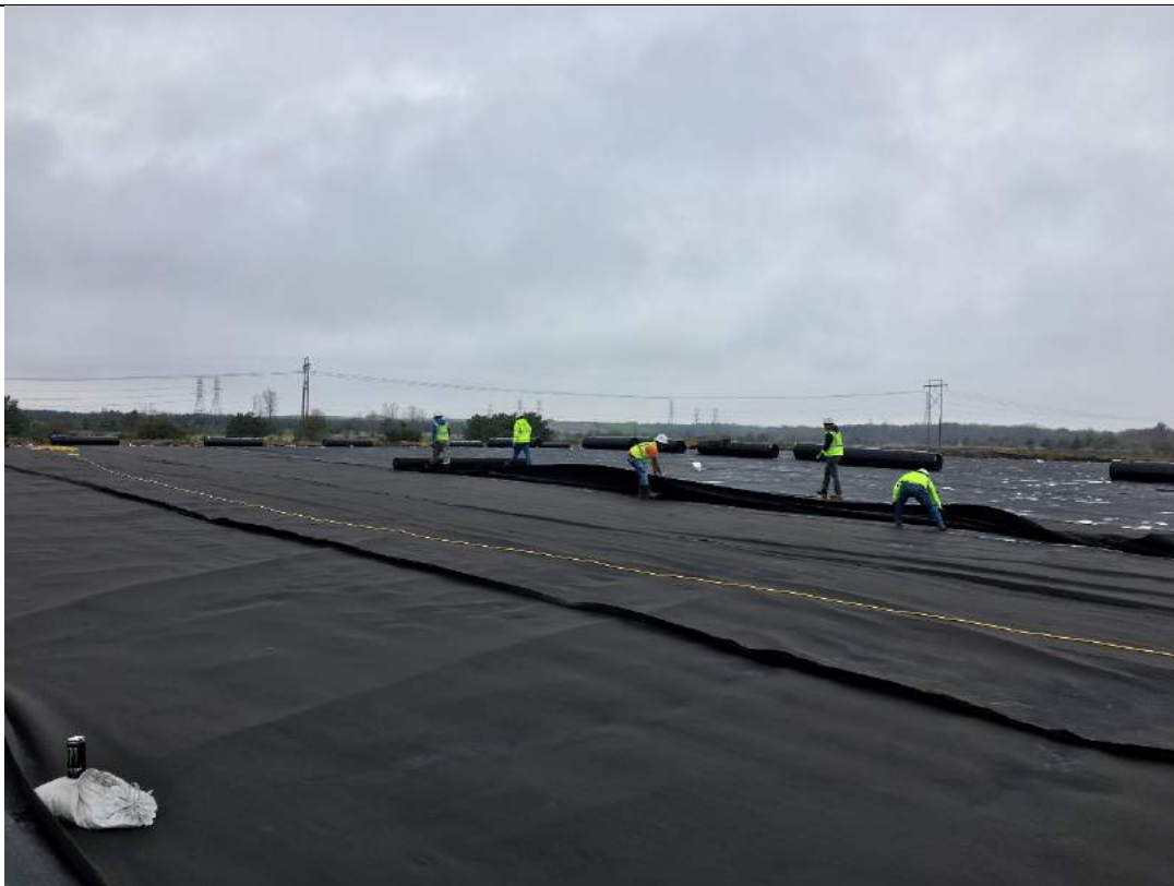
Deploying and sowing geotextile.
