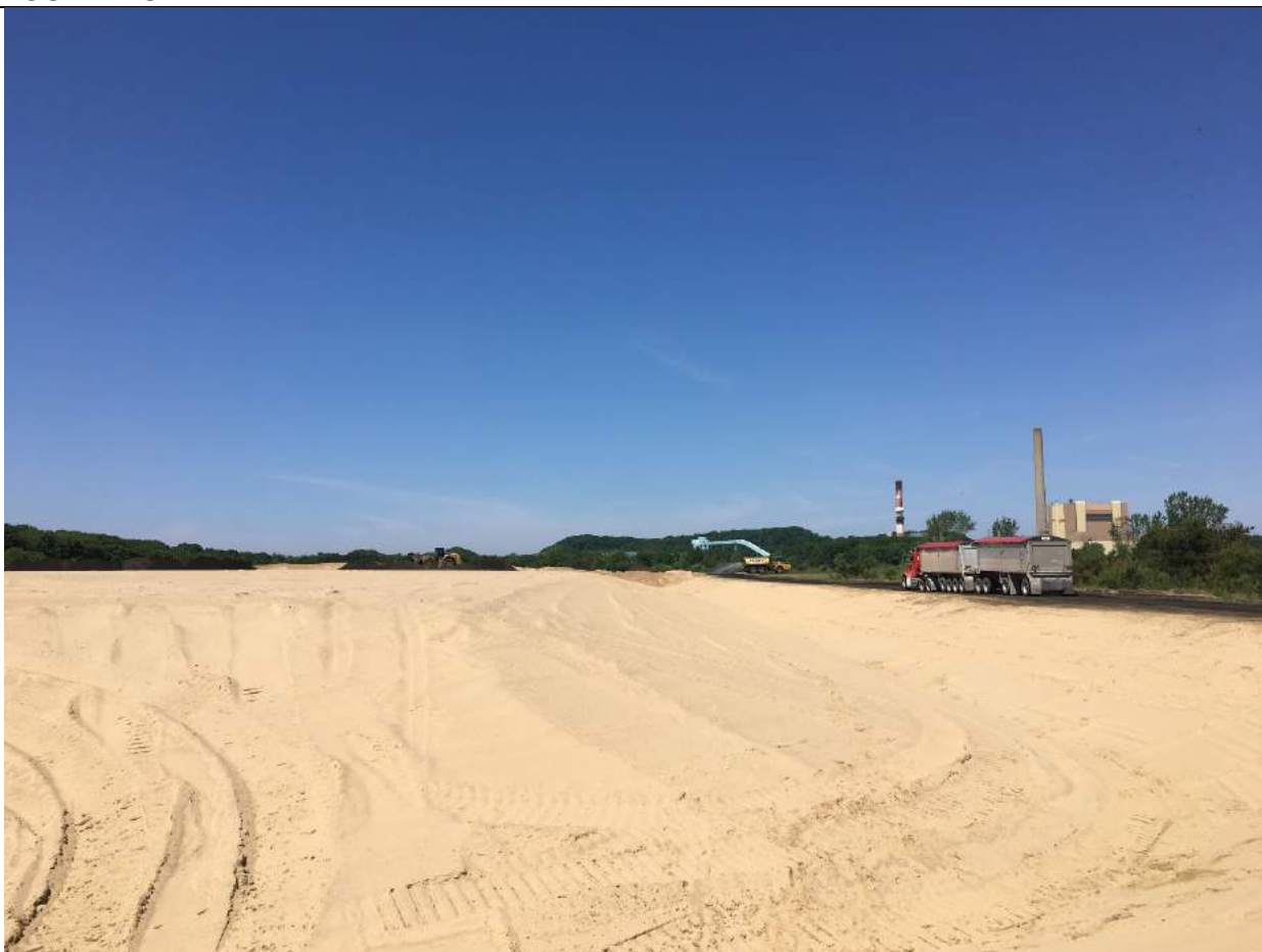
Placing and grading topsoil.
