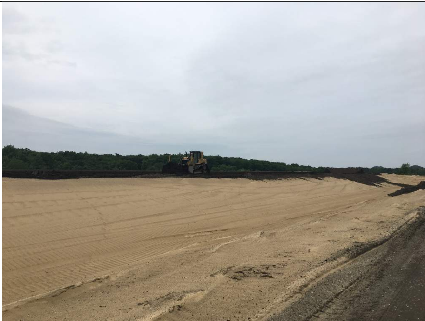
Delivery and grading of topsoil.
