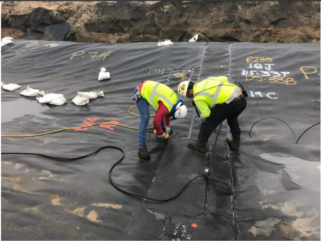
Extrusion welding repairs
