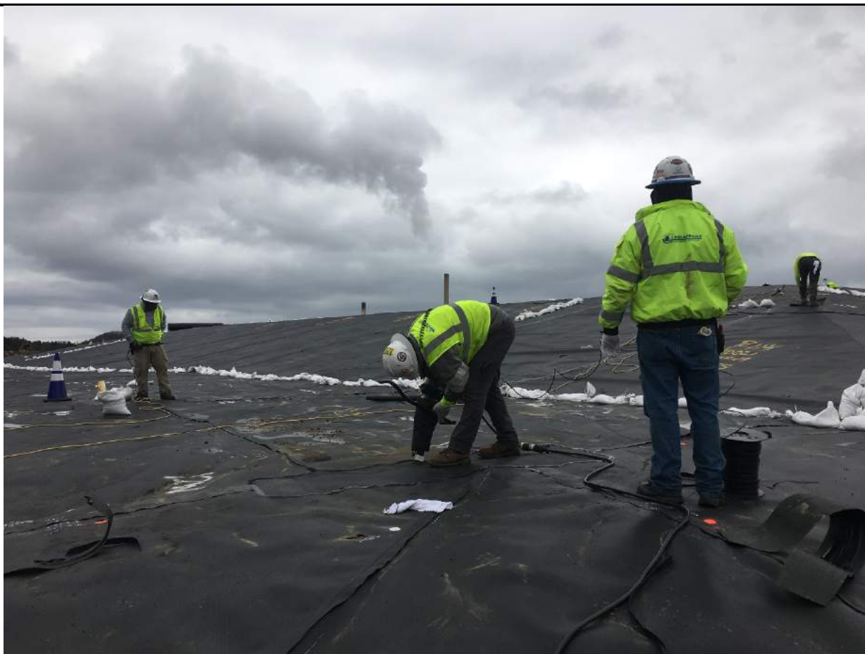
Extrusion welding repairs.
