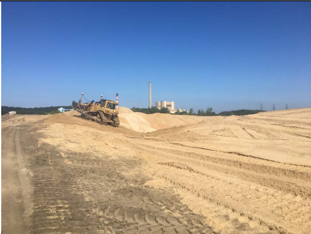
Dozer preparing subgrade at the west end of Pond A.
