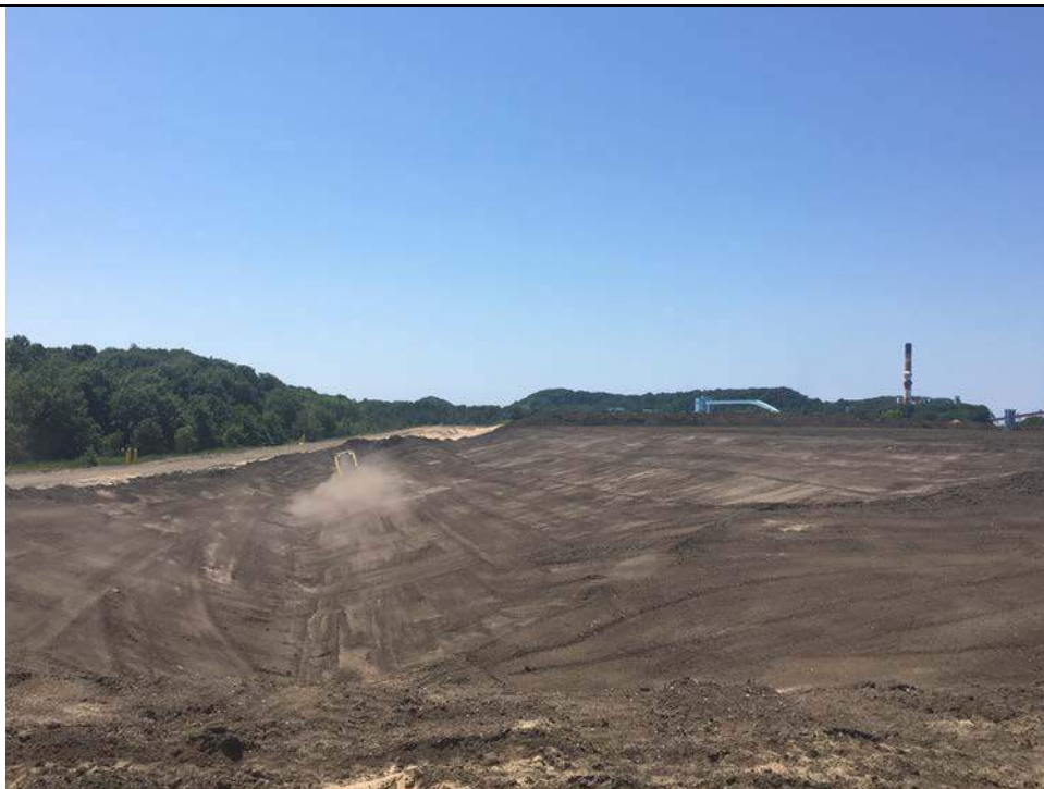
Grading cover material.
