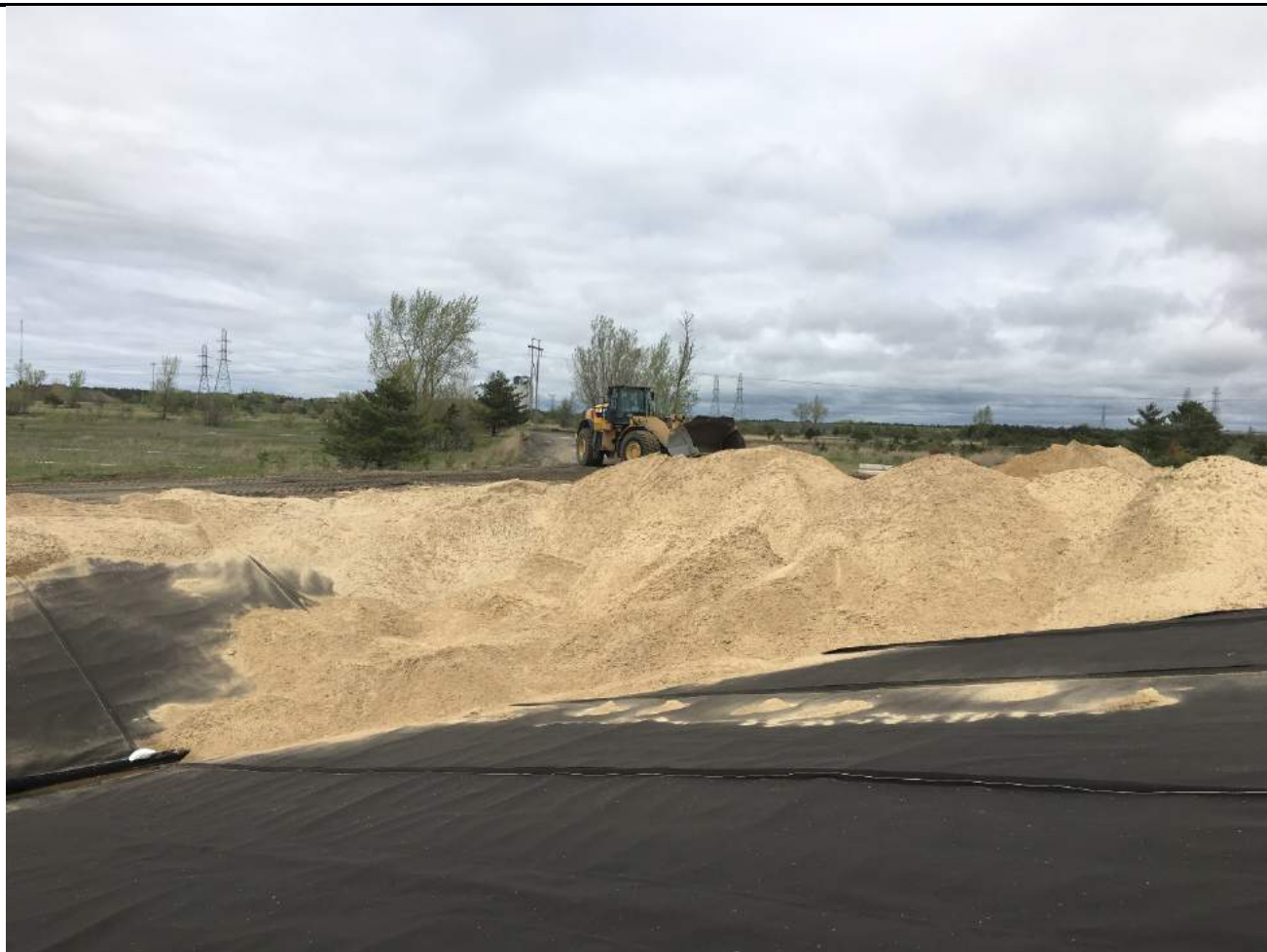
Building bridge of cover materials in the northwest corner of Pond A.
