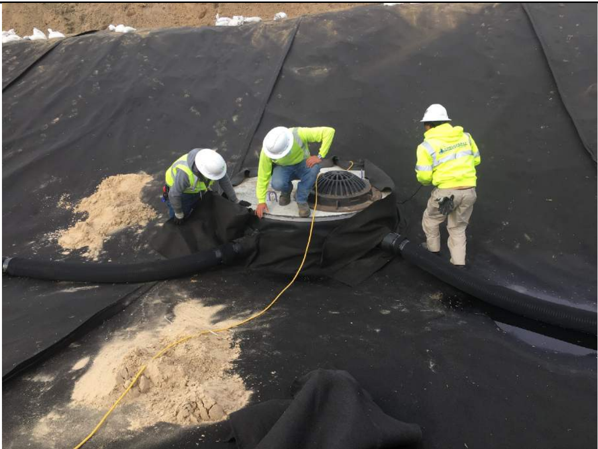
Wrapping western stormwater manhole in geotextile.
