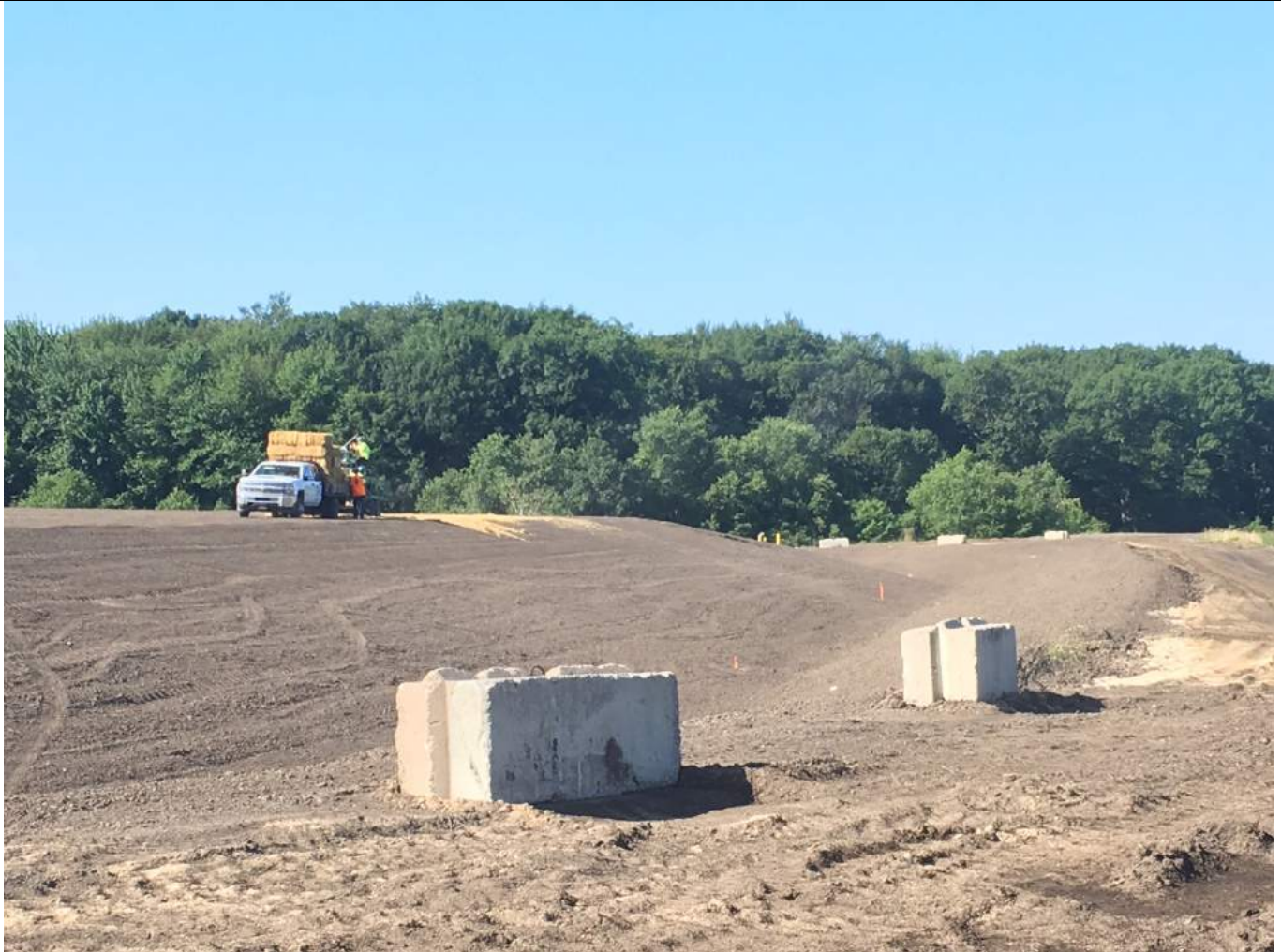
Placing straw over seeded topsoil at Pond A.
