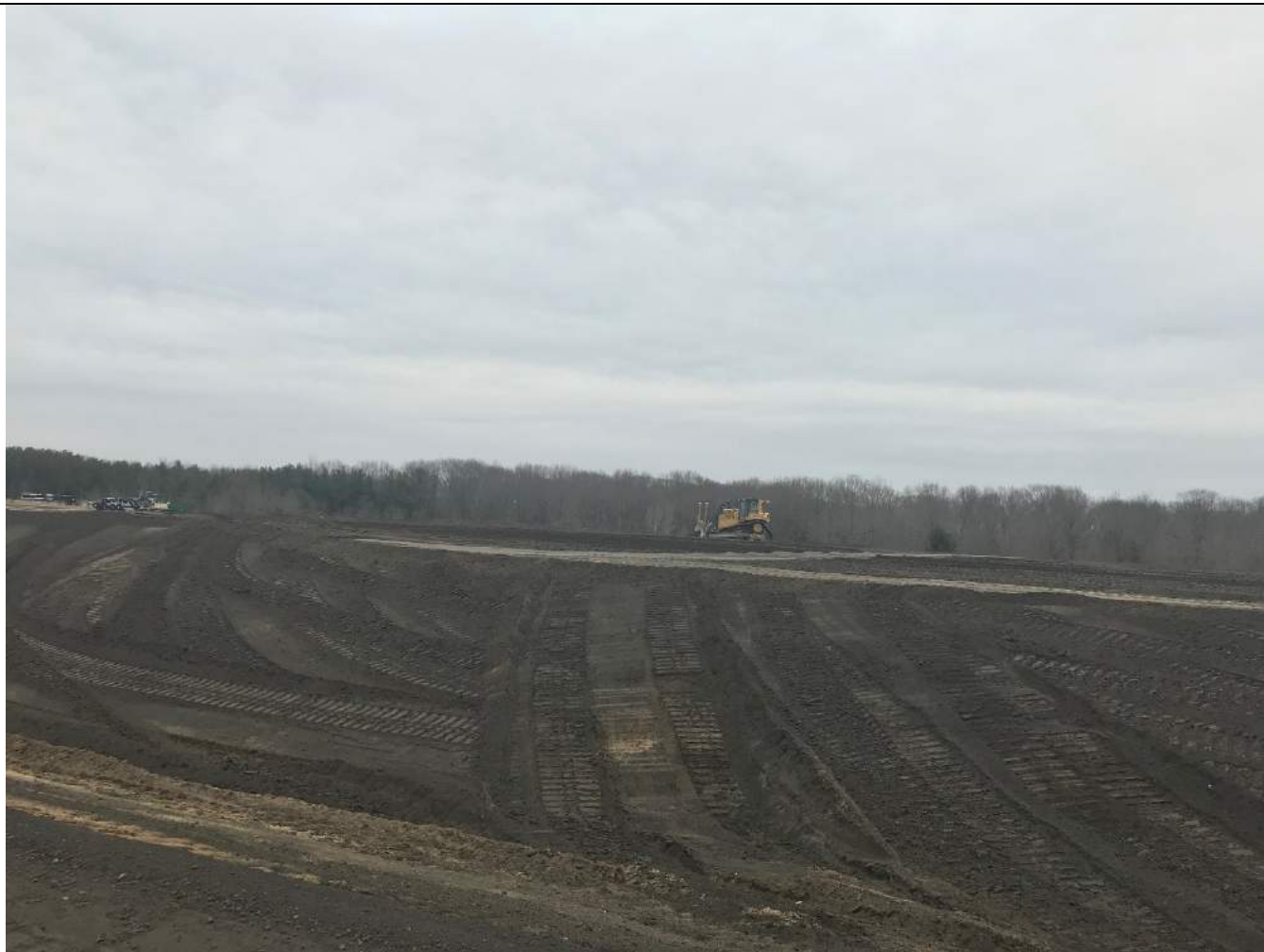
Dozer repairing subgrade.
