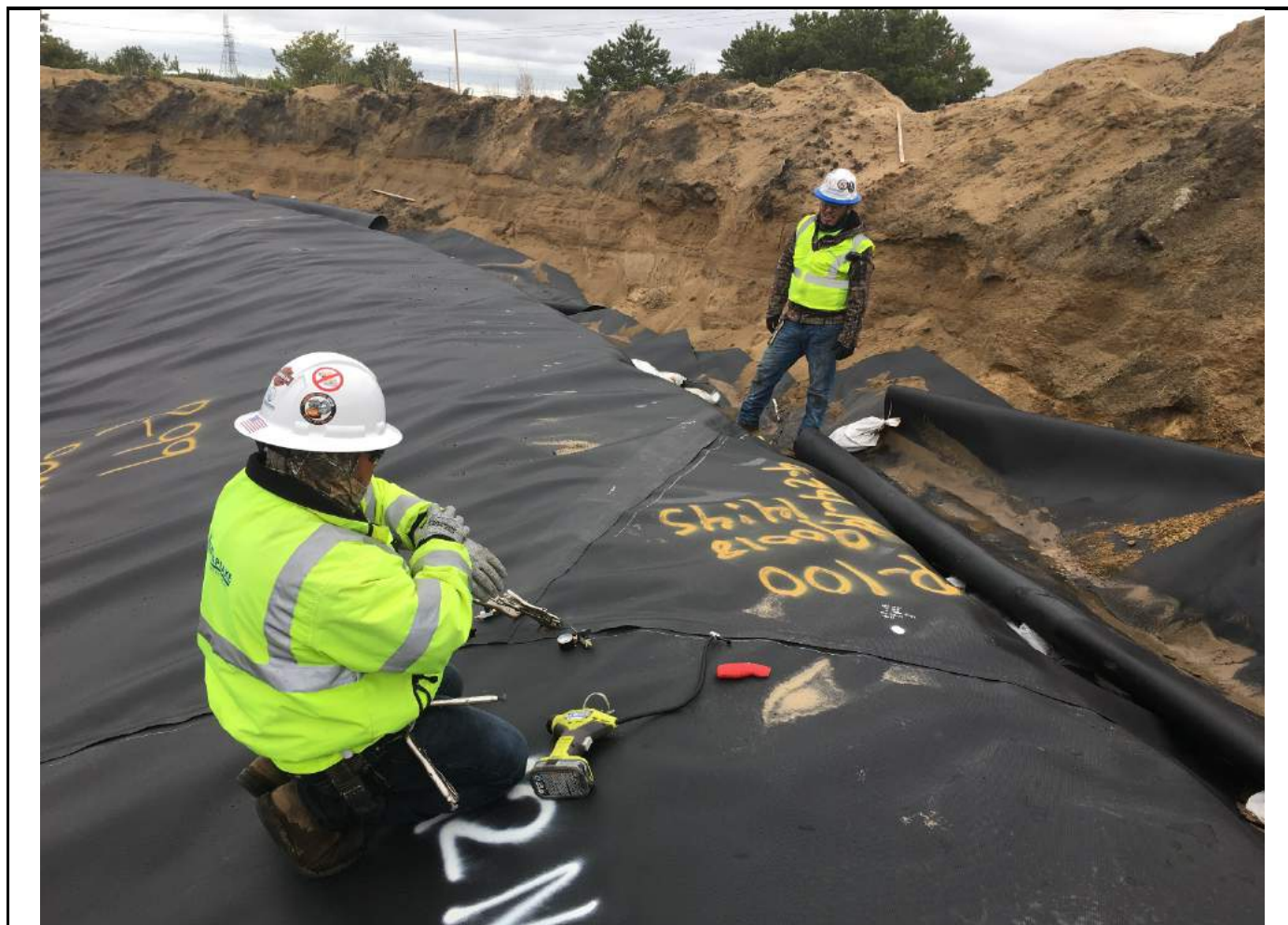
Pressure testing seams.
