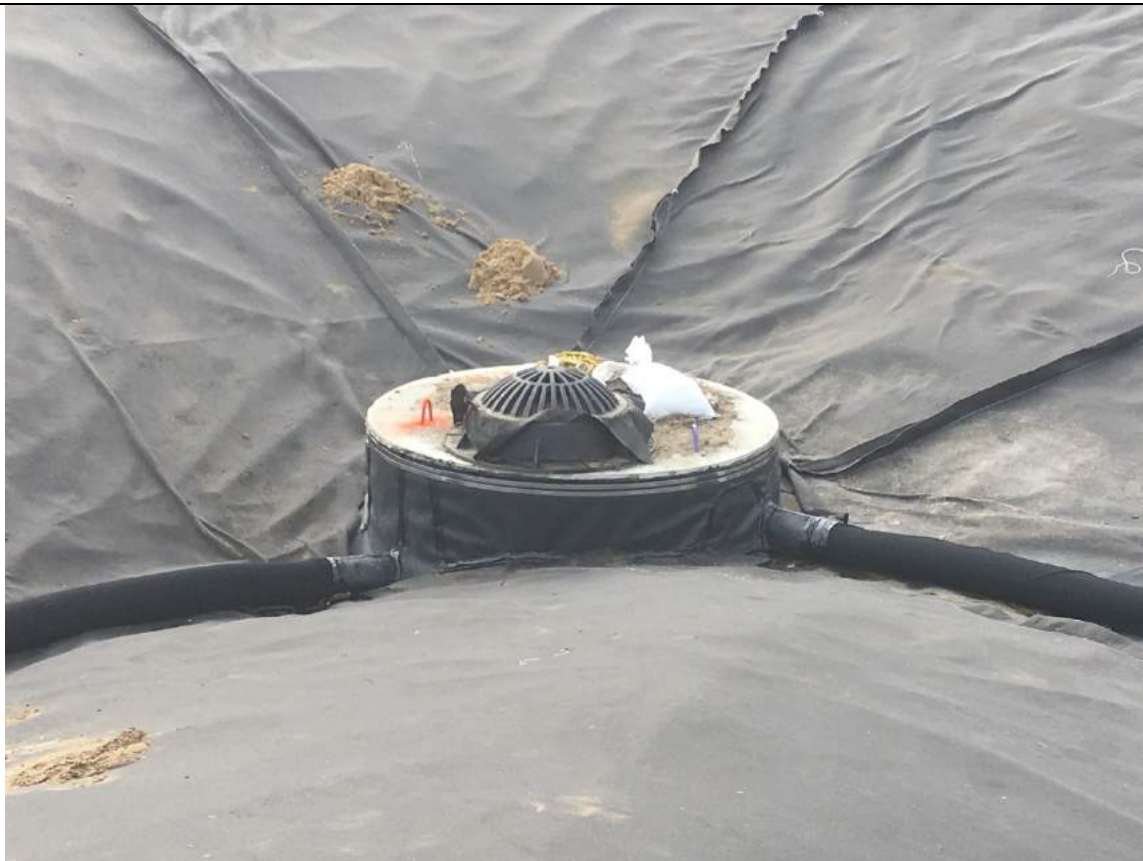
Eastern stormwater manhole without 6-inch drainage tile connected.
