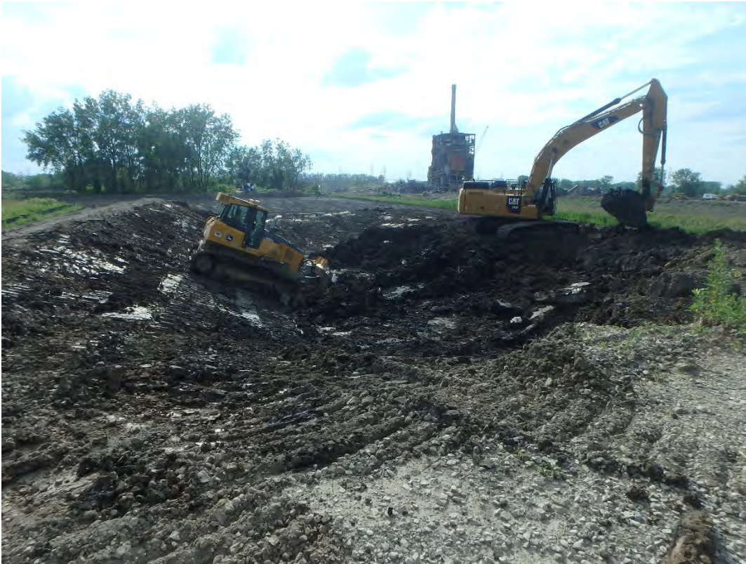
Removing residuals and cutting slopes down to clean sub-grade, Looking west.
