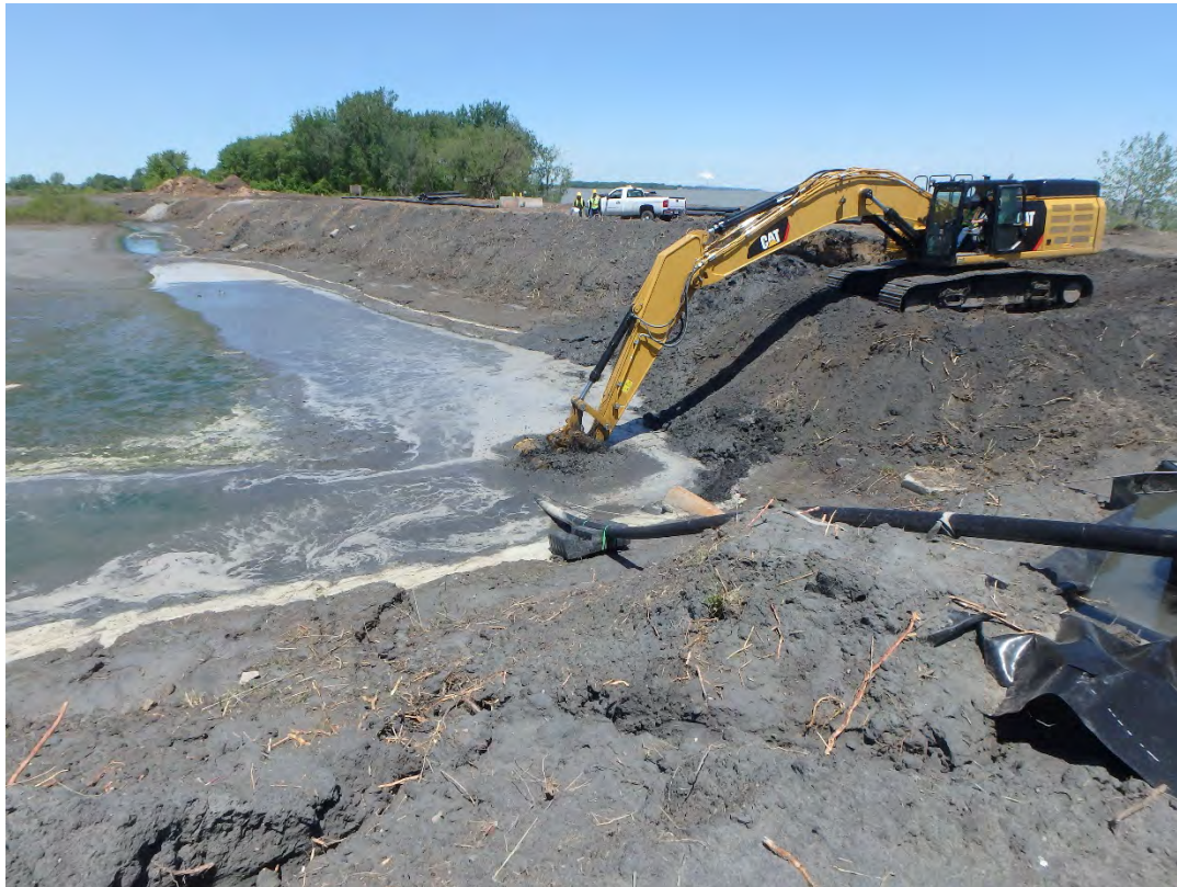
Excavating Sump in southeast corner of Pond 2
