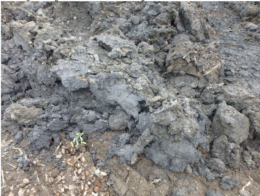
Screening cleared/grubbed material to remove organics
