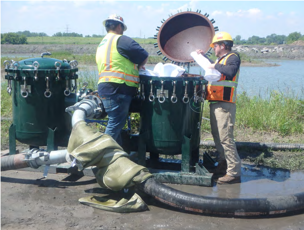
ProAct changing filters during dewatering of Pond 2, looking north.
