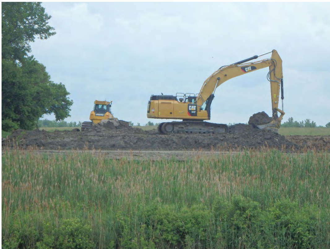
Removing structural fill from berm of Chemical Pond B, looking south.
