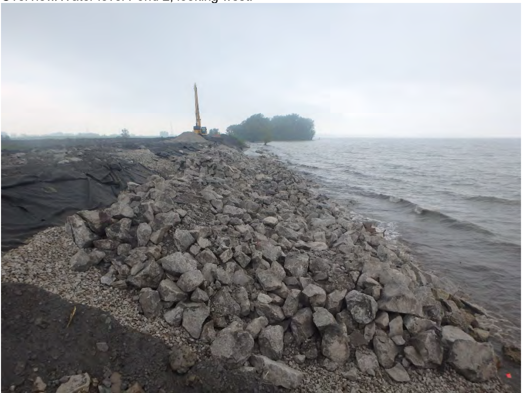
Southern end of shoreline, looking north.
