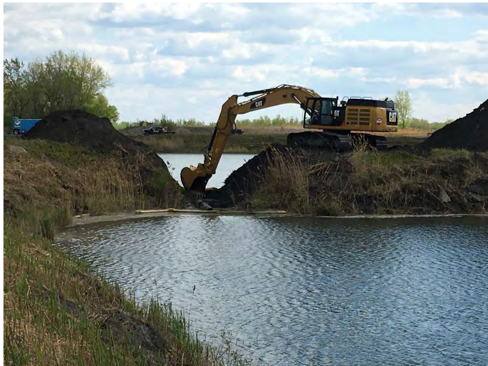
Ryan lowering culvert between Pond 1 and Pond 2.
