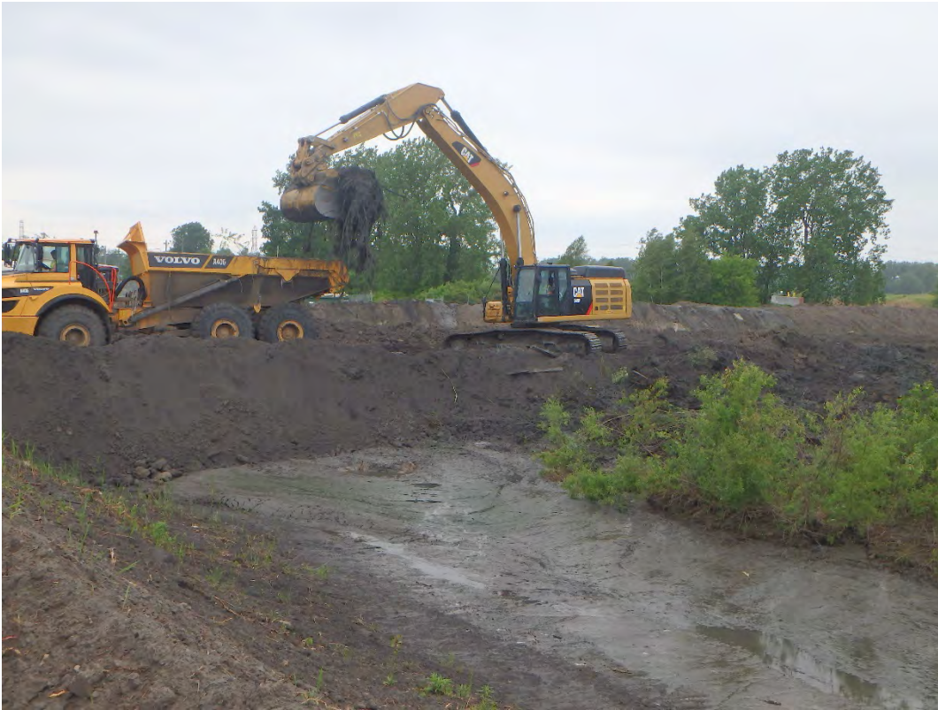
Clearing vegetation from Pond 1, looking west.
