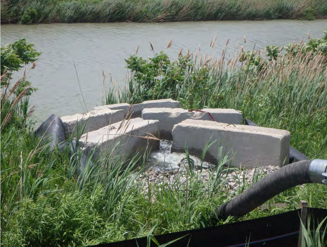
Discharge from dewatering of Pond 2 into discharge channel.
