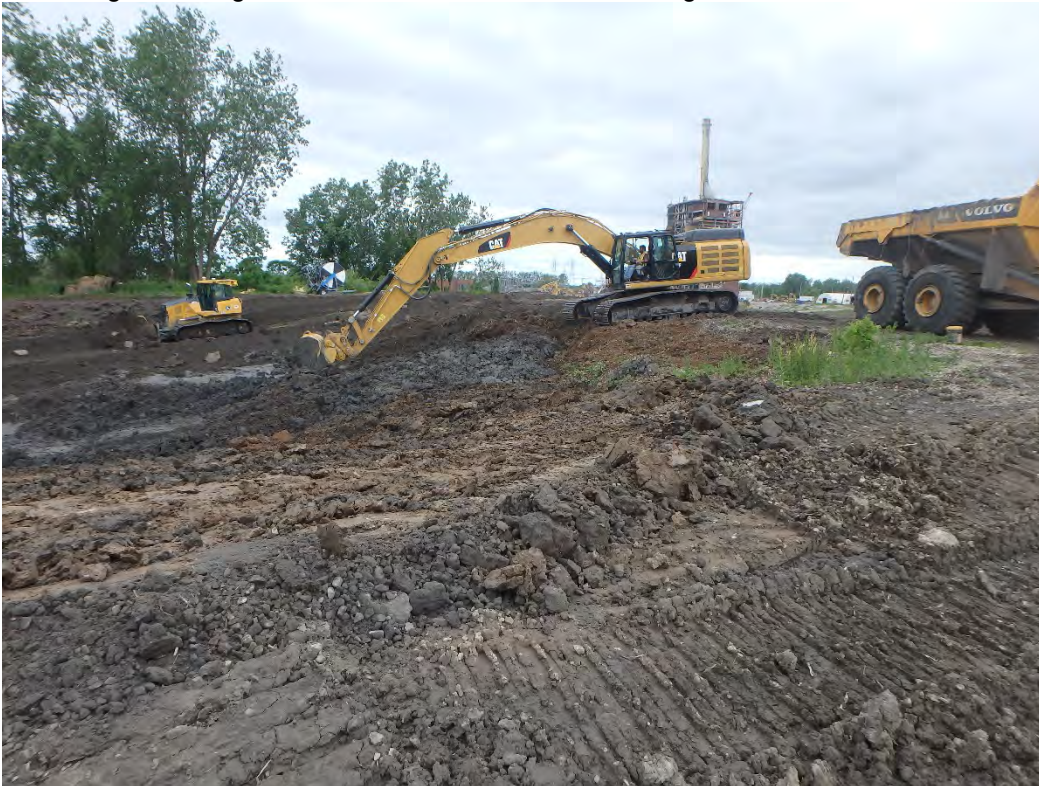
Loadout of residual from Chemical Pond A for transport to Pond 1, Looking West.
