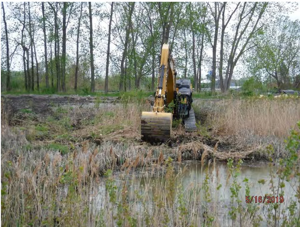
Chemical Pond A work to force water into northeast corner to enable dewatering into Chemical Pond B.
