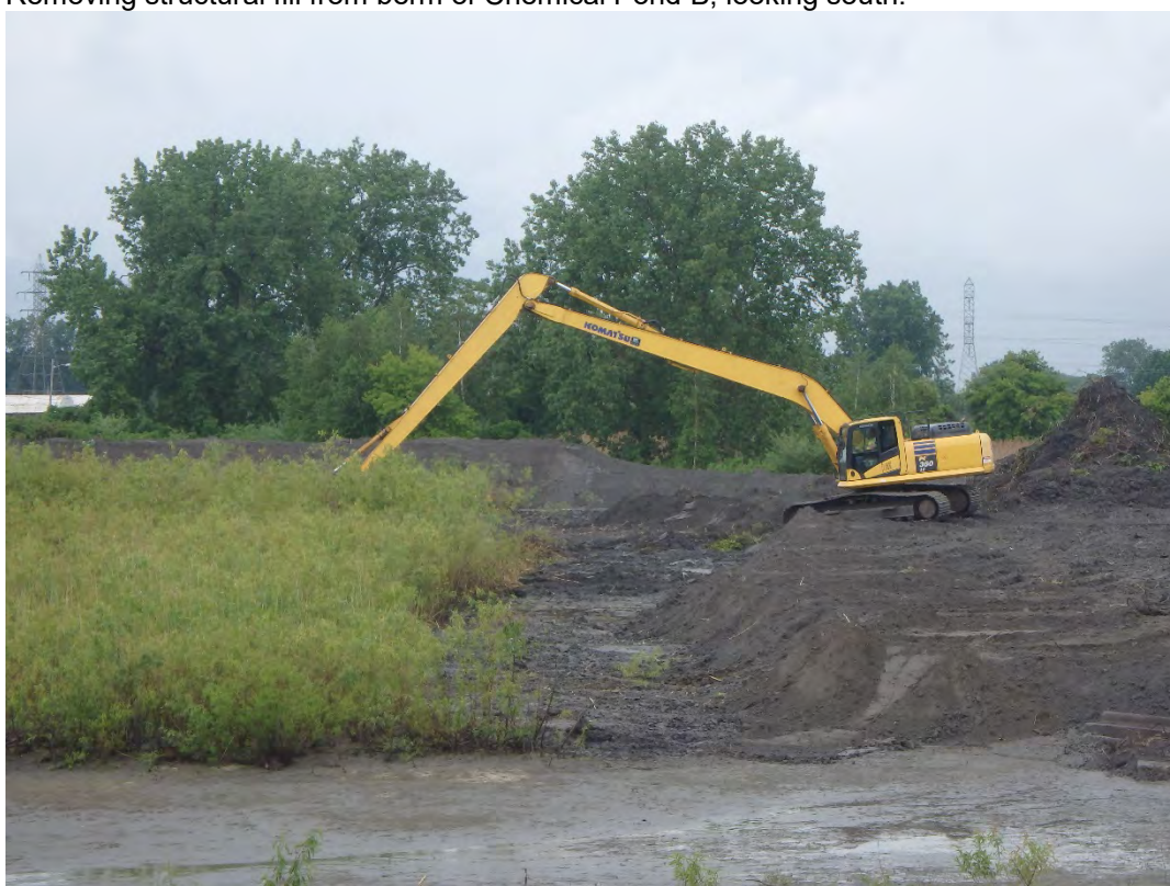
Removing vegetation from Pond 1, looking west.
