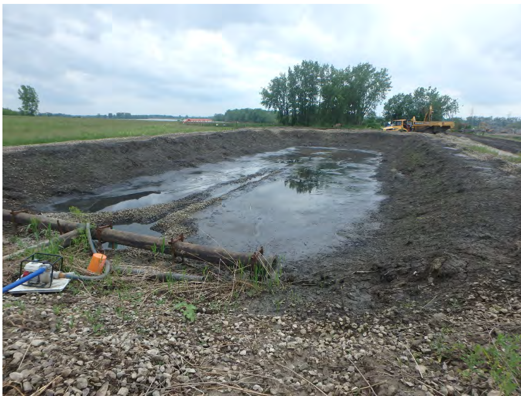
Water level in Chemical Pond B, Looking West
