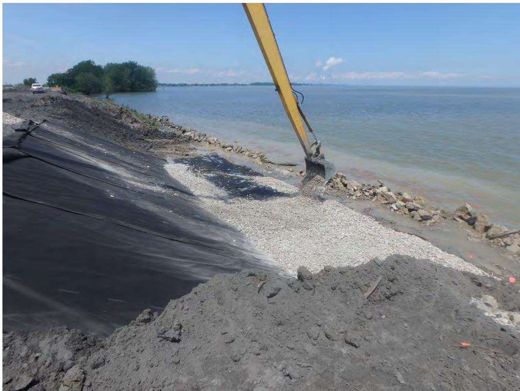
Placing D50-2 inch cushion layer, looking north.
