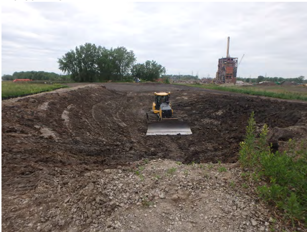
Cutting residual from Chemical Pond B, looking west.
