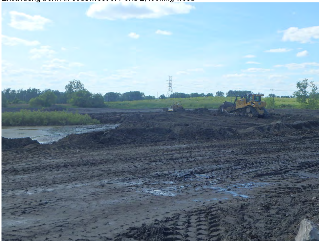
Placing bridging layer in Pond 1, looking northwest.
