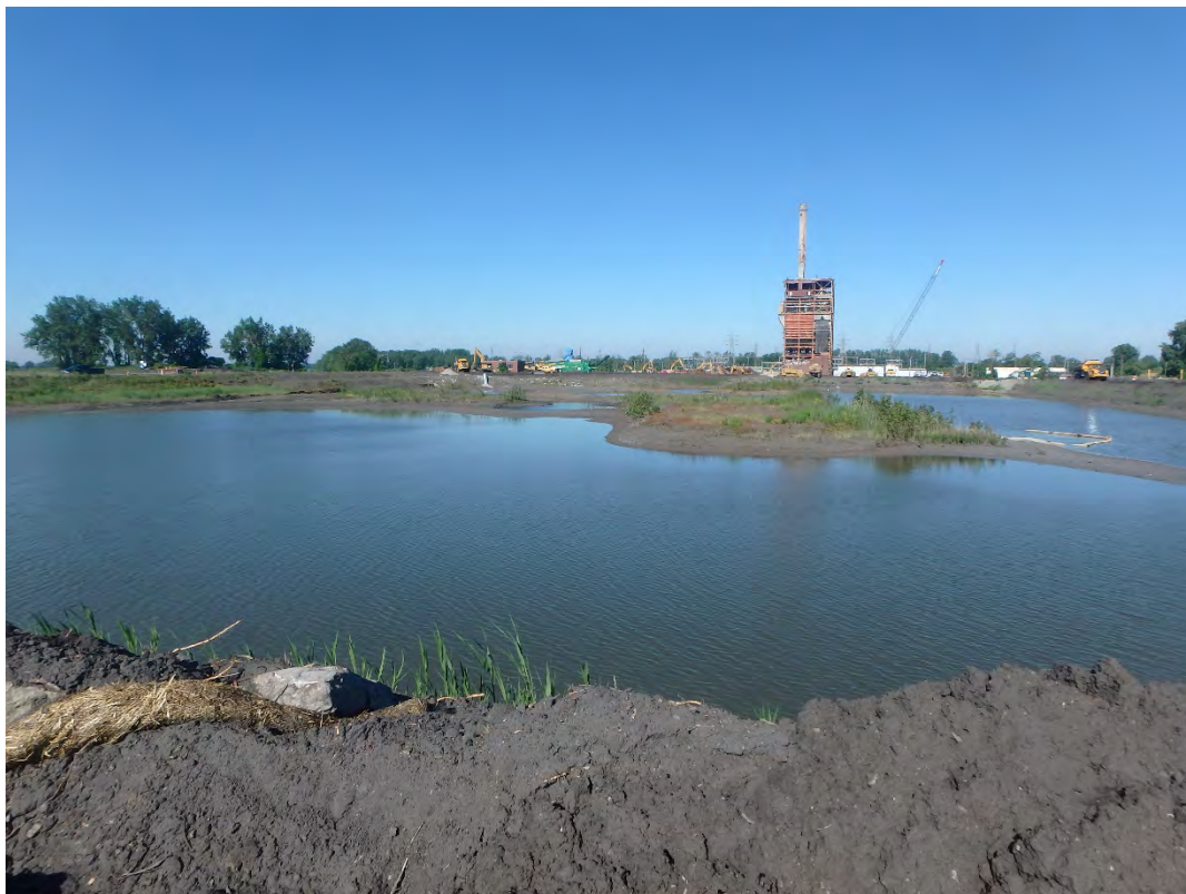
Overview / Water level of Pond 2, looking west.
