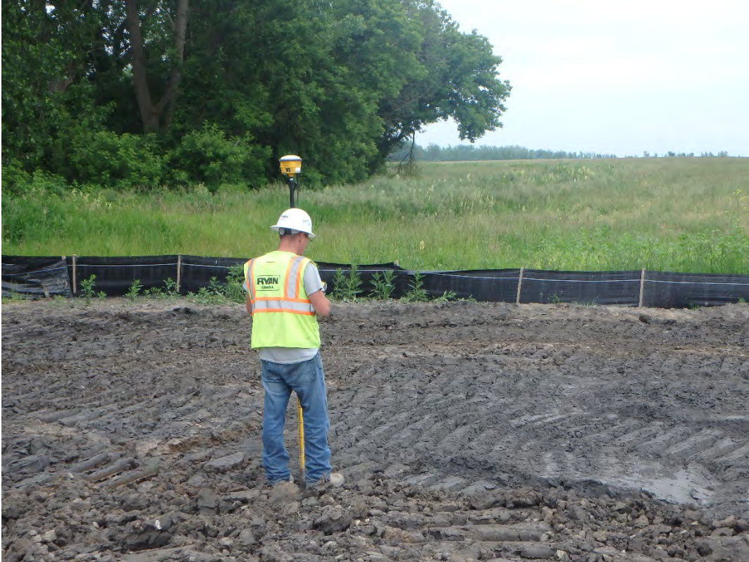
Checking grade at Chemical Pond B, looking south.
