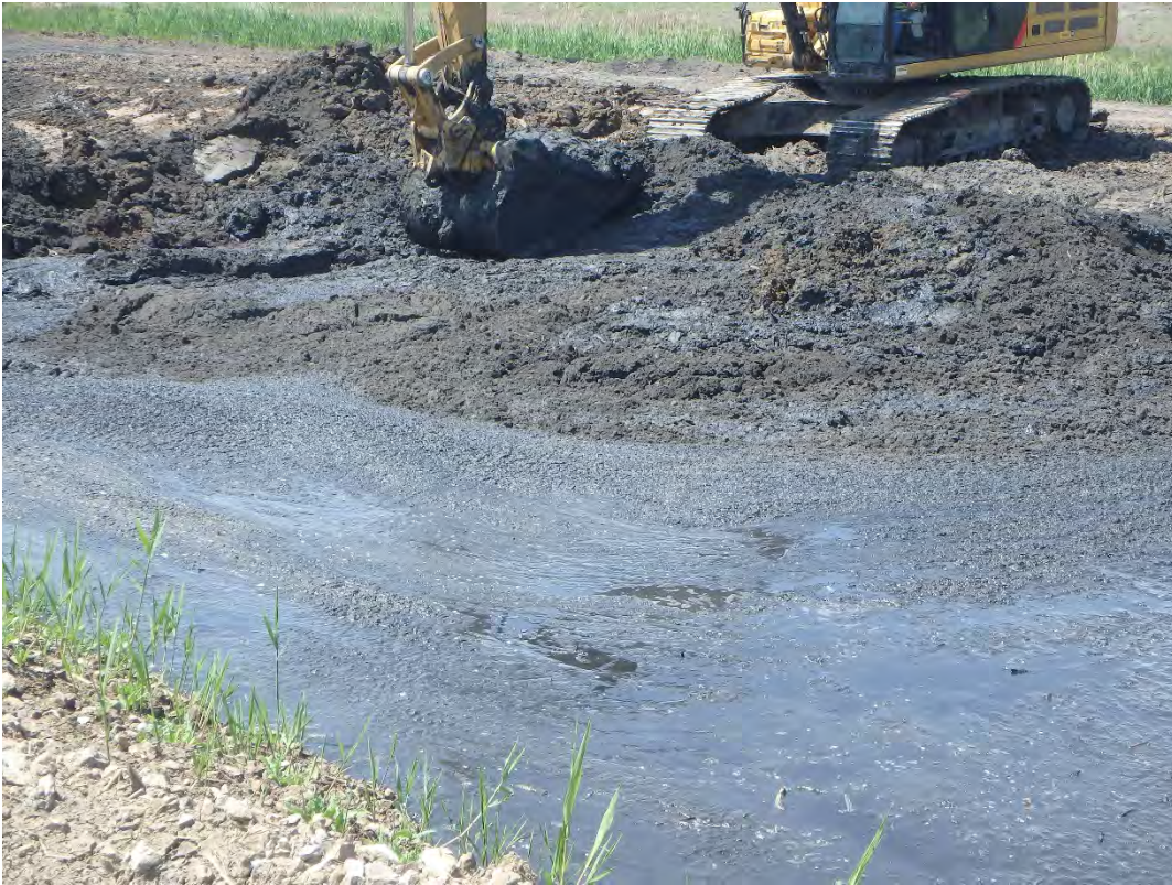
Mixing berm material with pond residuals to dry for transport to Pond 1, Looking north.
