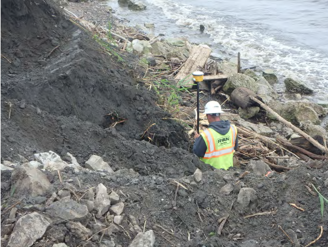
Checking grade in slope cut, looking northeast.
