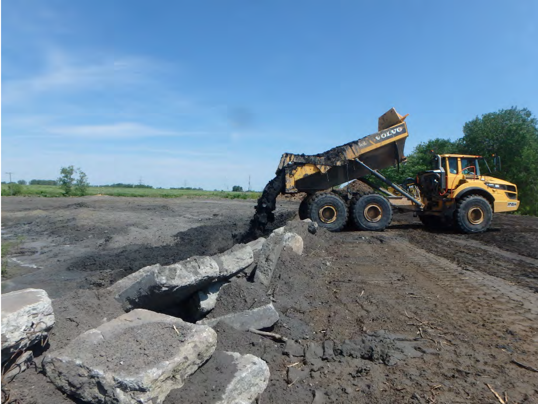
Placing Chemical Pond B residual material into Pond 1, Looking north.
