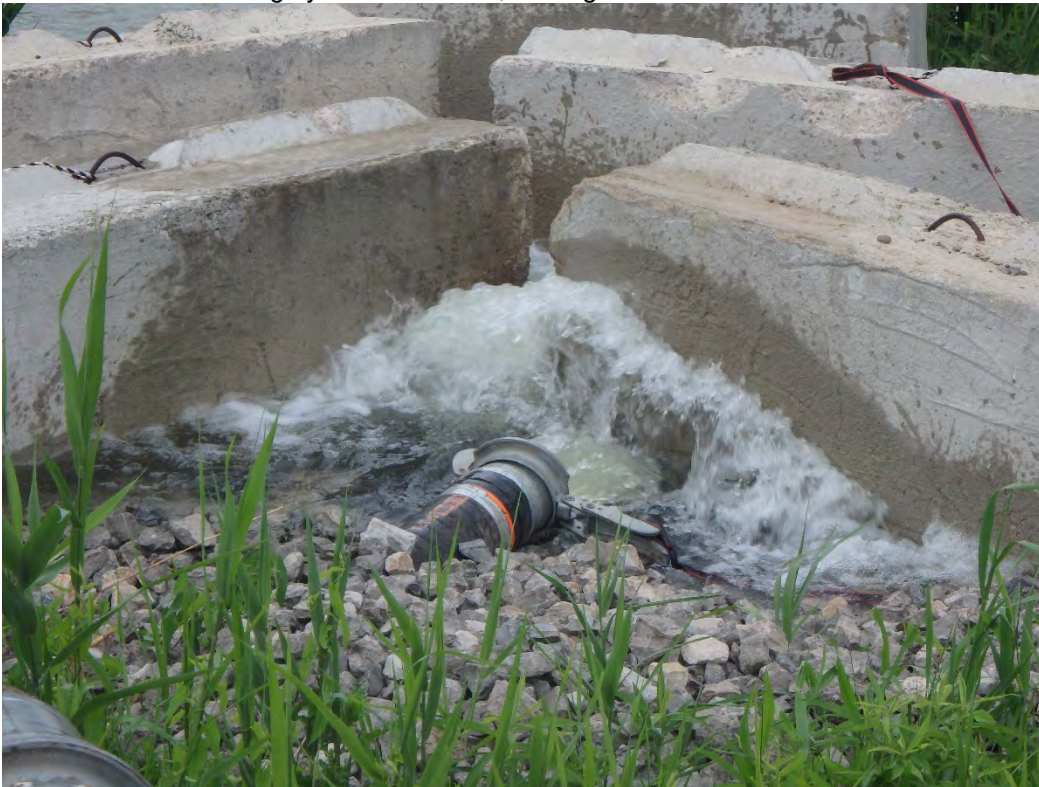
Discharge from pumping of Pond 2, looking south.
