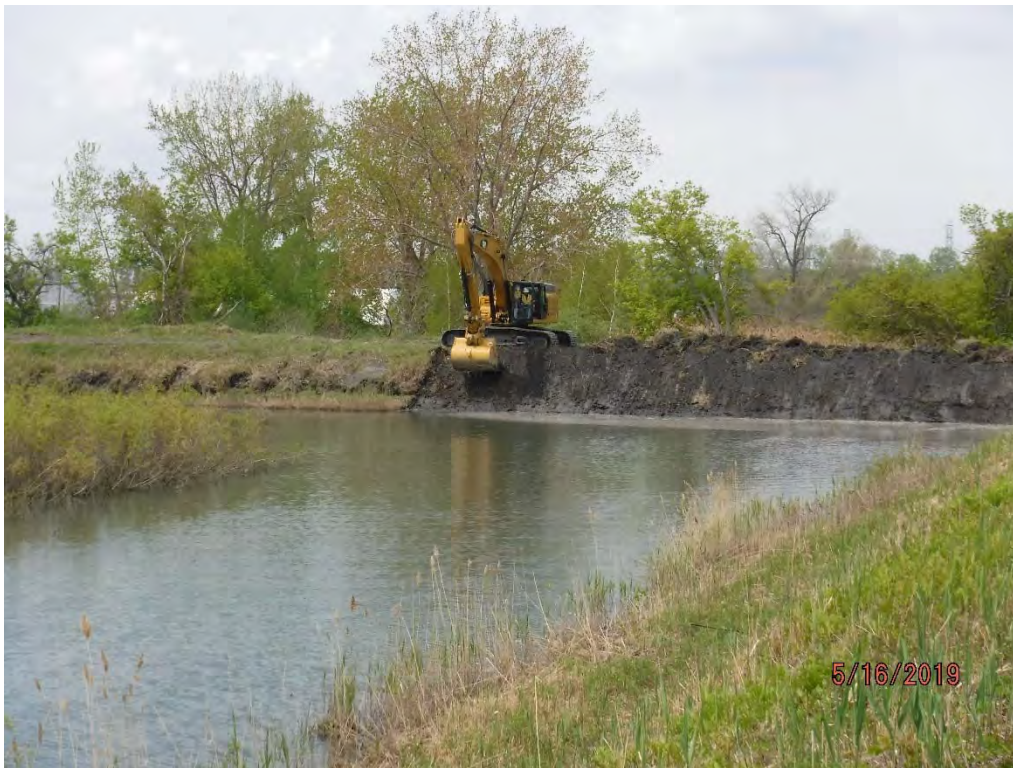
Removing vegetaion on west dike of Pond 1.
