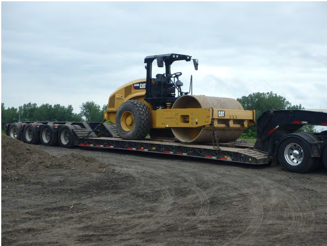
CS56B Smooth Drum mobilized to site, looking northeast.
