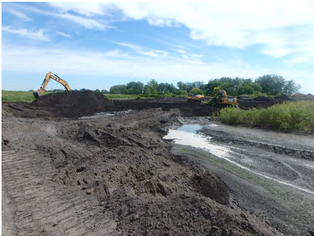
Removing north perimeter road, material to be used for bridging layer. Looking Northeast.
