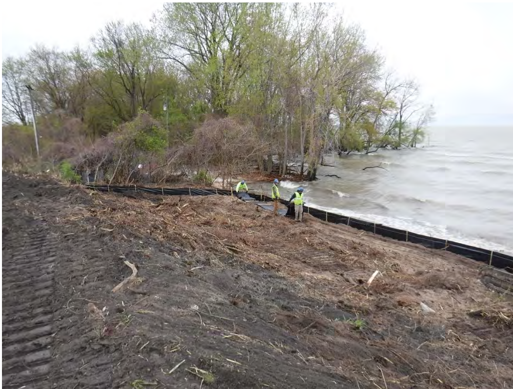
Silt fence diverted into slope to protect disturbed area from erosion.
