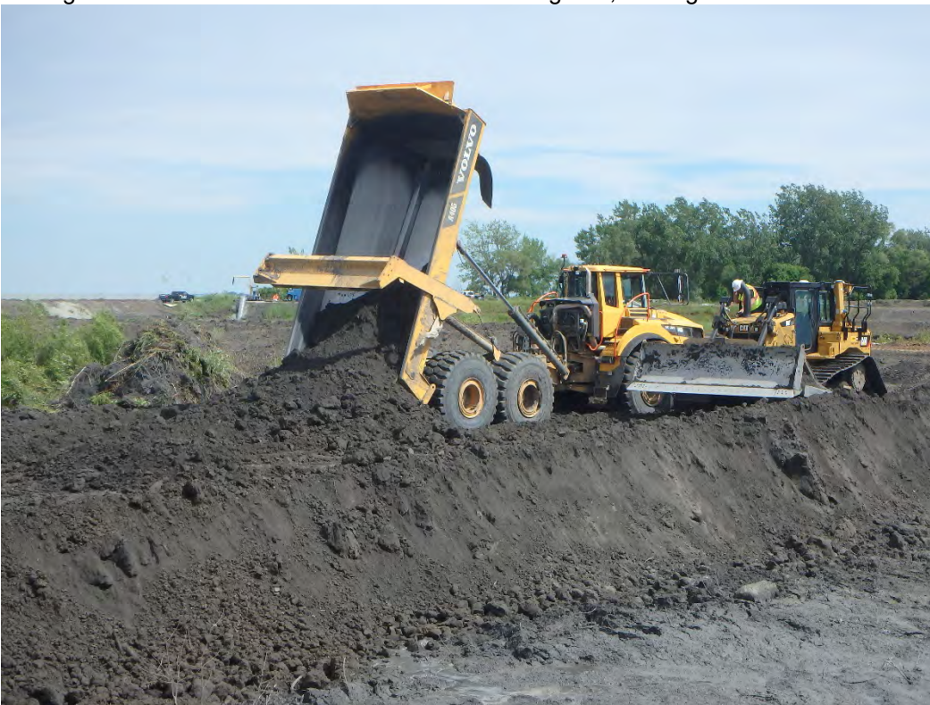
Placing bridging layer in Pond 1, looking southeast.
