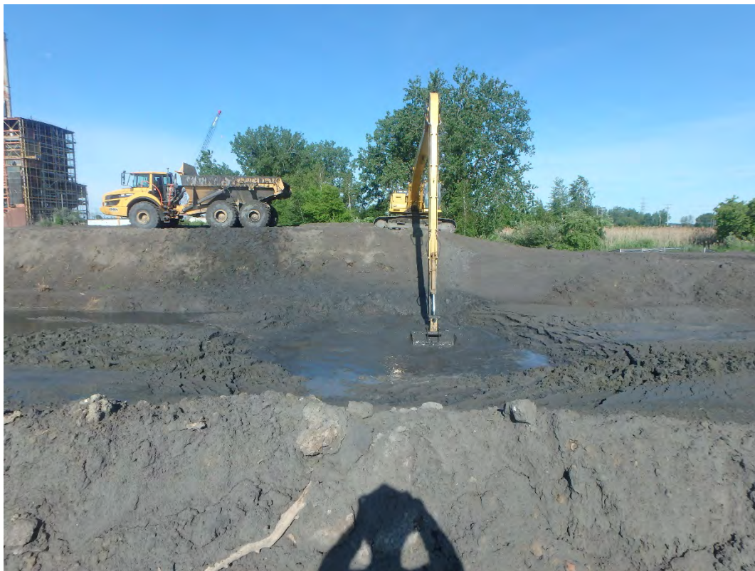
Over-Ex along toe of Pond 1 west slope, looking west.
