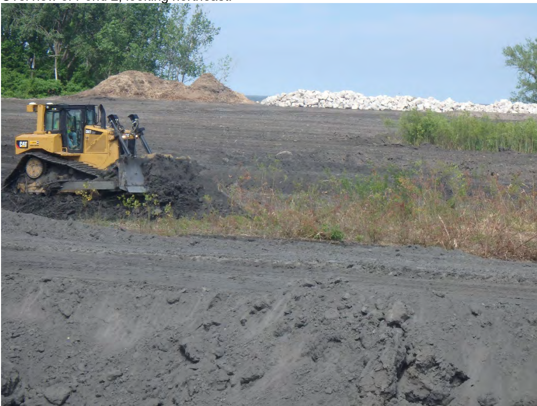
Placing bridging layer in Pond 1, looking east.
