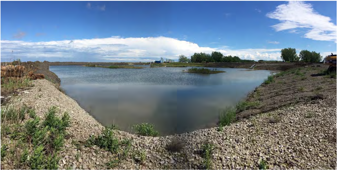
Pond 2 water level, looking southeast.
