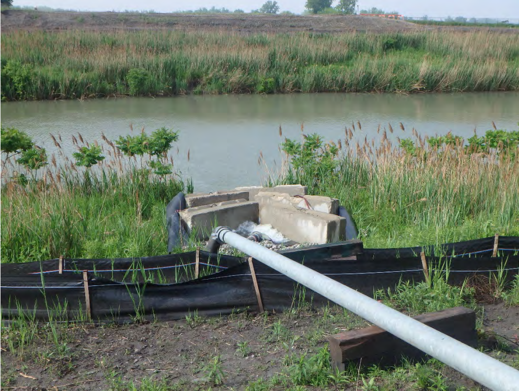
Dewatering of Pond 2 into Discharge Channel, Looking South
