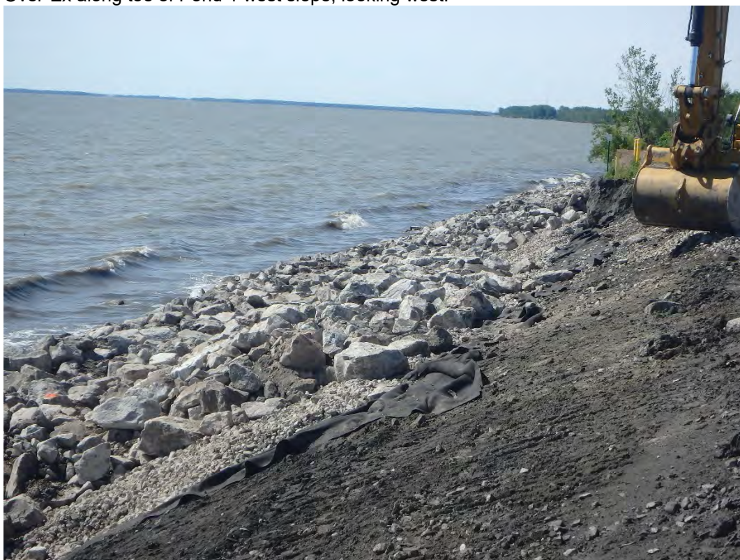
Placement of D50/30 inch riprap along shoreline slope, looking south.
