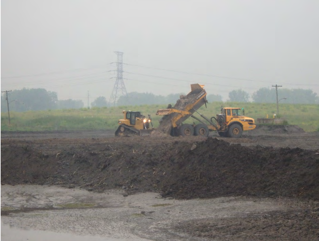
Placing bridging layer in Pond 1, looking northwest.
