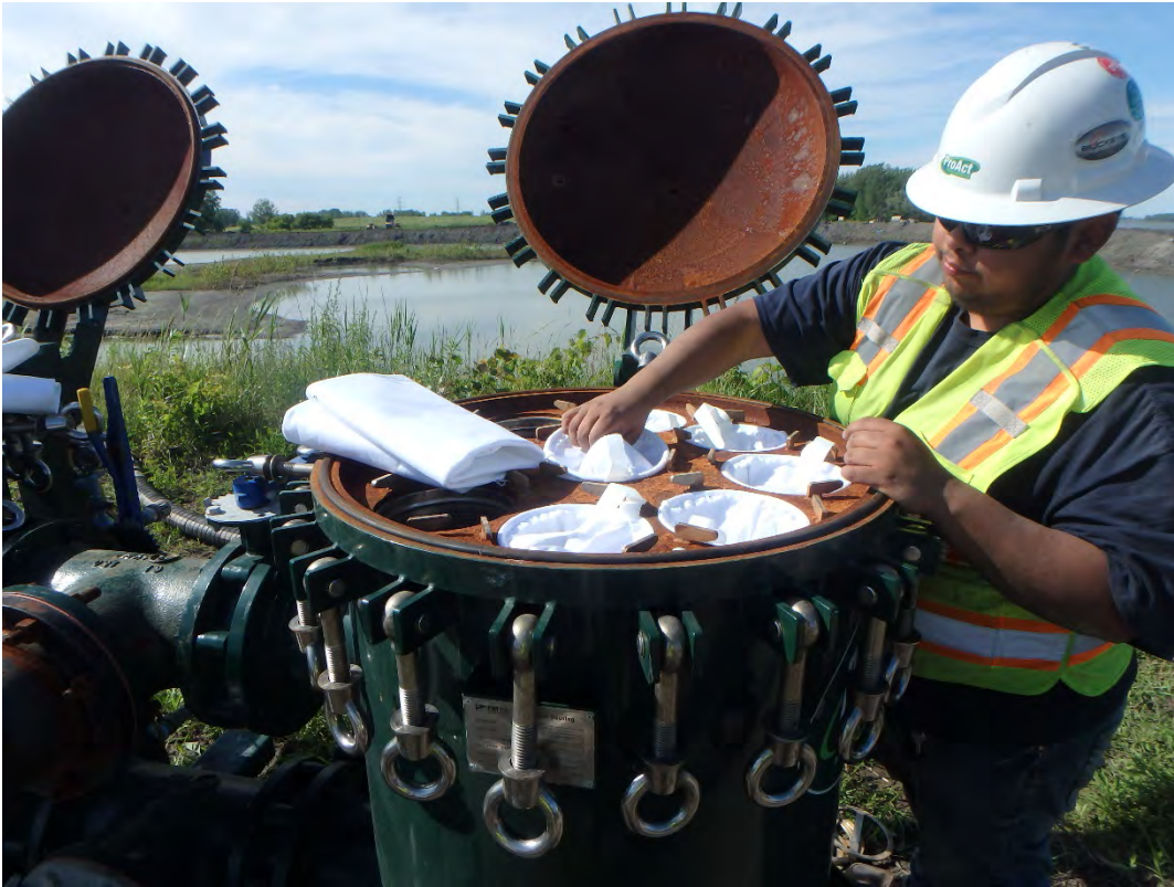
Installing filters on filtration system at Pond 2.
