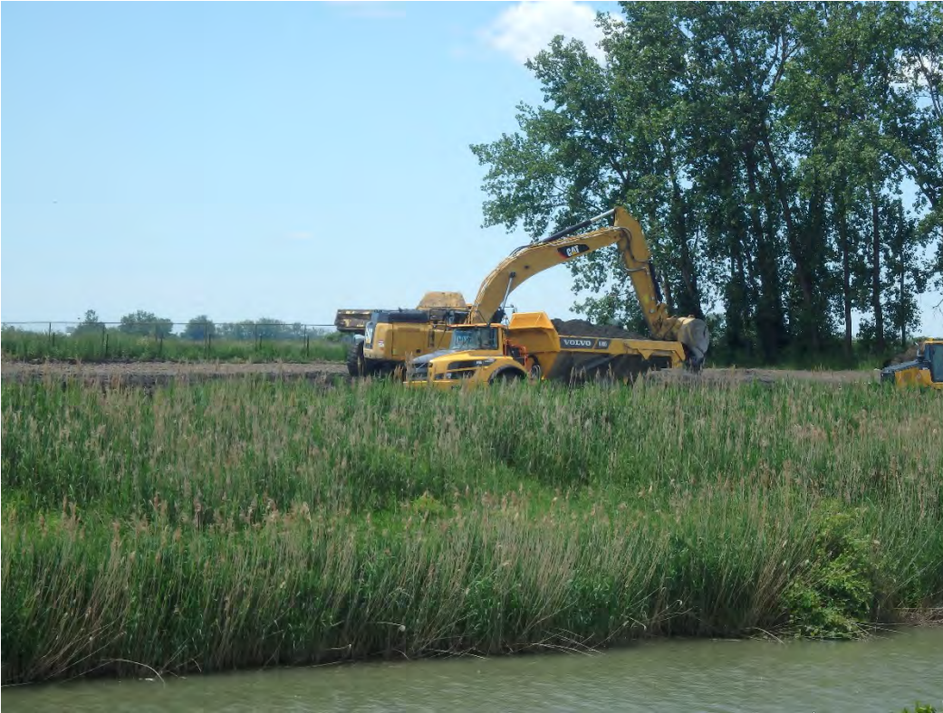
Cutting down Chemical Pond A to 2 feet below final grade, looking south.
