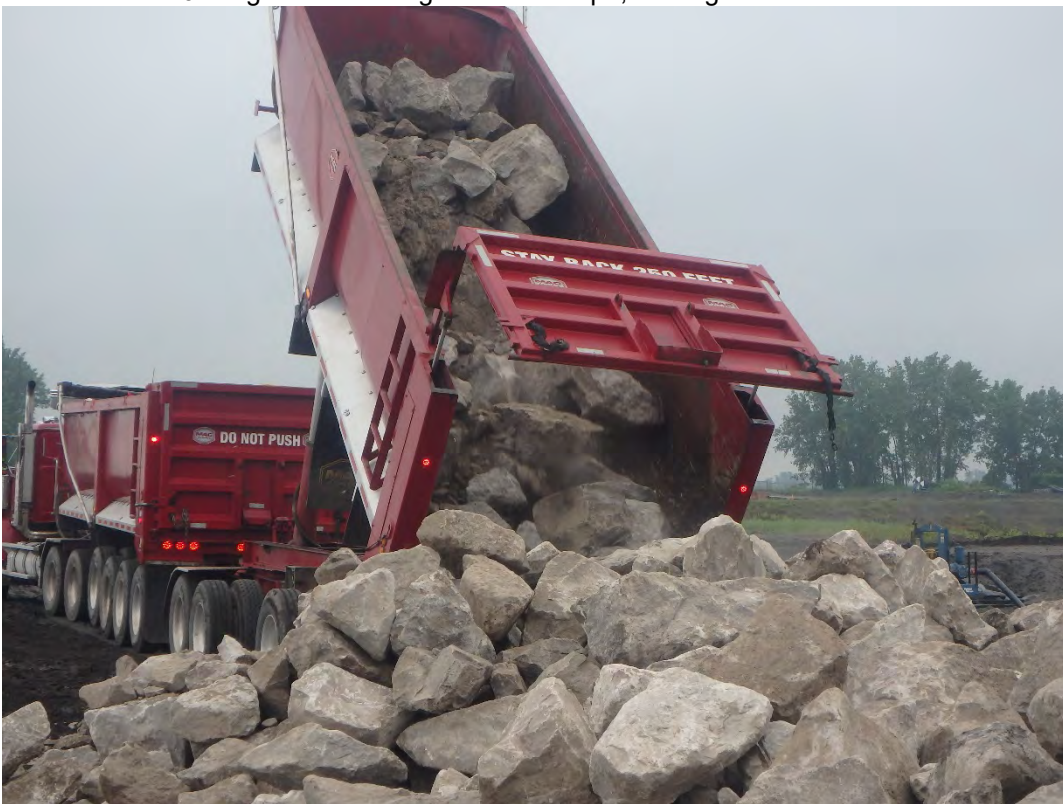
Delivery of D50-30 inch riprap, looking south.
