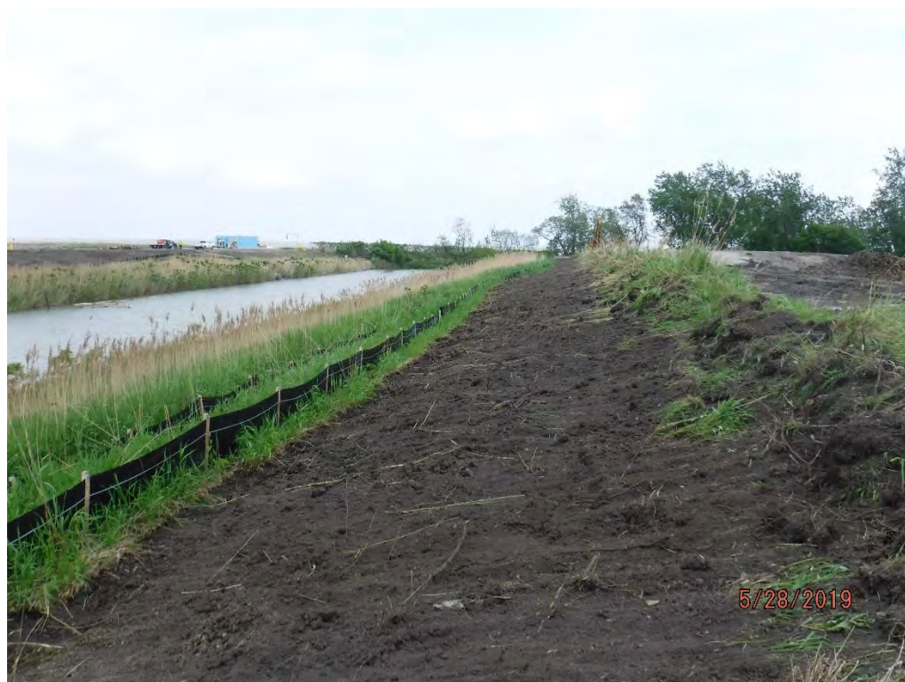
Vegetation removal on south dike of the discharge channel, looking east.
