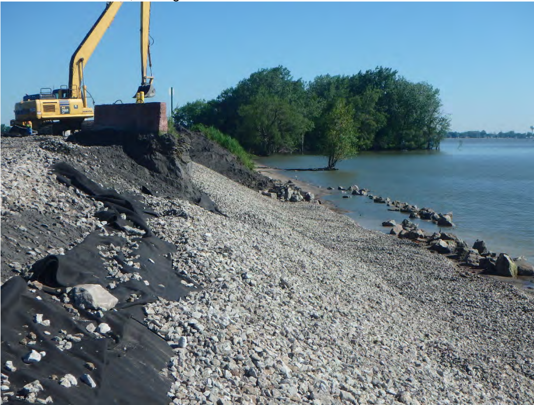
Placing D50/30 inch riprap along shoreline, looking north.
