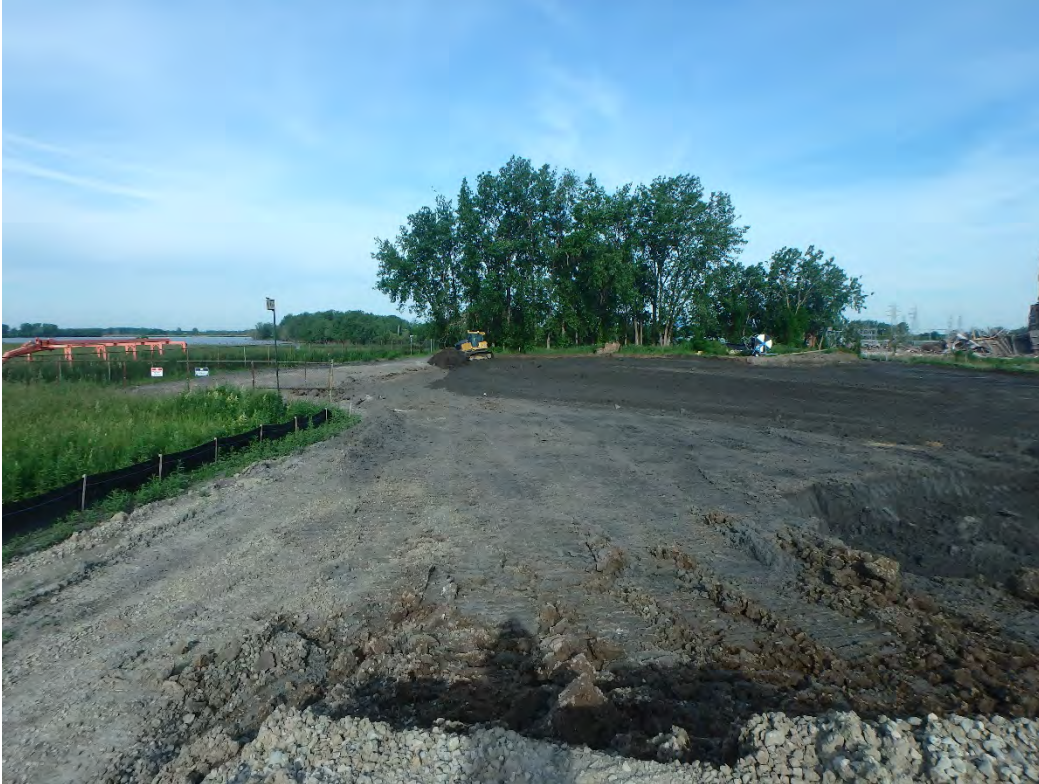
Backfilling Chemical Pond A with structural fill, Looking West.
