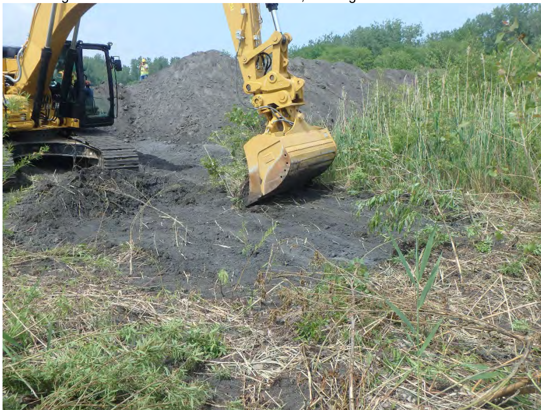
Clearing vegetation from floor of Pond 1
