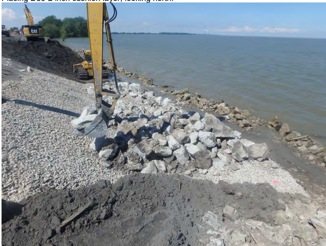
Placing D50-30 inch riprap, looking north.
