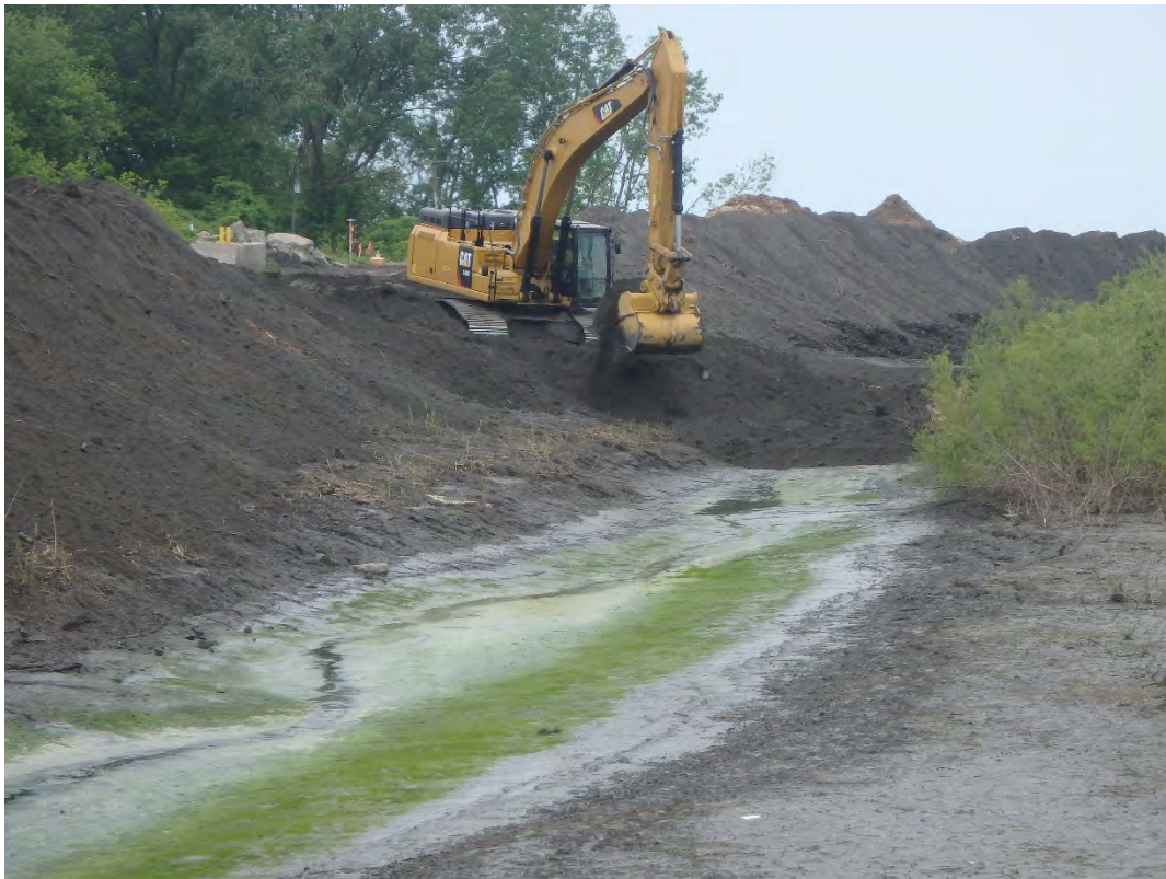
Bridging layer being placed in Pond 1
