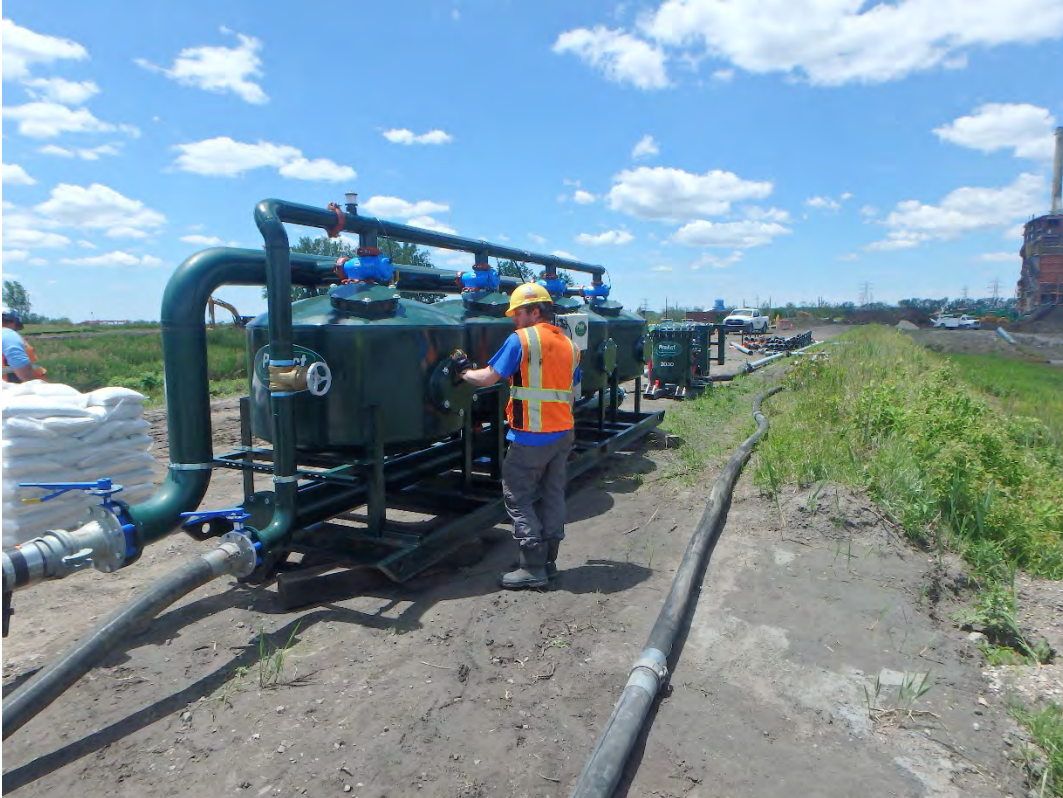
Set-up of sand pots at Pond 2, looking west
