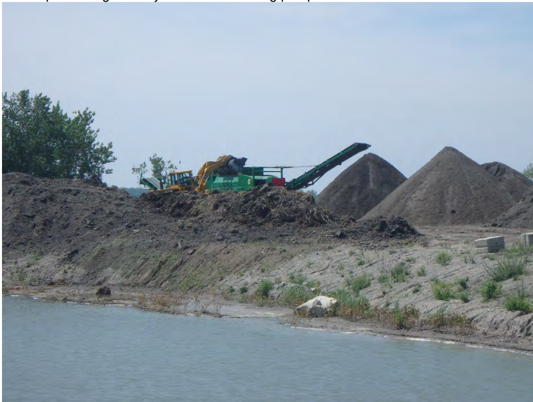
Screening of vegetation removed from Pond 1
