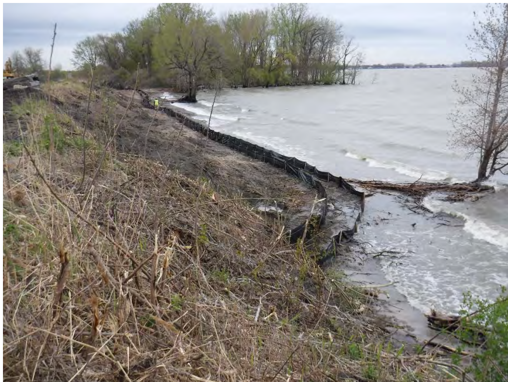
Silt fence diverted into slope to protect disturbed area from erosion.
