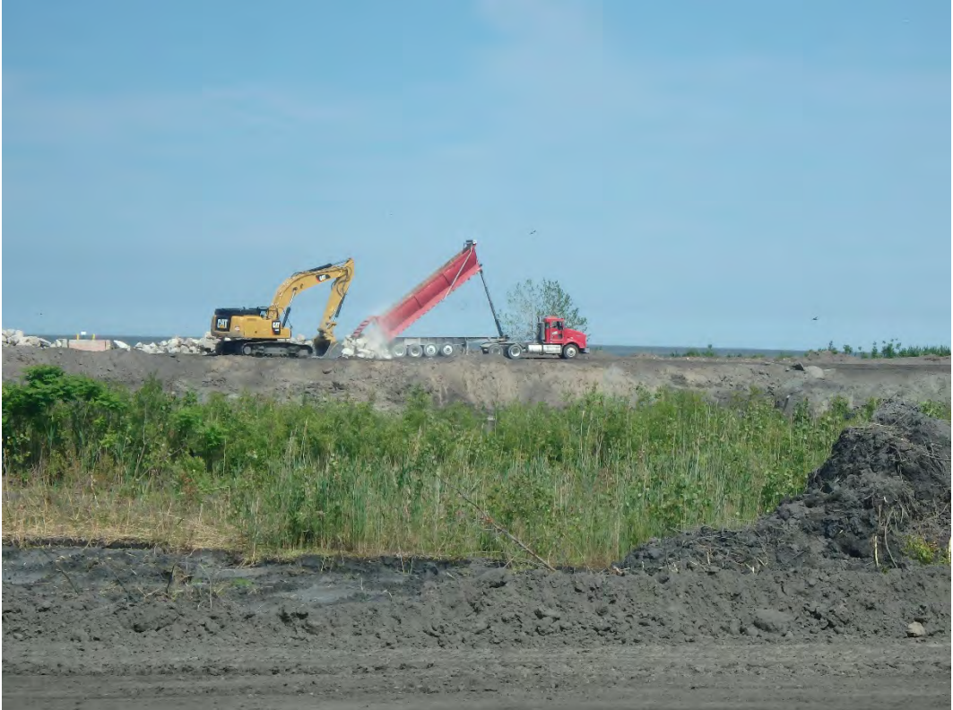
Delivery of D50-30 inch riprap, looking east.
