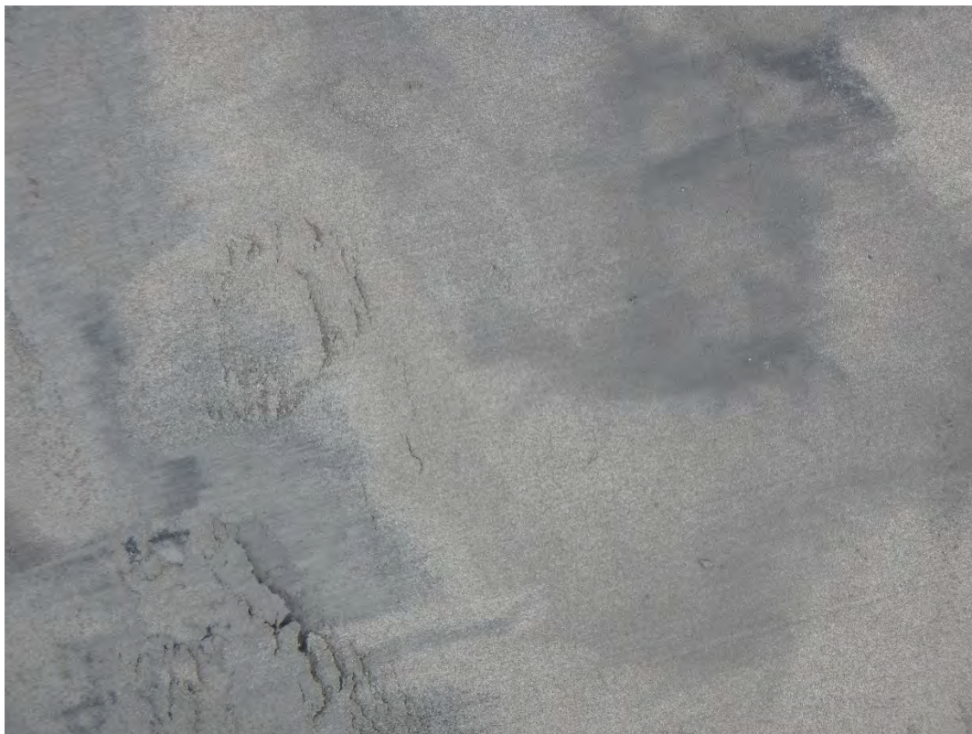
Chemical Pond A floor consisting of clean ash after removal of residual.
