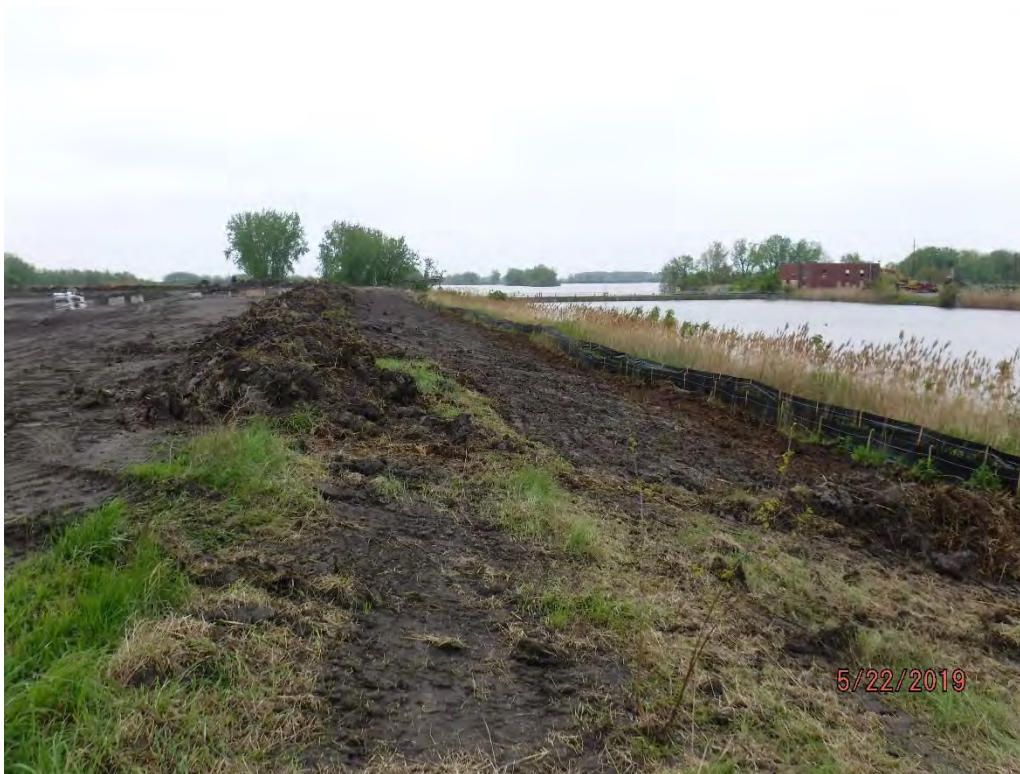
Vegetation removal from south dike of Pond 2 near discharge channel, looking west.
