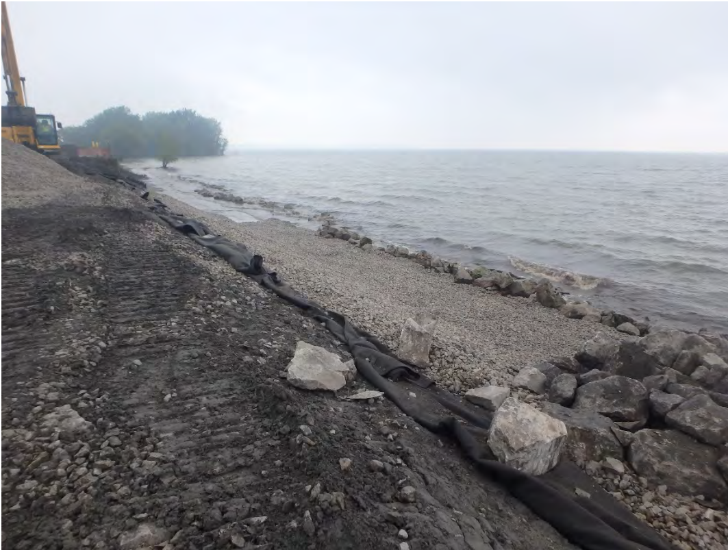
D50/2 inch placement along shoreline slope, looking north.
