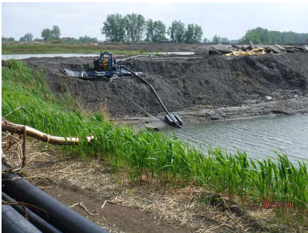
Pump system for pumping Pond 1 into Pond 2, looking south.
