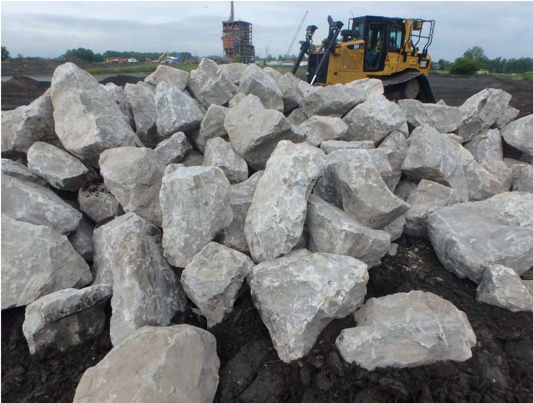
D50 – 30 inch riprap stockpile for shoreline, looking west.
