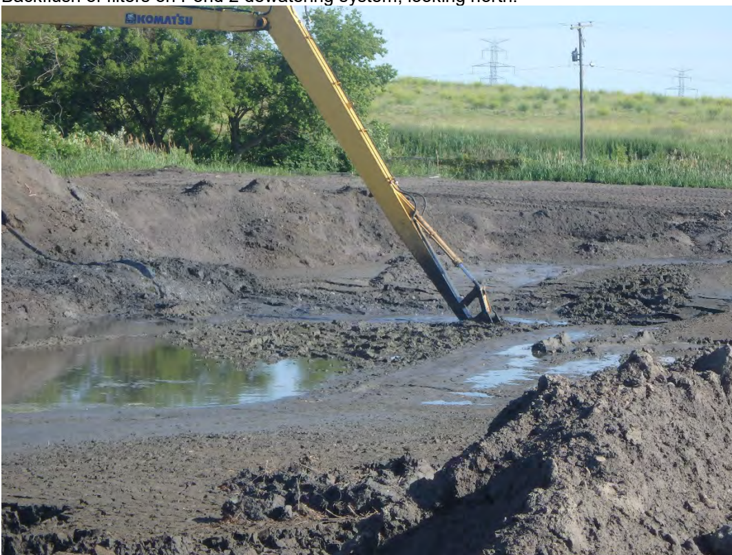
Over-Ex west side of Pond 1, looking north.
