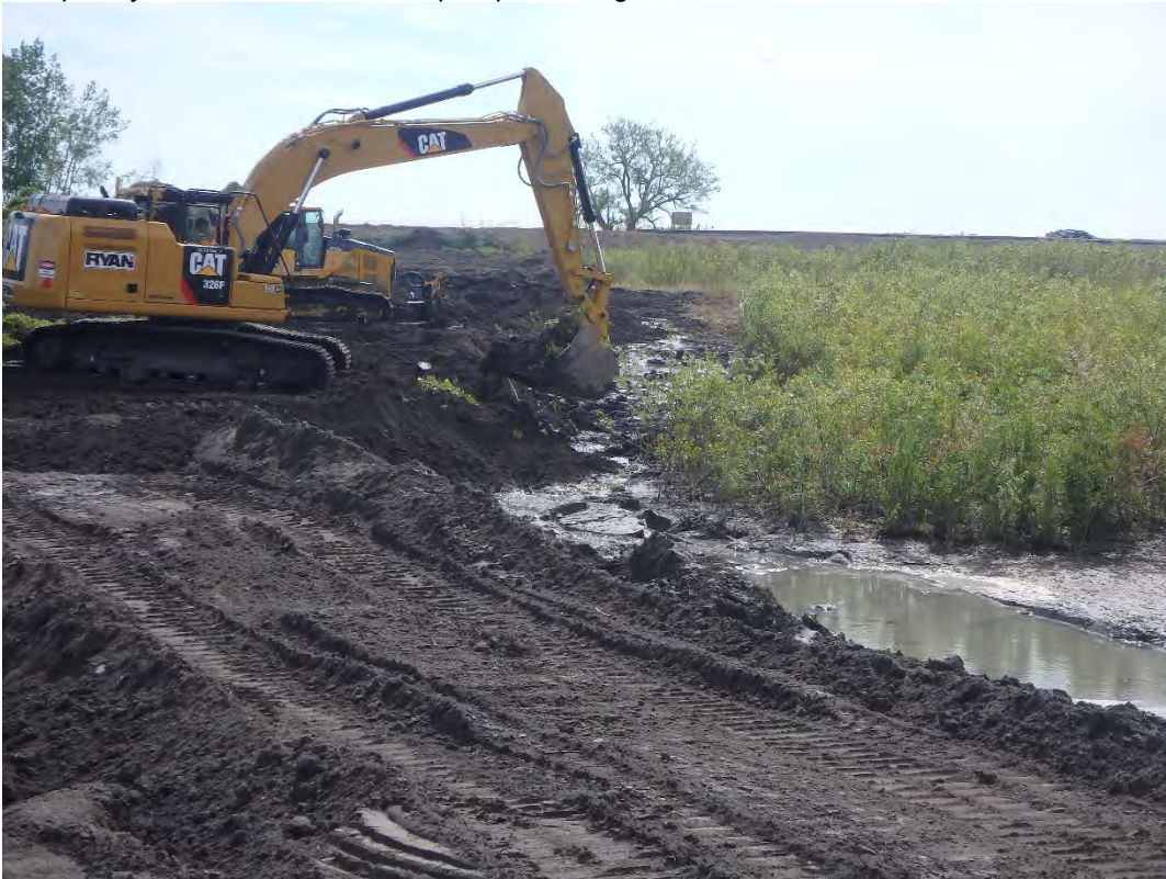
Removing vegetation from Pond 1
