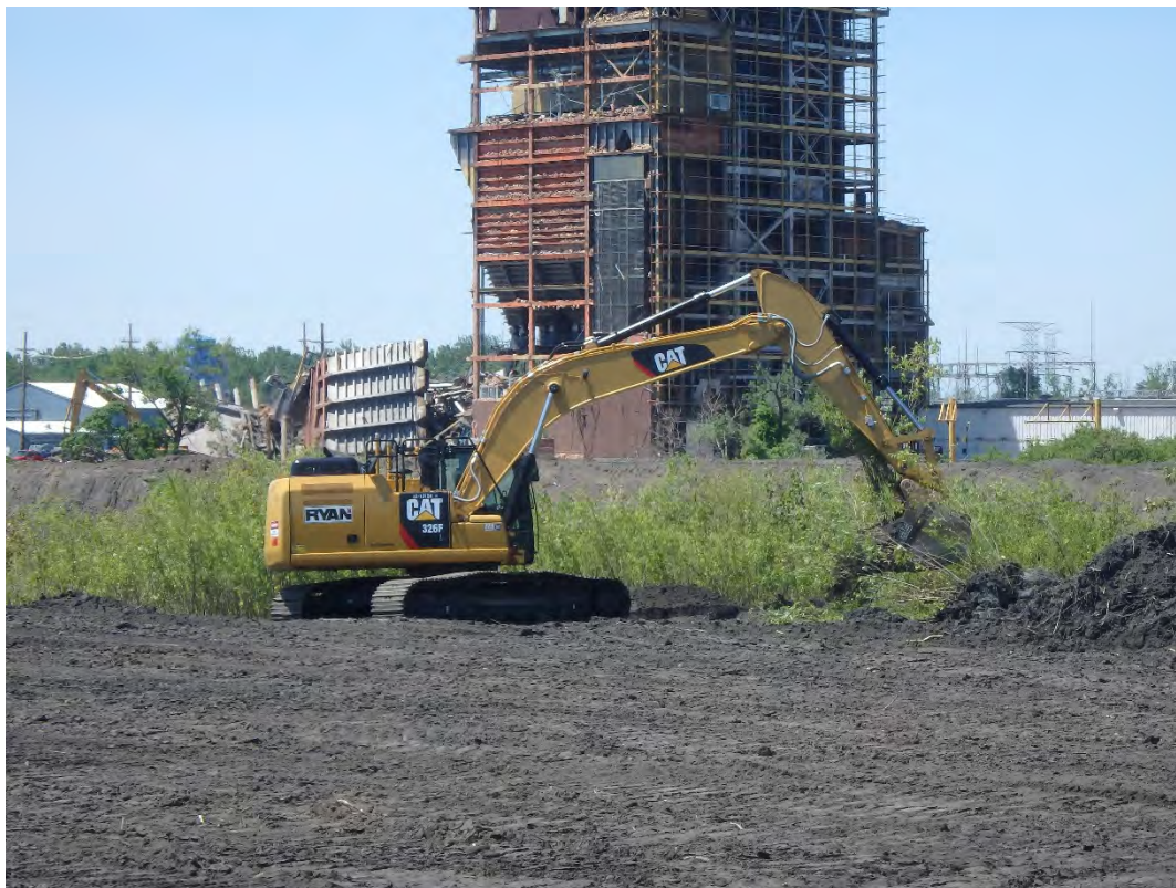
Clearing vegetation from Pond 1, Looking West.
