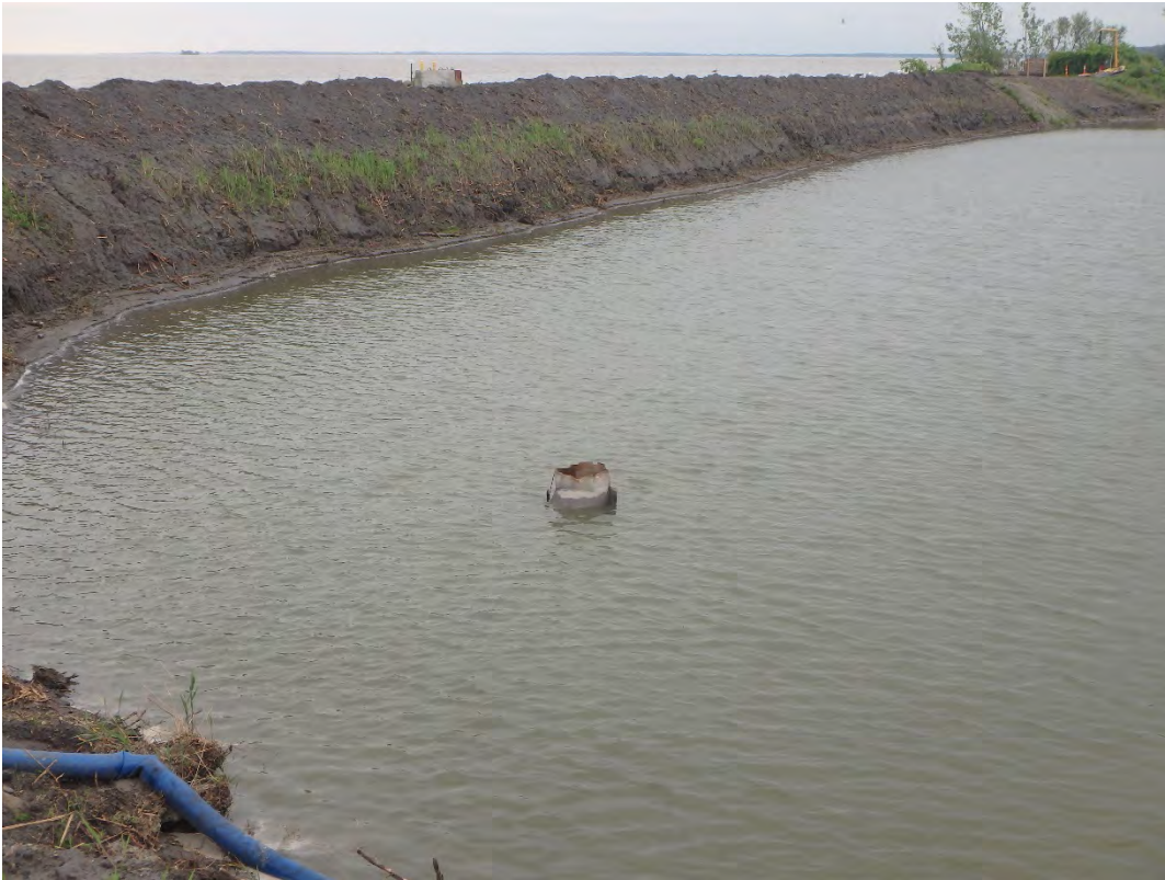
Water level of Pond 2, Looking Southeast.
