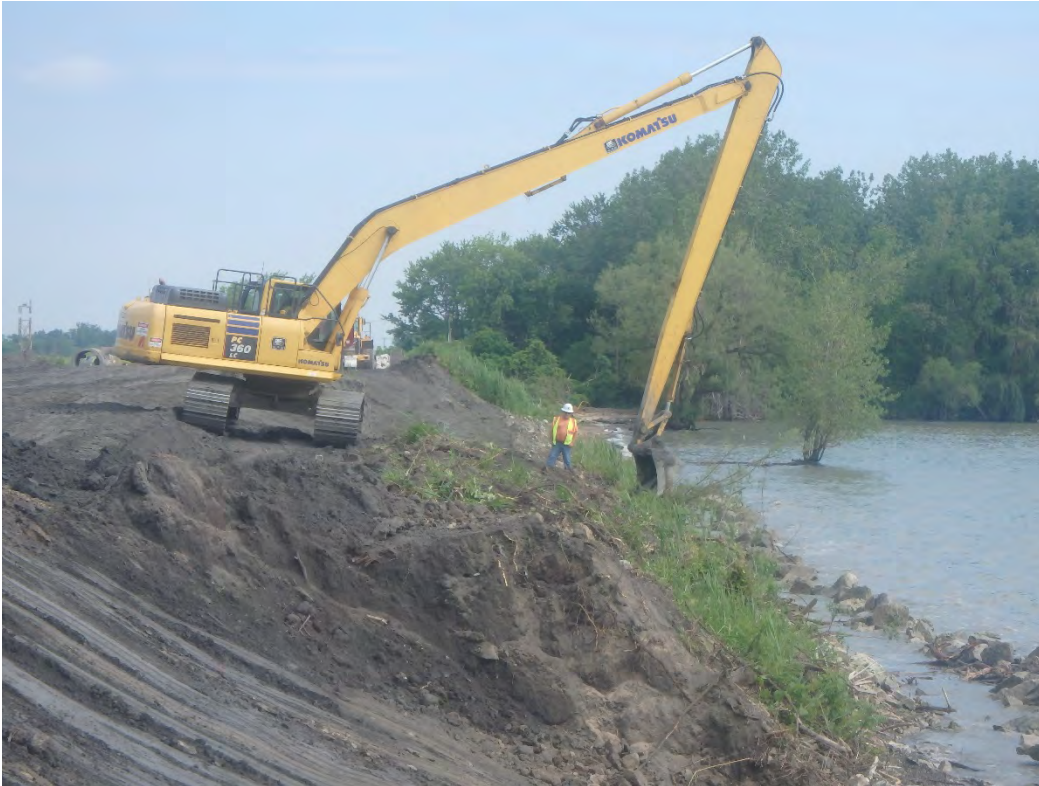
Removing vegetation along shoreline slope, looking north.
