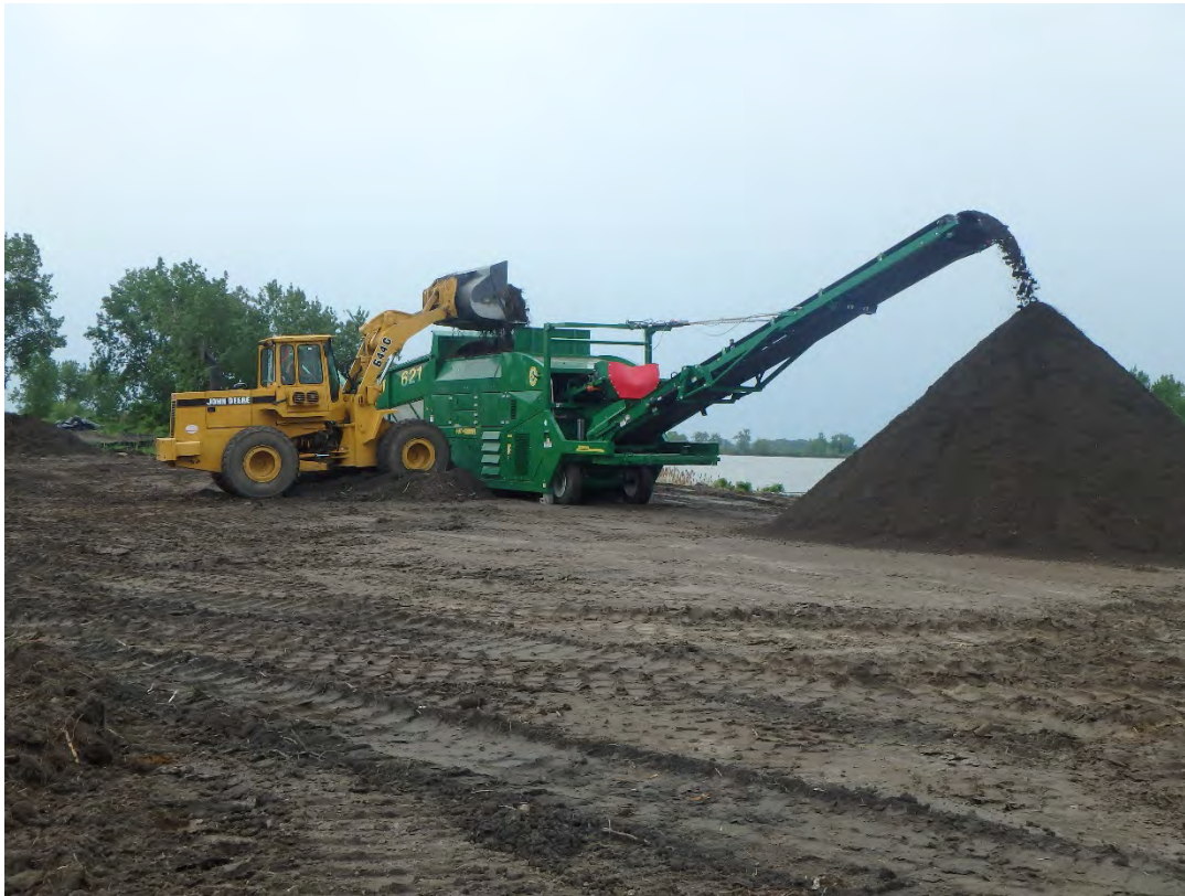
Screening cleared/grubbed material to remove organics
