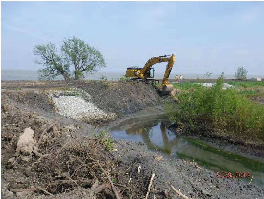
Vegetation removal on east dike of Pond 1, looking southeast.
