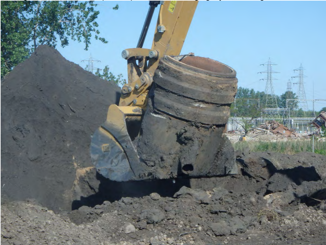
Removing manhole from north side of Chemical Pond A, Looking West.
