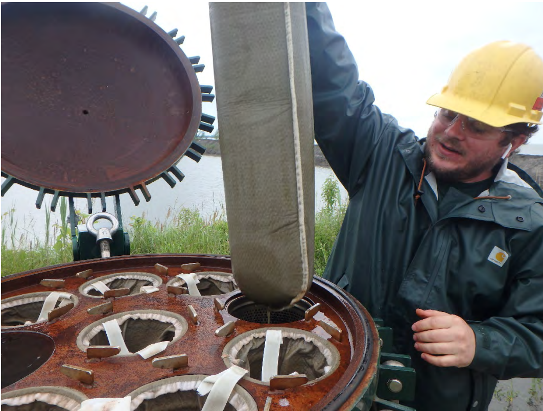
Changing cloth filters, looking northeast.
