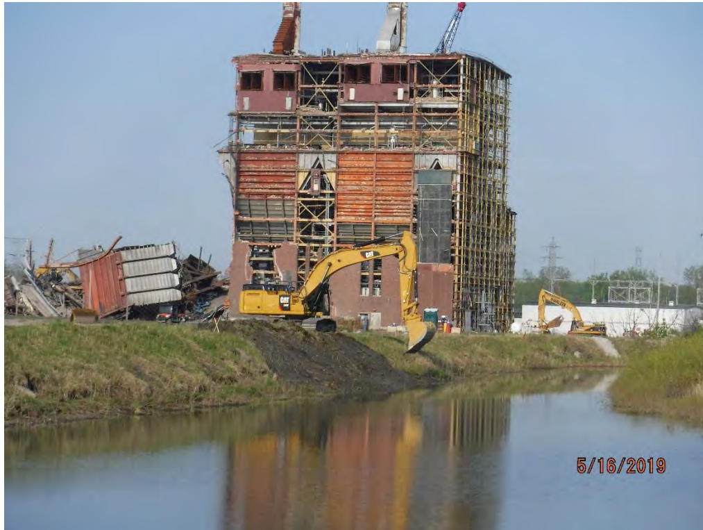
Removing vegetation north of center dike between Pond 1 and Pond 2.
