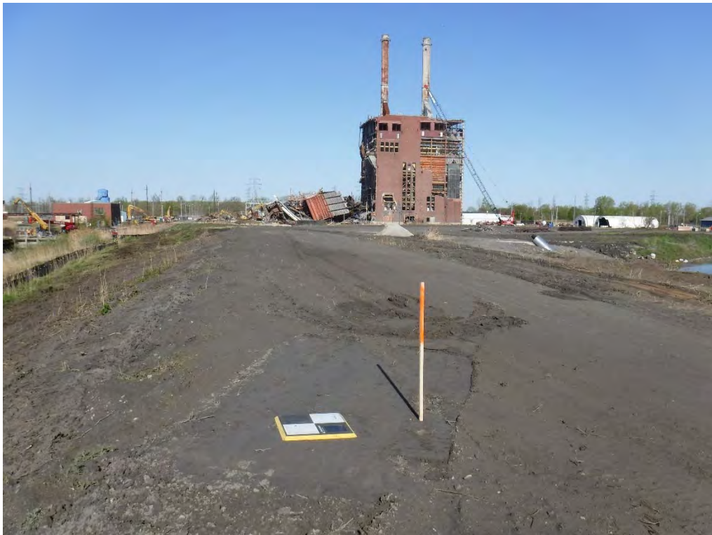
Control set for existing conditions drone survey.
