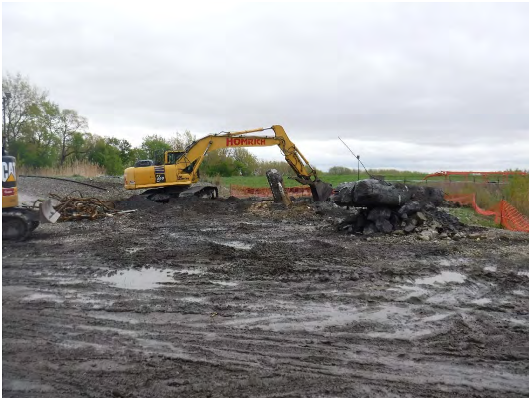
Homrich performing demo work of the Chemical Treatment Building.
