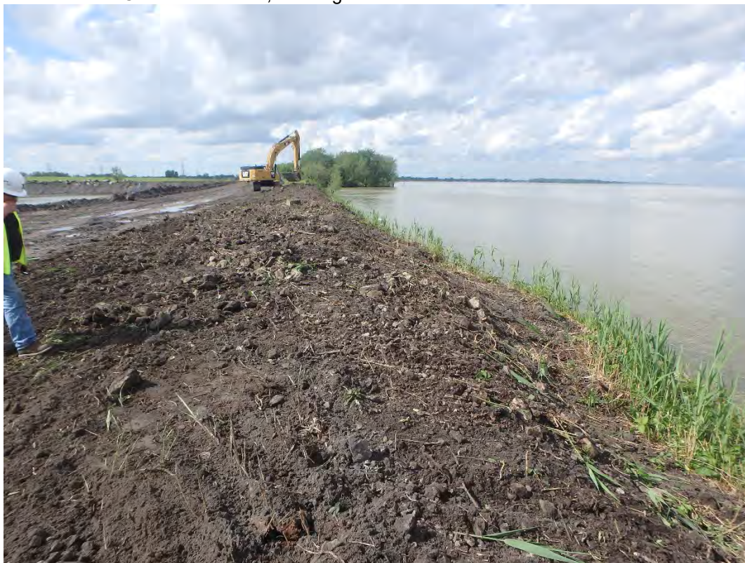
Clearing/Grubbing atop shoreline slope east of Pond 2
