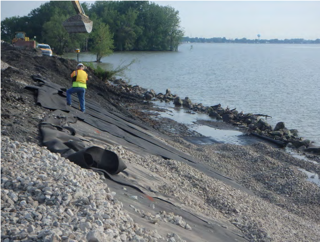
Checking grade atop geotextile, looking north.
