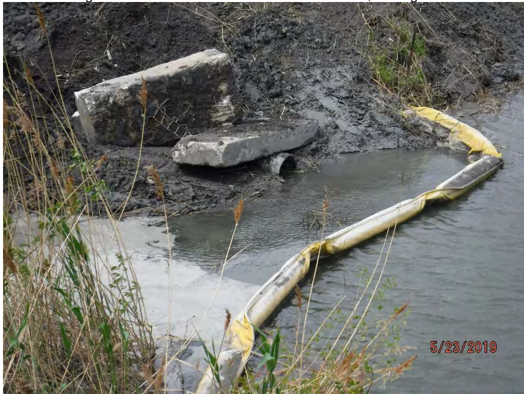
Culvert invert connecting Pond 1 and Pond 2 lowered on the north side, looking southwest.
