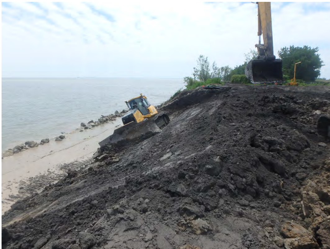
Grading shoreline slope, looking south.
