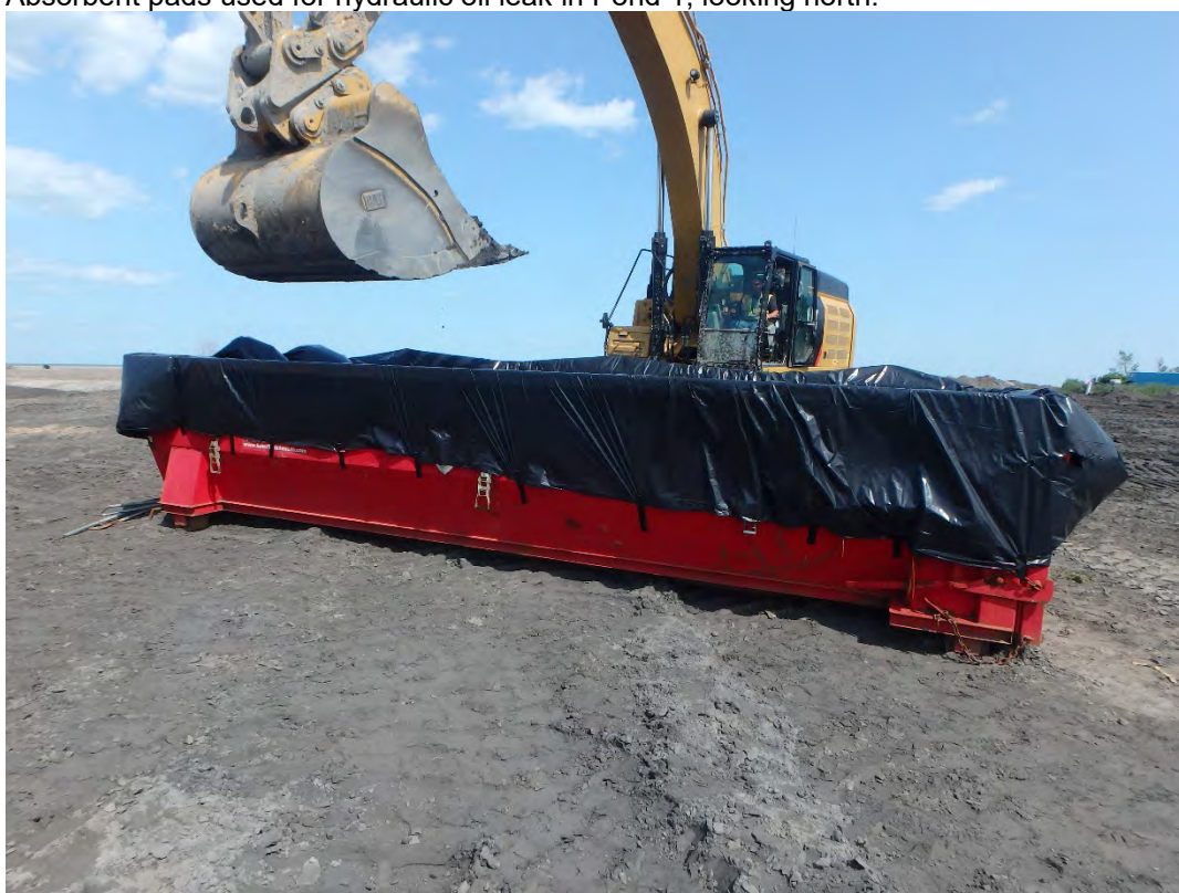
Lined dumpster used for disposal of contaminated soils excavated west of Pond 2, looking east.
