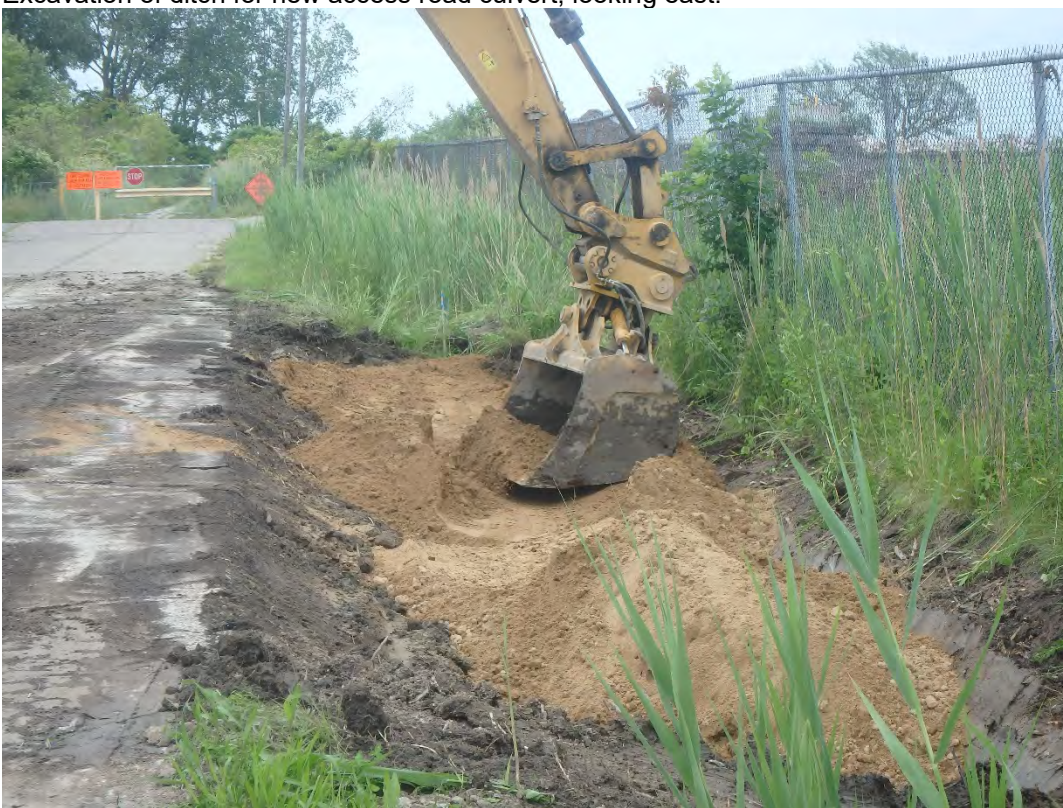
Placement of culvert bedding material, looking east.
