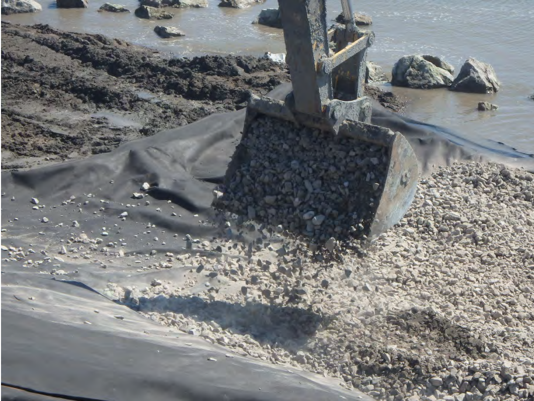
Placement of D50/2 inch cushion layer along shoreline, looking east.
