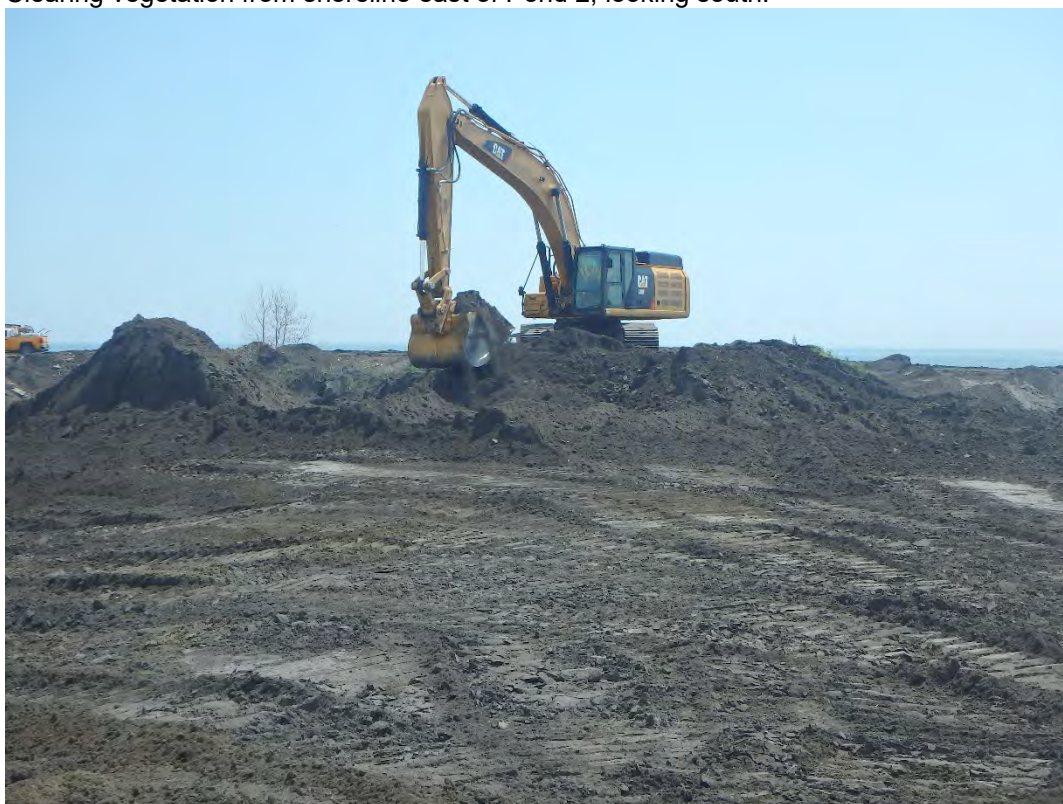
Excavating center dyke/access road down to grade, looking east.
