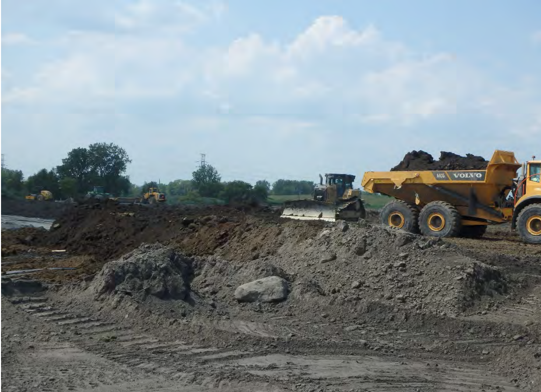
Placing bridging layer in Pond 2, looking west.
