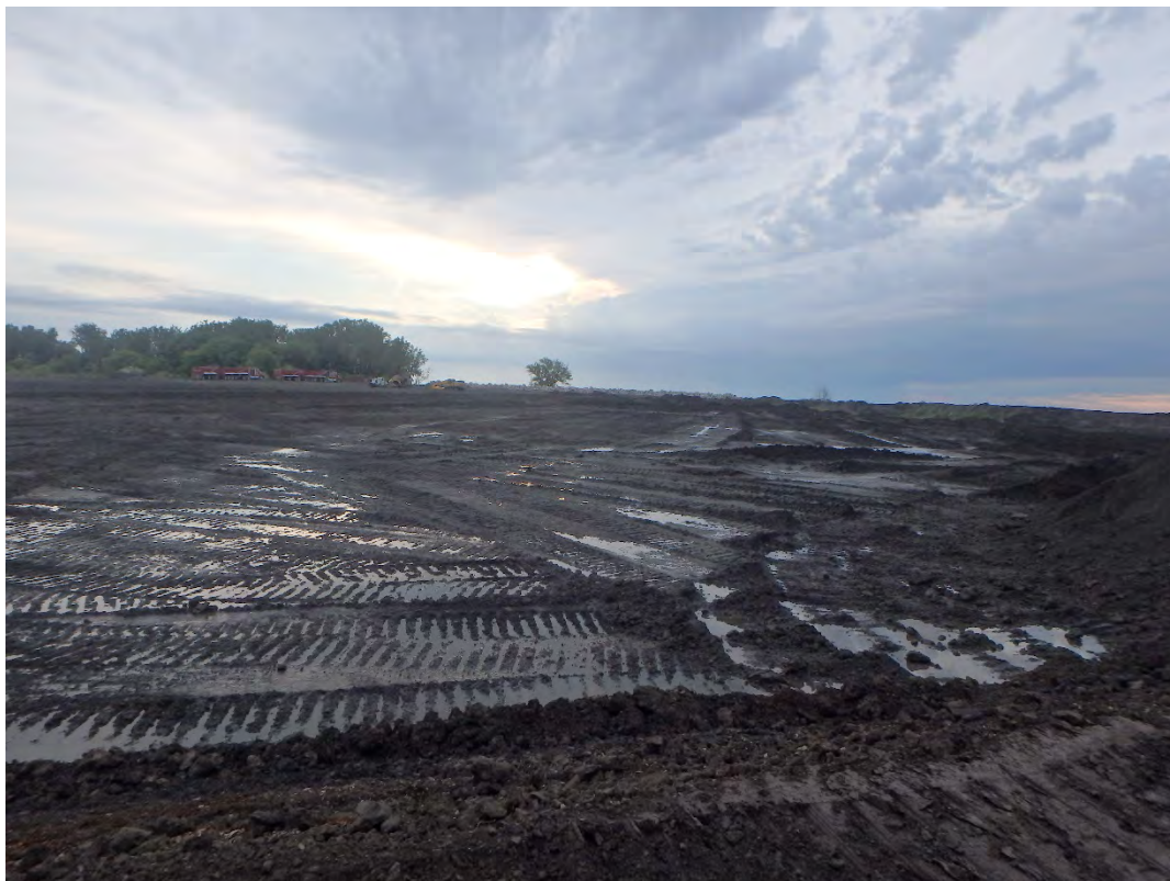
Overview of Pond 1, looking northeast.
