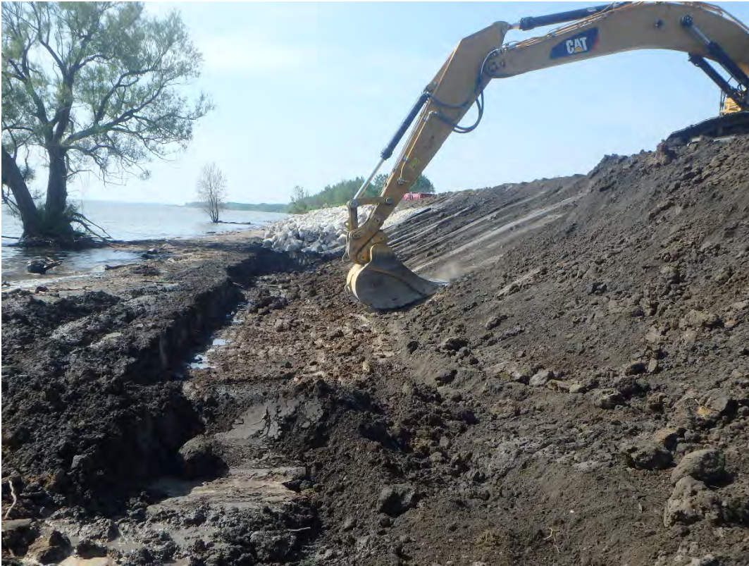
Cutting shoreline slope to sub-grade, looking south.
