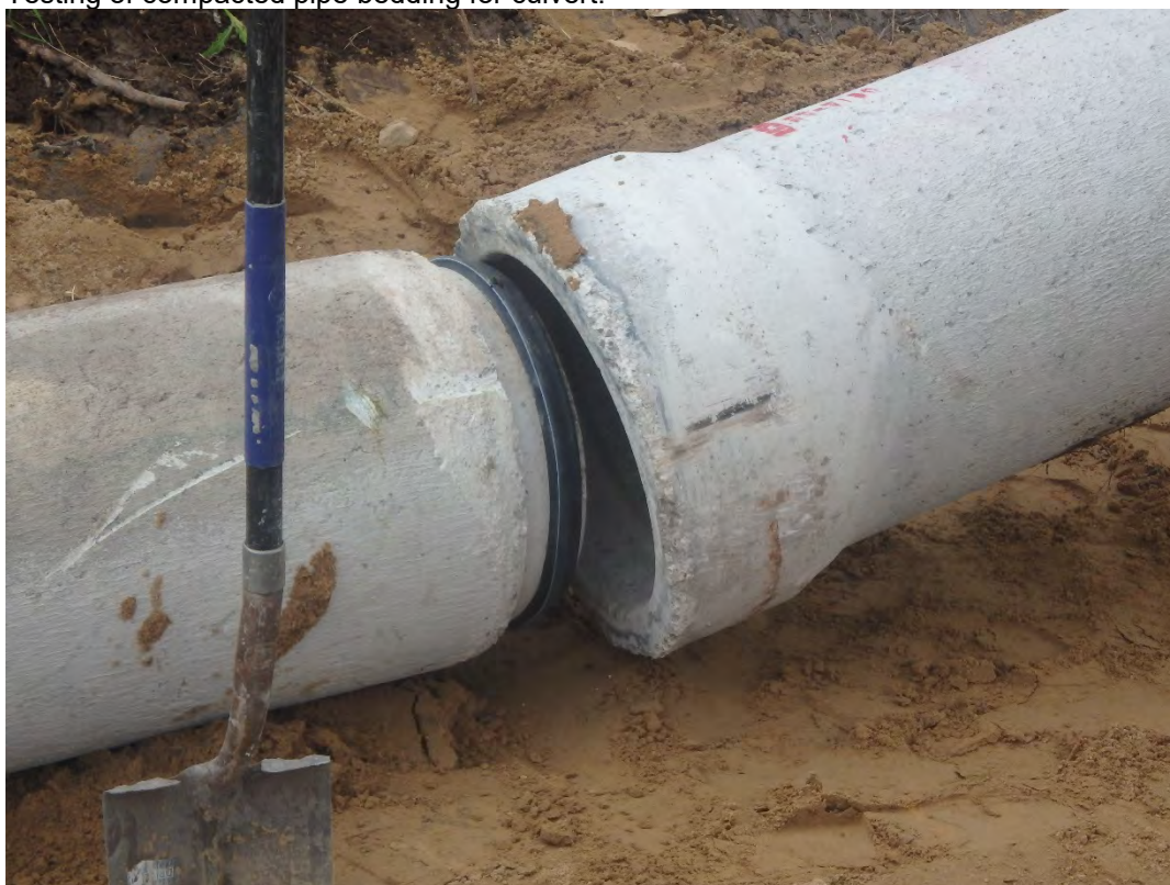
Installation of 12 inch RCP for access road culvert.
