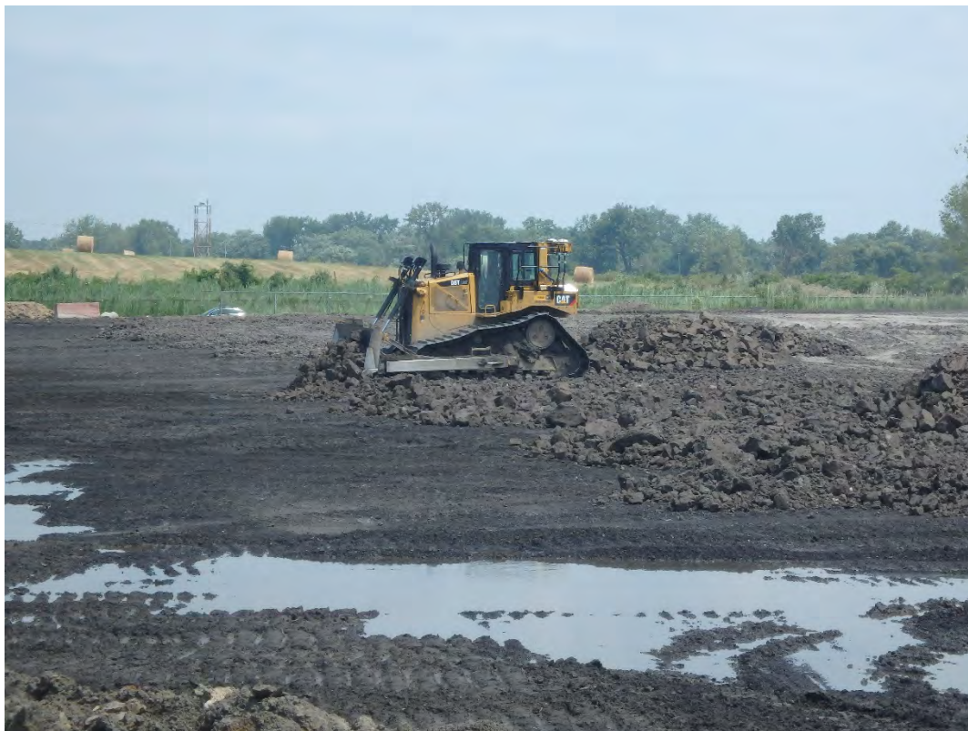
Placement of structural fill lift in Pond 1, looking north.
