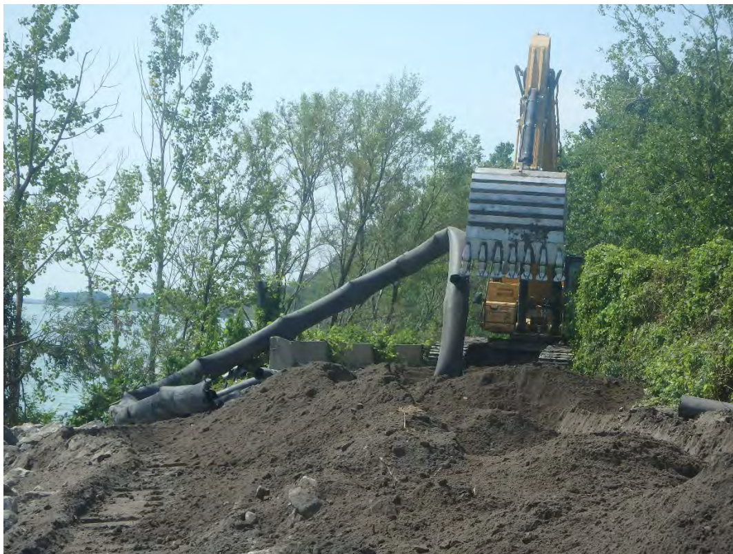
Removing utility pipe from Pond 2 to Chemical Ponds, looking south.
