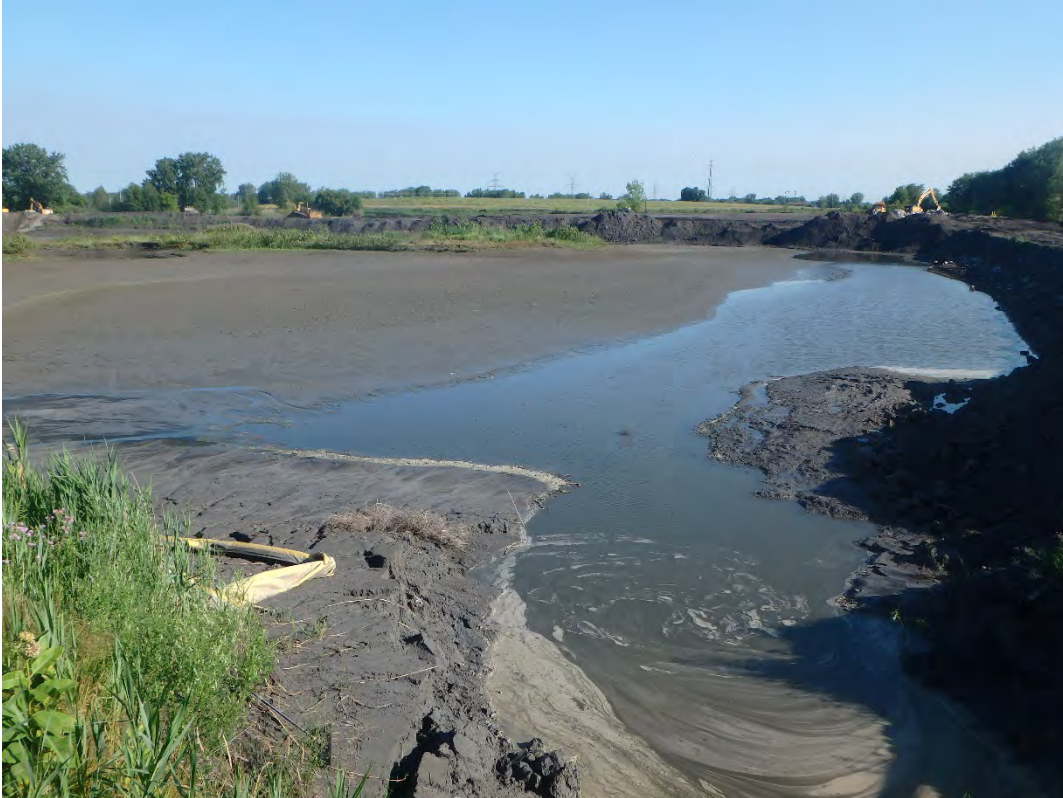
Overview/water level Pond 2, looking northern.
