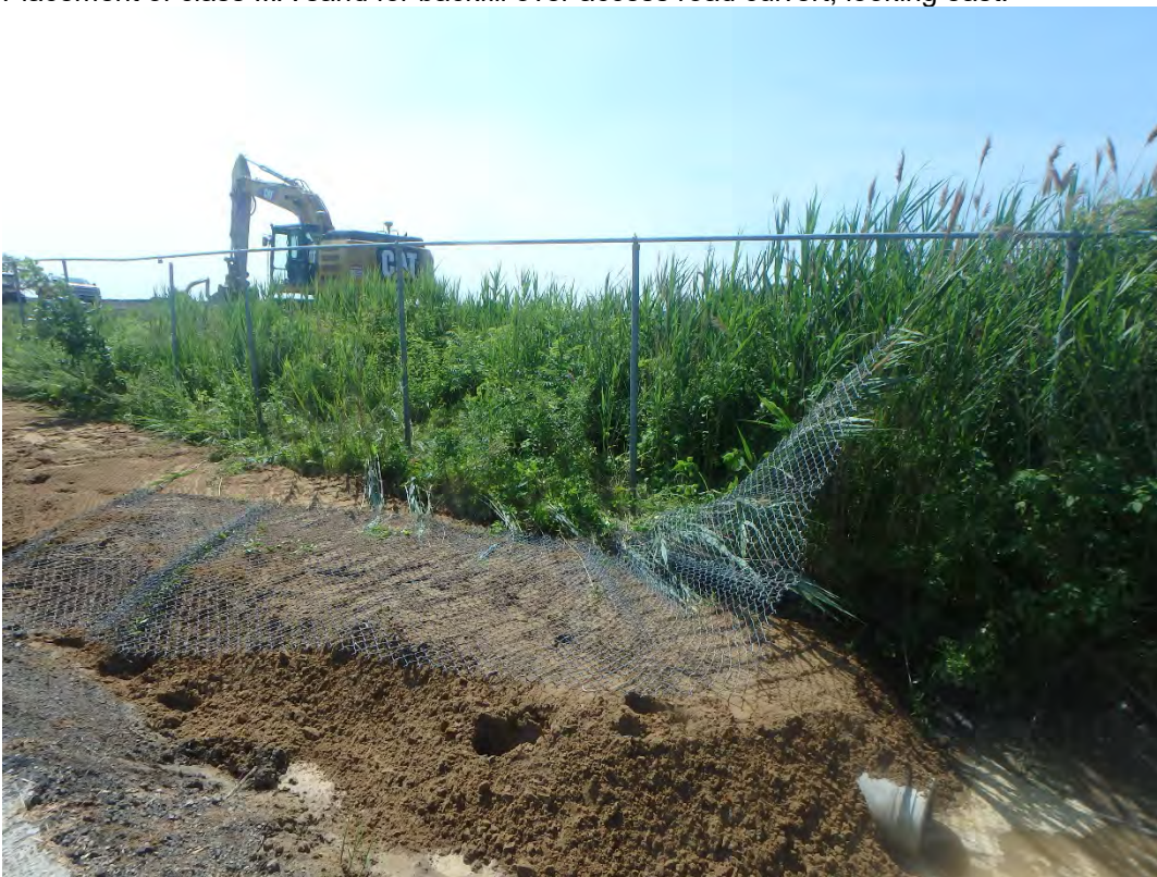
Removing fence for new entrance access road, looking southeast.
