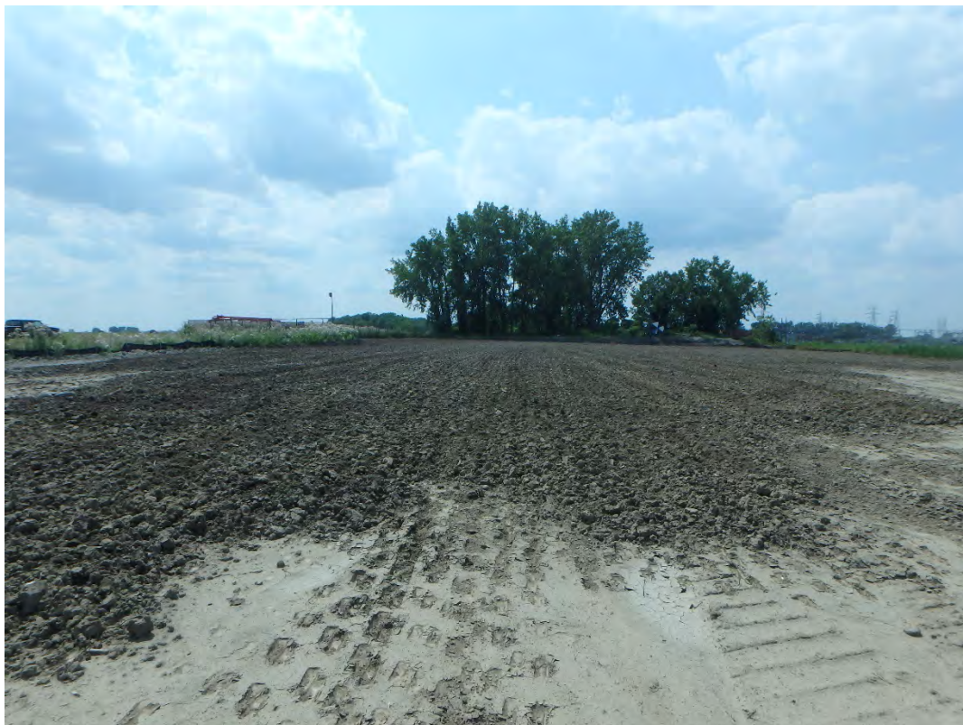
Overview of compacted structural fill at the Chemical Ponds, looking west.
