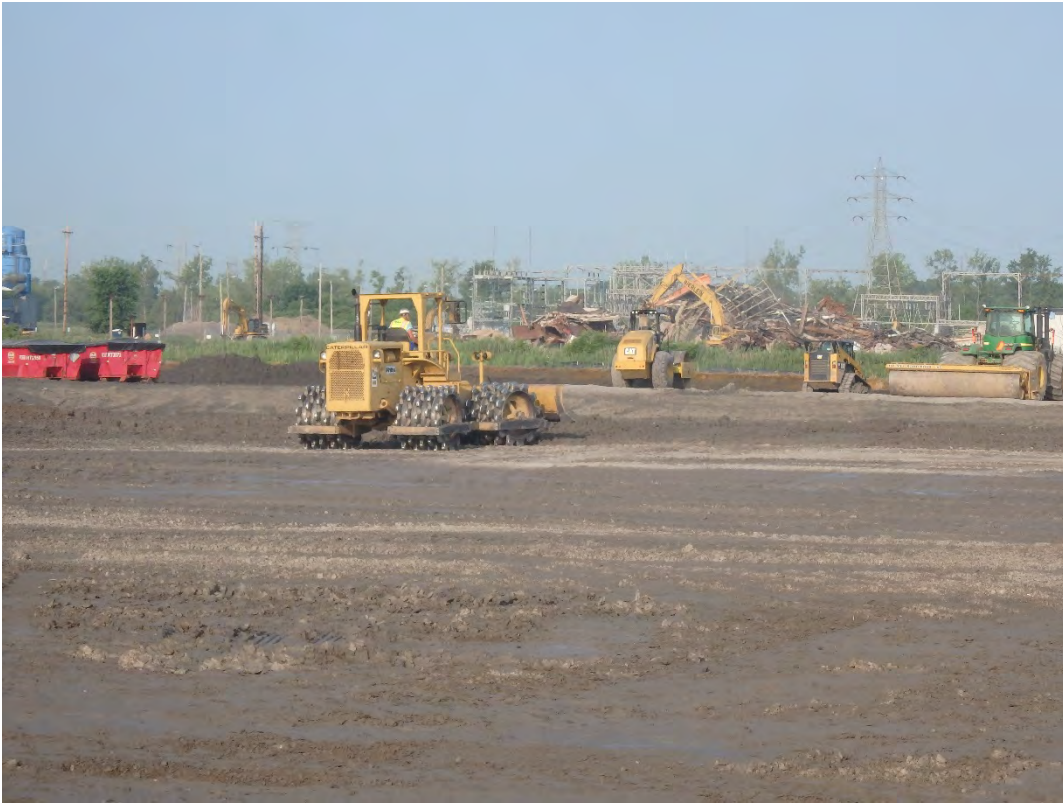
Compacting structural fill placed in Pond 1, looking southwest.
