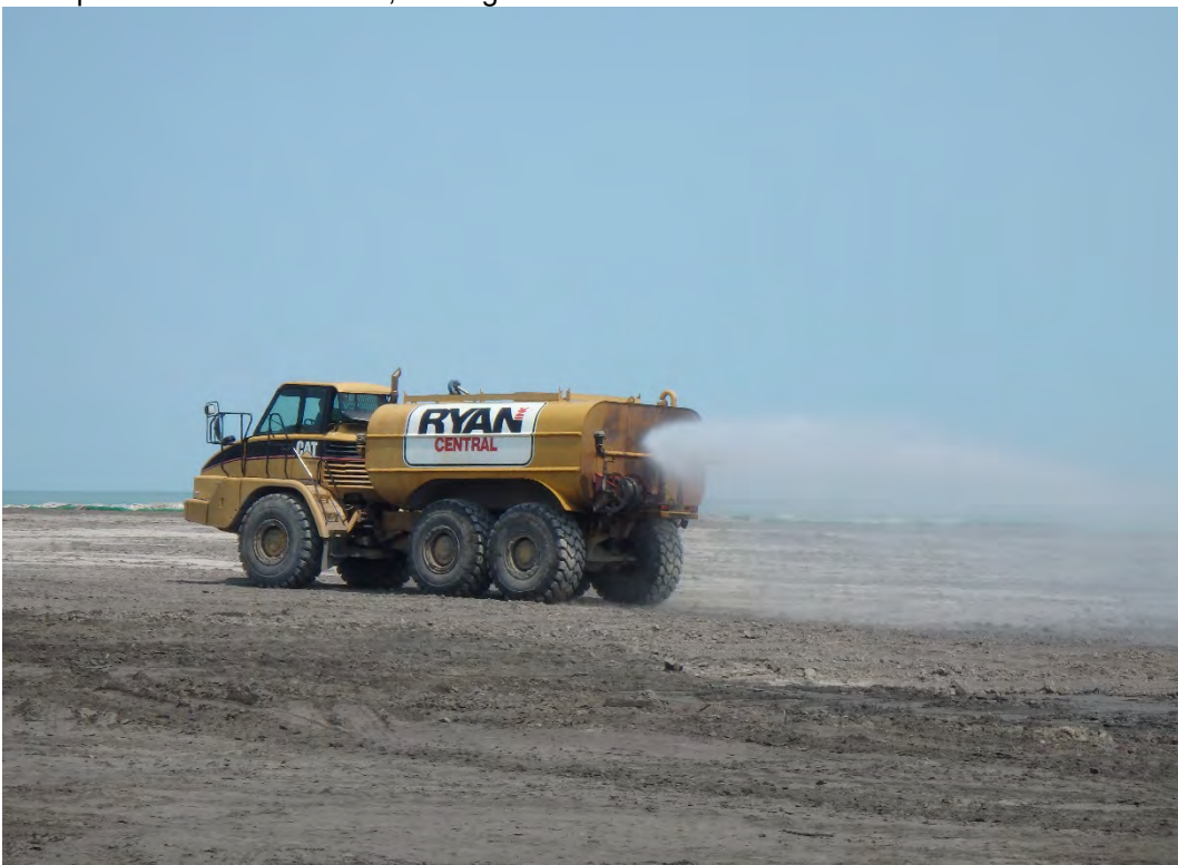
Dust control and maintaining moisture in placed structural fill, looking east.
