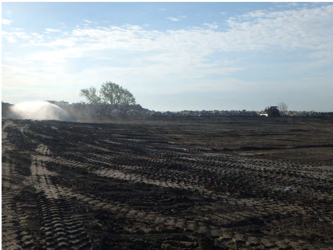
Dust control in Pond 1, looking east.
