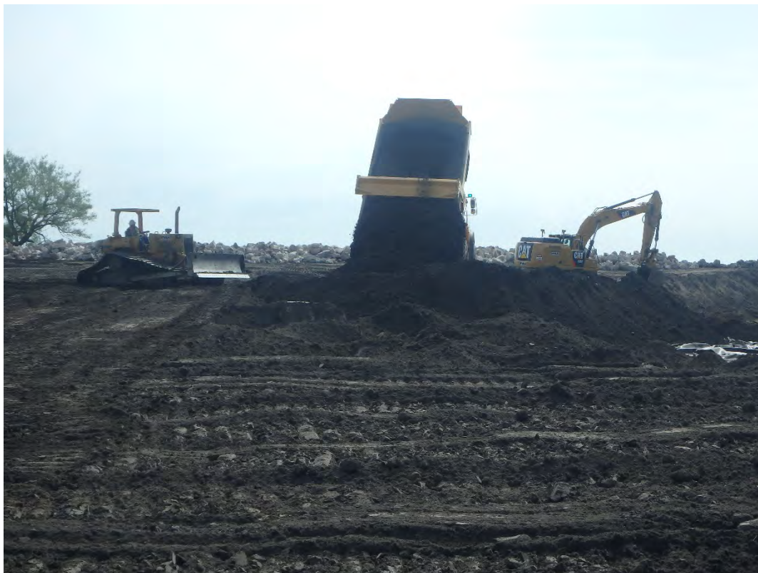
CCR regrading for bridging layer in Pond 1, looking east.
