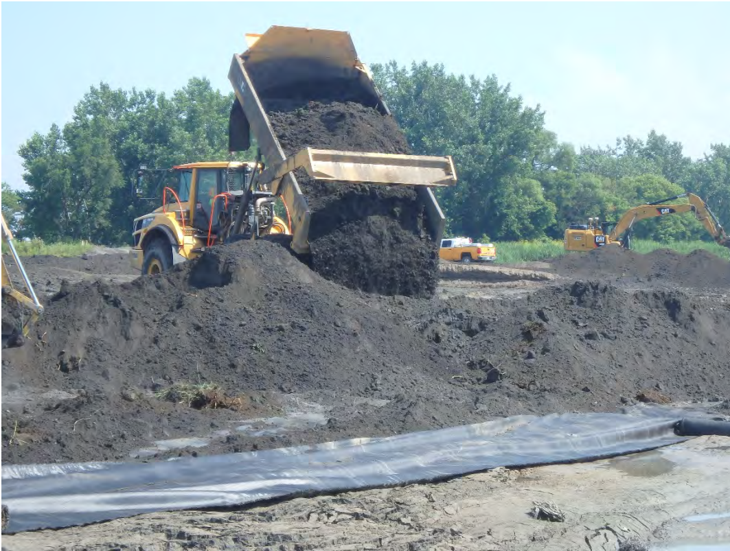
Bridging layer being placed in Pond 2, looking south.
