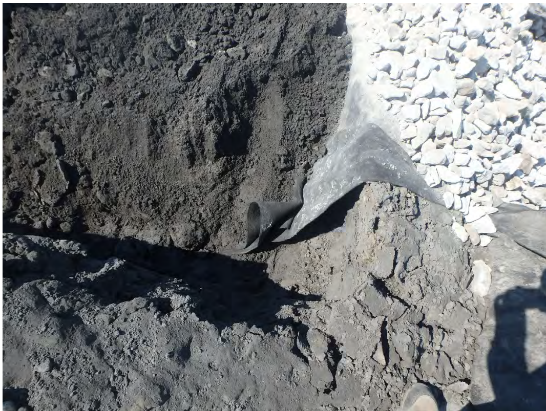
Shoreline geotextile in anchor trench with backfill.
