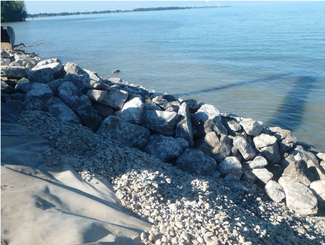
D50/30 inch riprap placed on shoreline southeast of Pond 2, looking northeast.
