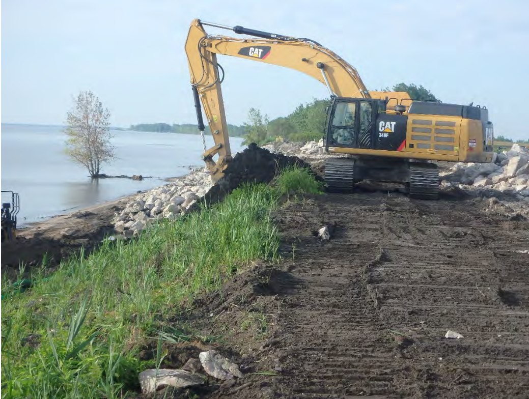
Clearing vegetation along shoreline, looking south.
