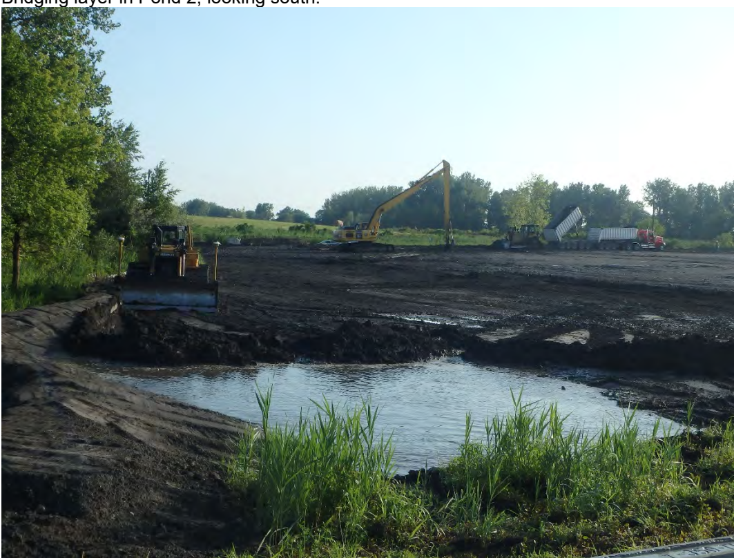
Charging standing water outside southwest corner of Pond 1, looking north.
