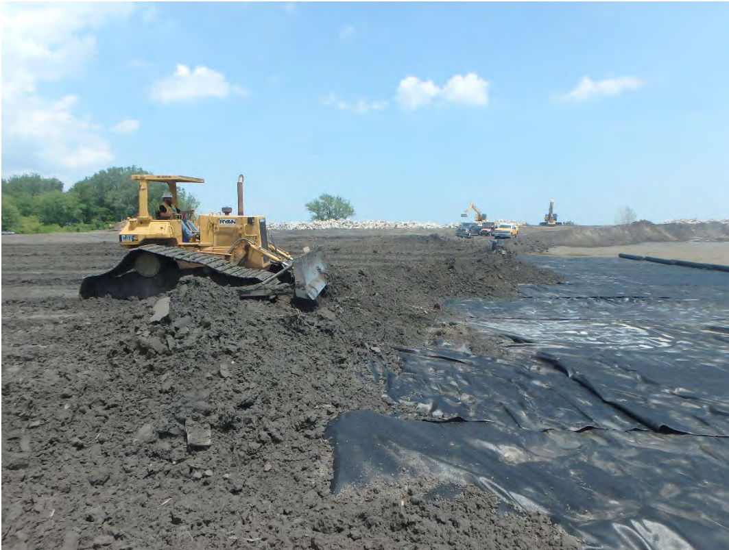
Placement of bridging layer above geotextile in Pond 1, looking east.
