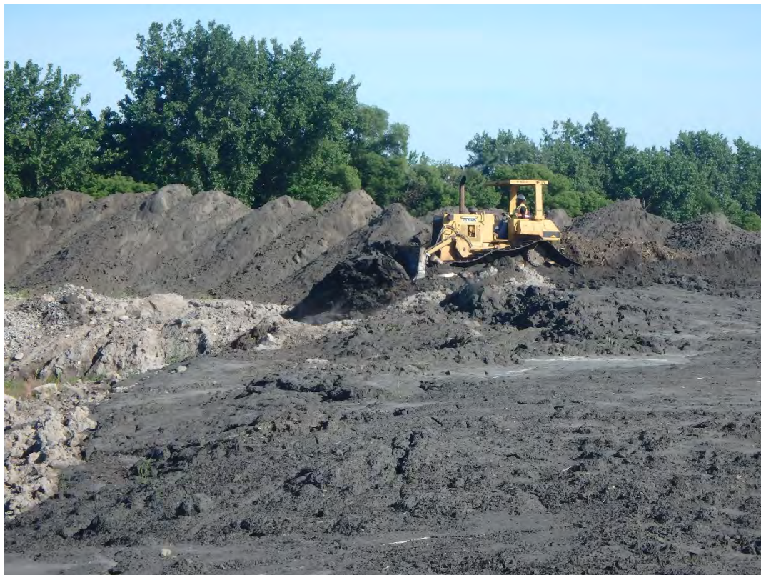
Placing bridging layer in Pond 2, looking south.
