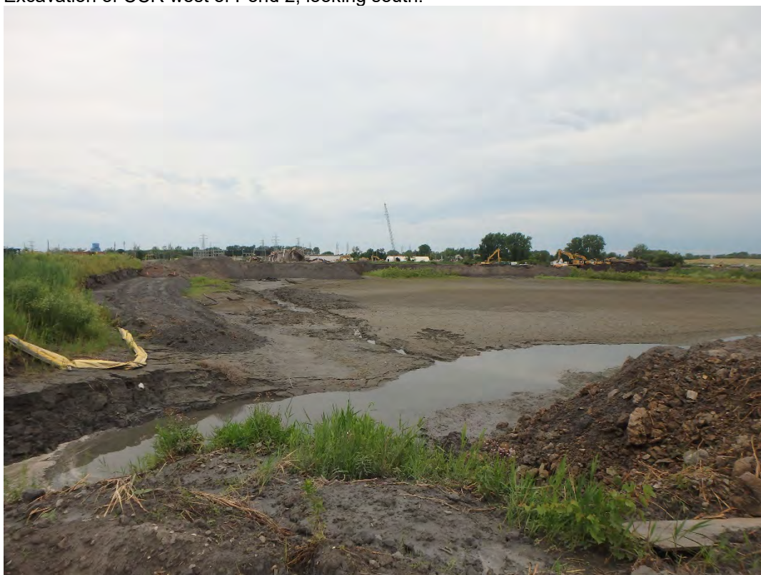
Overview of Pond 2, looking northwest.
