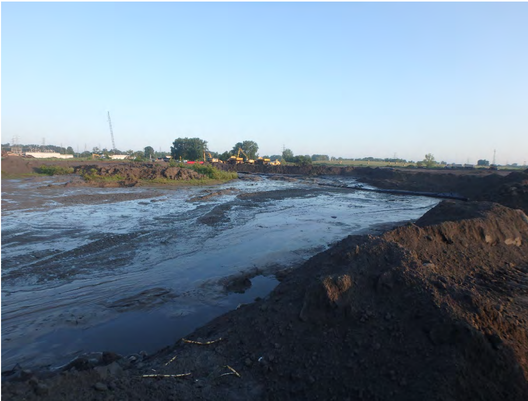
Overview of northeast corner of Pond 2, looking northwest.
