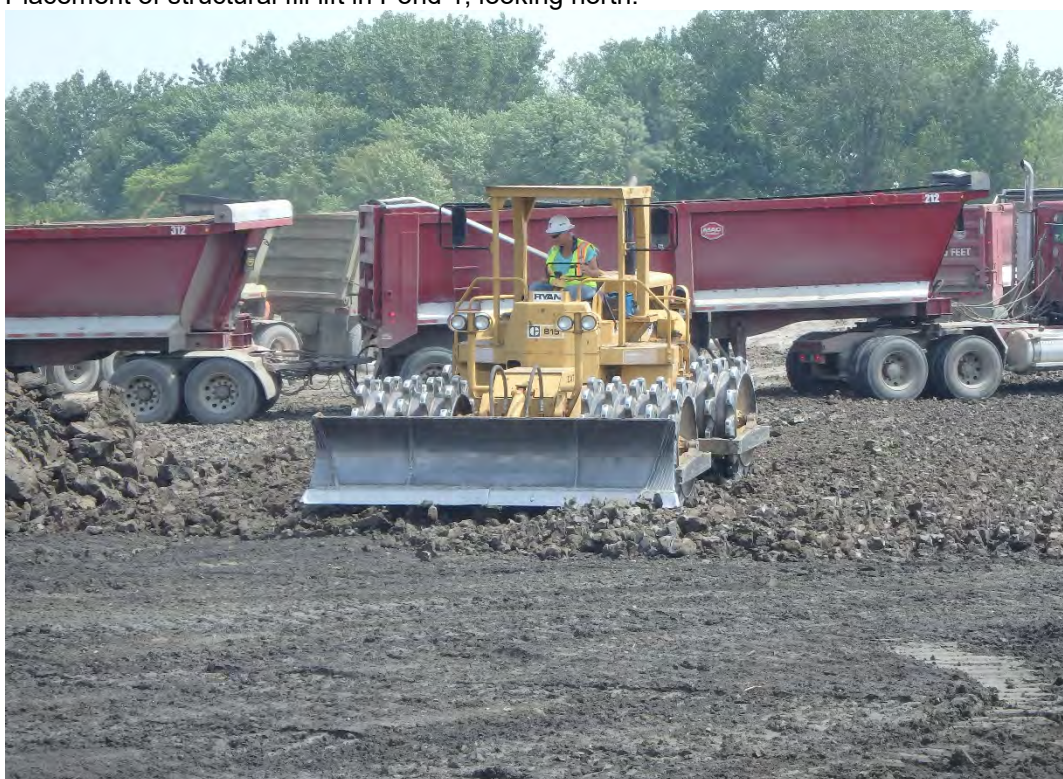
Compacting structural fill placed in Pond 1, looking northeast.
