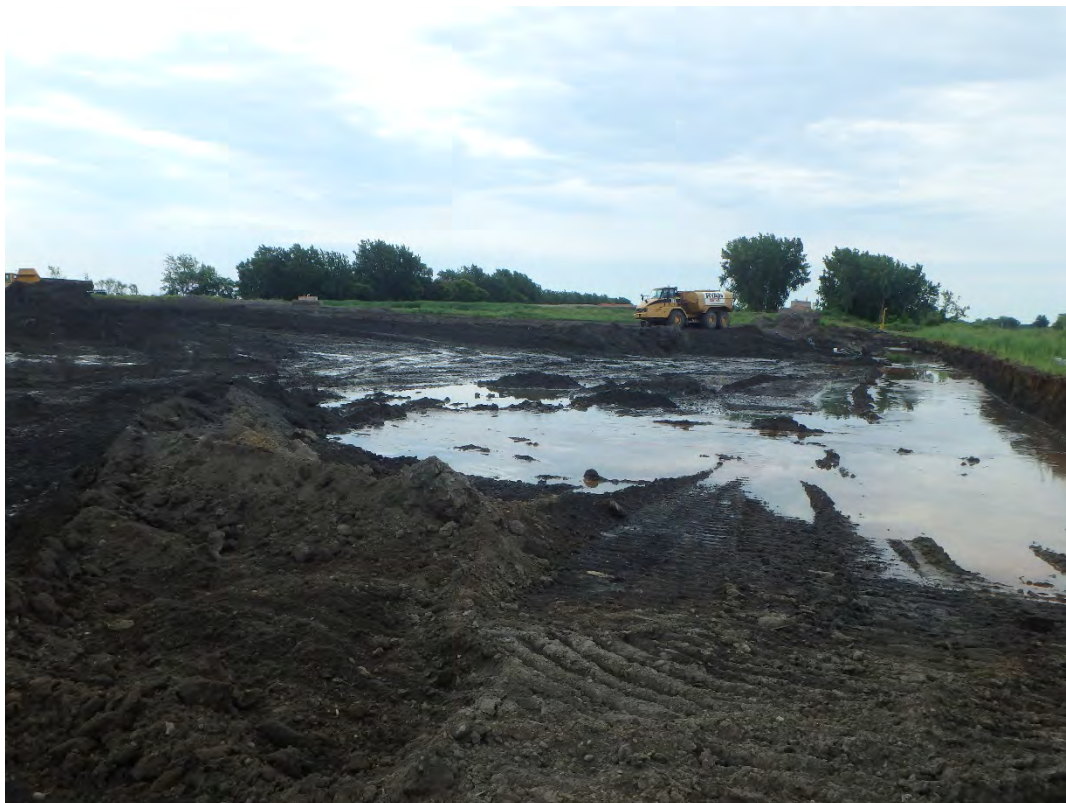
Excavation of CCR west of Pond 2, looking south.
