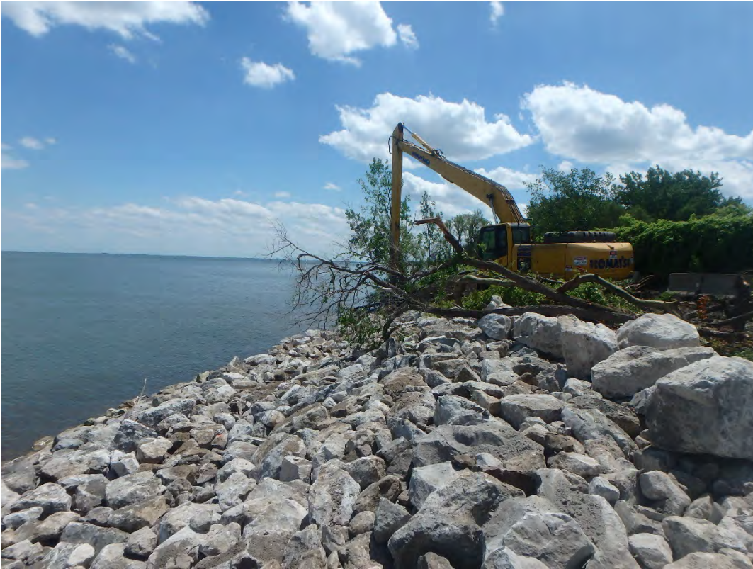
Clearing vegetation along shoreline southeast of Pond 2, looking south.
