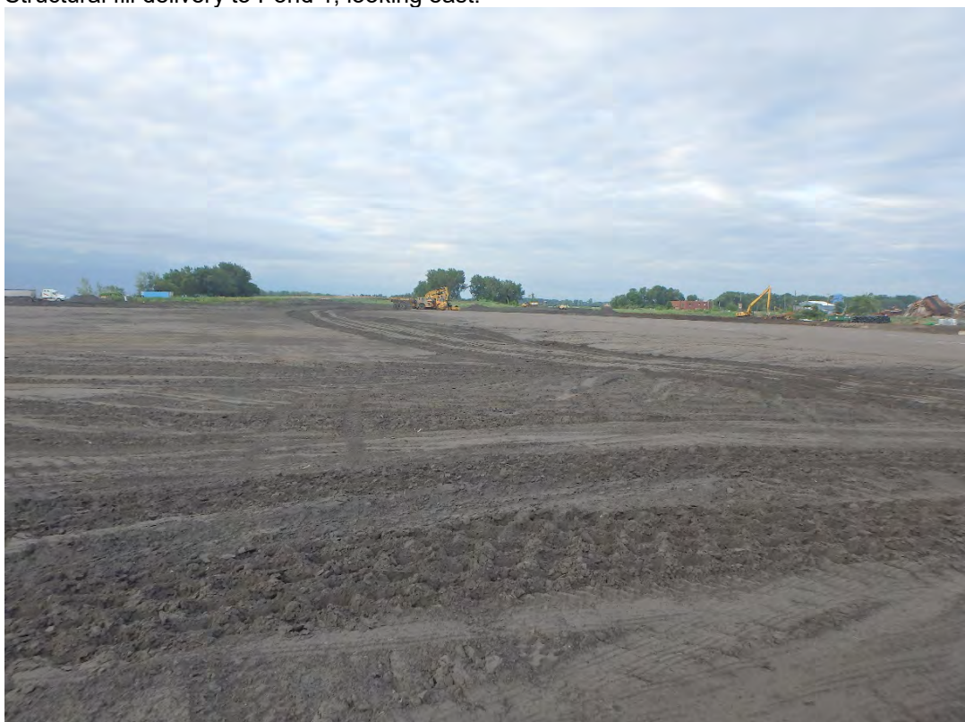
Overview of Pond 1 with single lift of structural fill, looking southwest.
