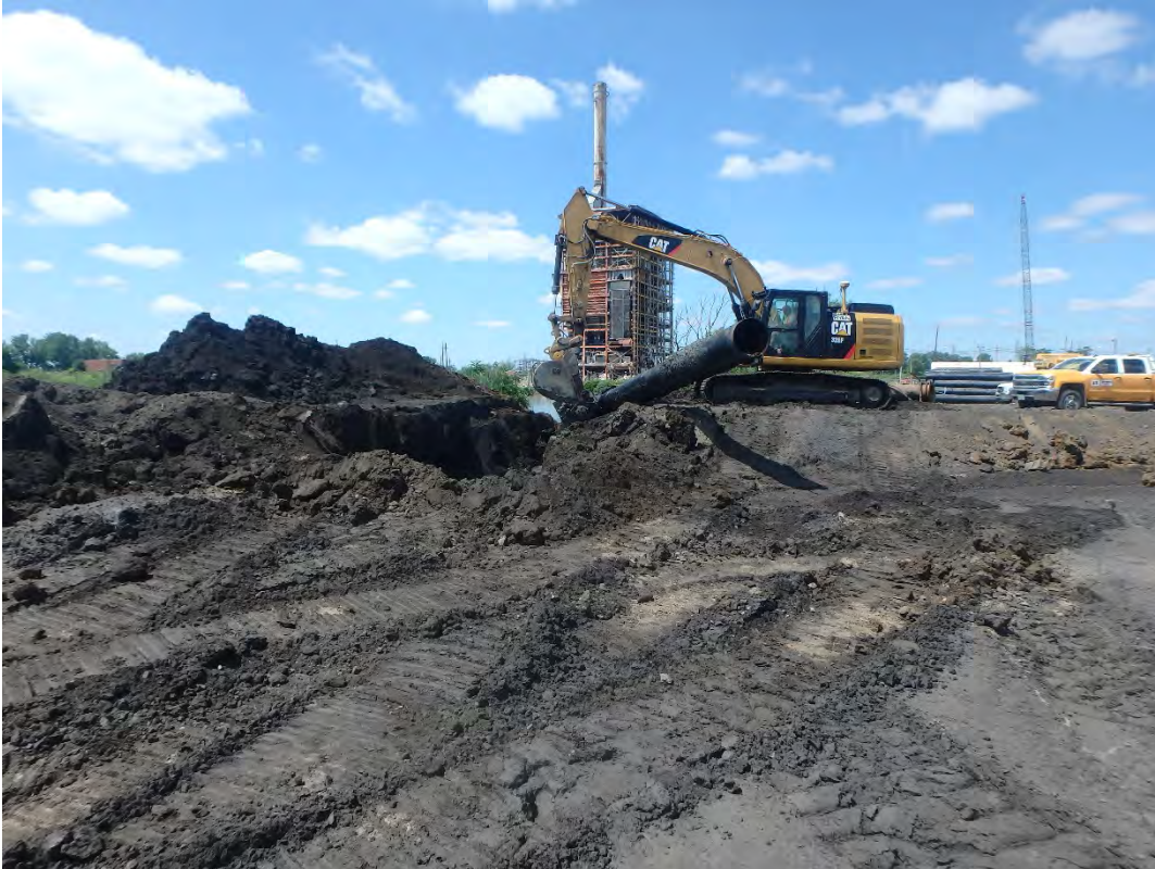
Removing standpipe running from Pond 1 to the Fore Bay, looking west.
