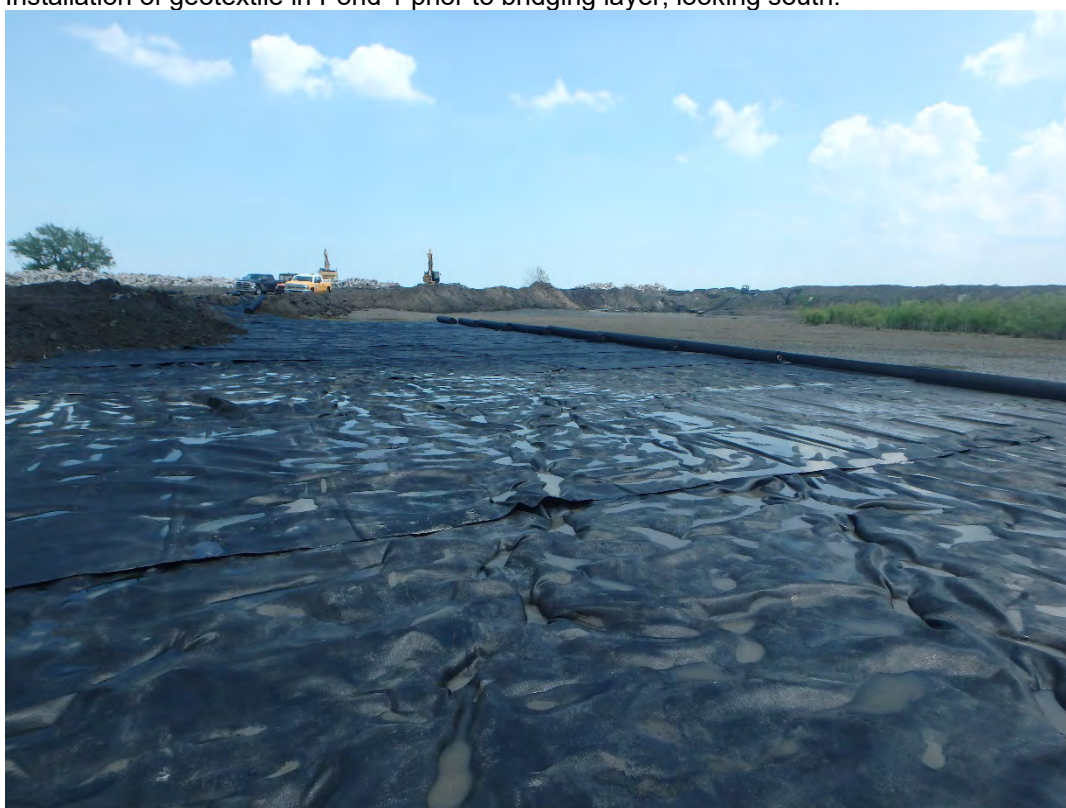
Geotextile installed across floor of Pond 1, looking east.
