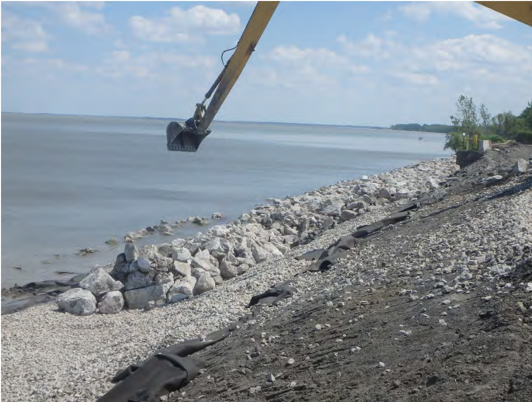
Placement of D50-30 inch riprap along shoreline, looking southeast.
