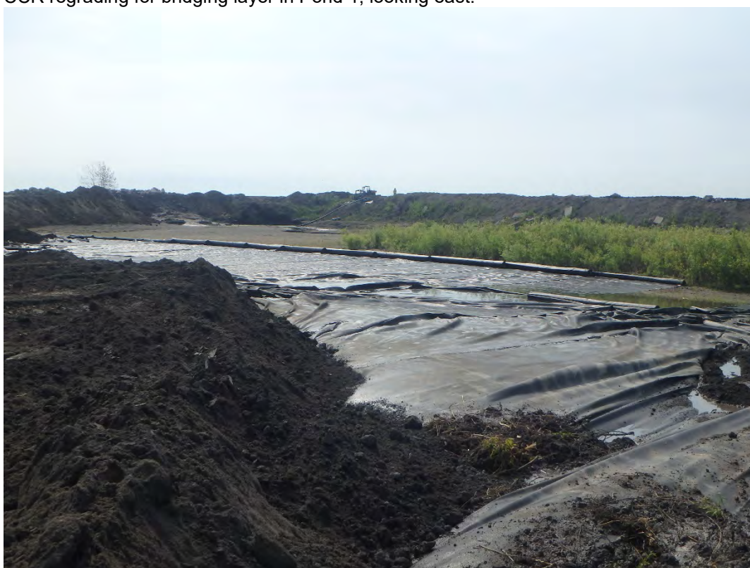
Textile deployed in Pond 1 for bridging layer, looking southeast.
