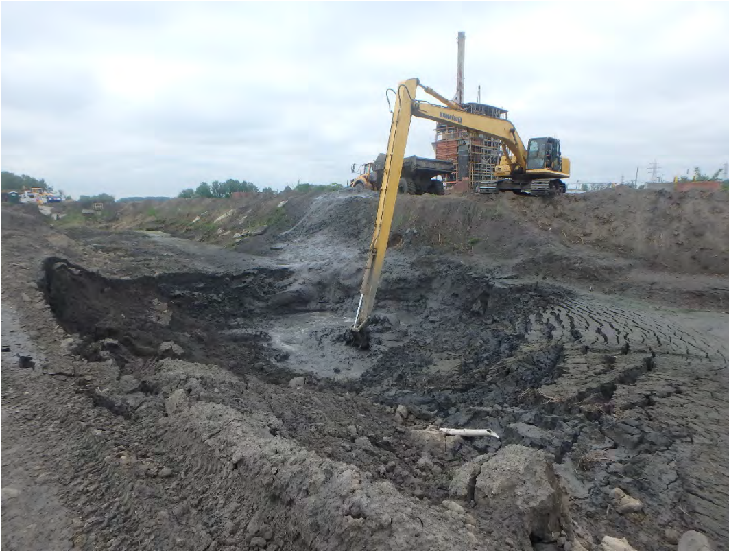
Over-Ex of saturated material from west side of Pond 1, looking south.
