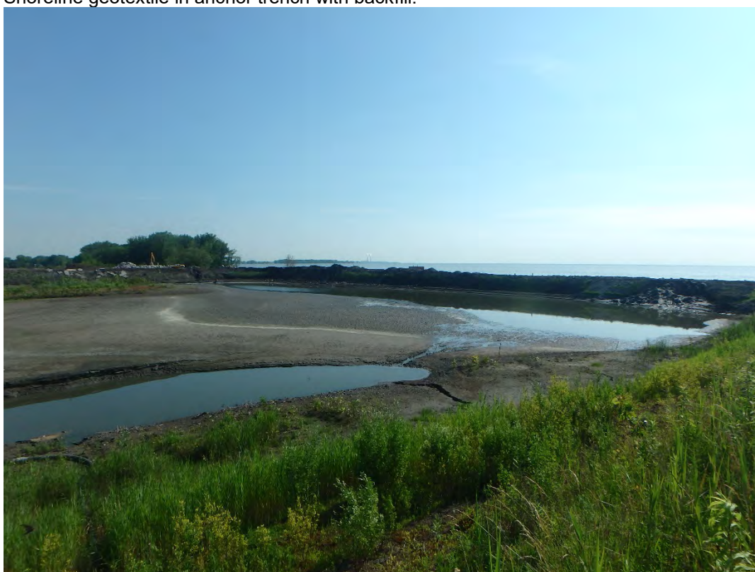
Overview and water level of Pond 2, looking northeast.
