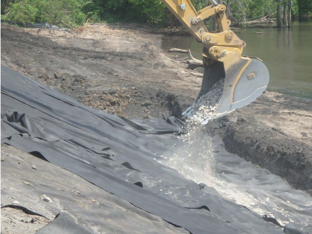
Placement of D50/2 inch cushion layer along shoreline, looking north.
