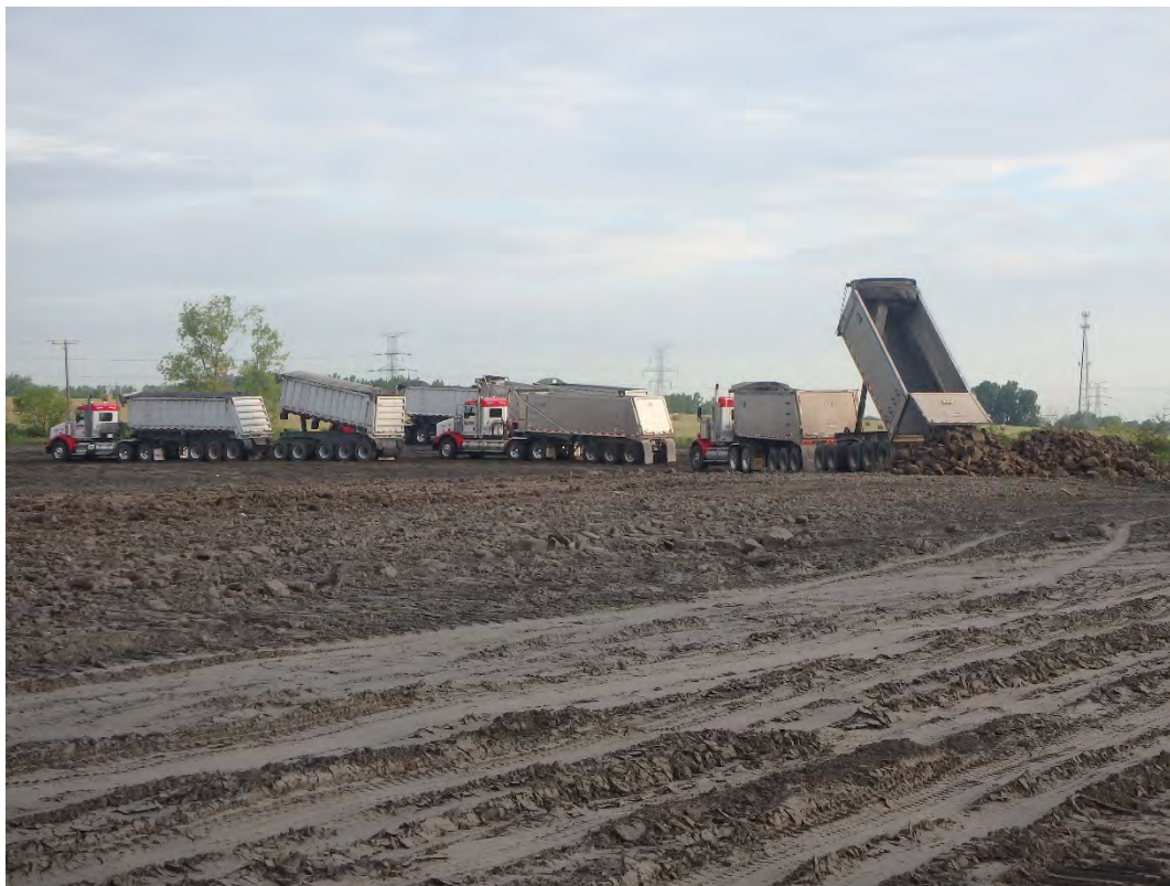
Delivery of structural fill to Pond 1, looking northwest.
