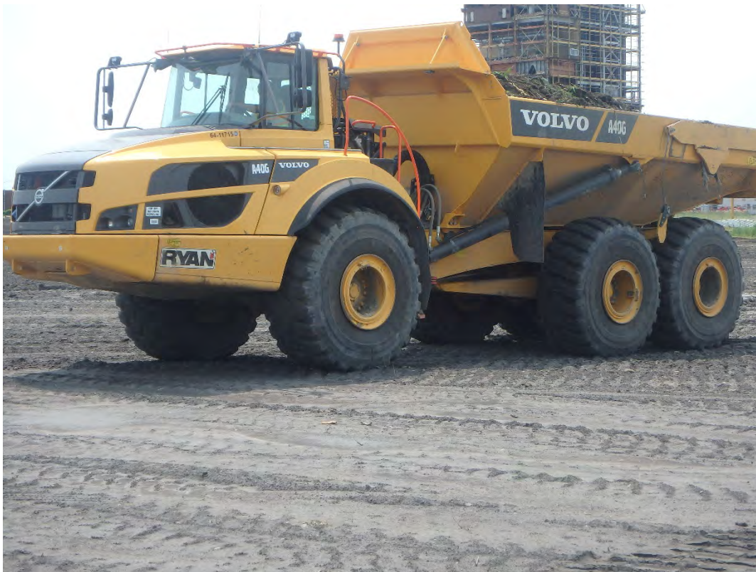
Proof roll in Pond 1 using loaded A40G haul truck, looking southwest.
