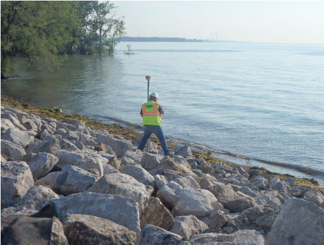
Ryan checking grade of riprap along shoreline, looking northeast.
