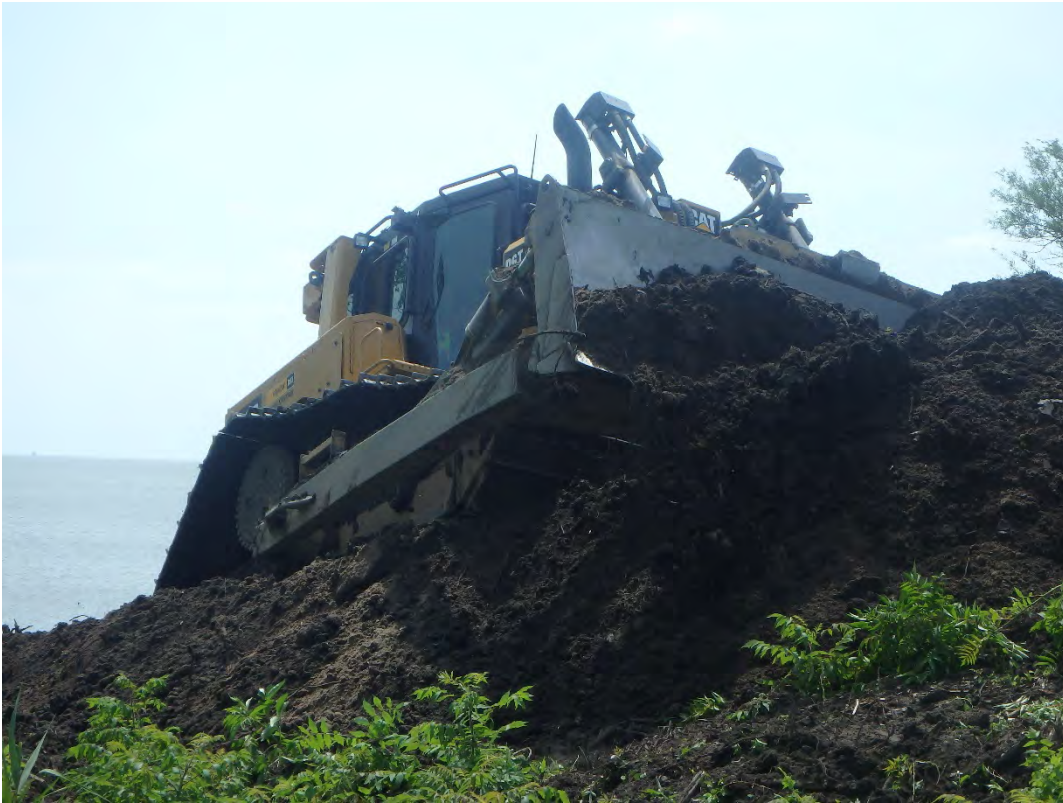
Cutting shoreline slope to sub-grade, looking east.
