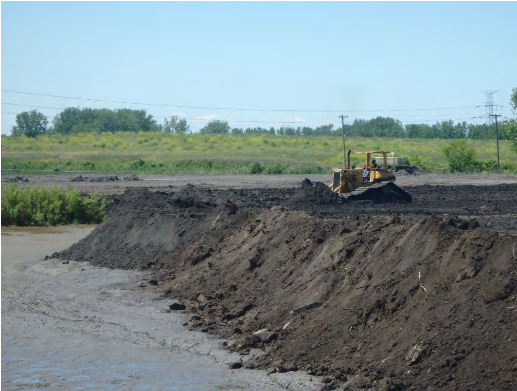
Placing bridging layer in Pond 1, looking north.
