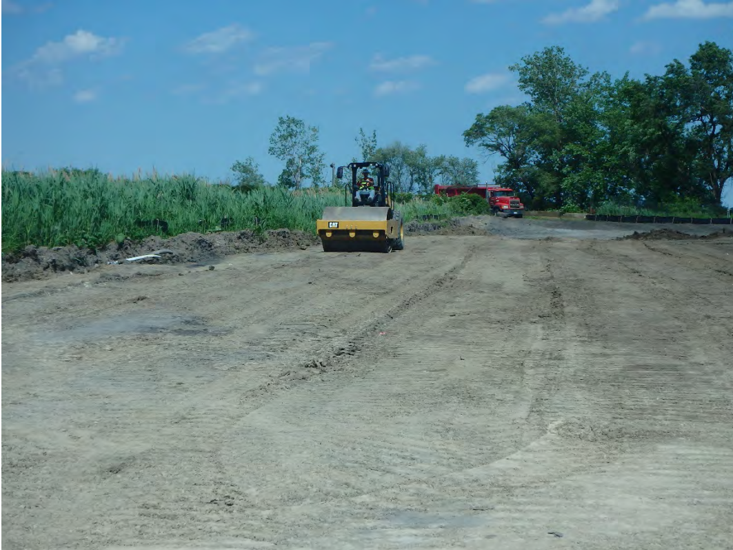
Compaction of placed structural fill at chemical ponds, looking east.
