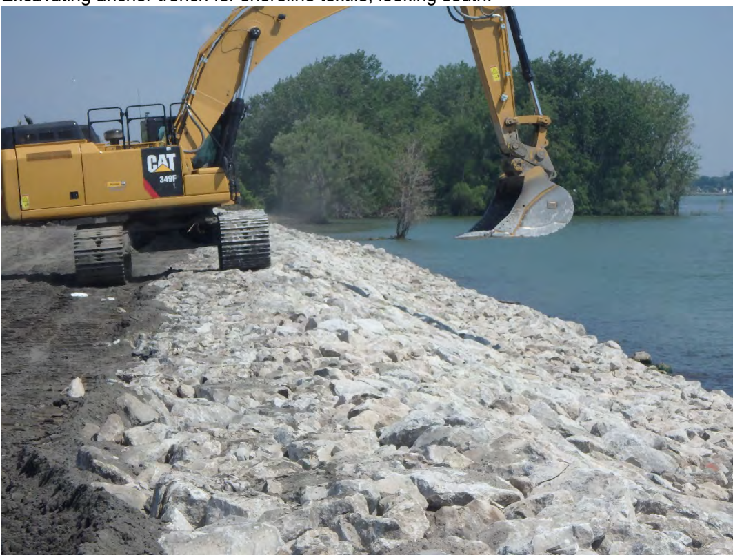
Filling voids in shoreline riprap using 8x16 inch riprap, looking north.
