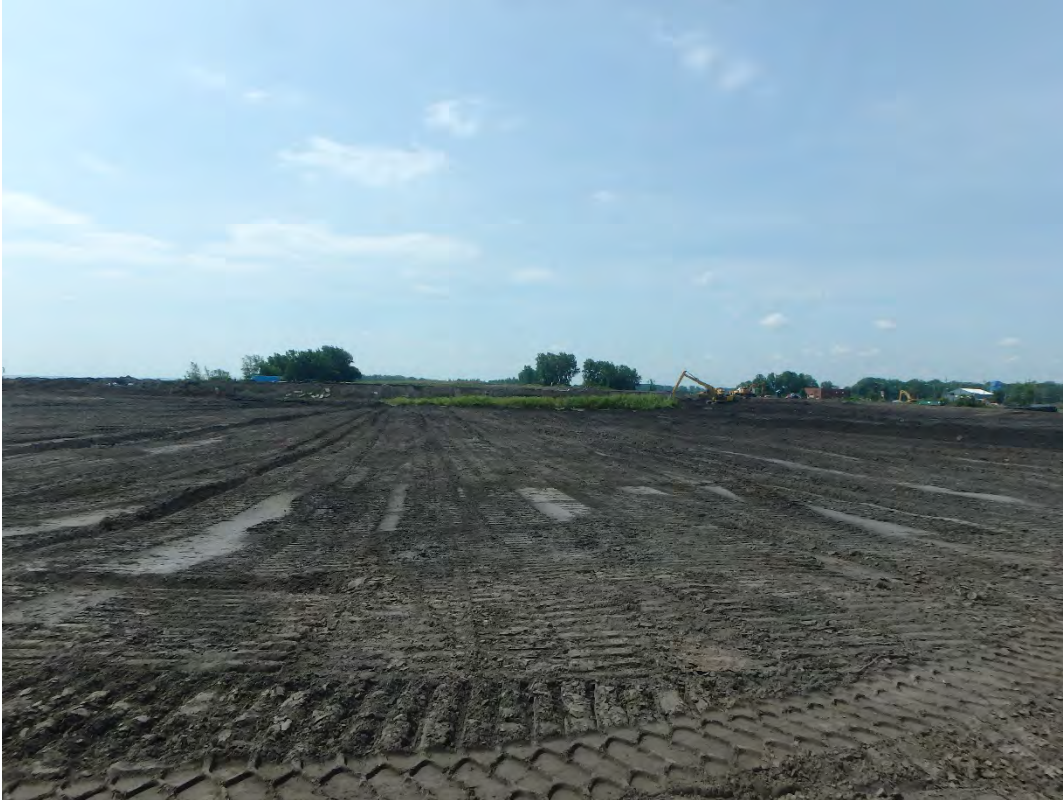
Overview of bridging layer in Pond 1, looking south.
