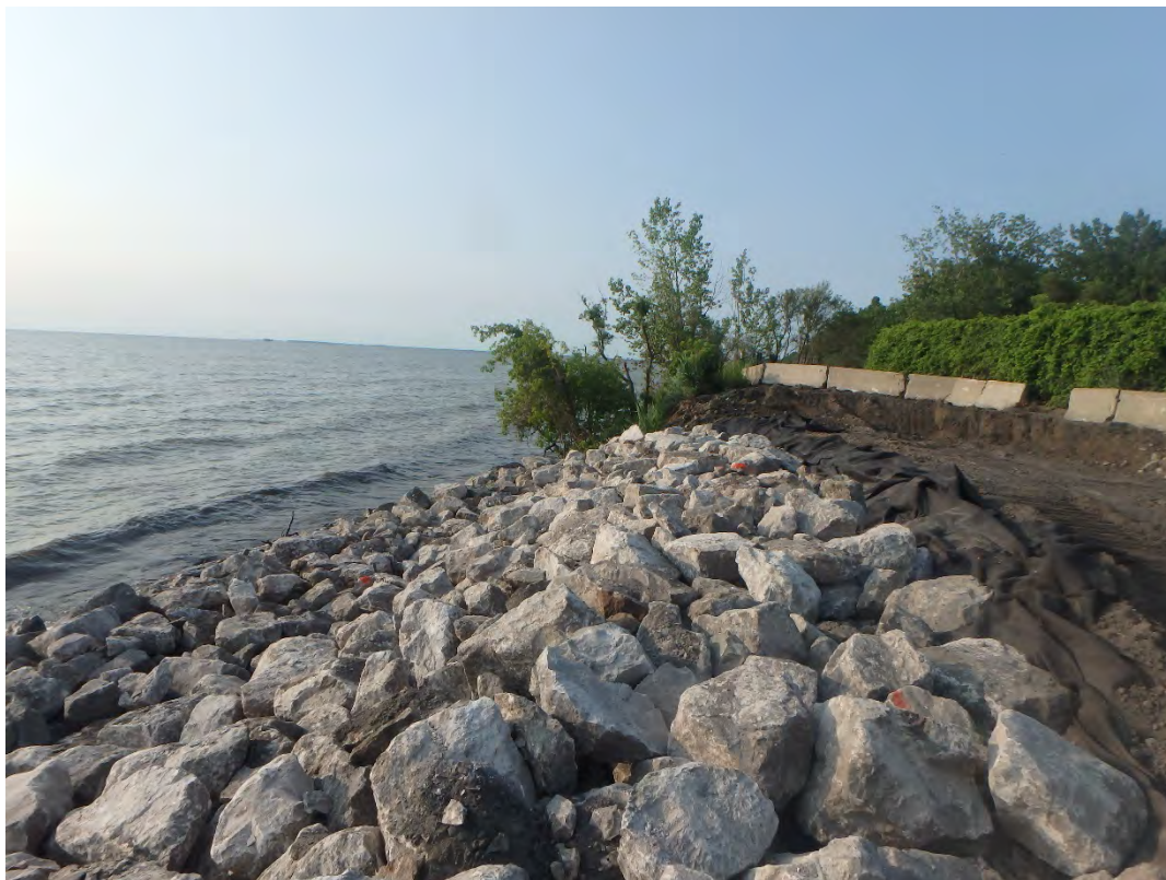
South end of shoreline riprap, looking south.
