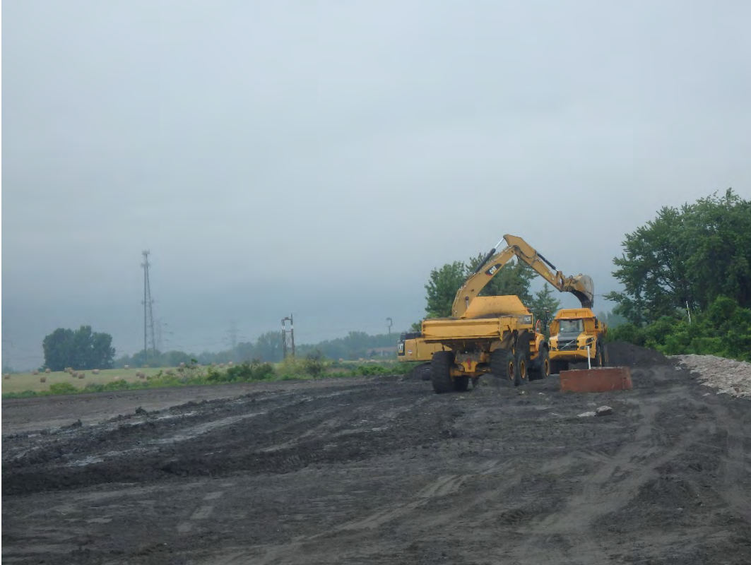
Excavating perimeter road east of Pond 1 down to sub-grade, looking north.
