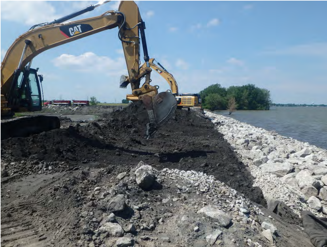
Excavating access road east of Pond 2 down to sub-grade, looking north.
