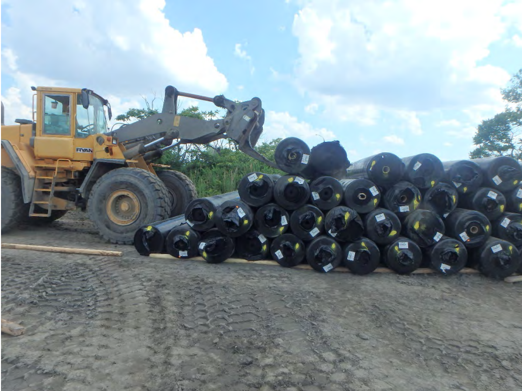
Off-loading of 8 oz. geotextile, looking south.
