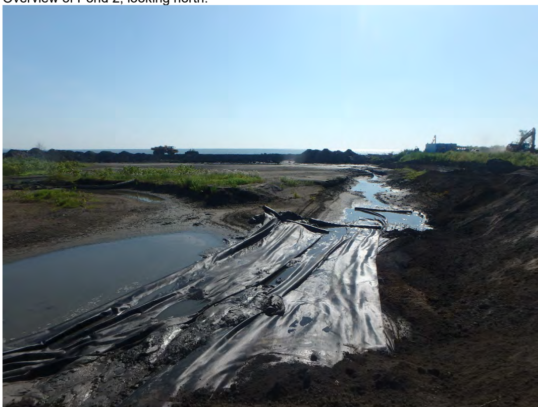
Textile for bridging layer deployed in Pond 2, looking east.
