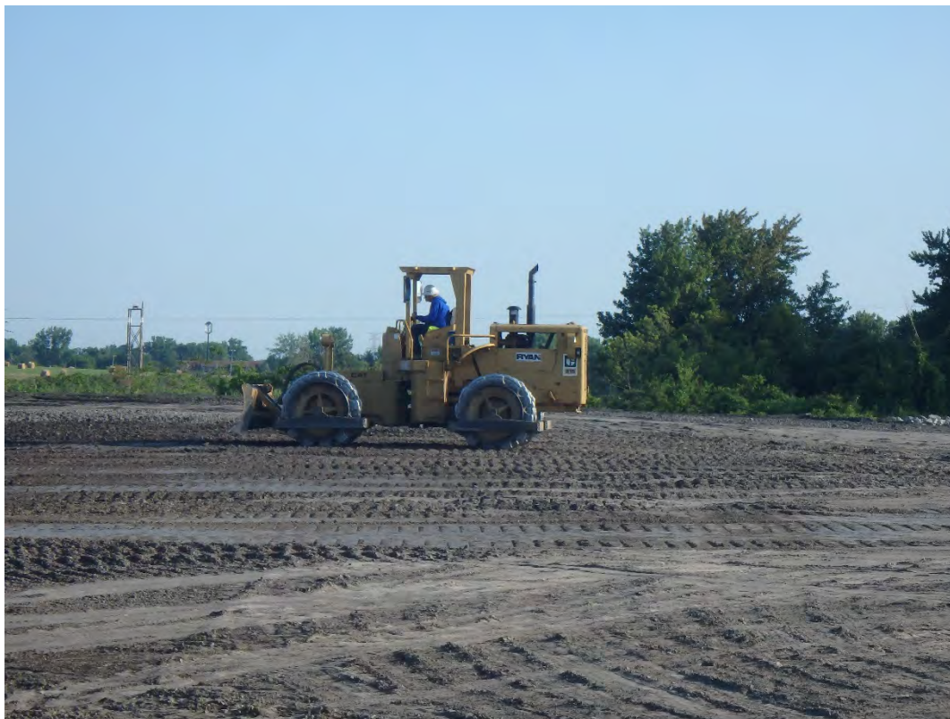
815 compacting placed structural fill in Pond 1, looking north.
