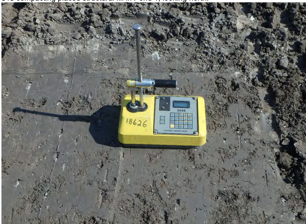
Density testing of compacted structural fill in Pond 1.
