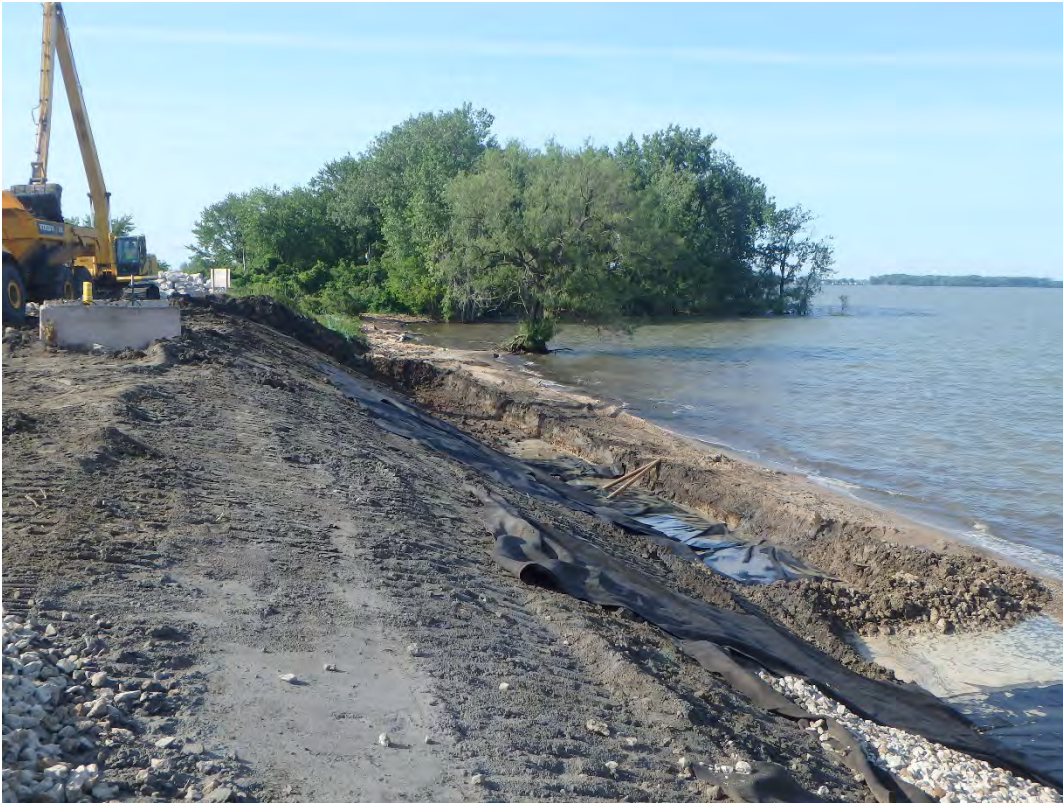
Cutting shoreline for installation of riprap, looking north.
