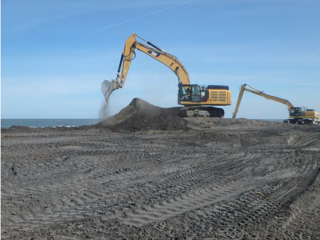
Excavating of Pond 1's east perimeter road, looking southeast.
