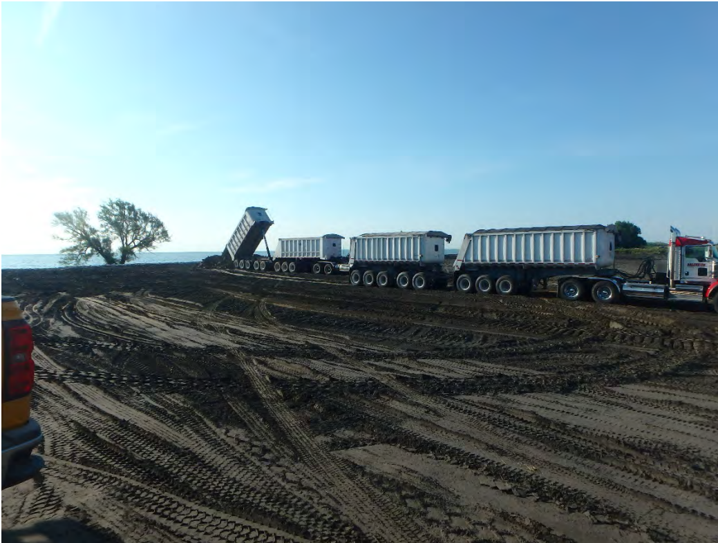
Structural fill delivered to Pond 1 by road trains, looking east.
