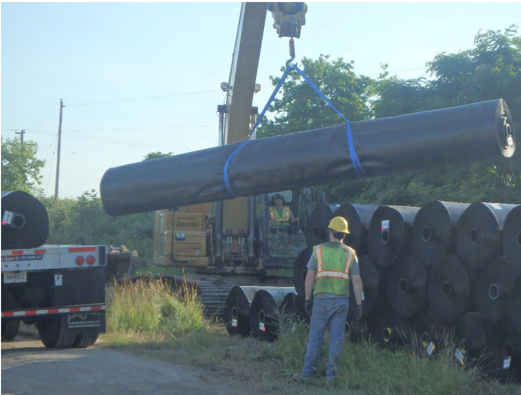
Off-loading 40mil geomembrane, looking north.
