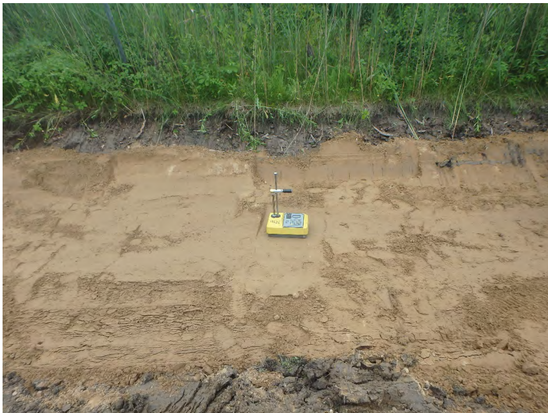
Testing of compacted pipe bedding for culvert.
