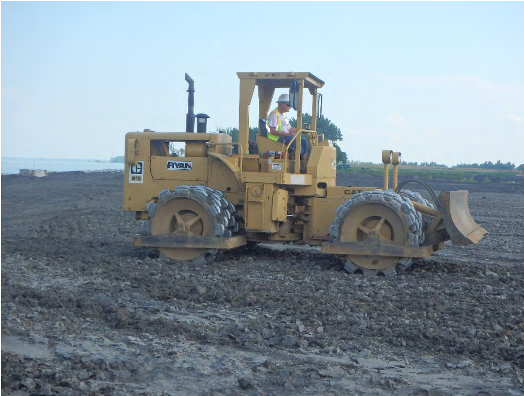
Compacting first lift of structural fill placed in Pond 1, looking south.
