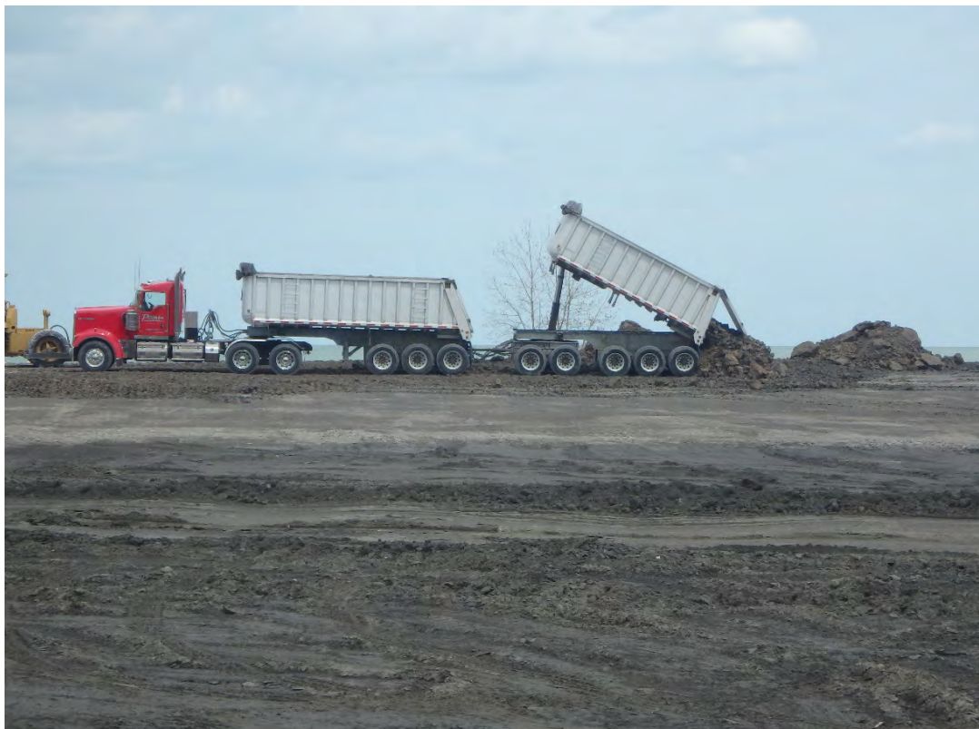
Structural fill delivery to Pond 1, looking east.
