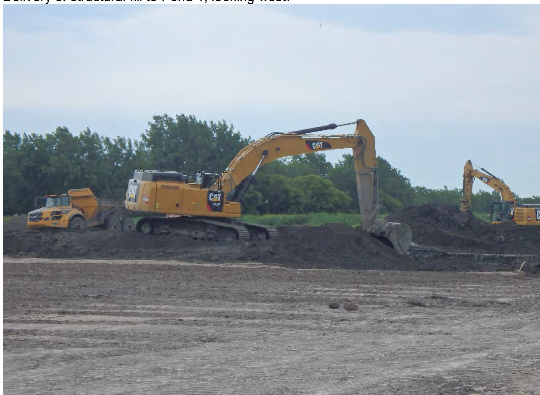
Excavation of dyke between Ponds 1 and 2, looking south.
