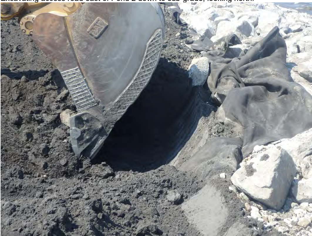
Excavating anchor trench for shoreline geotextile, looking north.
