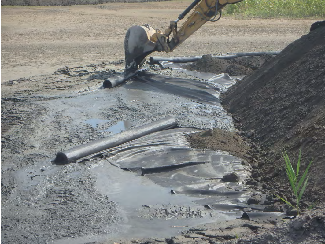
Deploying textile for bridging layer in Pond 2.
