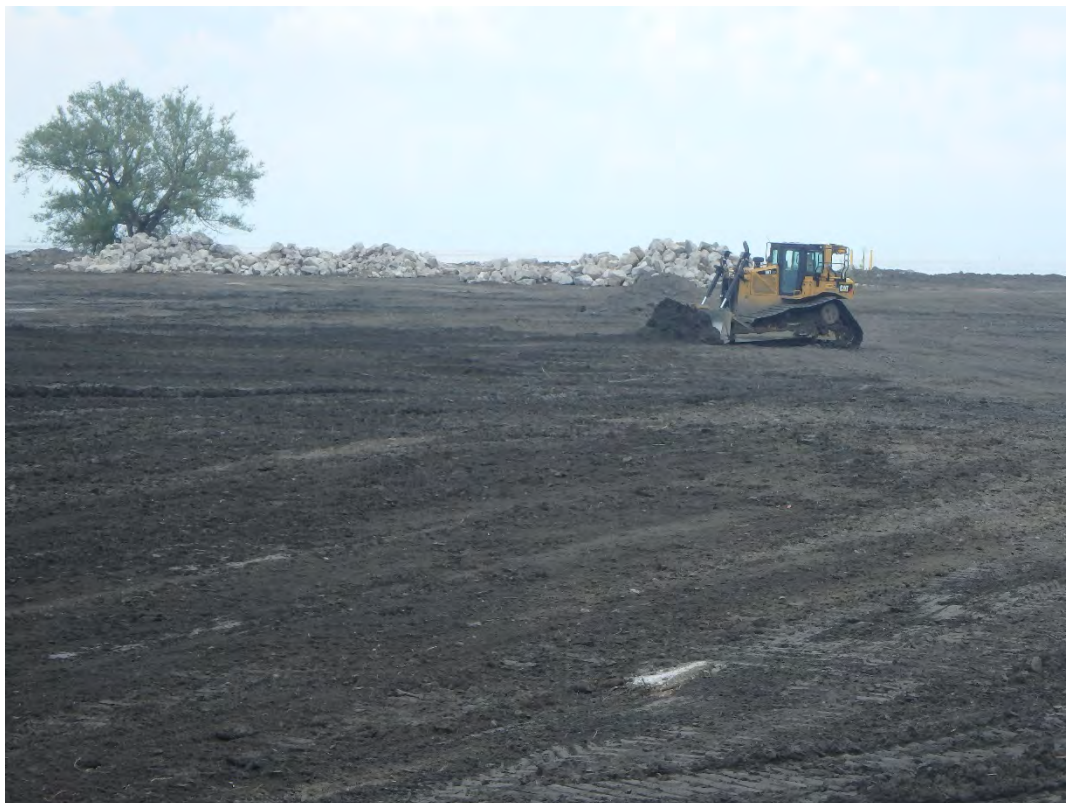
Pond 1 bridging layer being placed, looking east.
