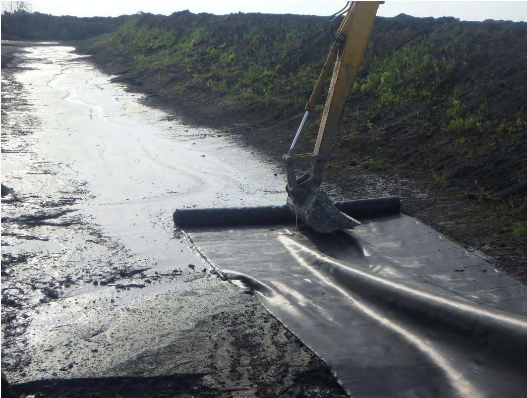
Installation of geotextile in Pond 1 prior to bridging layer, looking east.
