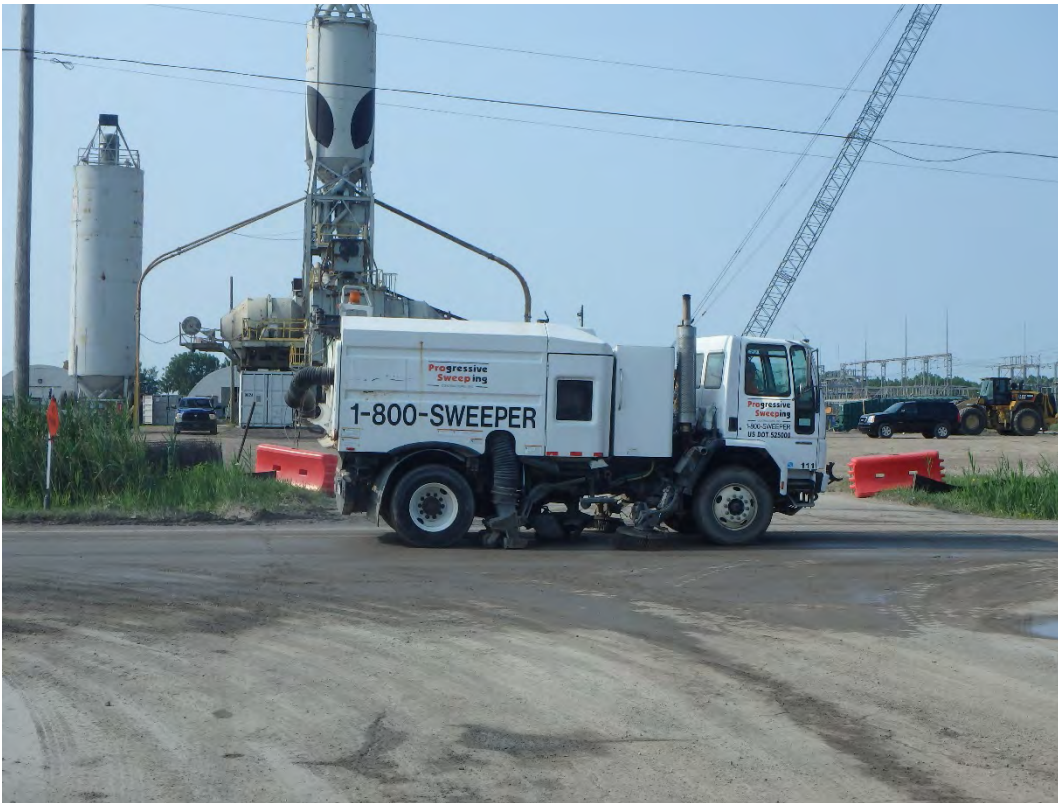
Sweeper to maintain Erie Rd., looking south.
