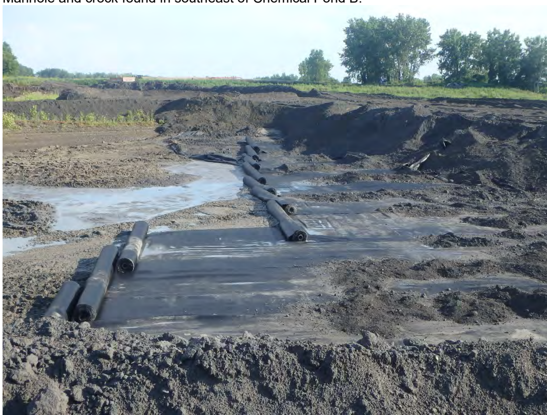
Textile for bridging layer deployed in Pond 2, looking south.
