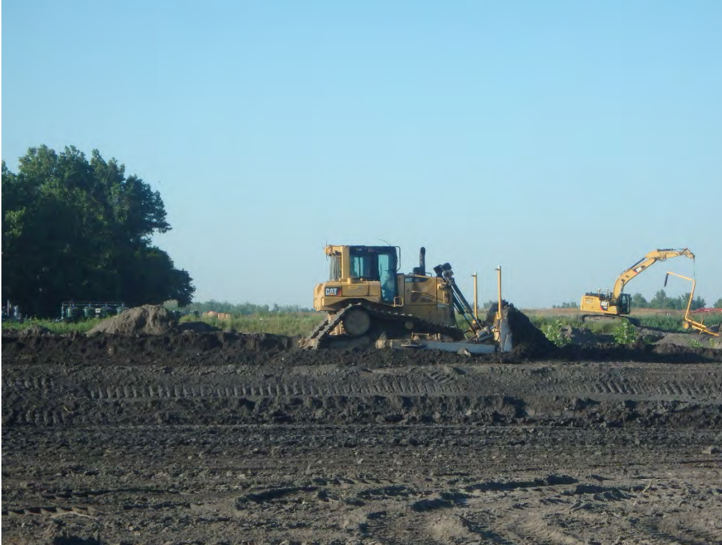
Placement of CCR for bridging layer in Pond 2, looking southwest.
