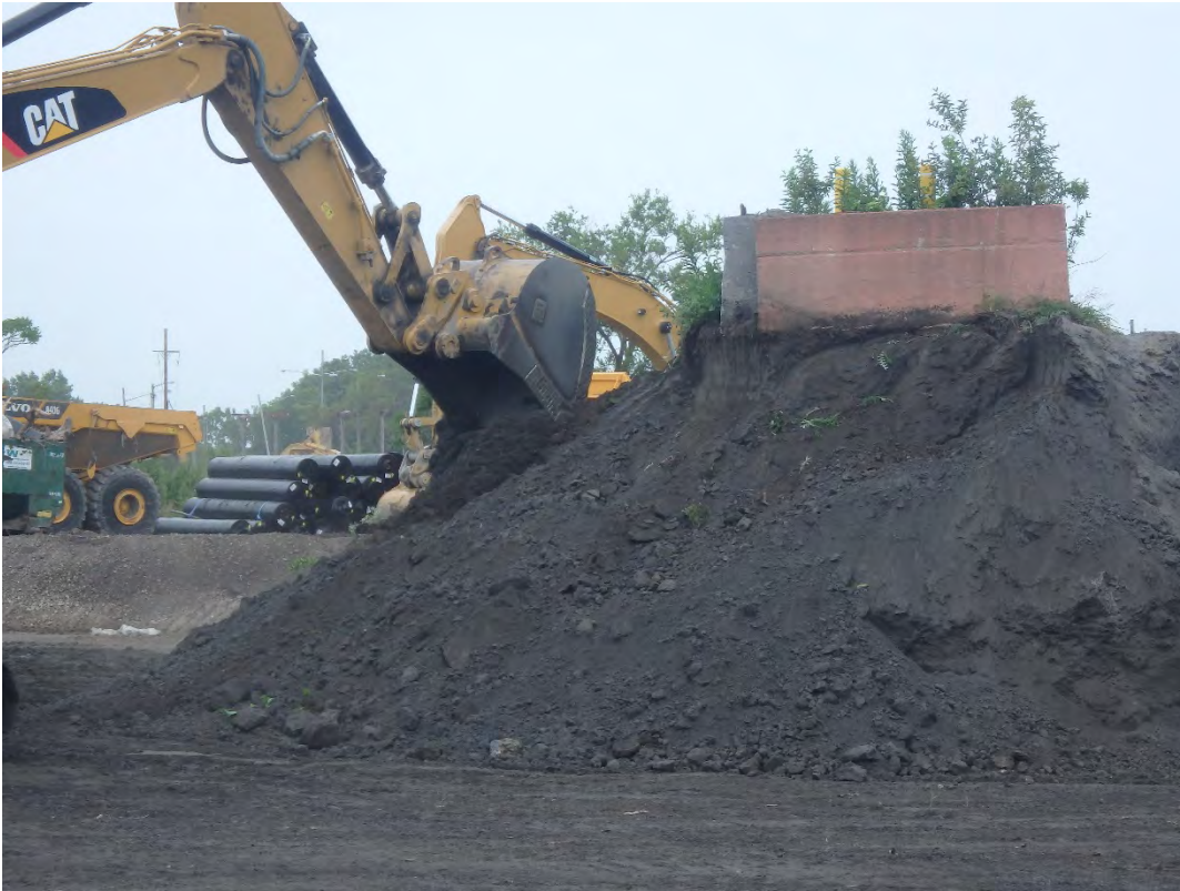
Excavating around MW-15001 prior to removing jersey barriers, looking southwest.
