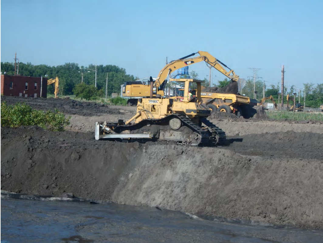
Placing bridging layer in Pond 2, looking southwest.
