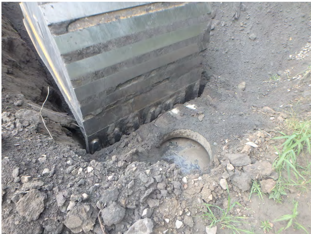
Manhole and crock found in southeast of Chemical Pond B.
