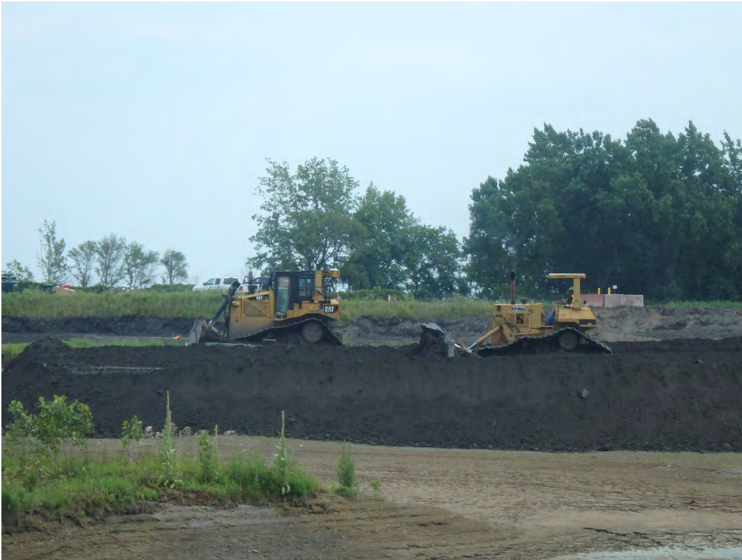
Placing bridging layer in Pond 2, looking south.
