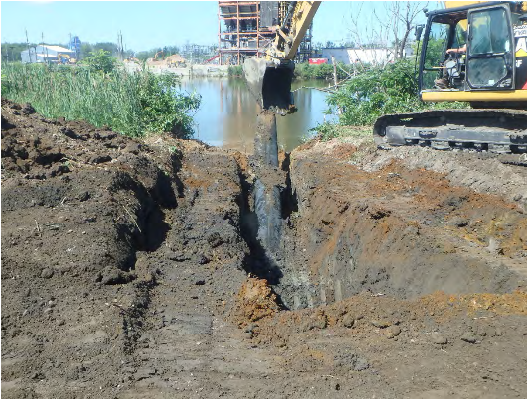
Removing standpipe into Fore Bay from Pond 1, looking west.
