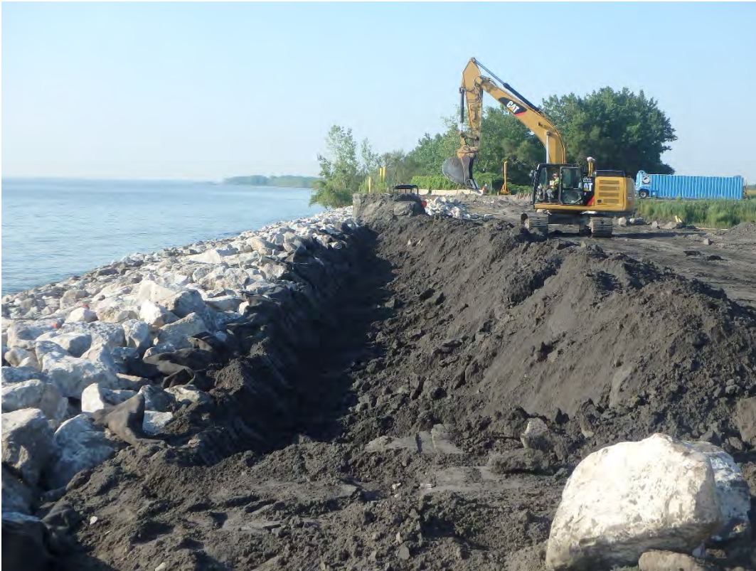
Excavating anchor trench for shoreline textile, looking south.
