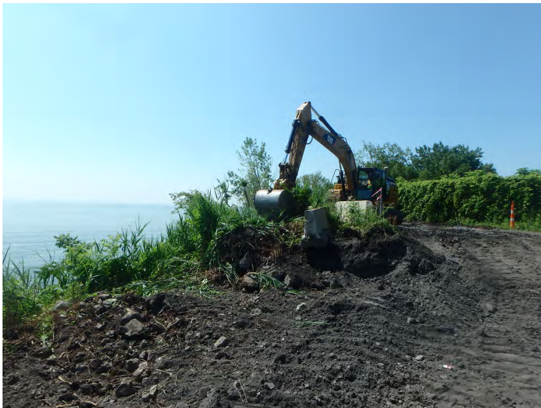
Clearing vegetation from shoreline east of Pond 2, looking south.
