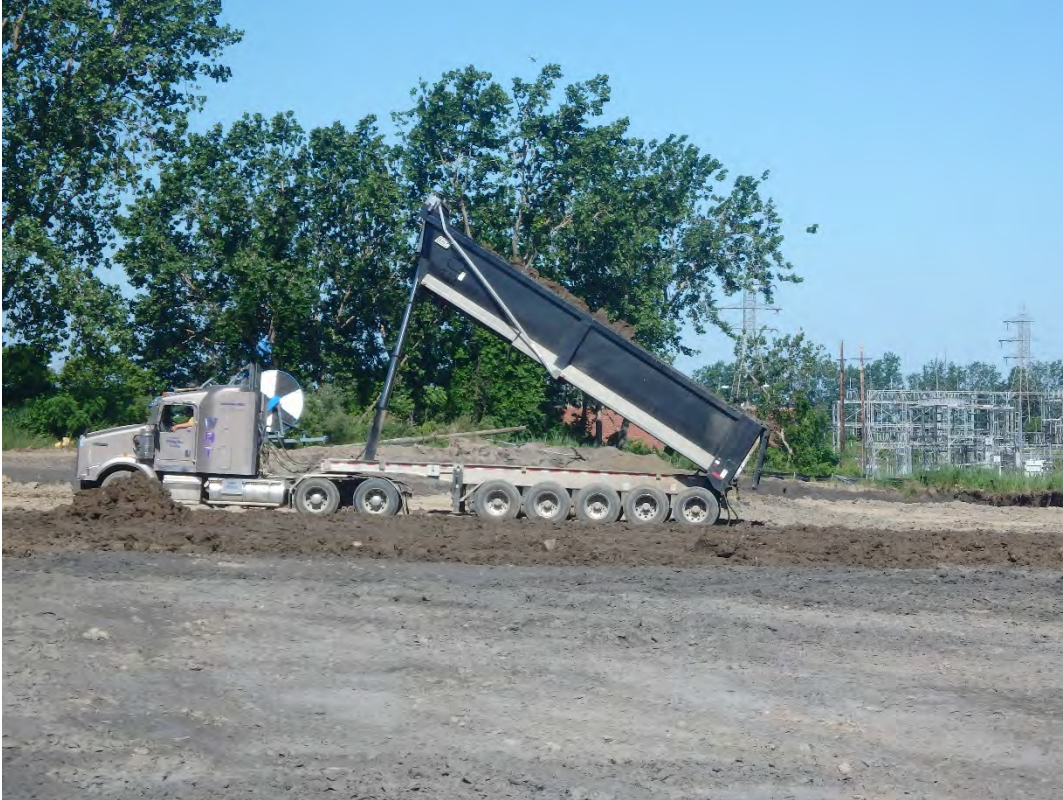
Structural fill hauled to chemical ponds, looking southeast.
