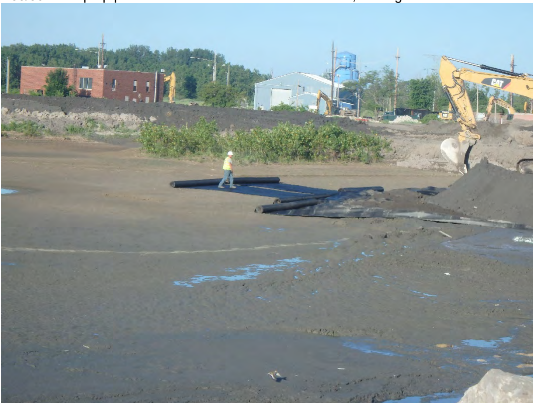
Deploying textile for bridging layer in Pond 2.
