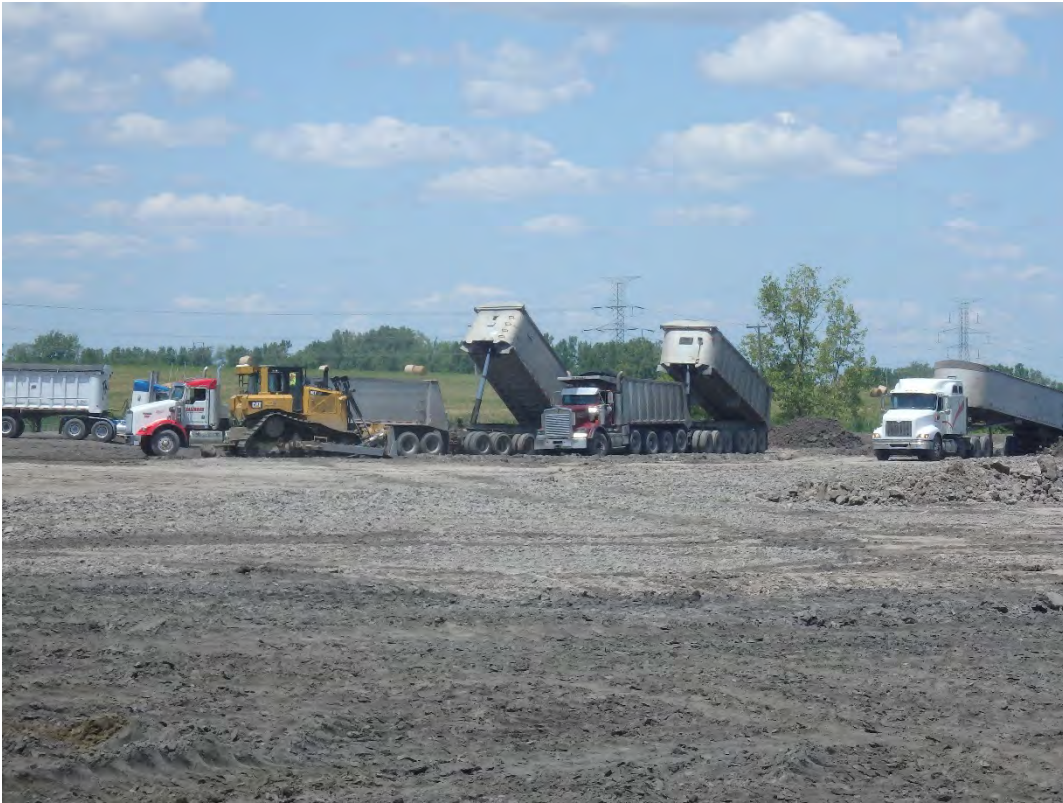
Structural fill import and placement in Pond 1, looking northeast.
