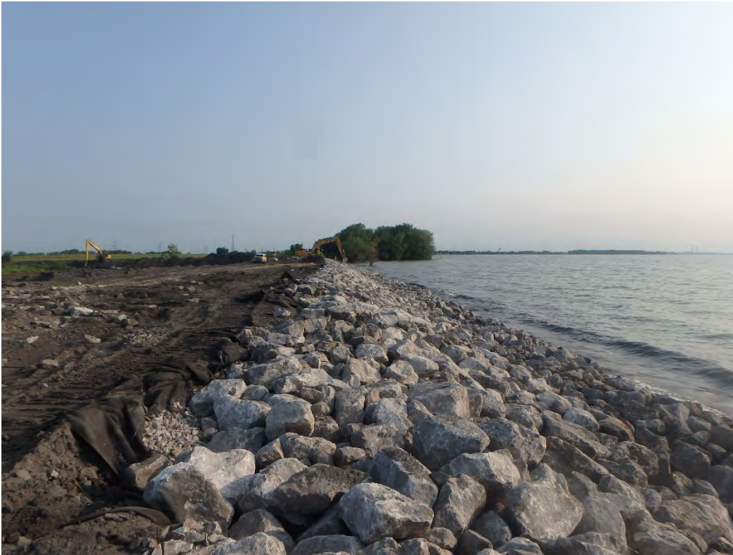
Overview of shoreline riprap, looking north.
