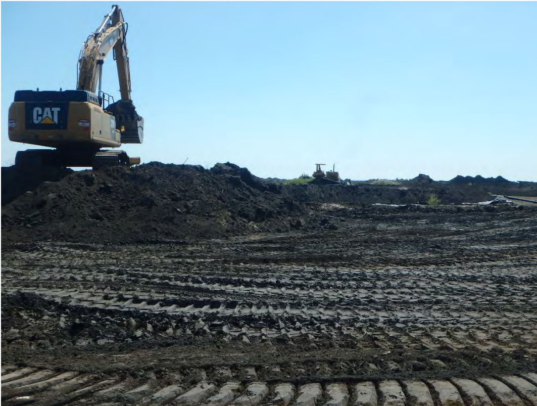
Excavation of dyke between Pond's 1 and 2, looking east.
