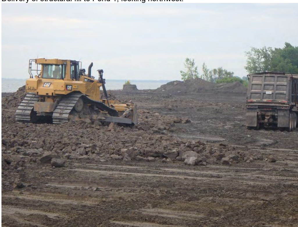
Placing lift of structural fill in Pond 1, looking southeast.
