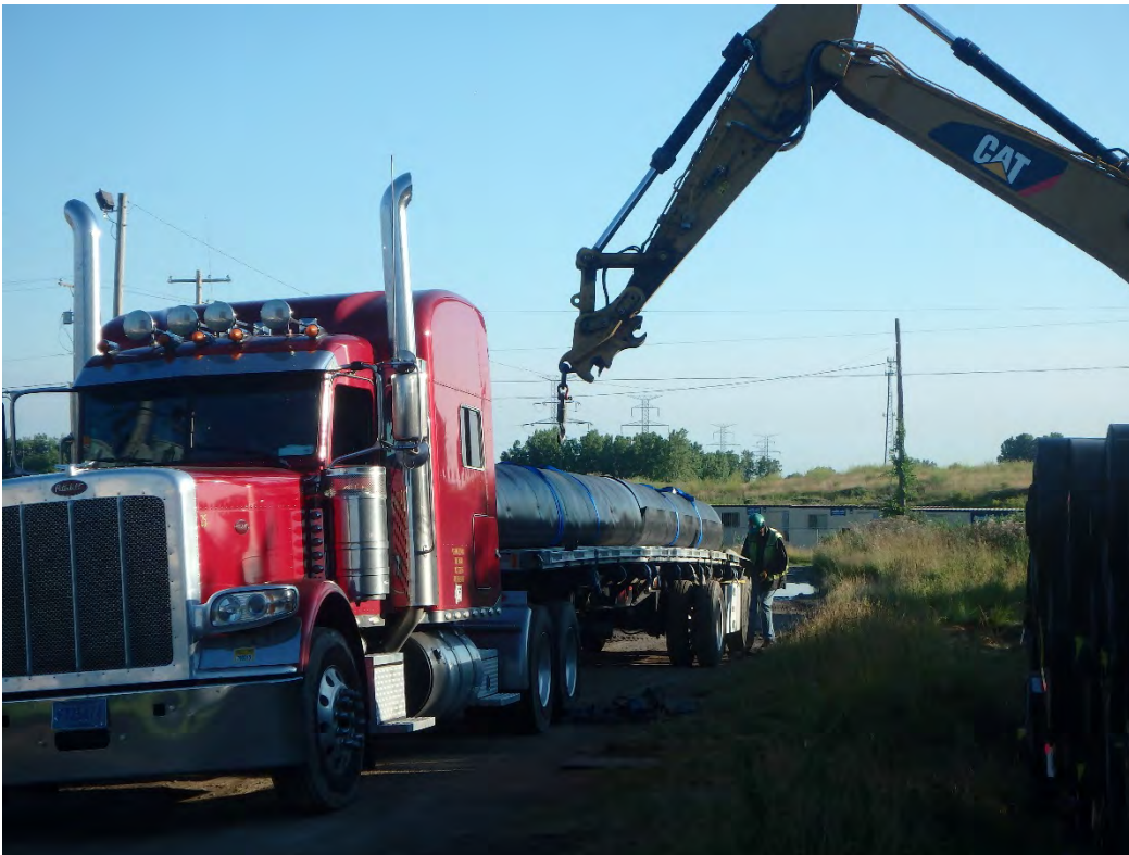
Offload of geomembrane, looking north.
