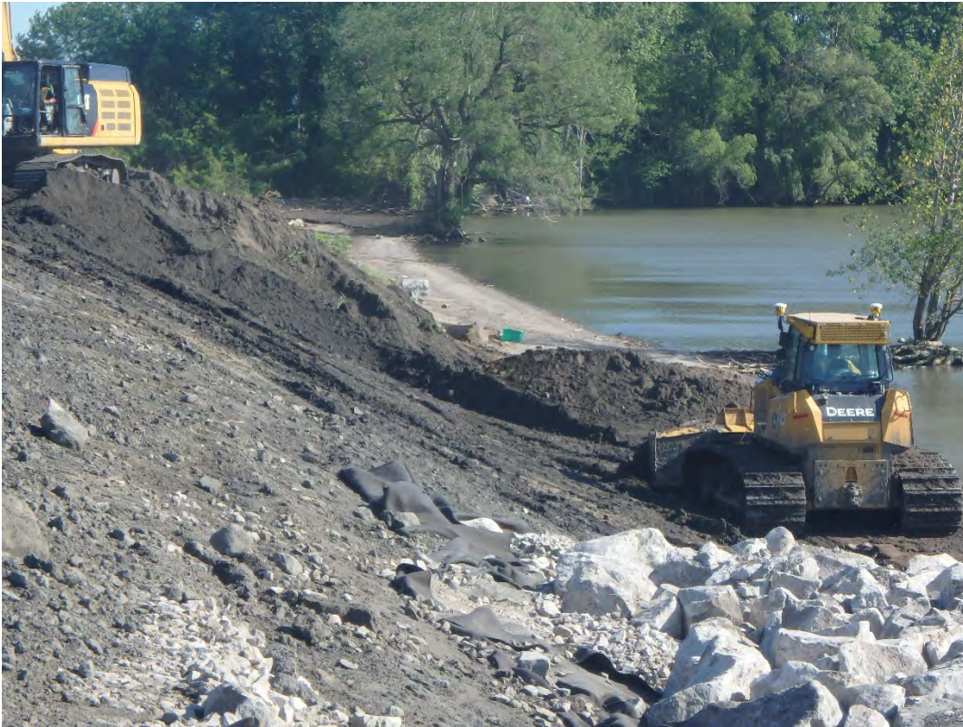
Grading shoreline slope, looking north.
