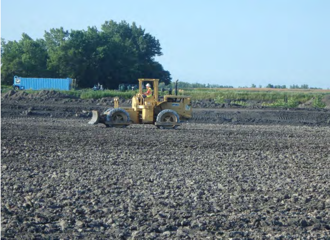
Compacting structural fill placed in Pond 1, looking south.
