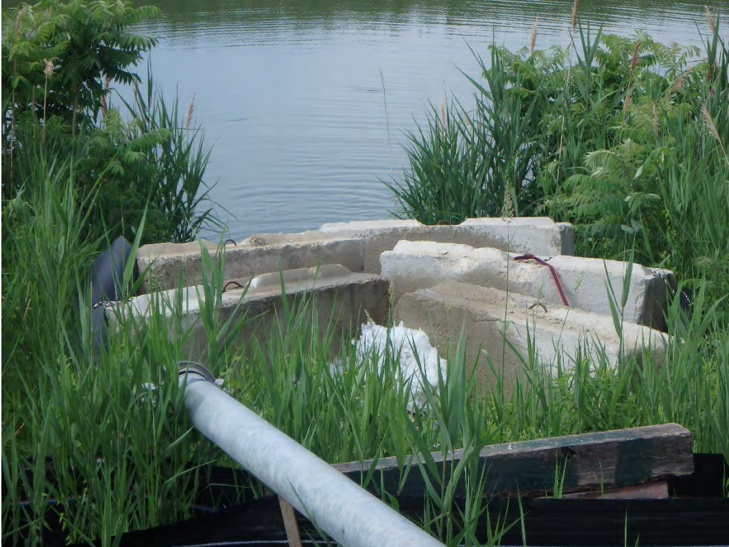
Discharge water from Pond 2, looking south.
