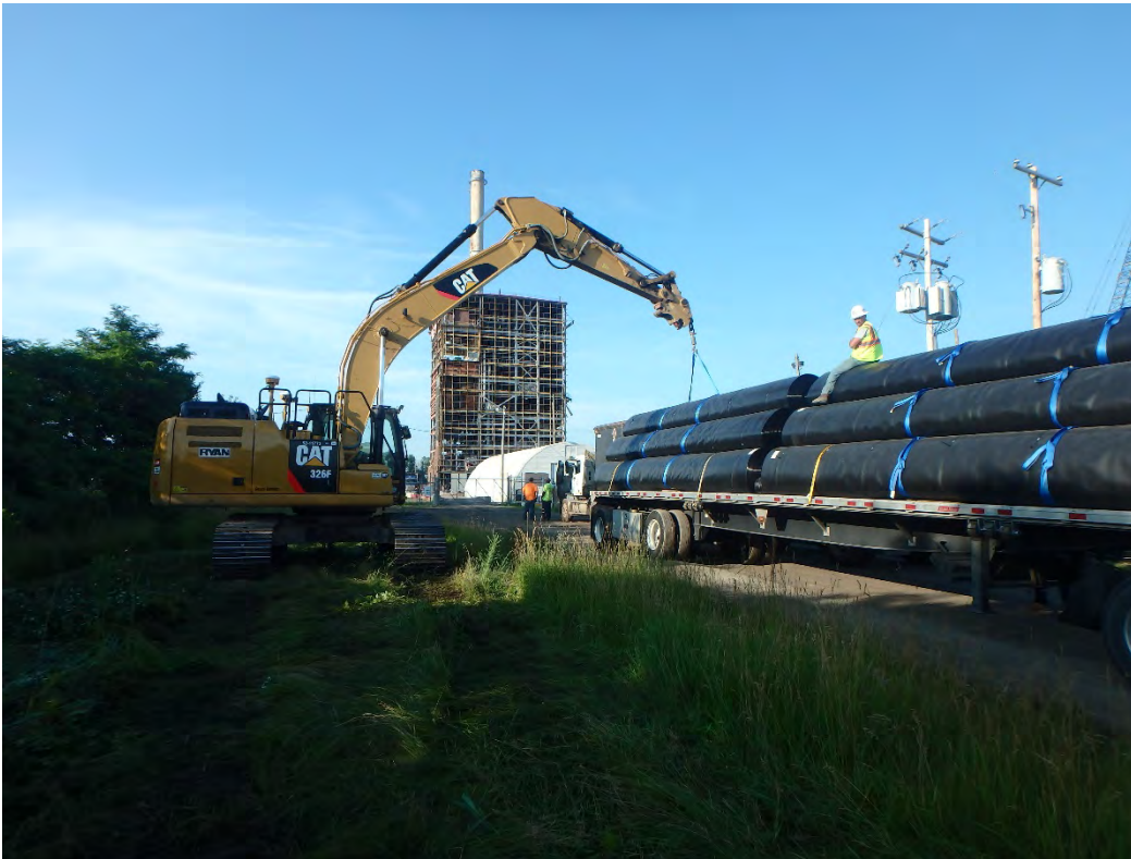
Off-loading 40mil geomembrane, looking south.
