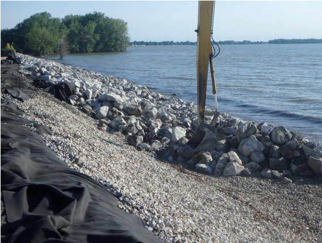
Placing D50/30 inch riprap along shoreline, looking northeast.
