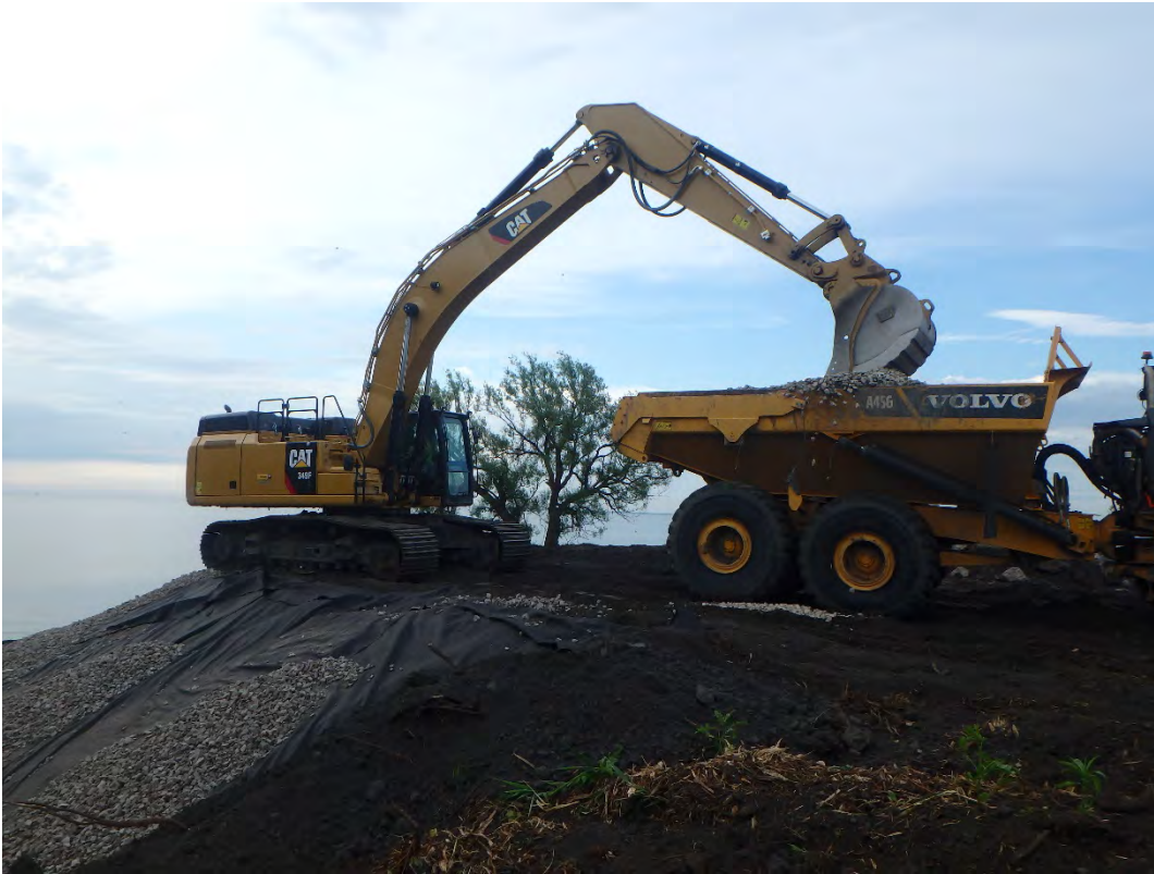
Placing D50/2 inch cushion layer on shoreline, looking east.
