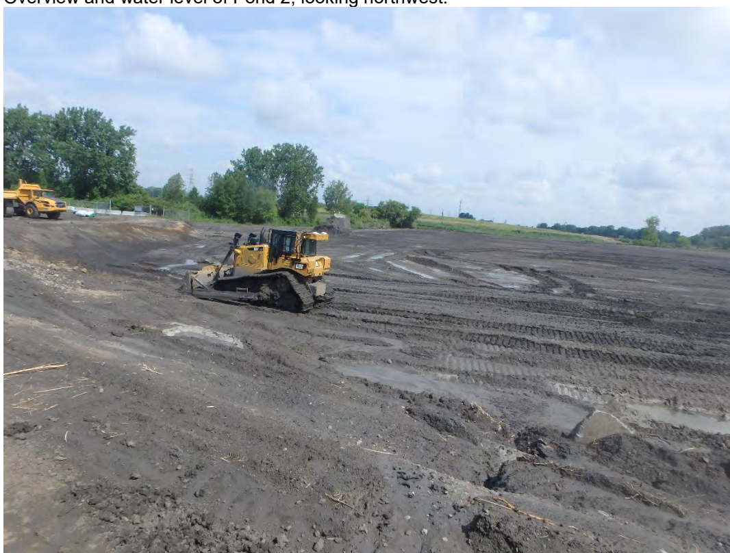
Re-grading of CCR in Pond 1 work area, looking northwest.
