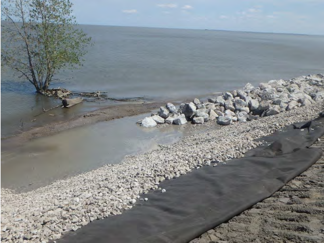
Geotextile and D50/2 inch cushion layer along shoreline, looking southeast.
