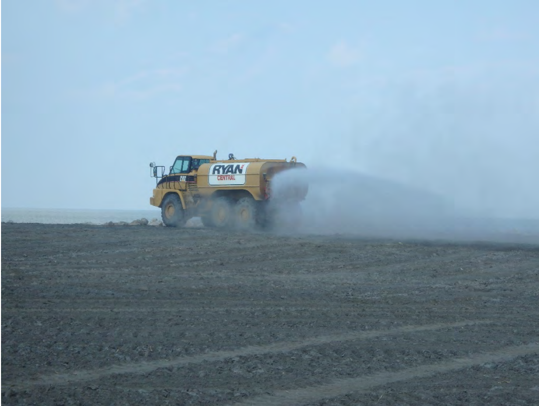
Water truck used for dust control, looking east.
