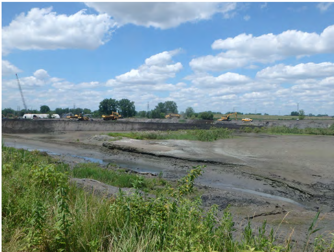
Overview/water level of Pond 2, looking northwest.
