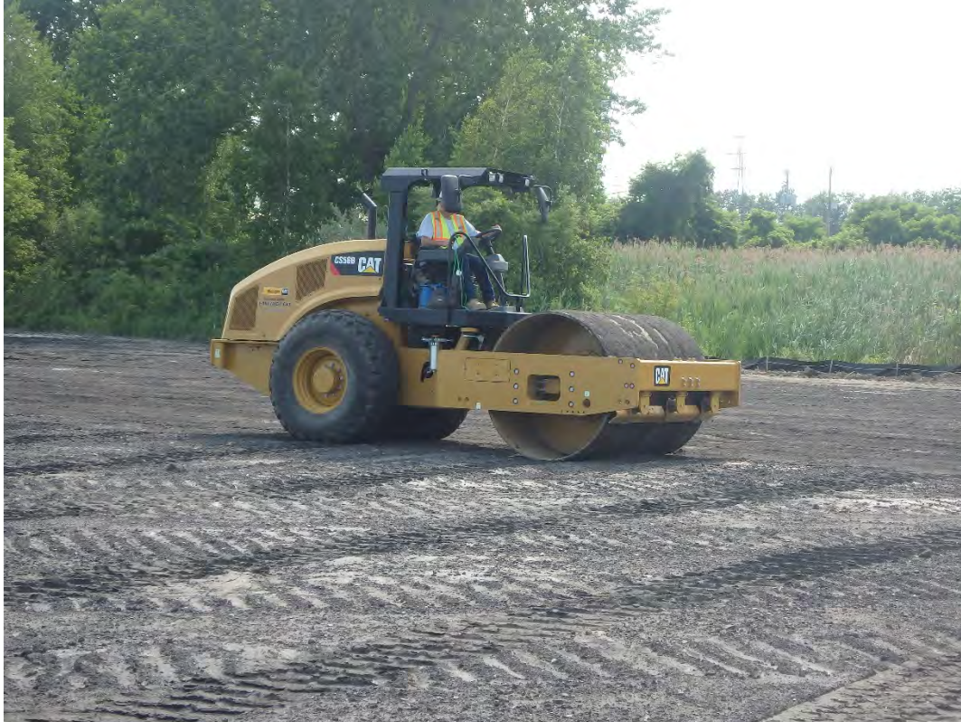
Smooth drum rolling bridging layer in Pond 1, looking west.
