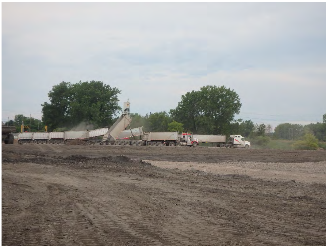
Delivery of structural fill to Pond 1, looking west.
