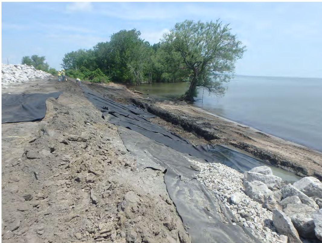
Textile placed along shoreline for D50/2 inch cushion layer, looking north.
