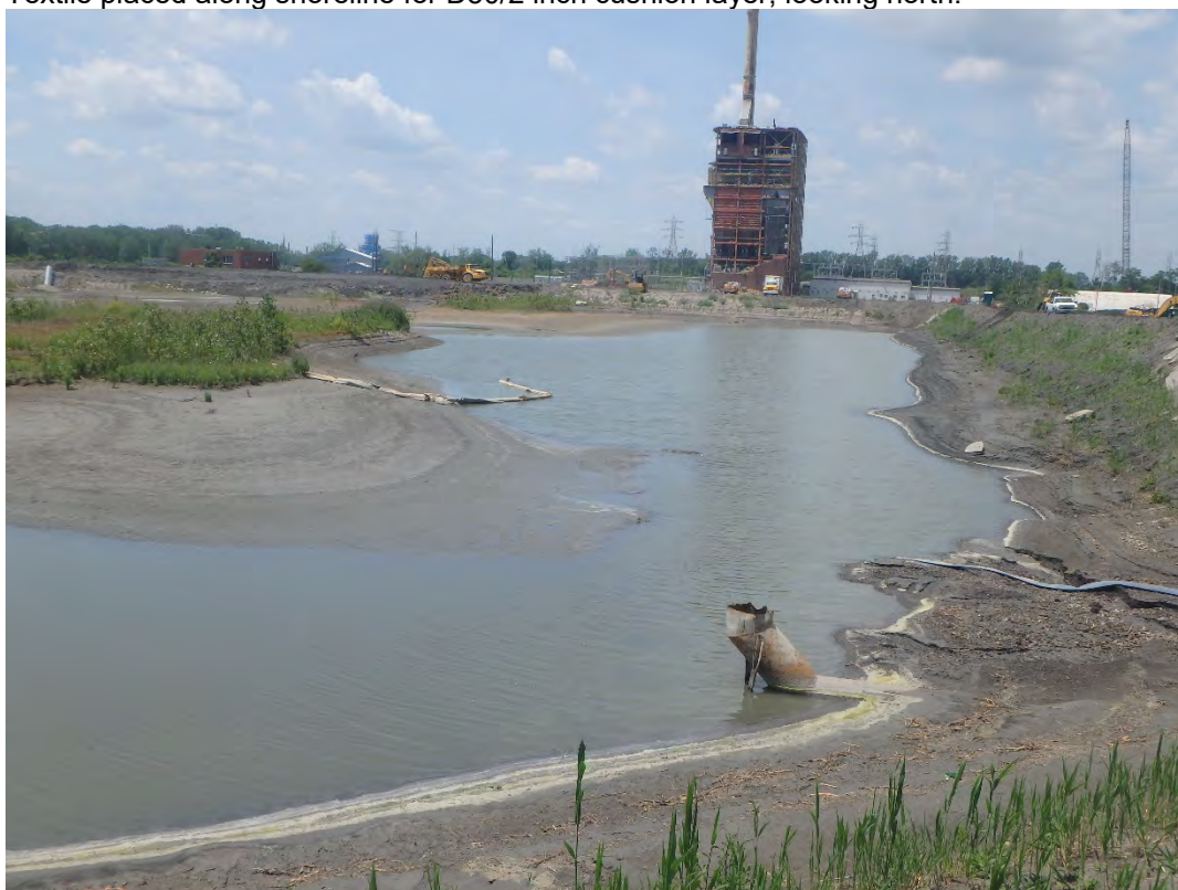
Overview and water level of Pond 2, looking west.
