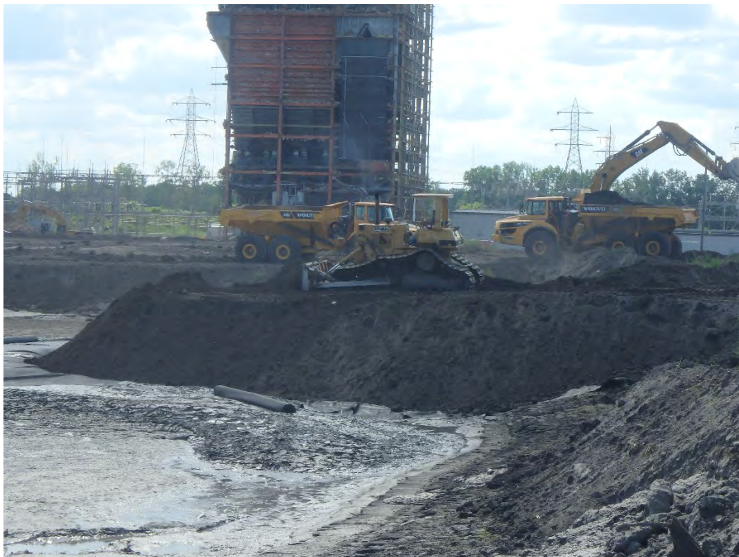
Placing bridging layer in Pond 2, looking west.
