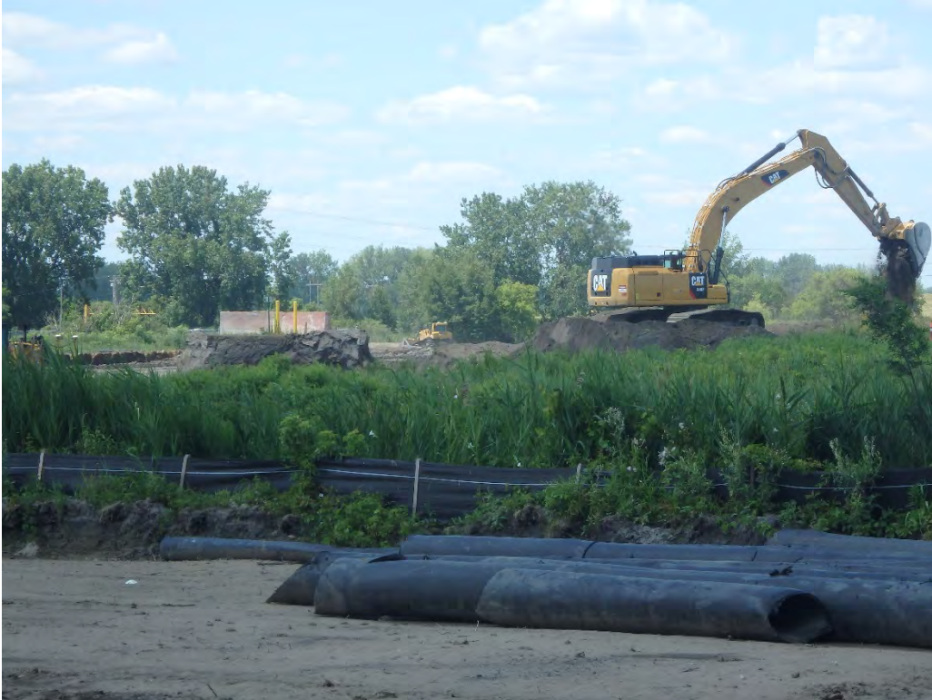
Excavating Pond 2's west dike, looking northwest.
