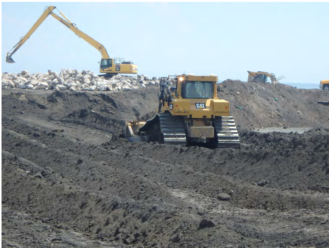
Pond 1 bridging layer being placed atop geotextile, looking east.
