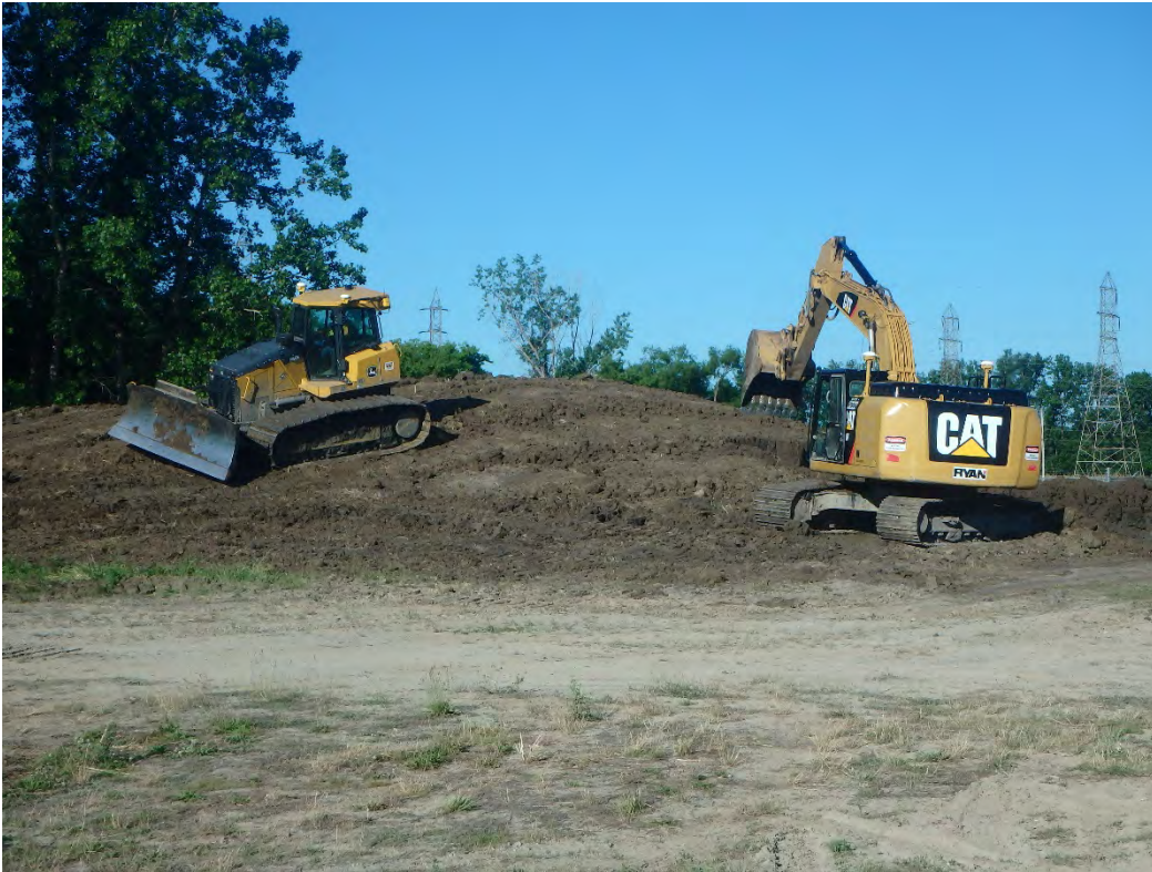
On-site structural fill stockpile stripped of vegetation, looking southwest.
