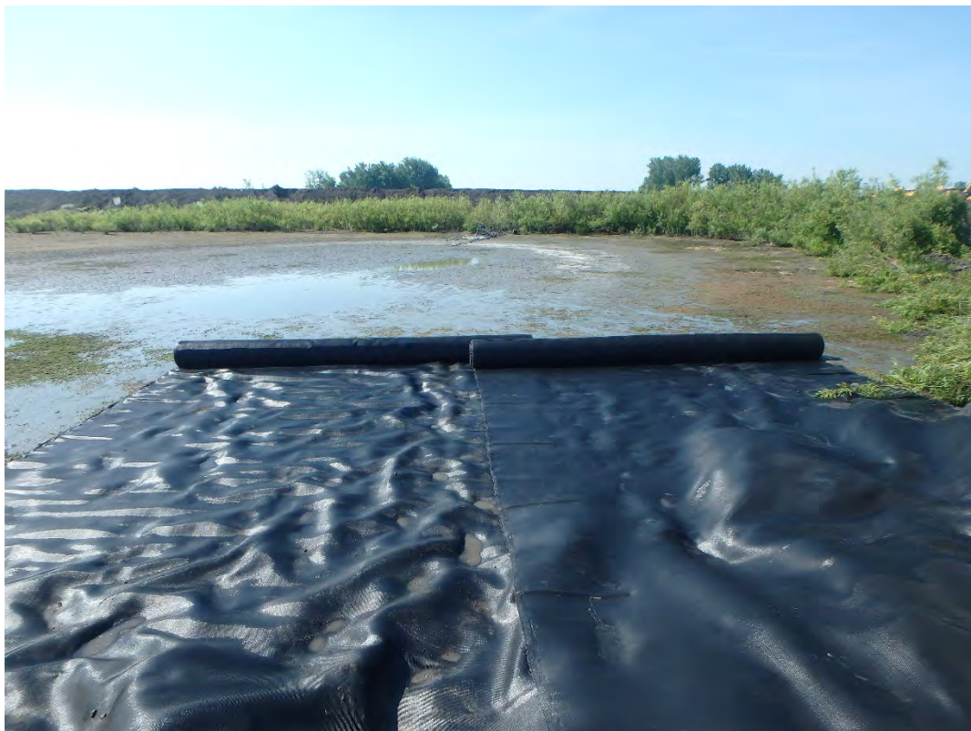
Installation of geotextile in Pond 1 prior to bridging layer, looking south.
