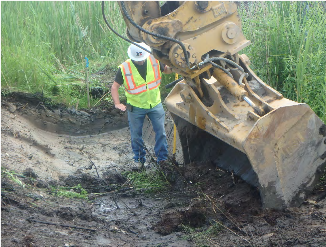
Excavation of ditch for new access road culvert, looking east.
