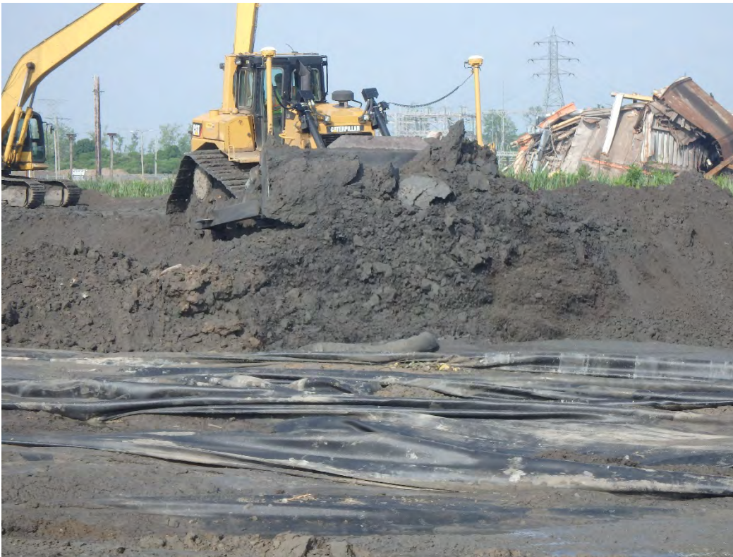
Placement of bridging layer in Pond 2, looking west.
