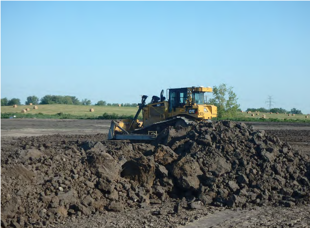
Placing lift of structural fill in Pond 1, looking north.
