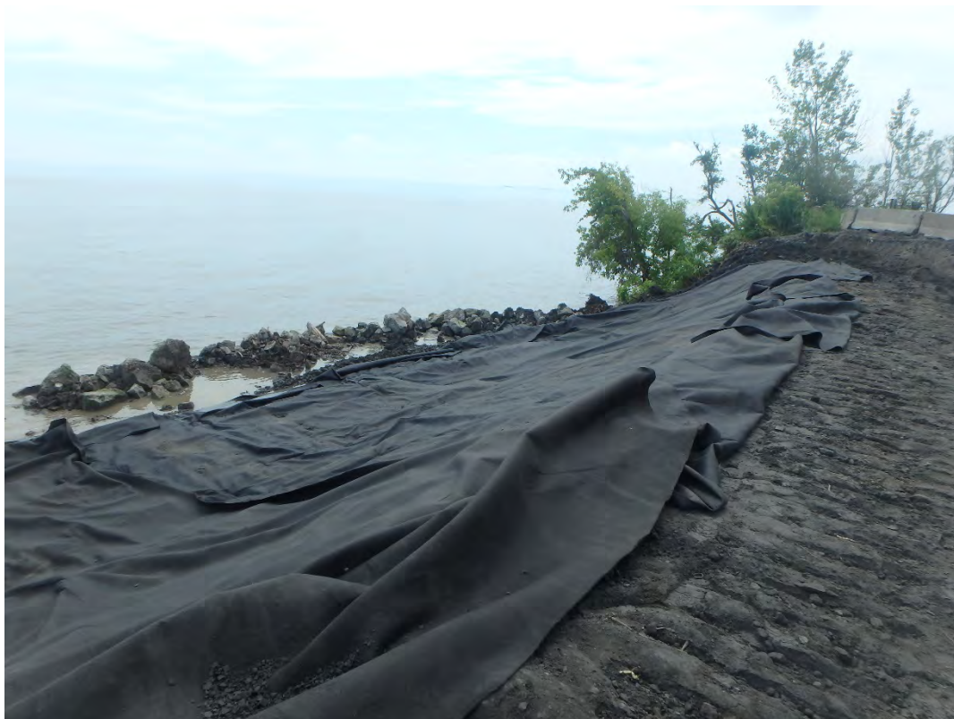
Textile deployed along shoreline, looking south.
