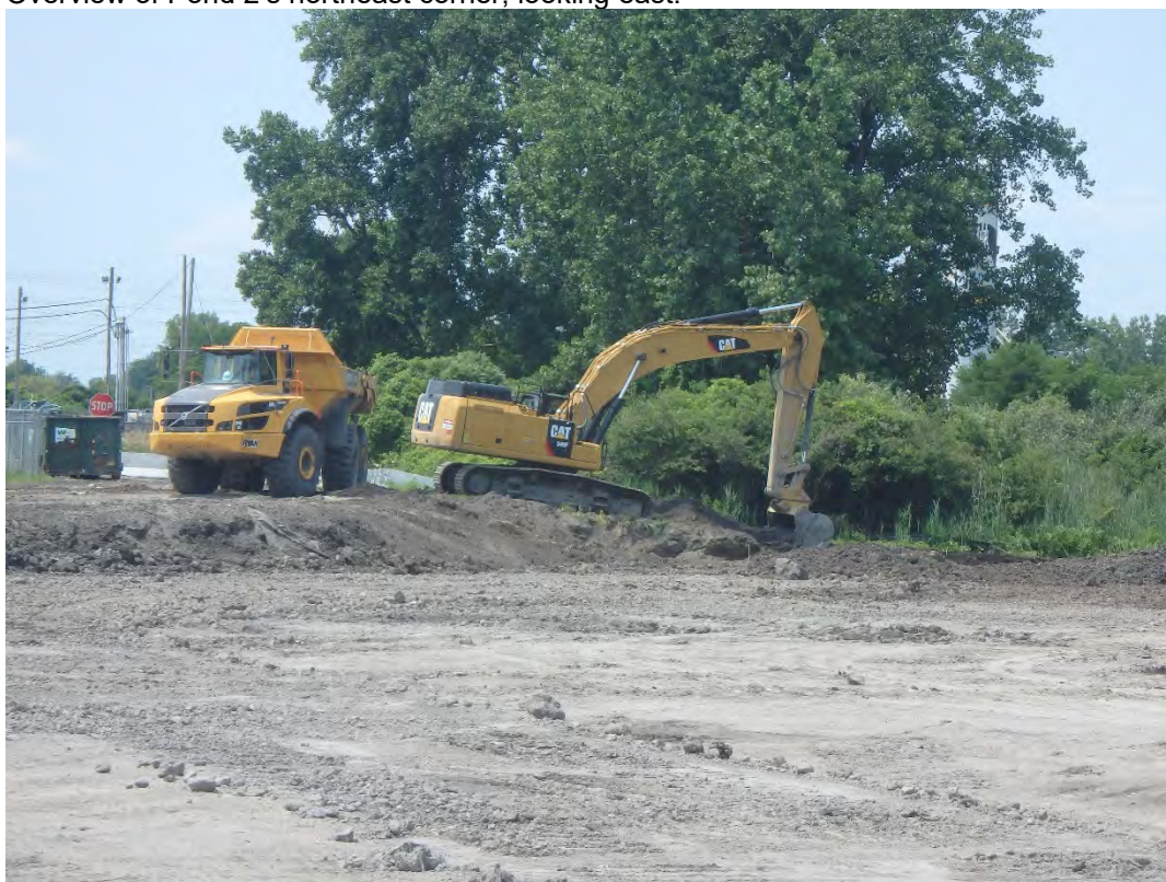
Excavation for the swale west of Pond 1, looking west.
