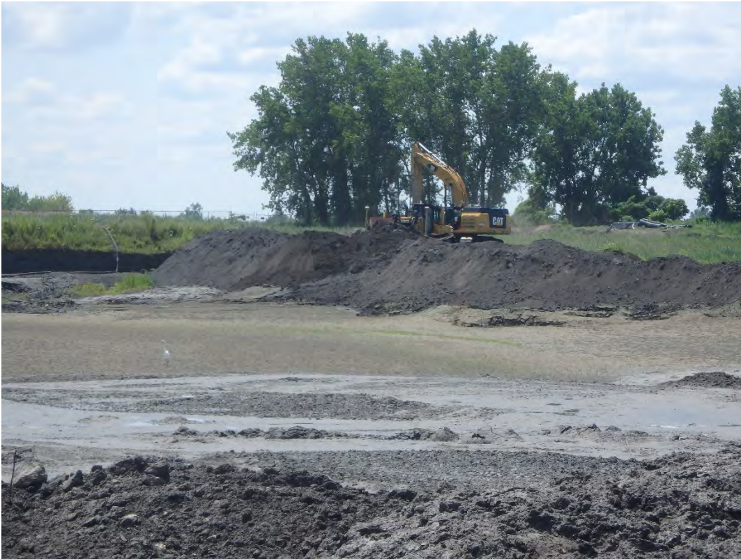
Bridging layer in Pond 2, looking south.
