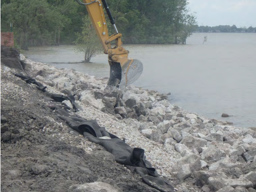
Placement of D50/30 inch riprap along shoreline, looking north.
