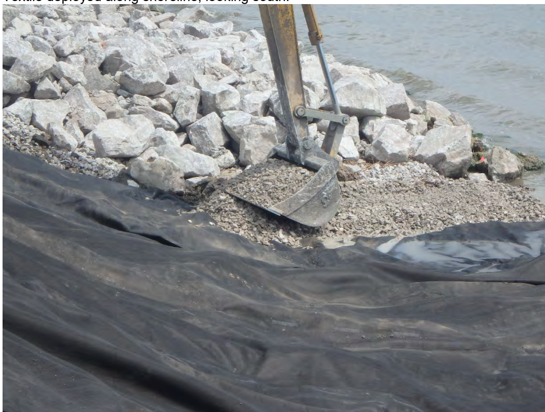
Placing D50-2 inch cushion layer atop textile on shoreline, looking north.
