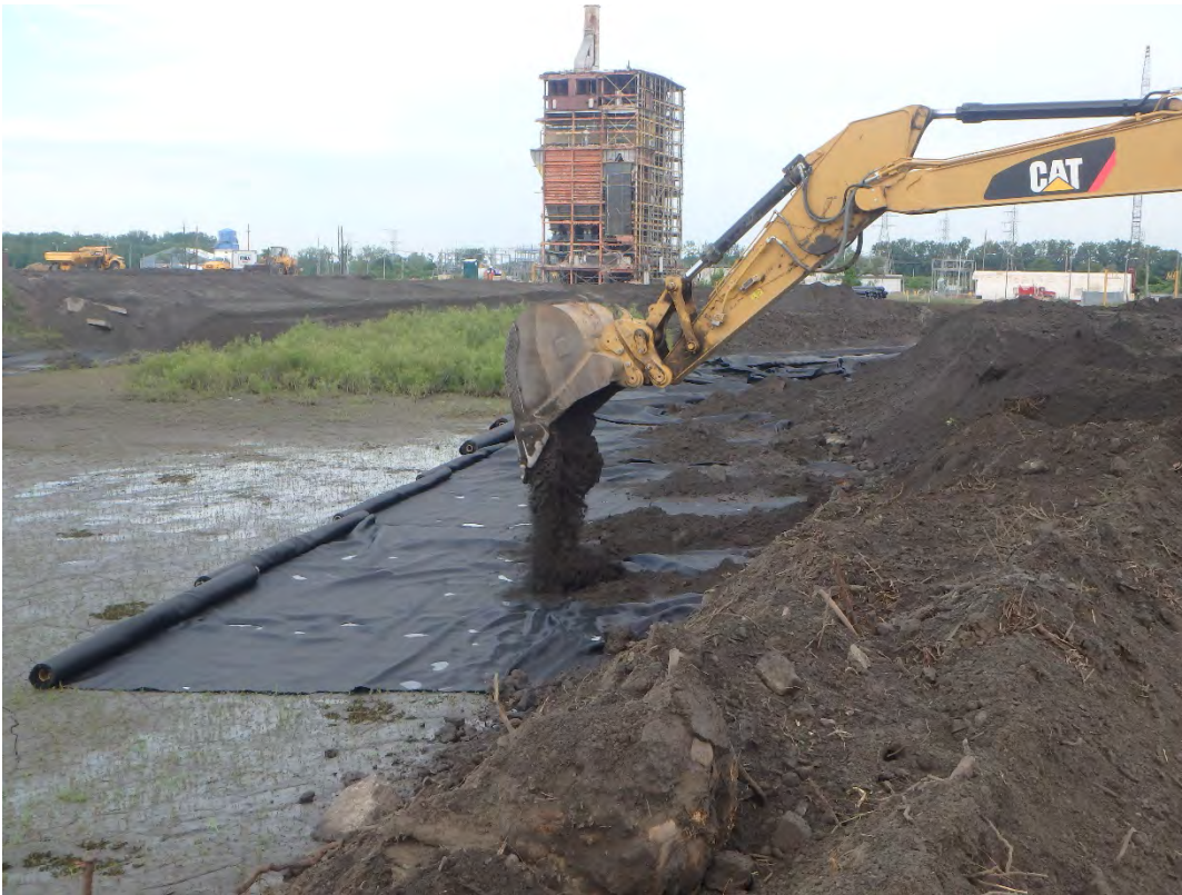
Pond 1 bridging layer being placed atop geotextile, looking west.
