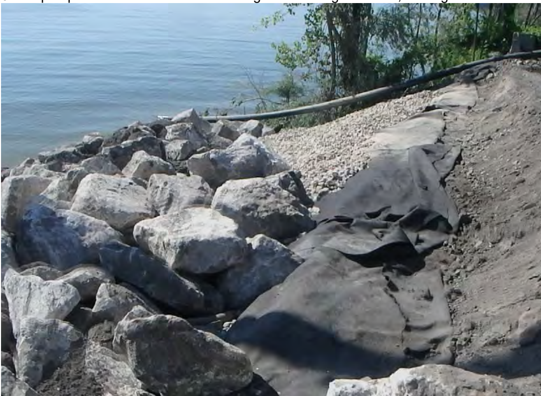
Riprap along shoreline southeast of Pond 2, looking south.
