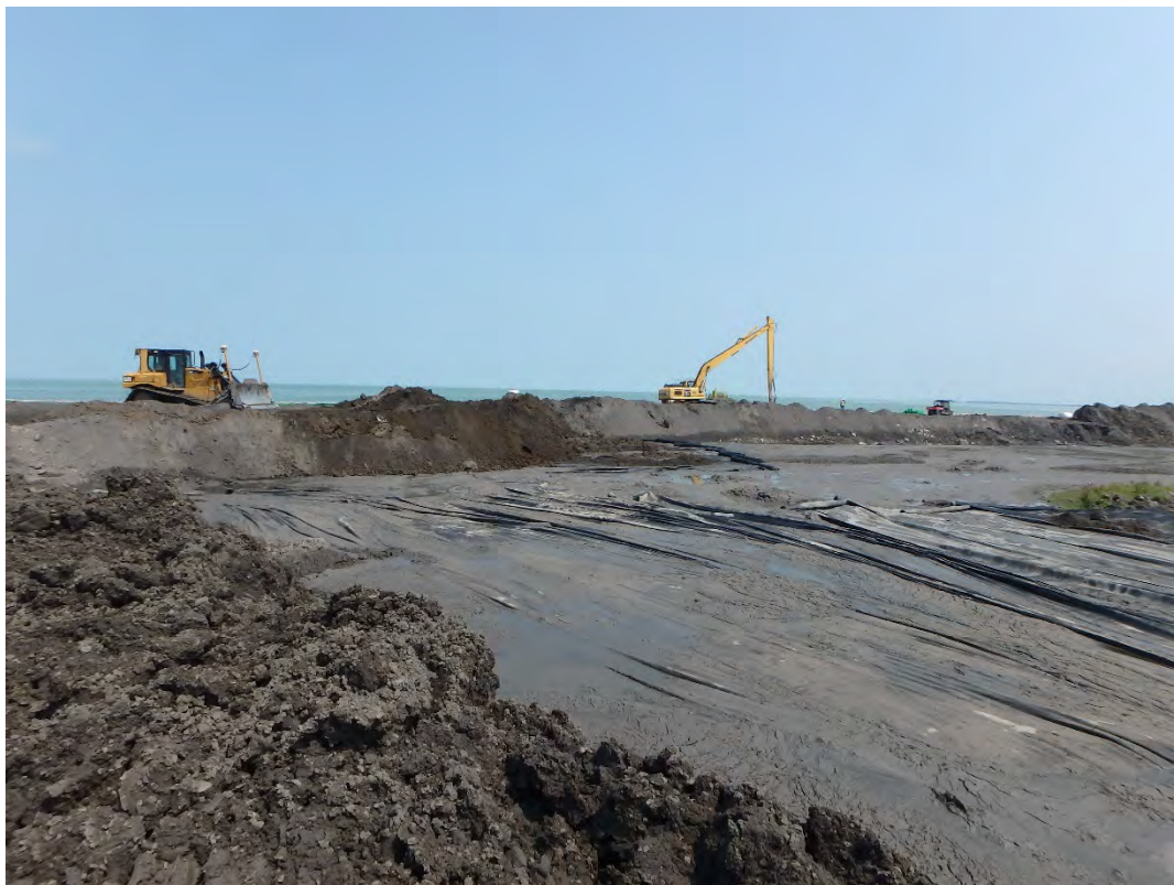
Overview of Pond 2's northeast corner, looking east.
