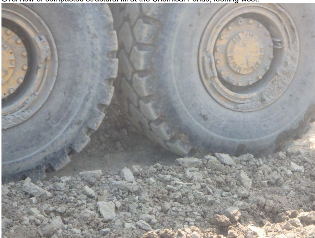
Proof roll of structural fill at the Chemical Ponds.
