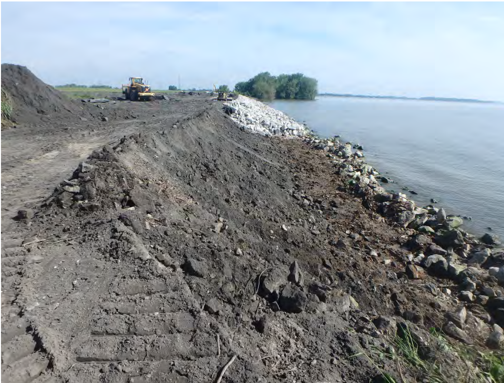
Cutting of shoreline east of Pond 2 to sub-grade, looking north.
