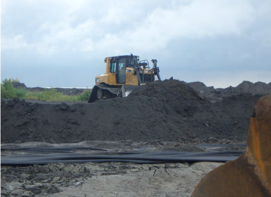
Placing bridging layer over textile in Pond 2, looking west.
