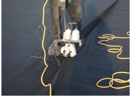
Sewing geotextile seam.
