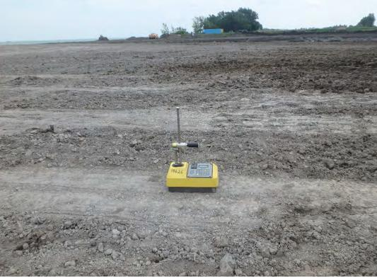
Density testing compacted lift of structural fill in Pond 1, looking south.
