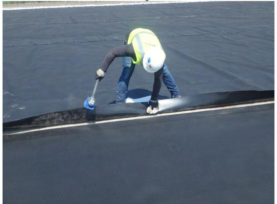
Cleaning liner overlap ahead of fusion seaming device.
