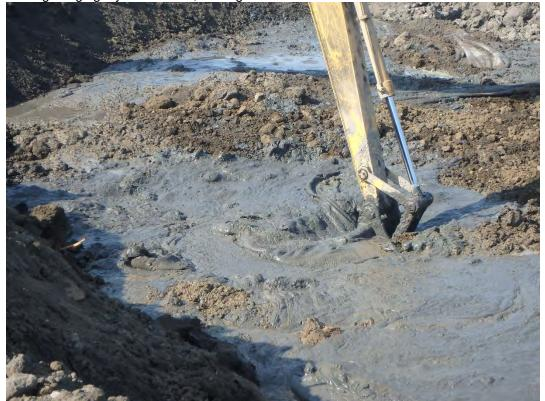
Removing saturated material from Pond 2 prior to bridging layer being placed.
