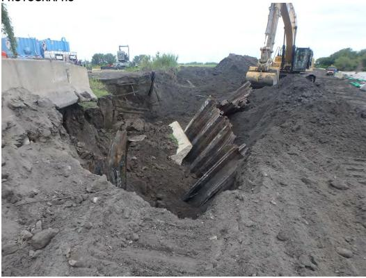
Removing sheet pylon east of Pond 2 and discharge channel, looking north.
