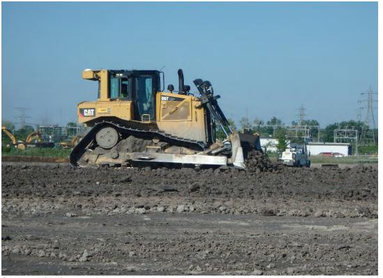
Structural fill lift being placed in Pond 1, looking west.
