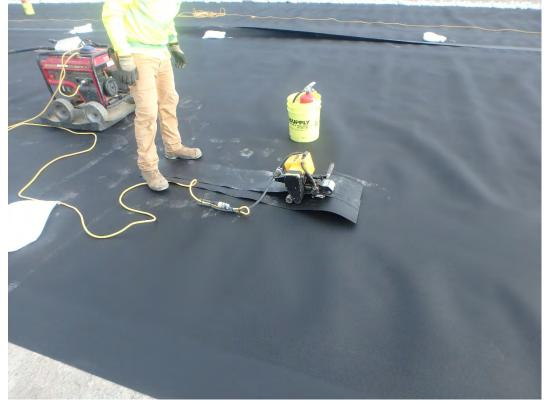
Producing trial weld for field testing.
