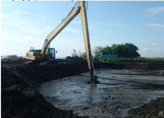
Removing saturated CCR from the northeast corner of Pond 2, looking southeast.
