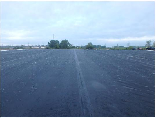
Overview of geomembrane deployed in Pond 1, looking west.
