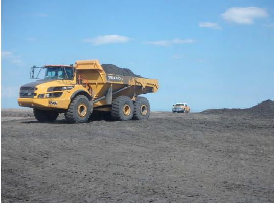
CCR excavated from south dike being placed in Pond 2 for bridging layer, looking east.
