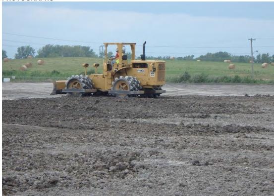
Compacting lift of structural fill in Pond 1, looking north.
