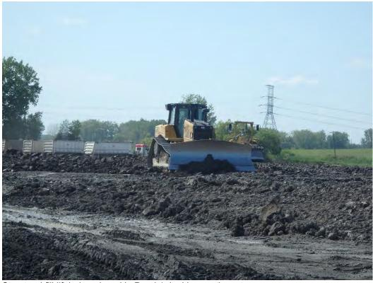
Structural fill lift being placed in Pond 1, looking northwest.
