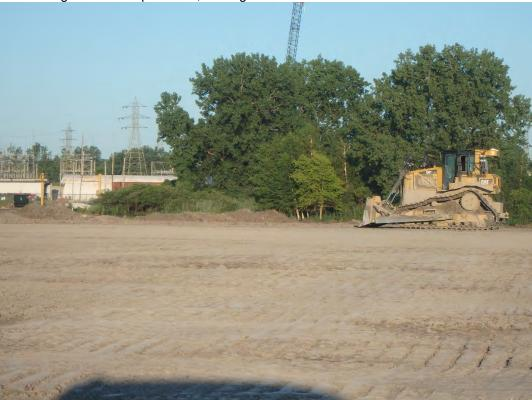
Finish grading of liner sub-grade in Pond 1, looking west.
