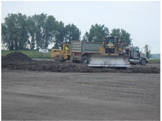
Placing structural fill lift in Pond 2, looking southwest.
