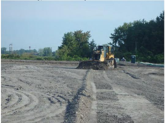
Cutting placed and compacted structural fill in Pond 1 to liner sub-grade, looking north.
