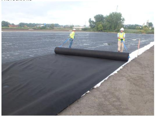
Deployment of 8oz. geotextile in Pond 1, looking west.
