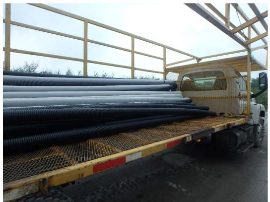
4 inch ADS pipe for above-cap drainage system.
