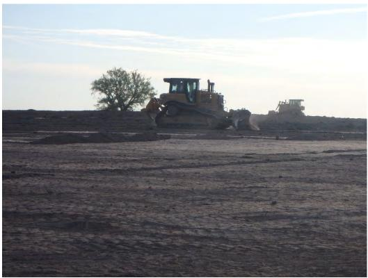
Finish grading structural fill in Pond 1, looking northeast.
