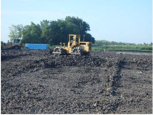
Compacting lift of structural fill in Pond 2, looking south.
