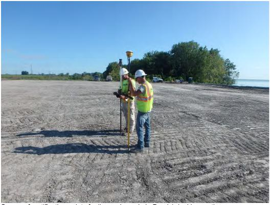
Survey of certification points for liner sub-grade in Pond 1, looking north.
