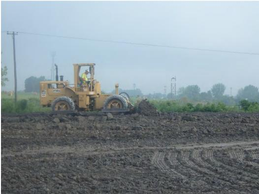
Compacting lift of structural fill in Pond 1, looking north.
