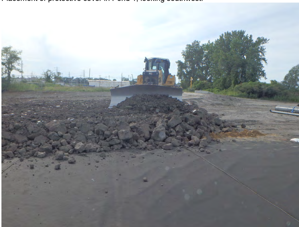
Protective cover being placed atop geosynthetics in Pond 1, looking west.
