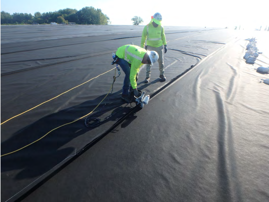
Sewing geotextile seam, looking northeast.
