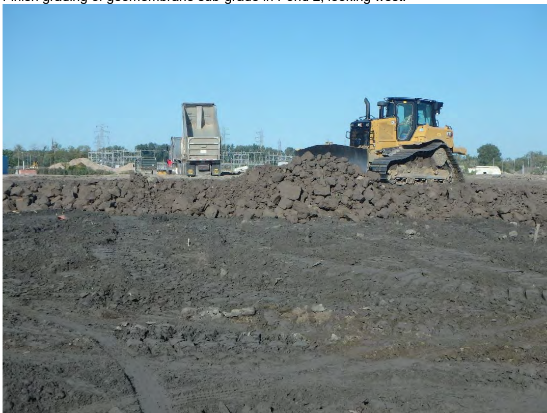
Placement of bridging layer in southeast corner of Pond 2, looking west.
