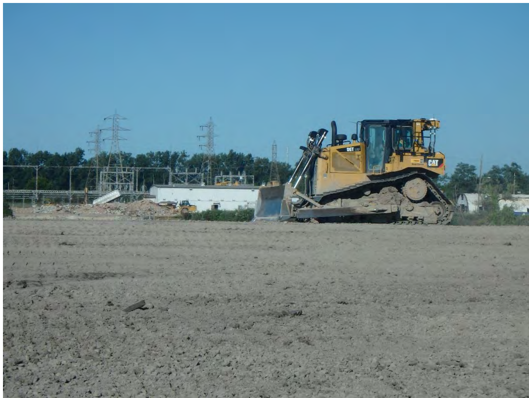
Finish grading of geomembrane sub-grade in Pond 2, looking west.
