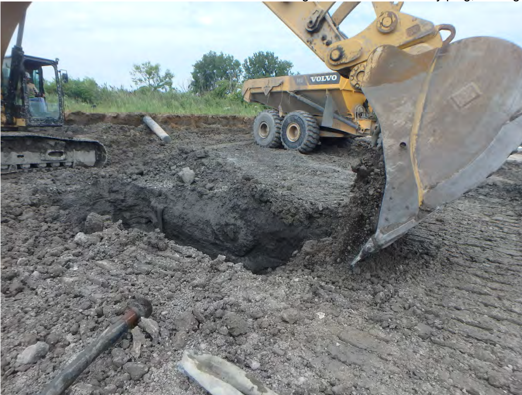
Installing clay plug in the French Drain trench, looking west.
