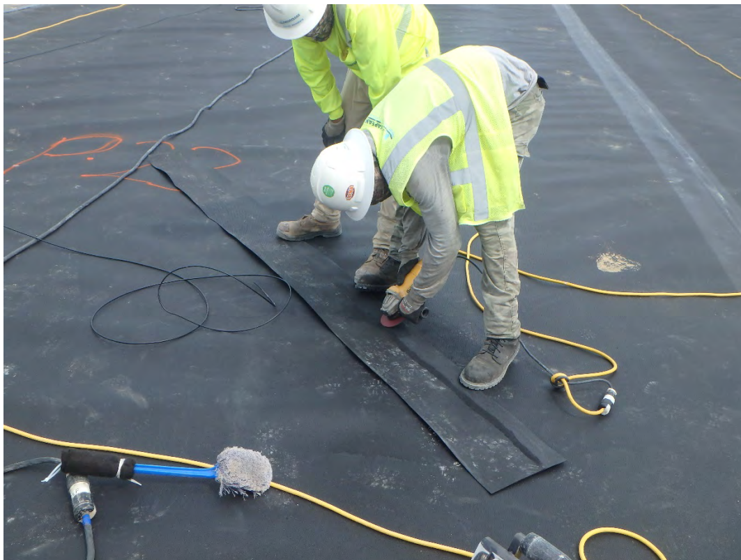
Preparing trial weld.
