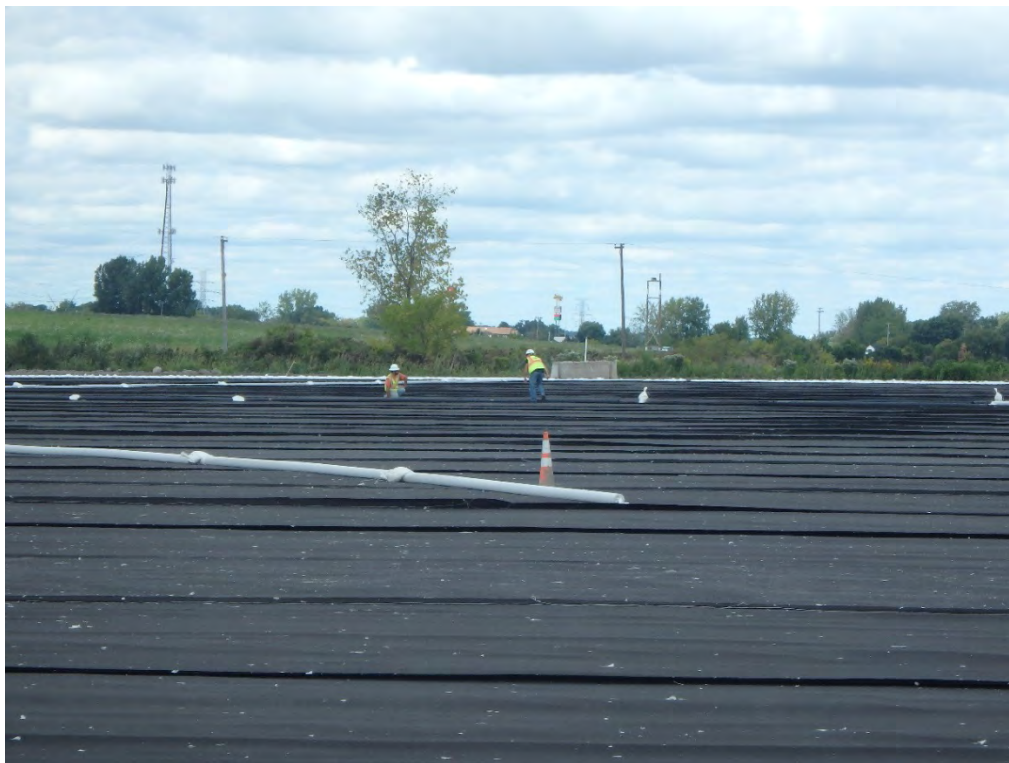
Installation of the above-cap drain pipe in Pond 1, looking north.
