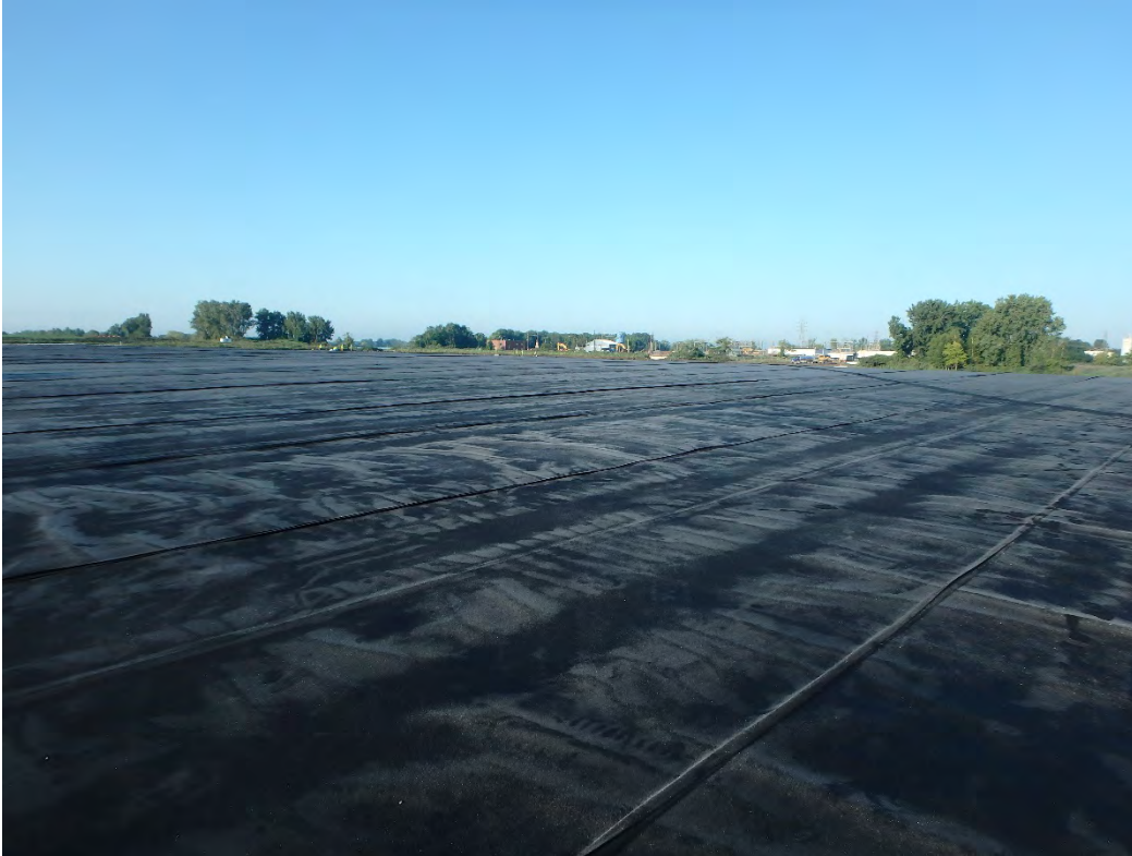
Overview of Pond 1, looking southwest.
