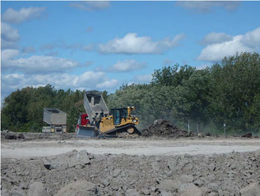
Protective cover import and placement in Pond 1, looking north.
