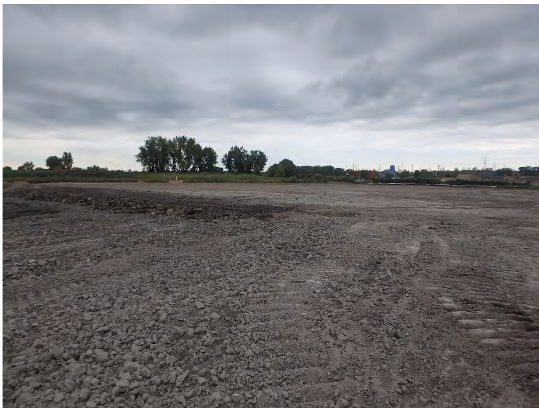
Overview of Pond 2, looking southwest
