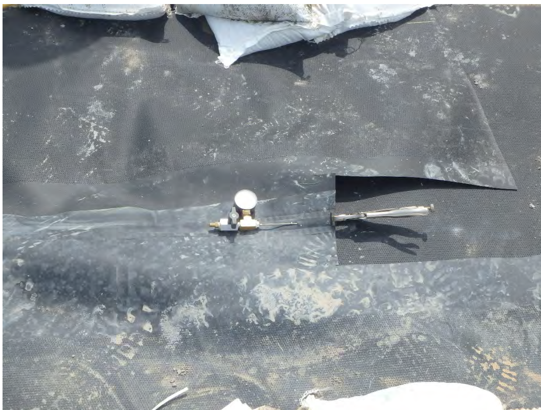
Pressure testing of fusion seam.
