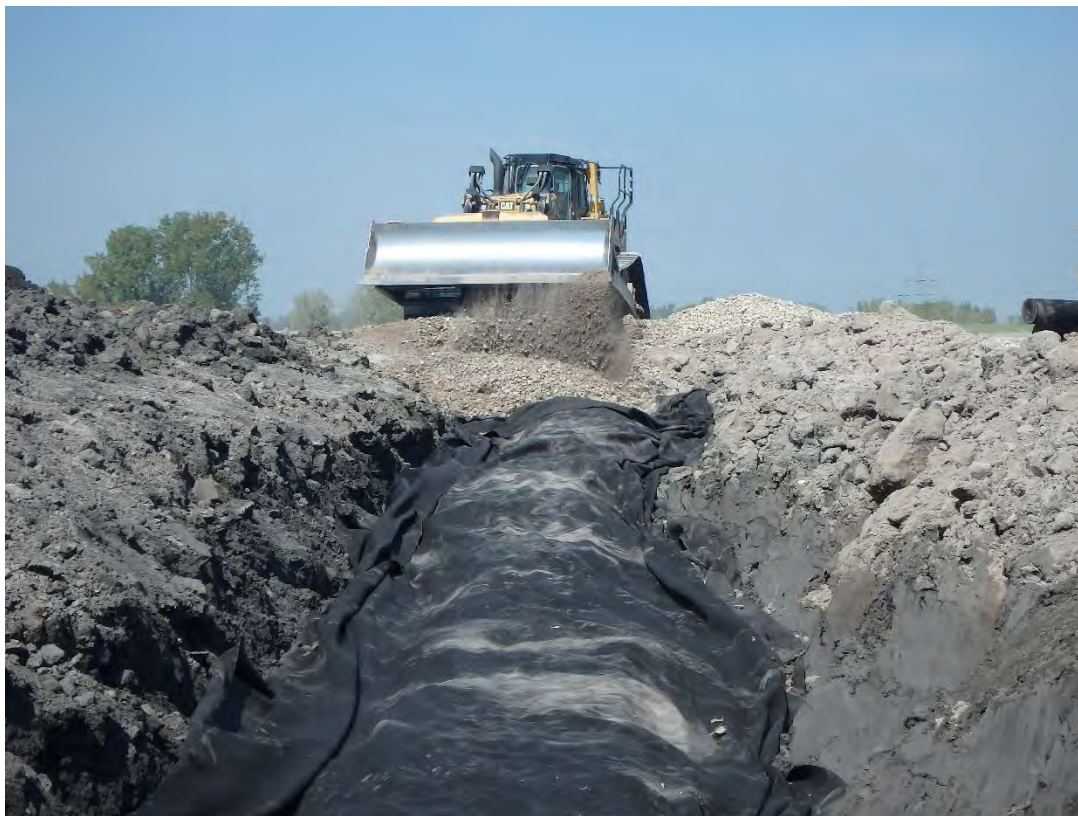
Backfilling trench in southeast corner of Pond 2, looking north.
