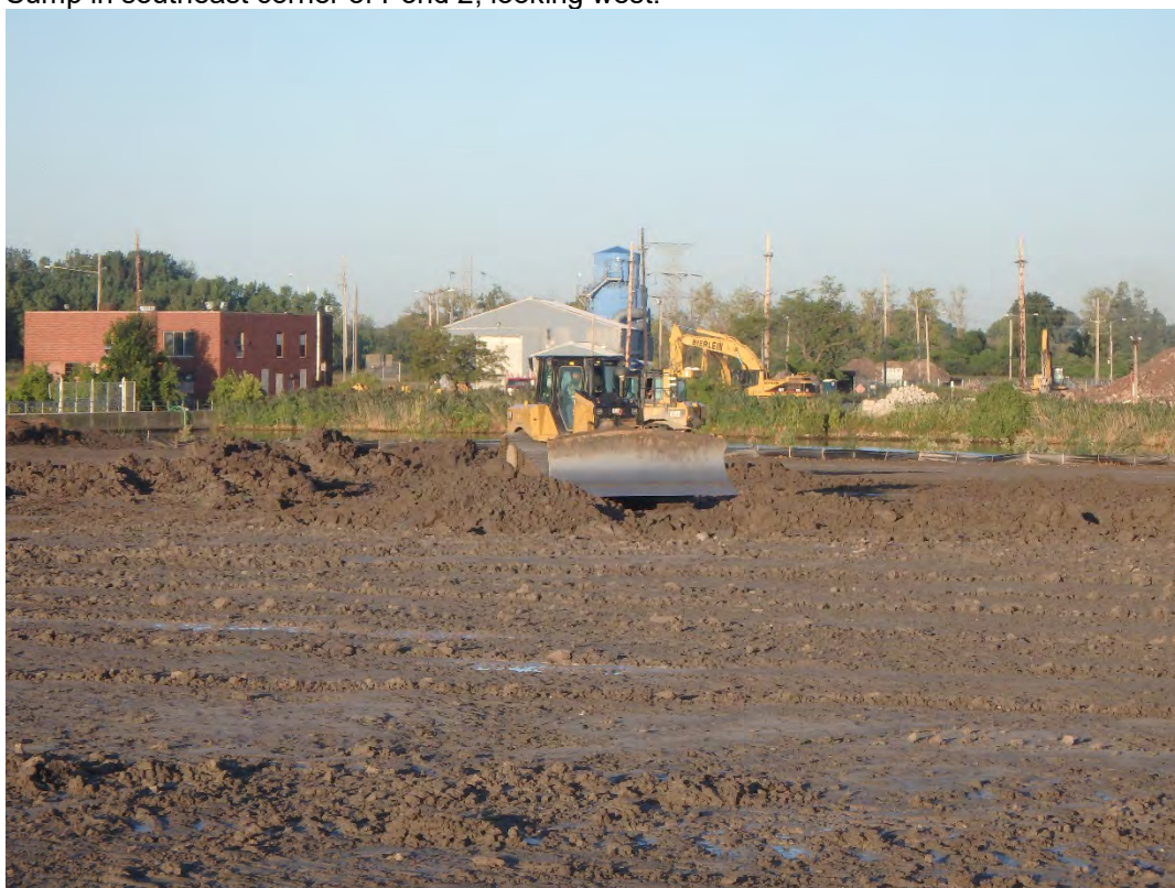
Placing structural fill in Pond 2, looking west.
