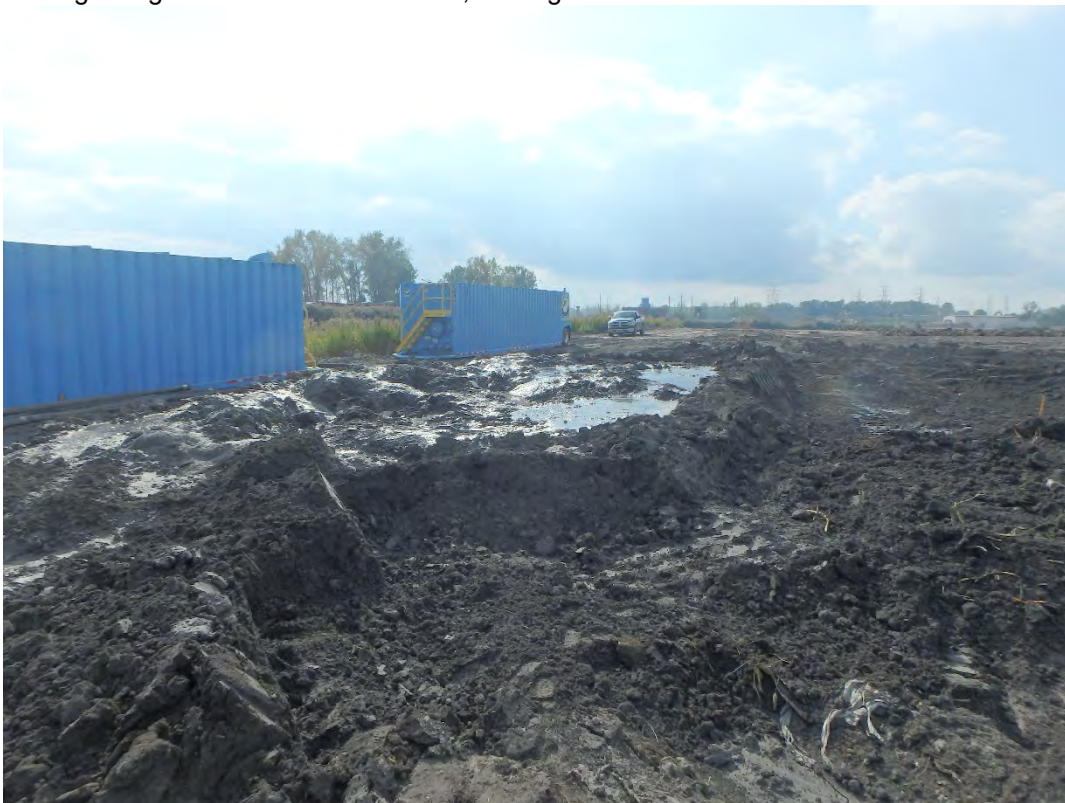
Saturated CCR removed from the sump area of Pond 2, looking west.
