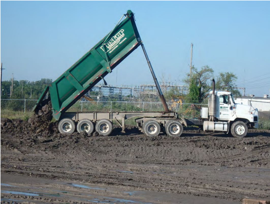
Structural fill import, looking southwest.
