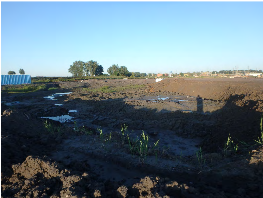
Sump in southeast corner of Pond 2, looking west.
