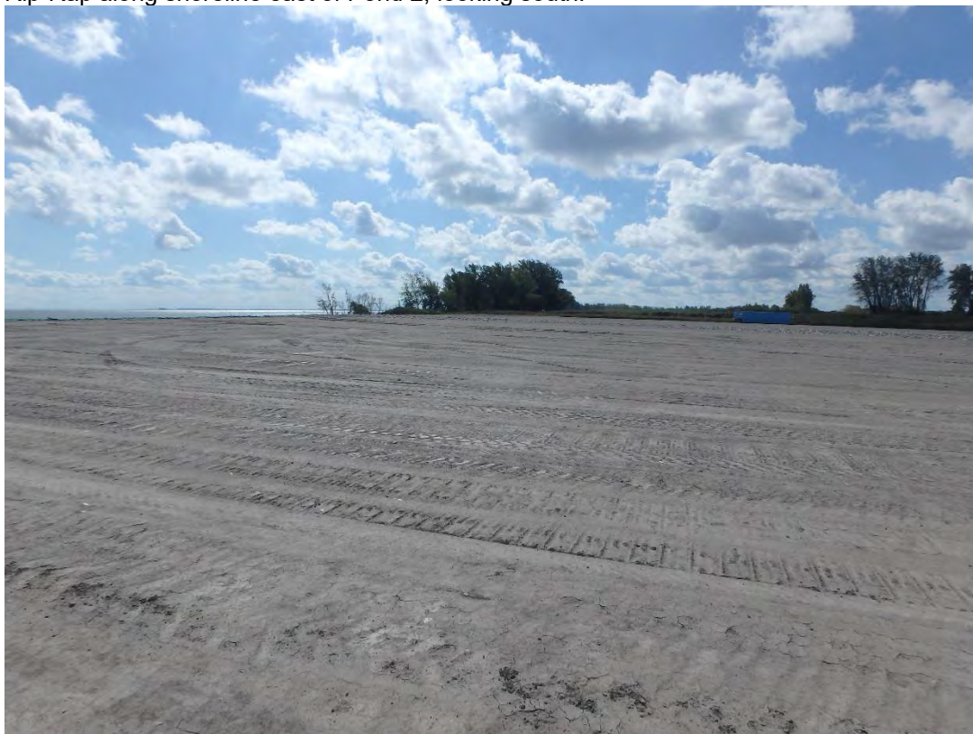
Overview of liner sub-grade in Pond 2, looking southeast.
