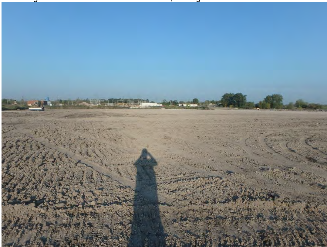
Overview of liner sub-grade in Pond 2, looking west.
