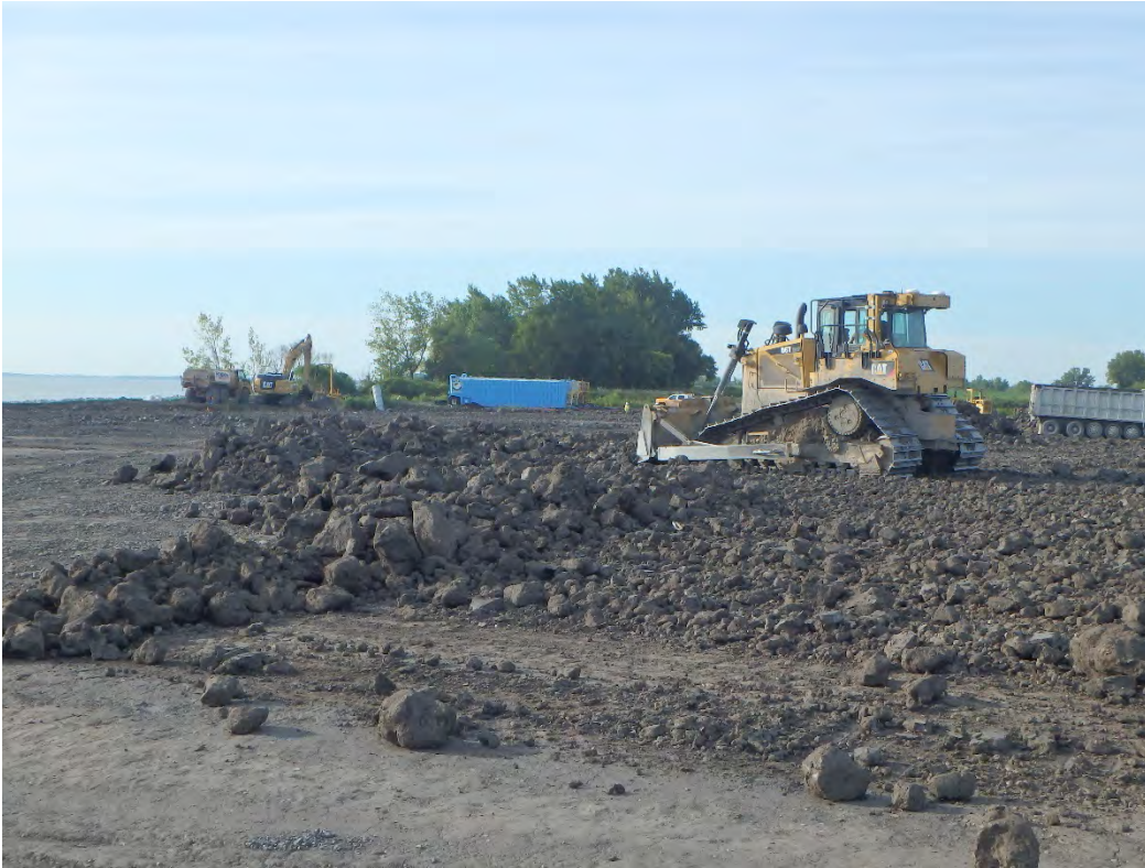
Placing lift of structural fill in Pond 2, looking south.
