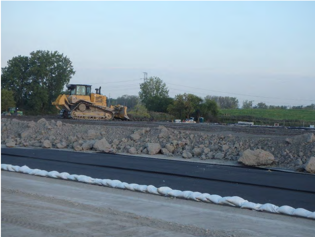
Placement of protective cover in Pond 1, looking northwest.
