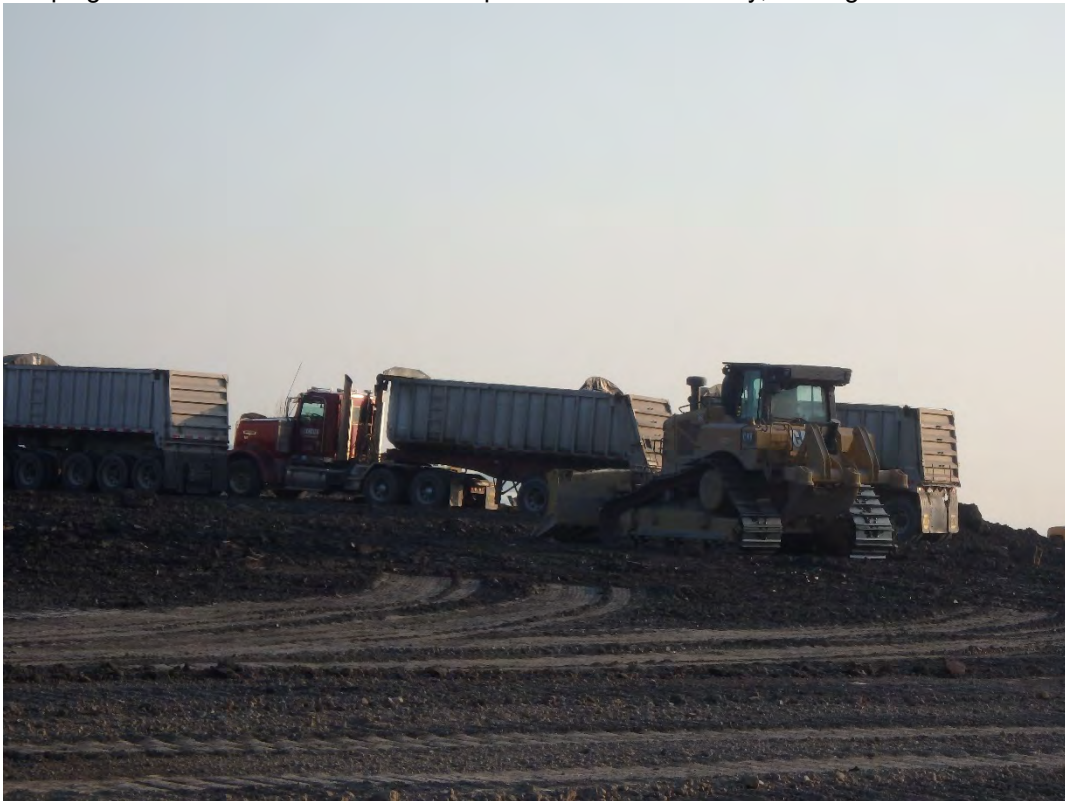
Import and placement of structural fill in Pond 2, looking east.
