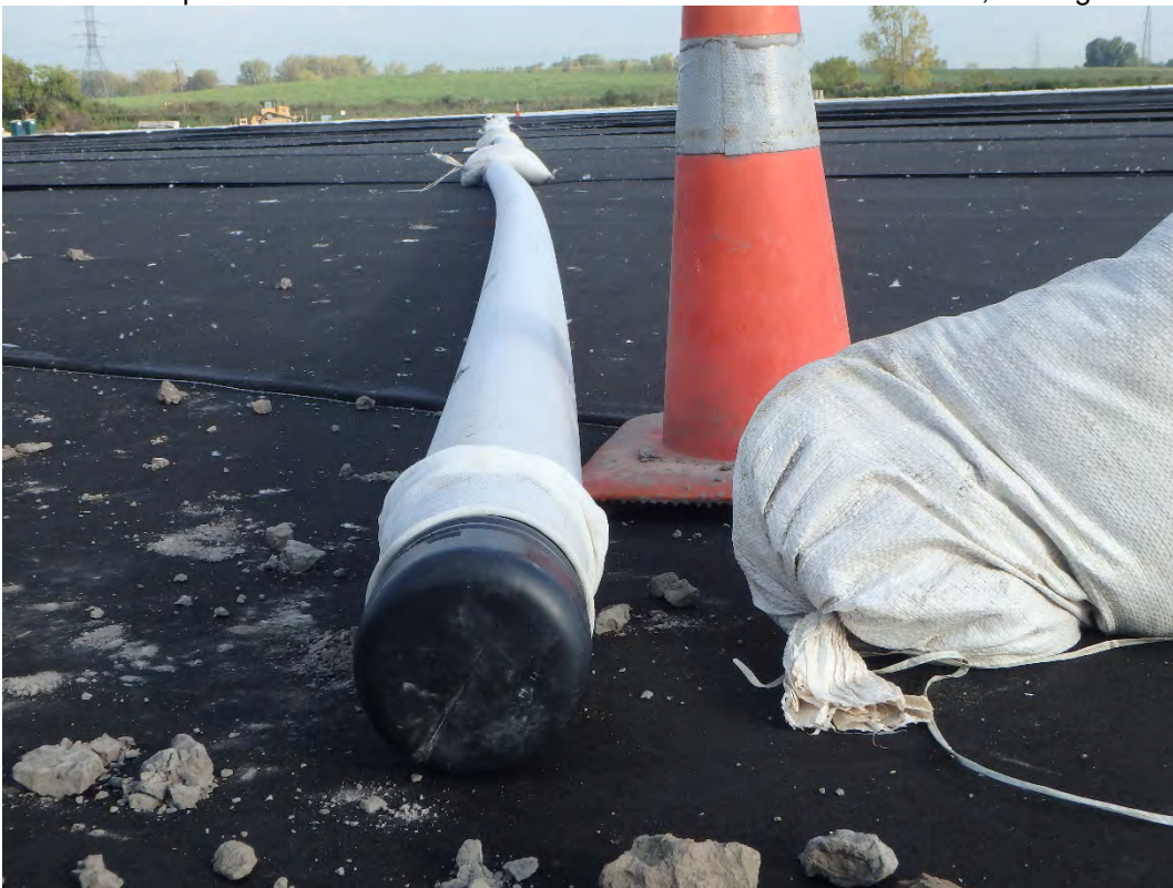
End caps on socked ADS perforated pipe, looking north.
