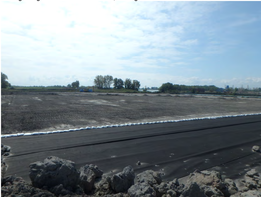
Overview of Pond 2, looking southwest.
