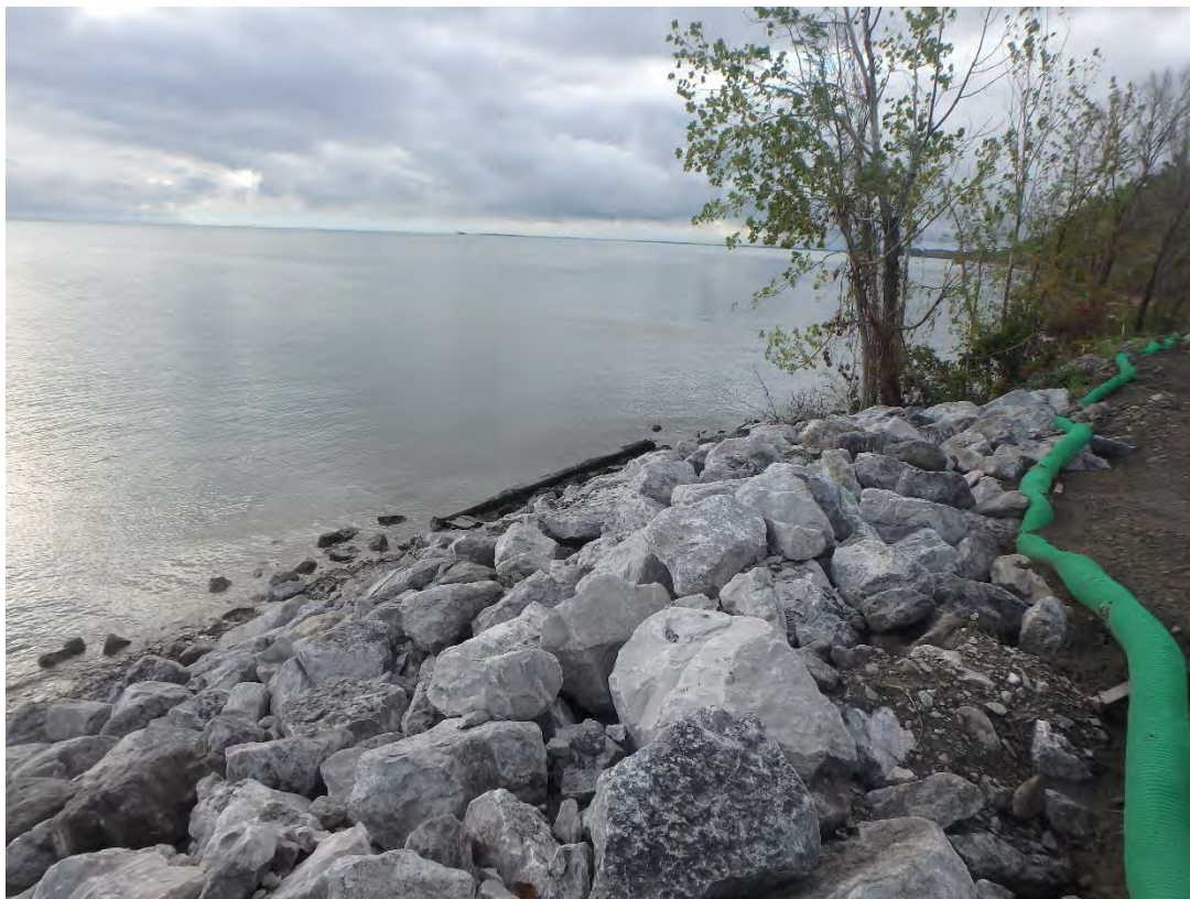
Rip-Rap along shoreline east of Pond 2, looking south.
