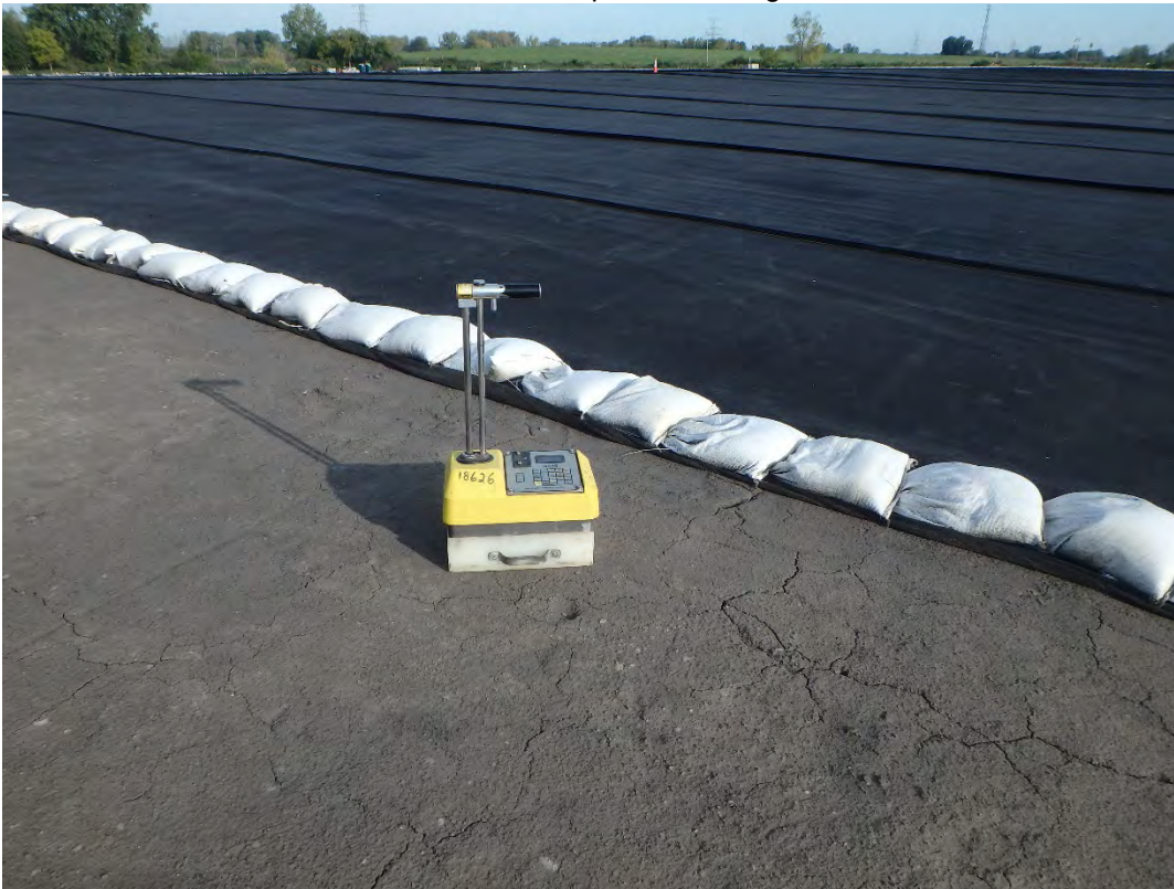
Performing standard test on density gauge prior to testing, looking northwest.
