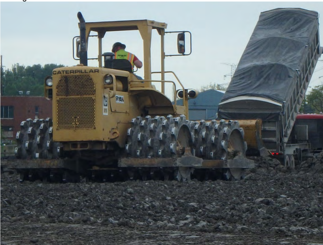
Compacting placed lift of structural fill in Pond 2, looking west.
