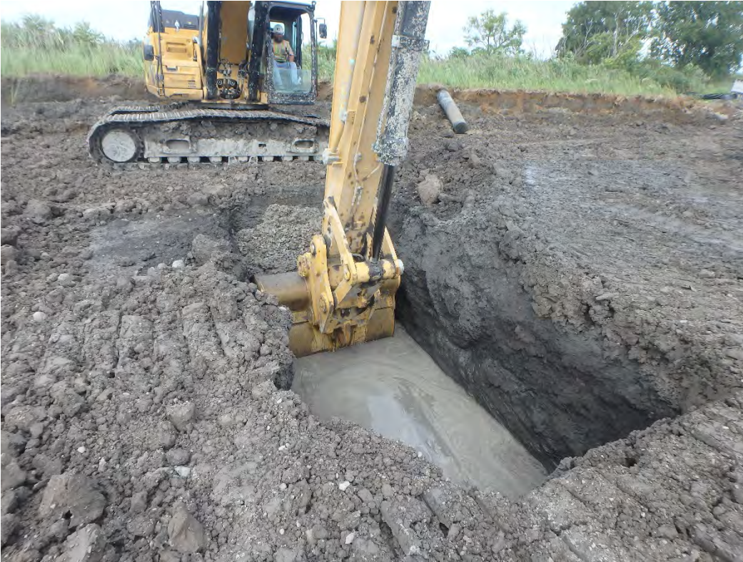
Excavation of French Drain trench to remove drainage stone and install clay plug, looking west.
