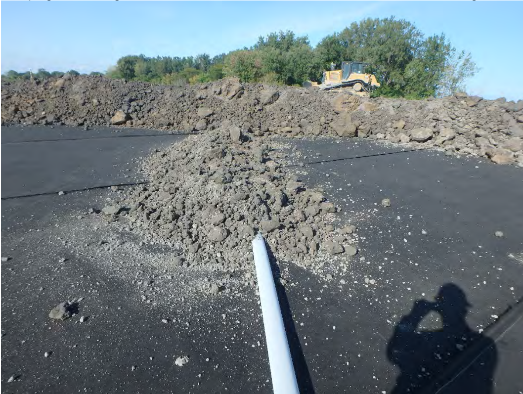
Protective cover placed atop the 4 inch ADS perforated drain pipe in Pond 1, looking northeast.
