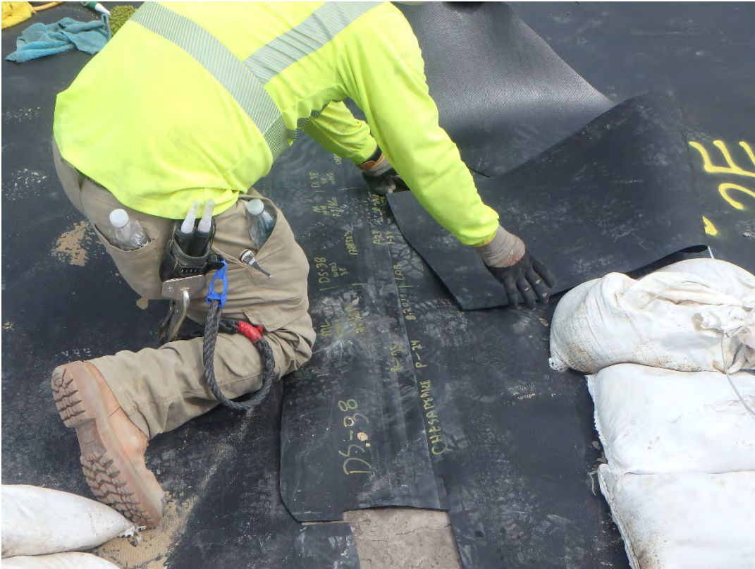
Removing marked destruct for field testing.
