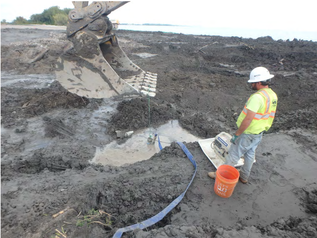
Pumping water from the southeast corner of Pond 2, looking northeast.
