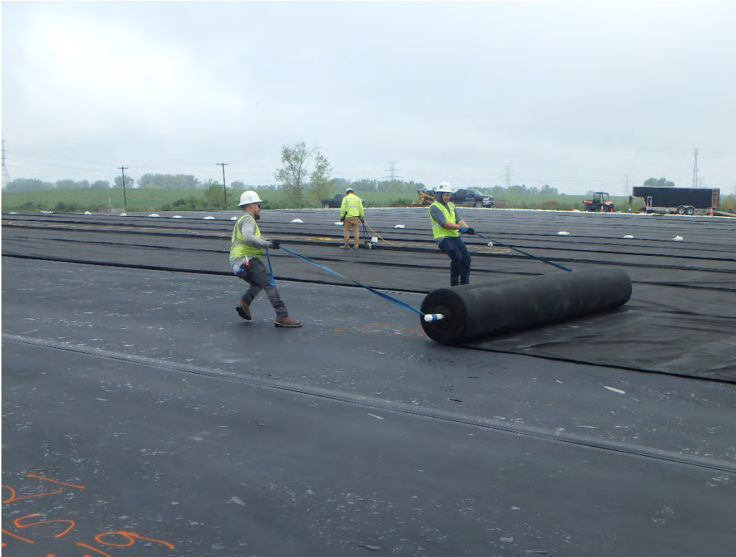
Deployment of geotextile in Pond 1, looking northwest.
