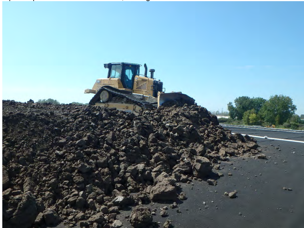
Placement of protective cover over geosynthetics in Pond 1, looking northwest.
