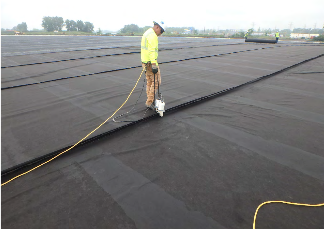
Sewing of geotextile panel seam, looking southwest.
