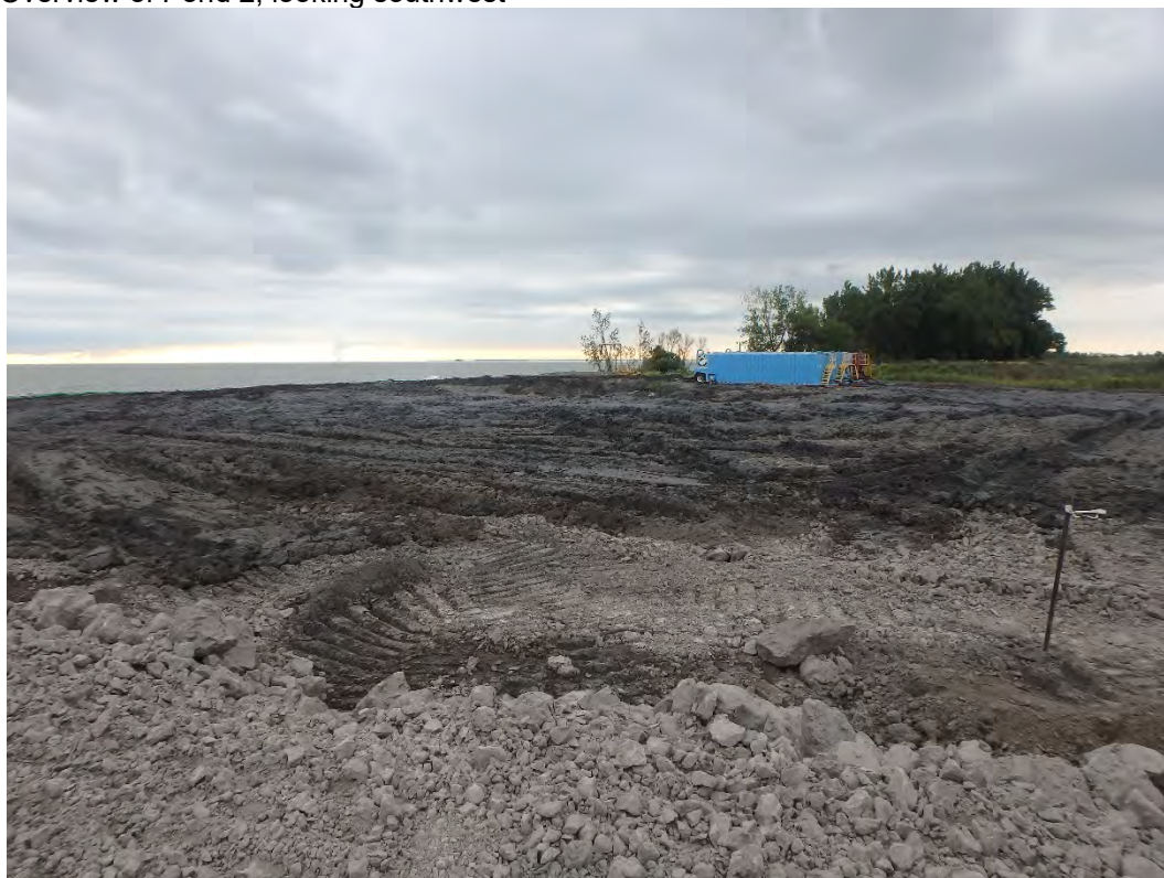
Overview of Pond 2's southeast corner, looking southeast.
