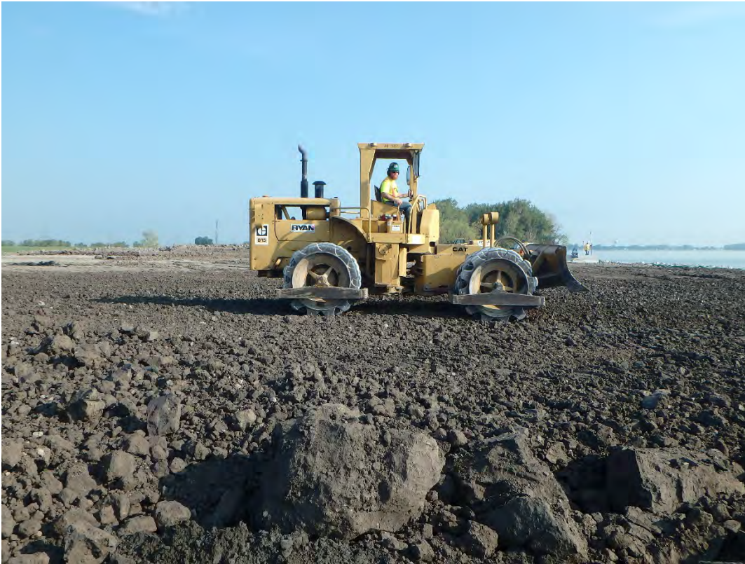
Compaction of placed structural fill in Pond 2, looking north.
