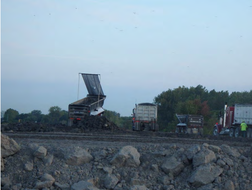
Protective cover import to Pond 1, looking north.
