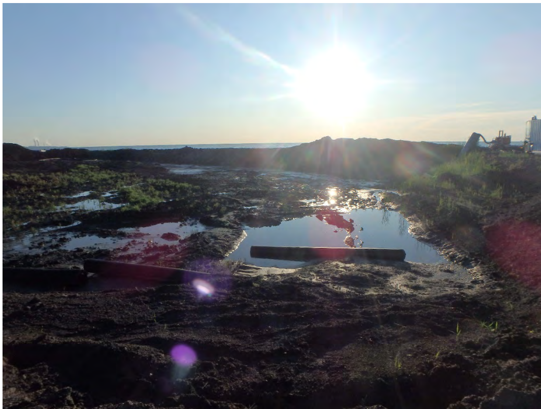
Southeast corner of Pond 2, looking east.
