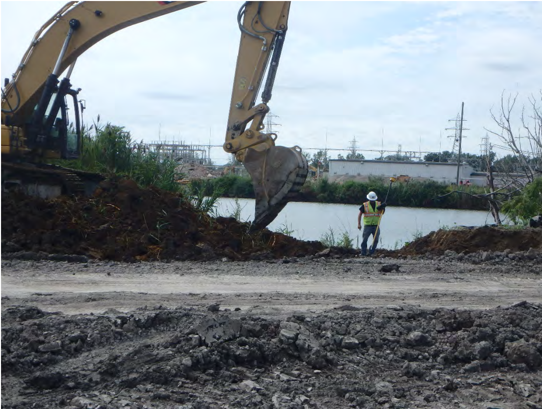
Excavating along fore bay west of Pond 2, looking west.
