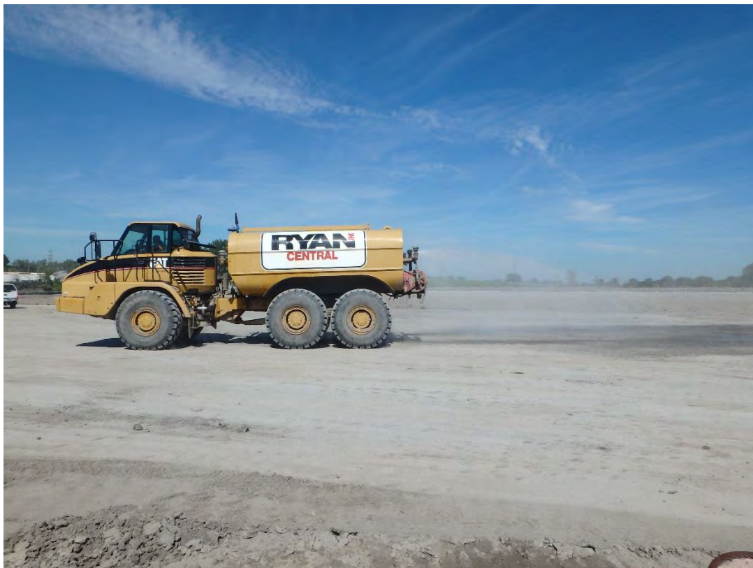
Water truck used for dust control and moisture conditioning of prepared sub-grade, looking north.
