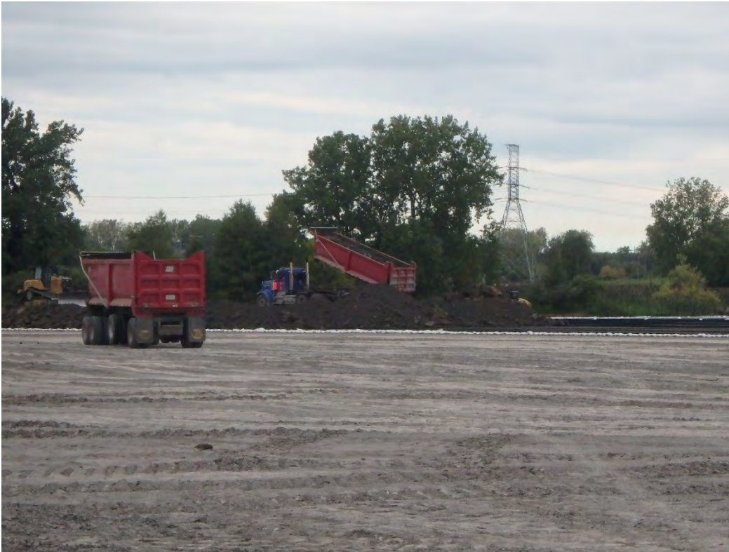
Protective cover import to Pond 1, looking northwest.
