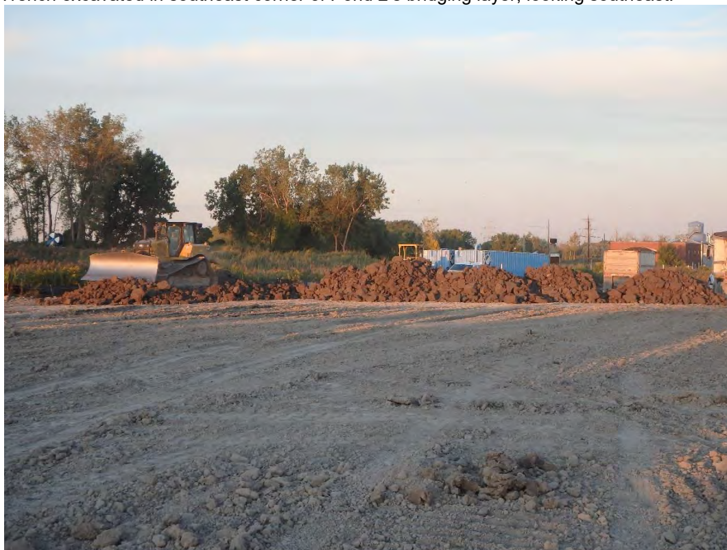
Placement of structural fill outside Pond 2 liner limits, looking southwest.
