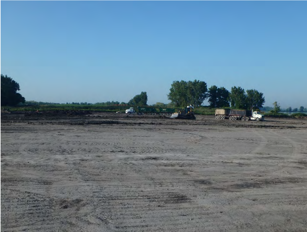
Deployment of geotextile in Pond 1, looking northwest.
