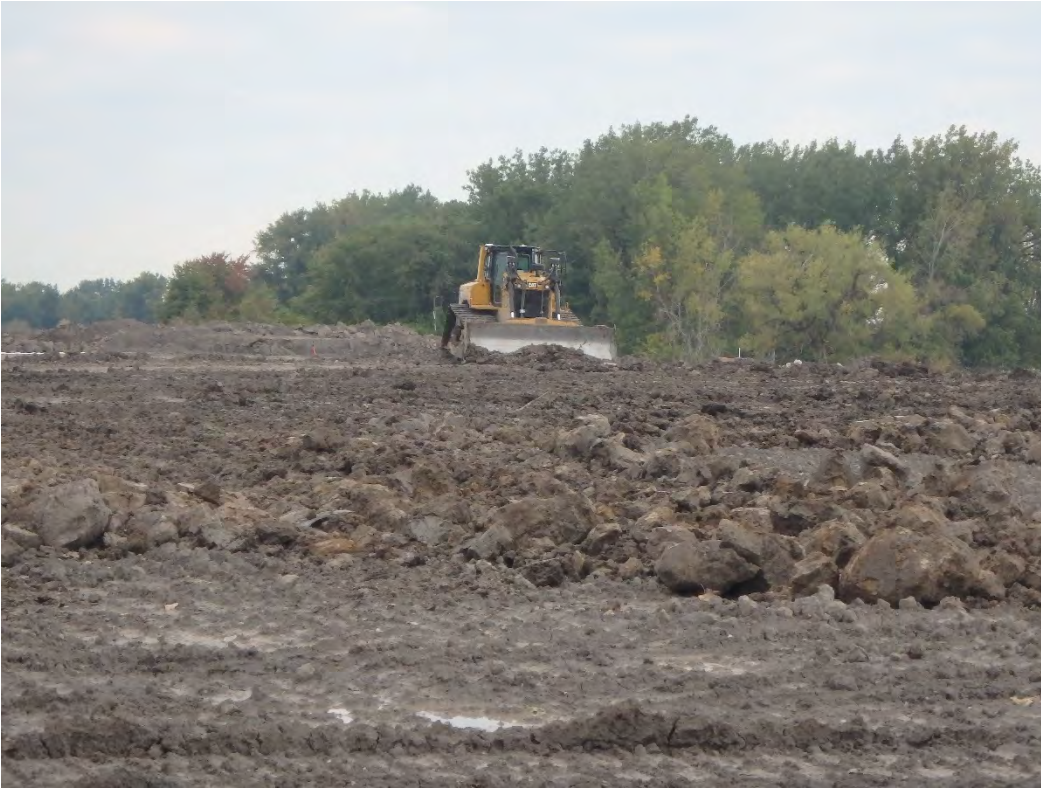
Finish grading of structural fill in Pond 2, looking north.
