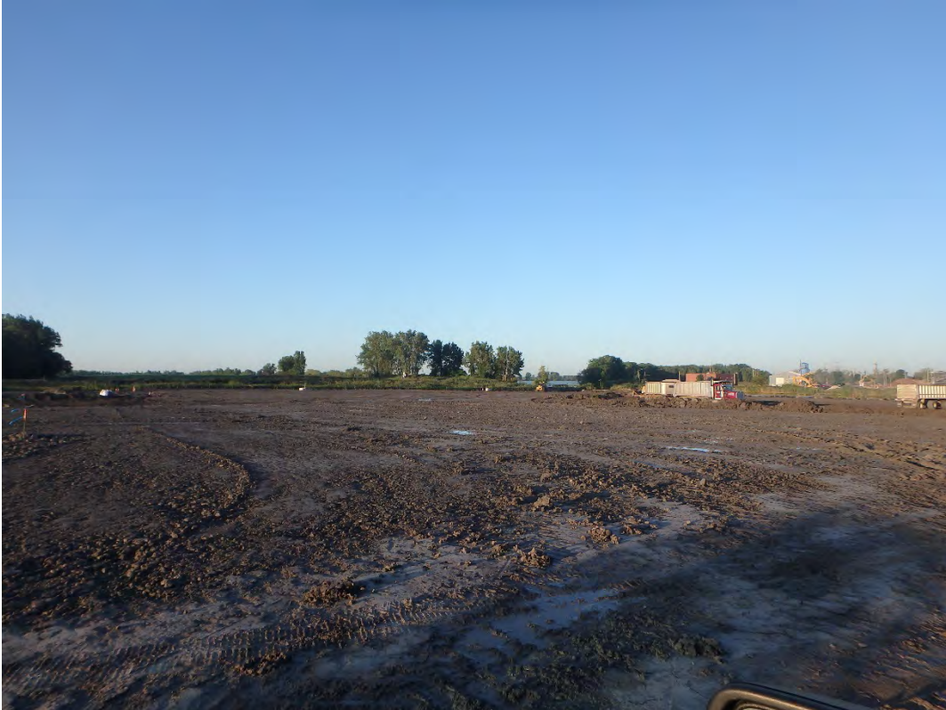
Overview of Pond 2, looking southwest.
