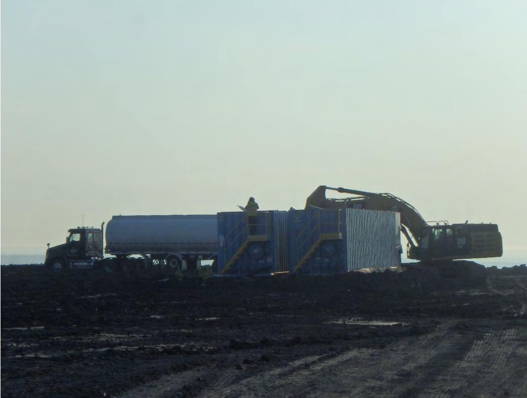
Pumping baker tanks into tanker for transport to treatment facility, looking east.
