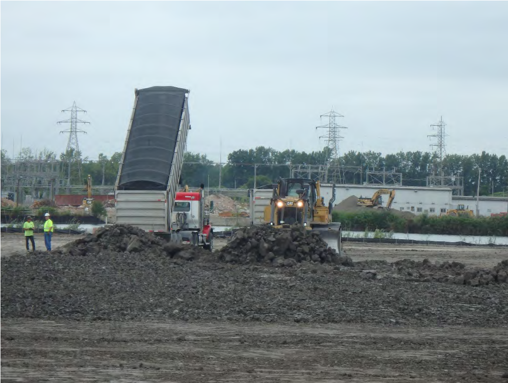
Placing lift of structural fill in Pond 2.
