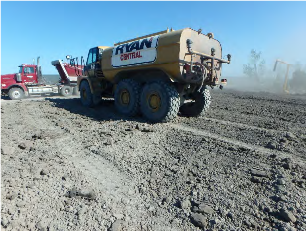
Water truck used for proof roll of bridging layer in Pond 2, looking east.
