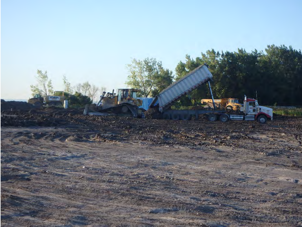
Structural fill import to Pond 2, looking southeast.
