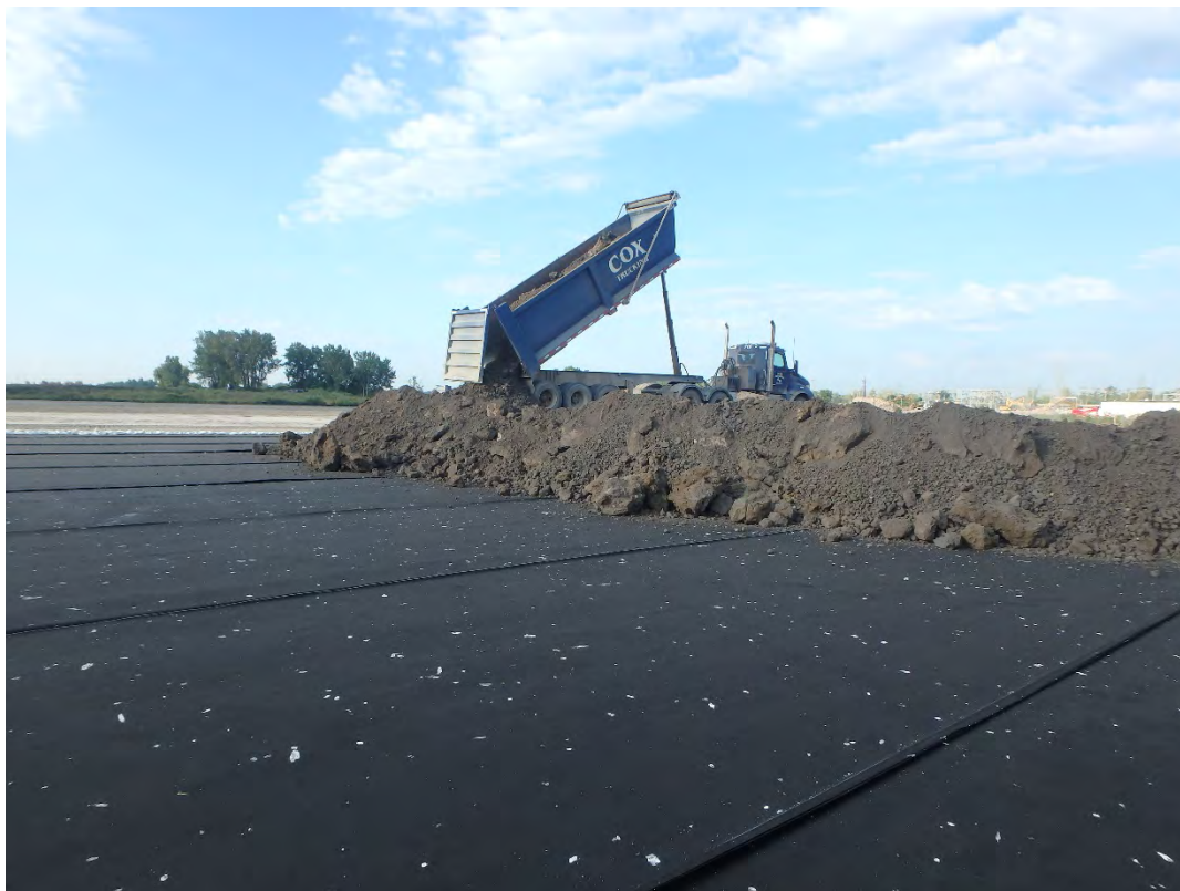
Import of protective cover to Pond 1, looking southwest.
