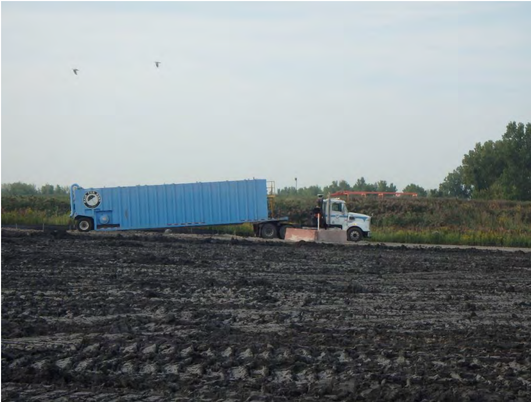
Demobilization of Baker Tank from Pond 2, looking south.
