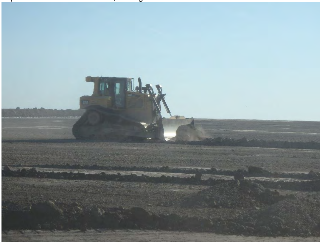
Finish grading of liner sub-grade in Pond 2, looking east.
