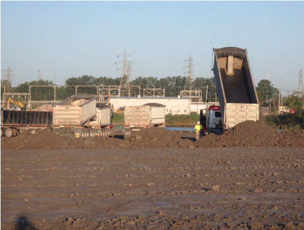
Structural fill import to Pond 2.
