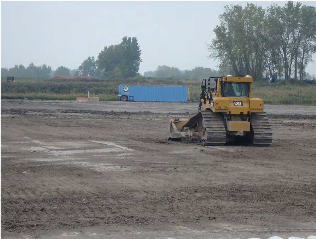
Finish grading of structural fill in Pond 2, looking South.
