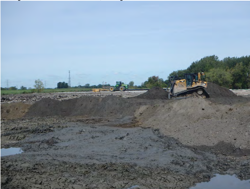
Placing bridging layer in Pond 2, looking north.
