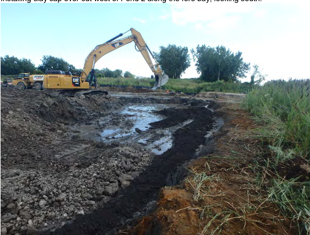
Excavating along fore bay west of Pond 2, looking south.
