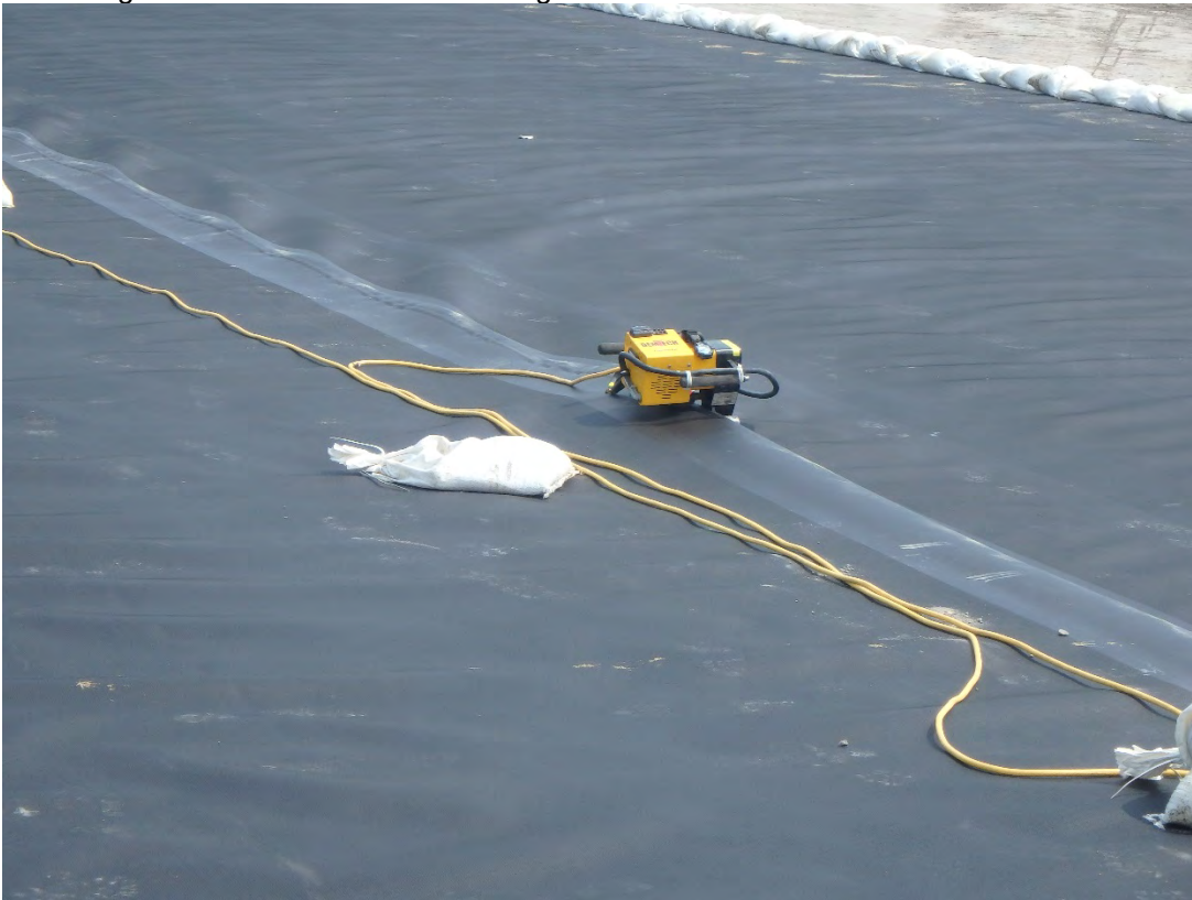
Seaming of geomembrane panels by fusion method.
