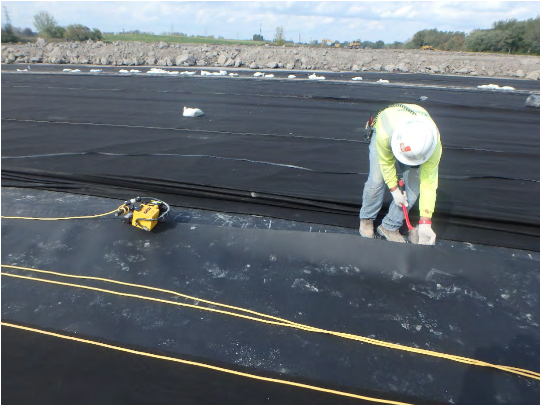
Fusion seaming of geomembrane panels.
