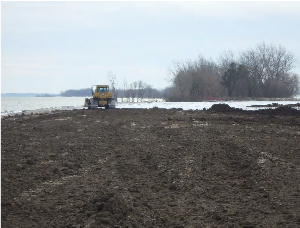
Placement of topsoil along east side of Ponds 1 and 2, looking south
