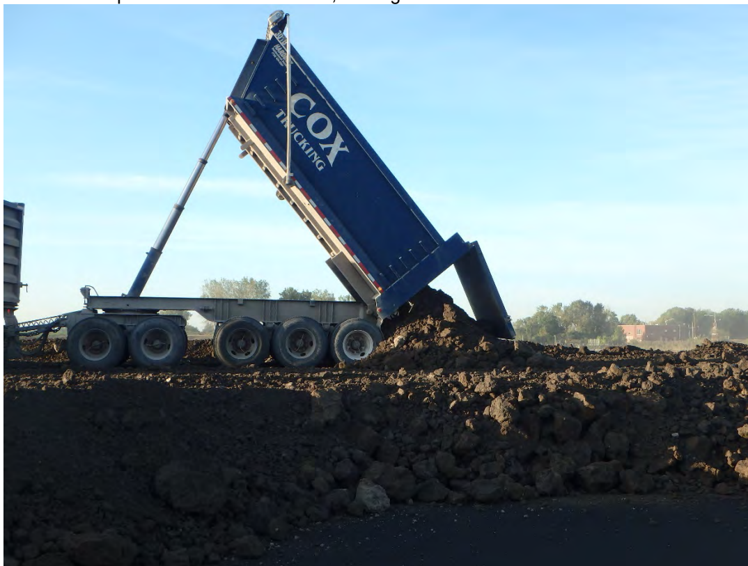
Import of protective cover in Pond 1, looking south.
