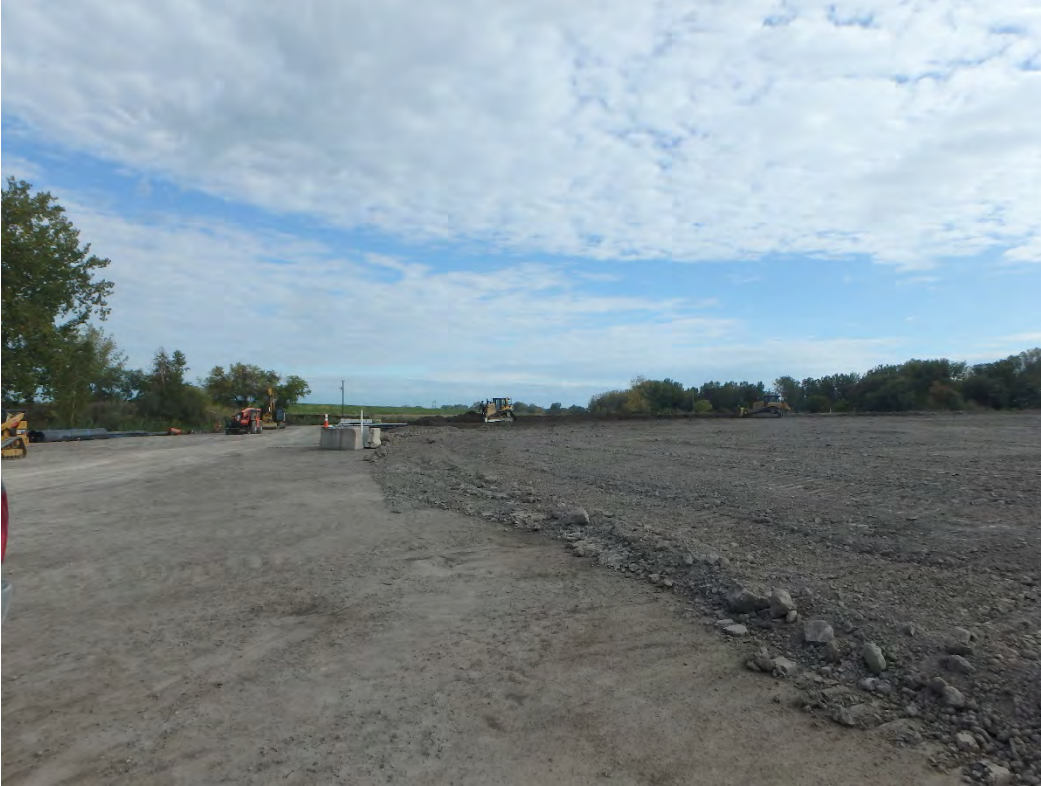
Protective cover in Pond 1, looking north.
