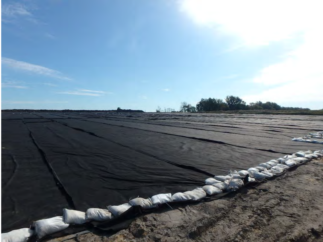
Overview of Pond 2, looking southeast
