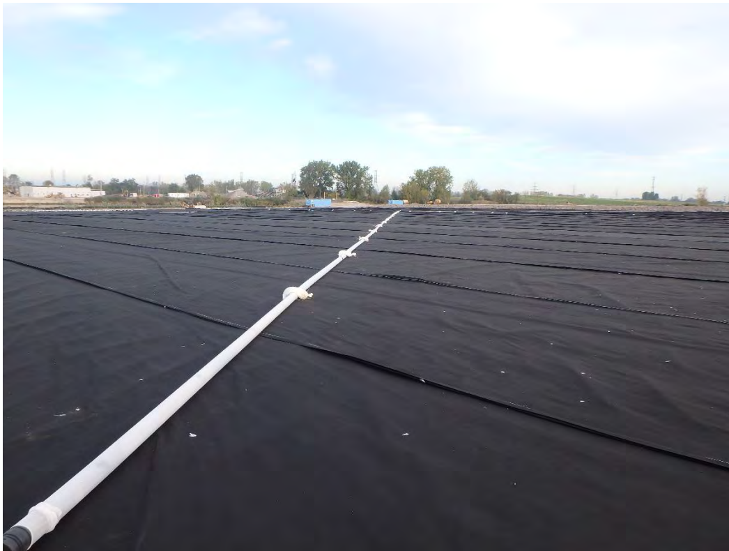
Above-cap drain pipe installed in Pond 2, looking northwest
