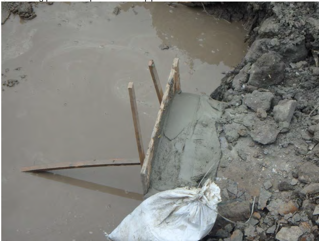
Finished 24 inch pipe cap
