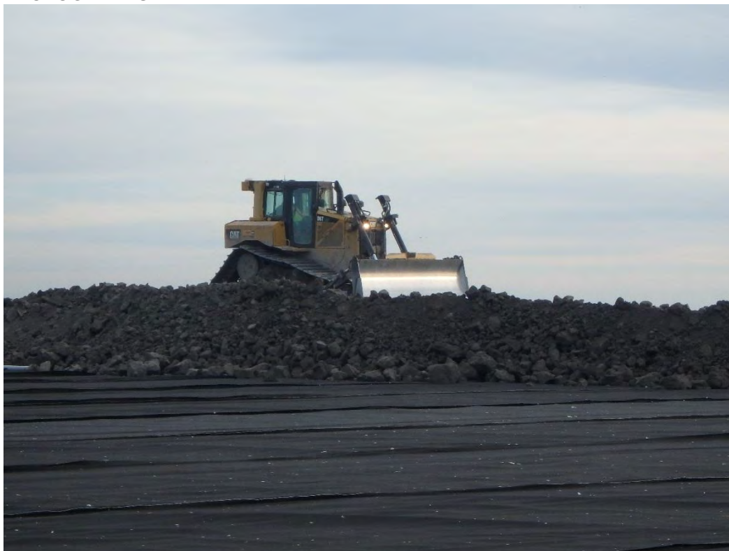
Placing protective cover in Pond 2, looking northeast
