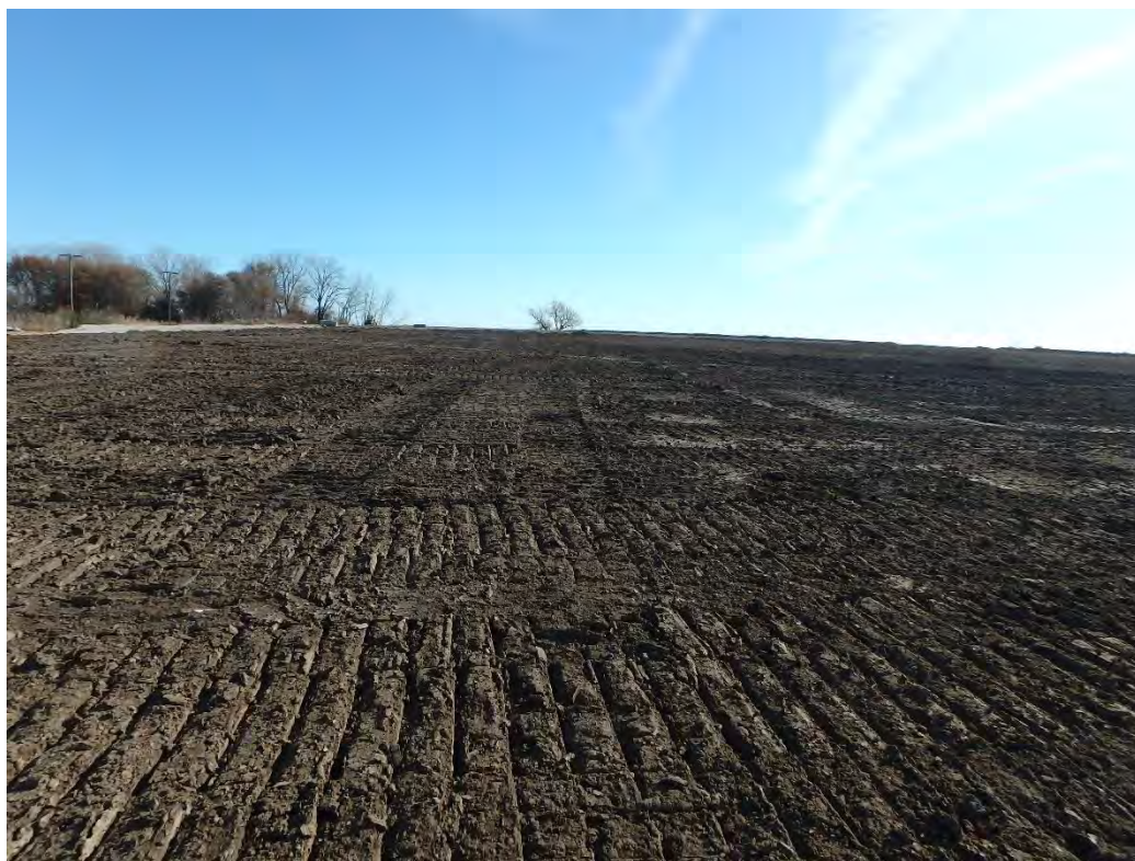
Overview of topsoil placement in Pond 1, looking east
