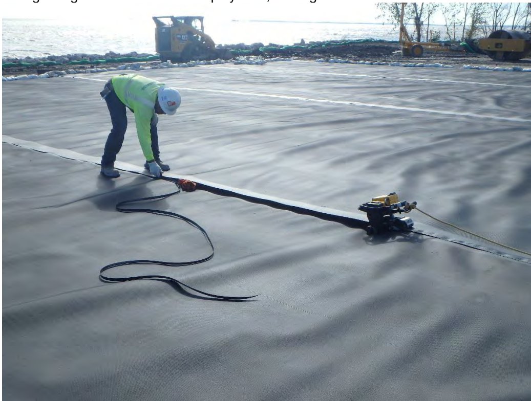
Fusion welding of seam in Pond 2, looking southeast
