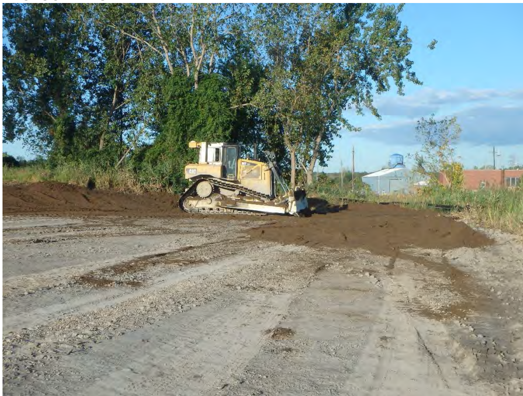
Placement of topsoil in the Chemical Pond work area, looking west.
