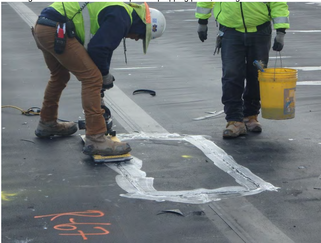
Vacuum testing of extrusion weld on repair patch
