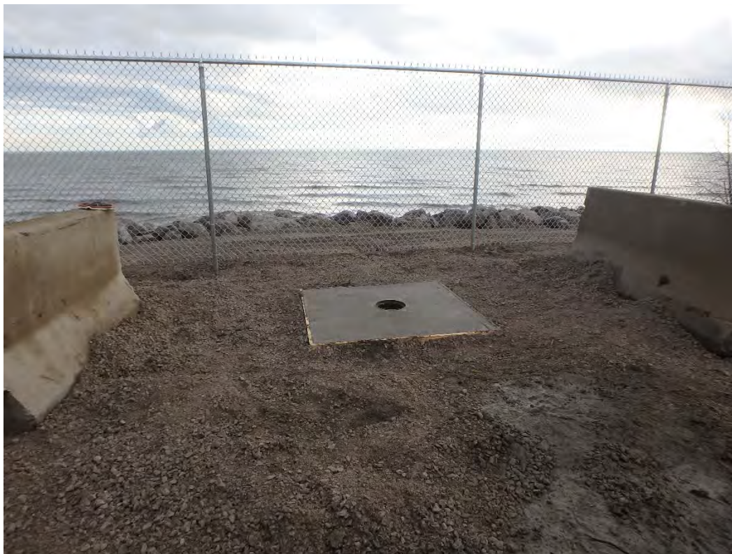
MW-15003 ground flush in east access road
