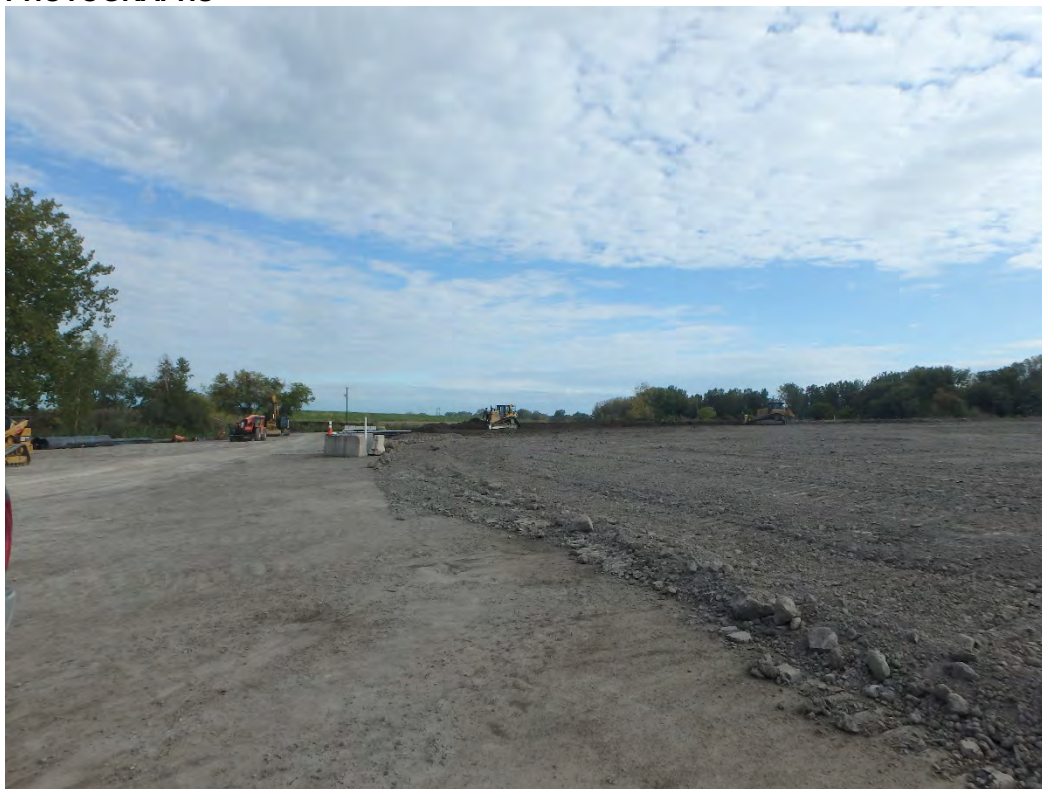
Protective cover in Pond 1, looking north.
