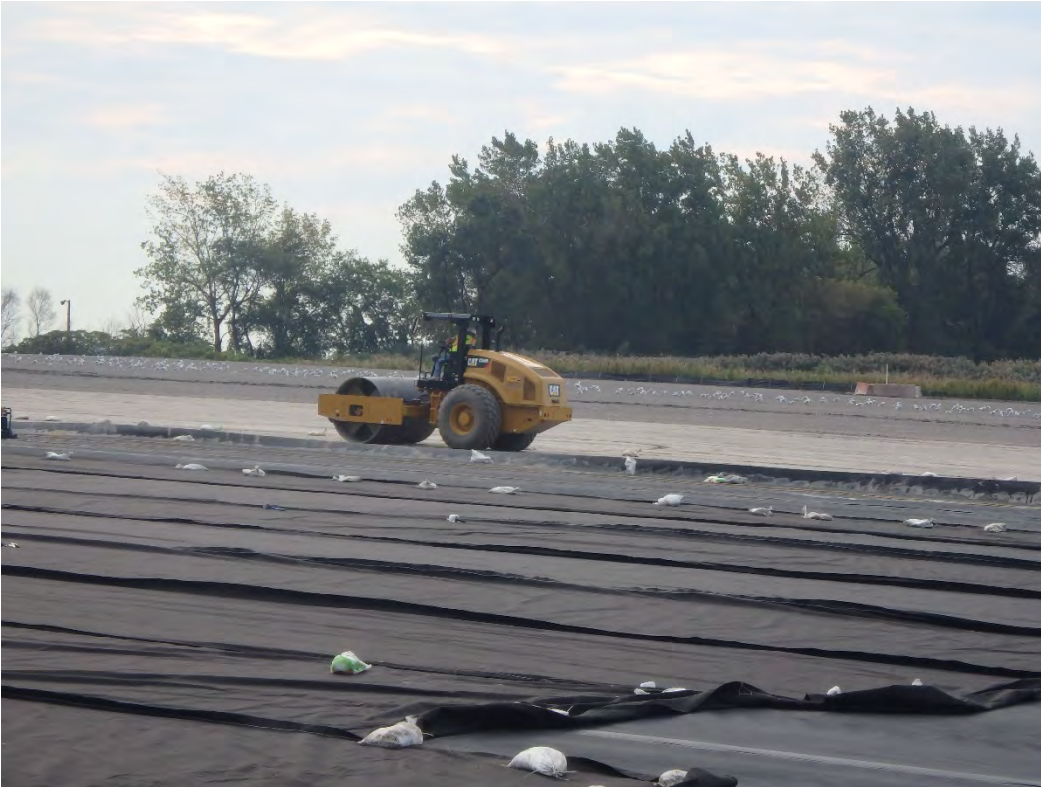
Rolling sub-grade ahead of liner deployment, looking south
