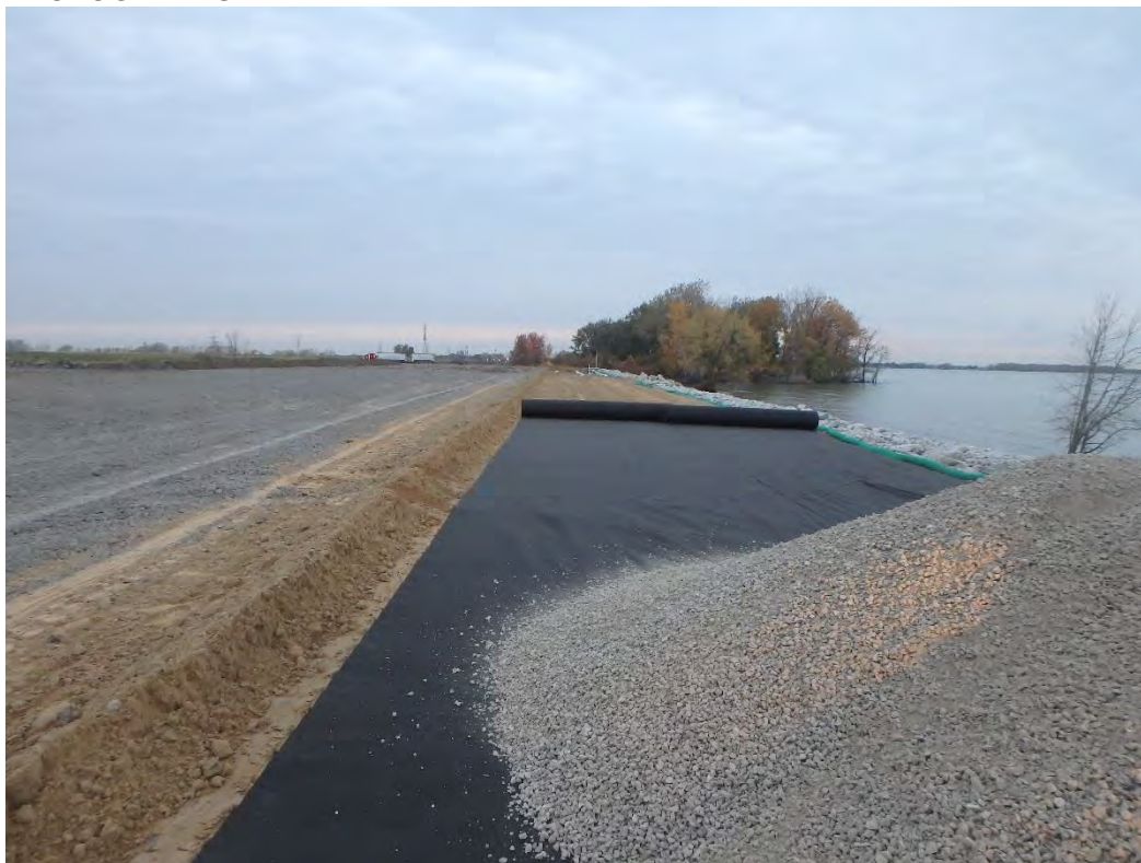
East access road, looking north
