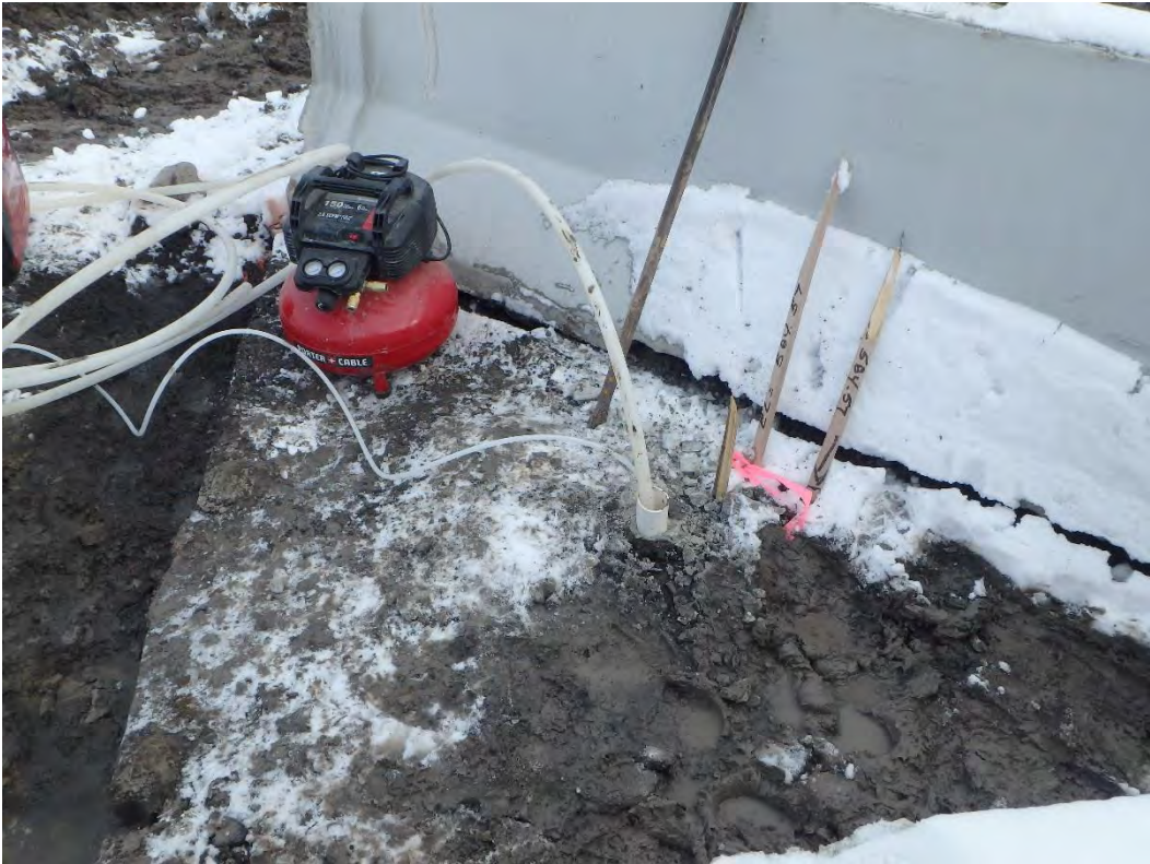
Preparing to flush MW-15006
