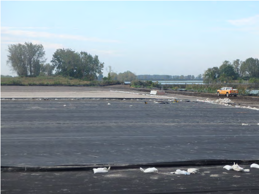
Overview of geosynthetics in Pond 2, looking south
