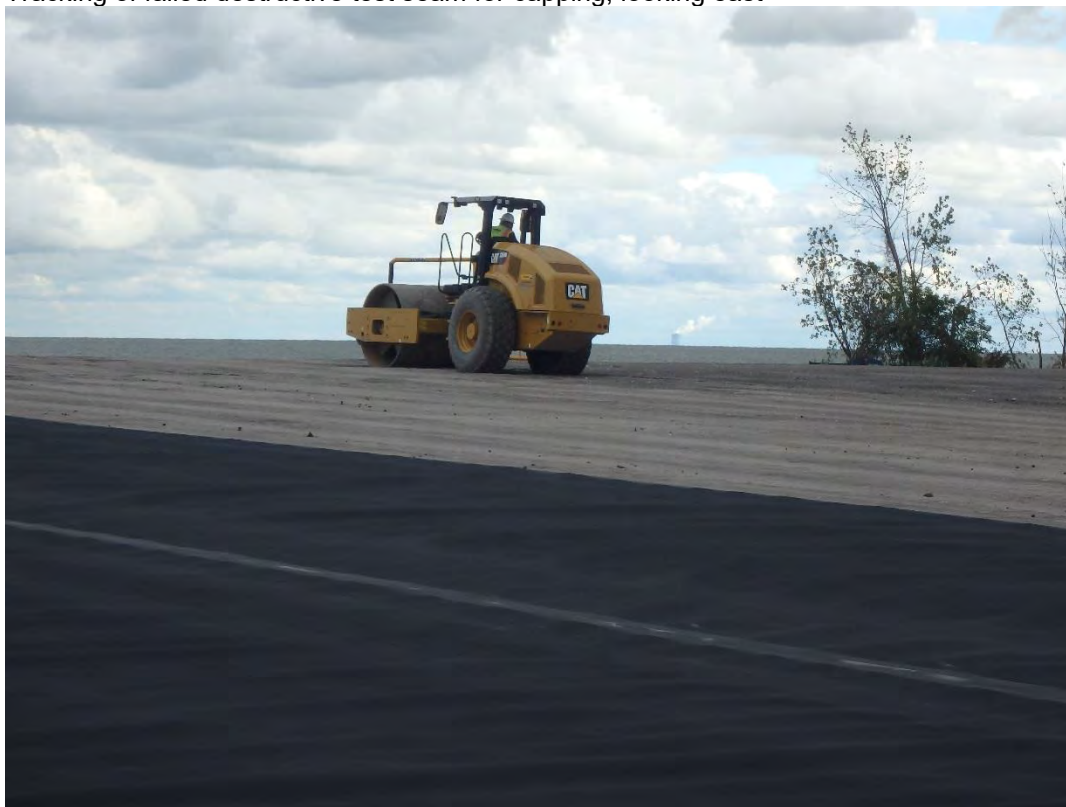
Rolling sub-grade ahead of liner deployment, looking southeast
