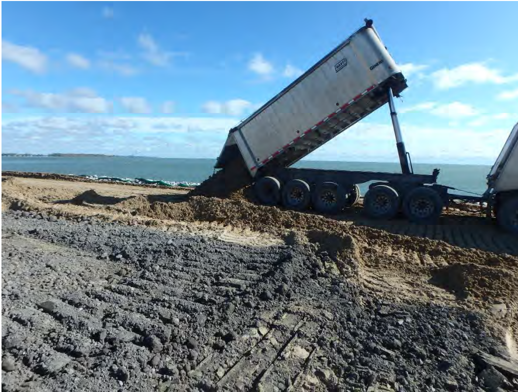
Class II sand imported for access road, looking east from Pond 2
