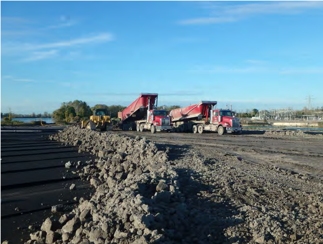
Protective cover import to Pond 2, looking southwest
