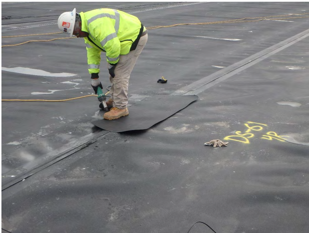
Leistering patch in preparation of extrusion welding
