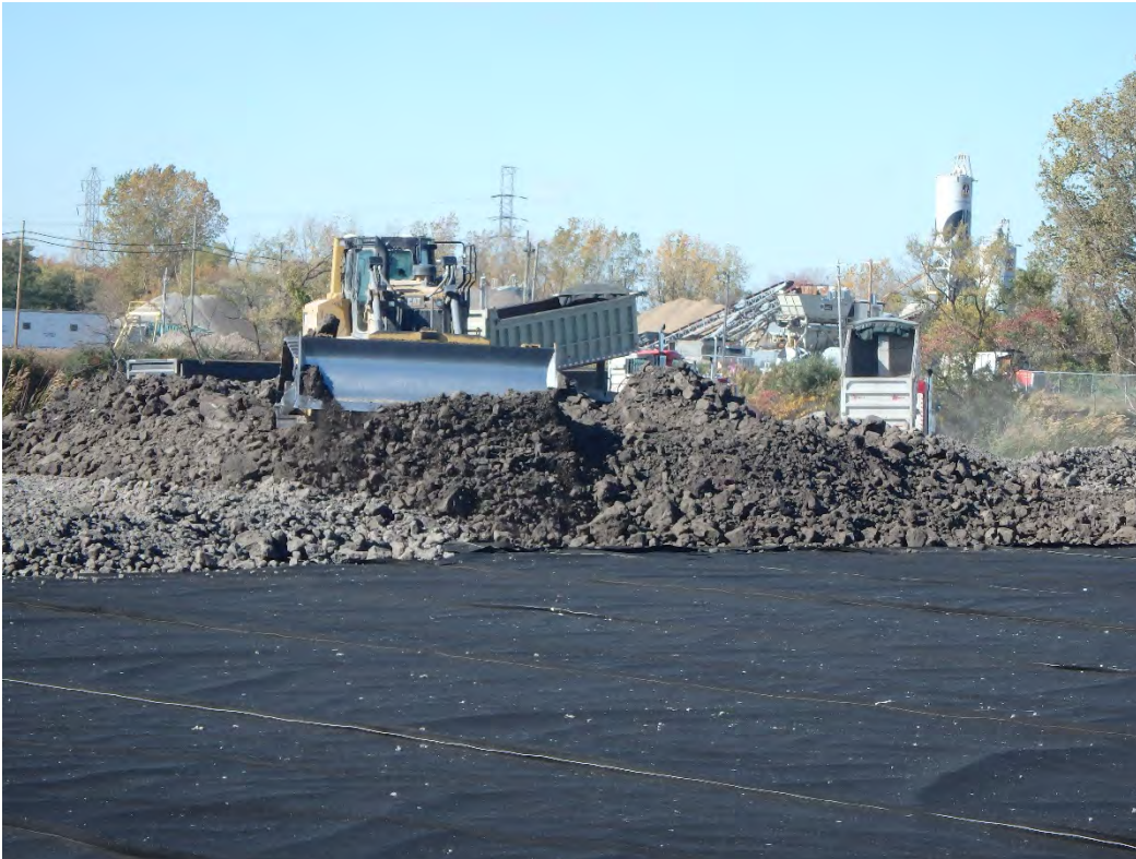
Placement of protective cover in Pond 2, looking northwest
