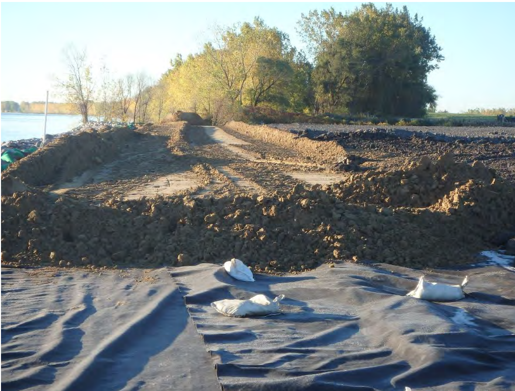
Class II placed for east access road sub-base east of Pond 2, looking south
