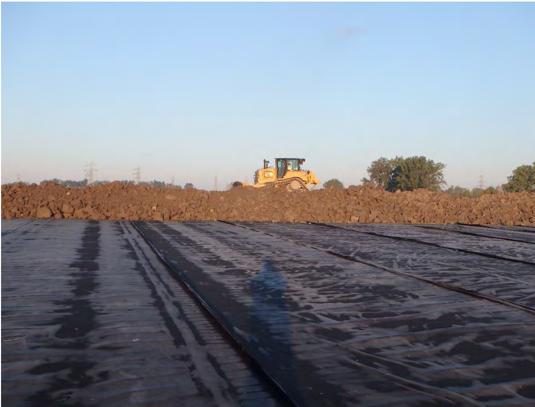
Placing protective cover in Pond 2, looking west
