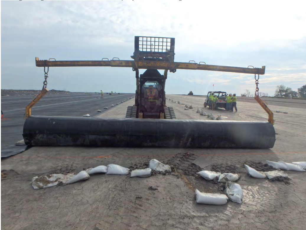
Deployment of geomembrane in Pond 2, looking east
