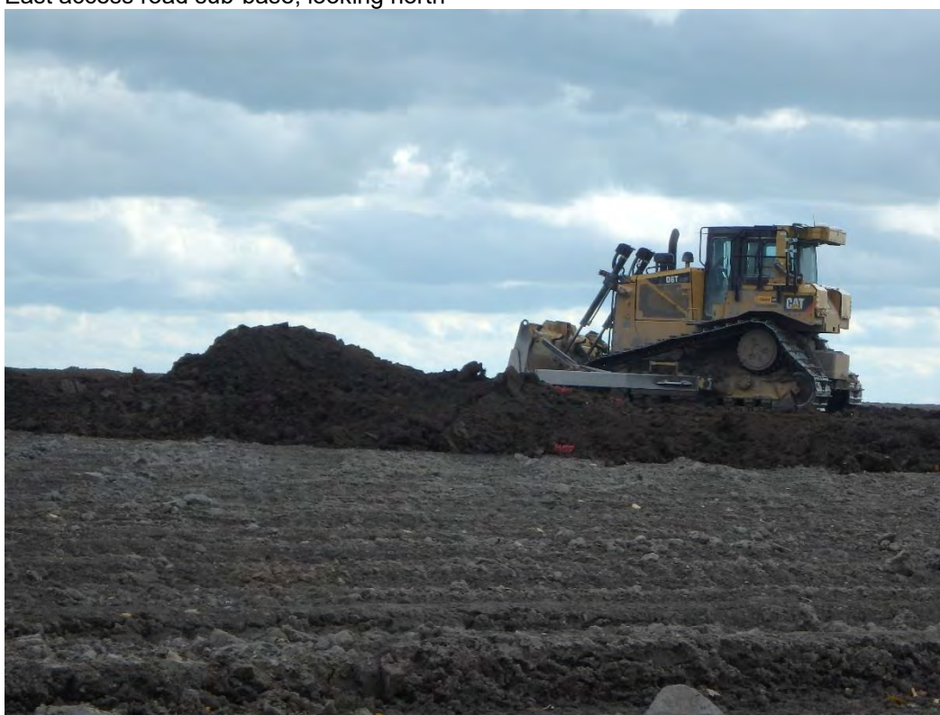
Building topsoil haul road in Pond 1, looking east
