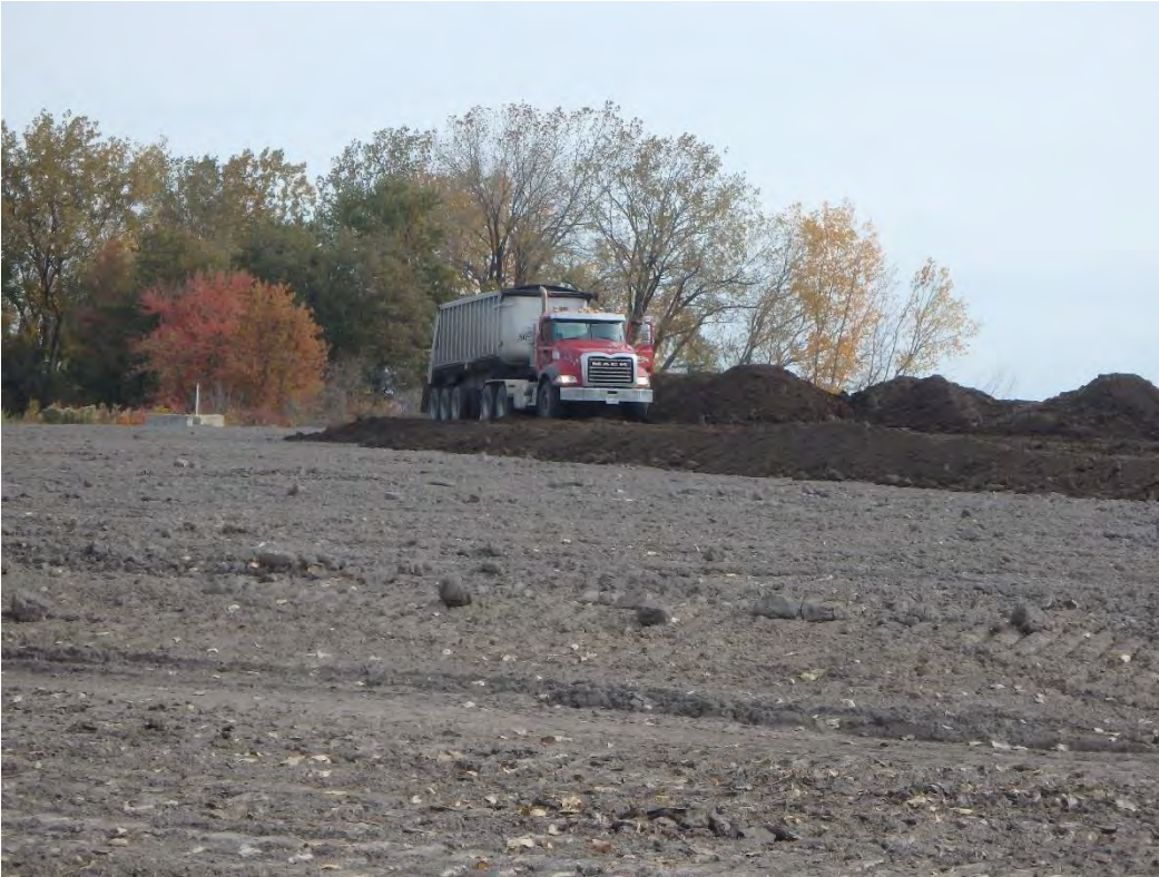
Topsoil import to Pond 1, looking northeast
