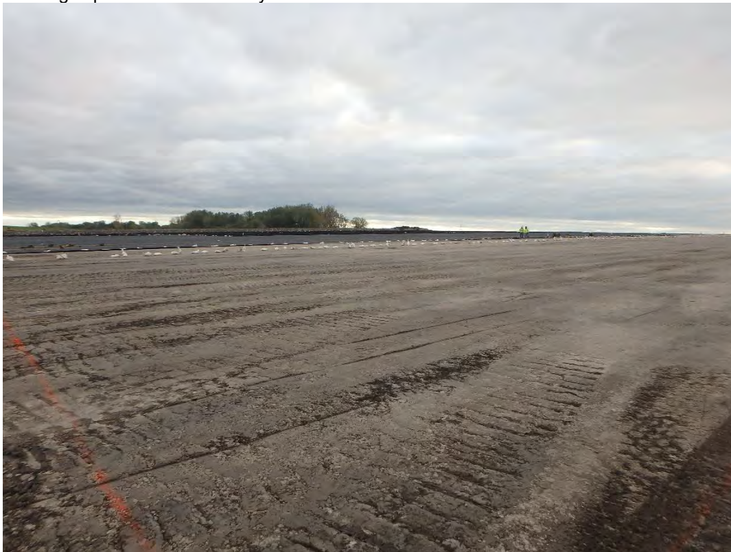
Overview of Pond 2, looking northeast
