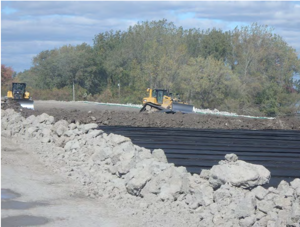
Placement of protective cover east side of Pond 2
