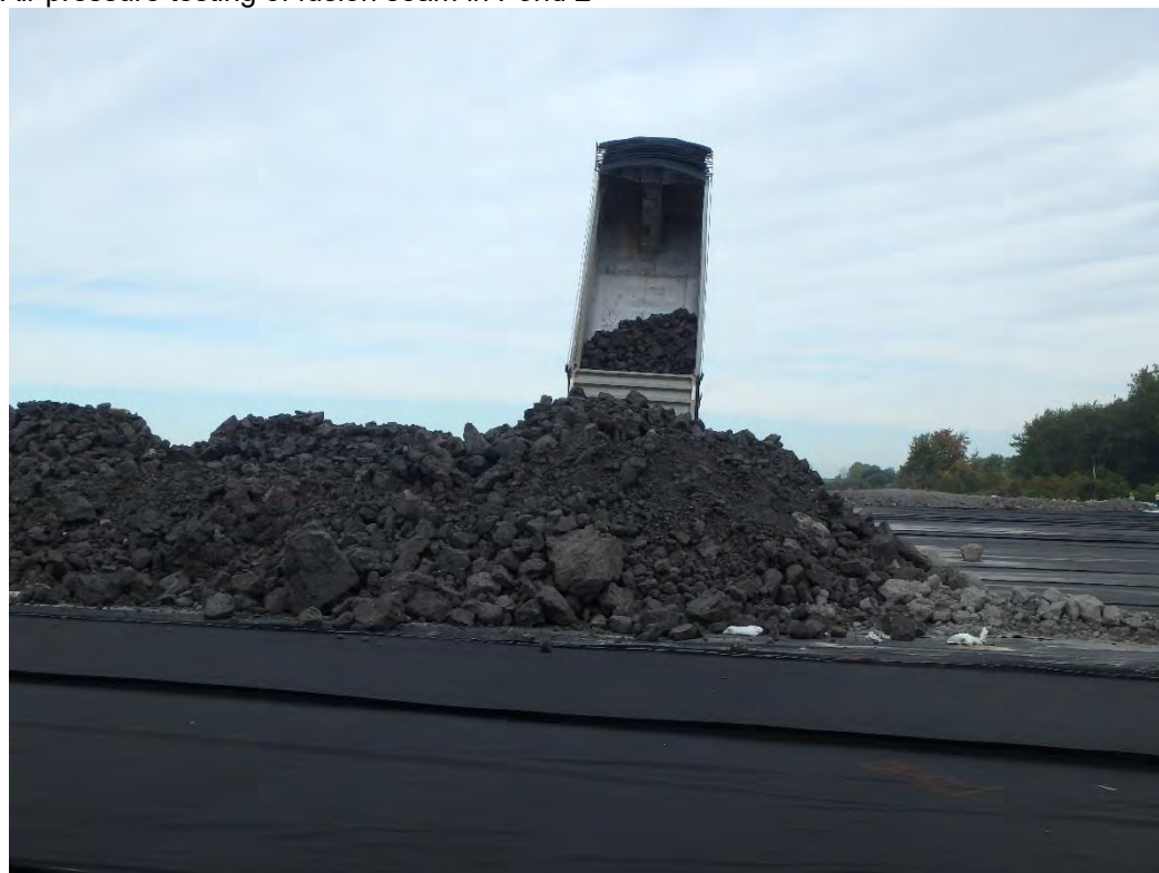
Import of protective cover in Pond 2, looking north
