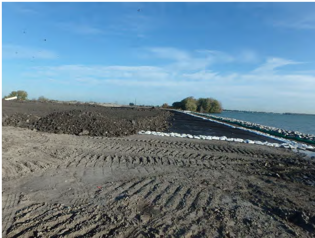
Overview of Pond 2's southeast corner, looking north
