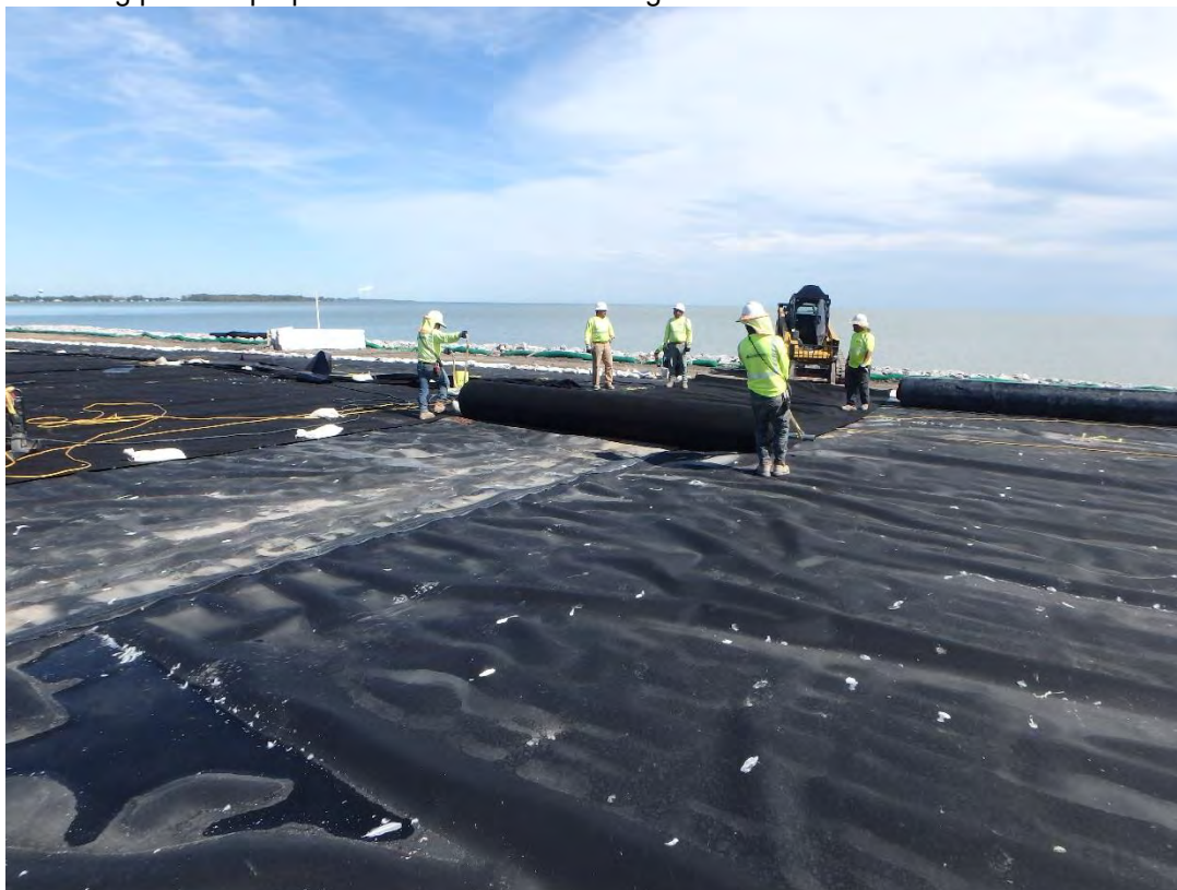
Deploying geotextile in Pond 2, looking east
