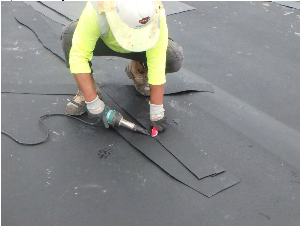
Preparing trial weld.
