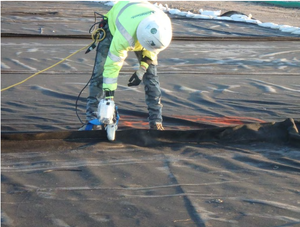
Sewing textile seam in Pond 2
