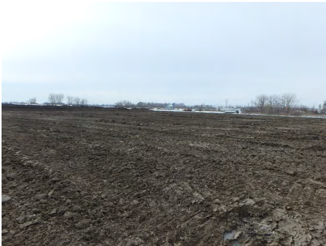
Overview of topsoil placed in Pond's 1 and 2, looking southwest
