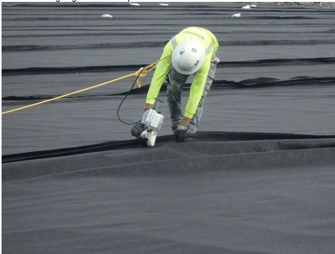
Sewing of geotextile panel seams in Pond 2.
