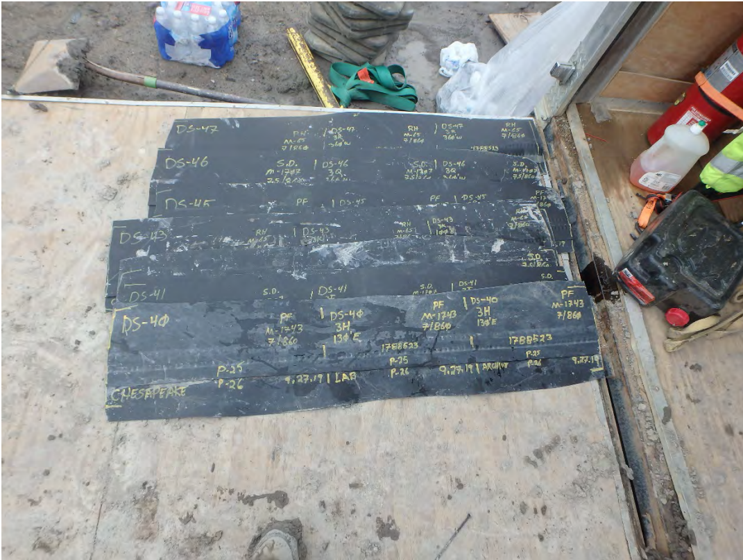
Destructive samples removed for sampling.
