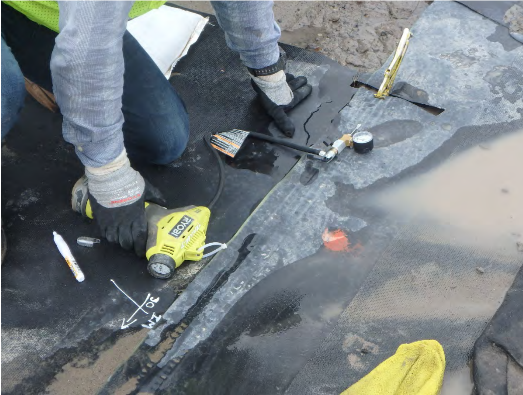
Air pressure testing of fusion seam.
