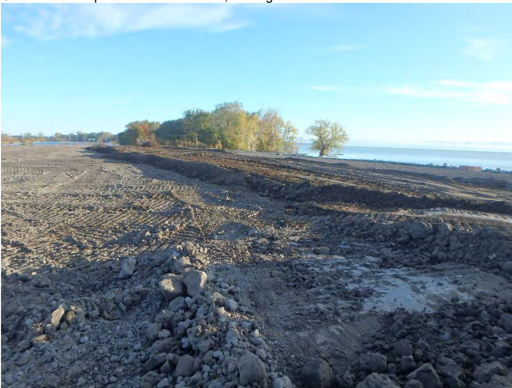
Topsoil placed in Pond 1, looking northeast
