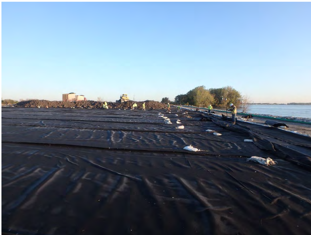
Deployment of geotextile in Pond 2, looking north
