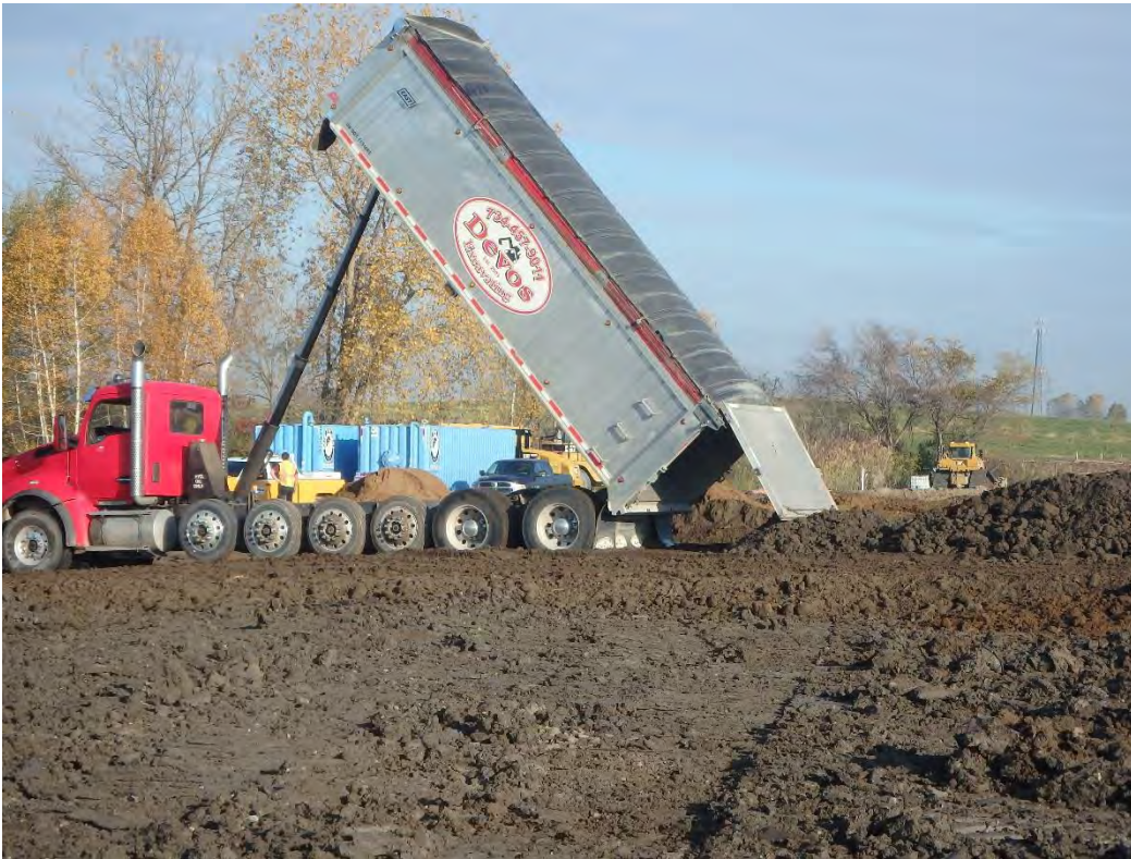
Import of topsoil to Pond 1, looking north
