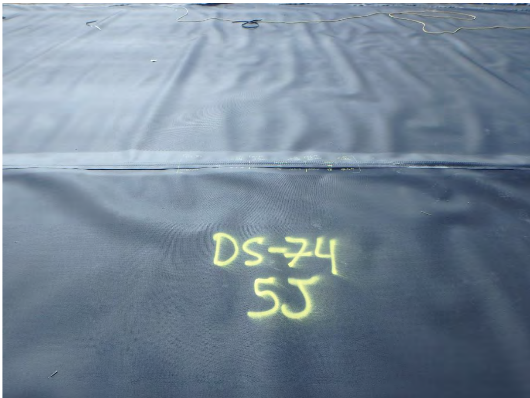
Destruct marked for removal and testing
