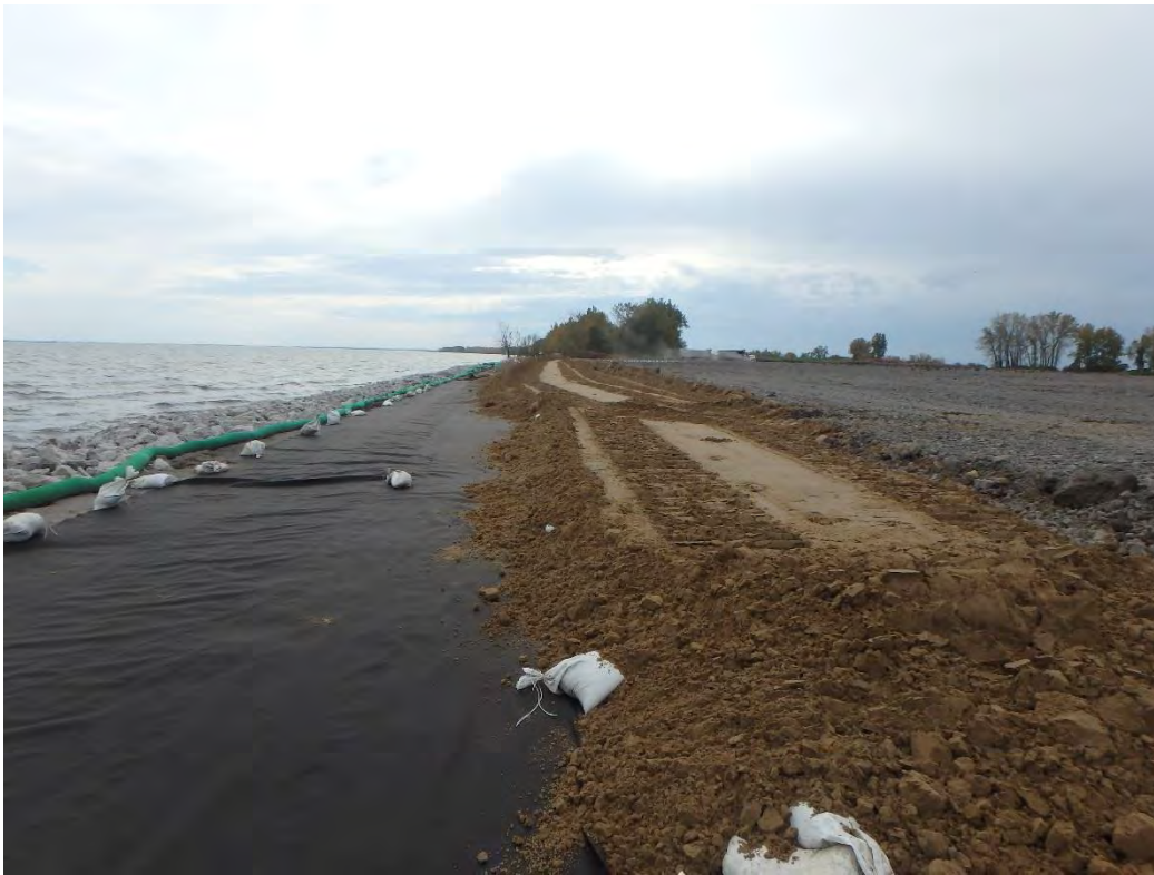
East access road sub-base, looking south
