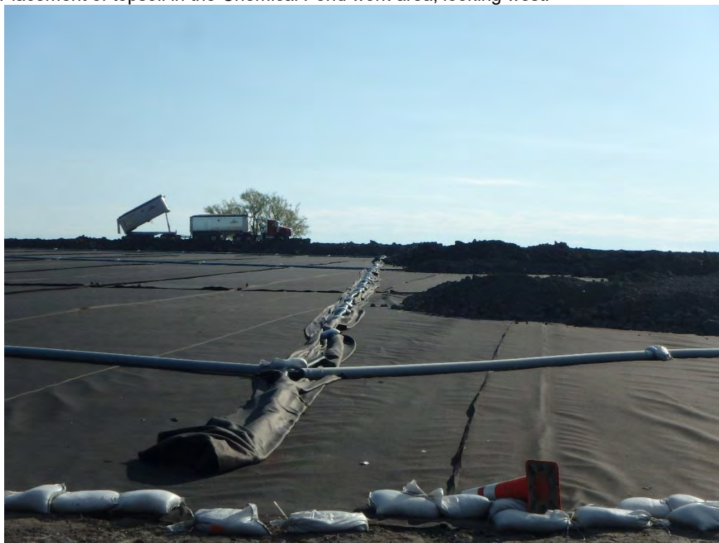
Protective cover on Pond 1 geotextile, looking east.
