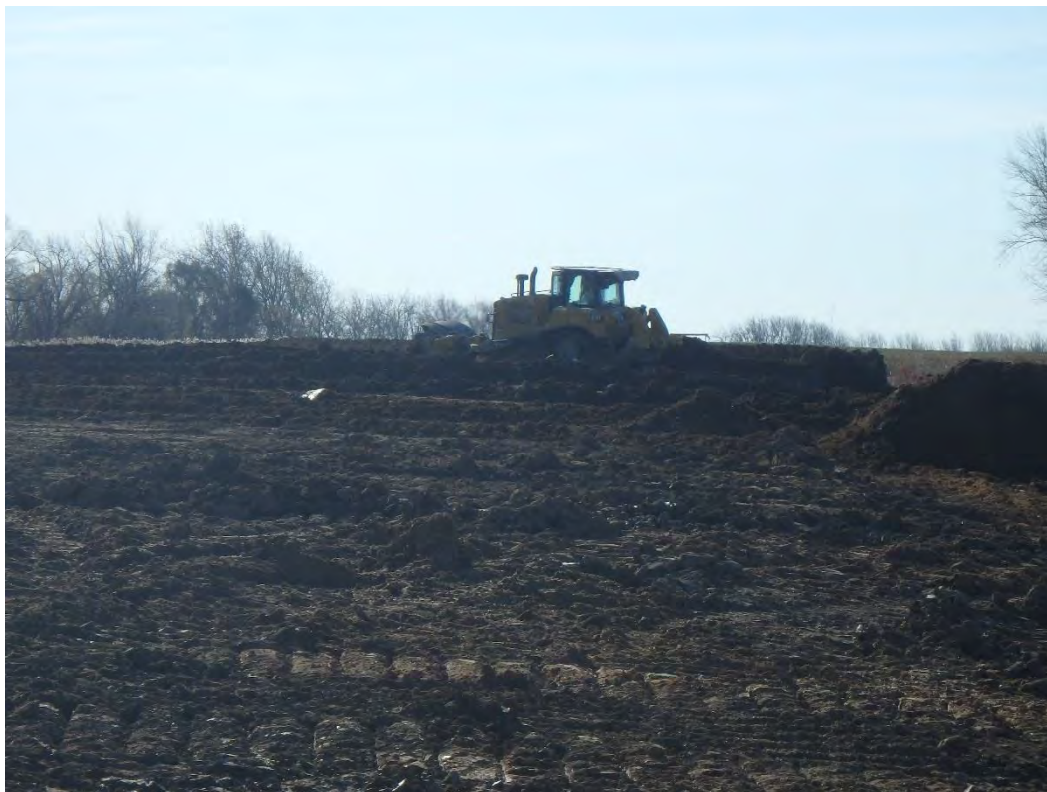
Placement of topsoil in Pond 2, looking south
