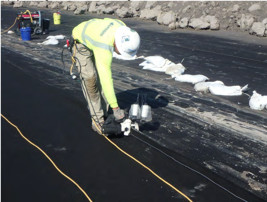
Sewing of geotextile panels.
