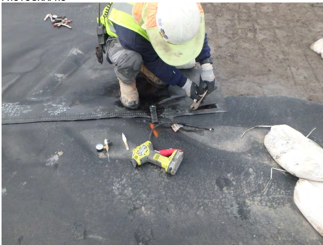
Air pressure testing of fusion seam in Pond 2
