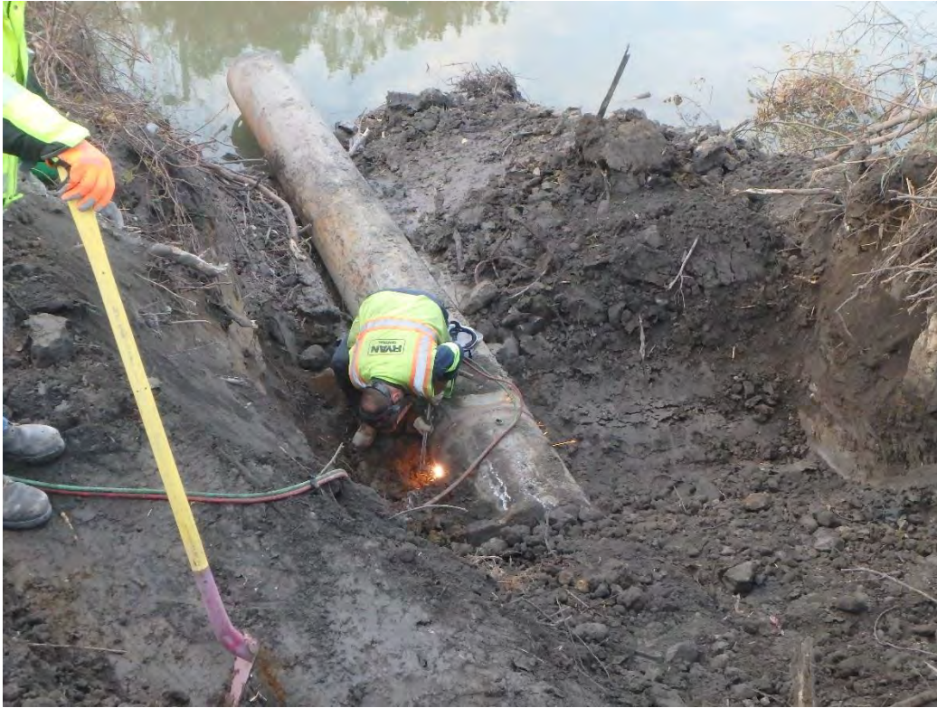
Cutting 24 inch pipe into discharge channel for removal, looking south
