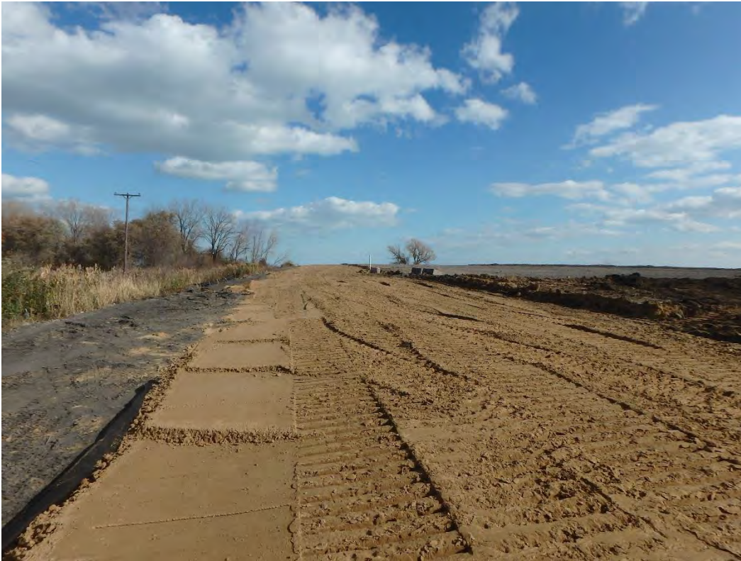
Overview of completed north access road sub-base, looking east
