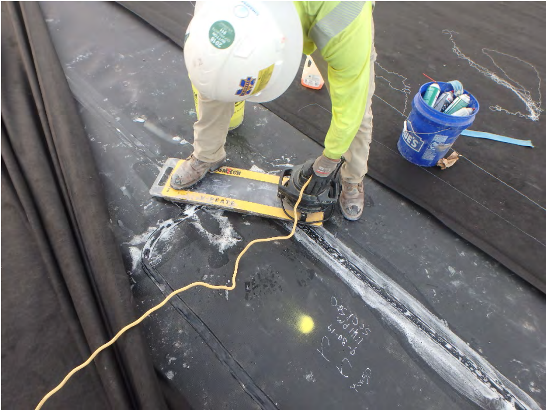
Vacuum testing of extrusion weld.
