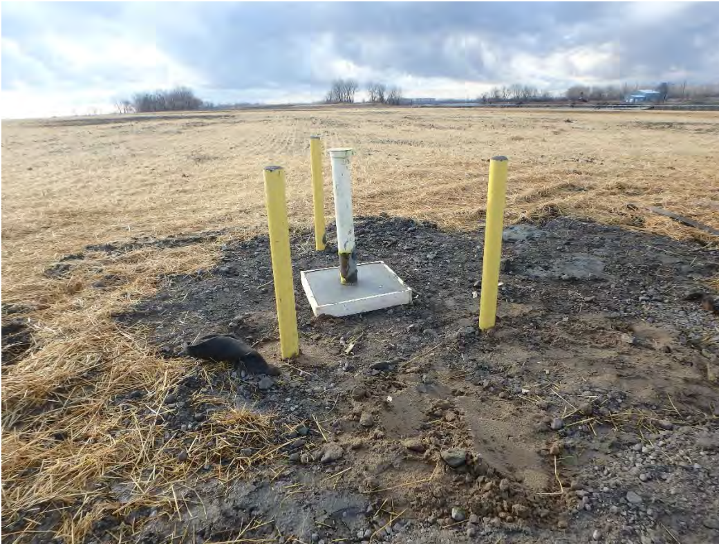
MW-15002 with protective casing and bollards installed
