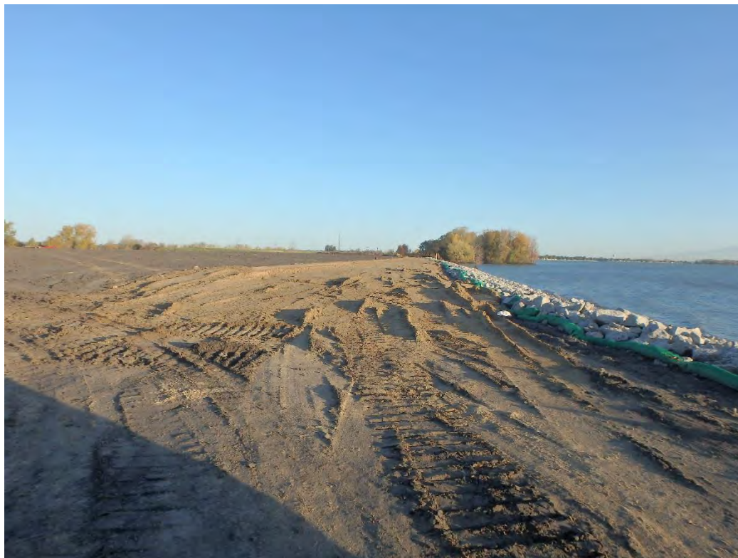
East access road sub-base, looking north
