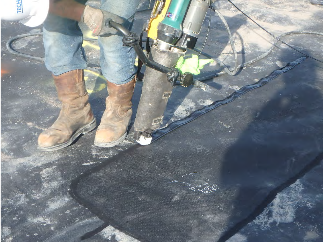
Repair using extrusion method.
