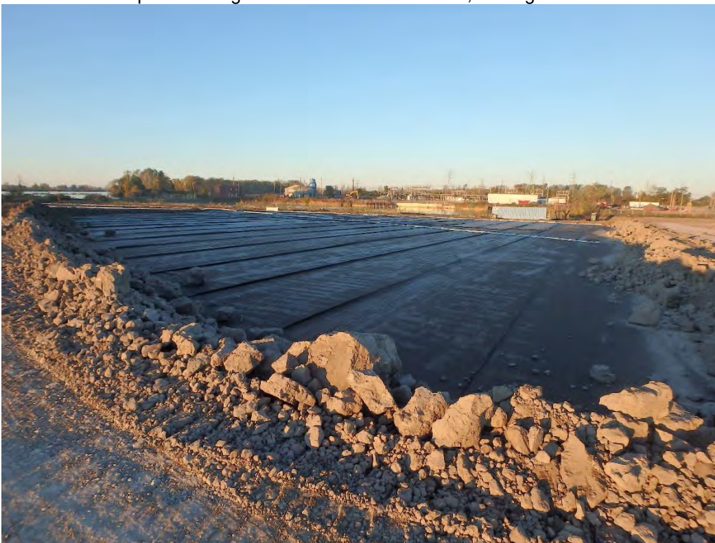
Overview of protective cover in Pond 2, looking southwest
