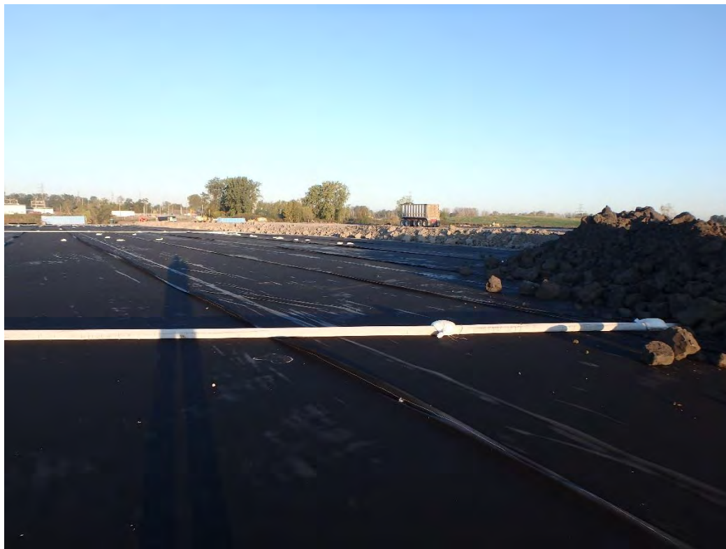
Above-Cap drain pipe installed in Pond 2
