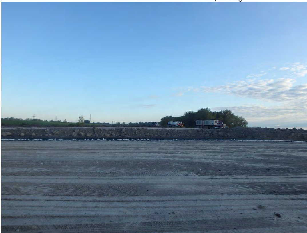
Finished liner sub-grade in Pond 2, looking north.
