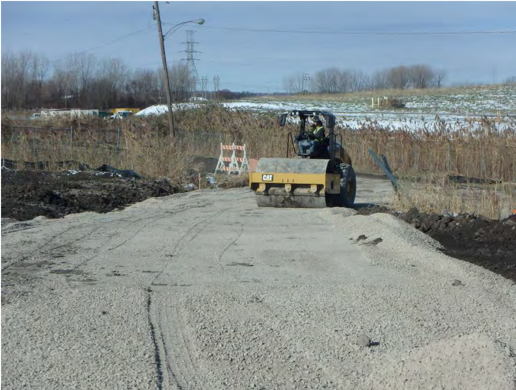
Compacting 21AA placed for access ramp using smooth drum roller, looking north
