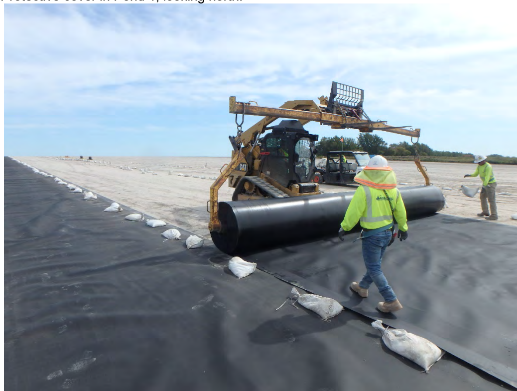
Deployment of 40mil geomembrane in Pond 2, looking southeast.
