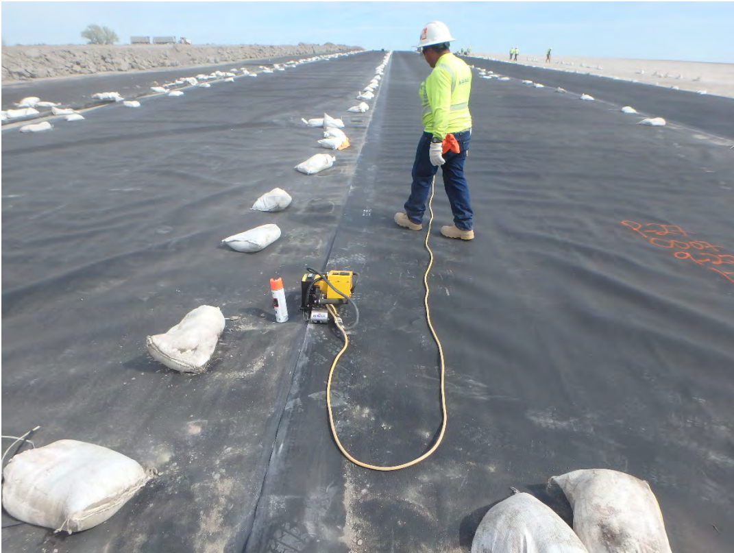
Seaming of geomembrane by fusion method, looking east.
