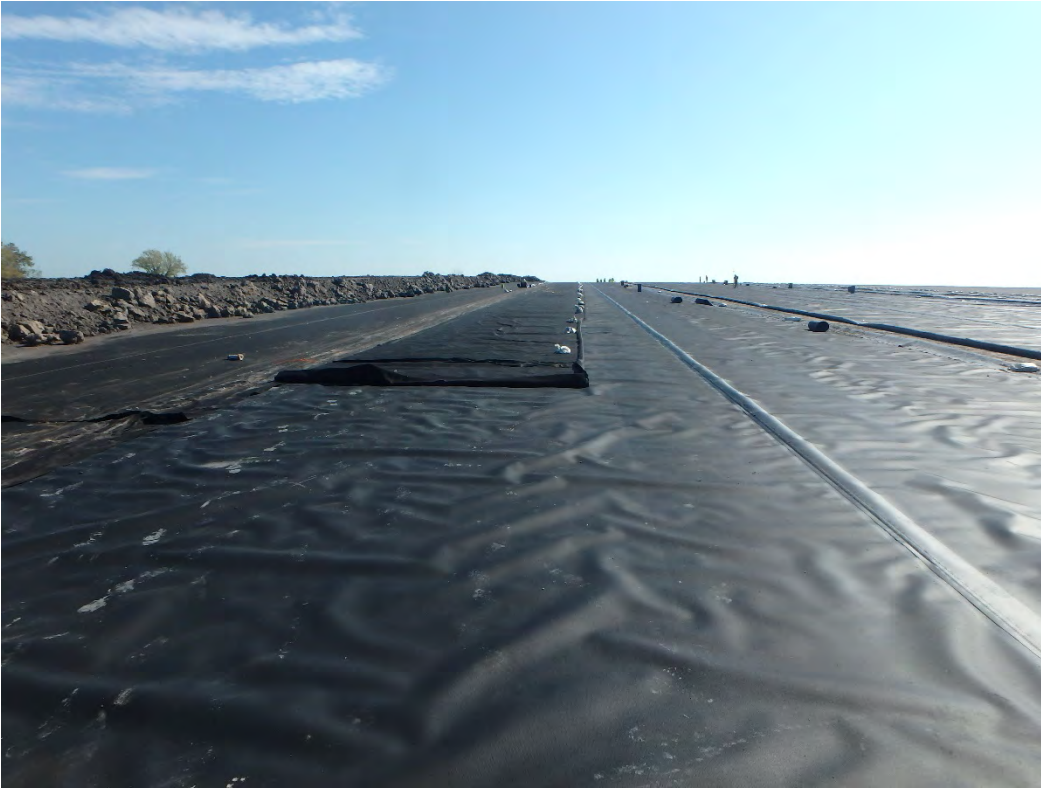
Deployment of geotextile in Pond 2, looking east.
