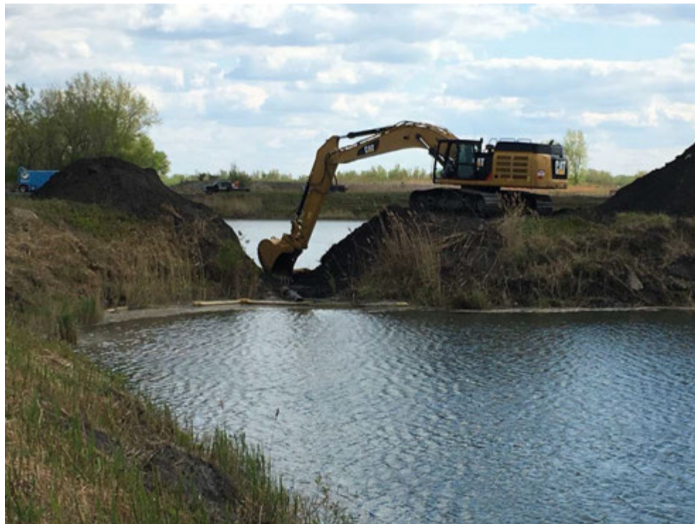
Ryan lowering culvert between Pond 1 and Pond 2.
