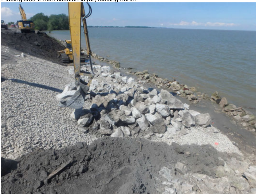
Placing D50-30 inch riprap, looking north.
