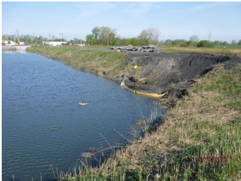
Pond 2 water level near the vertical pipe.
