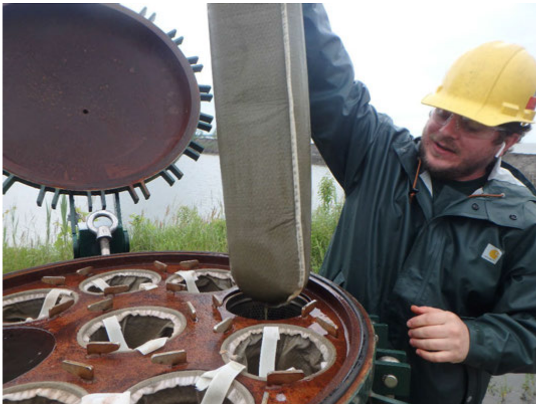
Changing cloth filters, looking northeast.
