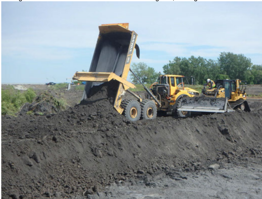
Placing bridging layer in Pond 1, looking southeast.
