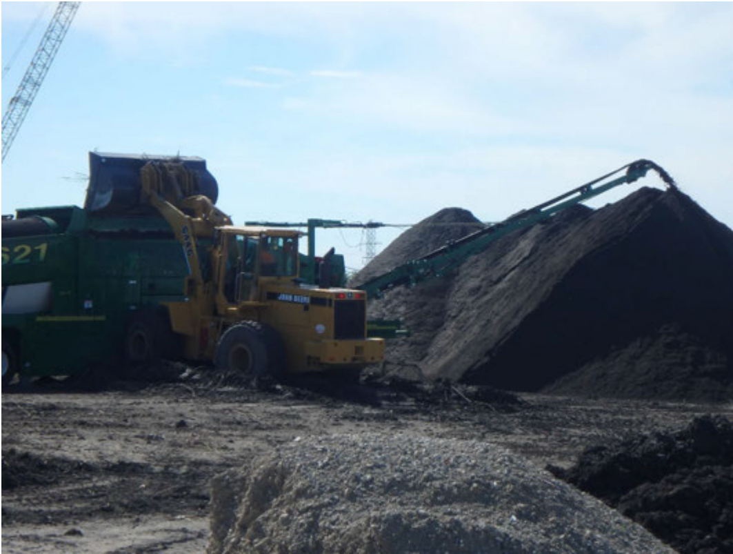
Screening of vegetation cleared from Pond 1, looking west.
