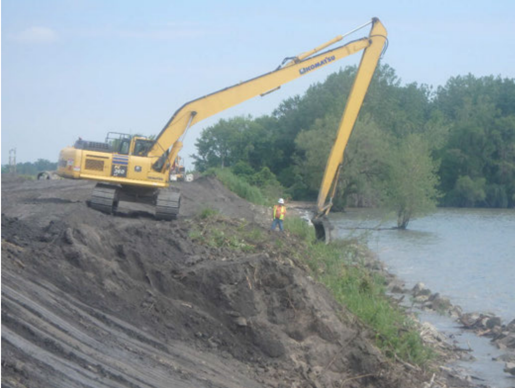
Removing vegetation along shoreline slope, looking north.
