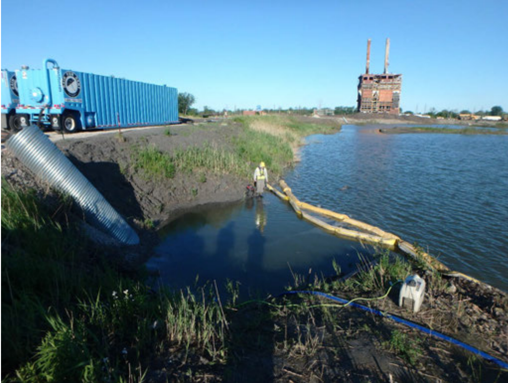
Dewatering Pond 2, Looking West
