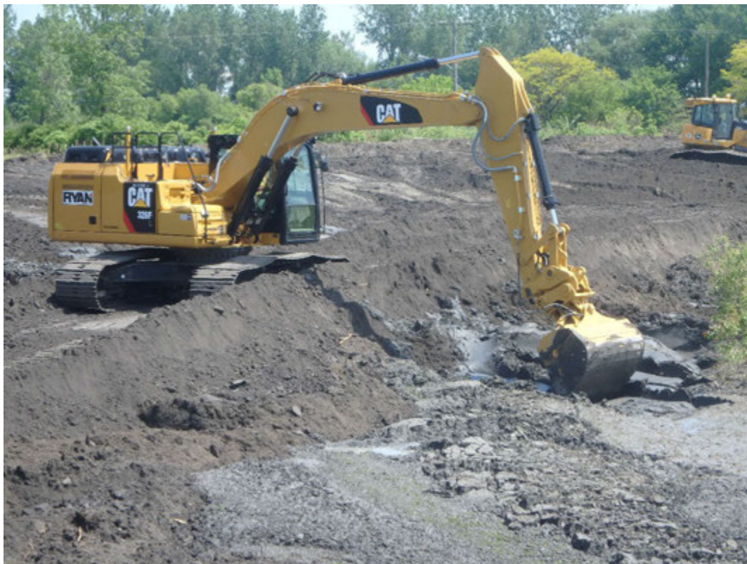
Removing saturated material from floor of Pond 1 prior to placement of bridging layer.
