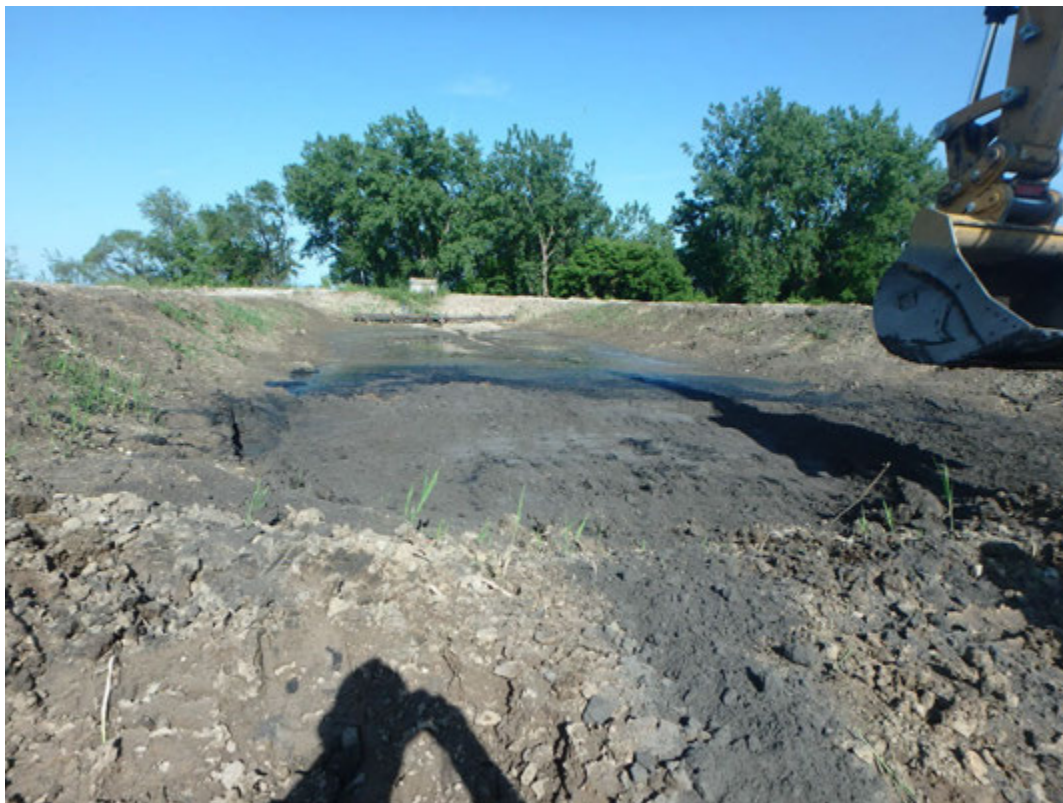
Adding material to Chemical Pond B residual to dry for transport to Pond 1, Looking South.
