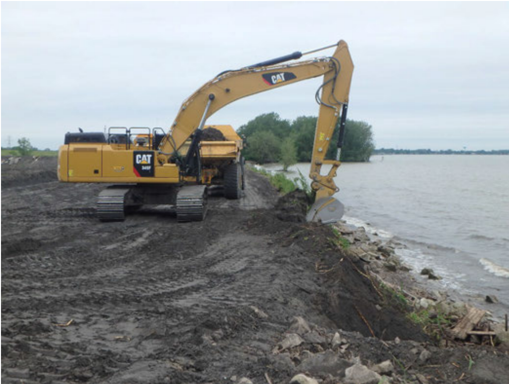
Removing vegetation from shoreline slope east of Pond 2, looking north.
