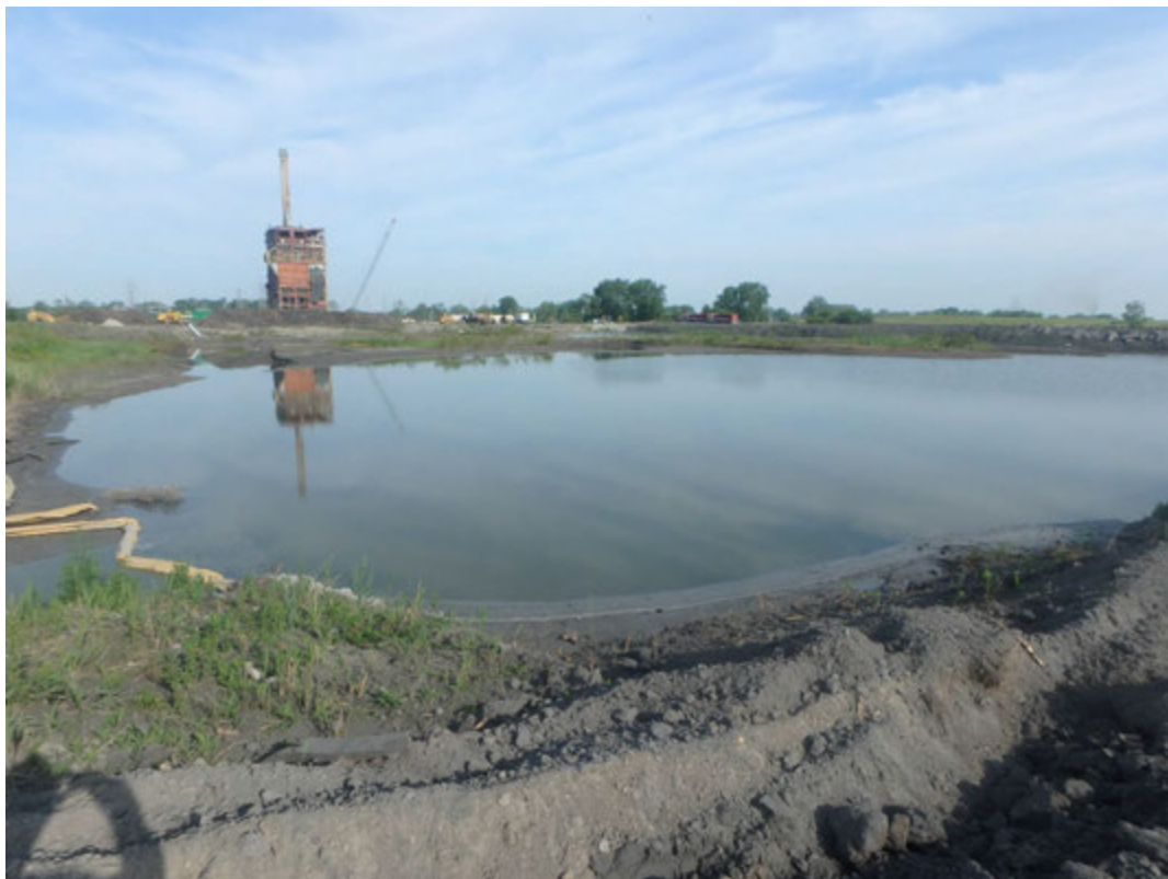
Overview of Pond 2, looking northeast.
