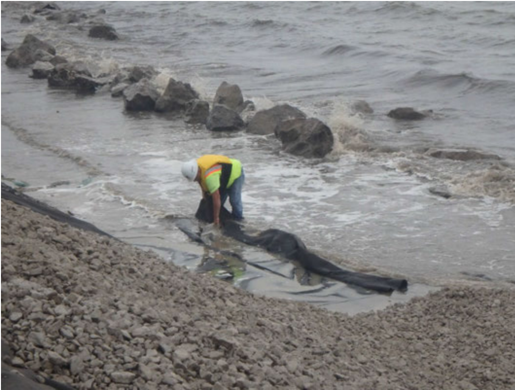
Installation of 16 oz. geotextile along shoreline slope, looking northeast.
