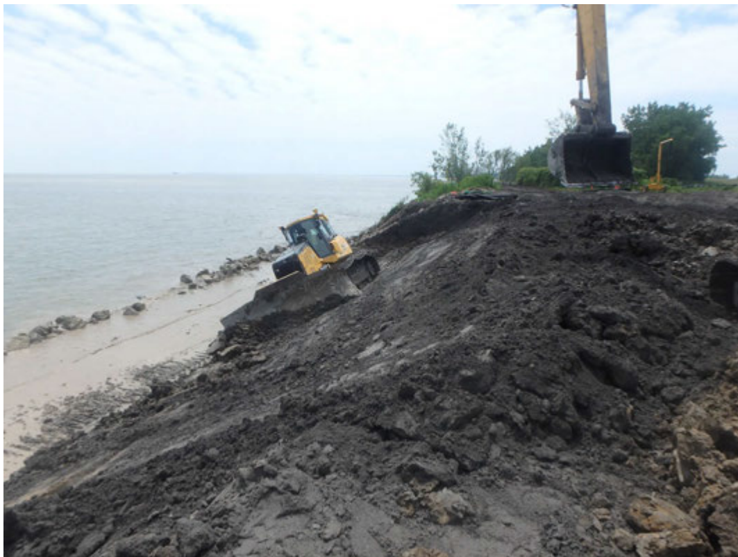
Grading shoreline slope, looking south.
