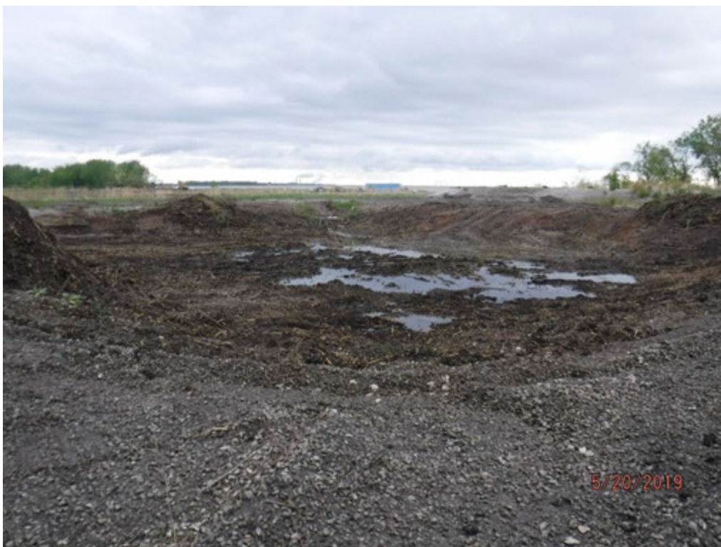
Chemical Pond A dewatering efforts and vegetation removal that took place on 05-18-19 looking northeast.
