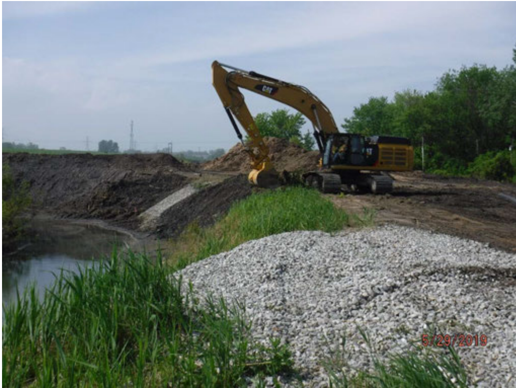
Vegetation removal on east dike of Pond 1, looking north.
