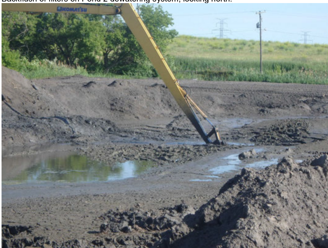
Over-Ex west side of Pond 1, looking north.
