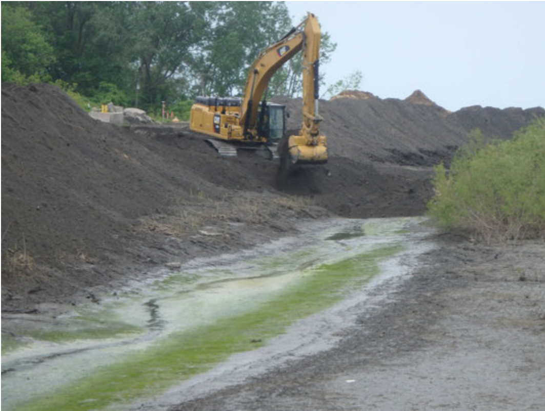
Bridging layer being placed in Pond 1
