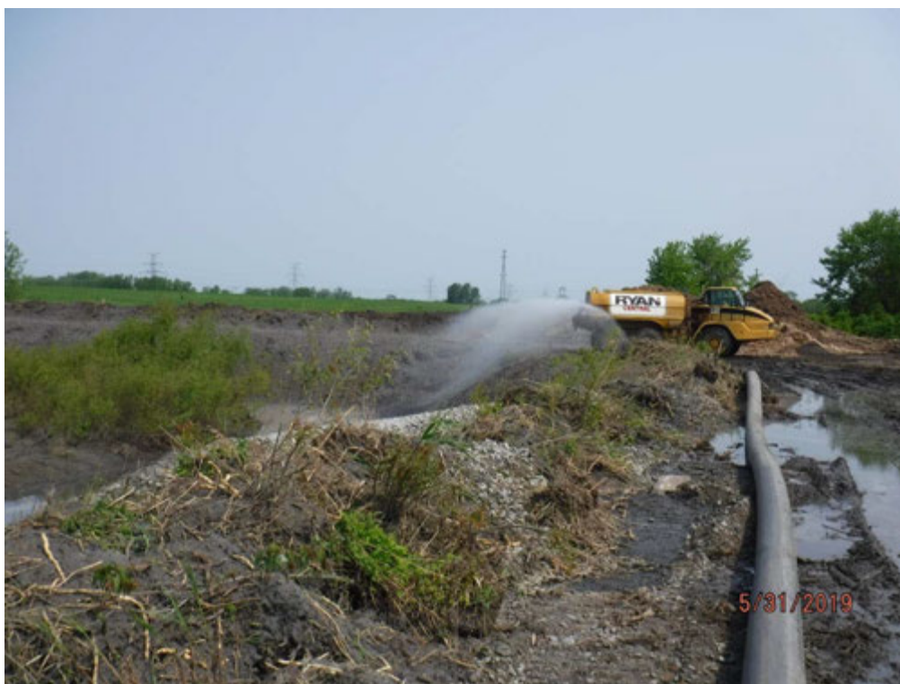
Dewatering of Chemical Pond B into Pond 1 via water truck, looking north.
