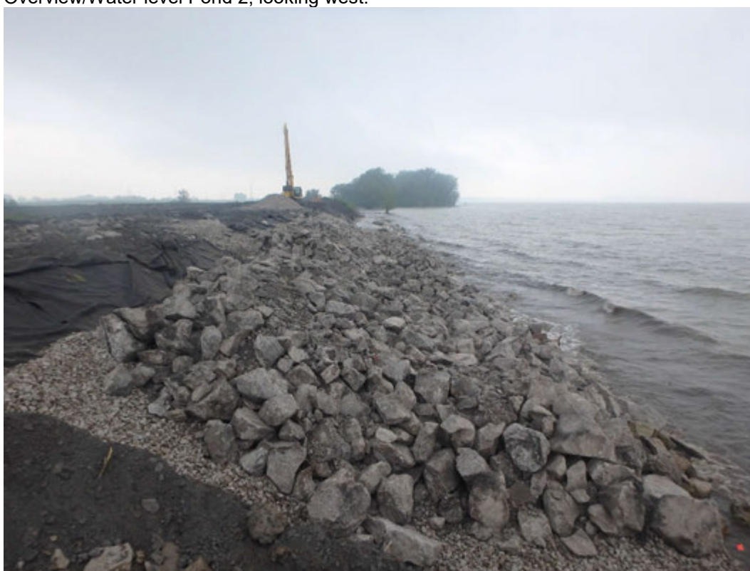
Southern end of shoreline, looking north.
