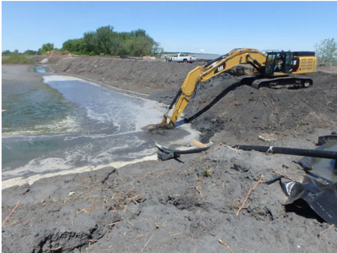
Excavating Sump in southeast corner of Pond 2
