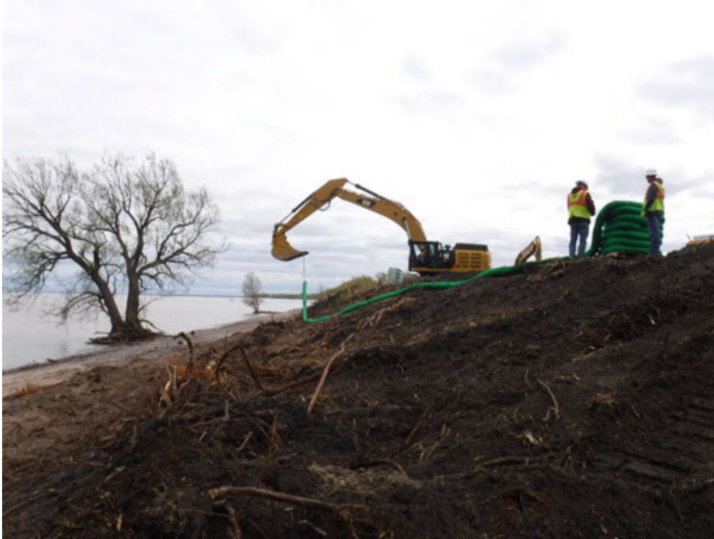
Ryan installing 8" straw wattle on the east dike.
