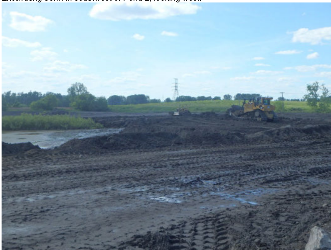
Placing bridging layer in Pond 1, looking northwest.
