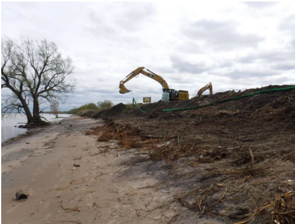
Ryan installing 8" straw wattle on the east dike.
