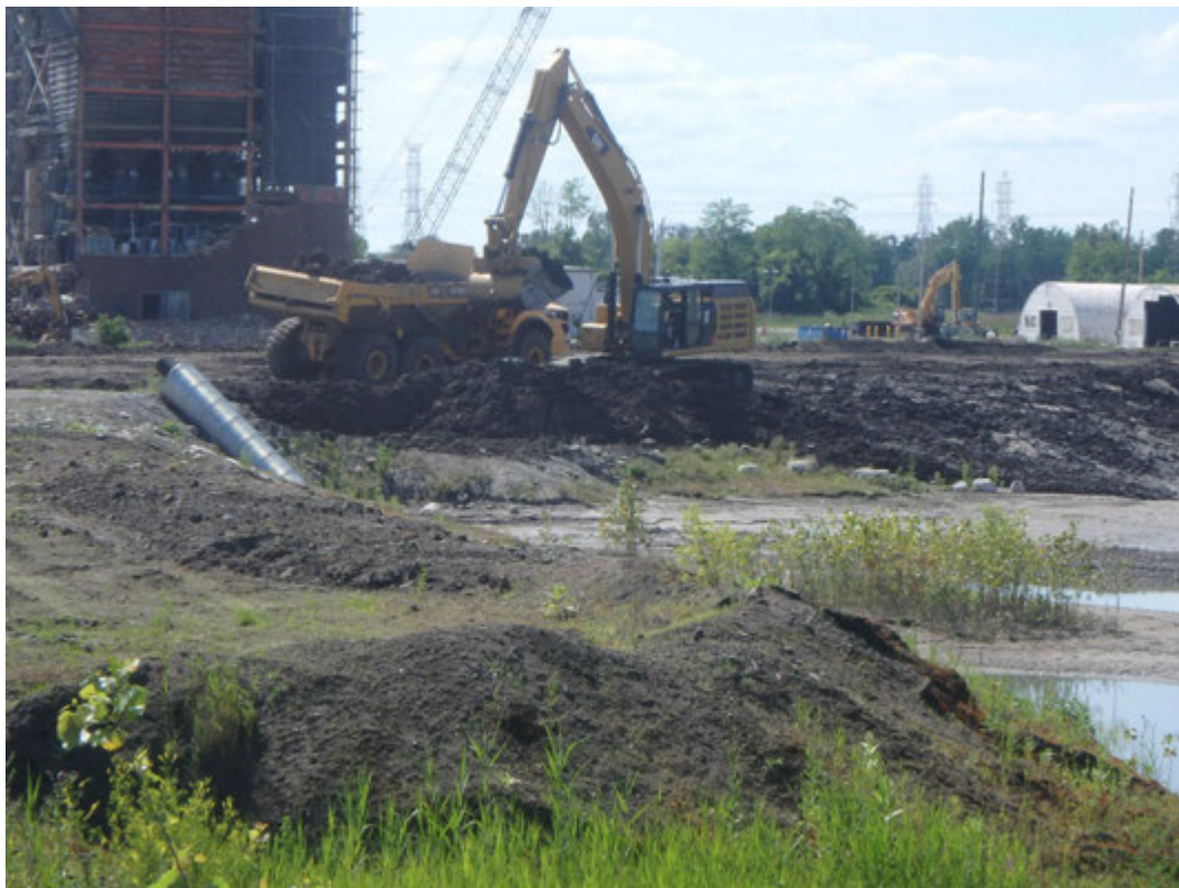
Excavating berm in southwest of Pond 2, looking west.
