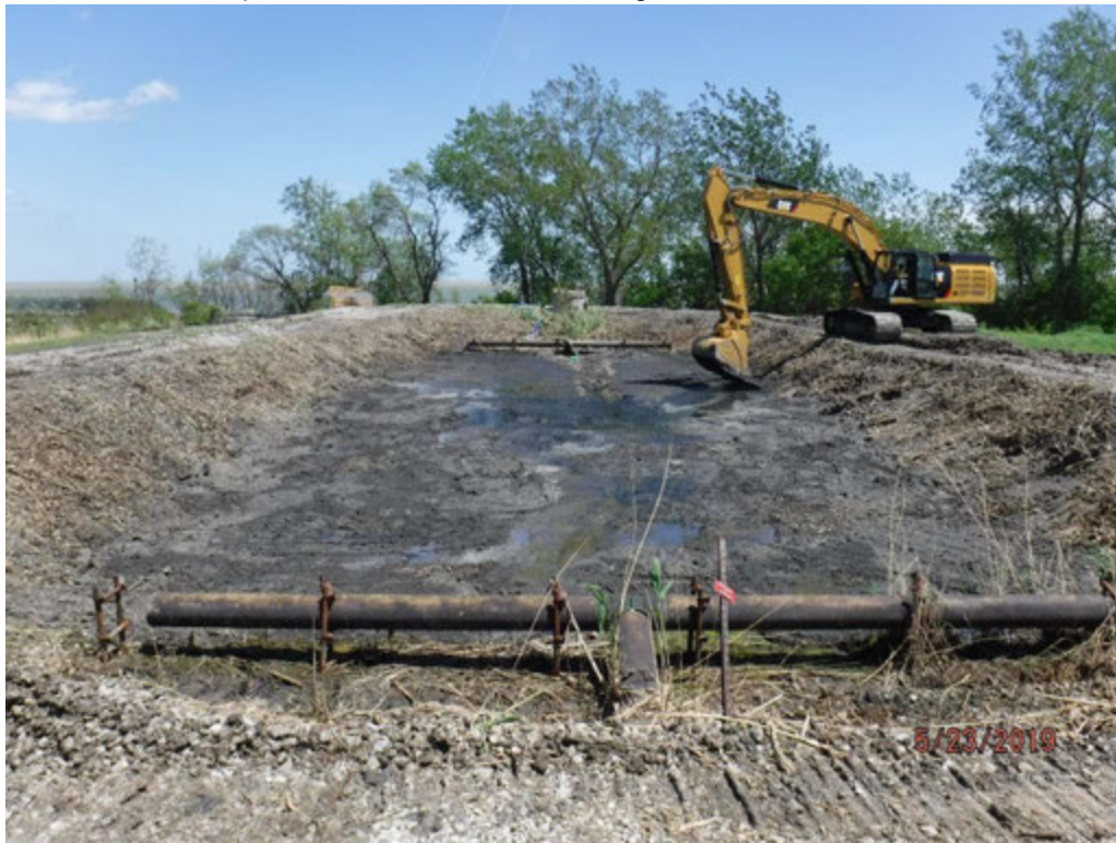
Chemical Pond B bottom ash placement on residuals, looking east.
