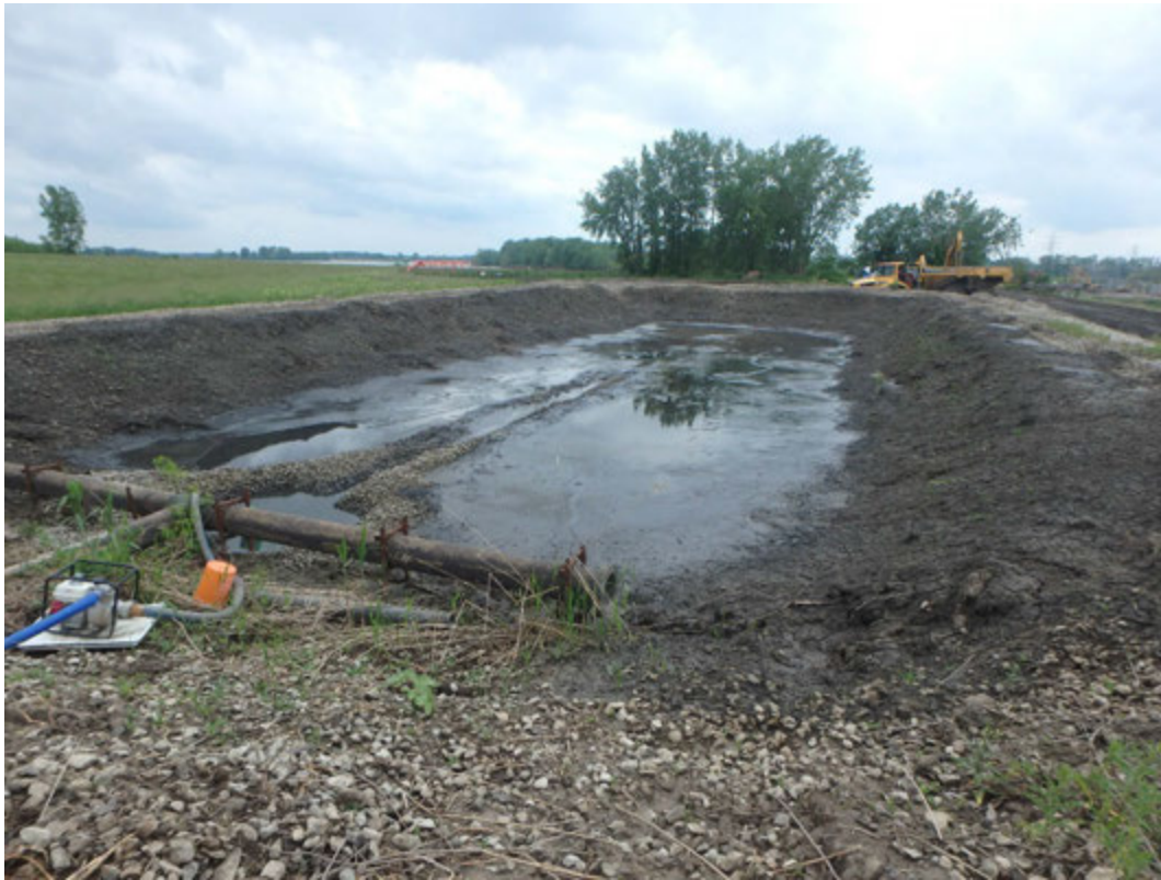
Water level in Chemical Pond B, Looking West
