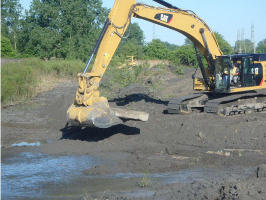
Placing concrete in Pond 1 prior to placement of bridging layer, Looking West.
