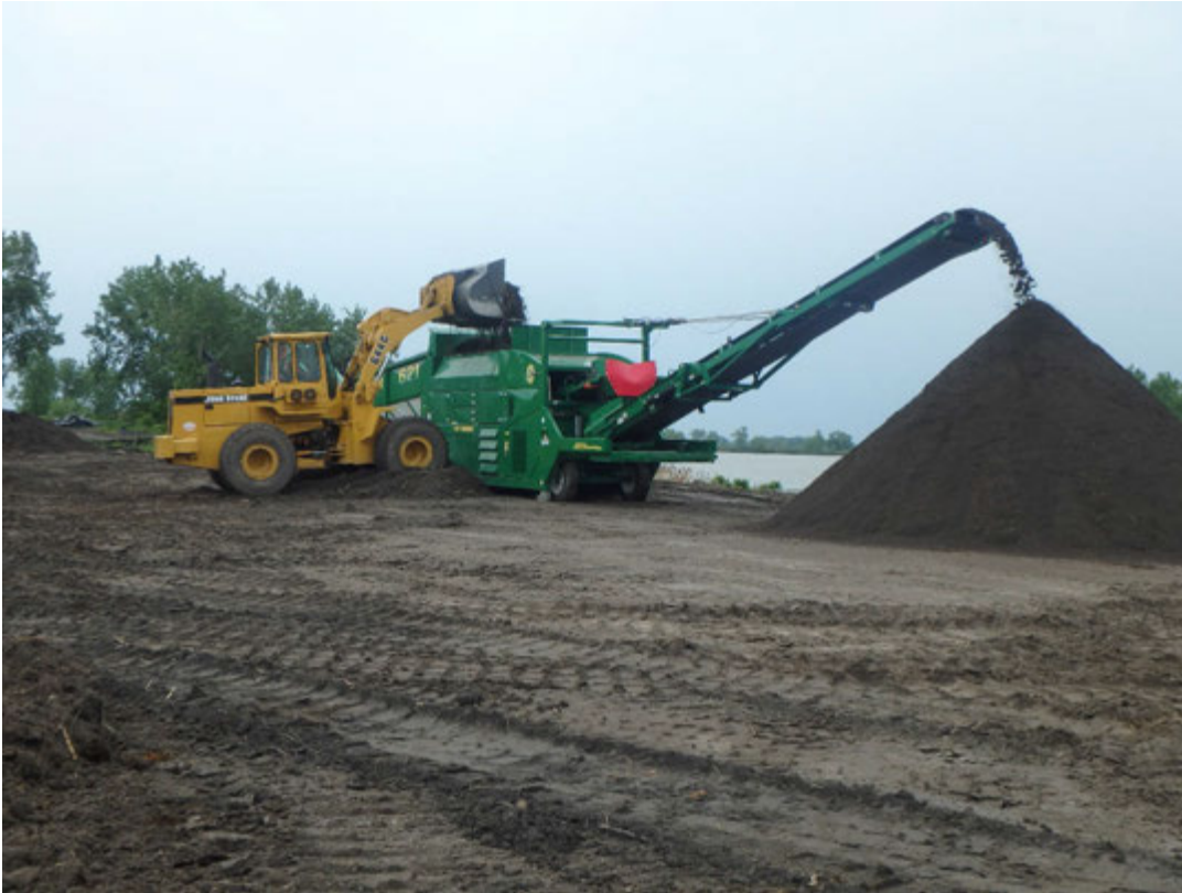
Screening cleared/grubbed material to remove organics
