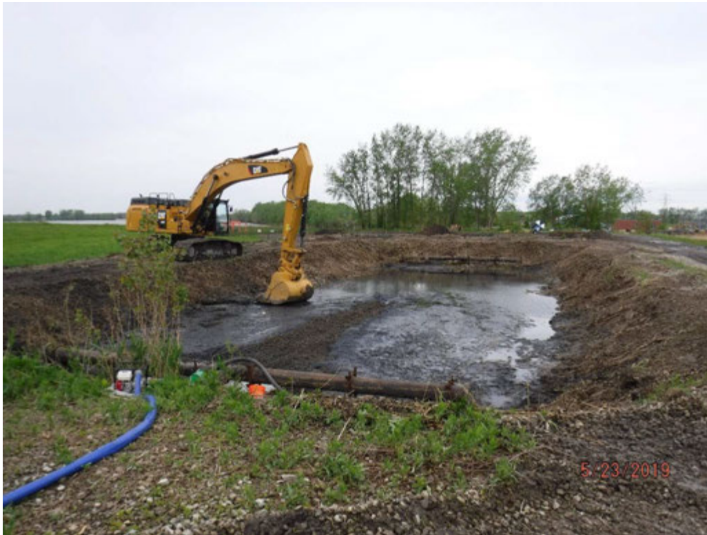
Chemical Pond B bottom ash placement on residuals, looking east.
