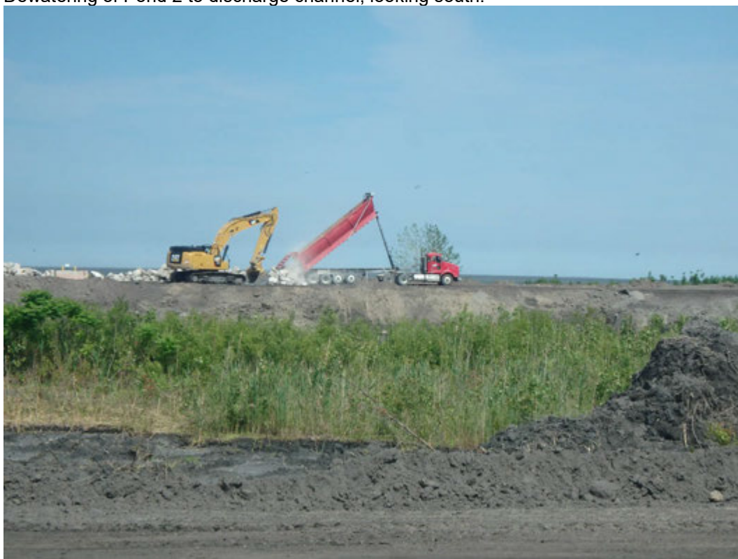
Delivery of D50-30 inch riprap, looking east.
