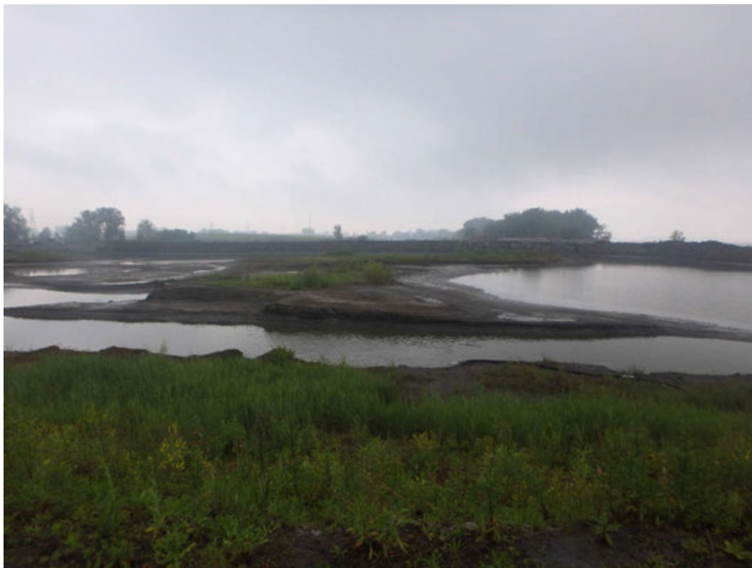
Overview/Water level Pond 2, looking west.
