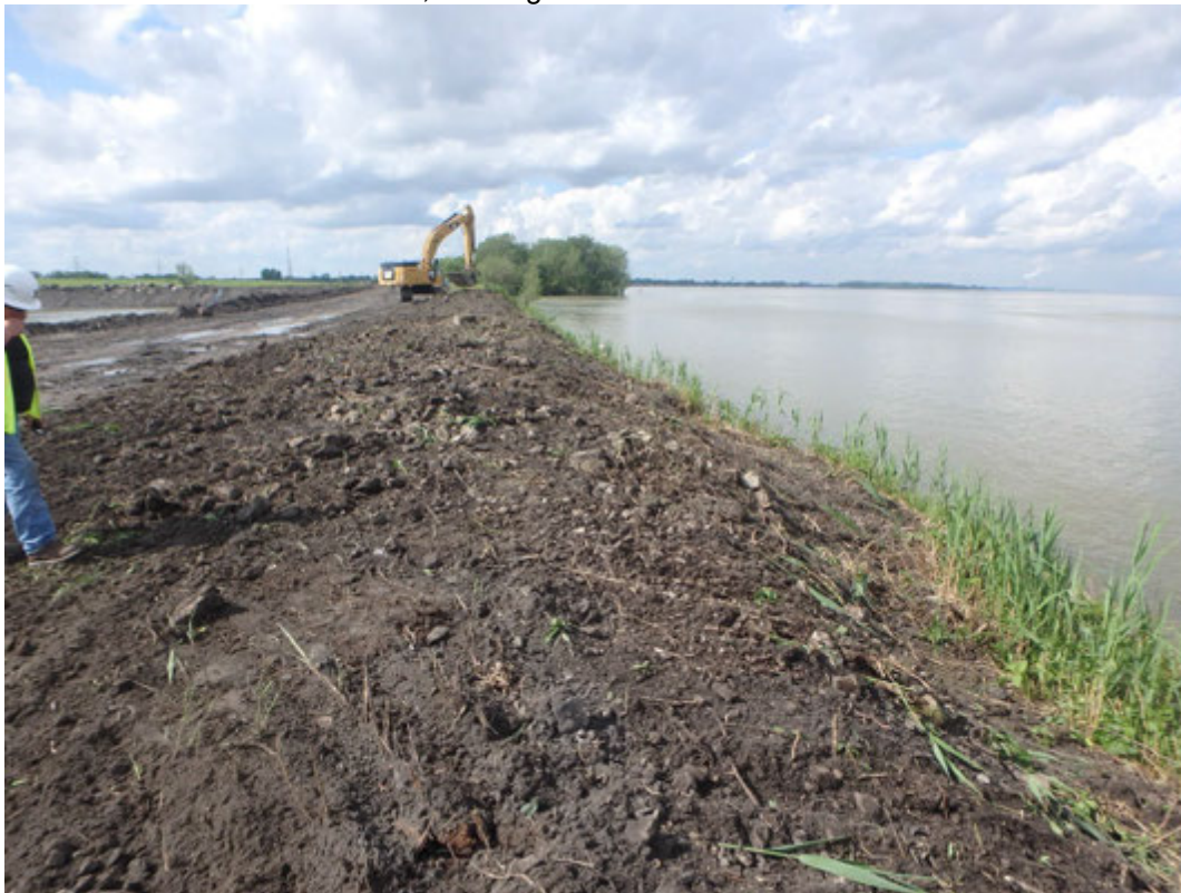
Clearing/Grubbing atop shoreline slope east of Pond 2
