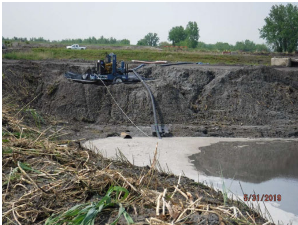
Dewatering Pond 1 into Pond 2 via 6-inch pump, looking south.
