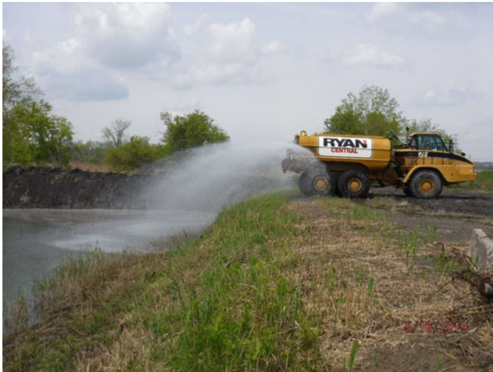
Discharging water from Chemical Pond B via the water truck into northwest corner of Pond 1.
