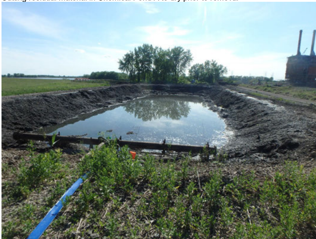
Water level Chemical Pond B, Looking West
