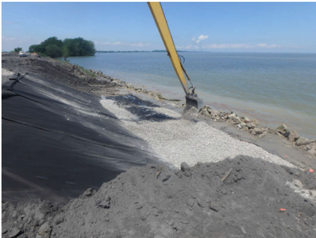
Placing D50-2 inch cushion layer, looking north.
