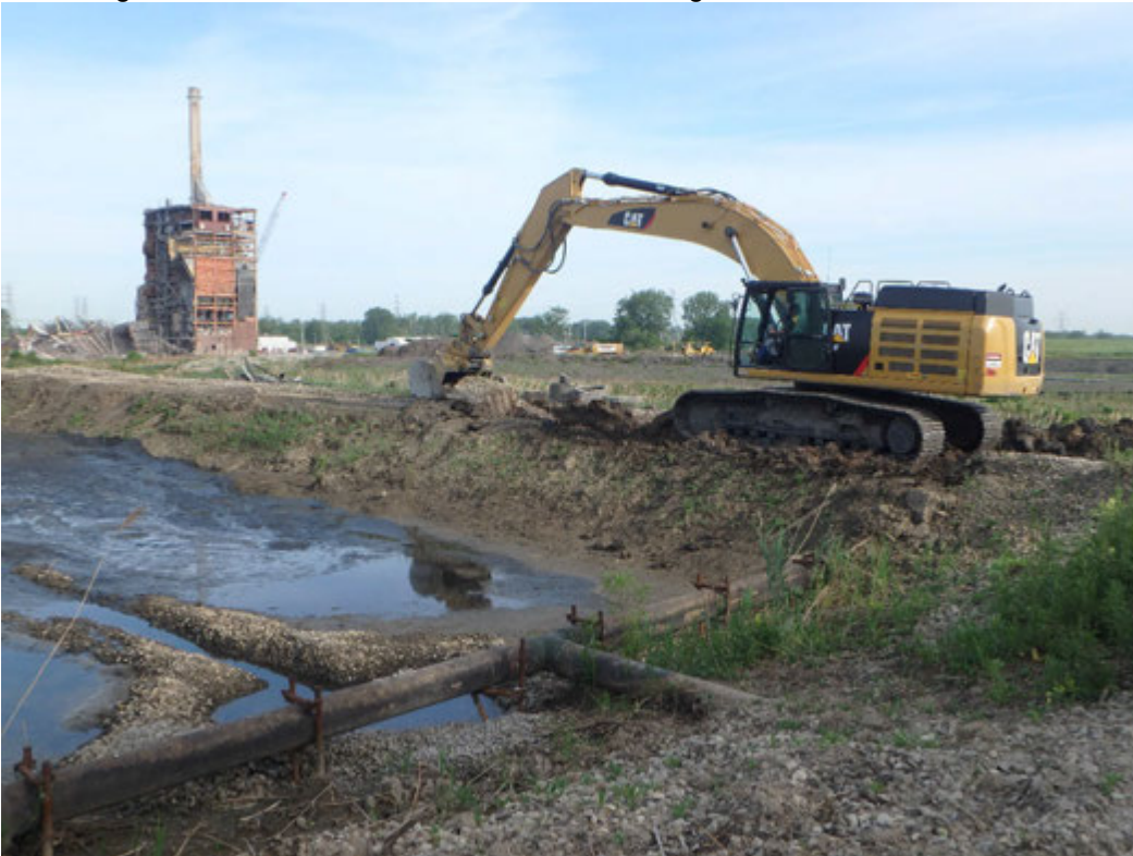
Cutting down north berm of Chemical Pond B, Looking northwest.
