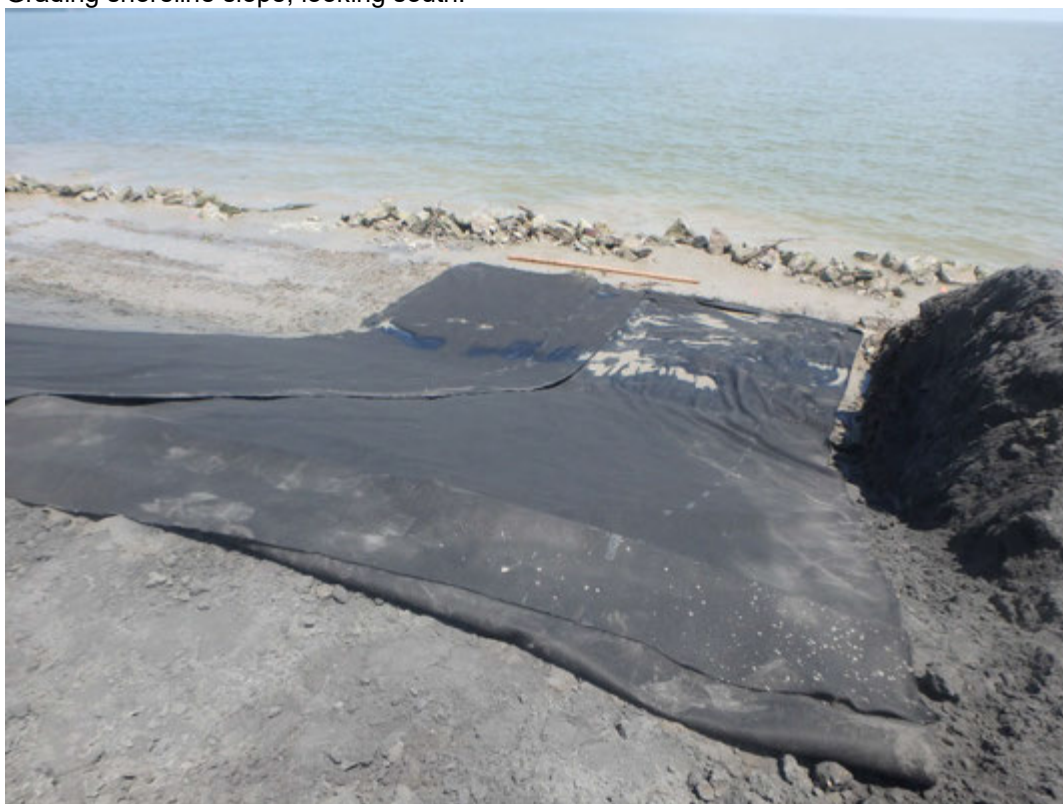
16 oz. geotextile installed along shoreline slope, looking east.
