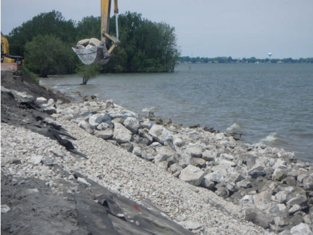
Placing D50-30 inch riprap atop cushion layer along shoreline slope.
