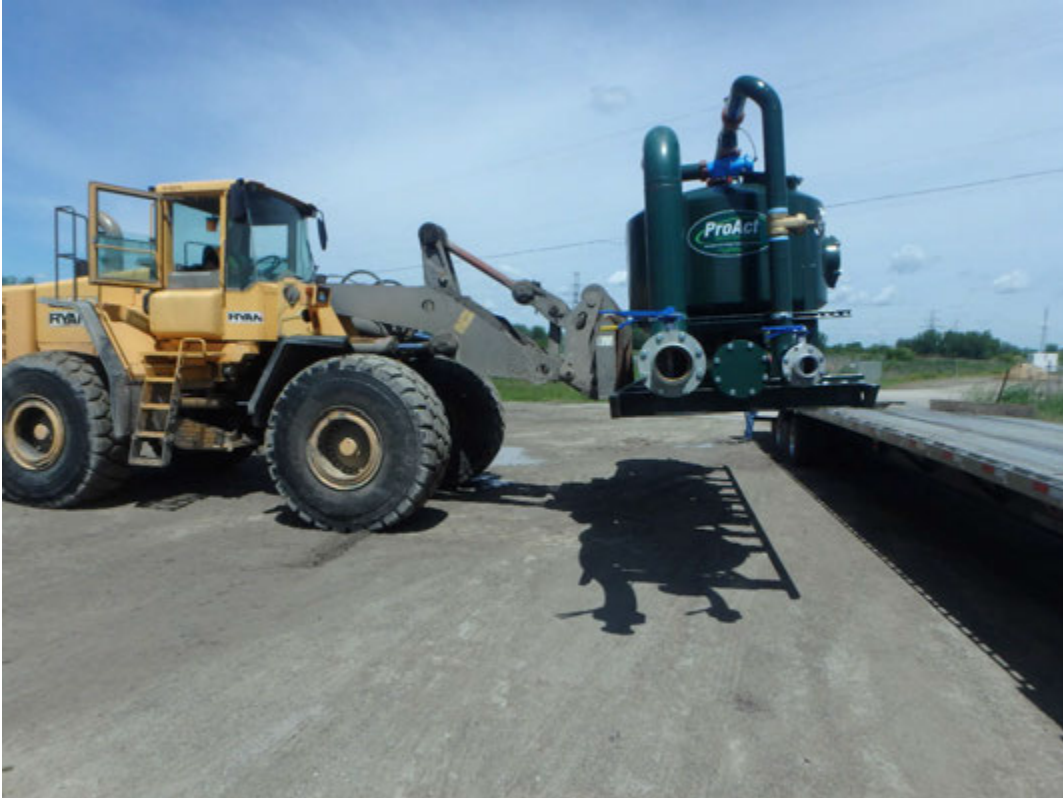
Off-loading sand pots from flat bed, looking north.
