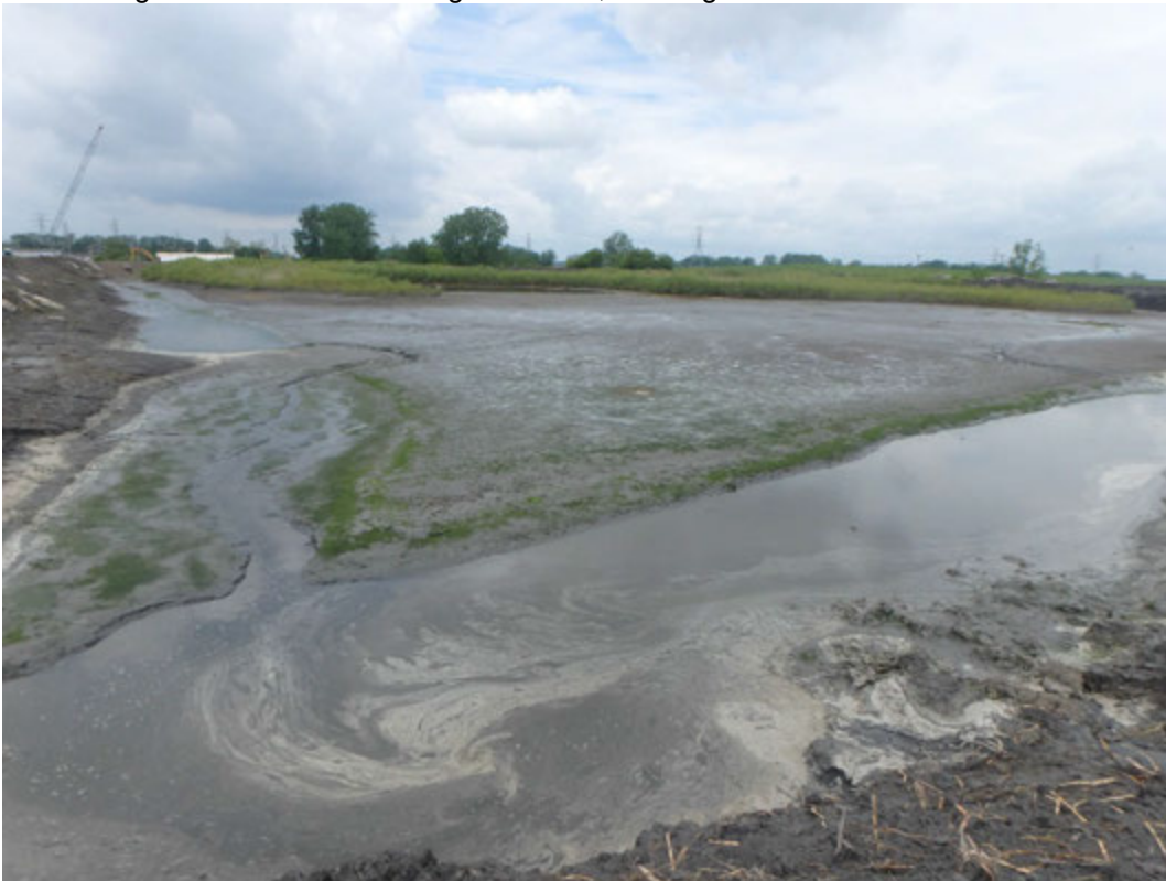
Water level Pond 1, Looking Northwest
