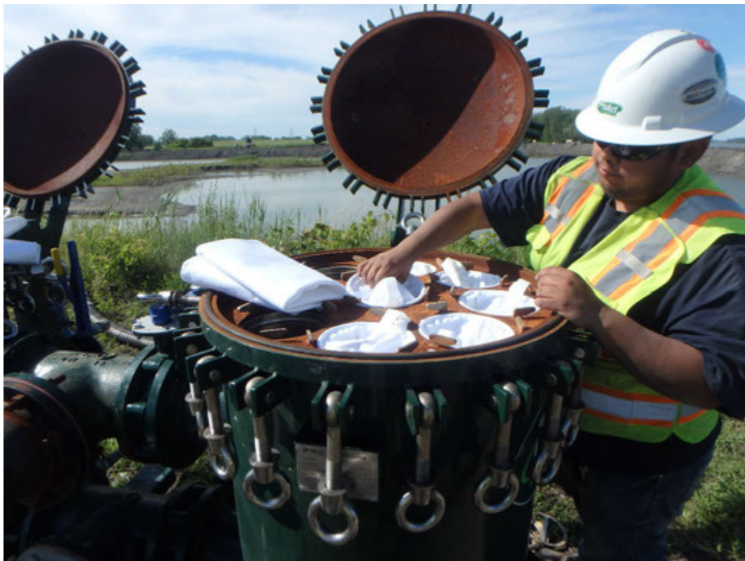
Installing filters on filtration system at Pond 2.
