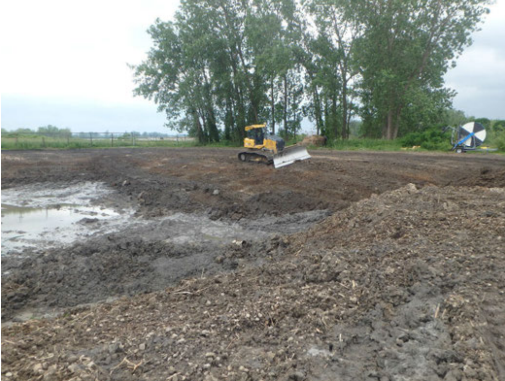
Removing remaining residual in Chemical Pond A, Looking Southwest.
