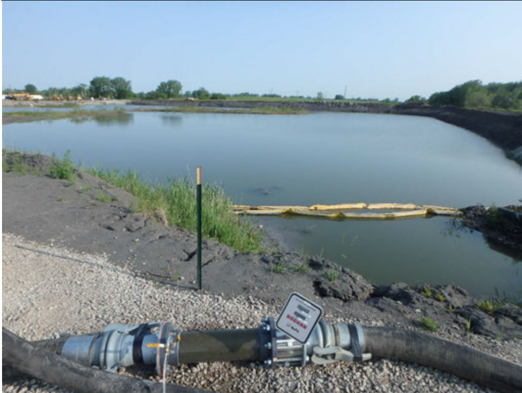
Water Level in Pond 2, Looking North
