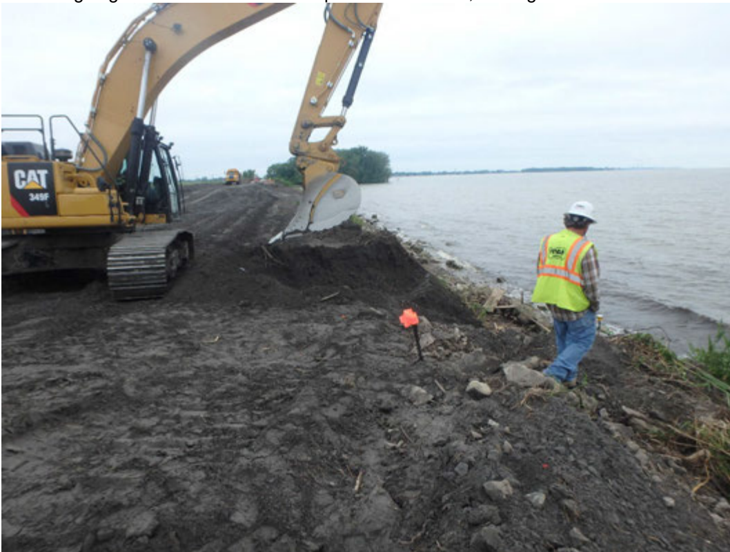
Cutting slope down to riprap sub-grade, looking northeast.
