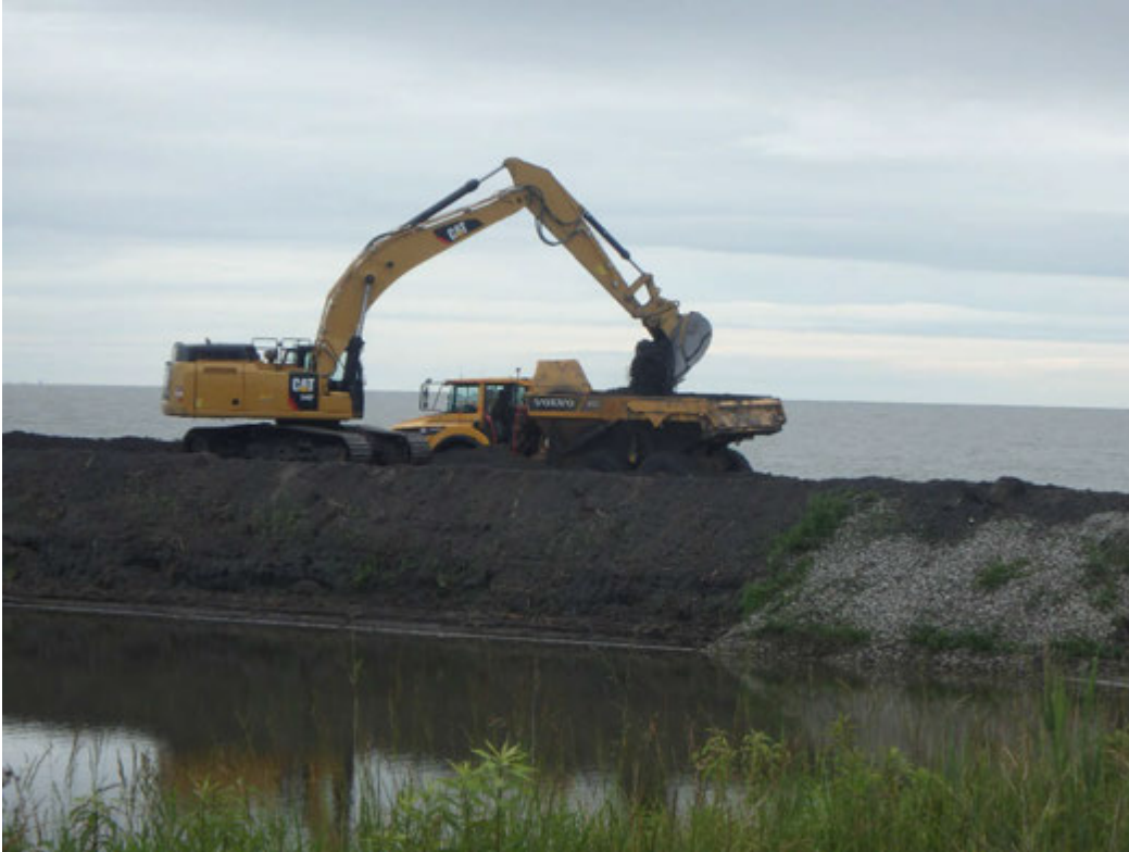
Cutting access road east of Pond 2 down to sub-grade, looking east.
