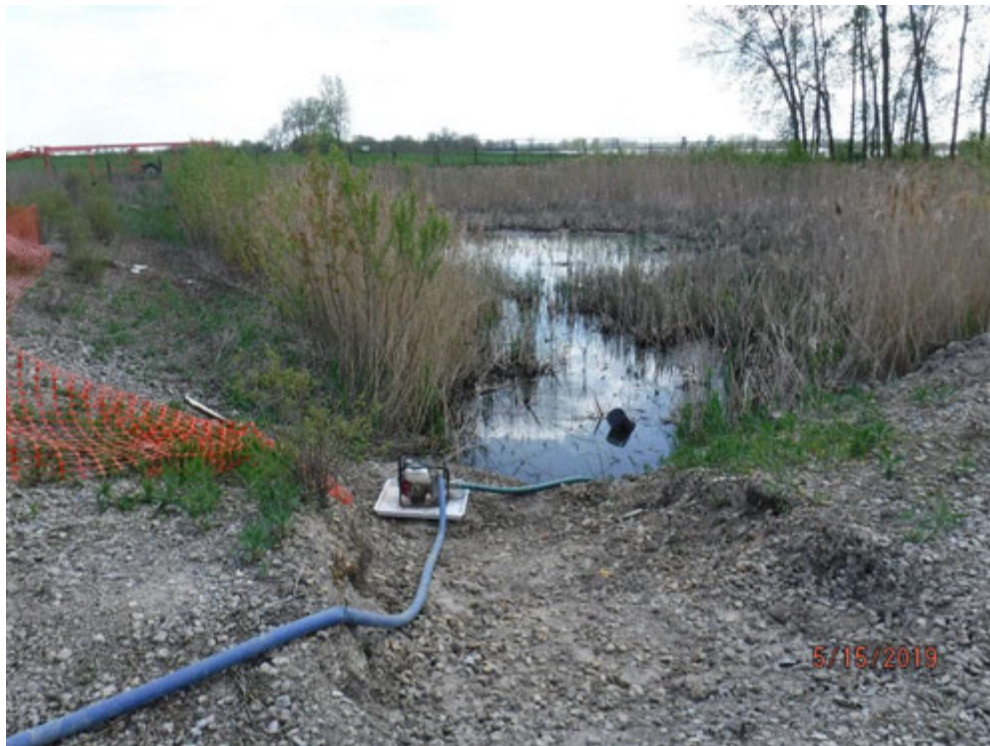
Dewatering of Chemical Pond B into water truck for discharge into northwest corner of Pond 1.
