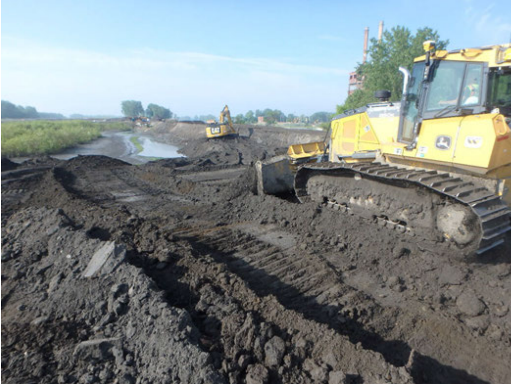
Placing bridging layer in northwest corner of Pond 1, Looking South
