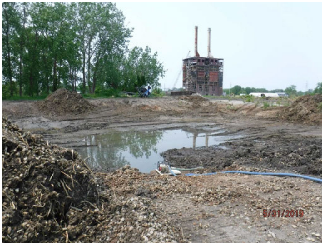
Dewatering Pond 1 into Pond 2 via 6-inch pump, looking south.
