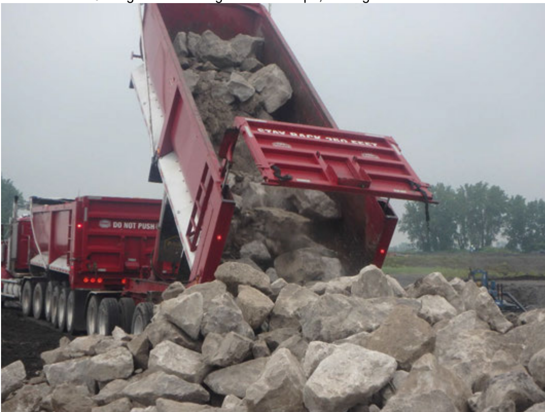
Delivery of D50-30 inch riprap, looking south.
