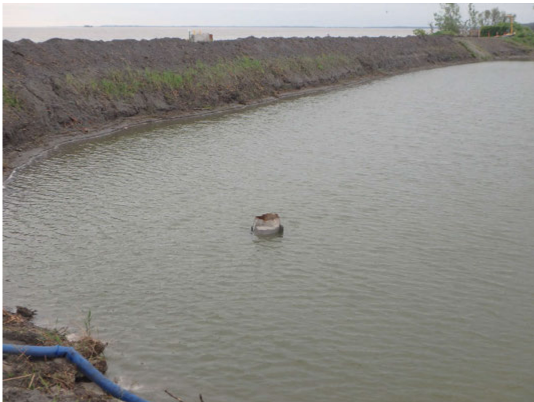
Water level of Pond 2, Looking Southeast.
