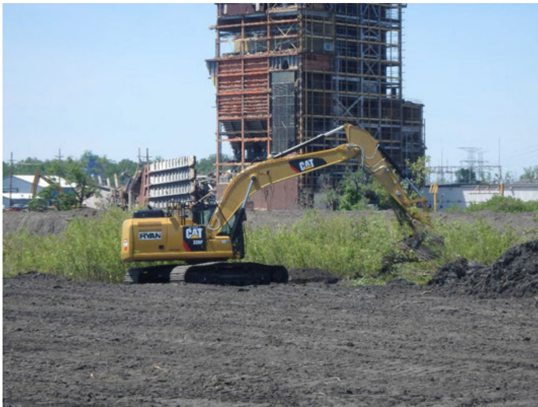
Clearing vegetation from Pond 1, Looking West.
