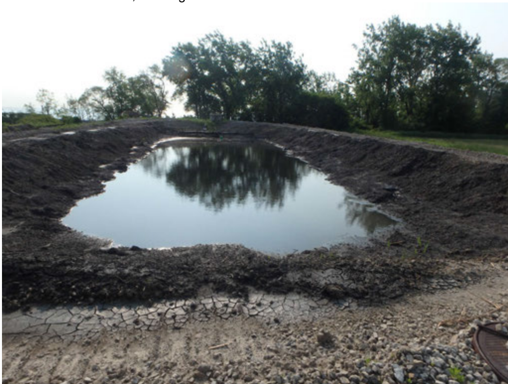
Water level Chemical Pond B, Looking West
