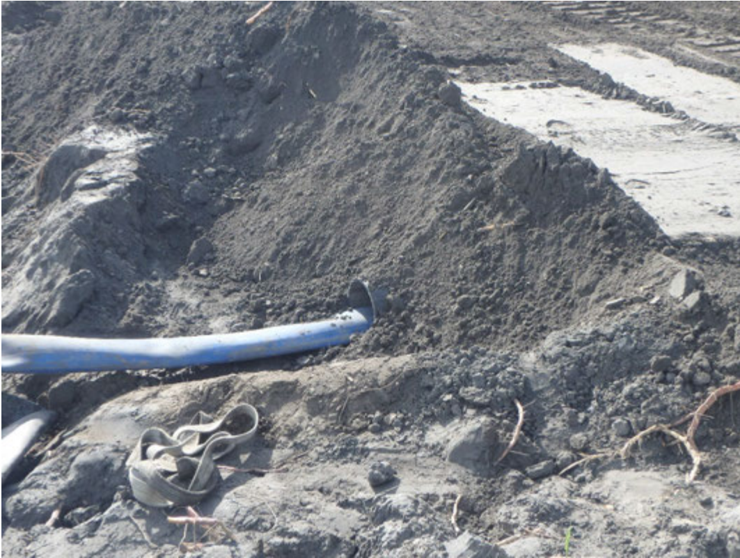
Temporary culvert installed for 6" pump discharge hose under access road between Ponds 1&2.
