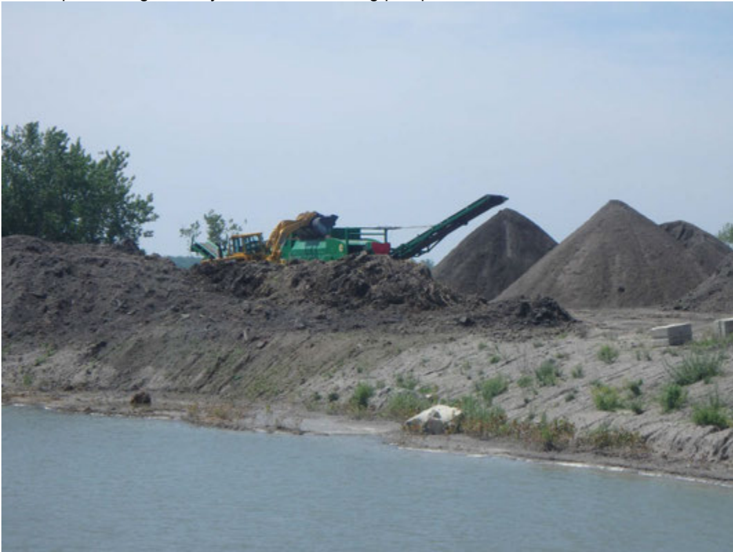
Screening of vegetation removed from Pond 1
