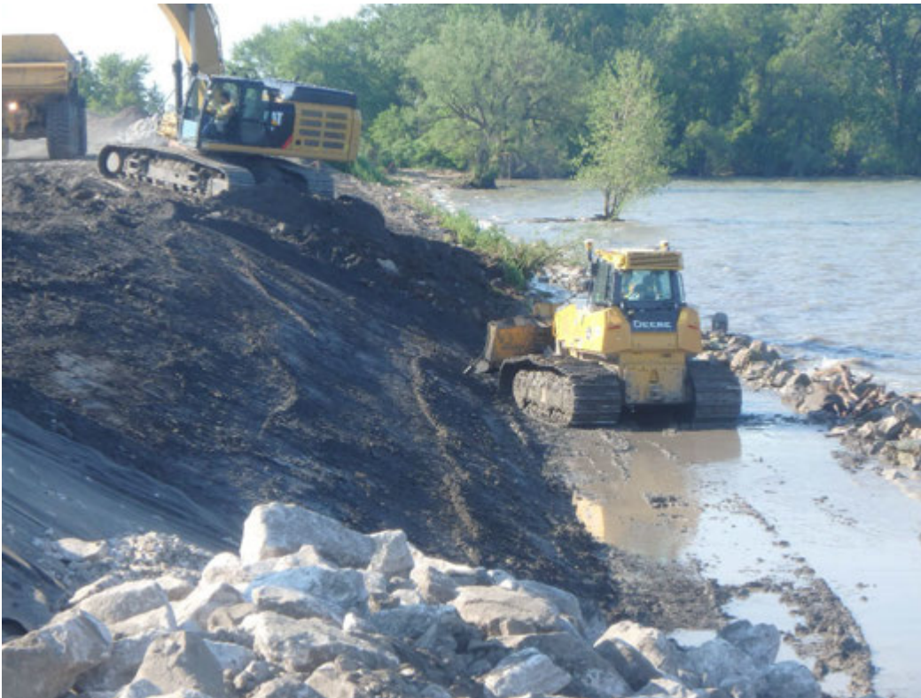
Grading shoreline slope to sub-grade for installation of geotextile, looking north.
