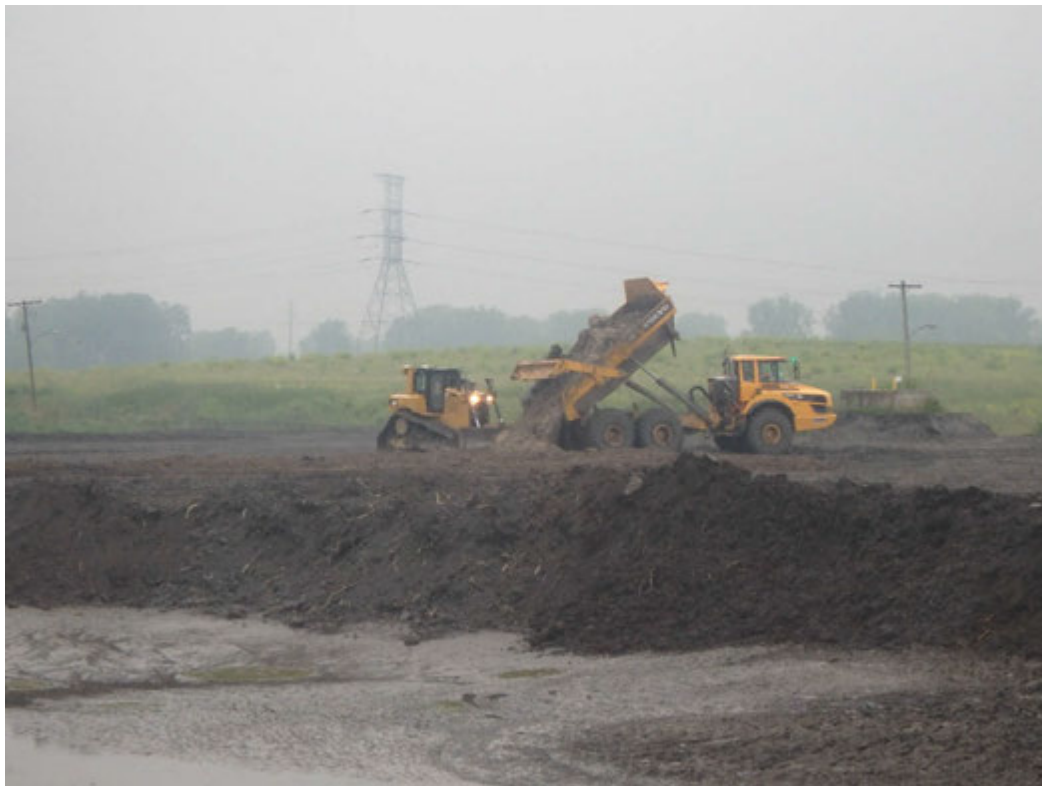
Placing bridging layer in Pond 1, looking northwest.
