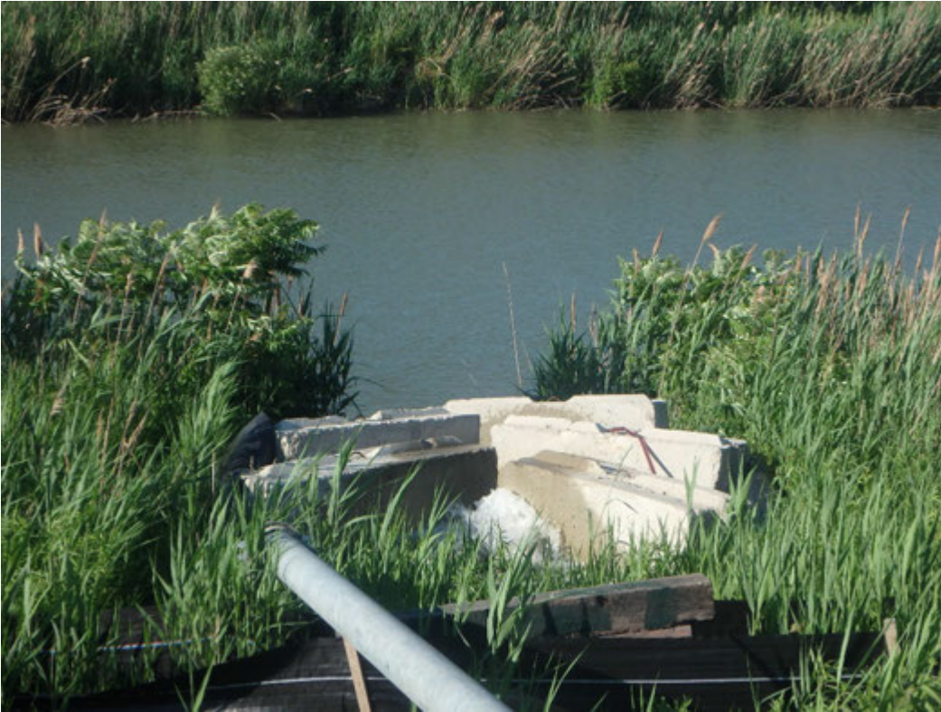
Outfall of water pumped from Pond 2 into discharge channel, looking south.
