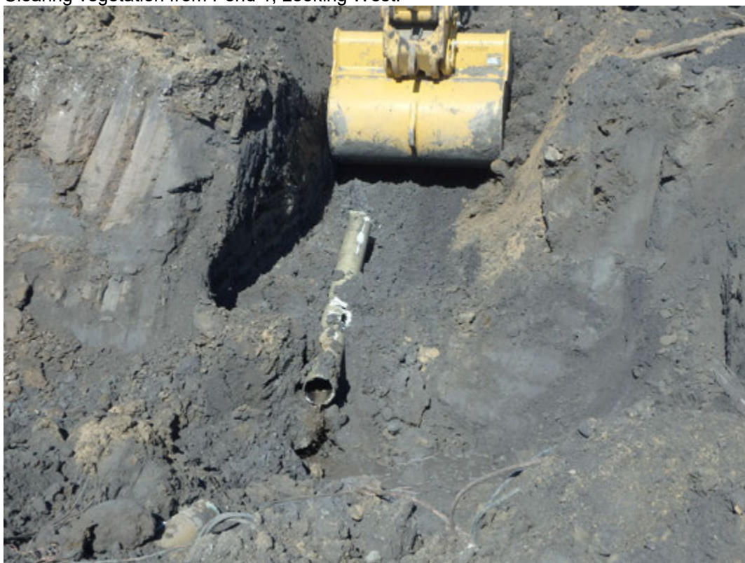
Removing drain pipe from manhole at Chemical Pond A.
