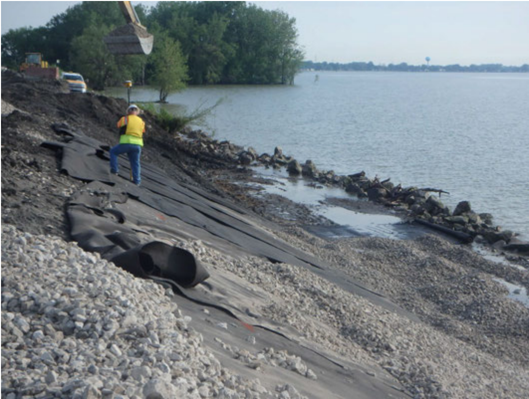
Checking grade atop geotextile, looking north.
