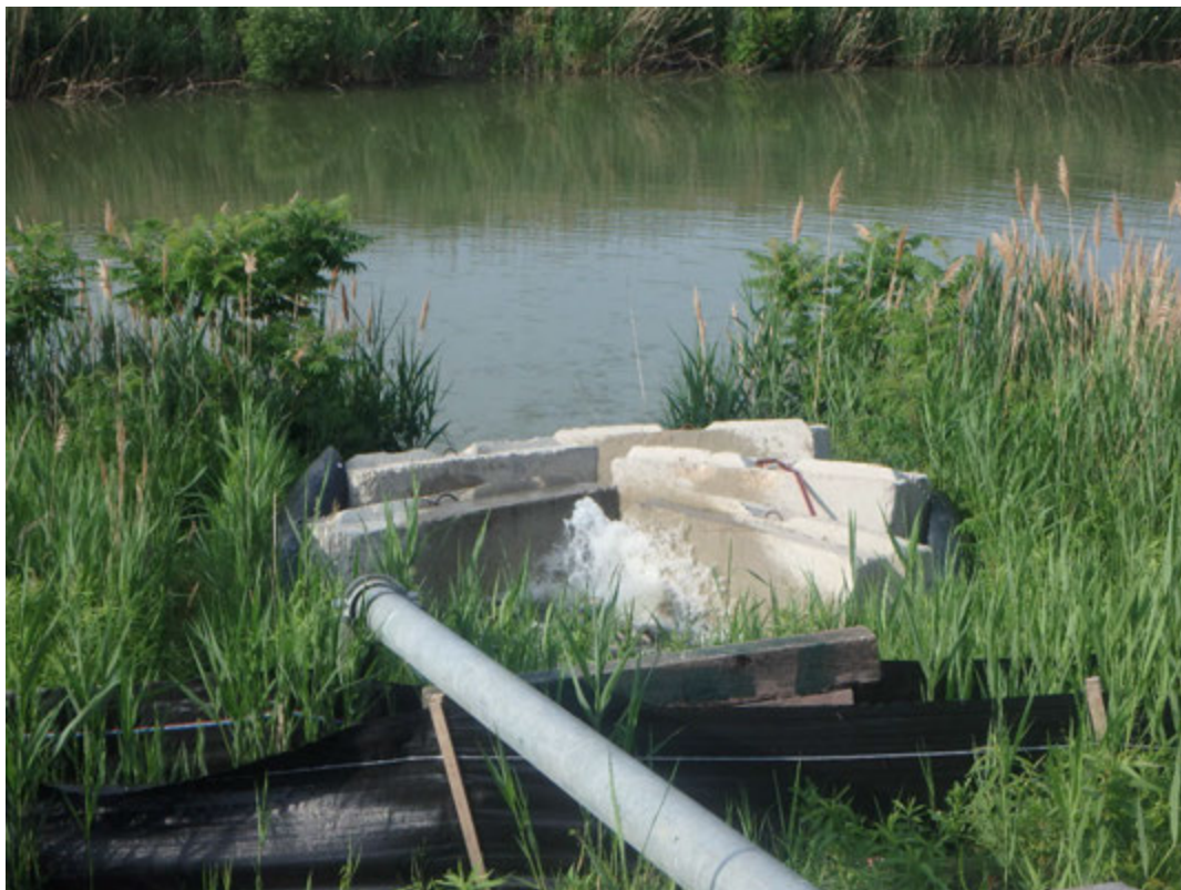
Dewatering of Pond 2 to discharge channel, looking south.
