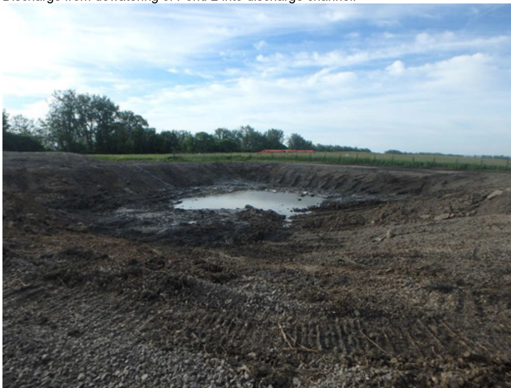
Chemical Pond A, Looking Southeast.
