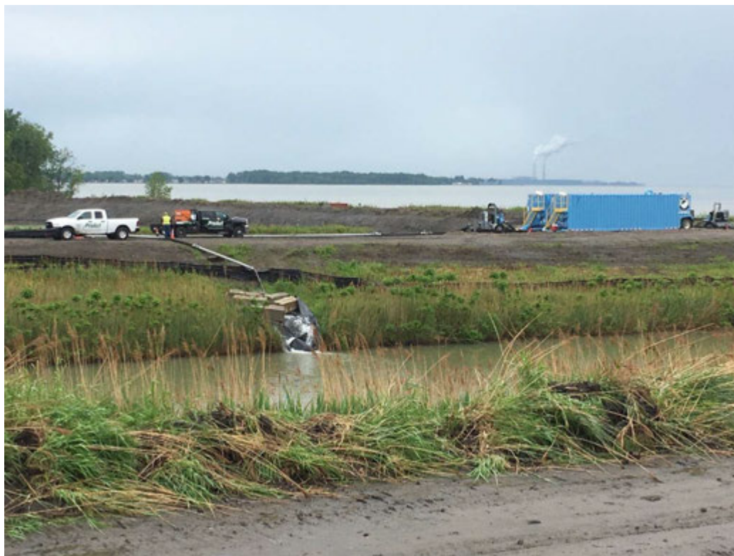
ProAct continued dewatering efforts, looking northeast across discharge channel.
