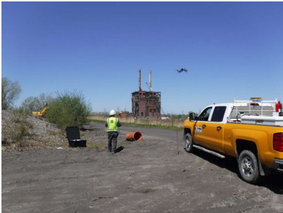
Rowe launching drone to perform existing conditions survey.
