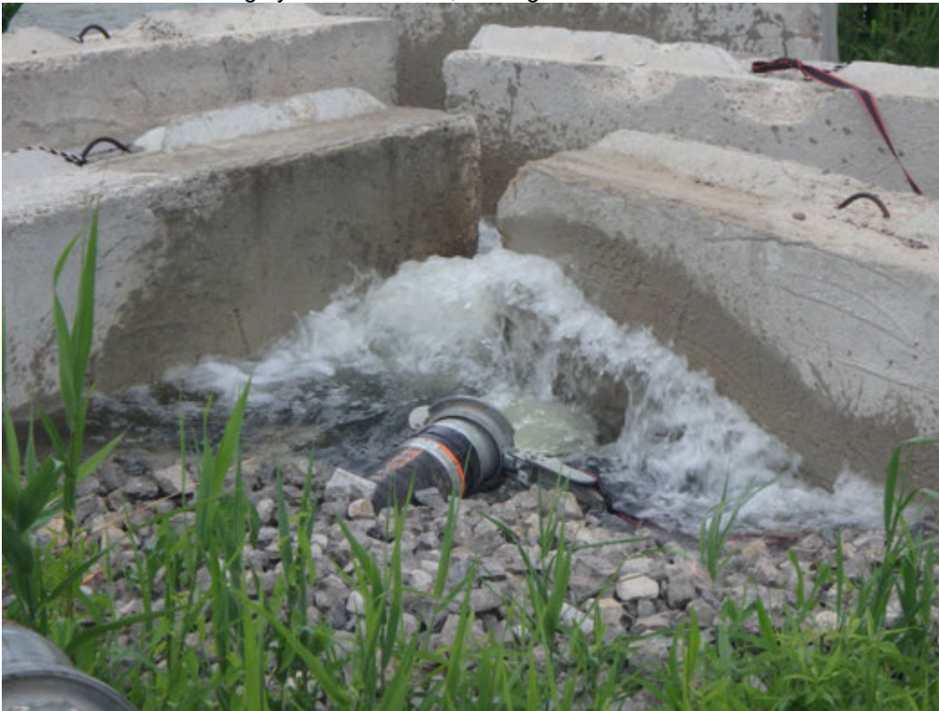
Discharge from pumping of Pond 2, looking south.
