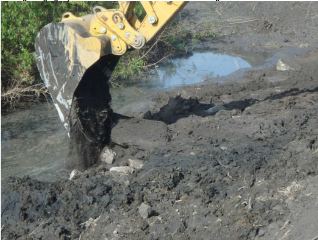
Placing concrete debris in Pond 1 prior to bridging layer
