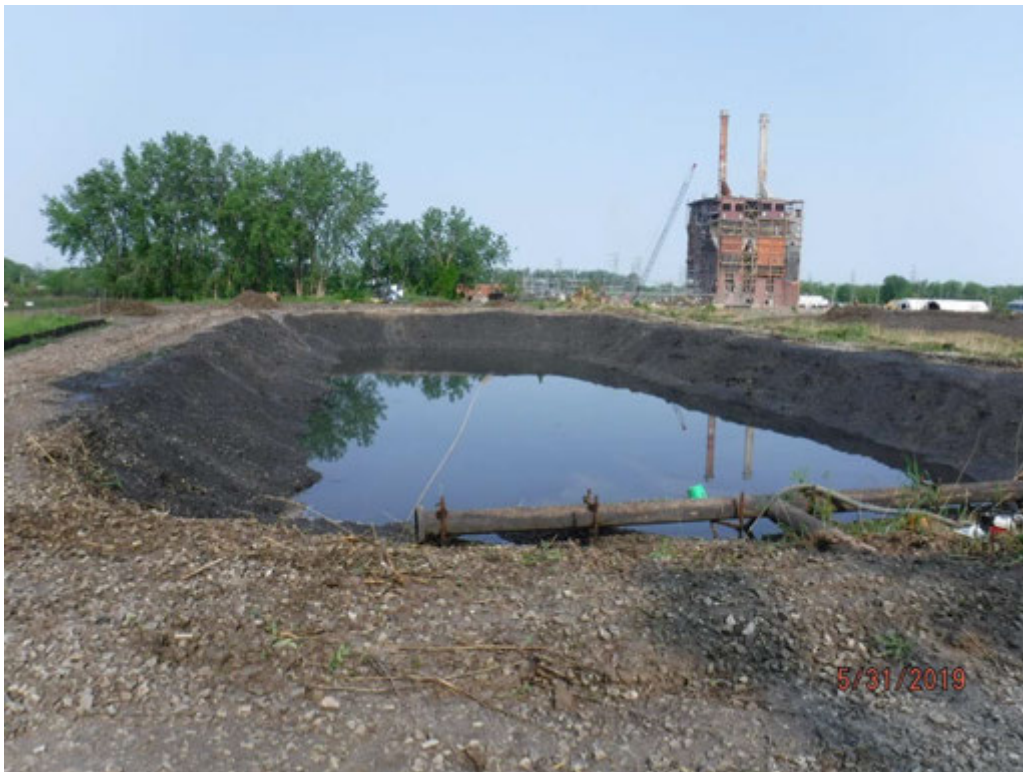
Dewatering of Chemical Pond B into Pond 1 via water truck, looking north.
