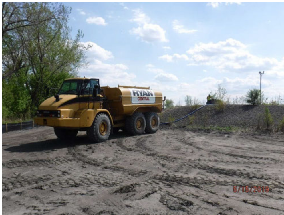
Dewatering of Chemical Pond B into water truck for discharge into northwest corner of Pond 1.
