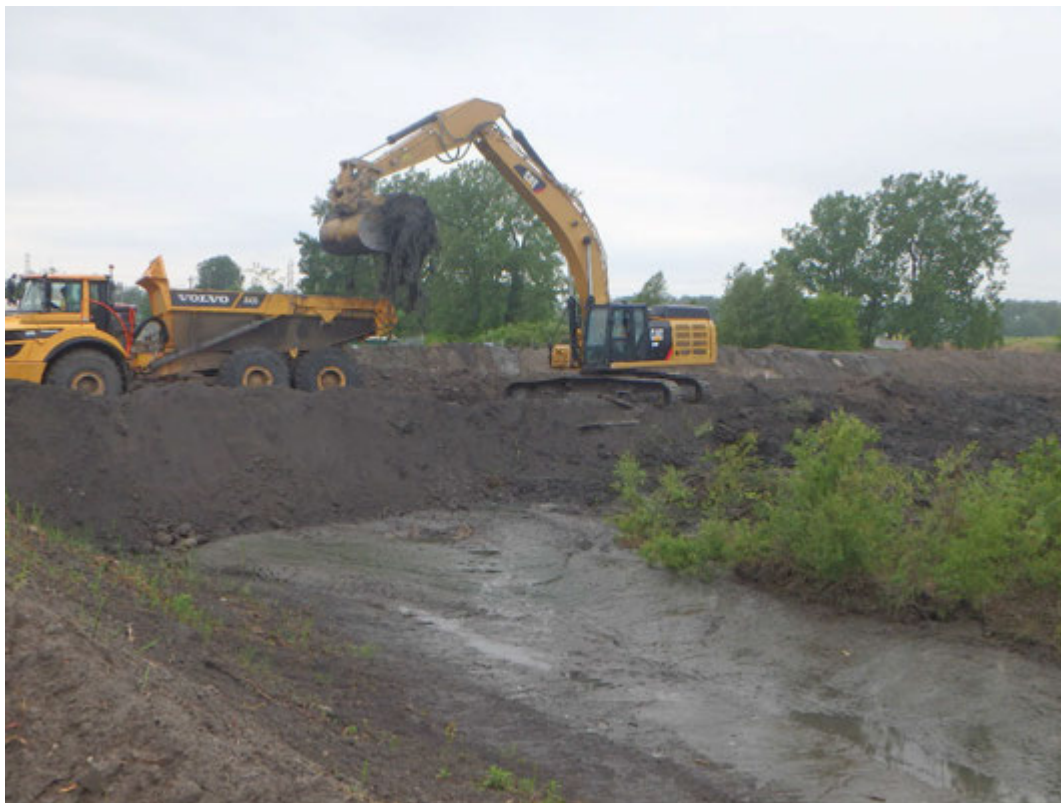
Clearing vegetation from Pond 1, looking west.
