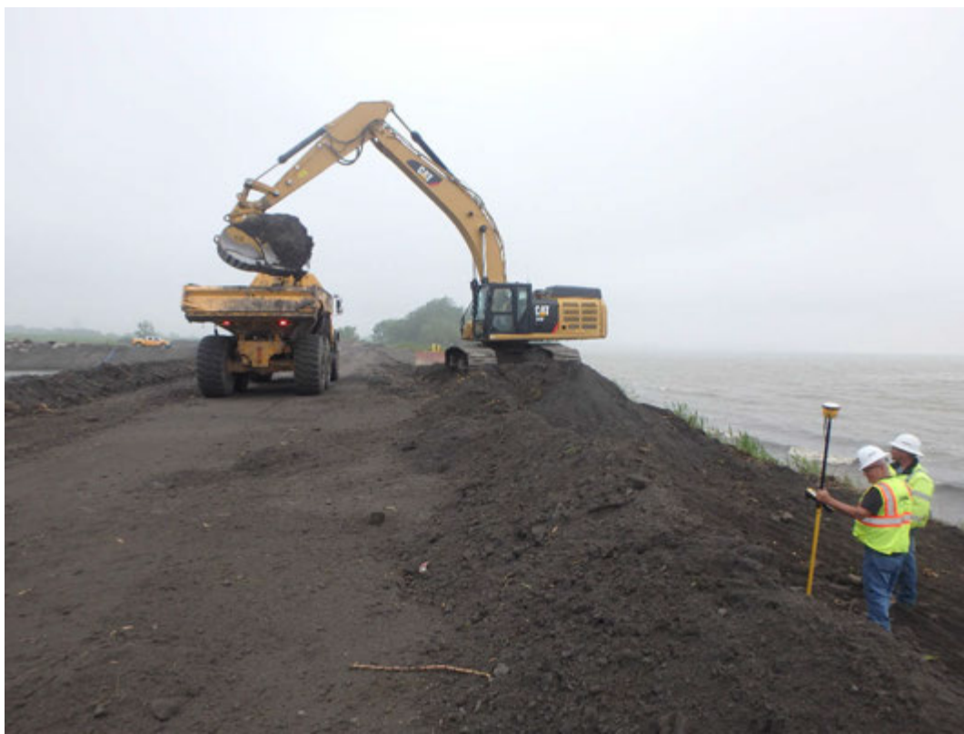
Excavating bench above shoreline east of Pond 2, Looking North
