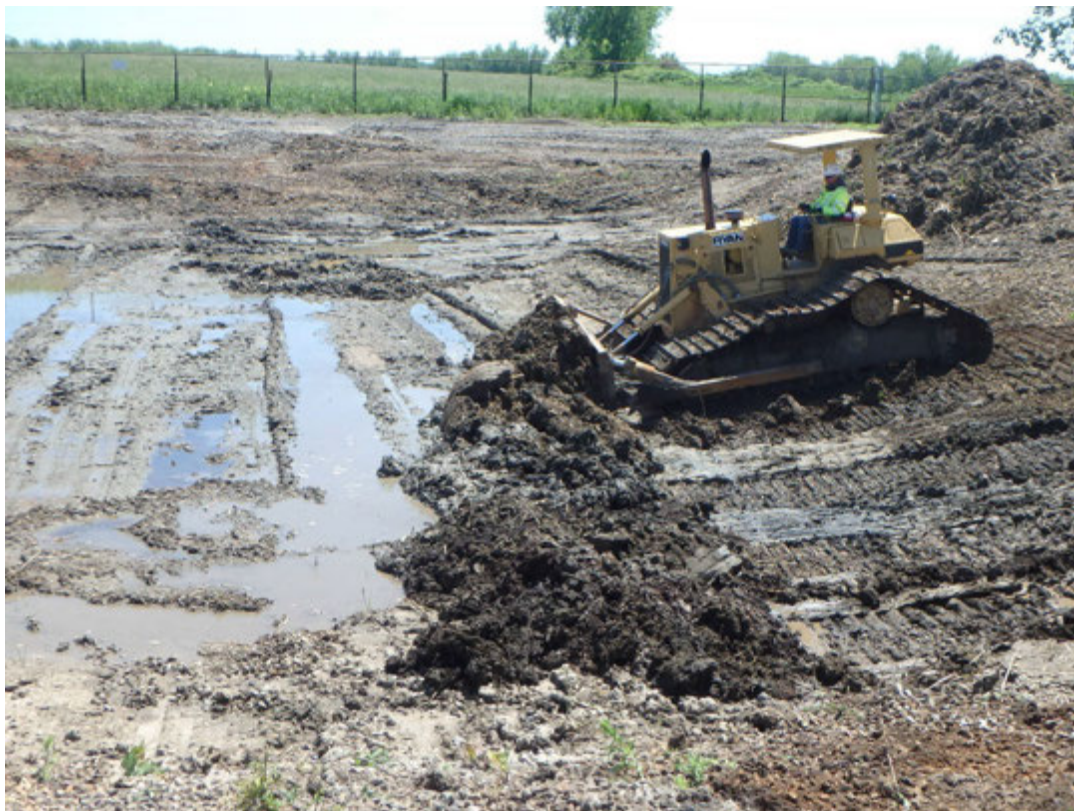
Cutting residual material in Chemical Pond A to dry prior to removal
