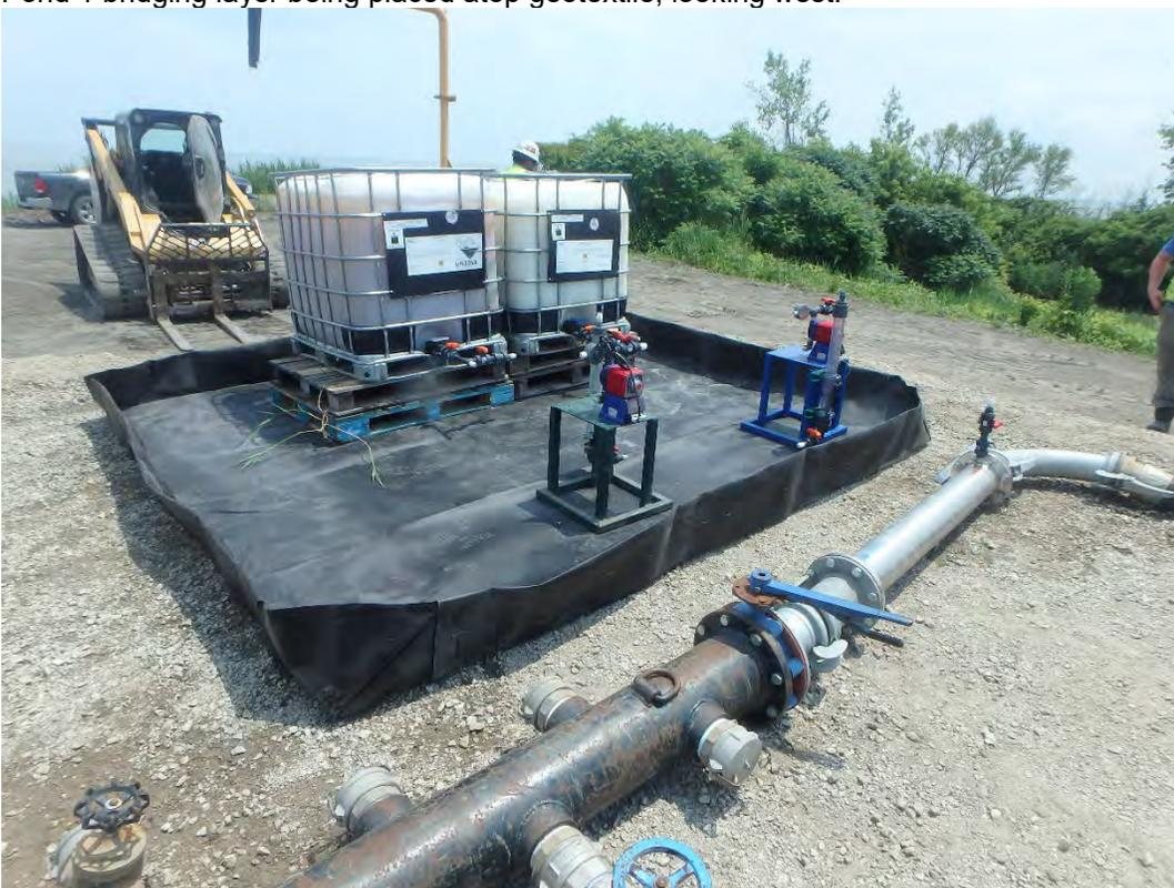
Installing equipment to supply Flocculant to supply side of Pond 2 dewatering system, looking southeast.
