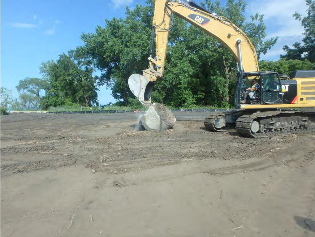
Removing utility pipe crock at the Chemical Ponds, looking east.
