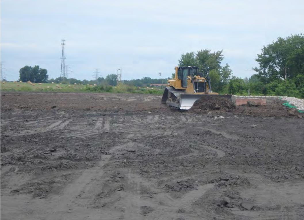
Placing lift of structural fill east of Pond 1 along top of shoreline slope, looking north.
