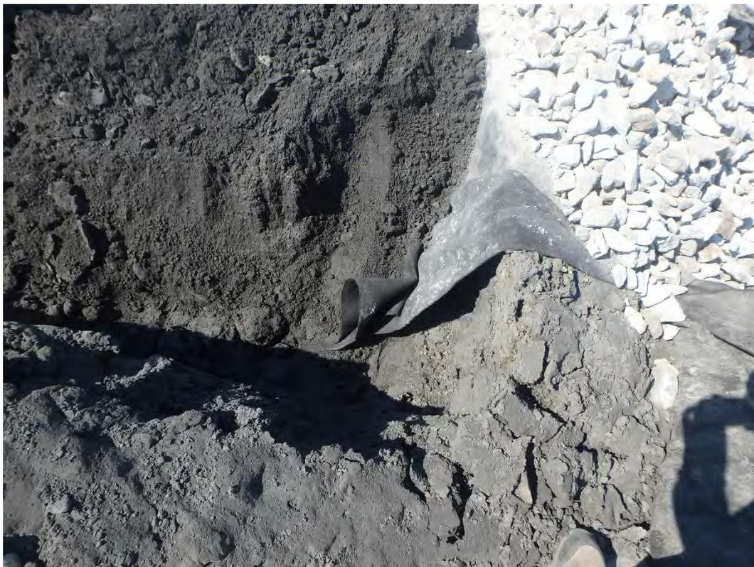
Shoreline geotextile in anchor trench with backfill.
