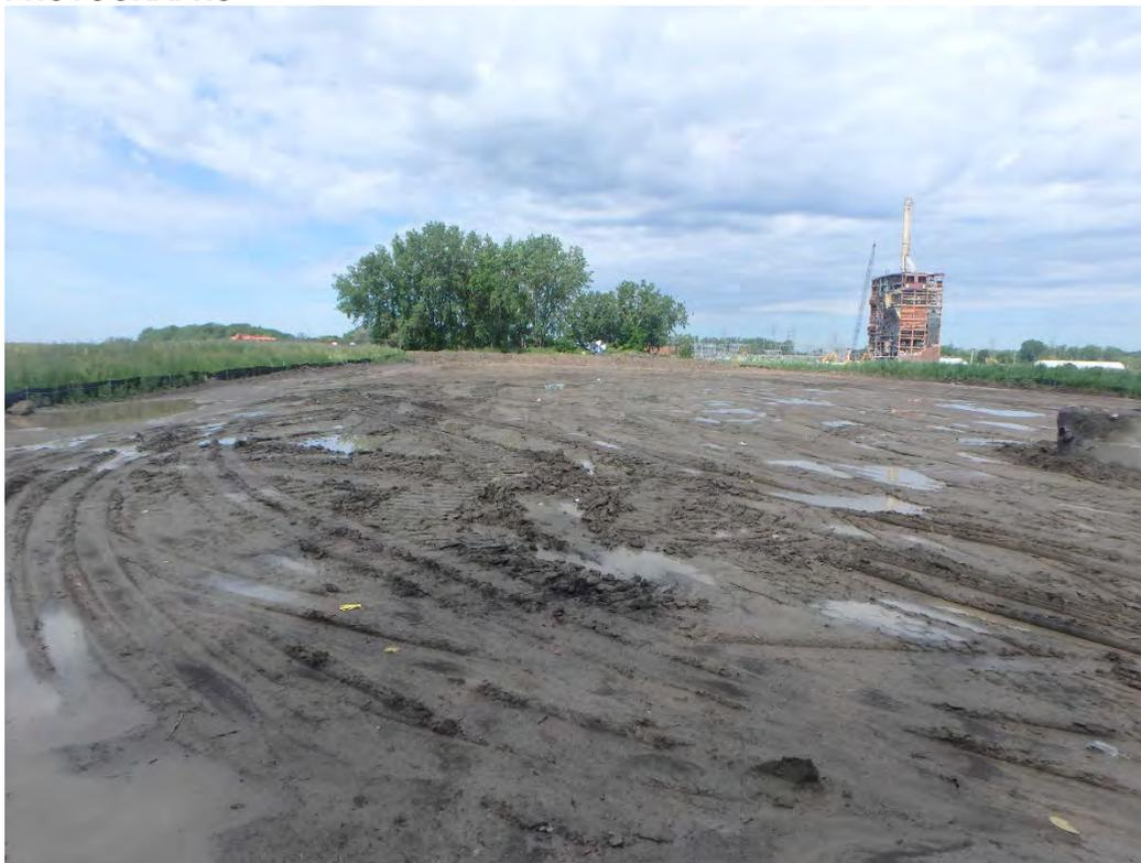
Chemical Ponds 1<sup>st</sup> lift of structural fill after previous night's rain, looking west.
