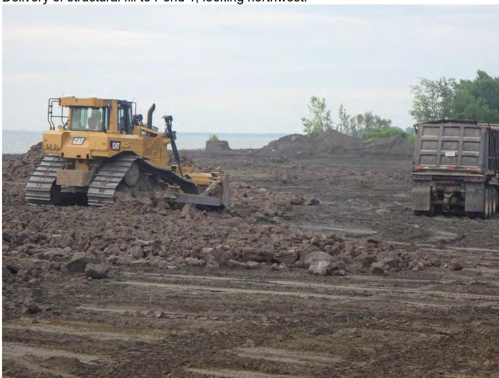
Placing lift of structural fill in Pond 1, looking southeast.
