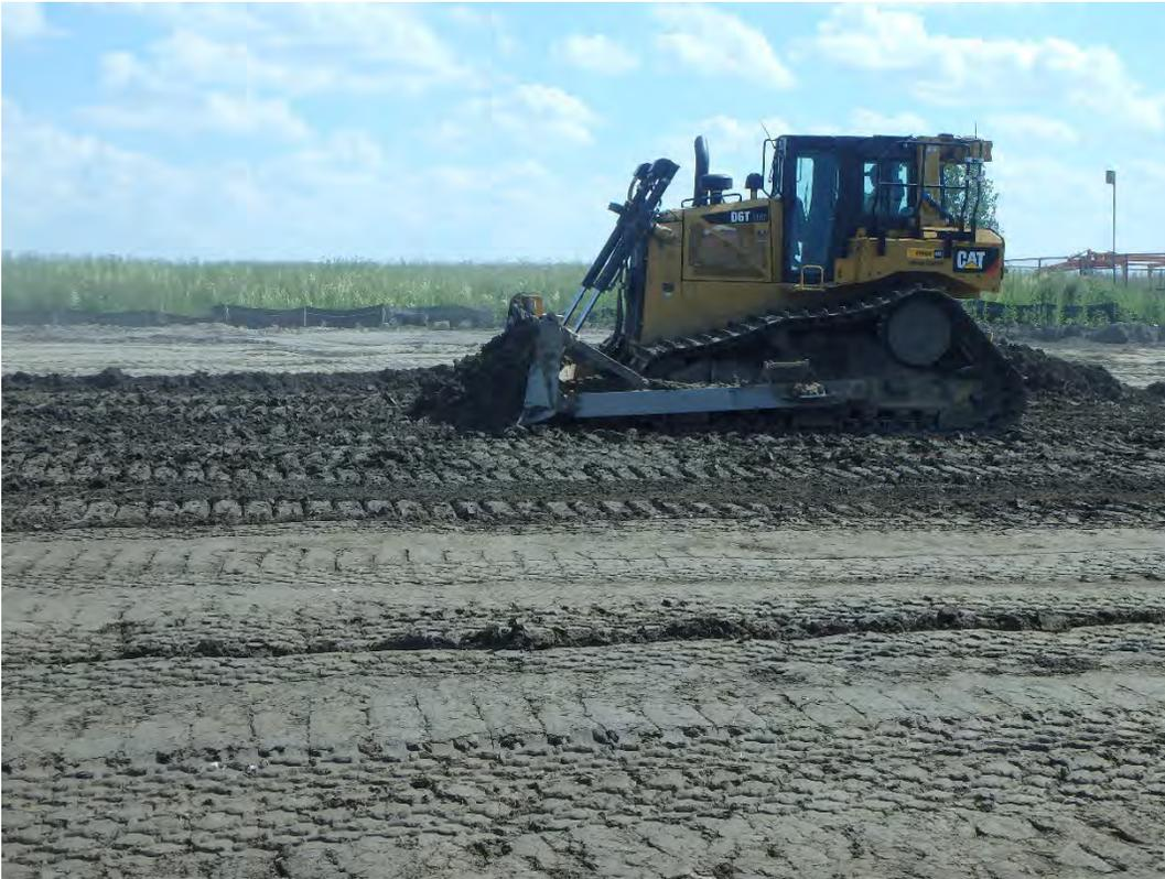
Placement of 12 inch loose lift of structural fill at chemical ponds, looking south.
