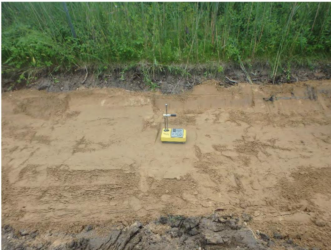
Testing of compacted pipe bedding for culvert.
