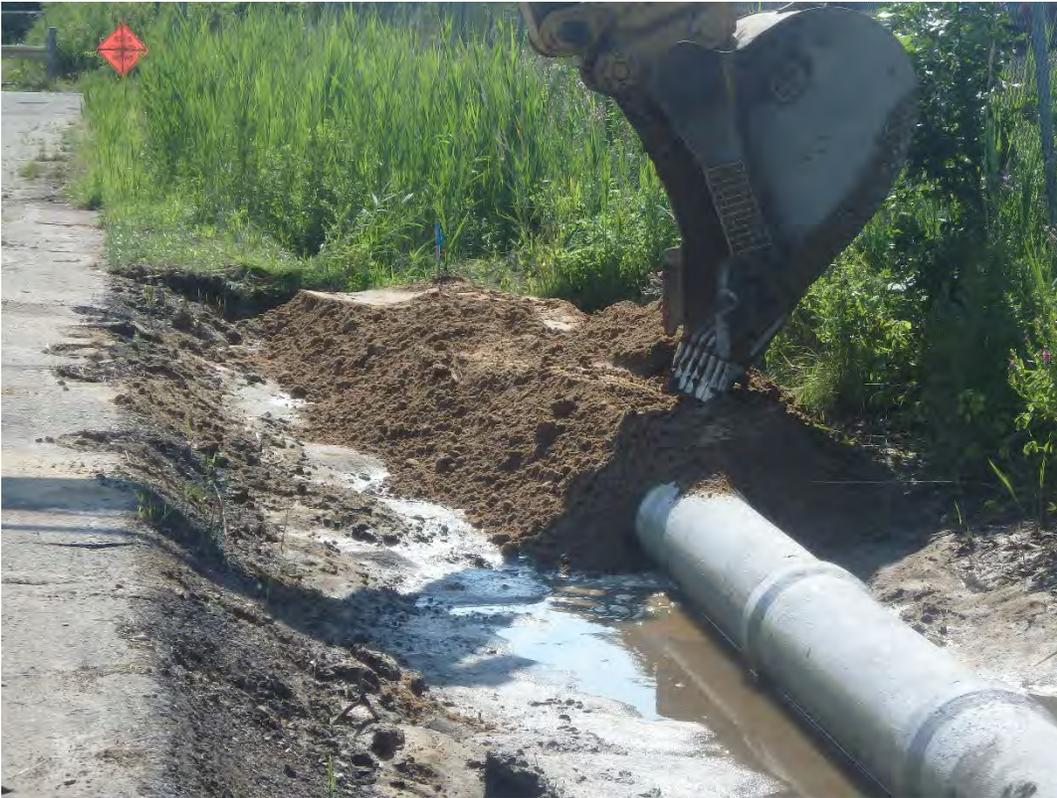
Placement of class IIIA sand for backfill over access road culvert, looking east.
