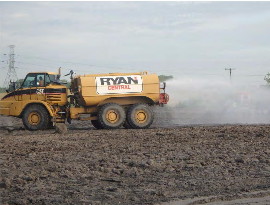
Water truck used to moisture conditioning of placed structural fill and dust control, looking west.
