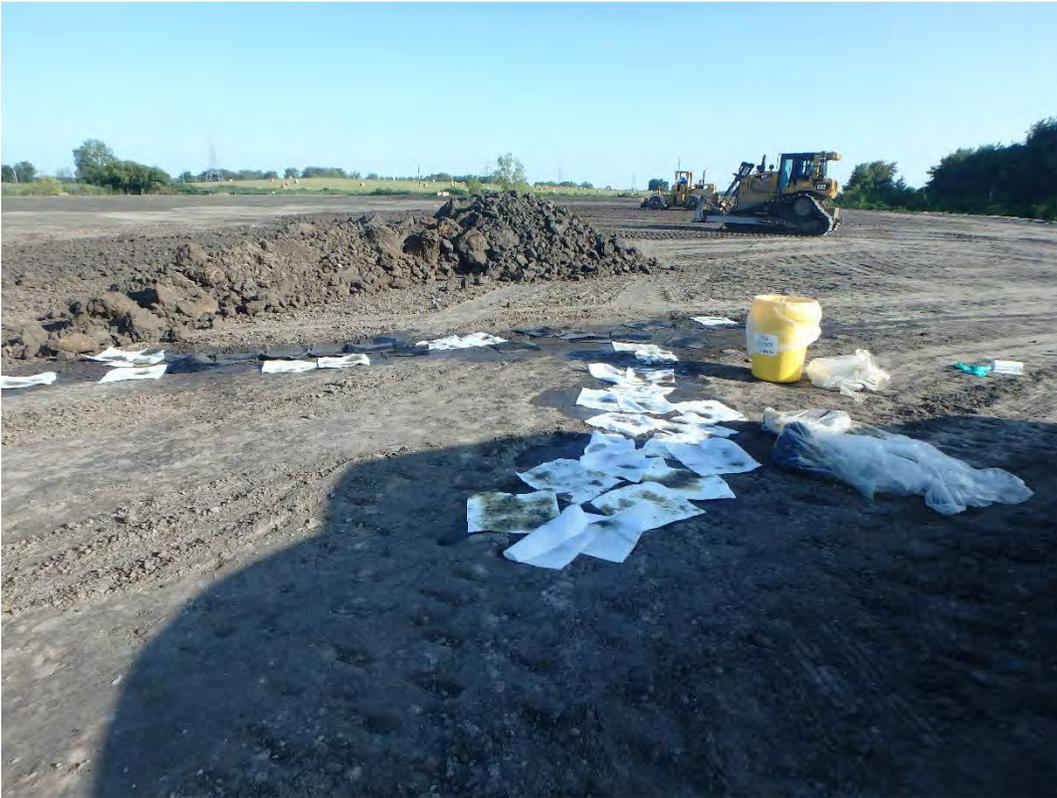
Absorbent pads used for hydraulic oil leak in Pond 1, looking north.
