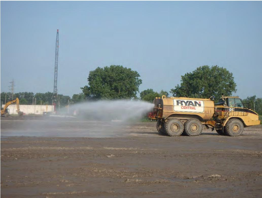
Dust control and moisture maintenance of fill placed in Pond 1, looking west.
