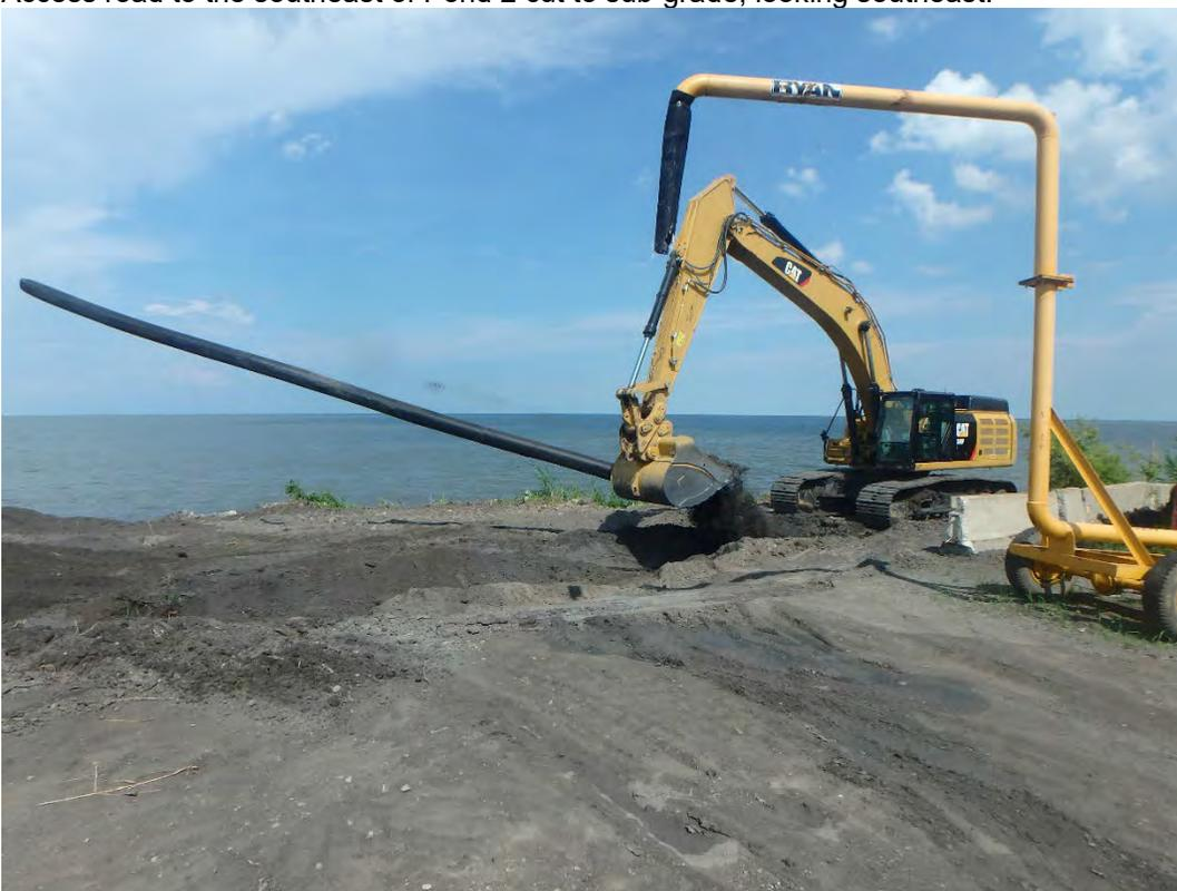
Removing utility pipe running from southeast corner of Pond 2 too Chemical Ponds, looking east.
