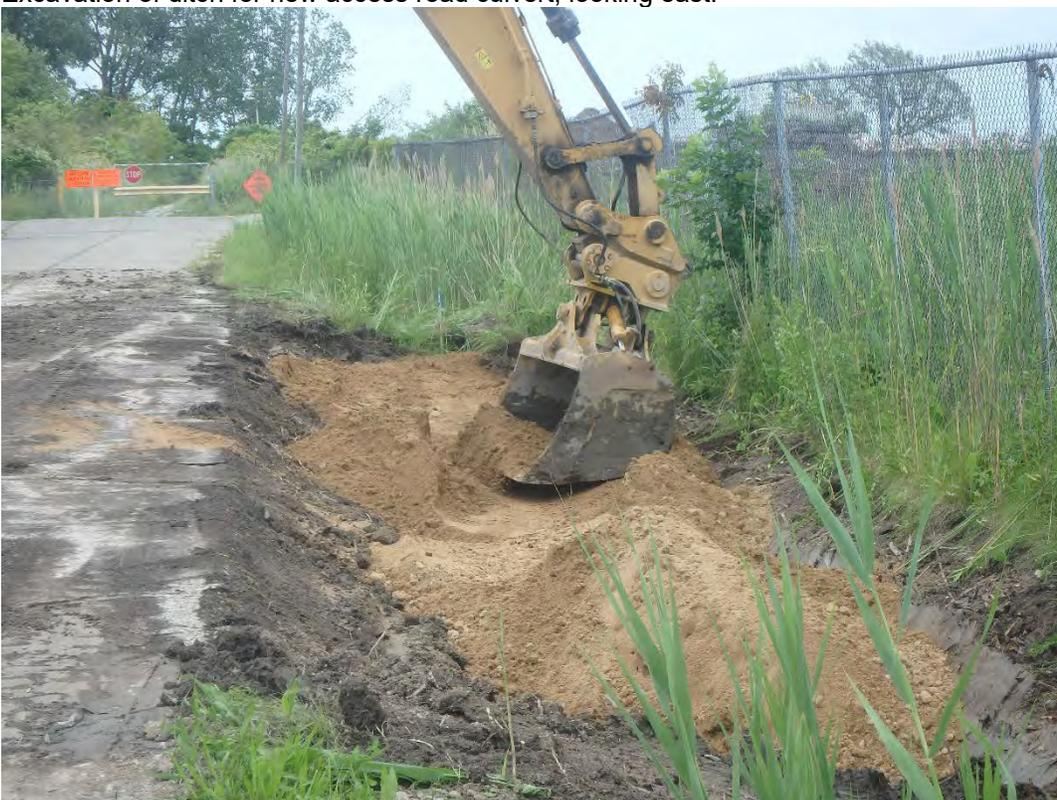
Placement of culvert bedding material, looking east.
