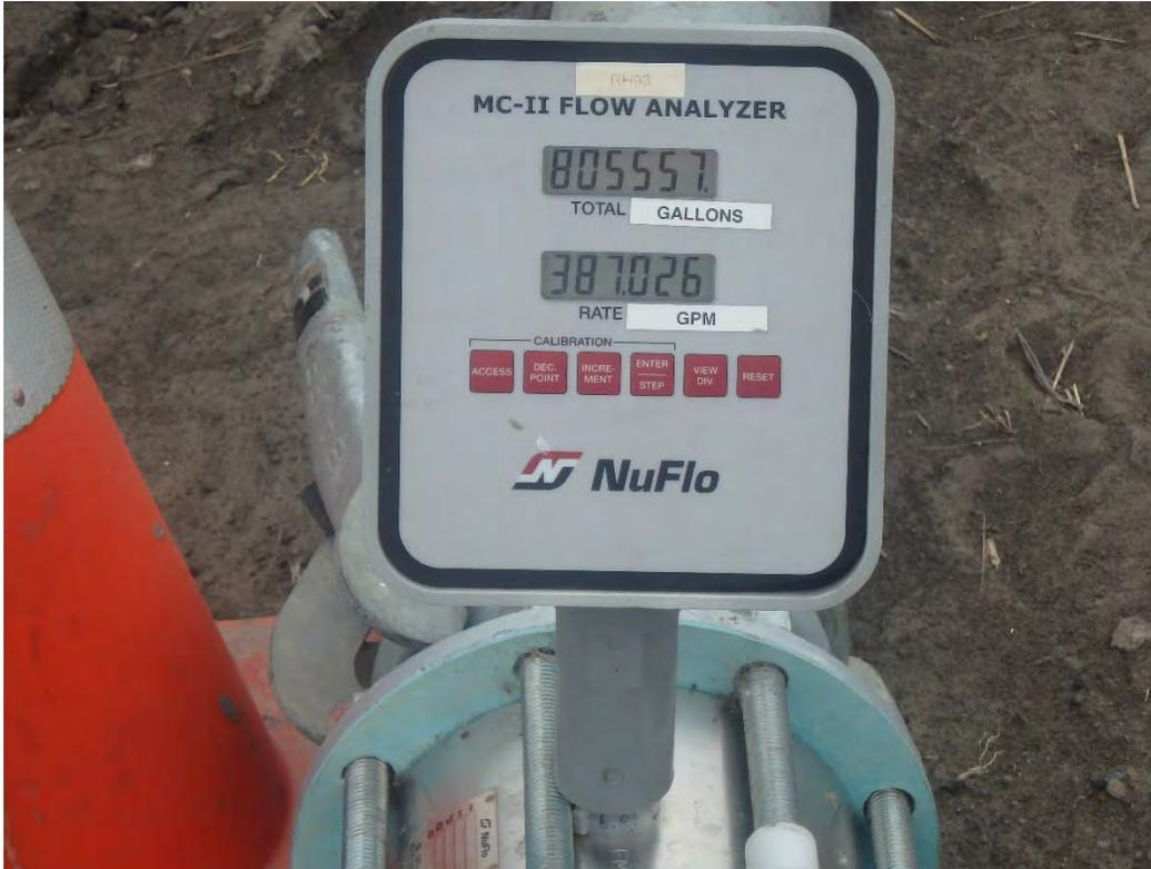
Discharge flowmeter on dewatering system in Pond 2.
