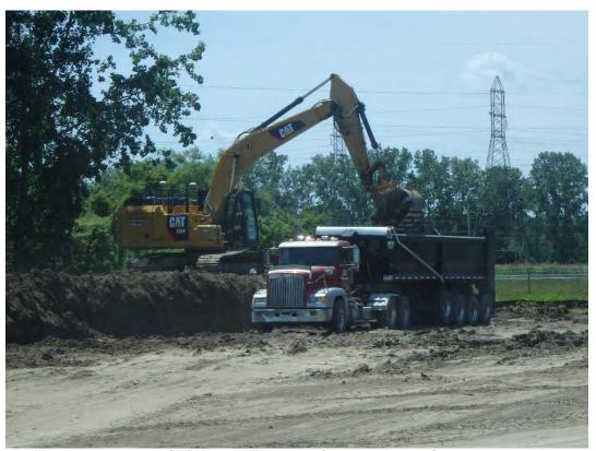
Loading onsite structural fill for stockpiling in the Chemical Ponds Grading area, looking west.
