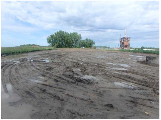
Chemical Ponds 1st lift of structural fill after previous night's rain, looking west.
