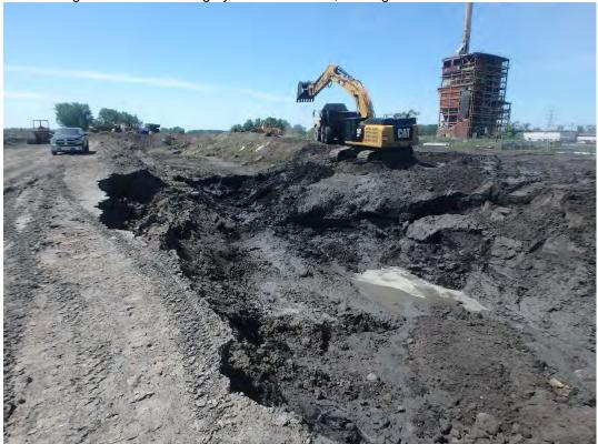
Removal of saturated material from along the west side of Pond 1, looking south.
