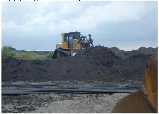
Placing bridging layer over textile in Pond 2, looking west.
