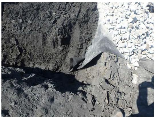
Shoreline geotextile in anchor trench with backfill.
