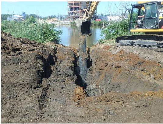
Removing standpipe into Fore Bay from Pond 1, looking west.
