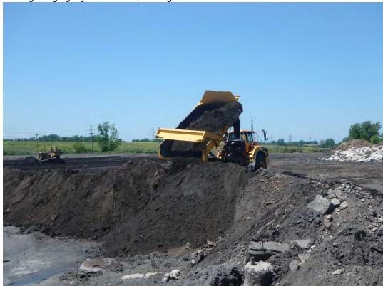
General fill from grading of shoreline being placed into Pond 1, looking north.
