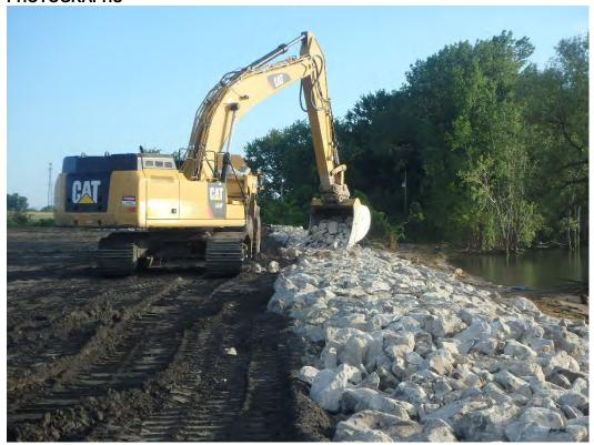
Placing 8 x 16 inch riprap to fill voids in the D50/30 inch along shoreline, looking north.
