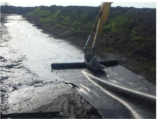
Installation of geotextile in Pond 1 prior to bridging layer, looking east.
