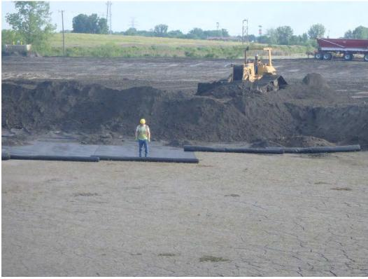
Deployment of geotextile and placement of bridging layer in Pond 1, looking north.
