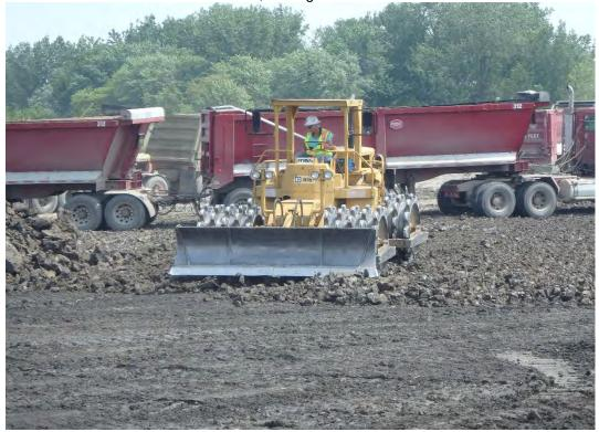
Compacting structural fill placed in Pond 1, looking northeast.
