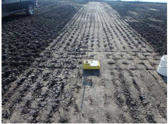
Density test of compacted structural fill in Pond 1, looking east.
