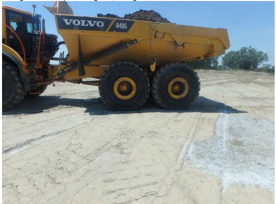
Proof roll of onsite structural fill placed over chemical ponds, looking west.
