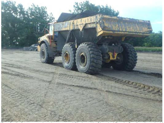
Proof roll of compacted onsite structural fill placed in Chemical Ponds Grading Area, looking west.
