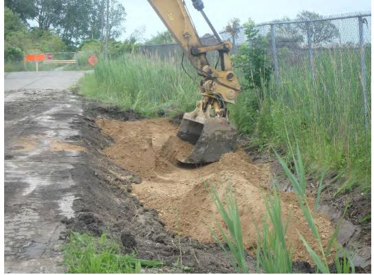
Placement of culvert bedding material, looking east.
