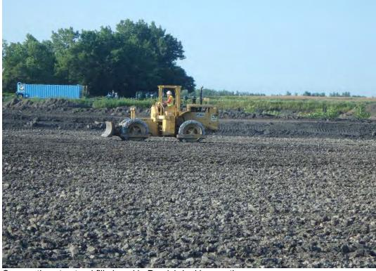
Compacting structural fill placed in Pond 1, looking south.
