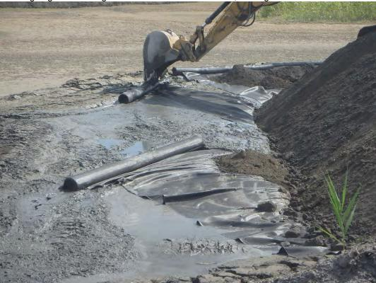
Deploying textile for bridging layer in Pond 2.
