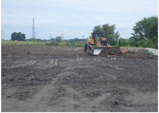
Placing lift of structural fill east of Pond 1 along top of shoreline slope, looking north.
