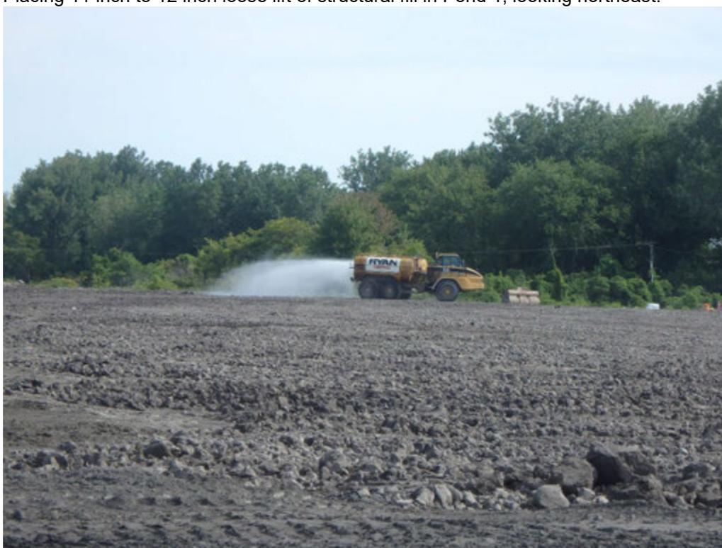
Moisture conditioning of structural fill in Pond 1, looking northeast.
