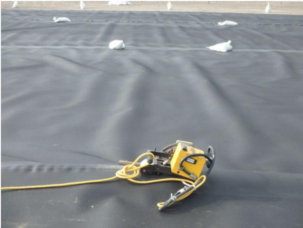
Seaming by fusion method of geomembrane.
