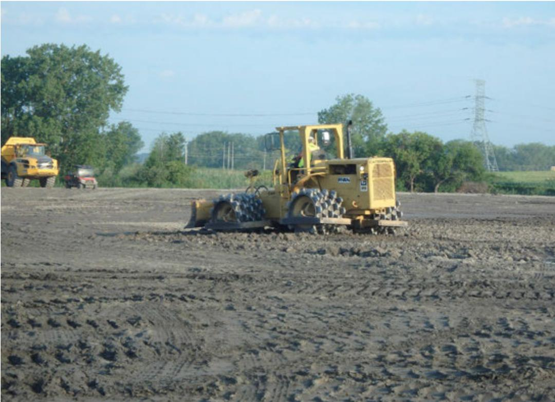
Compacting placed structural fill in Pond 1, looking northwest.
