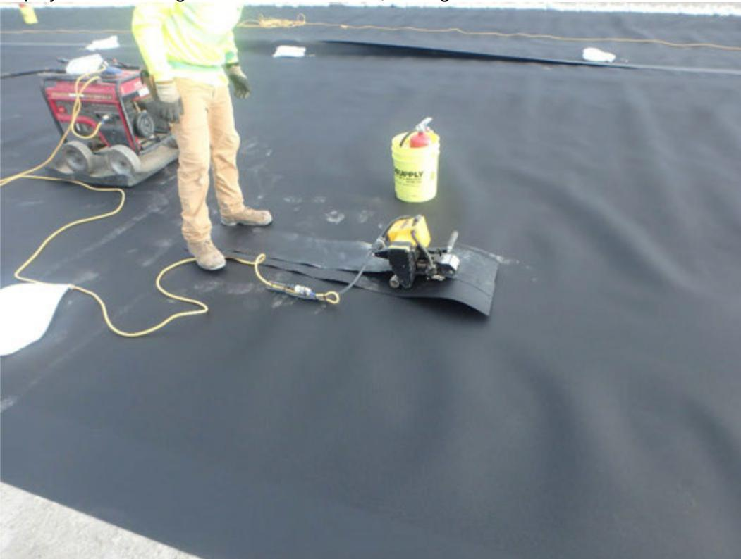
Producing trial weld for field testing.
