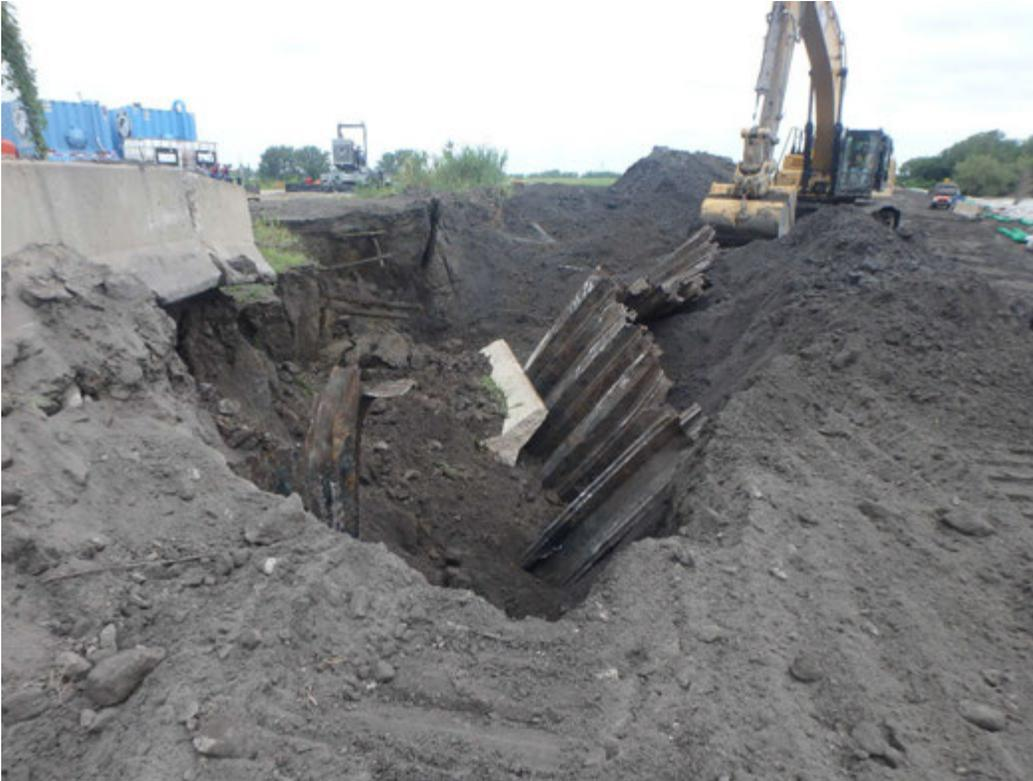
Removing sheet pylon east of Pond 2 and discharge channel, looking north.
