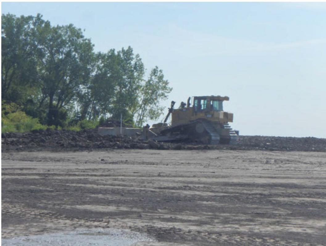
Placing 11 inch to 12 inch loose lift of structural fill in Pond 1, looking northeast.
