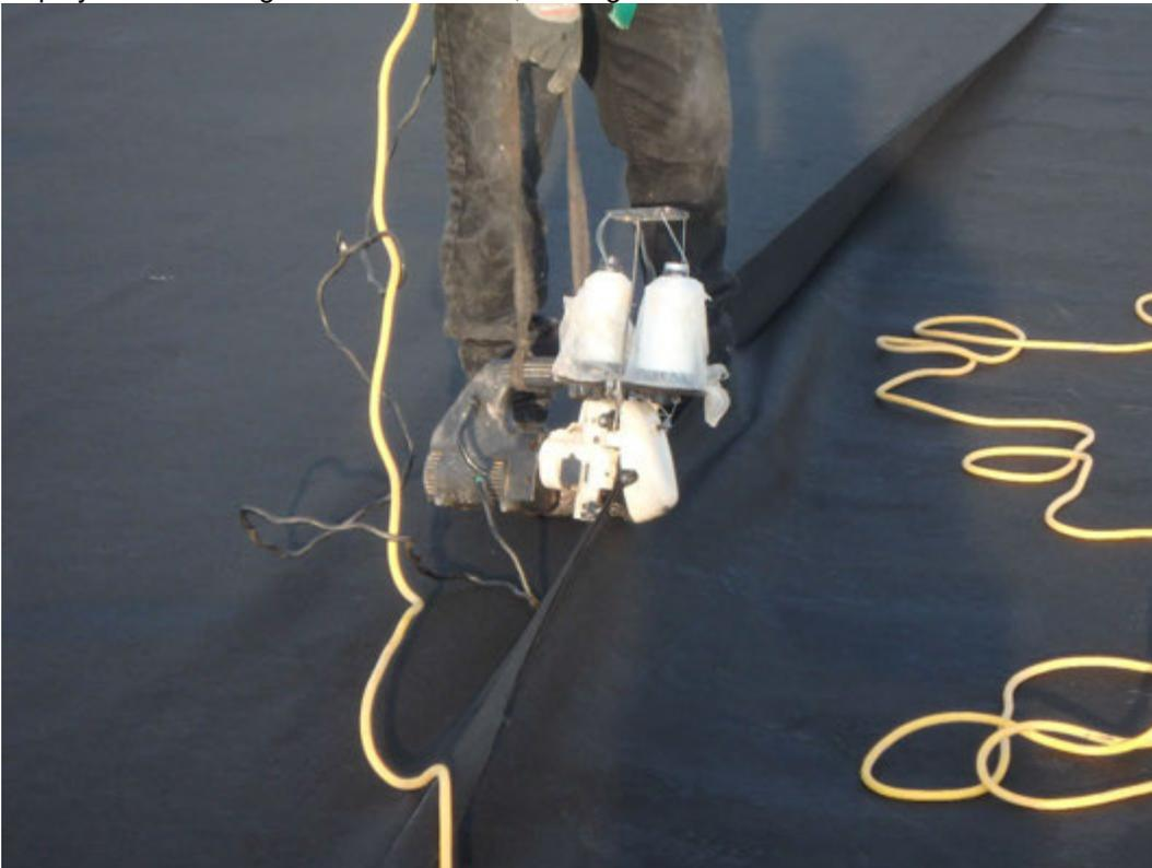
Sewing geotextile seam.
