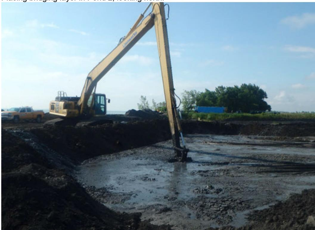
Removing saturated CCR from the northeast corner of Pond 2, looking southeast.
