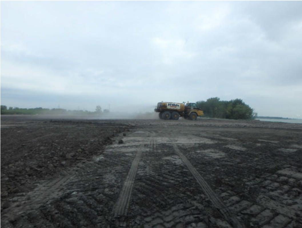
Maintaining moisture of placed fill and dust control, looking north.
