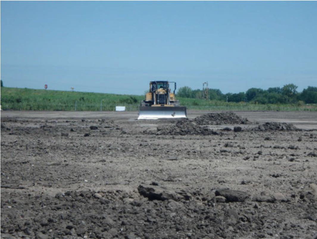
Finish grading Pond 1 liner sub-grade, looking north.
