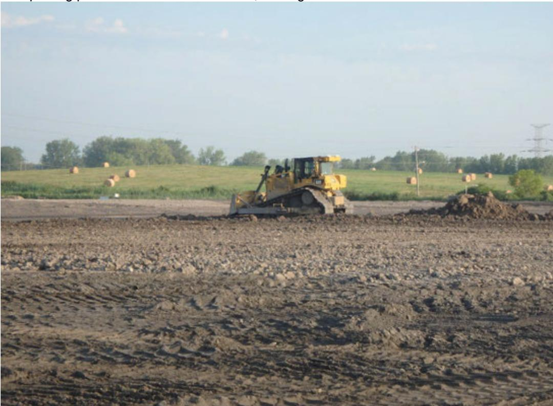
Placing structural fill in Pond 1, looking north.
