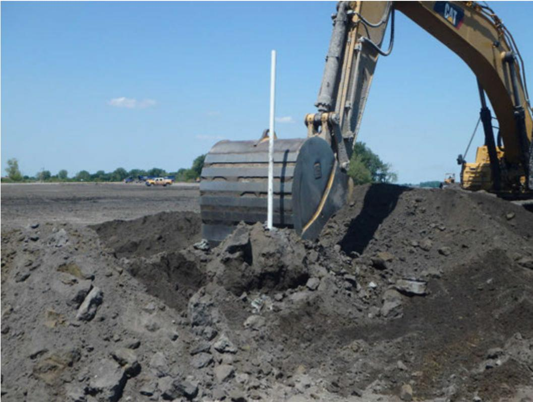
Removing remaining CCR from around MW-15005, looking northeast.
