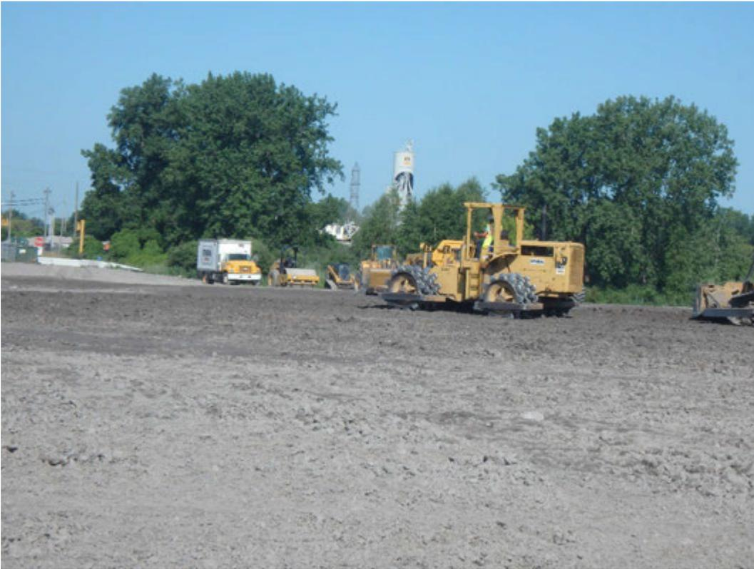
Compaction of structural fill placed in Pond 1, looking west.
