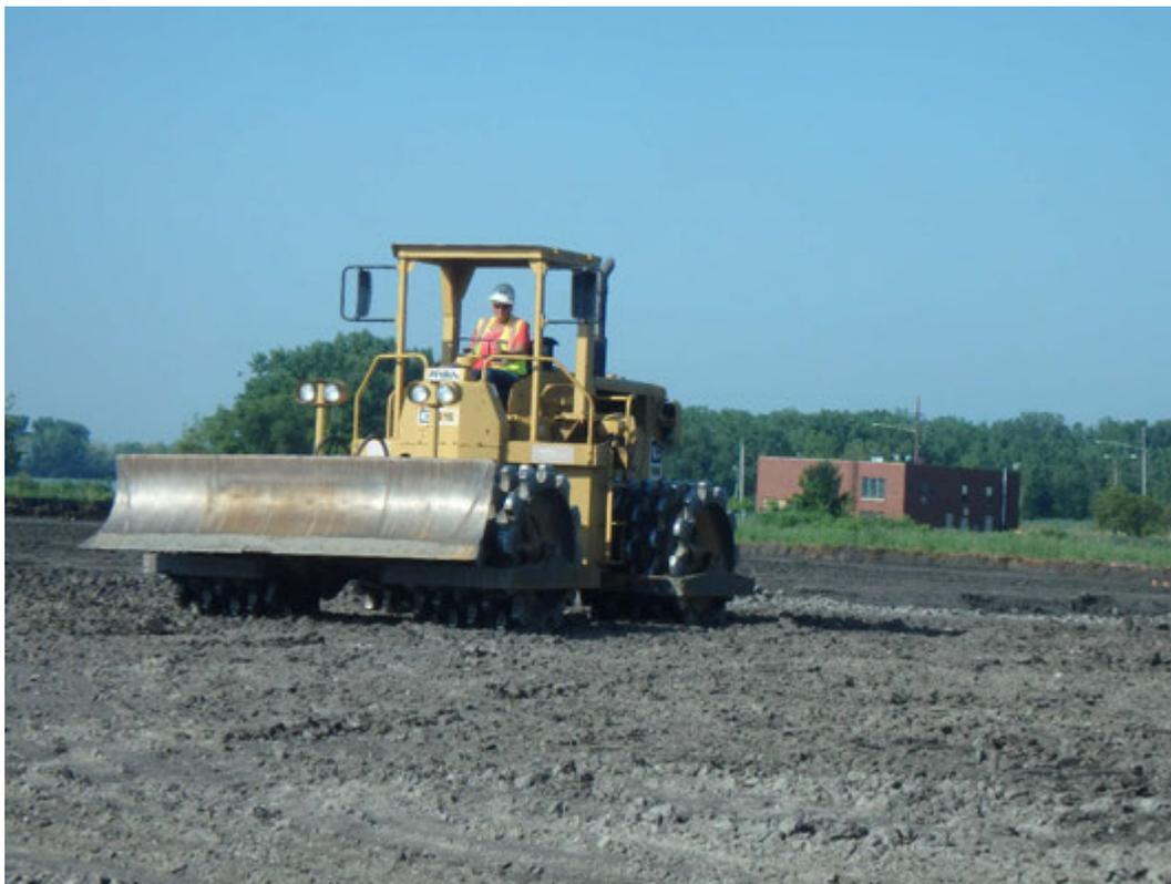
Compaction of placed lift of structural fill in Pond 1, looking west.
