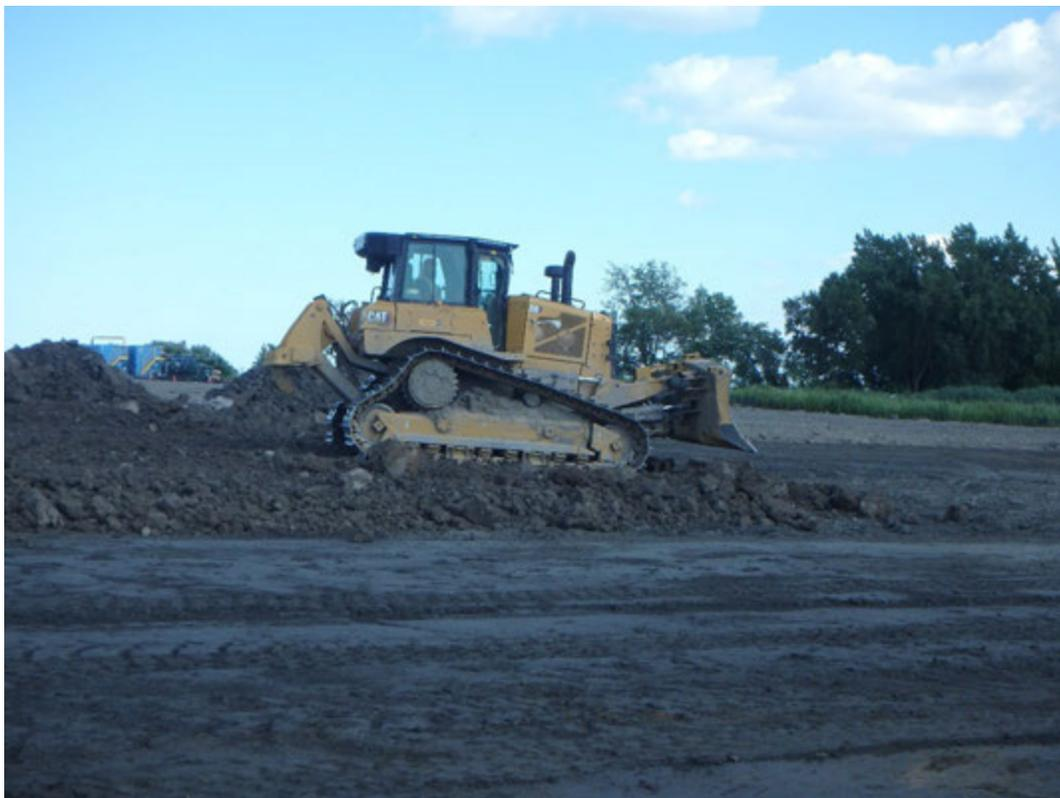
Placement of structural fill lift in Pond 2, looking south.
