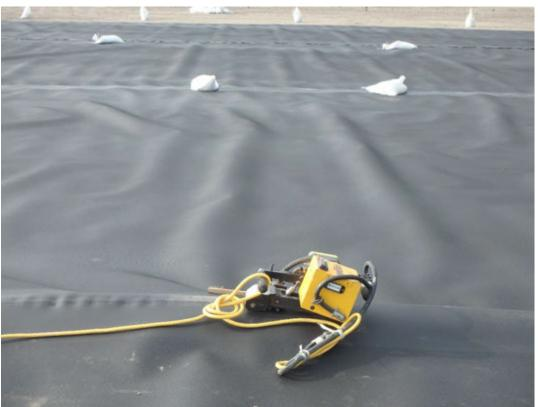
Seaming by fusion method of geomembrane.
