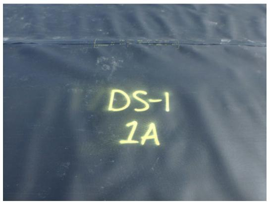
Destruct location marked for removal and testing.
