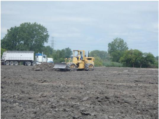
Compacting lift of structural fill placed in Pond 1, looking northeast.
