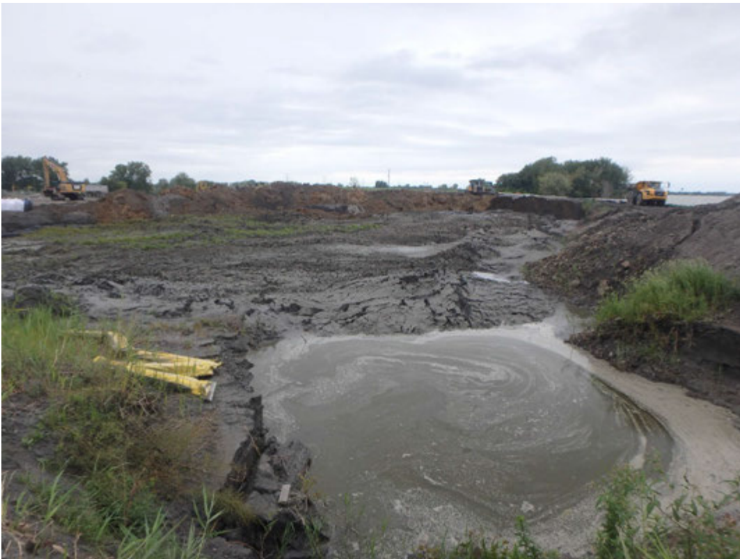
Southeast corner of Pond 2, looking north.
