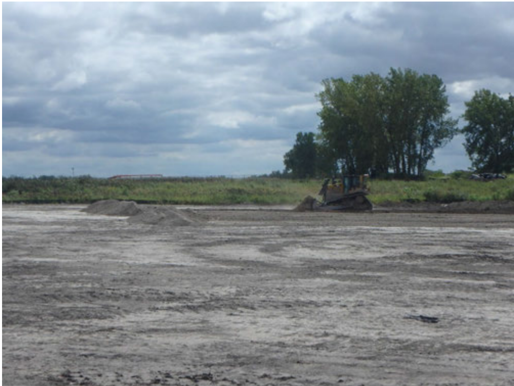
Finish grading of Pond 2's liner sub-grade, looking south.
