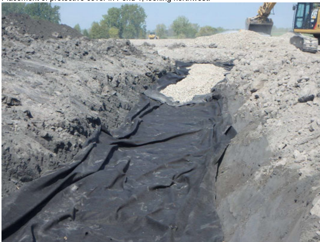
Placing 1x3 inch stone in trench excavated in southeast corner of Pond 2's bridging layer, looking north.
