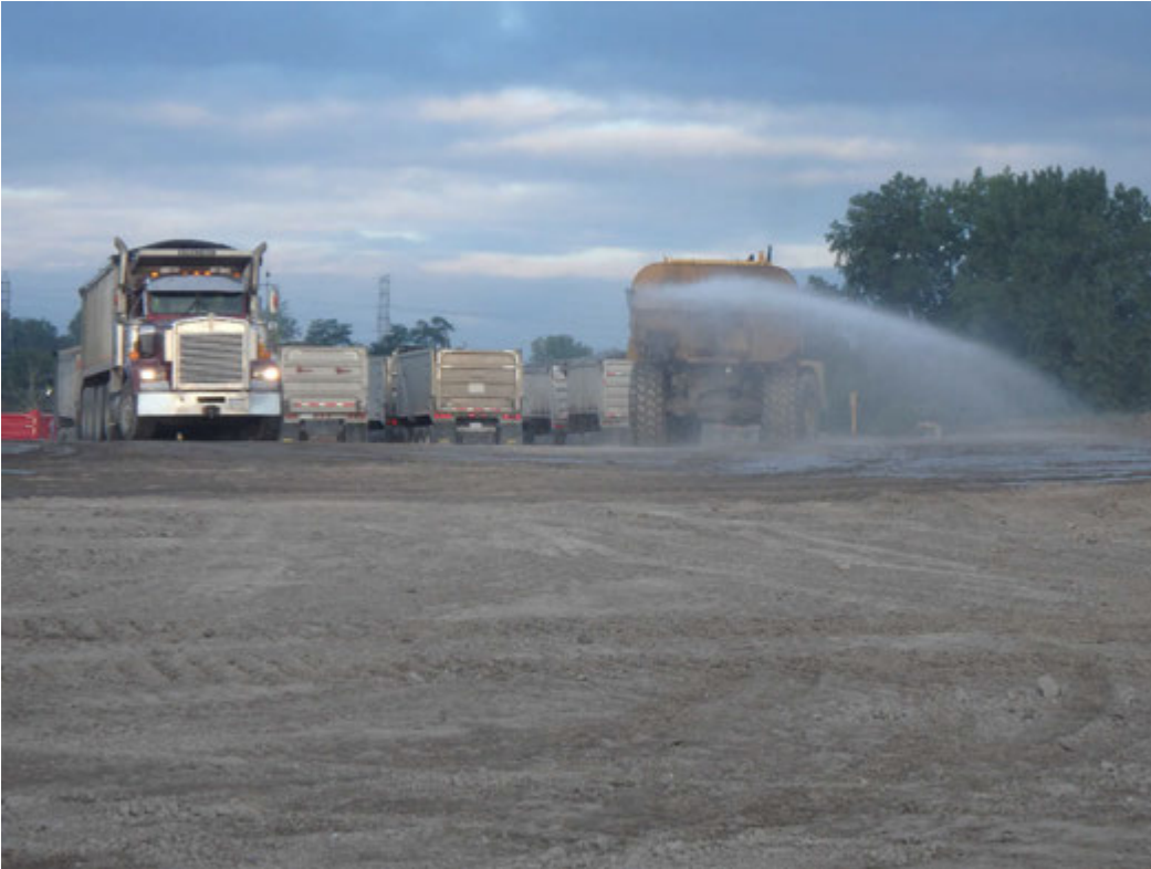
Water truck for dust control and maintain fill moisture, looking west.
