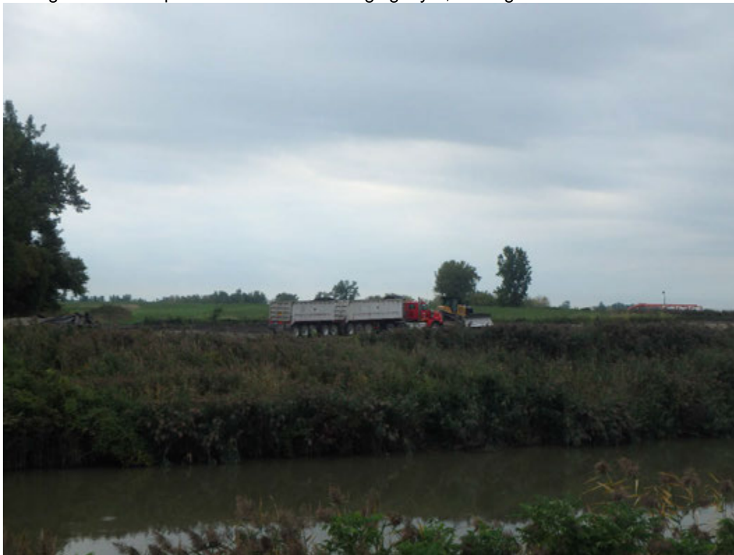
Structural fill being placed in the Chemical Ponds work area, looking south.
