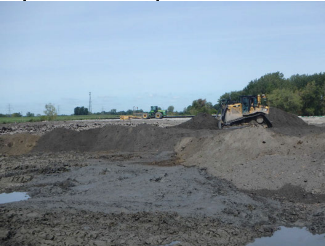
Placing bridging layer in Pond 2, looking north.
