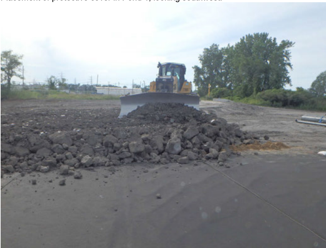
Protective cover being placed atop geosynthetics in Pond 1, looking west.
