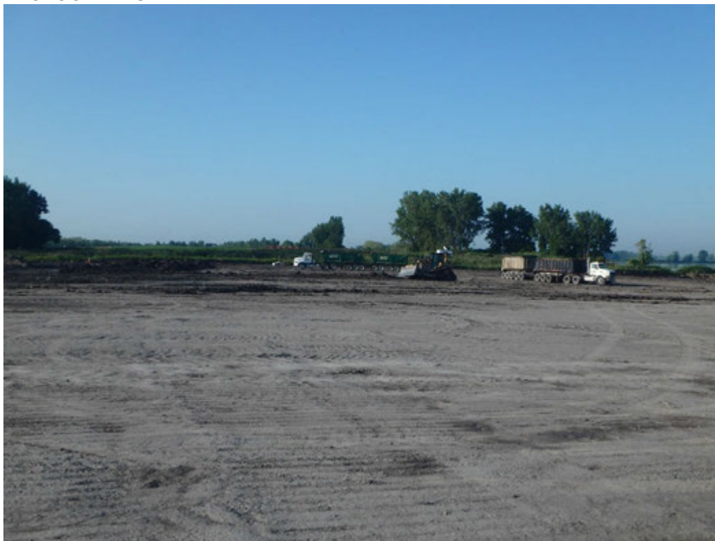
Deployment of geotextile in Pond 1, looking northwest.
