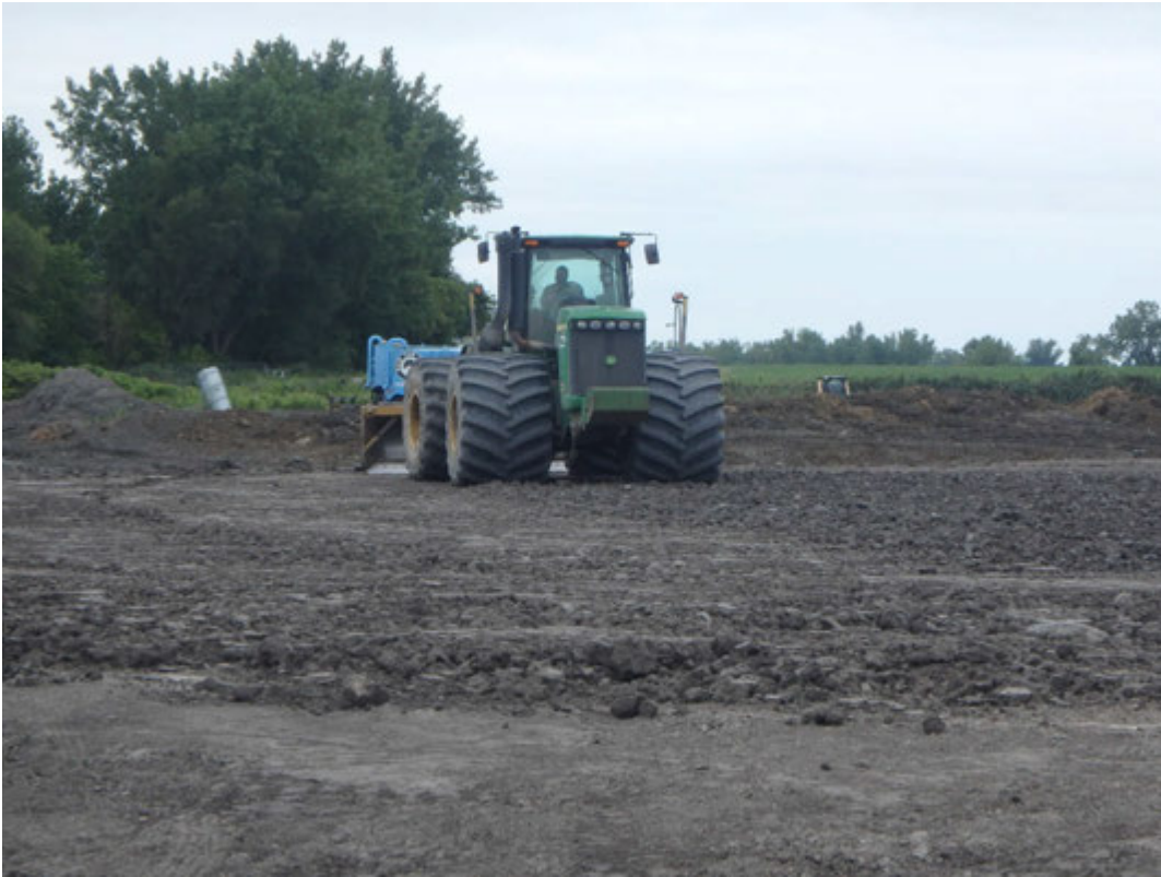
Sealing placed structural fill using towed box-blade with roller, looking south.
