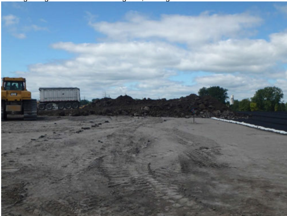
2 nd ramp built using protective cover over Pond 1 geosynthetics, looking west.
