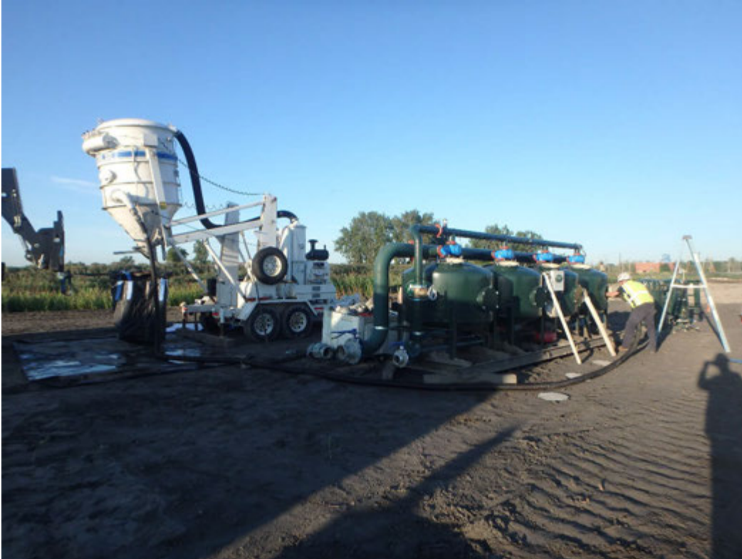
Cleaning out sand pots of filter system for demobilization, looking southwest.
