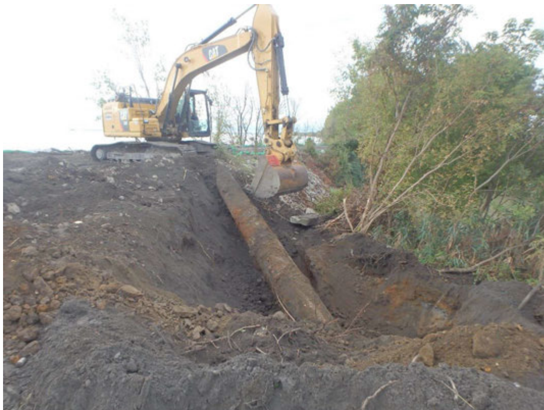
Removal of 24 inch pipe southeast of Pond 2, looking southeast.
