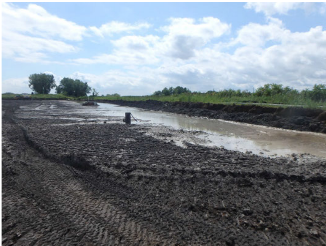
West side of Pond 2 after previous night's rain, looking south.
