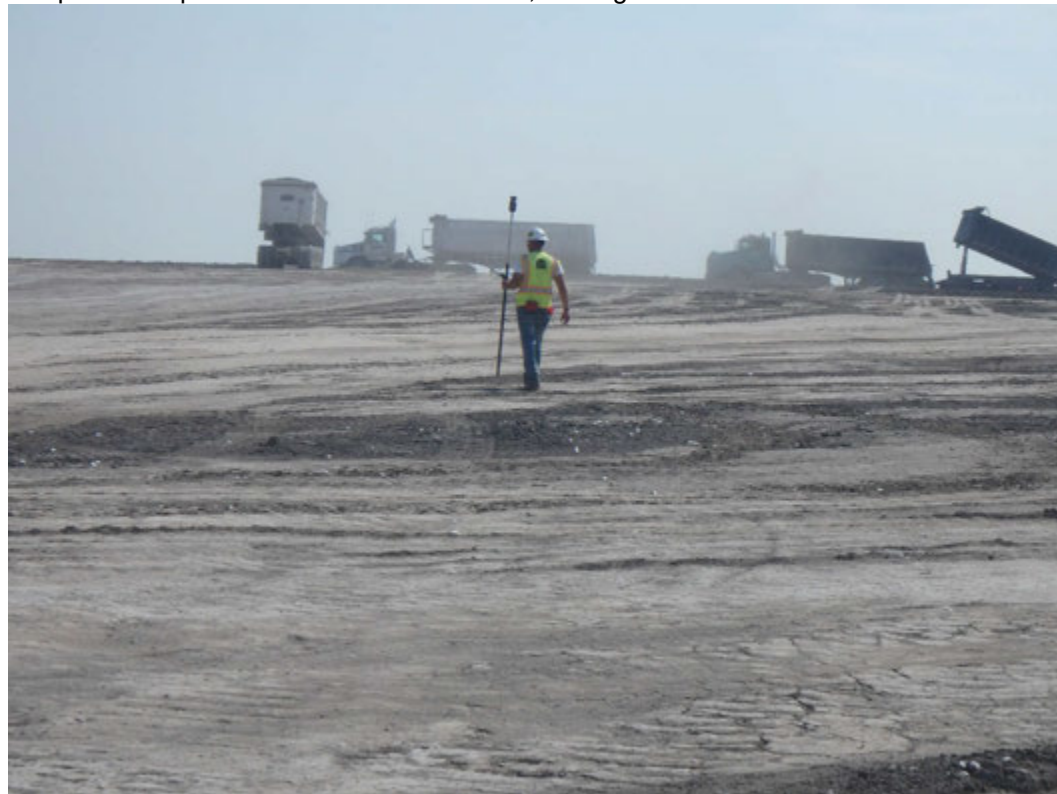
Rowe surveyor shooting sub-grade certification points in Pond 2, looking east.
