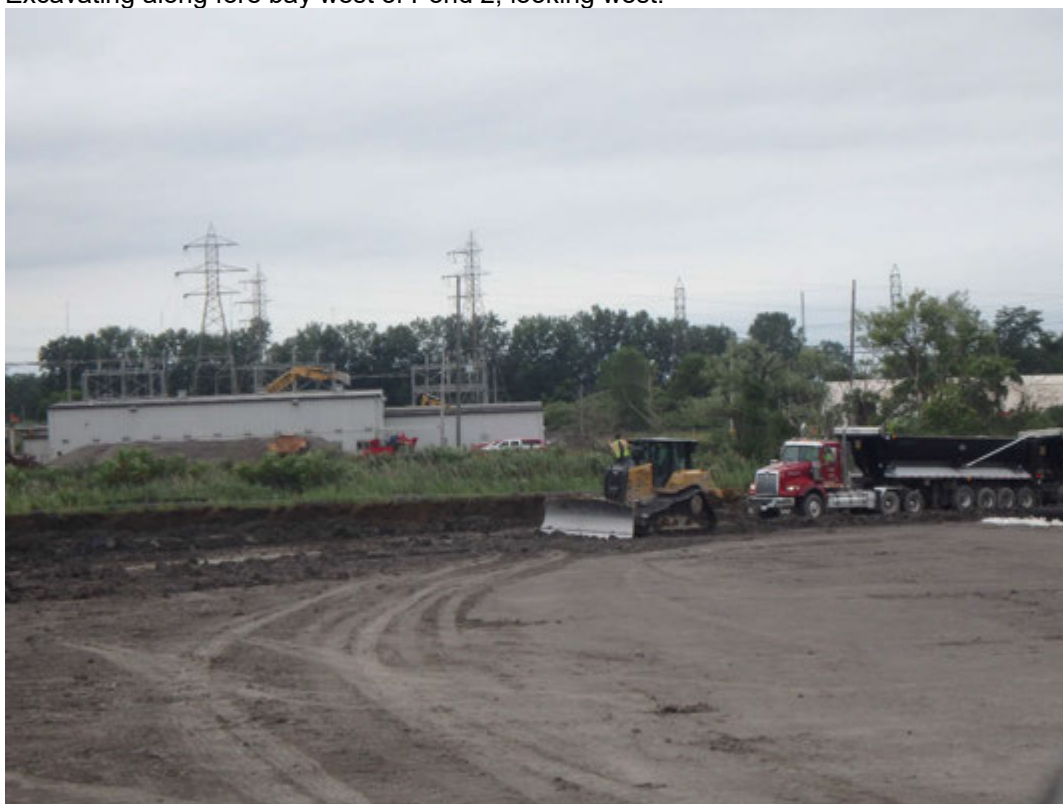
Import of structural fill to Pond 2, looking west.
