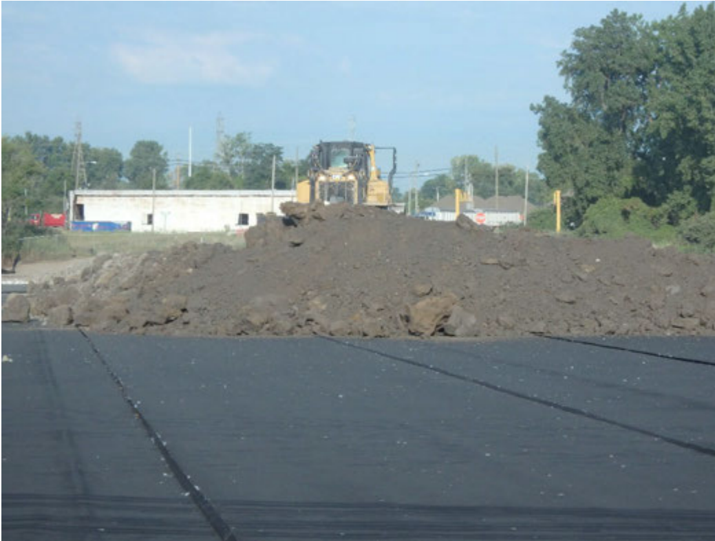
Placement of protective cover for construction of 4 foot haul road in Pond 1, looking west.
