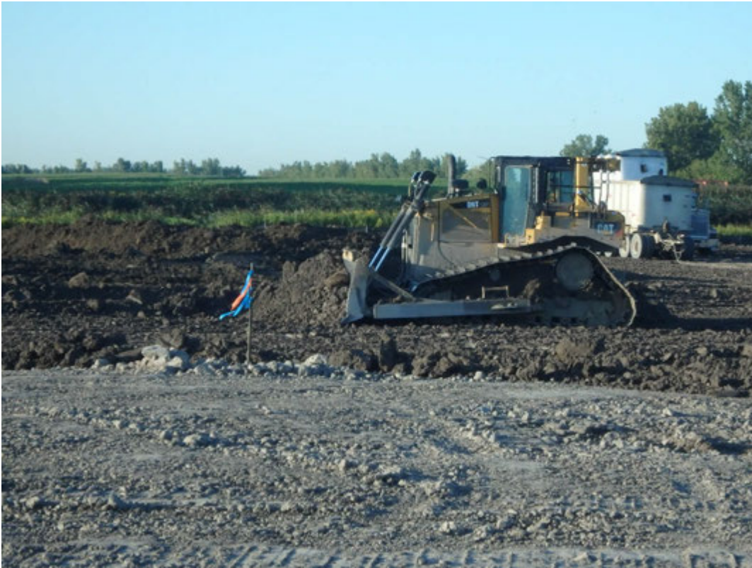
Placement of structural fill in Pond 2, looking south.
