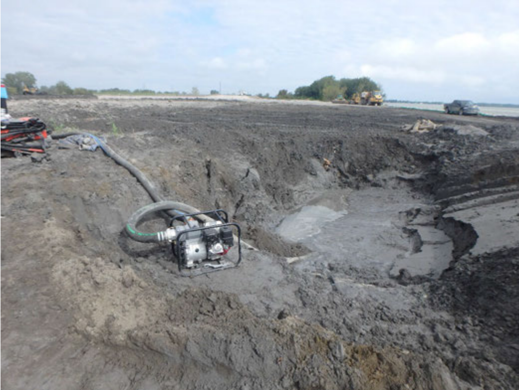
Pumping of standing water from southeast corner of Pond 2 to baker tank, looking northeast.
