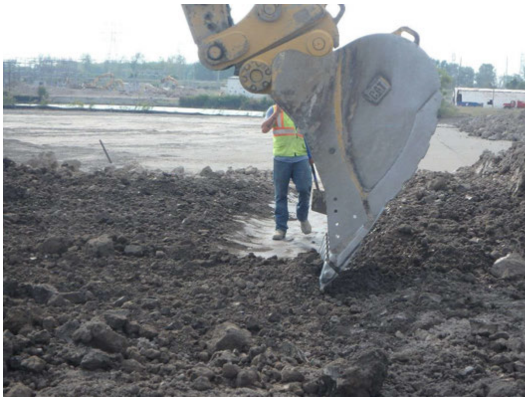
Removing temp ramp atop liner tie-in along south side into Pond 1, looking west.
