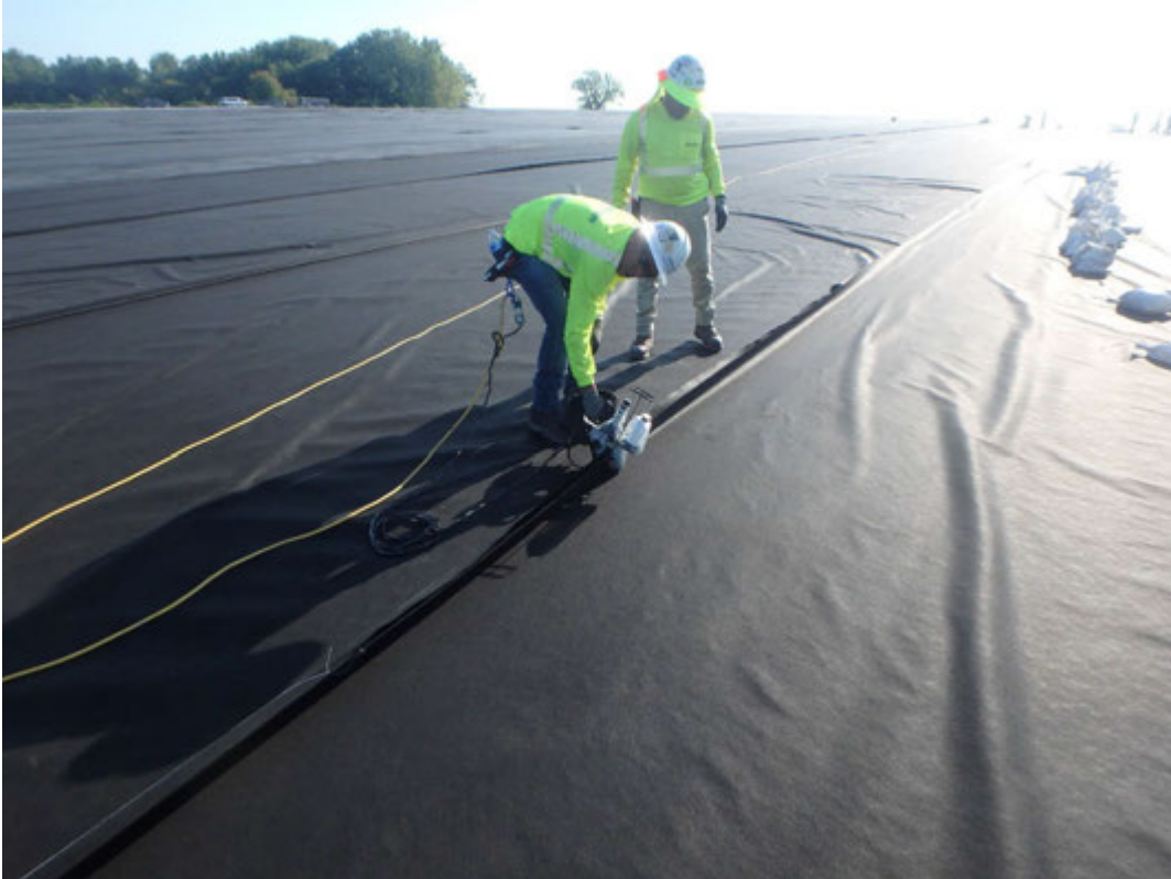
Sewing geotextile seam, looking northeast.
