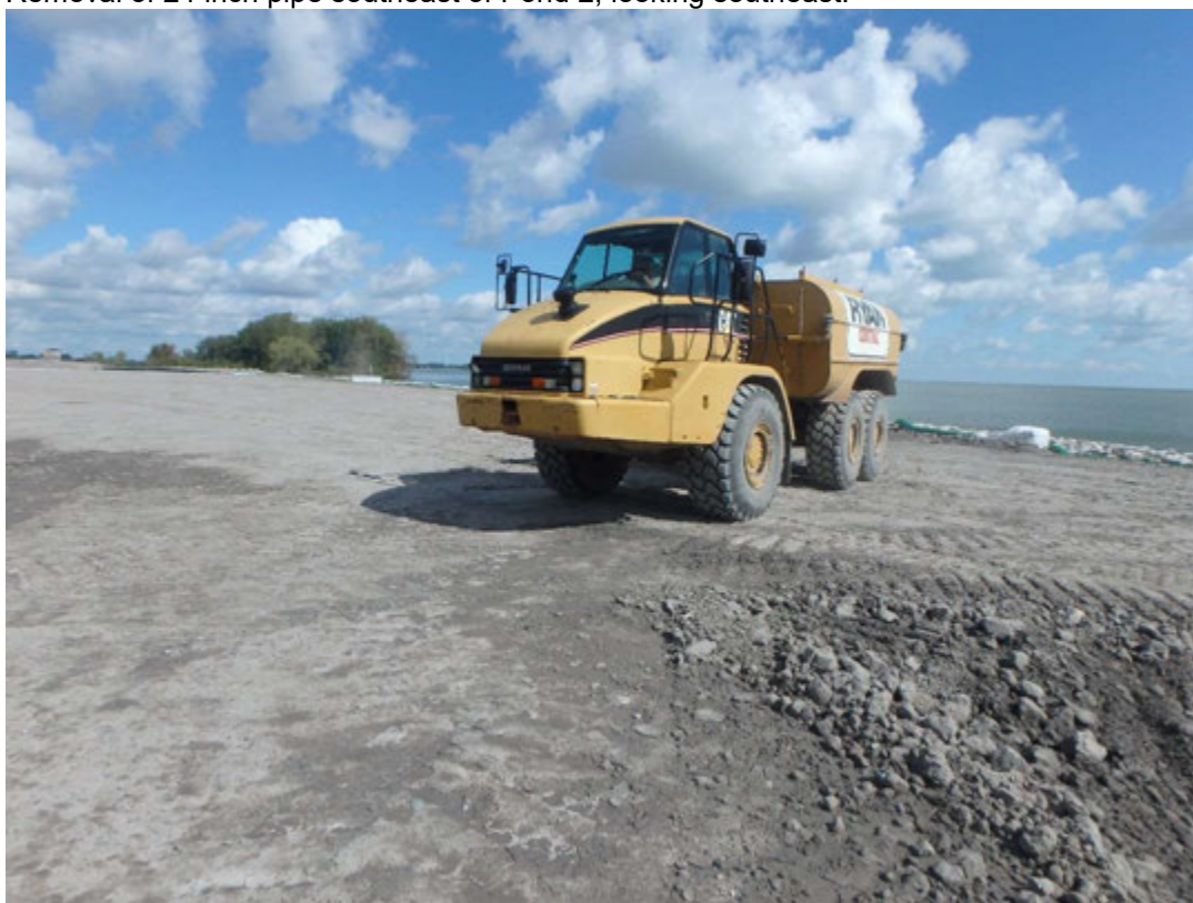
Proof roll of bridging layer in southeast corner of Pond 2, looking northeast.
