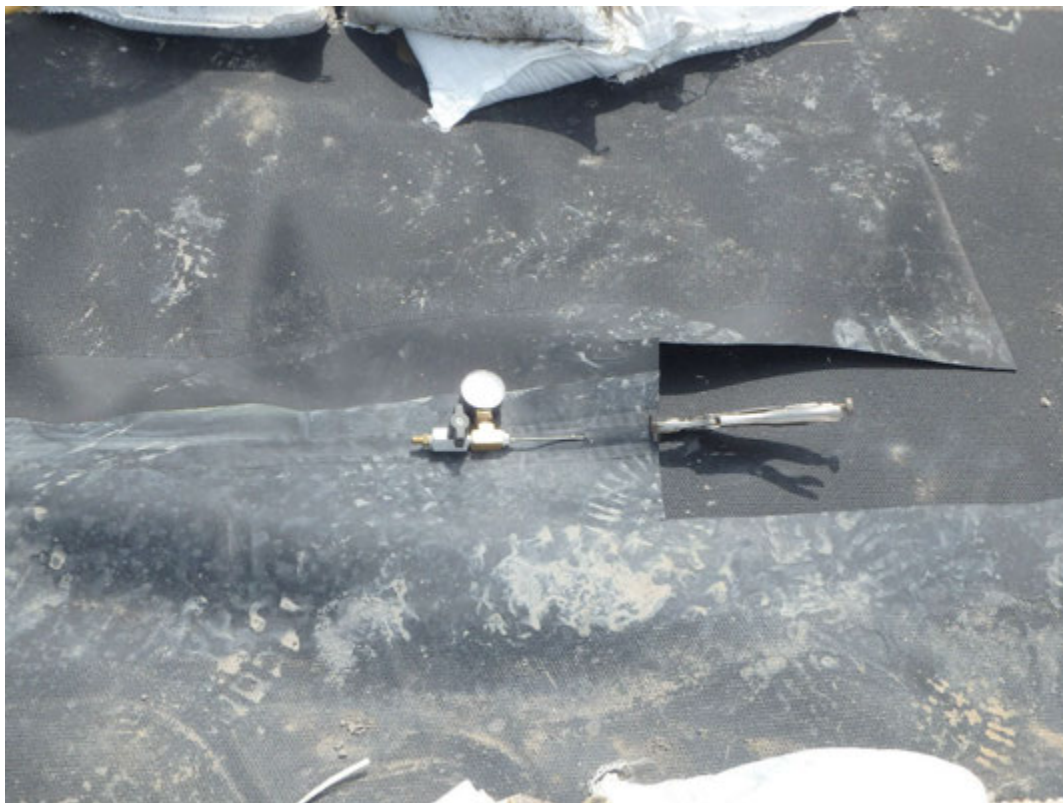
Pressure testing of fusion seam.
