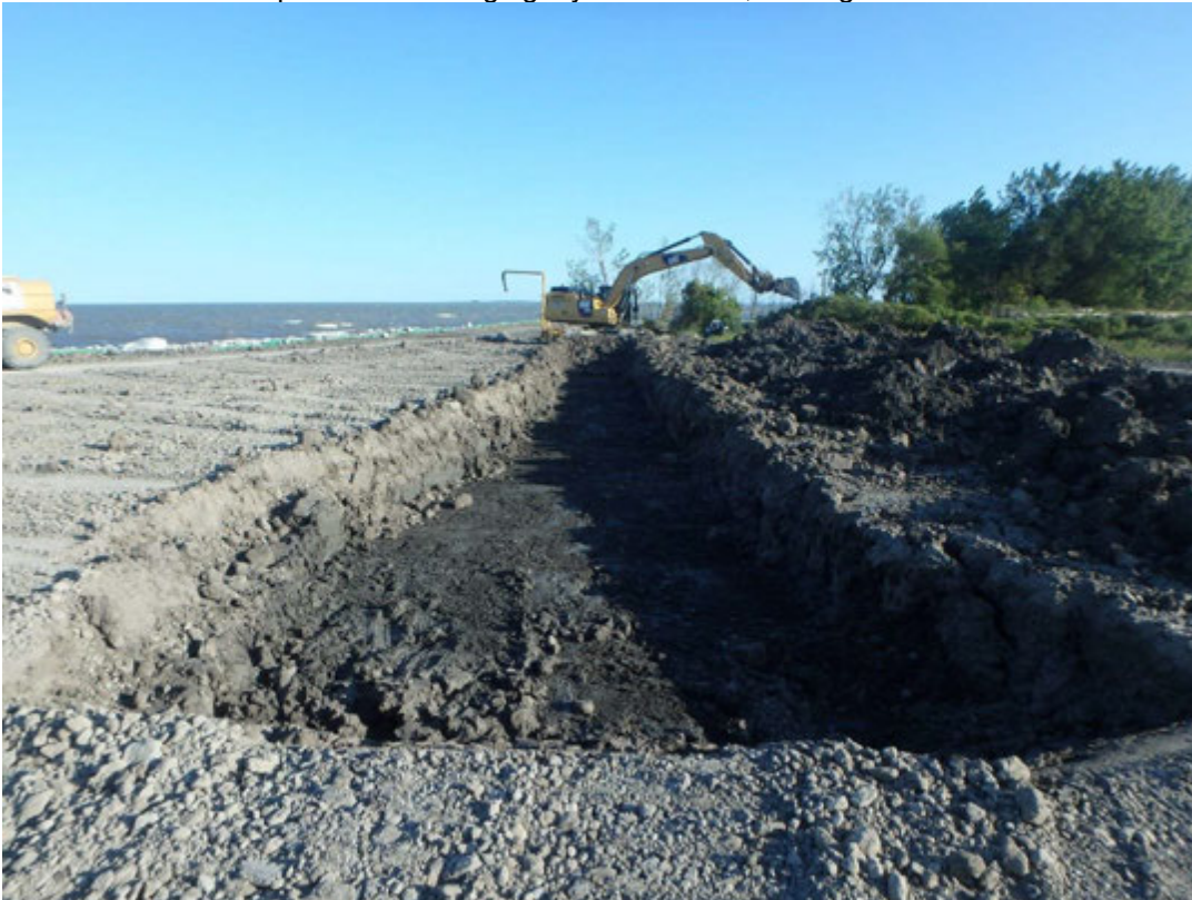
Excavating area of bridging layer in Pond 2 that failed proof roll, looking southeast.
