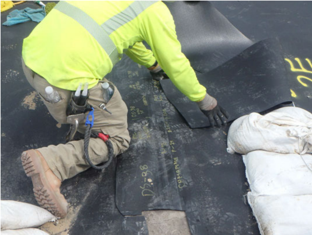
Removing marked destruct for field testing.
