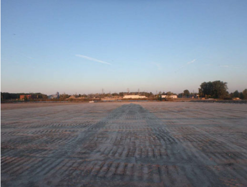
Overview of Pond 2's geomembrane sub-grade ready for survey, looking west.
