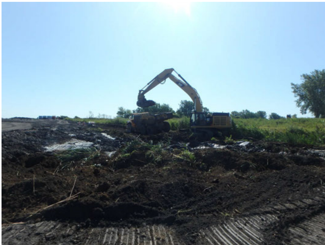
Excavating CCR from area between Pond 2's southwest corner and Fore Bay, looking south.
