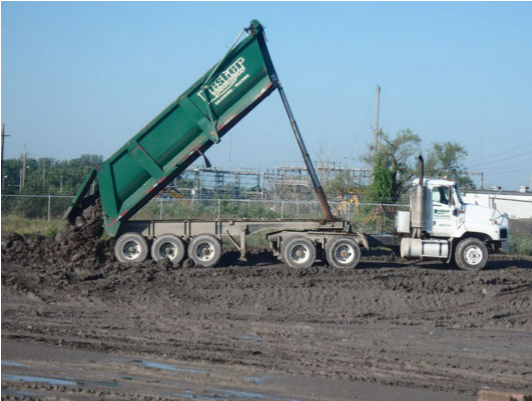
Structural fill import, looking southwest.
