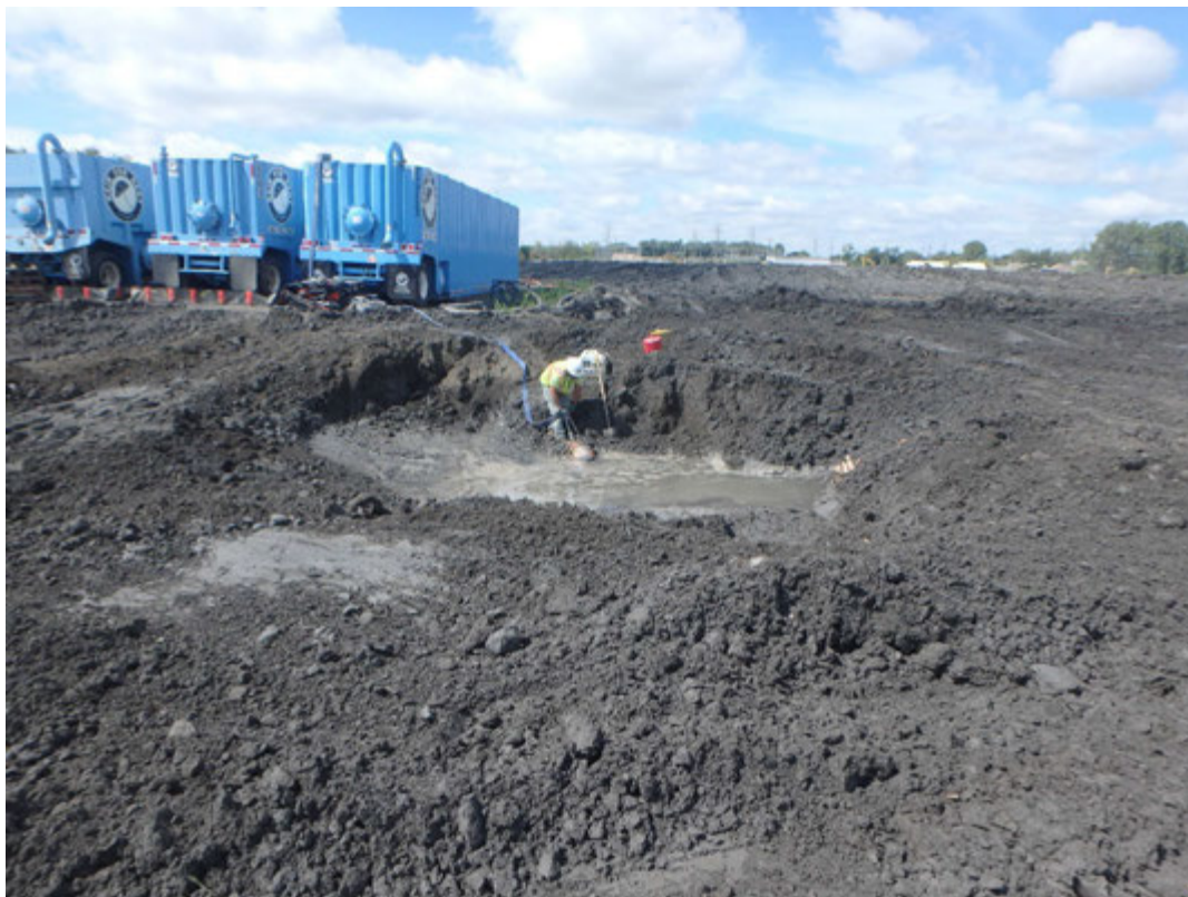
Pumping standing water from southeast corner of Pond 2 into baker tank, looking west.
