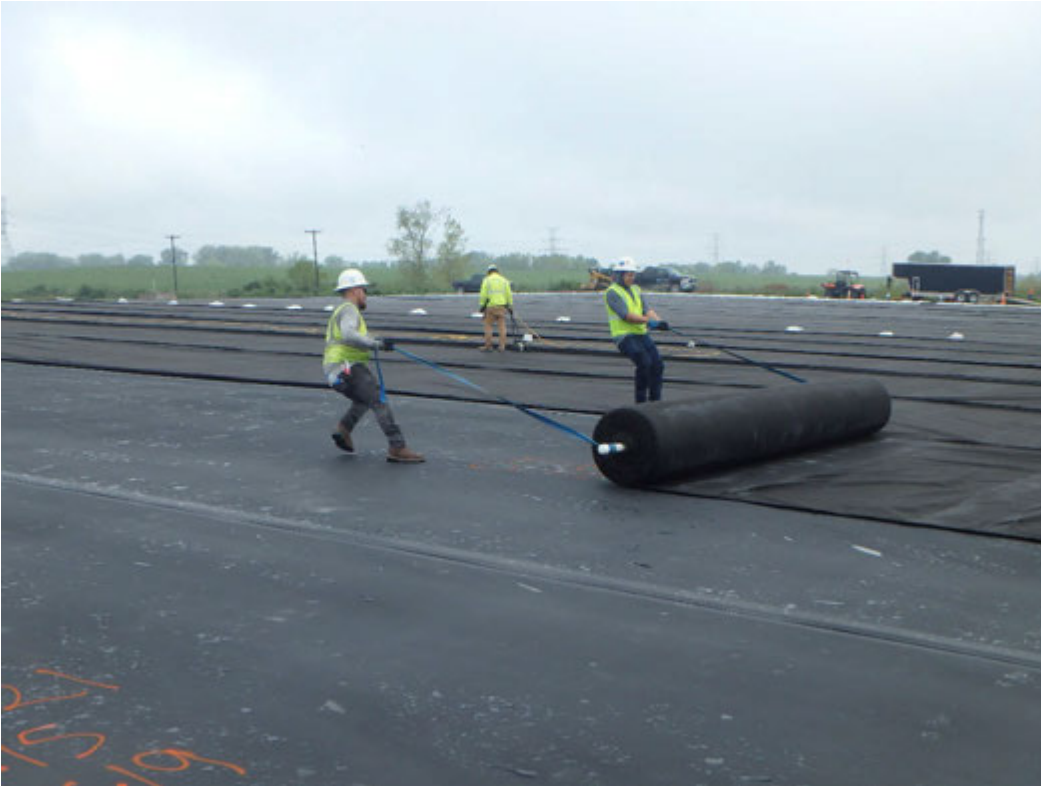
Deployment of geotextile in Pond 1, looking northwest.
