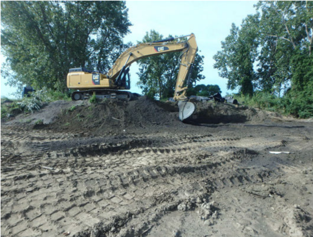
Removal of CCR from area west of chemical ponds, looking south.
