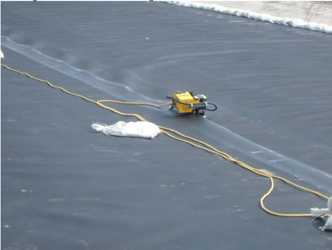
Seaming of geomembrane panels by fusion method.
