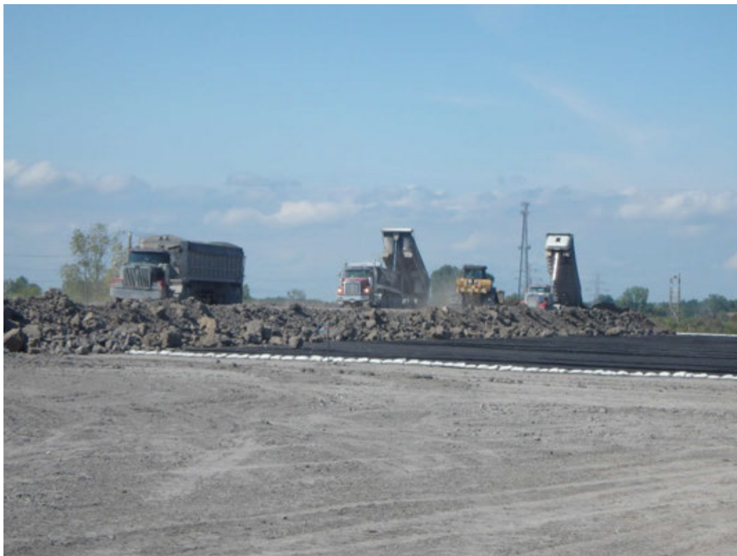
Import of protective cover to Pond 1, looking north.
