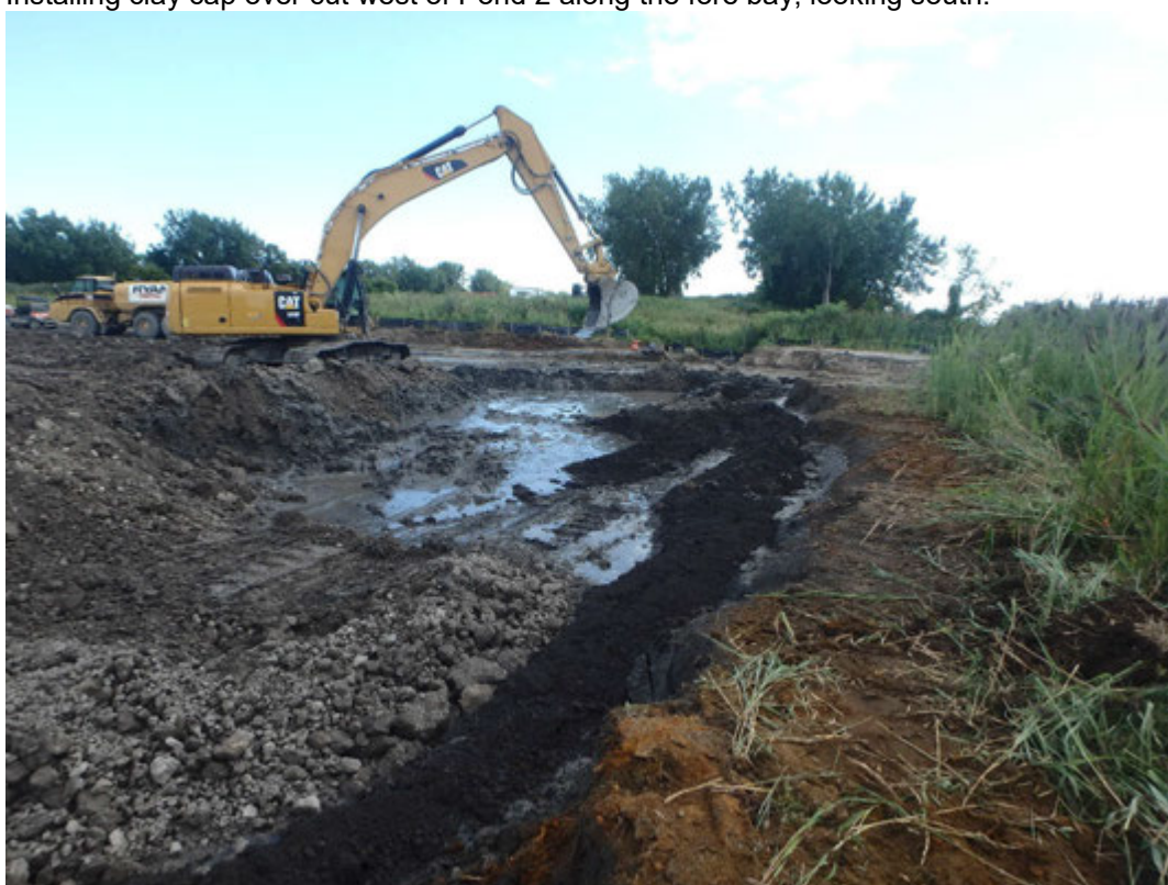
Excavating along fore bay west of Pond 2, looking south.
