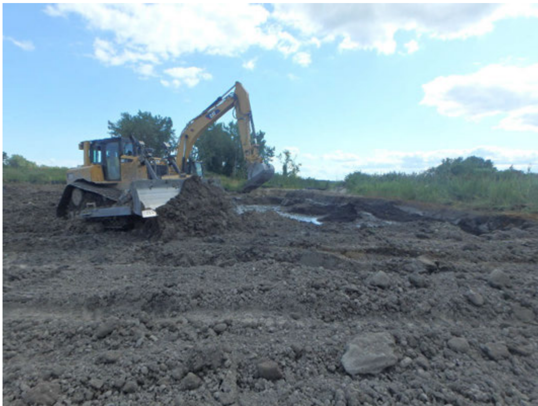
Installing clay cap over cut west of Pond 2 along the fore bay, looking south.
