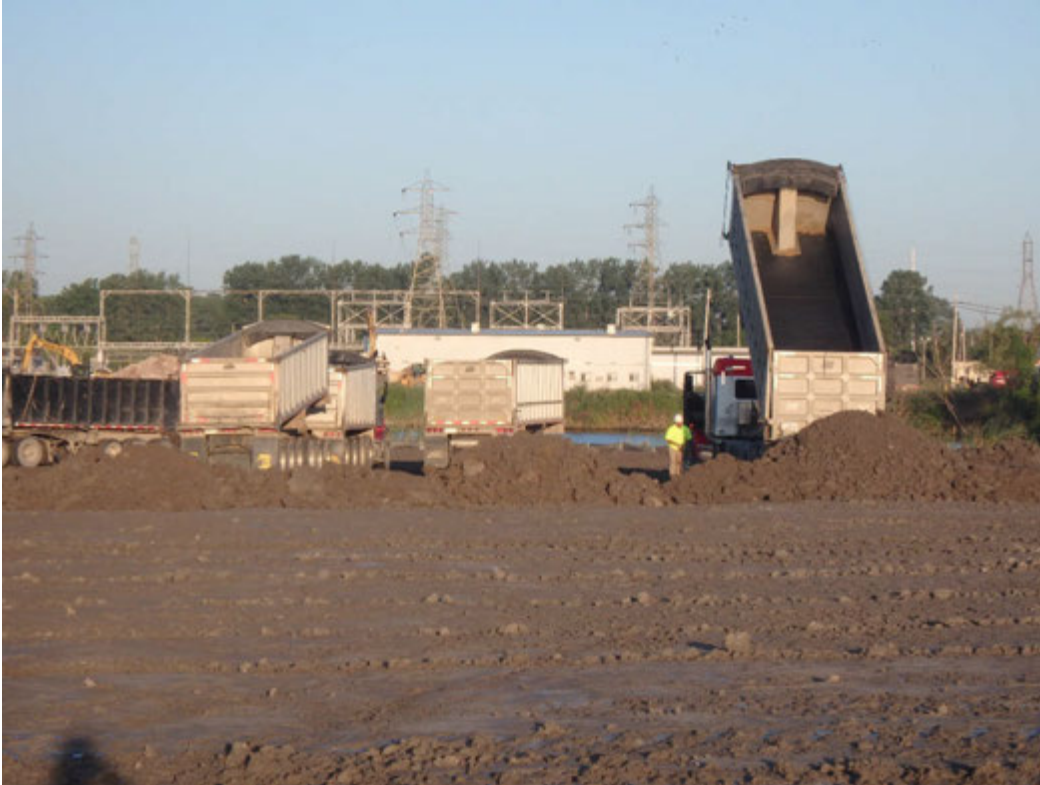
Structural fill import to Pond 2.
