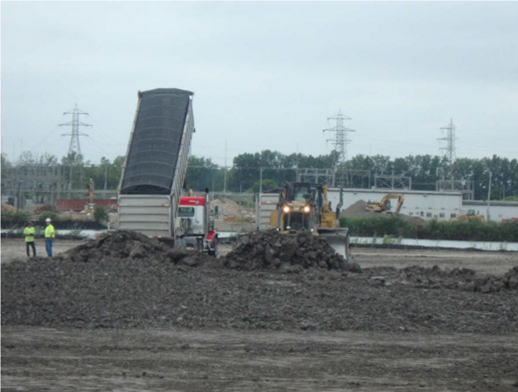
Placing lift of structural fill in Pond 2.
