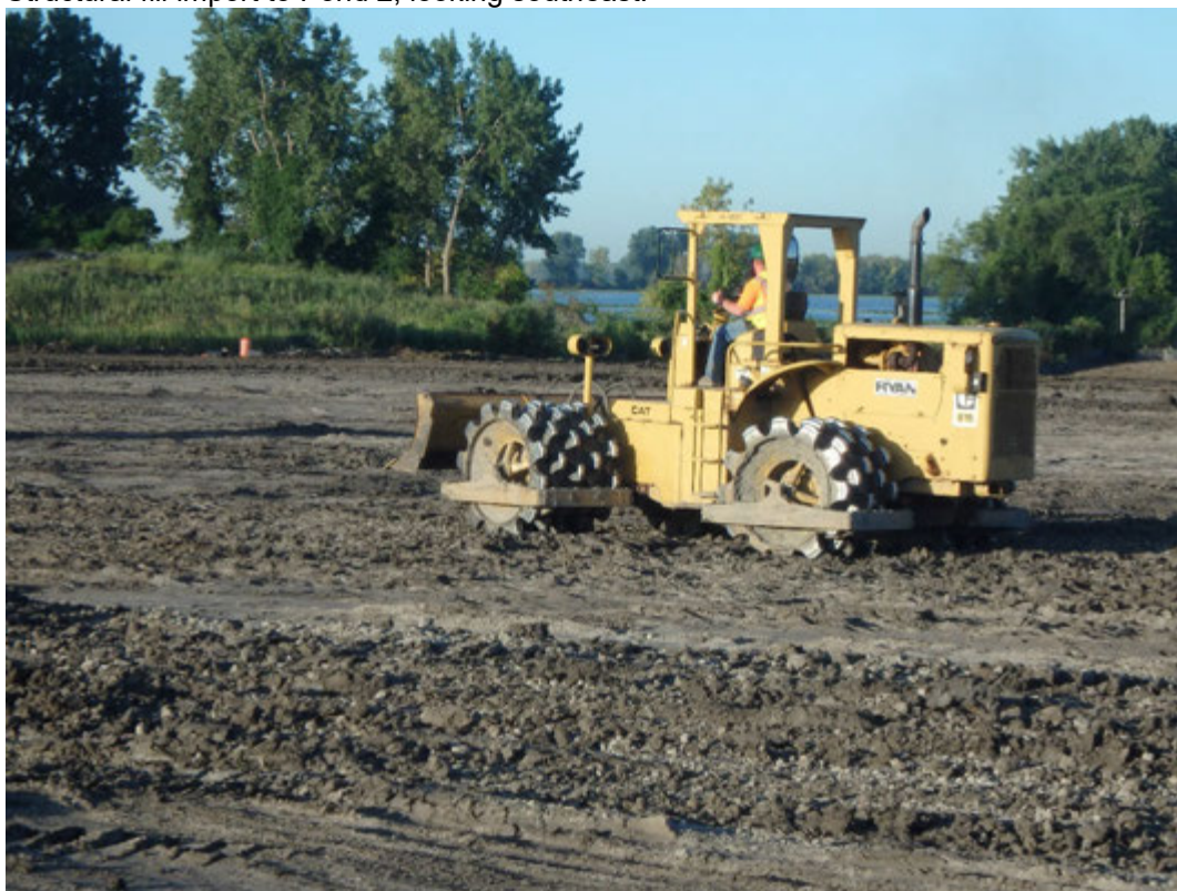
Compaction of structural fill lift in Pond 2, looking southwest.
