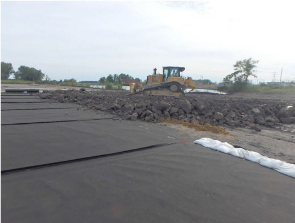
Placement of protective cover in Pond 1, looking southwest.
