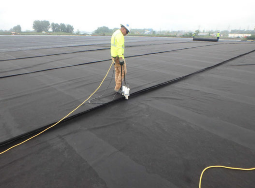
Sewing of geotextile panel seam, looking southwest.
