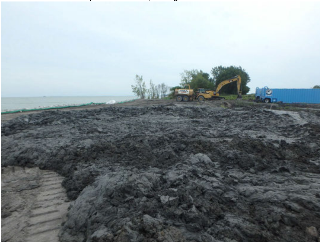
Saturated CCR removed from southeast corner of Pond 2, looking southeast.
