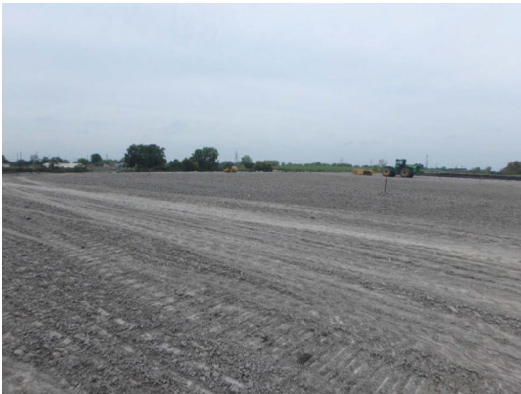
Overview of structural fill placed in Pond 2, looking northwest.
