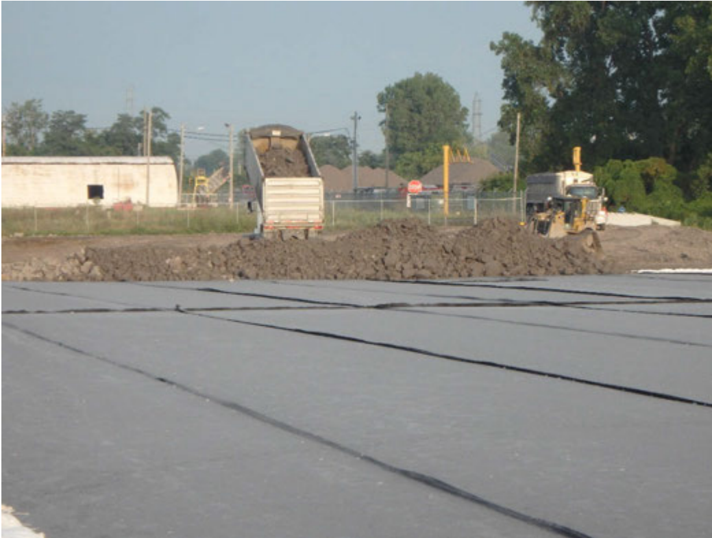
Placement of protective cover over Pond 1 geosynthetics, looking west.
