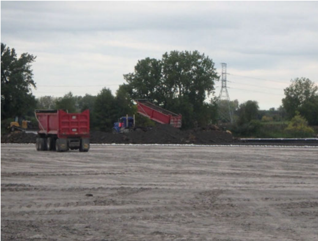
Protective cover import to Pond 1, looking northwest.
