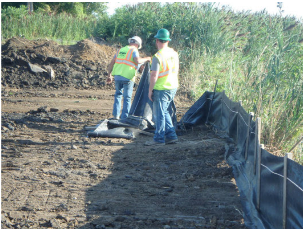
Installing silt fence west of excavation along fore bay, looking south.
