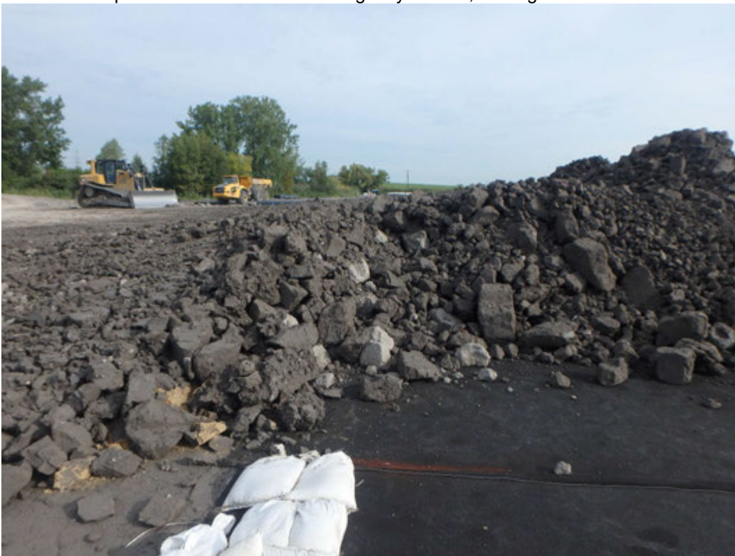
Ramp built using protective cover over Pond 1 geosynthetics, looking north.
