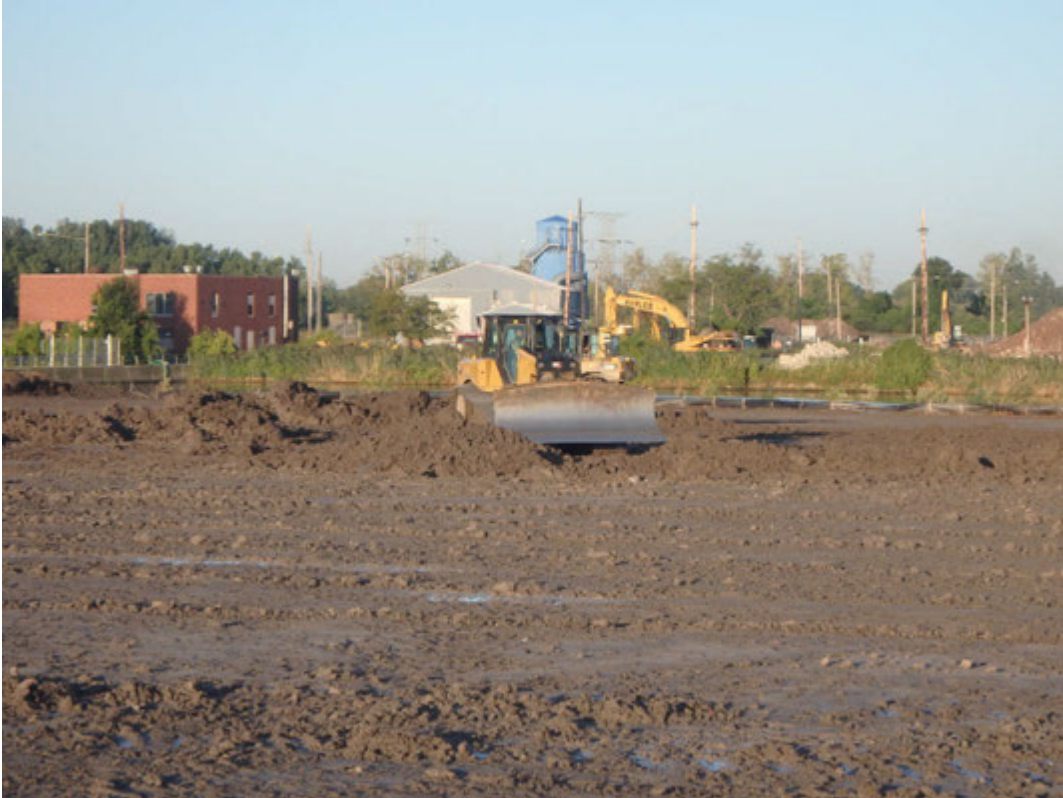
Placing structural fill in Pond 2, looking west.
