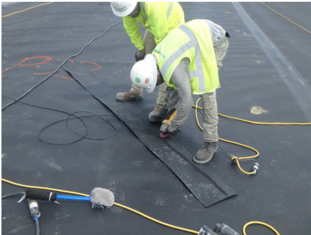
Preparing trial weld.
