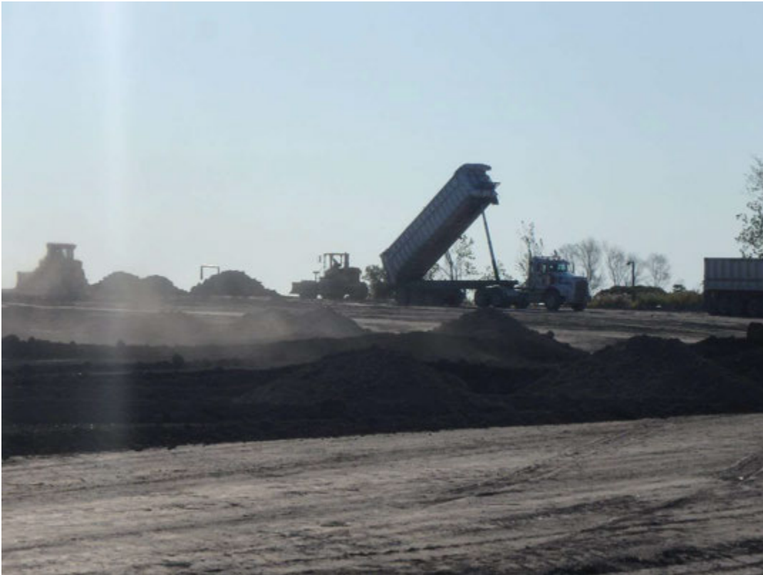
Import of structural fill to Pond 2, looking southeast.
