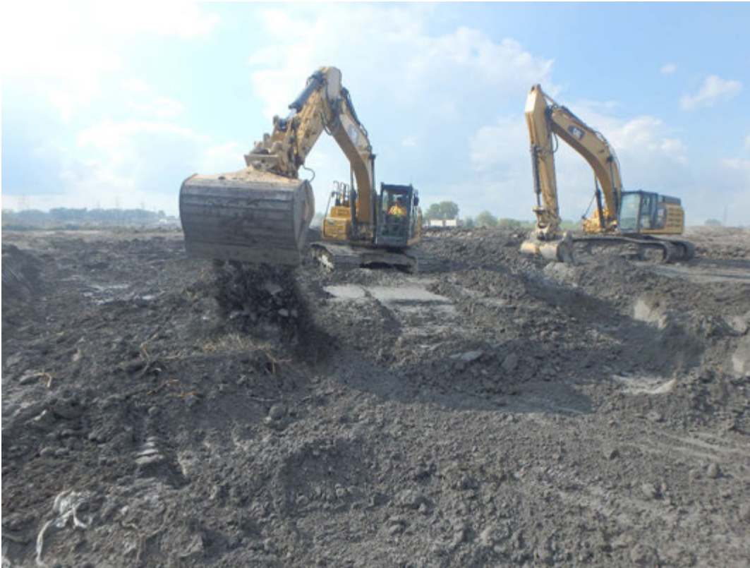
Placing CCR in sump area of Pond 2 for bridging layer, looking northwest.
