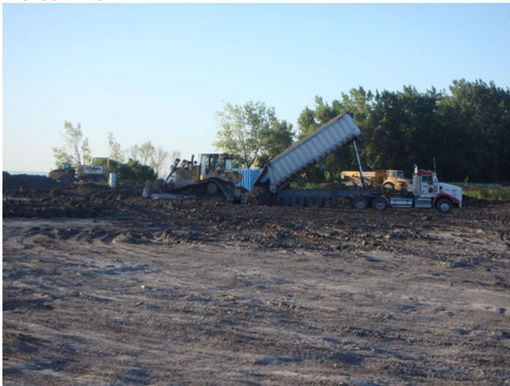
Structural fill import to Pond 2, looking southeast.
