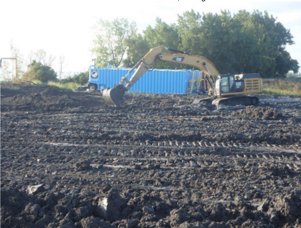
Removing saturated CCR from southeast corner of Pond 2, looking south.
