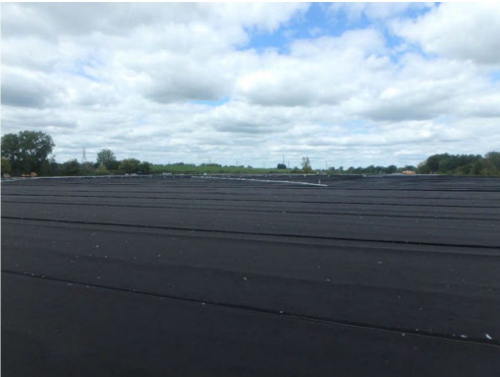
Overview of Pond 1 with above-cap drain pipe, looking north.
