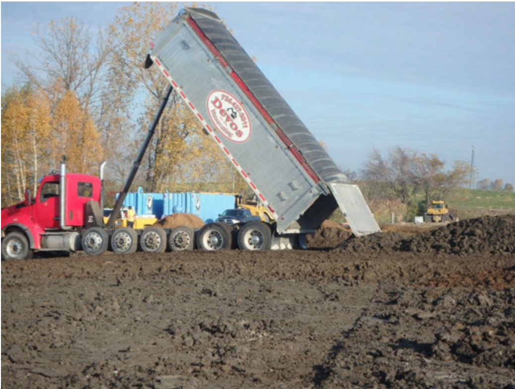
Import of topsoil to Pond 1, looking north
