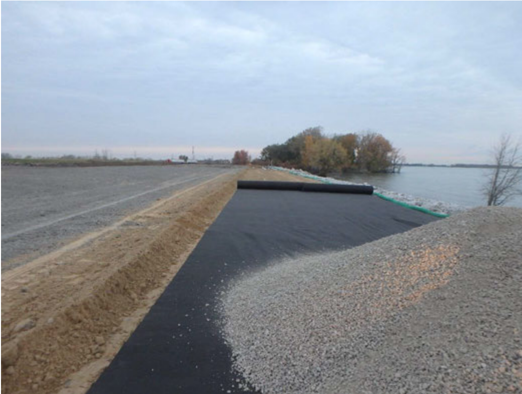
East access road, looking north
