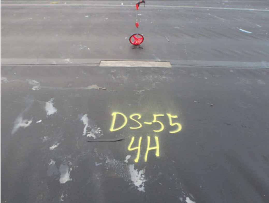
Destructive sample removed for field and lab testing
