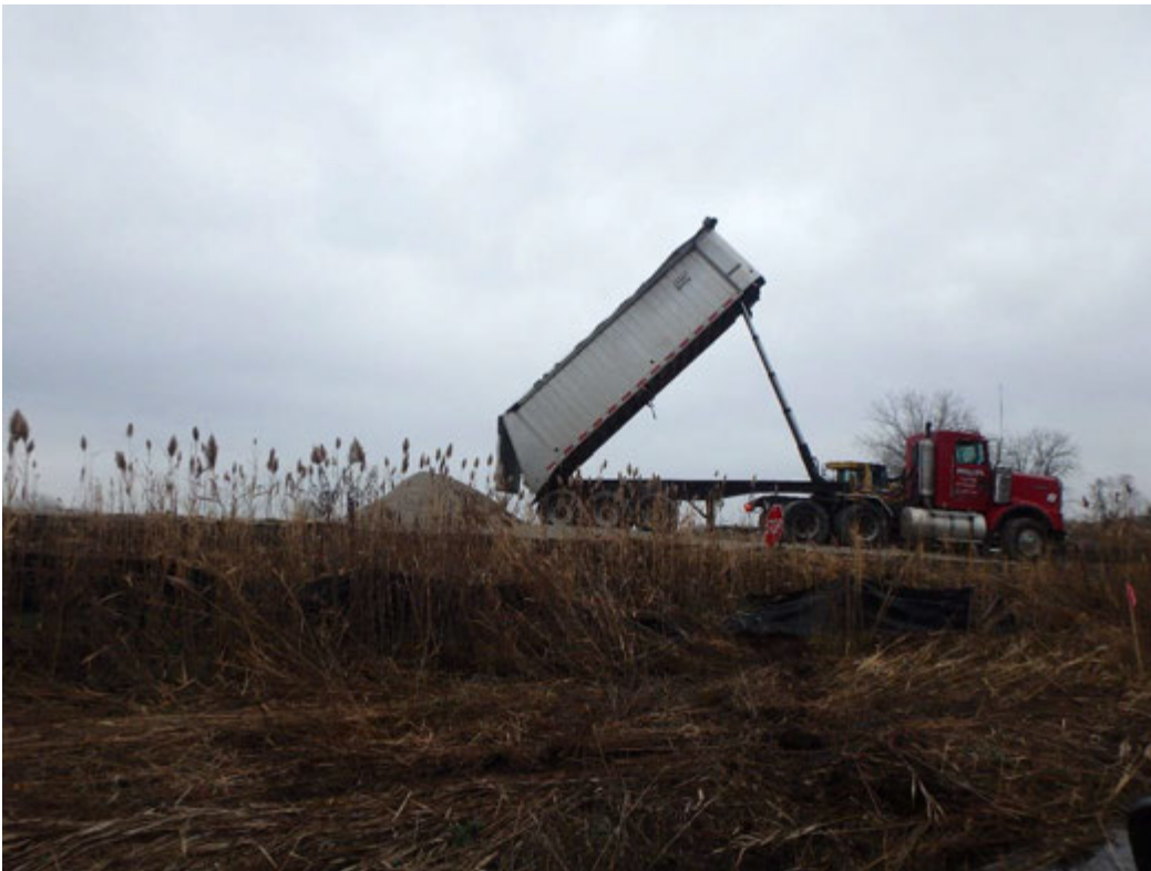
Import of 23AA for shoulder of asphalt access ramp, looking south
