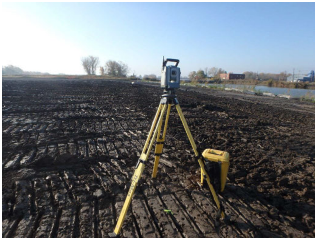
Rowe set-up for survey of protective cover, looking south
