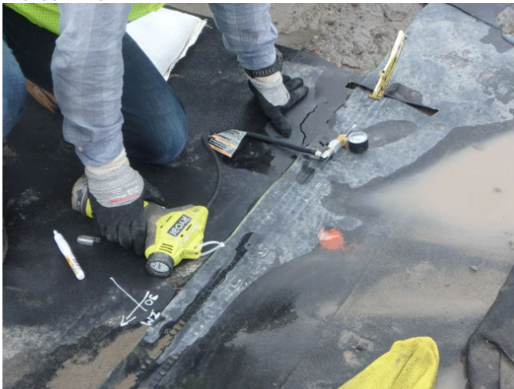
Air pressure testing of fusion seam.
