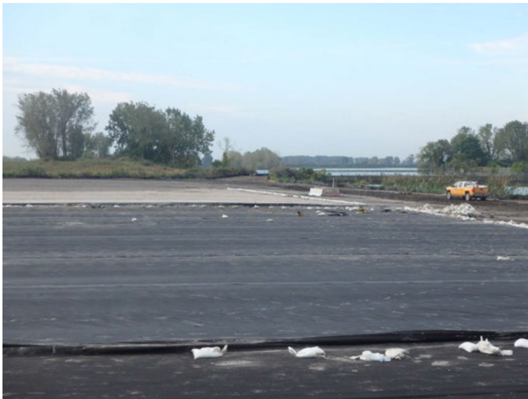
Overview of geosynthetics in Pond 2, looking south
