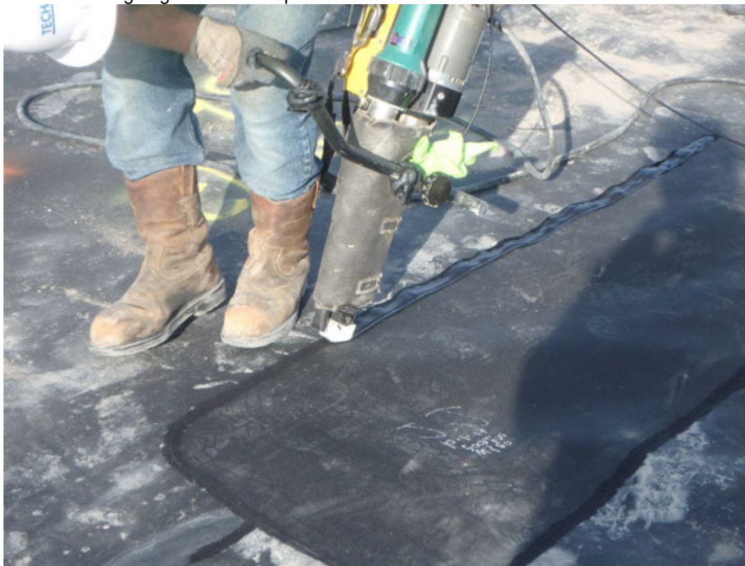
Repair using extrusion method.
