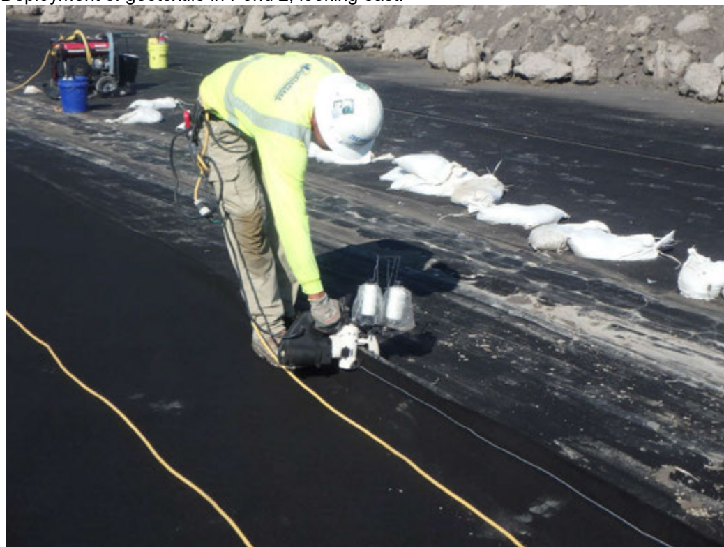
Sewing of geotextile panels.
