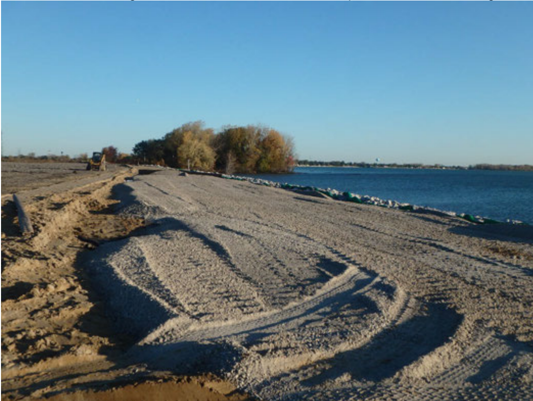
Road base placed for east access road, looking north
