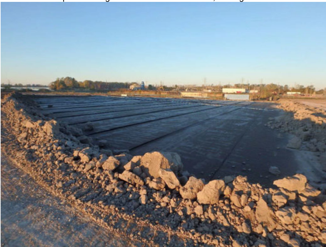
Overview of protective cover in Pond 2, looking southwest
