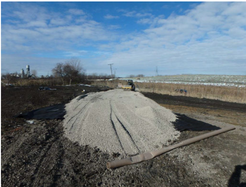
Fabric and 21AA placed for Access Ramp, looking northwest
