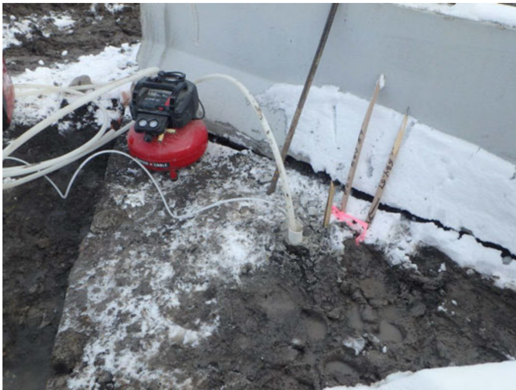
Preparing to flush MW-15006
