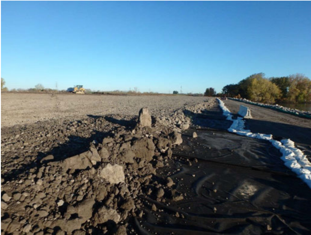
Protective cover placed along east side of Pond's 1 and 2, looking north
