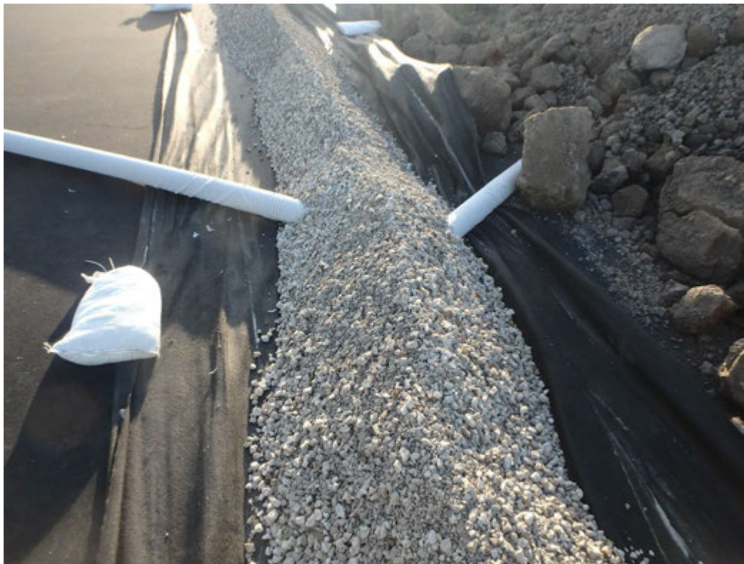
6AA placed around the solid above-cap drain pipe in Pond 1, looking east.
