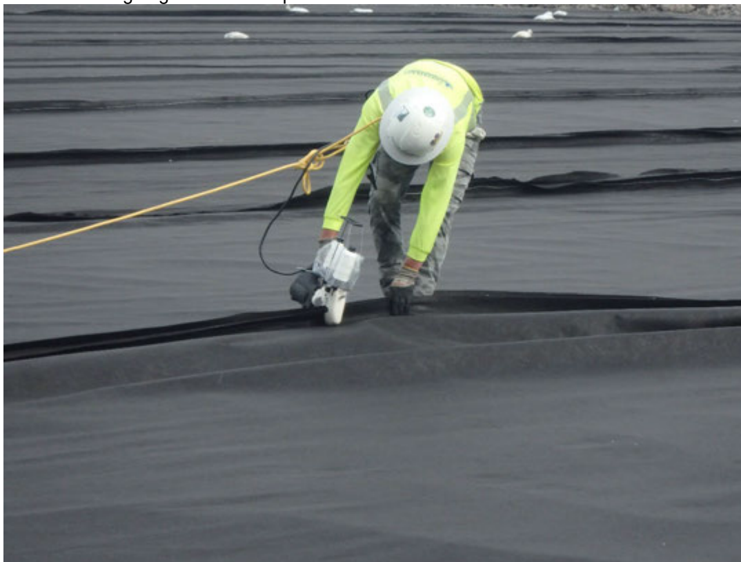
Sewing of geotextile panel seams in Pond 2.
