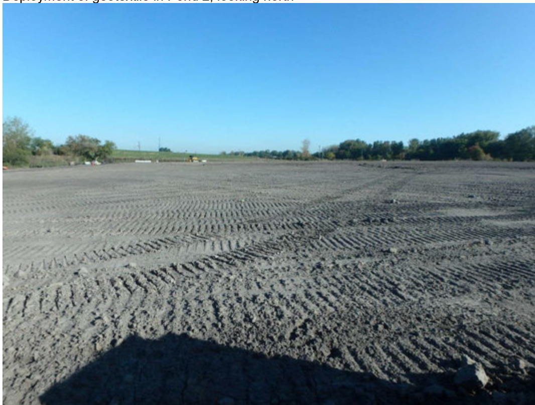
Overview of protective cover in Pond 1, looking north
