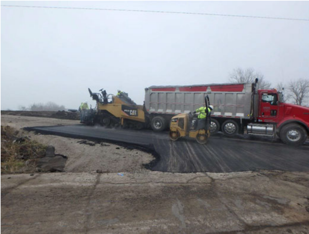
Placement and compaction of asphalt for access ramp, looking southwest
