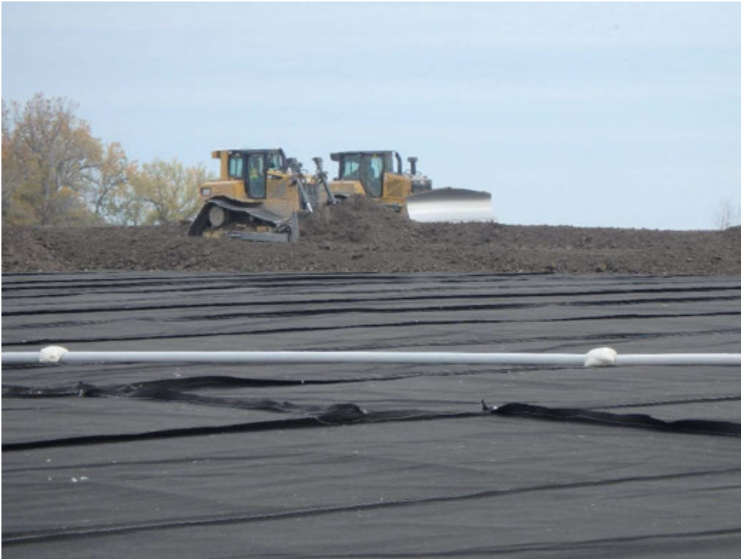
Placement of protective cover over Pond 2 geosynthetics, looking northeast
