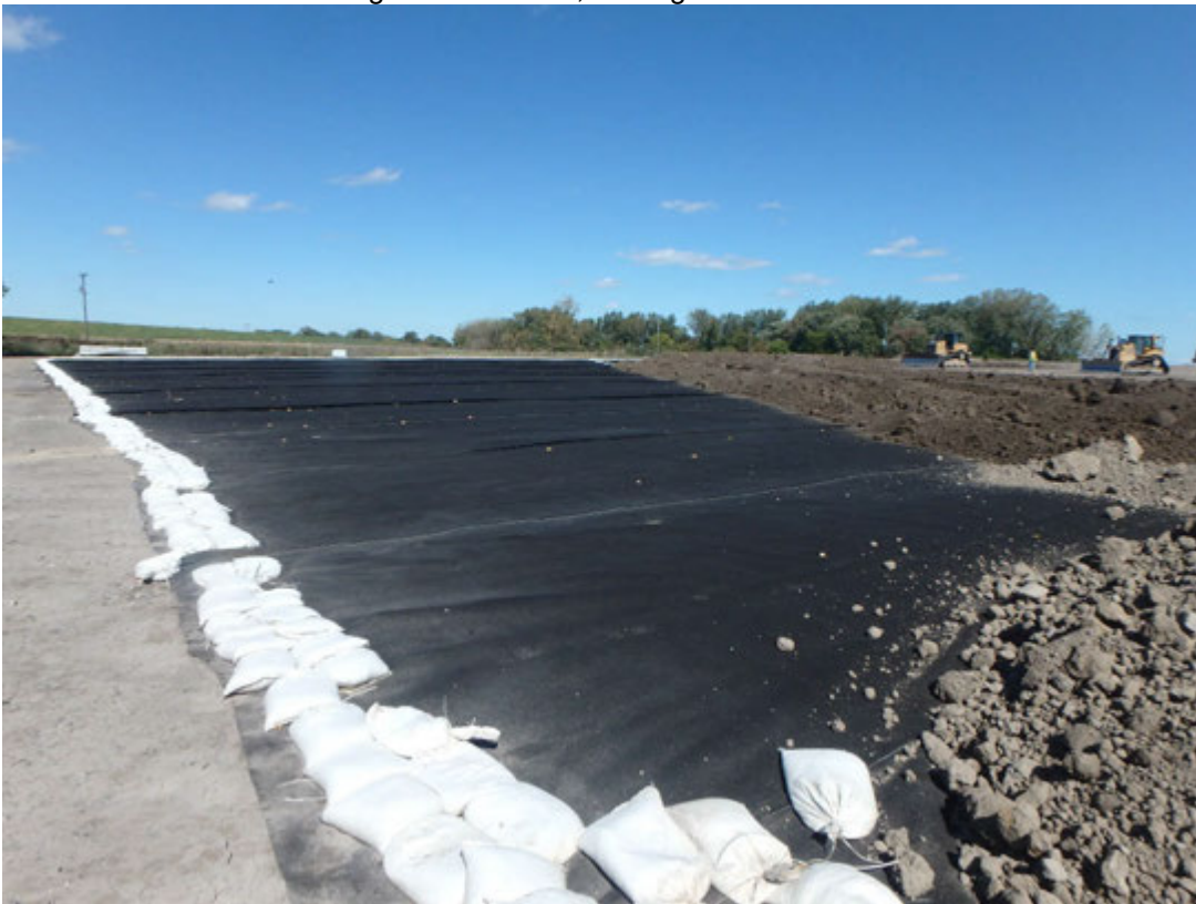
Overview of protective cover being placed in Pond 1, looking northeast.
