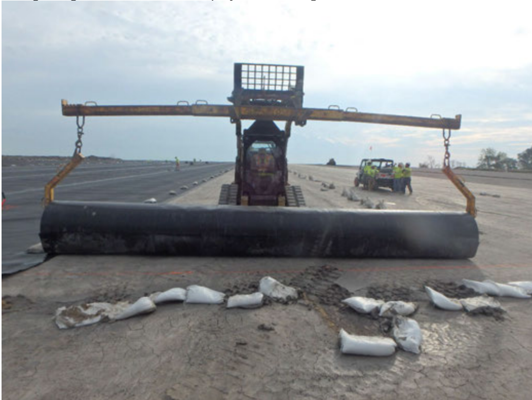
Deployment of geomembrane in Pond 2, looking east
