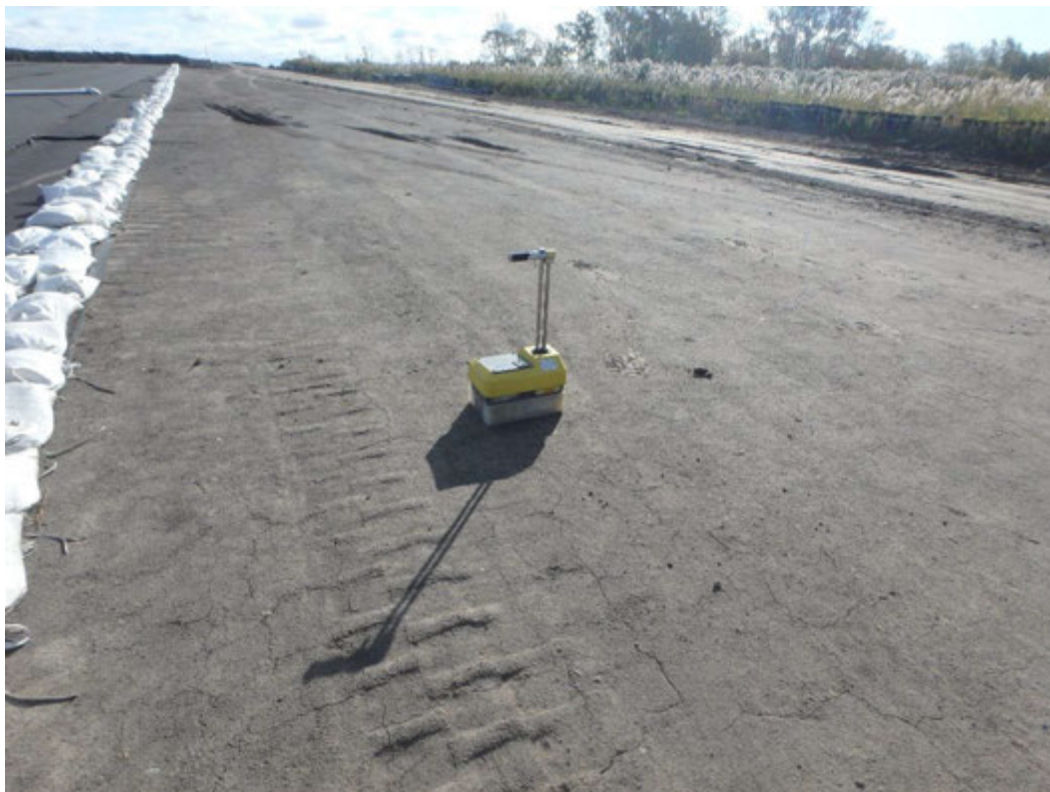
Performing standard on nuclear density gauge prior to testing, looking east
