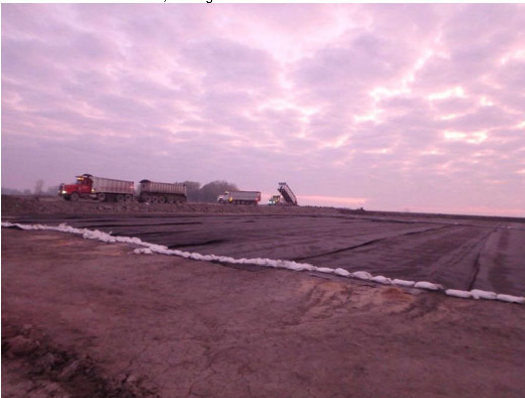
Import of protective cover to Pond 2, looking northeast
