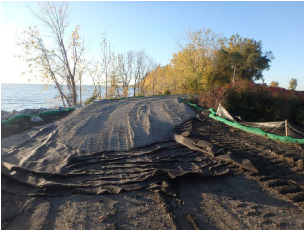
Resurfacing of access road to chemical ponds, looking south
