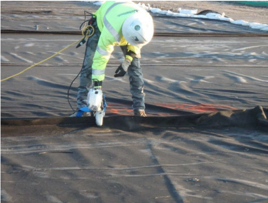
Sewing textile seam in Pond 2
