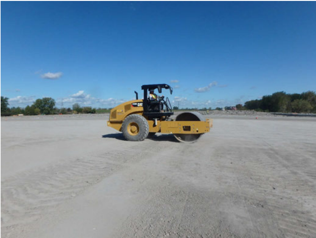
Rolling of liner sub-grade in Pond 2, looking north.
