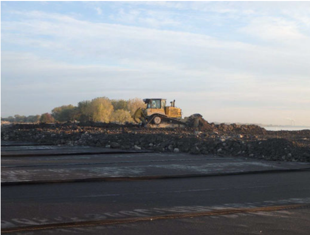
Placement of protective cover in Pond 2, looking northeast
