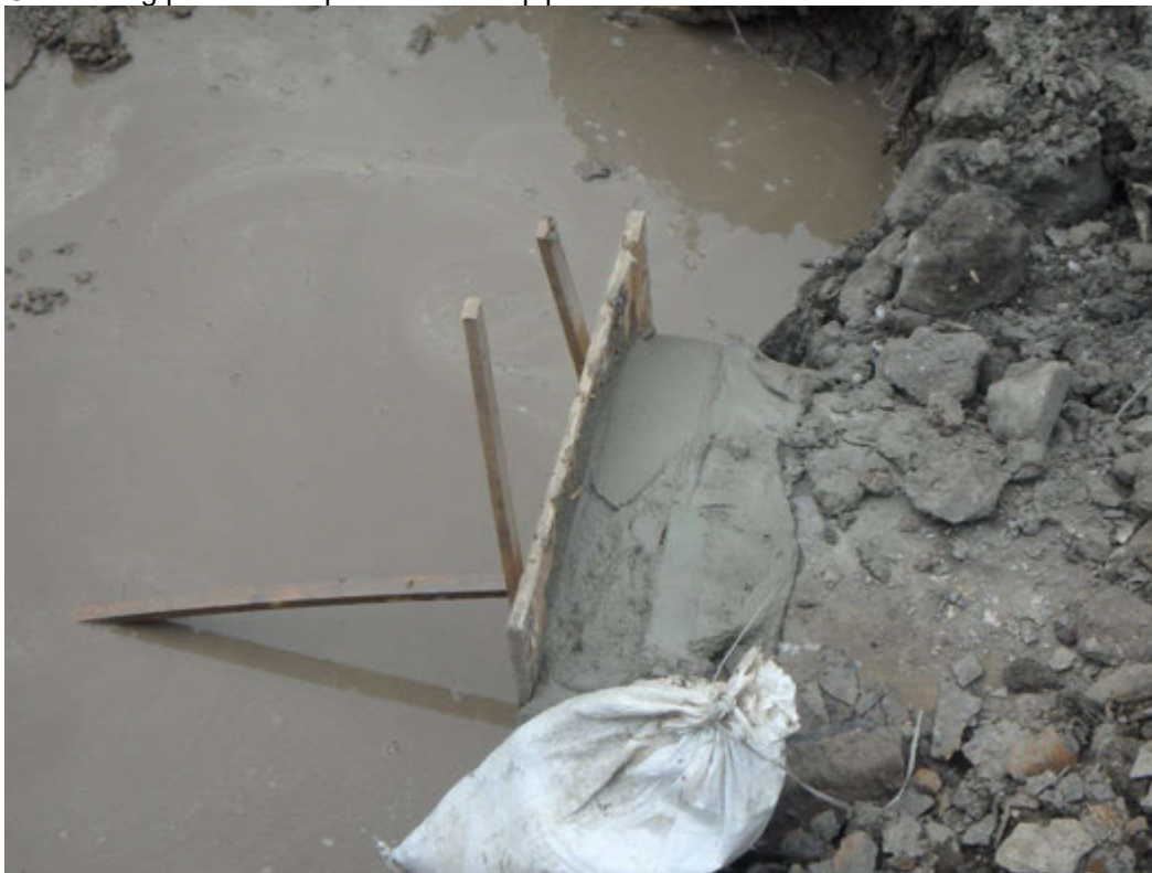
Finished 24 inch pipe cap
