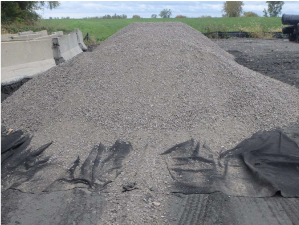
23A imported stone for access road placed atop 10 oz. textile in chemical ponds, looking south
