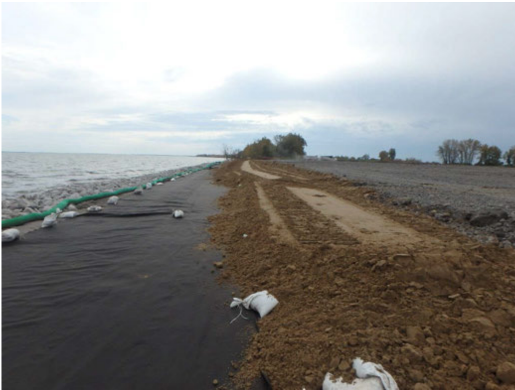
East access road sub-base, looking south
