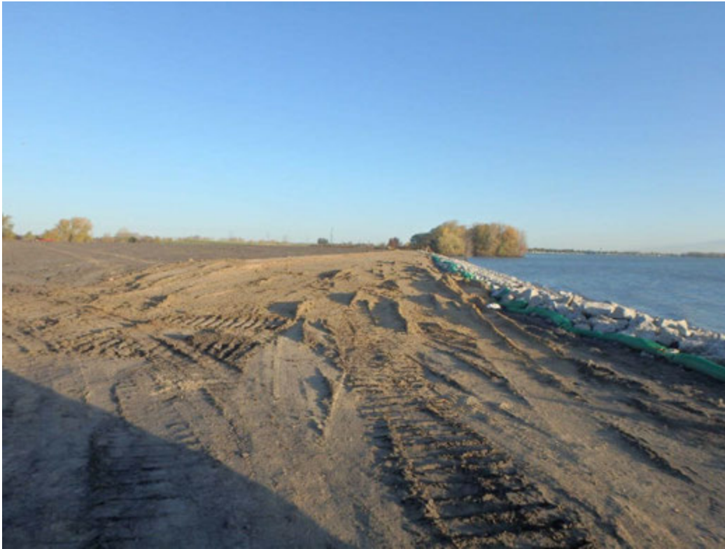
East access road sub-base, looking north
