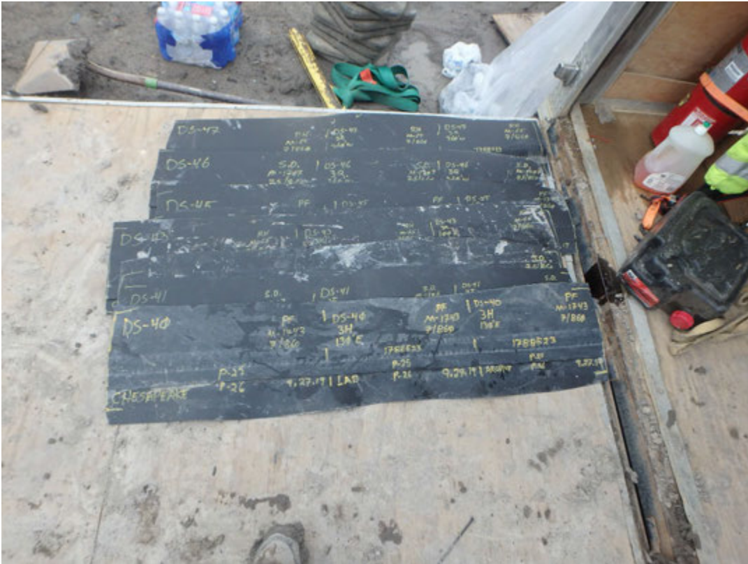
Destructive samples removed for sampling.
