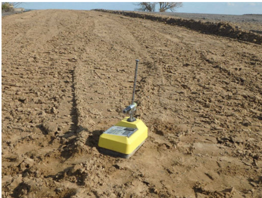
Density testing of north access road sub-base, looking east
