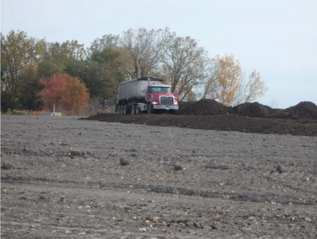
Topsoil import to Pond 1, looking northeast
