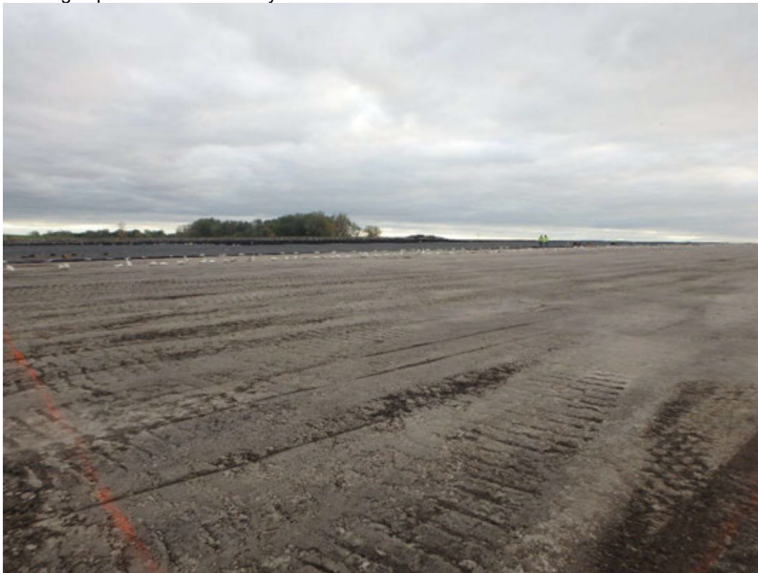
Overview of Pond 2, looking northeast
