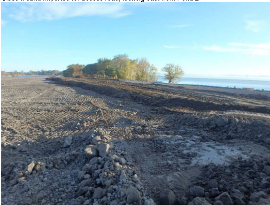
Topsoil placed in Pond 1, looking northeast
