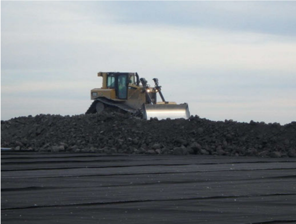
Placing protective cover in Pond 2, looking northeast
