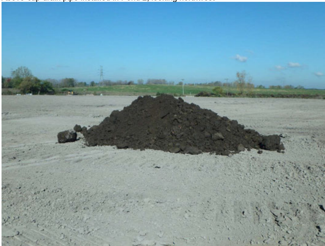
First load of topsoil received and placed in Pond 1, looking northwest
