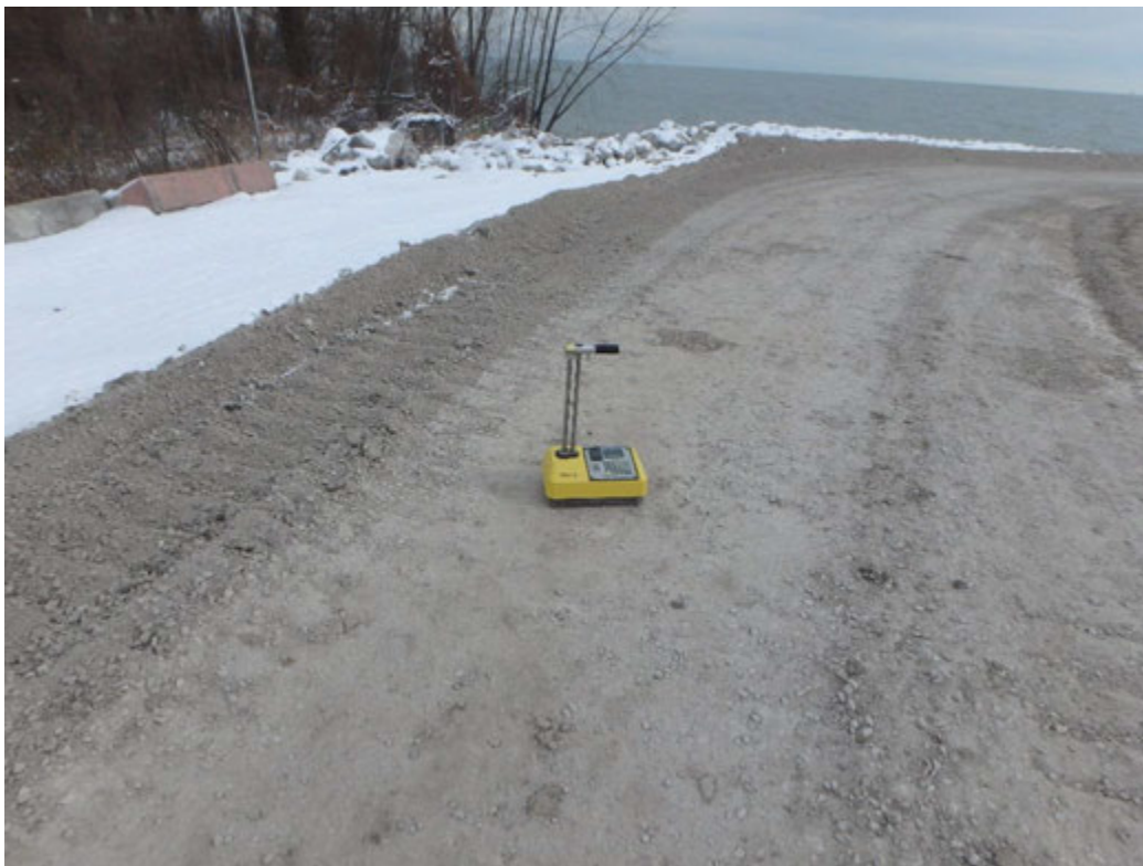
Density testing of road base material for north access road, looking east
