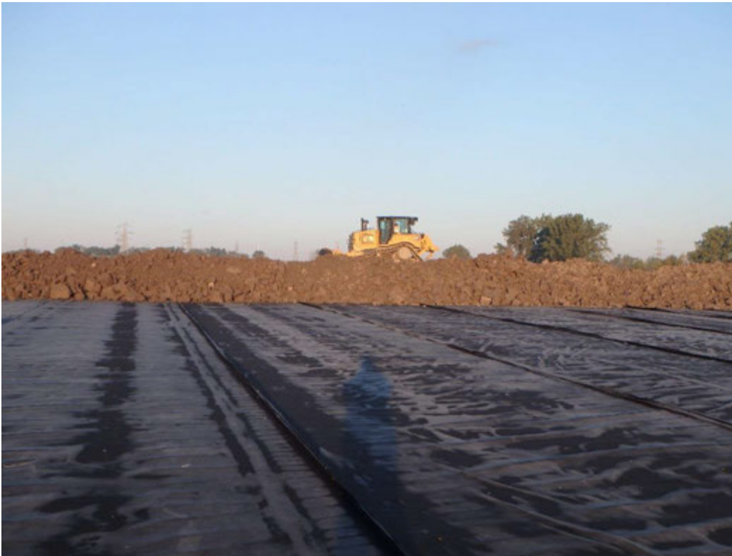
Placing protective cover in Pond 2, looking west
