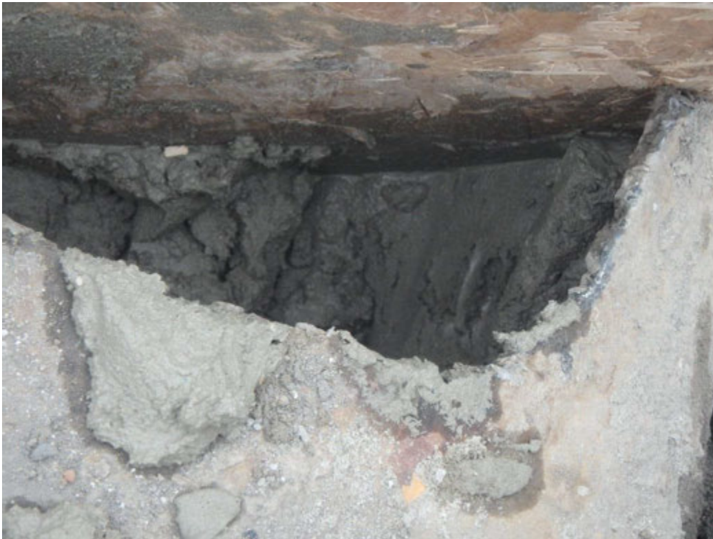
Grout being placed to cap 24 inch steel pipe
