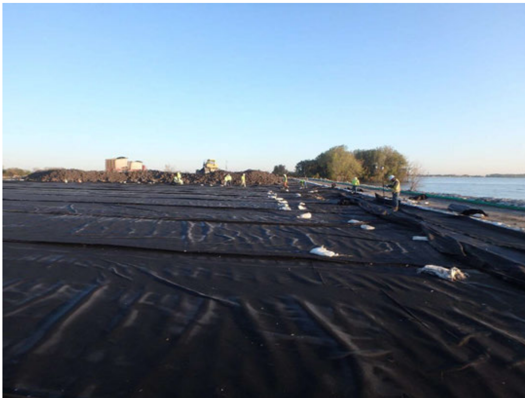
Deployment of geotextile in Pond 2, looking north
