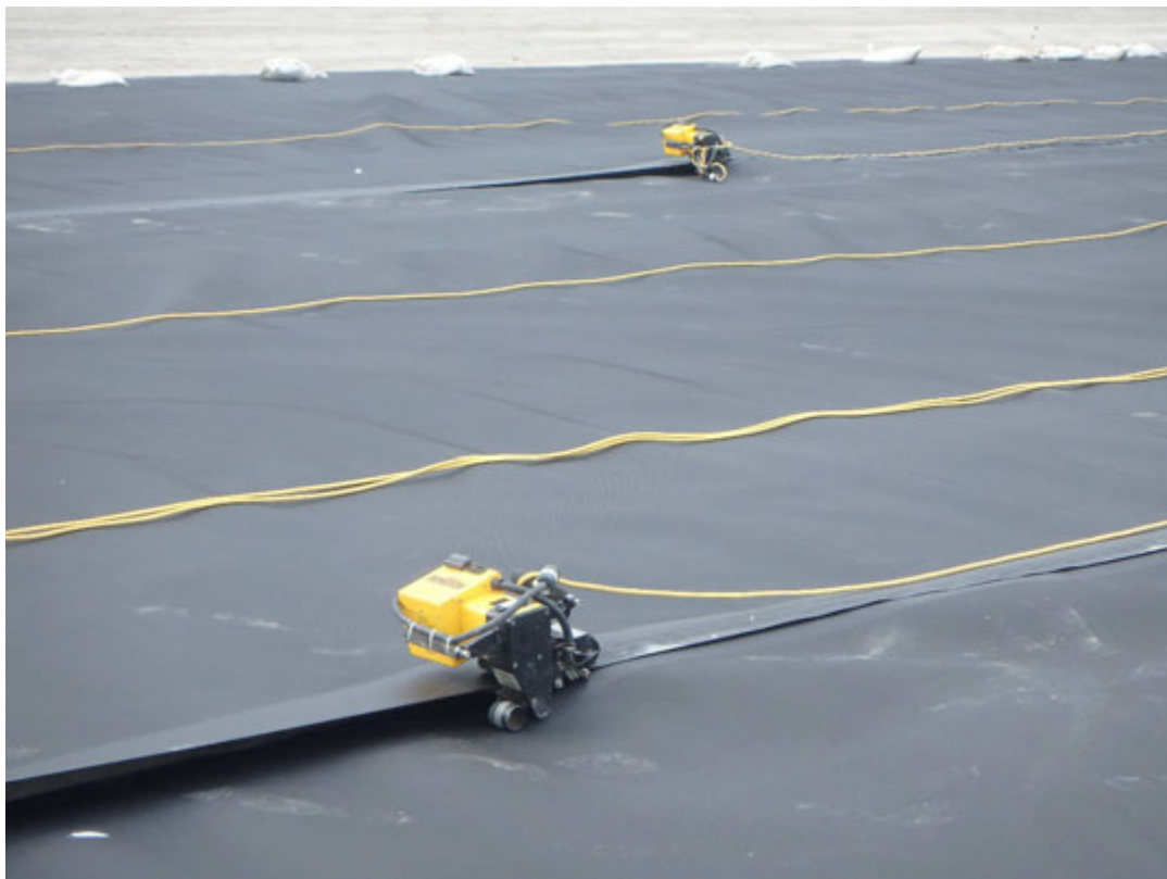
Fusion seaming of geomembrane panel seam in Pond 2.
