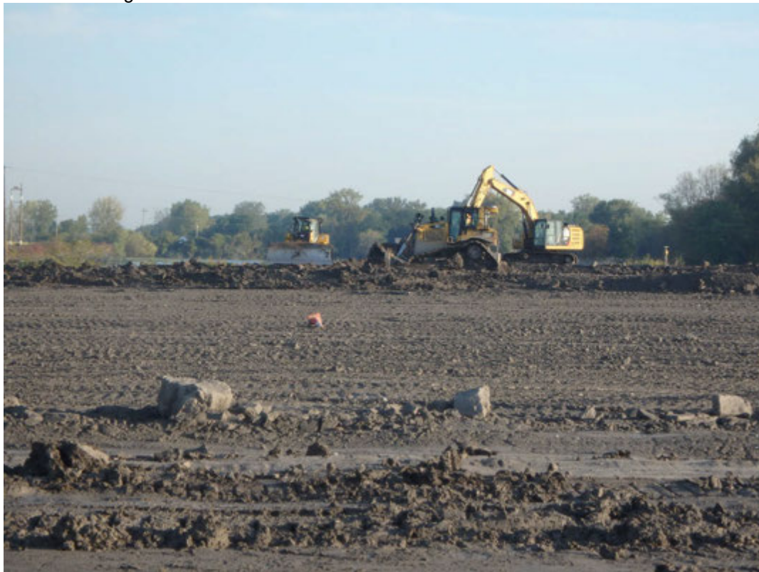
Placement of protective cover in Pond 1, looking north.
