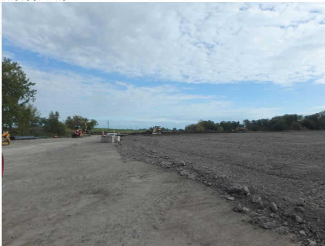
Protective cover in Pond 1, looking north.
