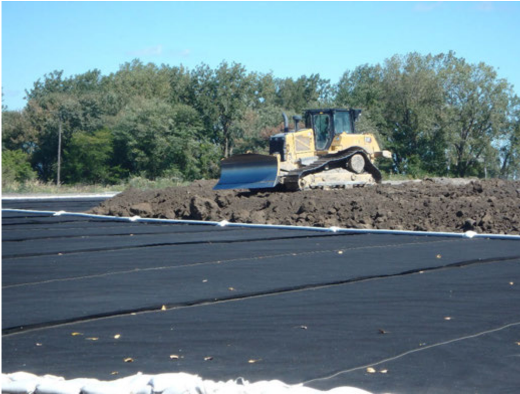
Placement of protective cover in Pond 1, looking northeast.
