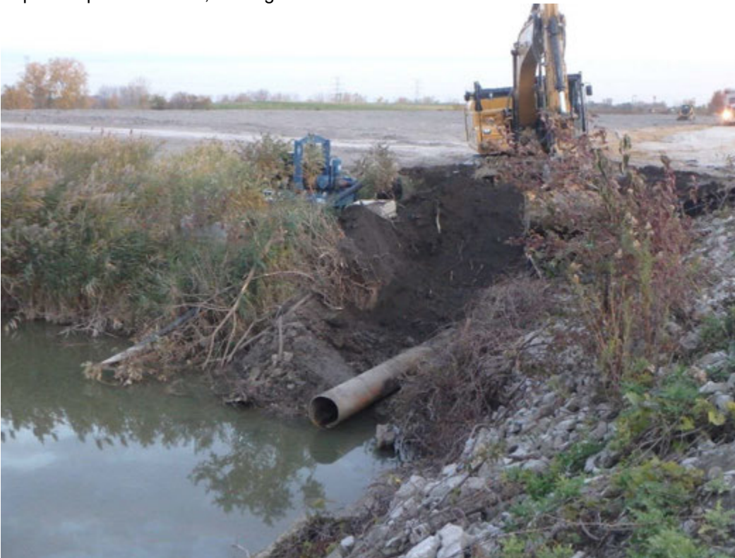
24 inch steel pipe discovered in the northeast corner of the discharge channel, looking north
