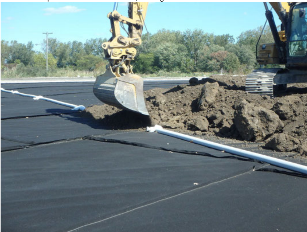
Placement of protective cover over the above-cap drain pipe in Pond 1, looking northeast.
