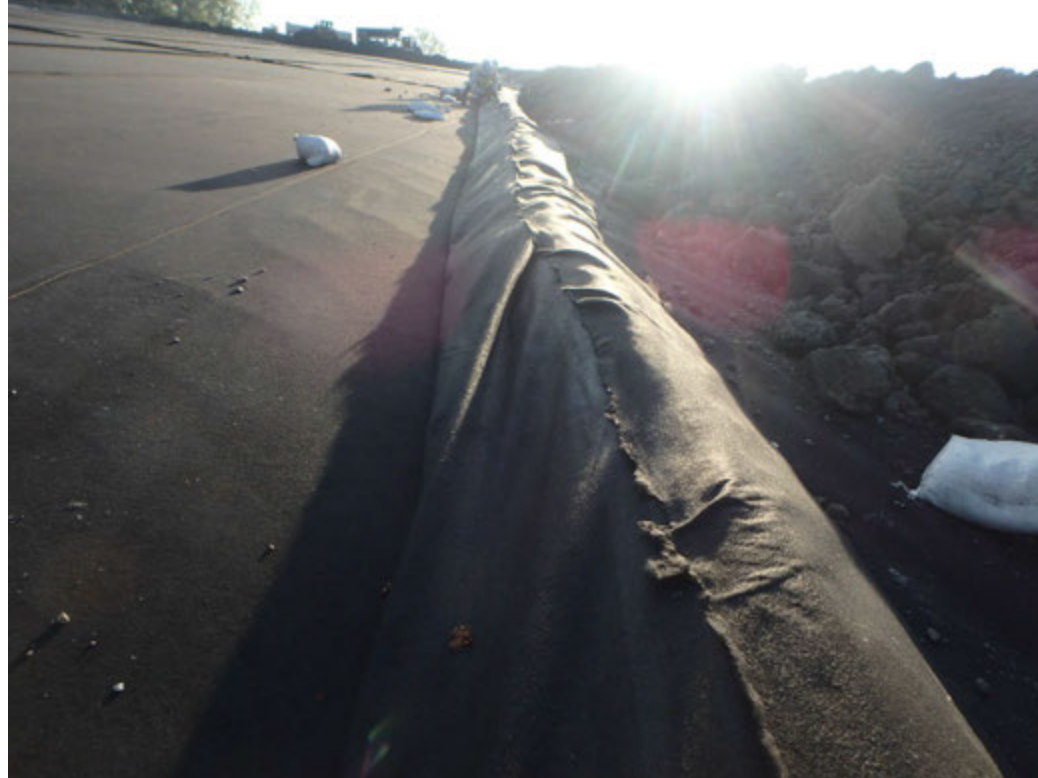
Burrito of the above-cap drain pipe stone, looking east.
