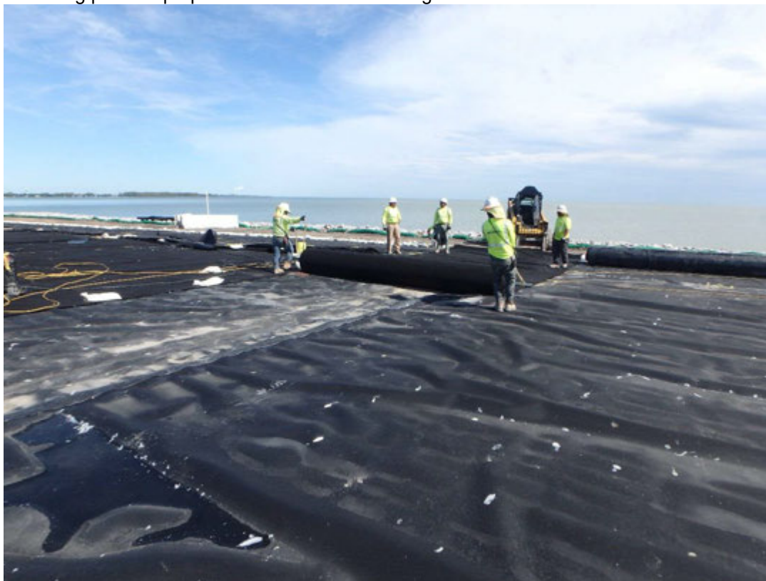
Deploying geotextile in Pond 2, looking east
