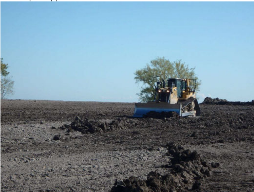
Finish grading of protective cover in Pond 1, looking east
