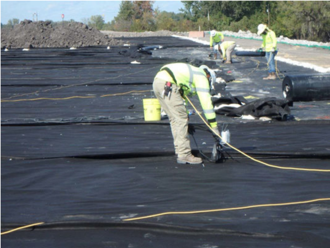
Sewing of geotextile seam in Pond 2, looking north
