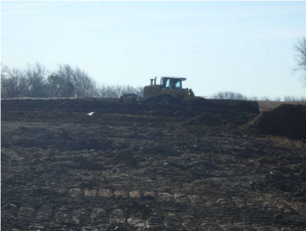
Placement of topsoil in Pond 2, looking south
