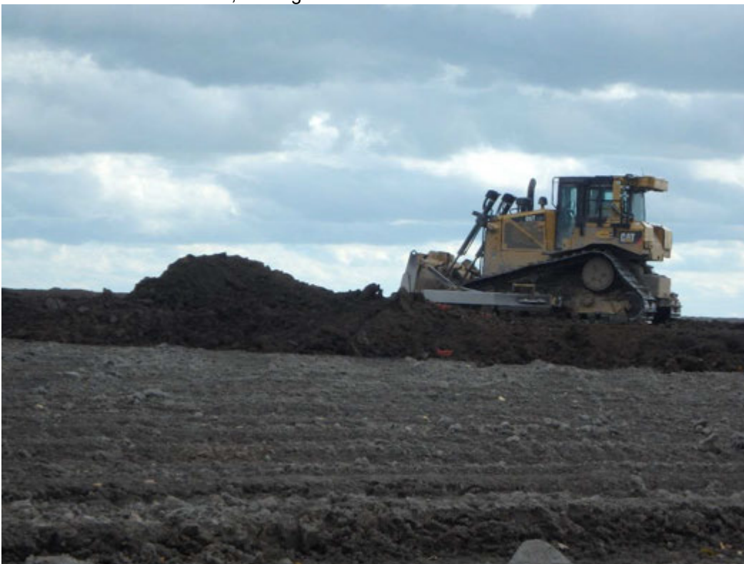
Building topsoil haul road in Pond 1, looking east
