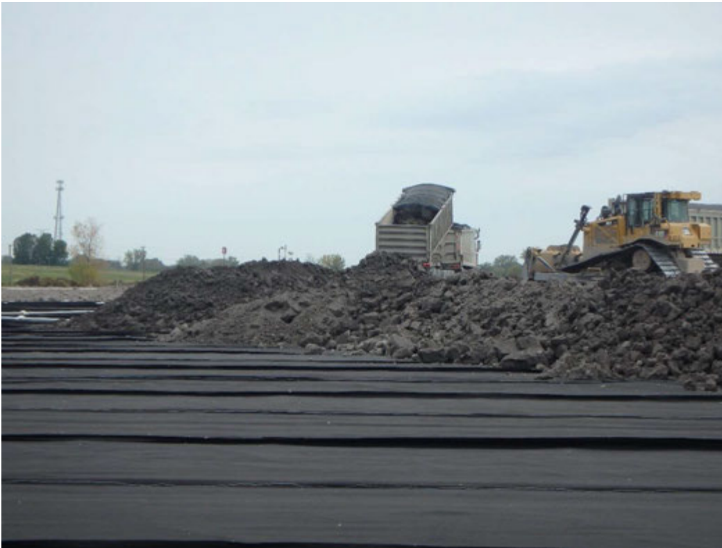
Import and placement of protective cover in Pond 2, looking north
