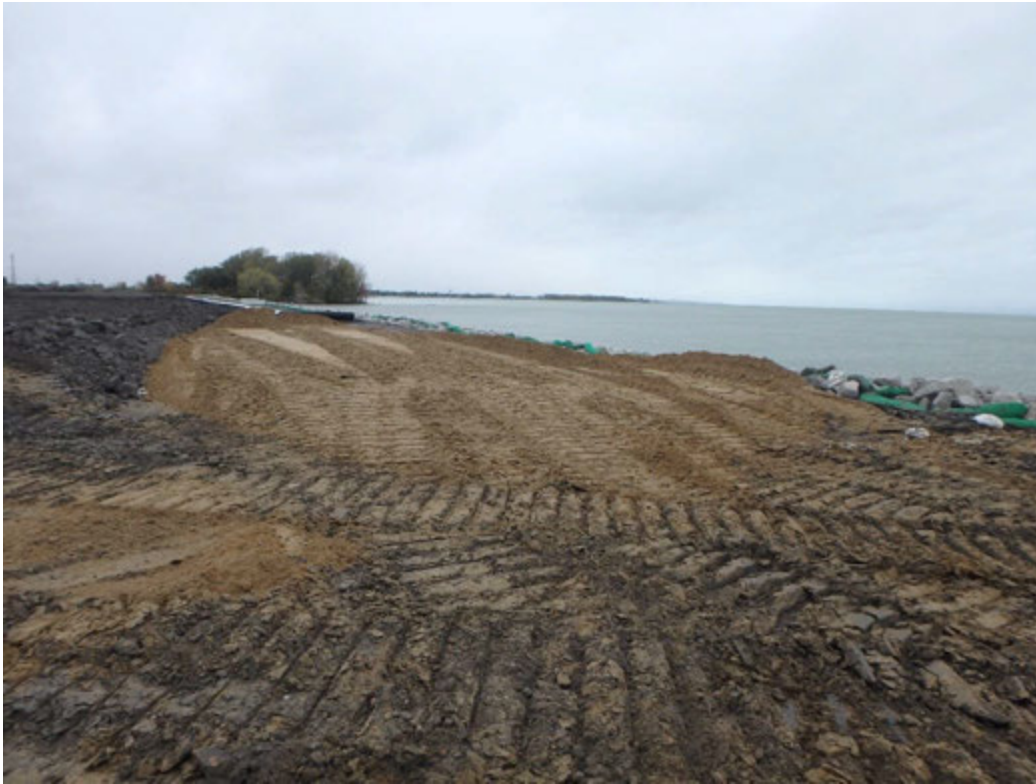
Class II sand imported for access road, looking north from southeast corner of Pond 2
