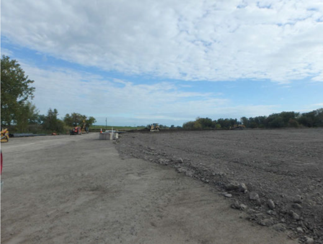
Protective cover in Pond 1, looking north.
