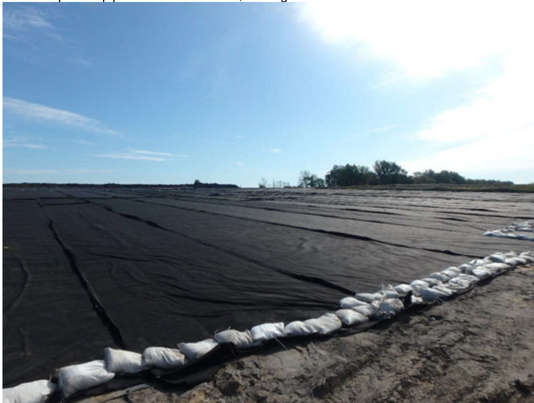
Overview of Pond 2, looking southeast
