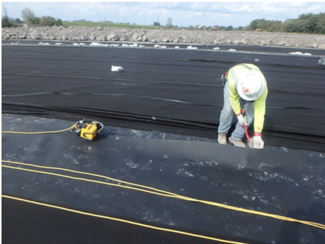
Fusion seaming of geomembrane panels.
