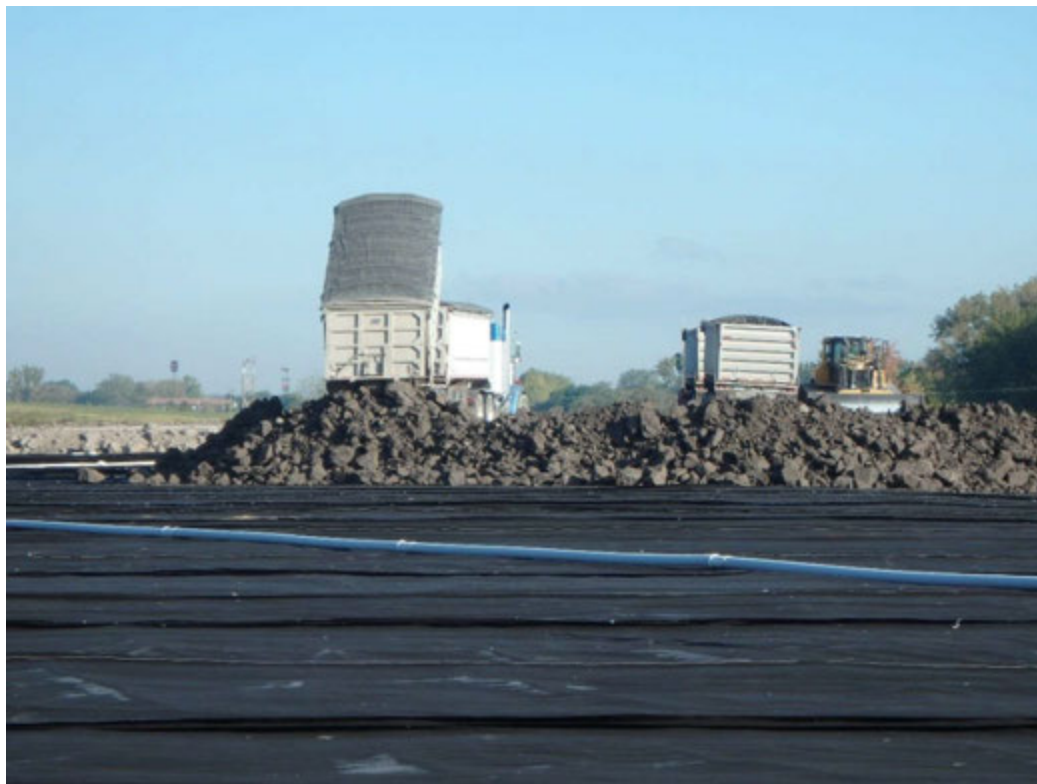
Import of protective cover to Pond 2, looking north
