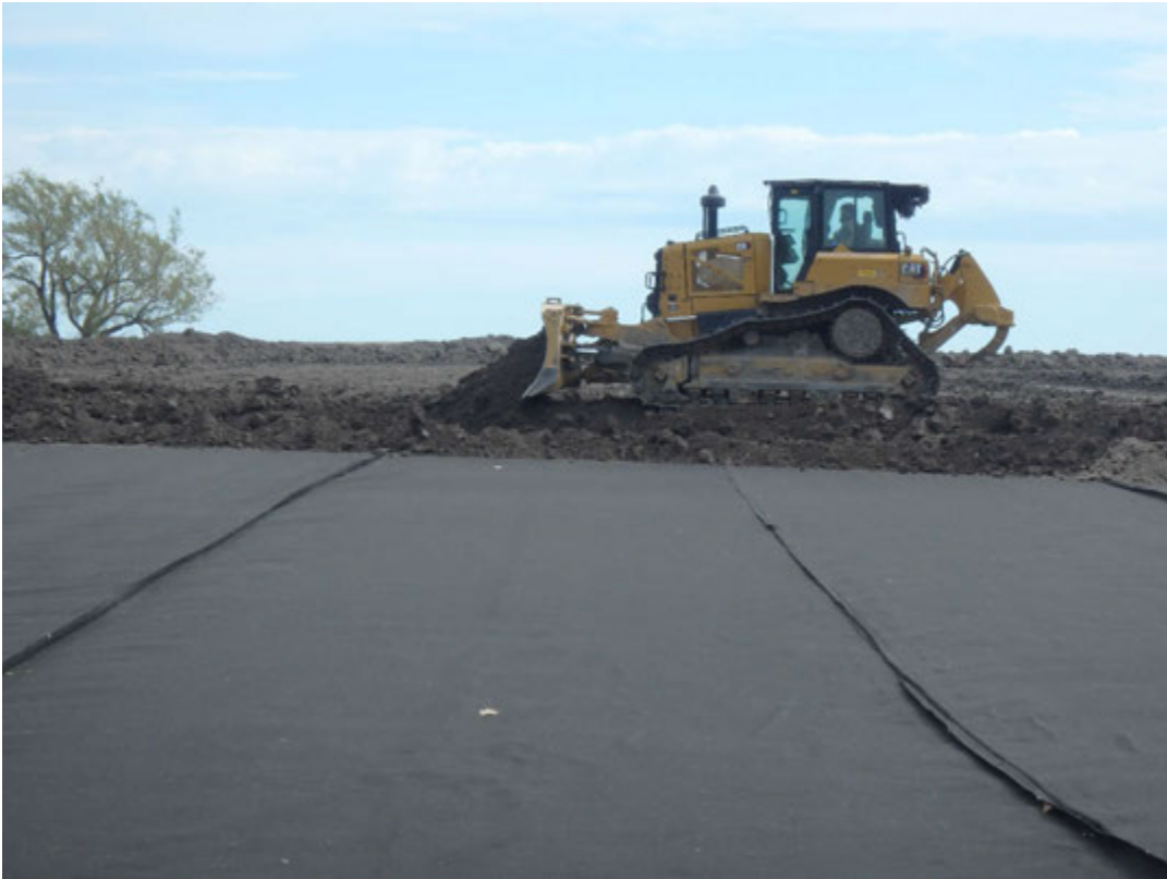
Placement of protective cover in Pond 1, looking east.
