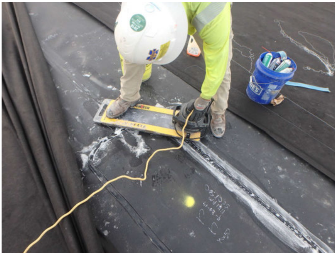
Vacuum testing of extrusion weld.
