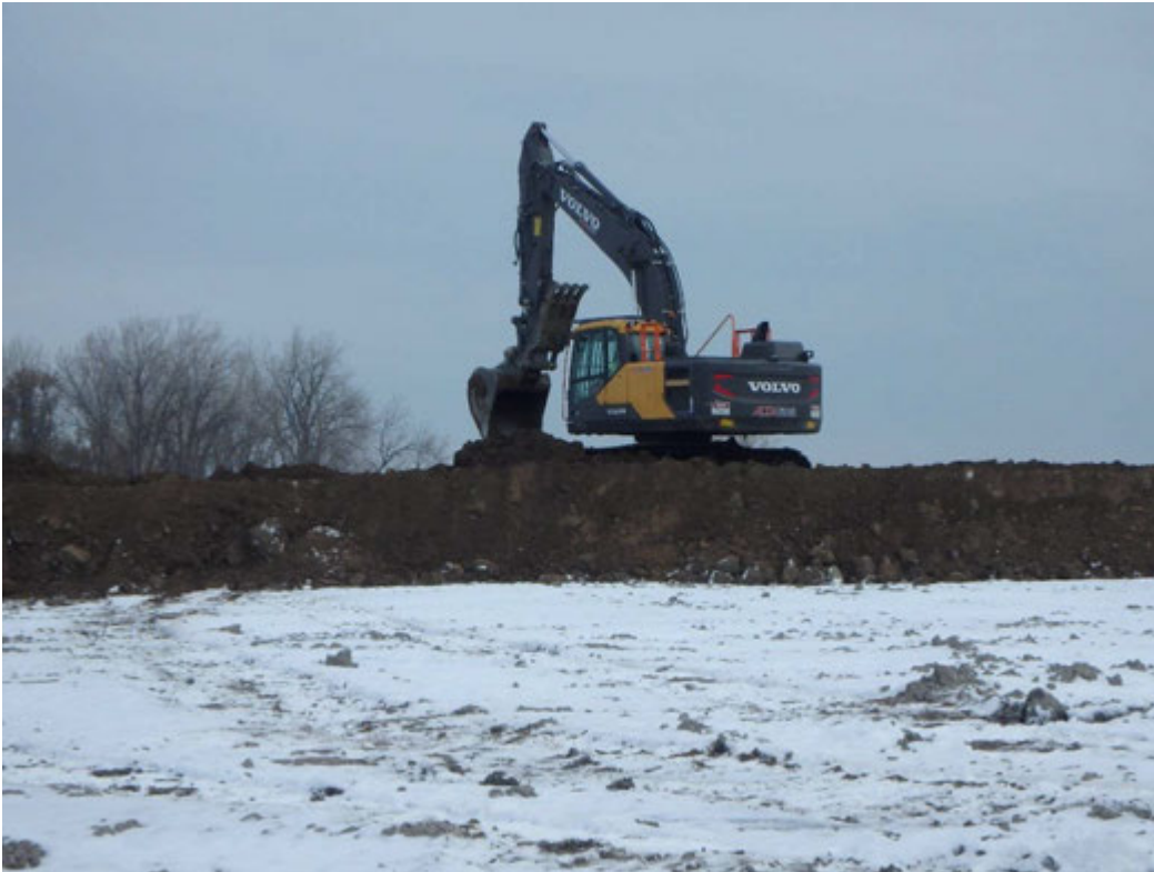
Loading topsoil from onsite stockpile for placement in Pond 2, looking northeast
