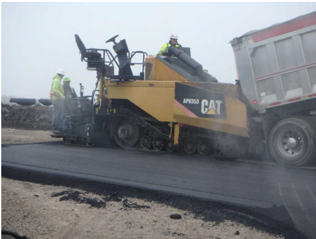
Asphalt being placed for access ramp, looking southwest
