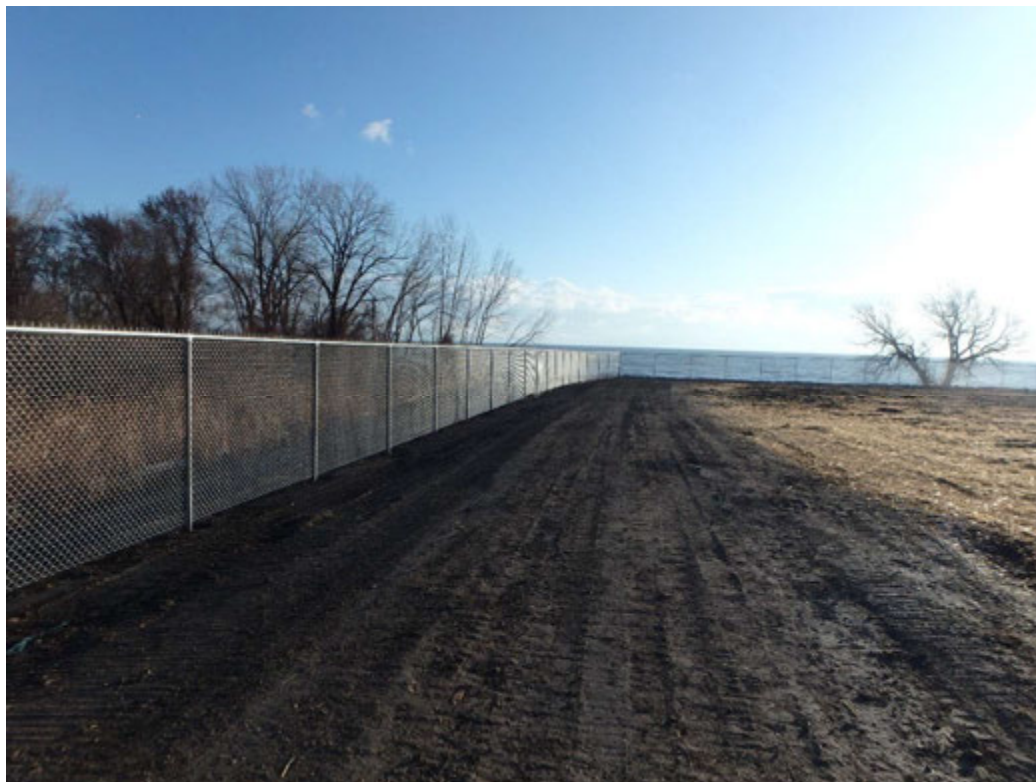
Overview of perimeter fence along north side of Pond 1
