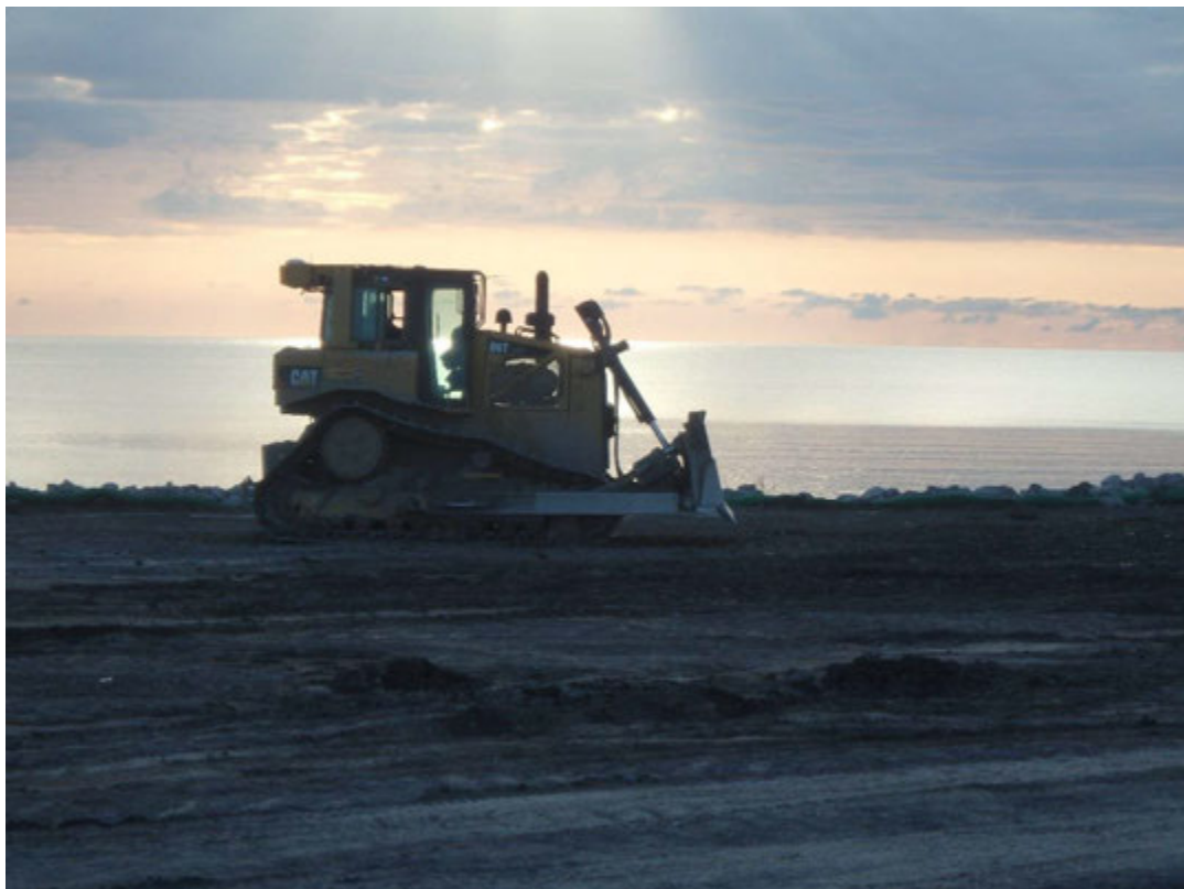
Placement of structural fill outside of Pond 2's southeast corner, looking east.
