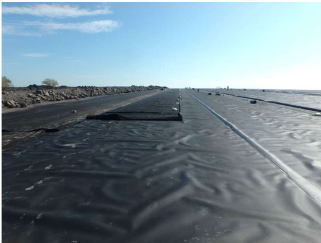
Deployment of geotextile in Pond 2, looking east.
