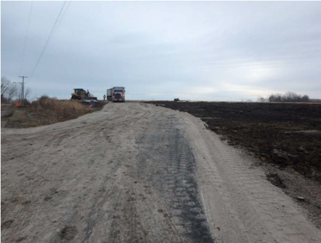
23AA placed along shoulder of asphalt access ramp, looking southeast
