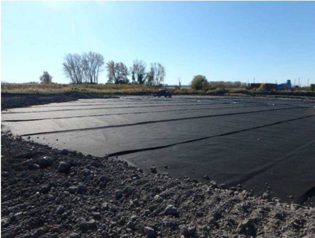
Overview of remaining area of Pond 2 to be covered with protective cover, looking southwest
