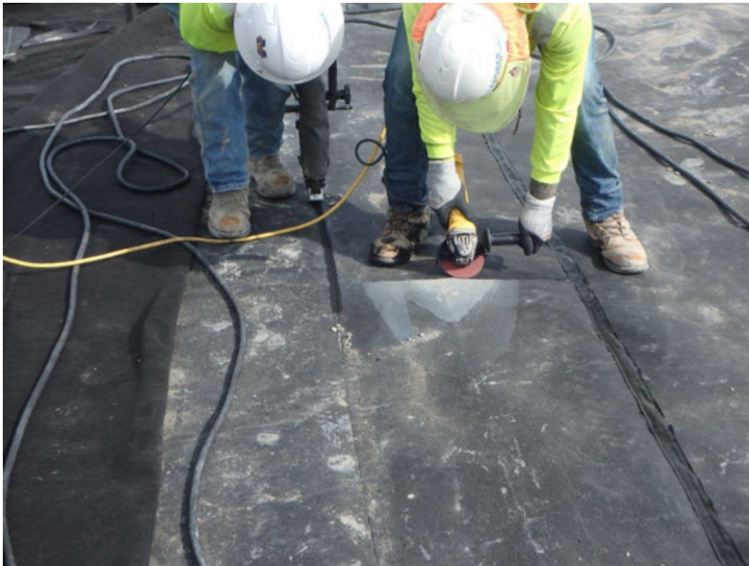
Welding cap over failed seam by extrusion method
