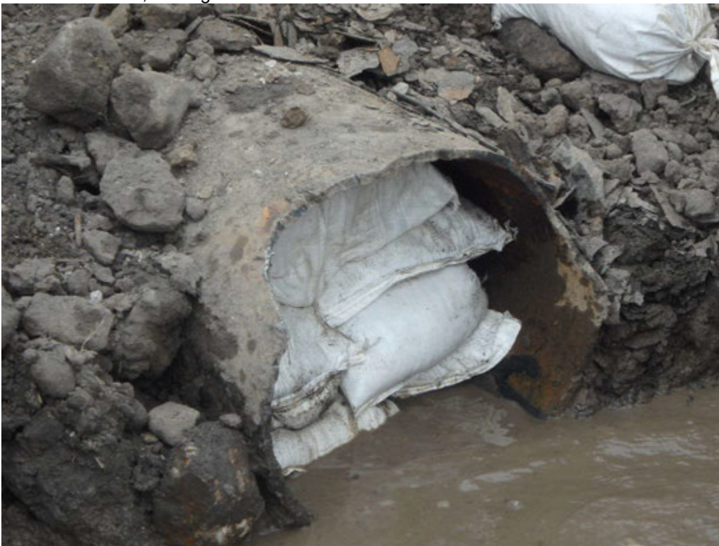
Sandbags placed in 24 inch steel pipe being capped
