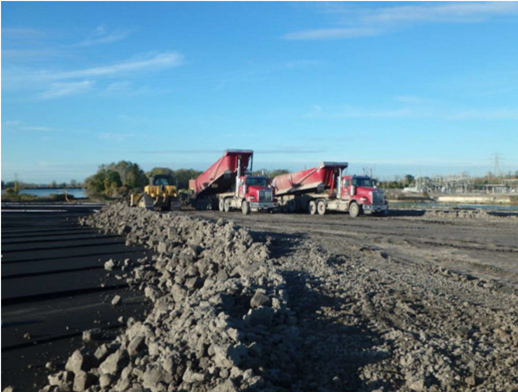
Protective cover import to Pond 2, looking southwest
