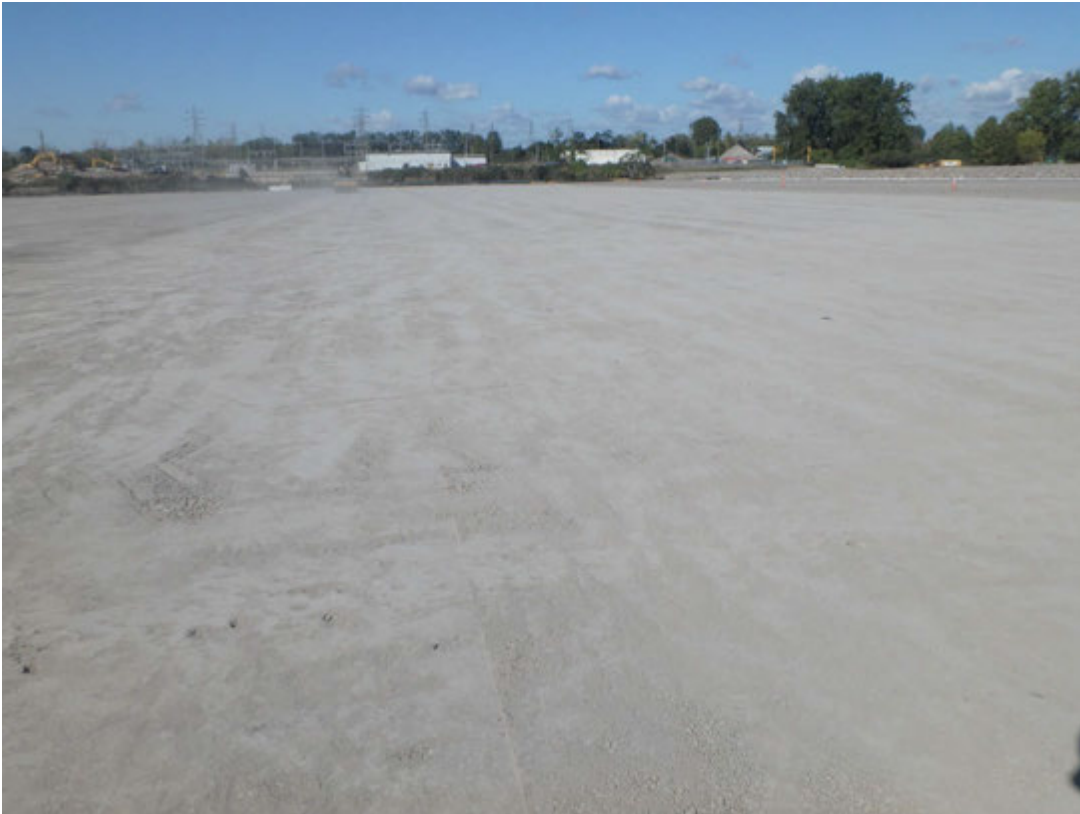
Overview of rolled liner sub-grade in Pond 2, looking west.
