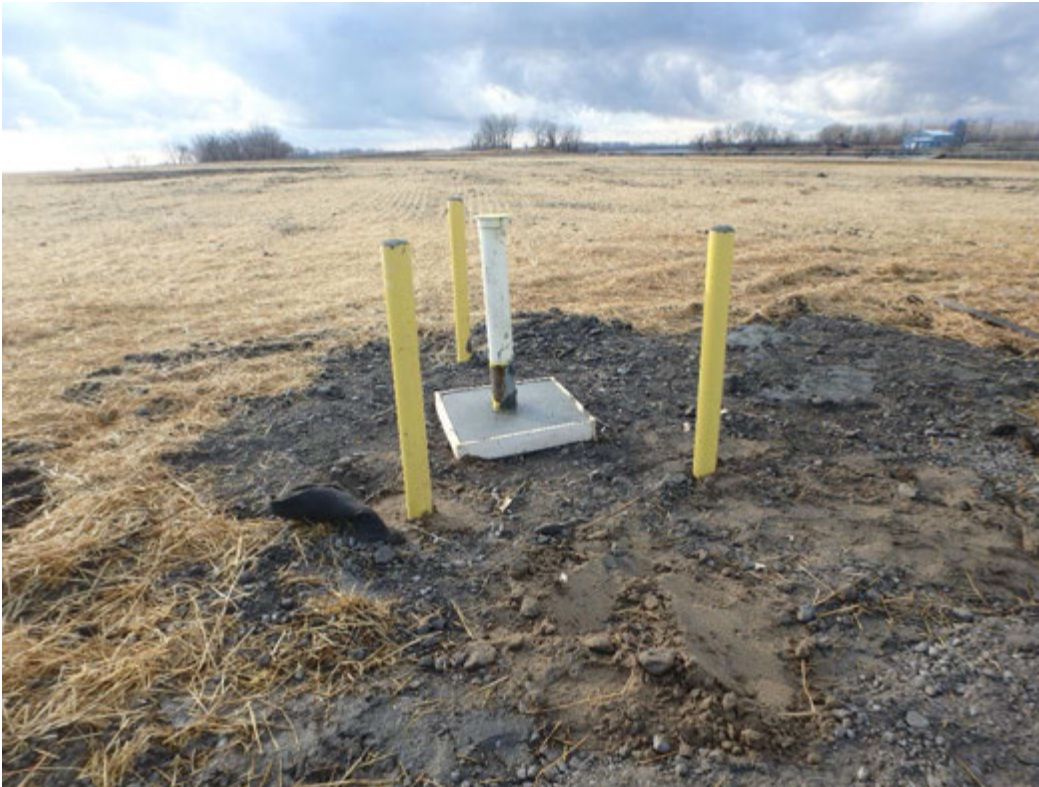
MW-15002 with protective casing and bollards installed
