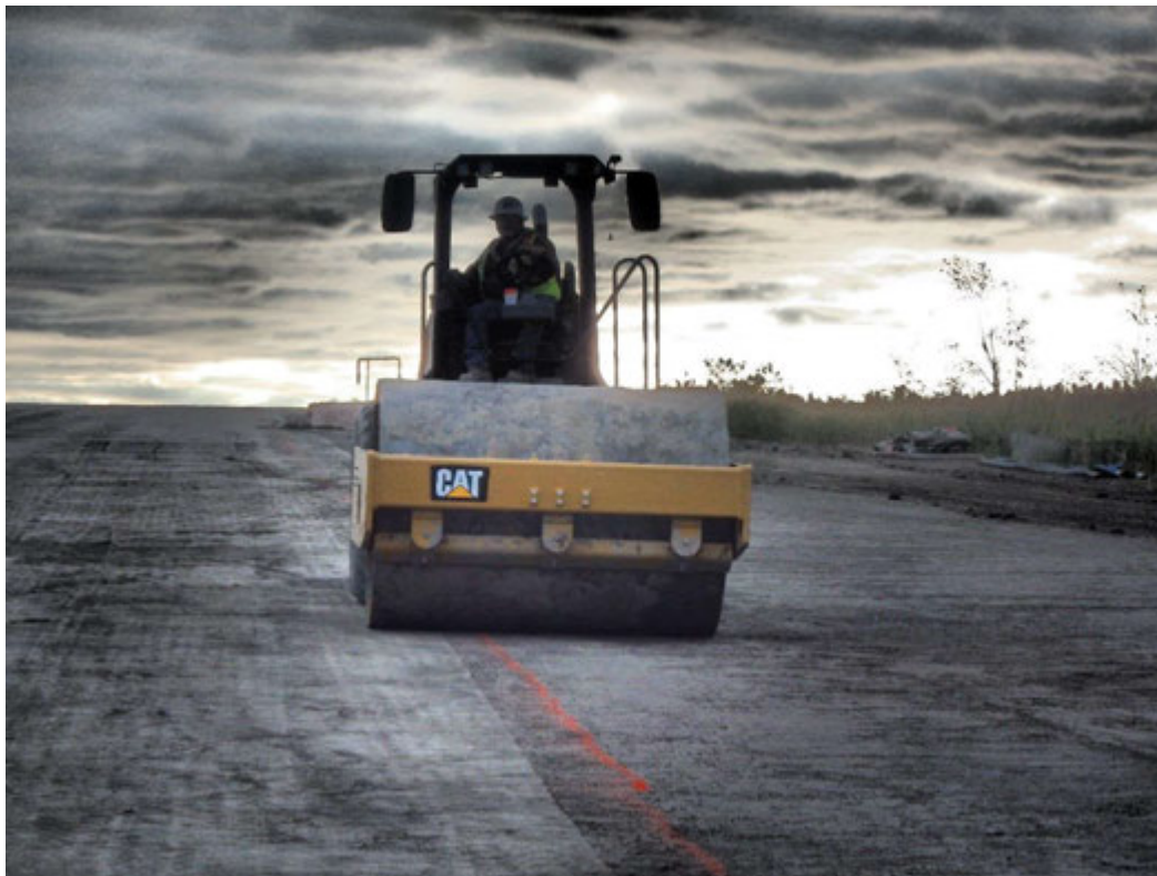
Rolling sub-grade ahead of liner deployment, looking east
