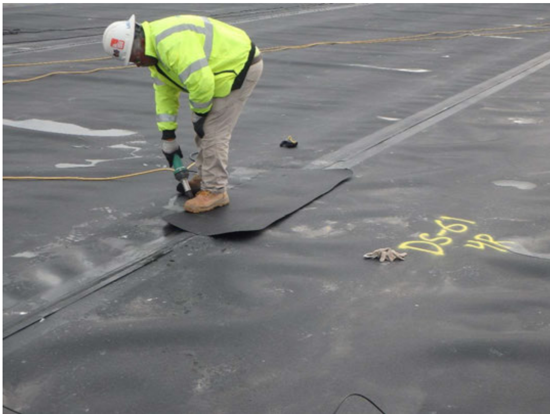
Leistering patch in preparation of extrusion welding
