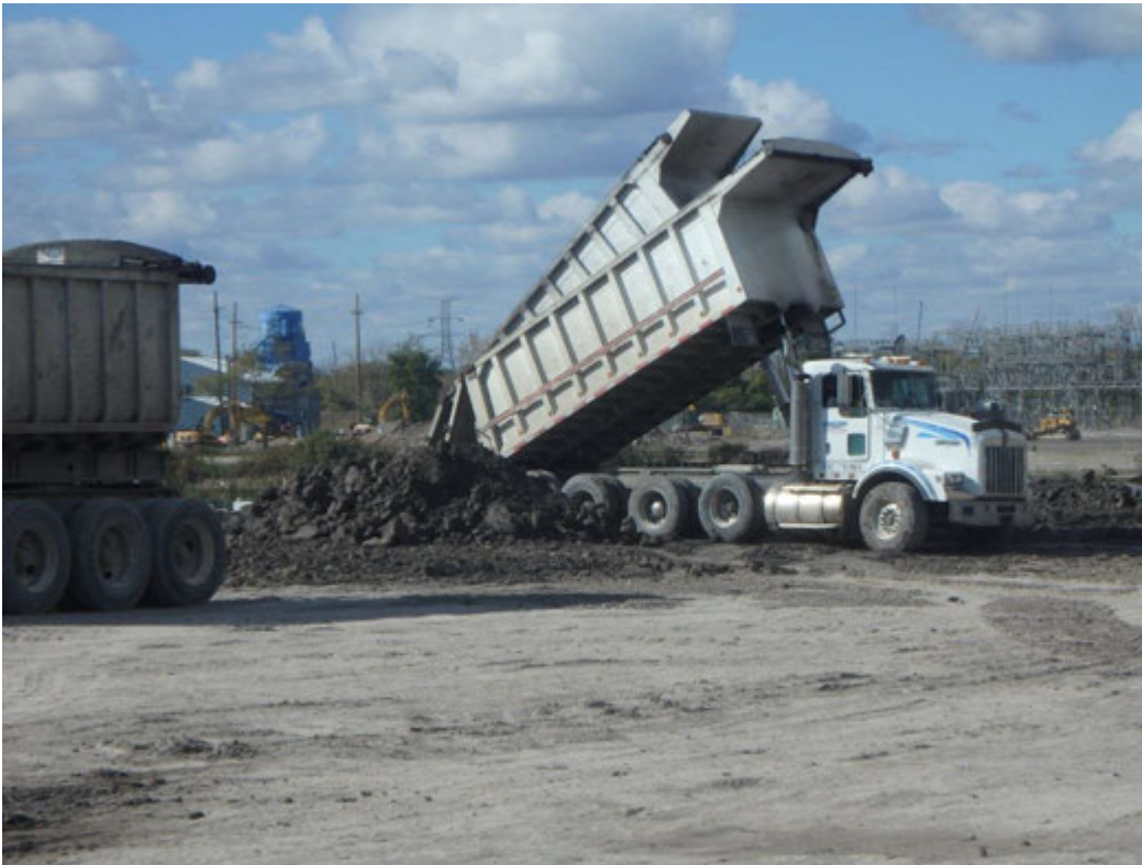
Import of protective cover to Pond 2, looking southwest
