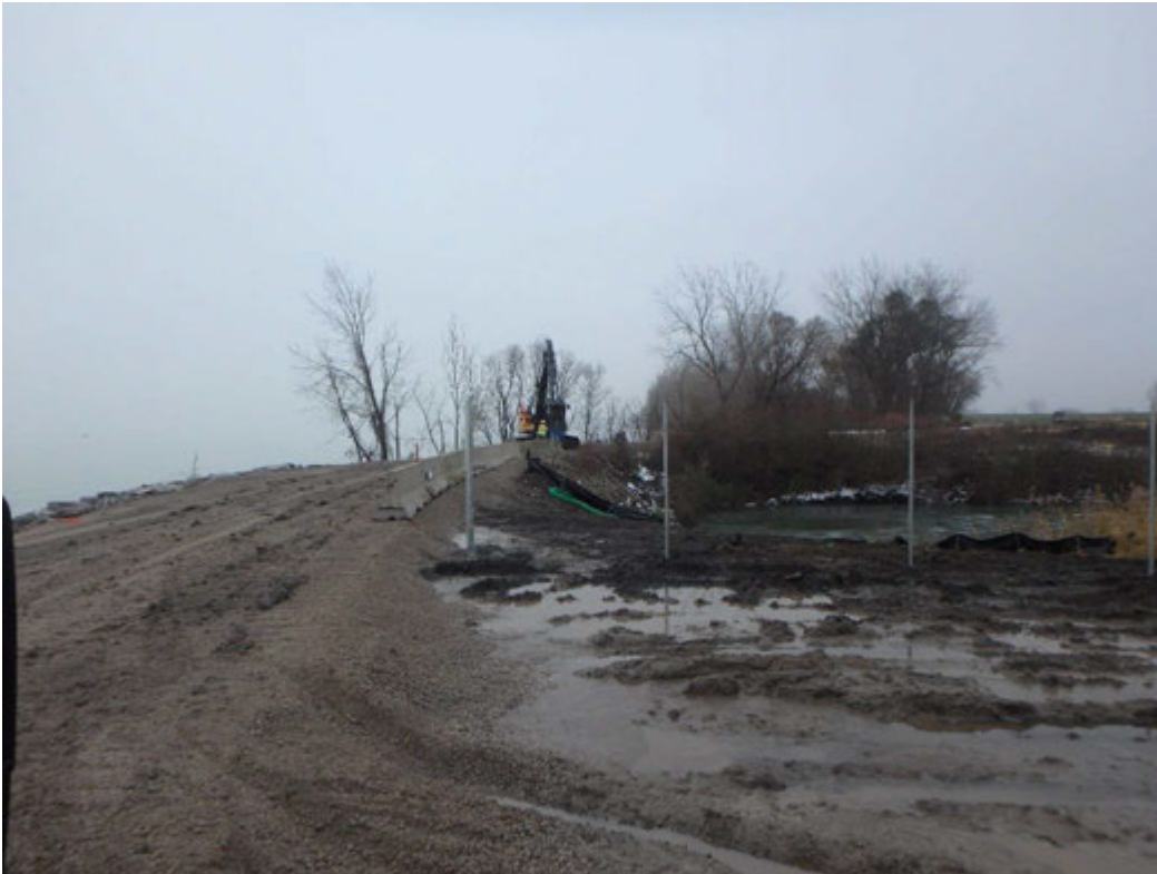
Installing Jersey barriers around horseshoe between Pond 2 and Chemical Pond, looking south
