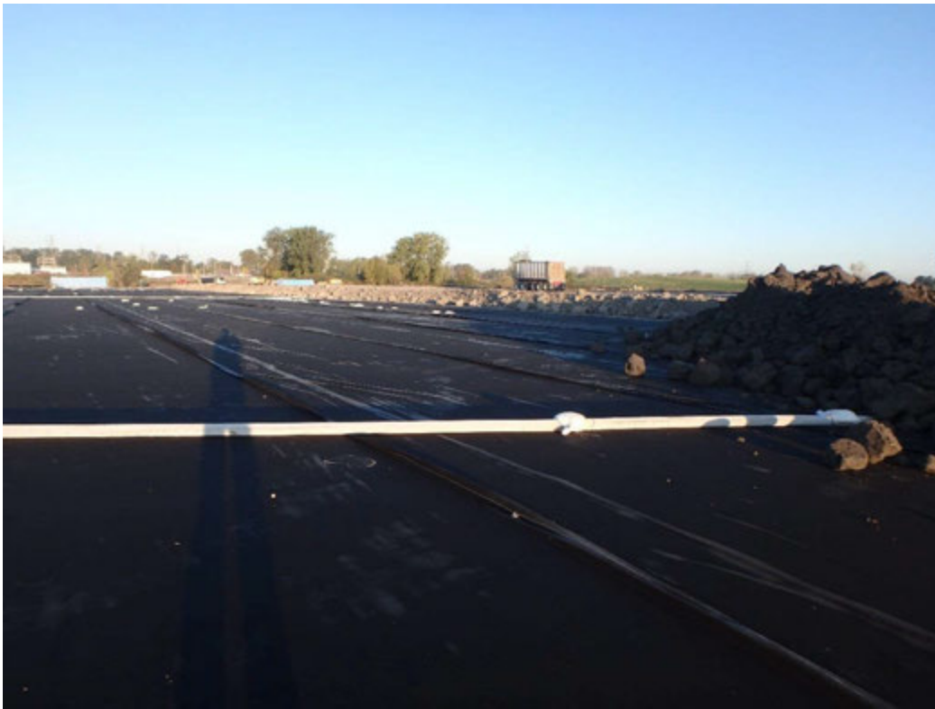
Above-Cap drain pipe installed in Pond 2
