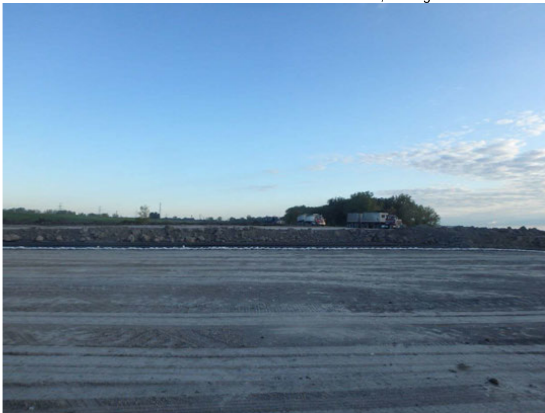
Finished liner sub-grade in Pond 2, looking north.
