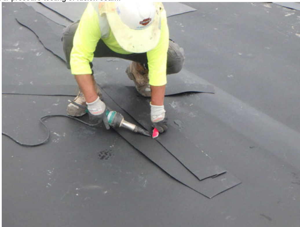
Preparing trial weld.
