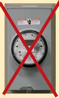
Consumers Energy recommends not pulling any meter due to the safety hazards associated with this activity. There are varying meter configurations that could result in a structure still being energized even with a meter being pulled.
